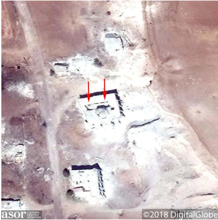
Increased damage to the mosque as indicated by red arrows. It appears that the central portion of the roof has collapsed (©2018 DigitalGlobe; September 11, 2018)
