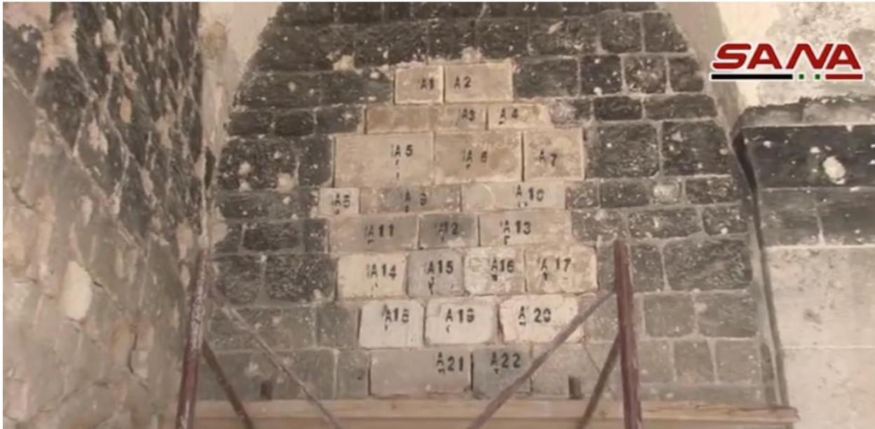
A video still of numbered stones replaced at the al-Umayyad Mosque (SANA; September 25, 2018)
