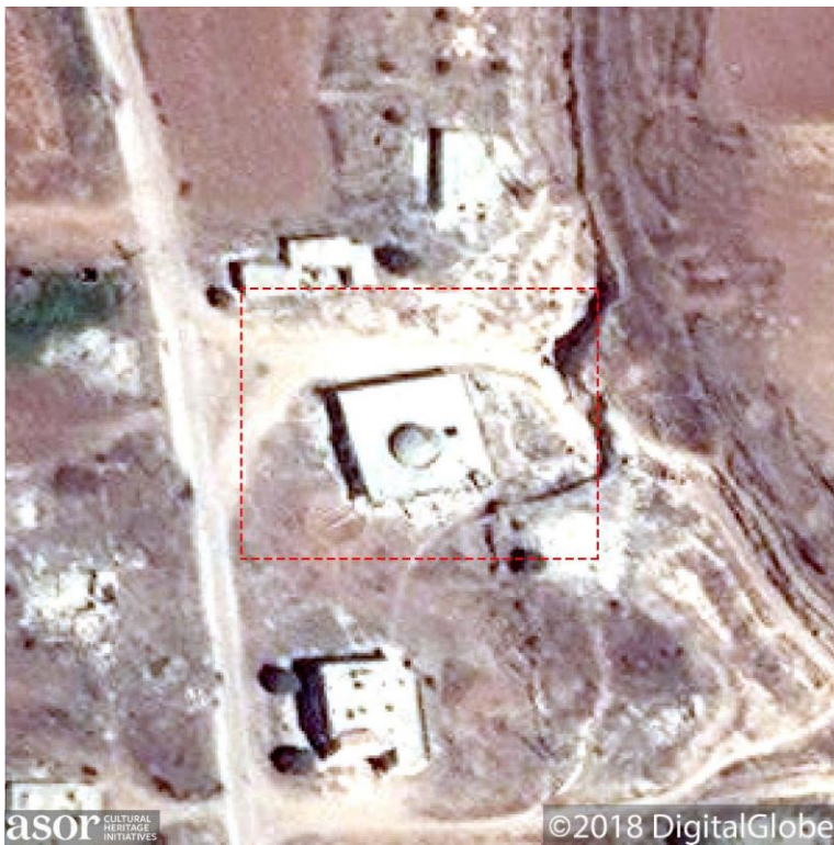
The Hasraya Village Mosque showing prior minor damage to the roof, and military trenching to the east of the mosque (©2018 DigitalGlobe; August 27, 2018)
