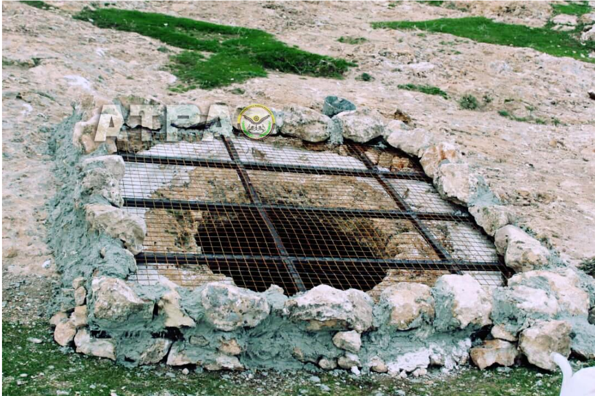
Conservation work at Qalaat Sukara with the application of plaster to stabilize metal grates that show the underground chambers (ATPA; November 26, 2018)
