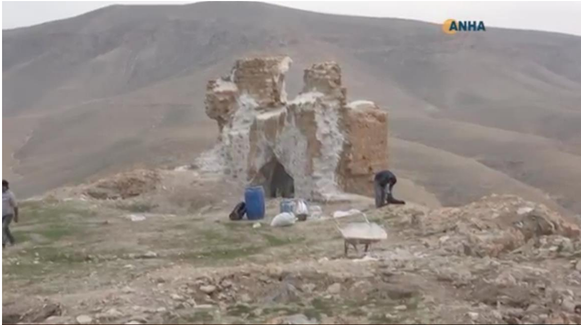
Conservation work in progress at Qalaat Sukara (Hawar News; November 22, 2018)
