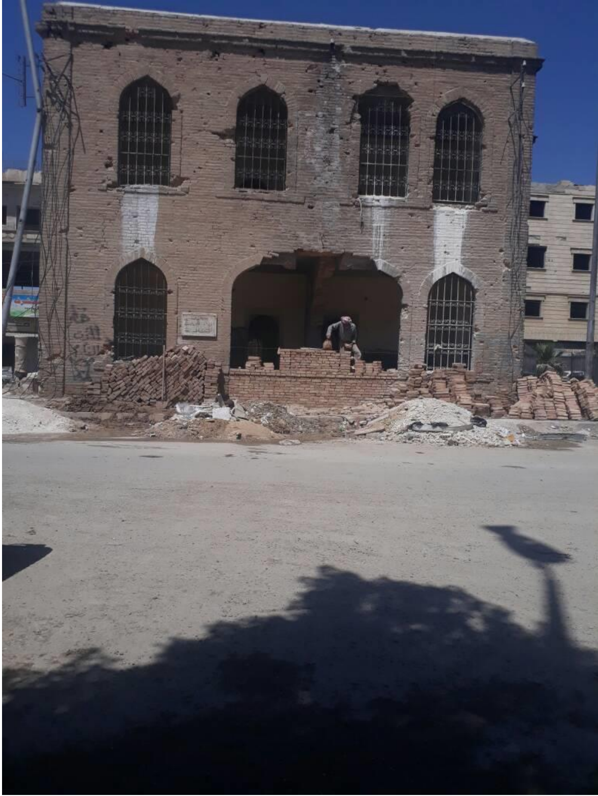
The ASOR CHI sponsored project to rebuild the east wall of the heavily damaged Raqqa Museum. This construction was one part of a much larger stabilization effort focused on the building's interior, exterior, and gardens (ASOR CHI).
