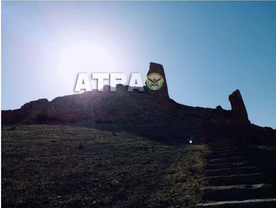
Qalaat Sukara before cleaning and restoration (ATPA; October 31, 2018)
