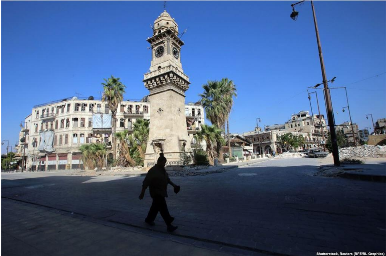
The Bab al-Faraj Clock Tower showing the missing clock faces and piles of rubble in the background (Radio Free Europe Radio Liberty; November 4, 2016)
