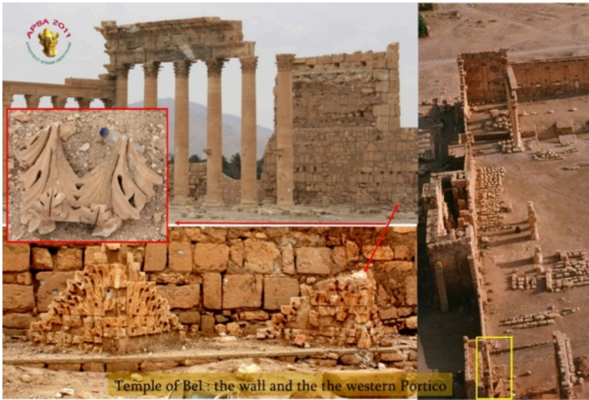
Figure 25: Damage to the capital of a column previously restored (Source: APSA)
