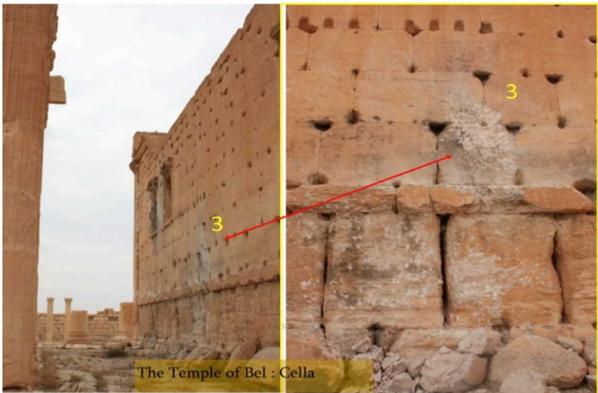
Figure 44: Sanctuary of the temple, shell traces on the outer facade of the eastern wall (Source: APSA)
