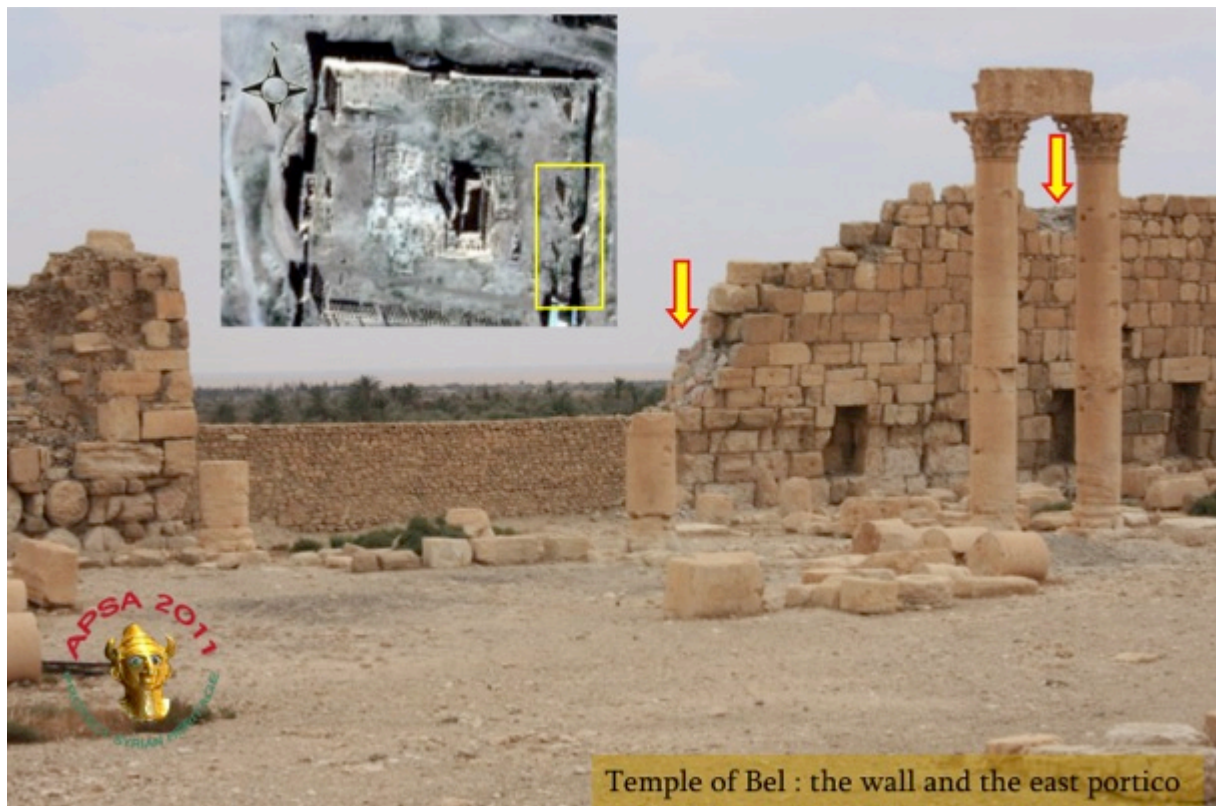
Figure 37: Traces of shrapnel in the eastern wall (Source: APSA)
