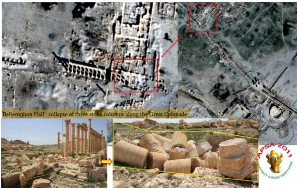
Figure 50: The colonnaded street; damage to three columns and the shifting of a drum of the fourth column (Sources: APSA and HRW)
