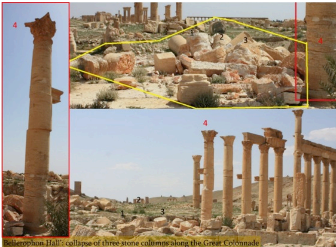
Figure 52: The colonnaded street; damage to three columns and the shifting of a drum of the fourth column (Source: APSA)
