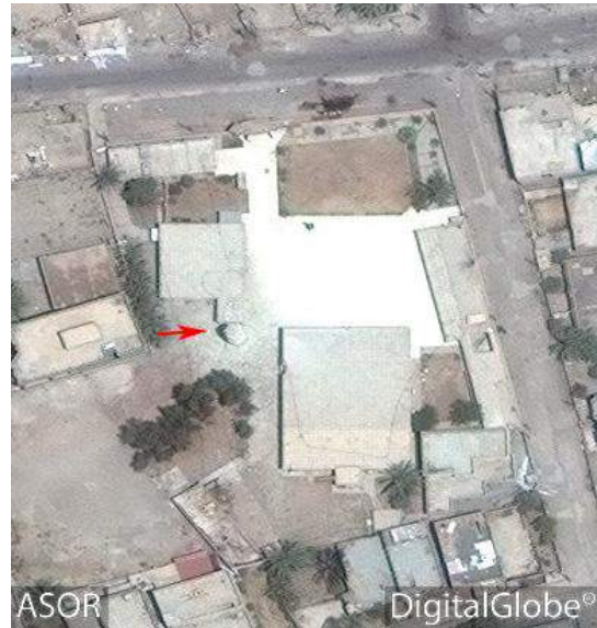
Visible damage to the minaret and corners of two buildings closest to the minaret (DigitalGlobe; June 28, 2016)
