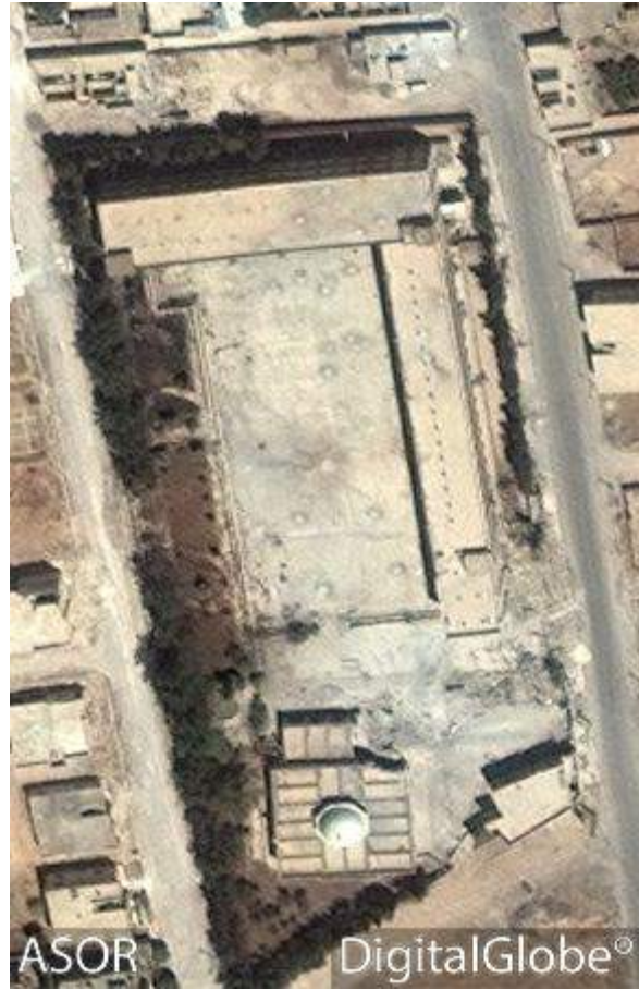
al-Miqdad Mosque complex with visible damage due to airstrikes. The minaret has been destroyed on the northeast corner of the mosque (DigitalGlobe; June 26, 2016)
