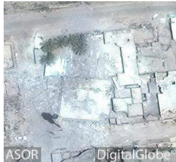
Extensive damage to al-Mudallal Mosque and complex which occurred between June 13 and 28th. (DigitalGlobe; June 28, 2016)
