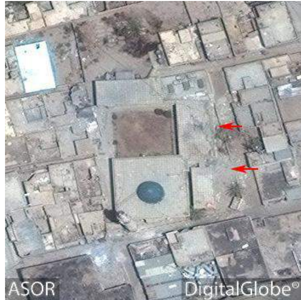
al-Fayad Mosque with damage to the eastern portion of the buildings (DigitalGlobe; June 28, 2016)
