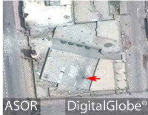
al-Furqan Mosque with new damage to the roof (DigitalGlobe; June 28, 2016)
