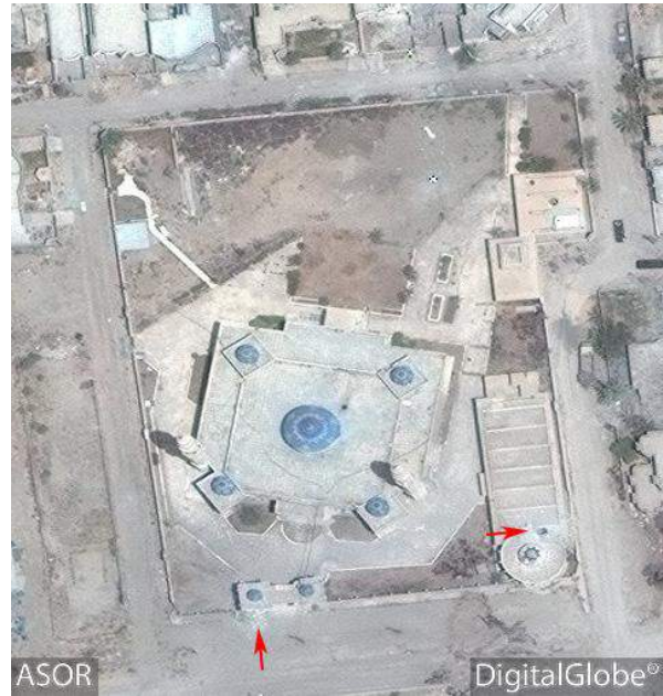
Mosque of the Caliphs with damage to the entrance gate and roof (DigitalGlobe; June 28, 2016)
