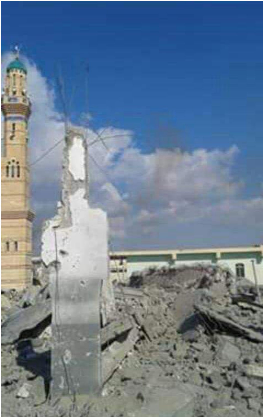
Severe damage to Hassan bin Ali Mosque (Twitter; January 28, 2016)
