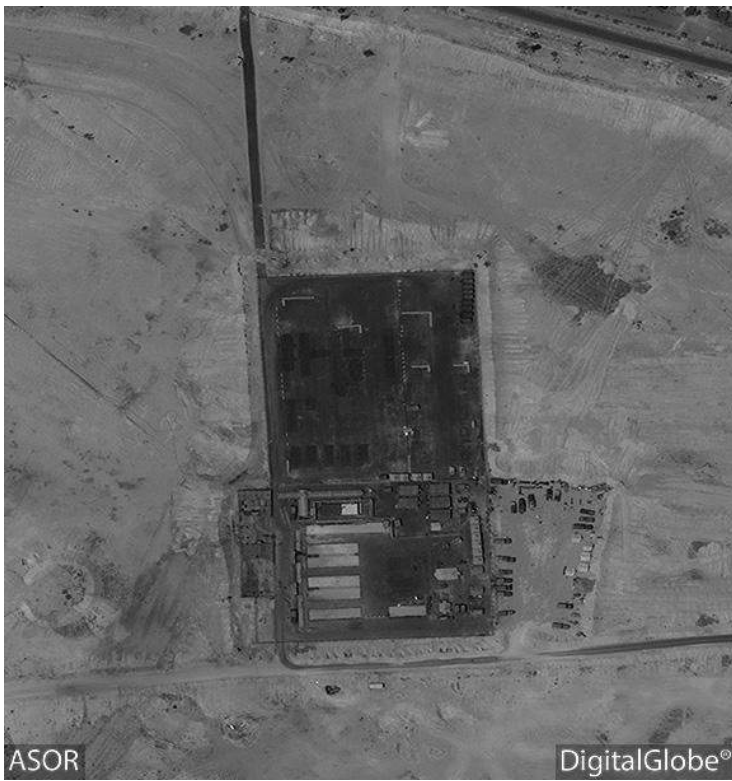
The military base after the removal of buildings from the northern portion (DigitalGlobe; June 23, 2016)
