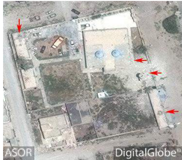
al-Taqwa Mosque with severe damage to the minaret, the mosque, and exterior buildings (DigitalGlobe; June 28, 2016)
