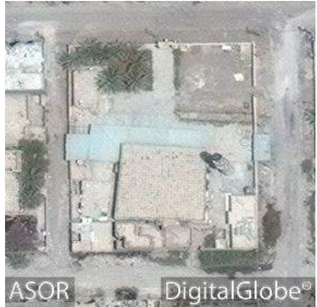
Minor damage to the mosque from the exterior (DigitalGlobe; June 28, 2016)
