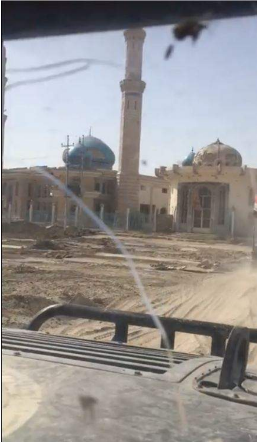
Damage to facade and domes of Mosque of the Caliphs as seen from the inside of a passing vehicle (AP; June 22, 2016)
