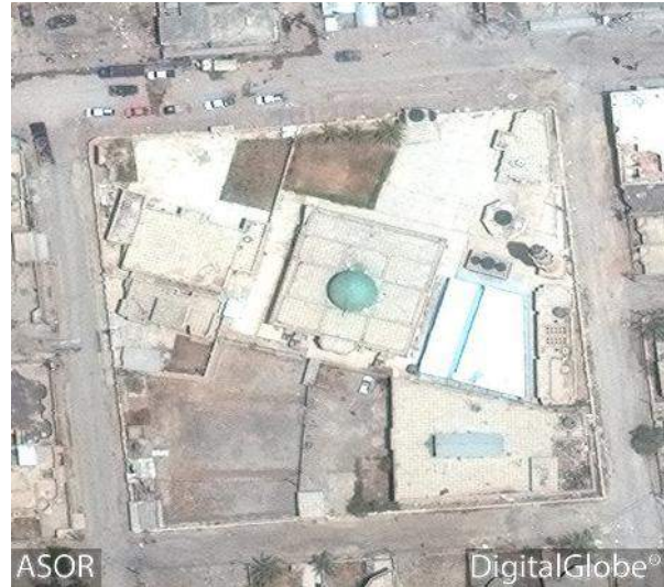
No visible exterior damage to the mosque (DigitalGlobe; June 28, 2016)
