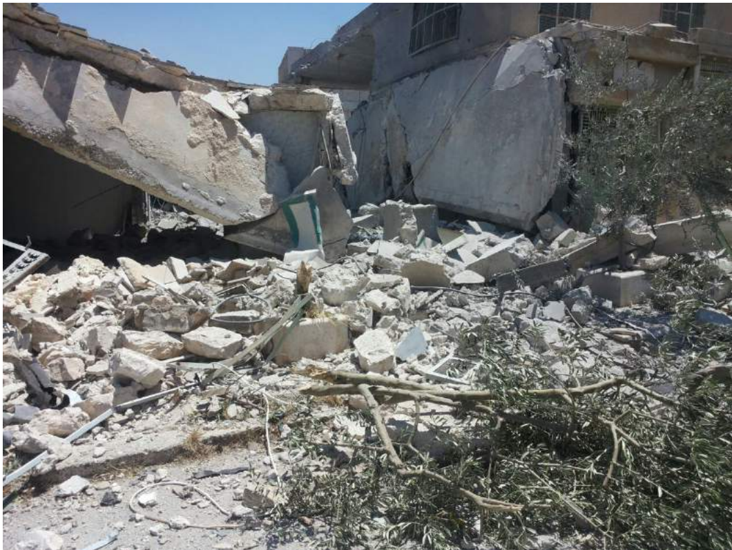
Exterior view of damage to Ammar bin Yasser Mosque (Mahmud al-Jurh Abu Malik/Twitter; July 1, 2016)
