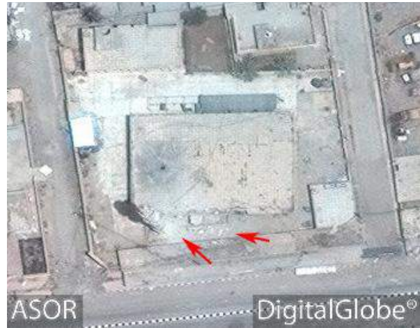
New damage to the mosque with visible debris from the front facade and the minaret (DigitalGlobe; June 28, 2016)
