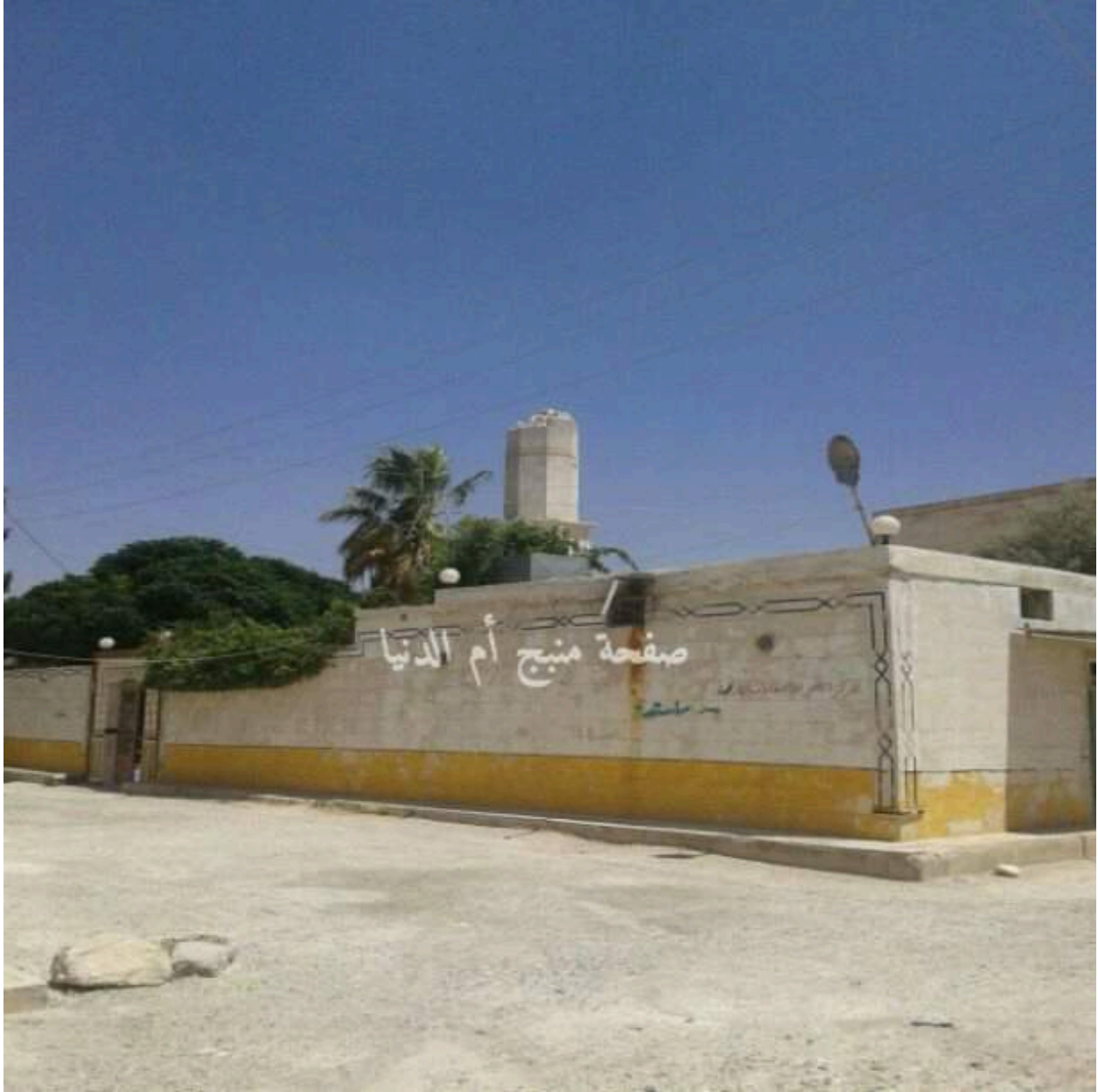
Damage to the minaret of al-Miqdad Mosque (Manbij Om al-Duonia; June 30, 2016)
