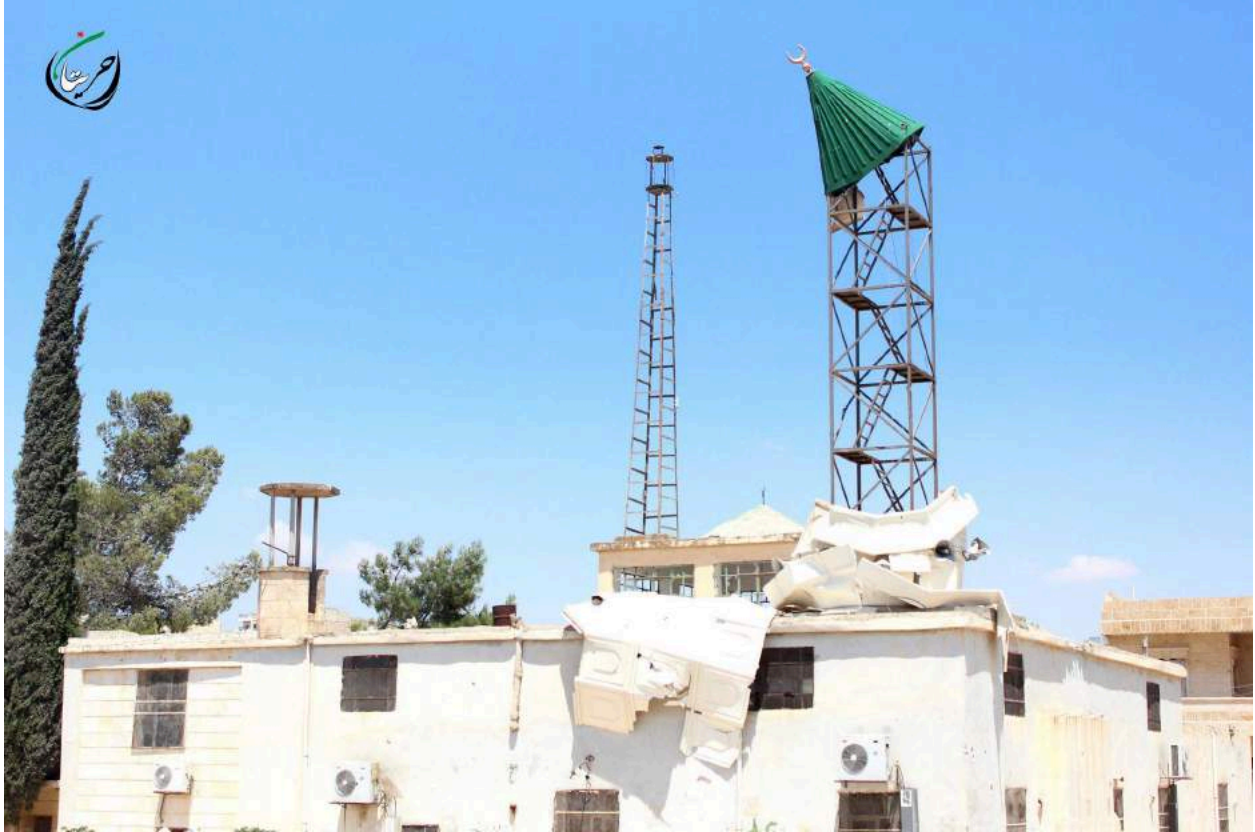
Damage to Ali Sayyad Mosque (Syrian Revolution Network; June 30, 2016)
