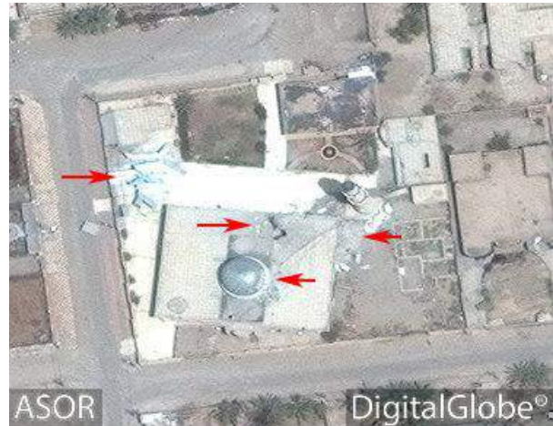
Damage to the metal roof of an exterior building, the roof and the dome of the mosque (DigitalGlobe; June 28, 2016)
