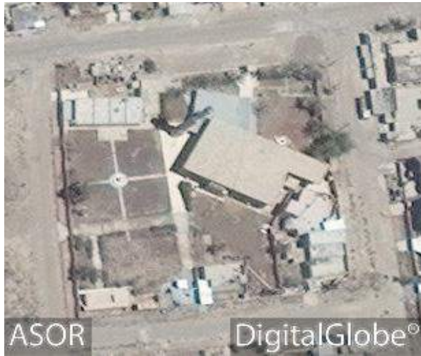
Hassan bin Ali Mosque with no visible damage (DigitalGlobe; June 13, 2016)
