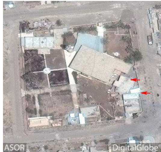
Visible damage to Hassan bin Ali Mosque (DigitalGlobe; June 28, 2016)
