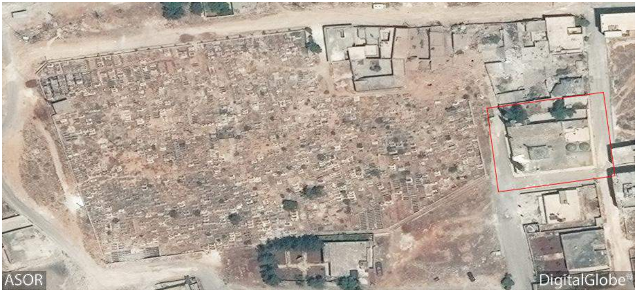
Ali Sayyad Mosque (outlined in red) with the minaret and corner of the mosque badly damaged (DigitalGlobe; June 30, 2016).
