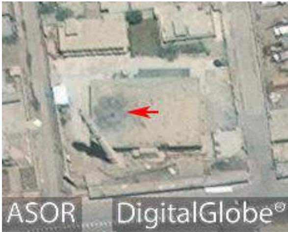
Damage to the roof of Abu Obeida Mosque between May 20 and 31st in 2016 (DigitalGlobe; May 31, 2016)
