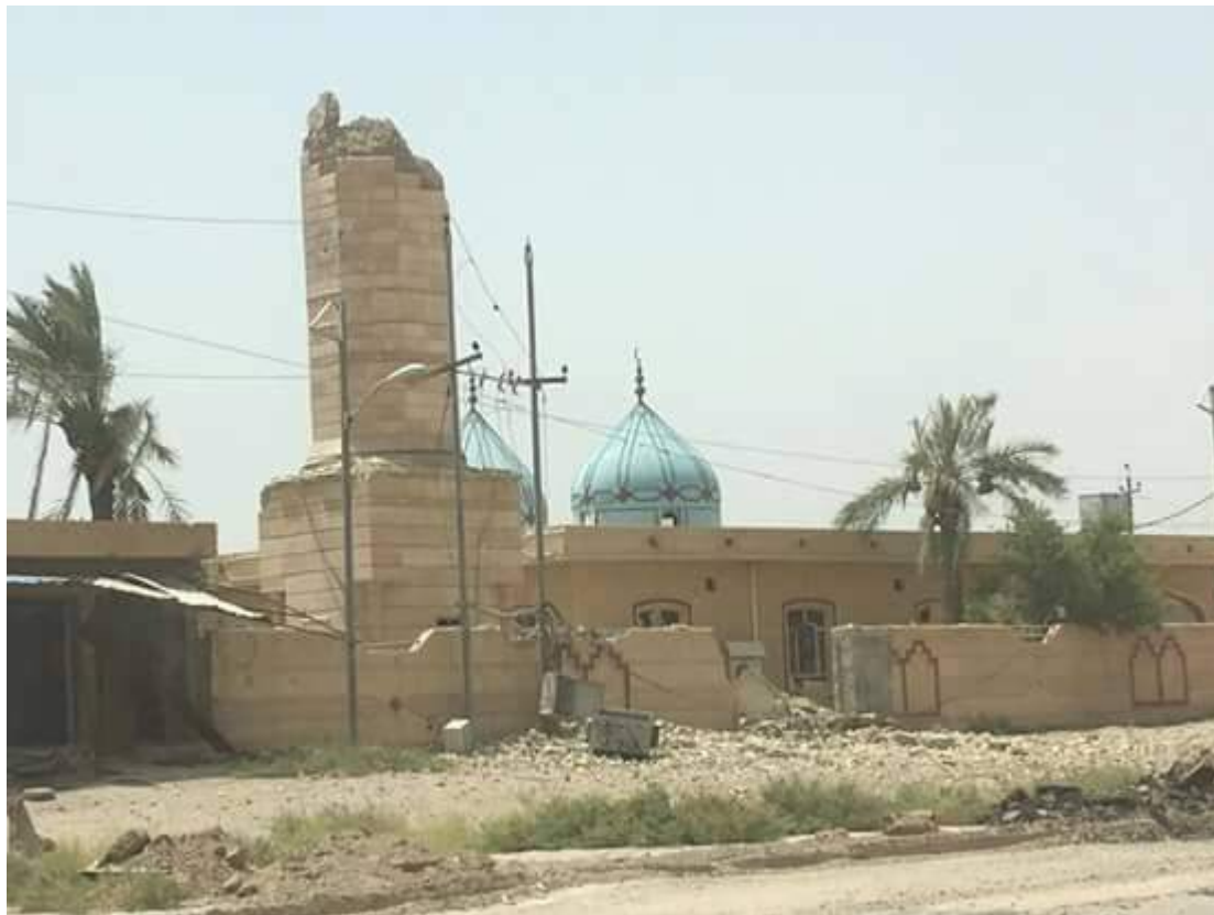
Damage to the fence and minaret of al-Taqwa Mosque (Twitter; June 22, 2016)
