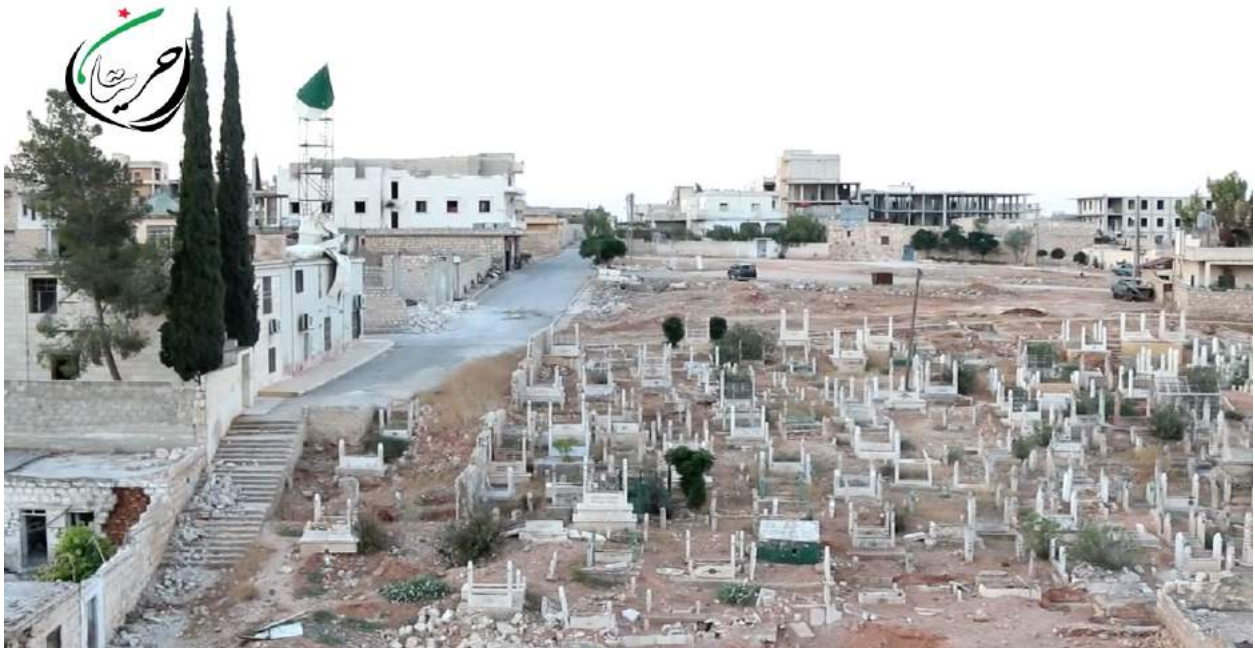
A video still showing an overview of damage to Ali Sayyad Mosque and Martyrs Cemetery (Hraytan City; July 5, 2016)
