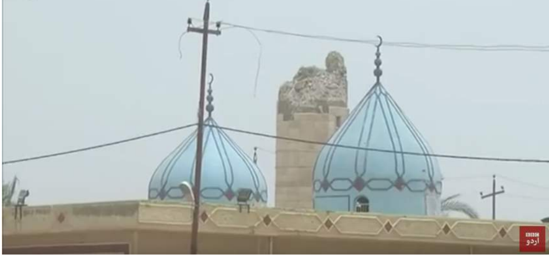
Severe damage to the minaret of al-Taqwa Mosque (BBC Urdu; June 21, 2016)
