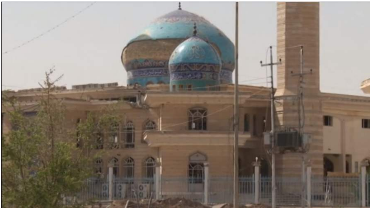
Video still of damage to the Mosque of the Caliphs (AP; June 22, 2016)
