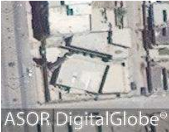
al-Furqan Mosque with minor damage to the roof (DigitalGlobe; June 13, 2016)
