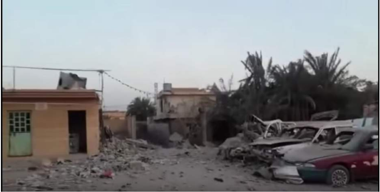
Video still of damage on street outside of entrance to Ali bin Abu Talib Mosque complex (Iraqi Spring Media Center; July 21, 2015)
