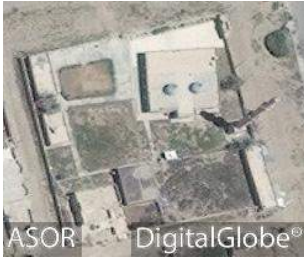
al-Taqwa Mosque with little visible damage (DigitalGlobe; June 13, 2016)
