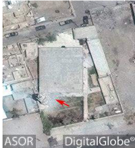
al-Sheikh Hamza Abbas Mosque with visible damage to the minaret and the wall closest to it (DigitalGlobe; June 28, 2016)
