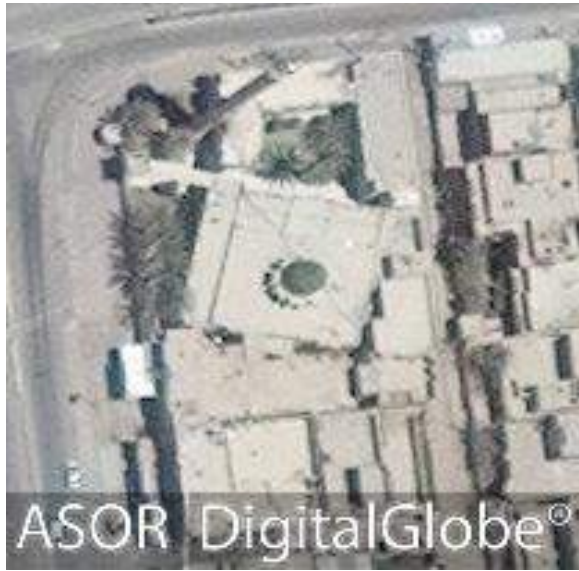
al-Hadra Mosque with no visible damage (DigitalGlobe; June 13, 2016)
