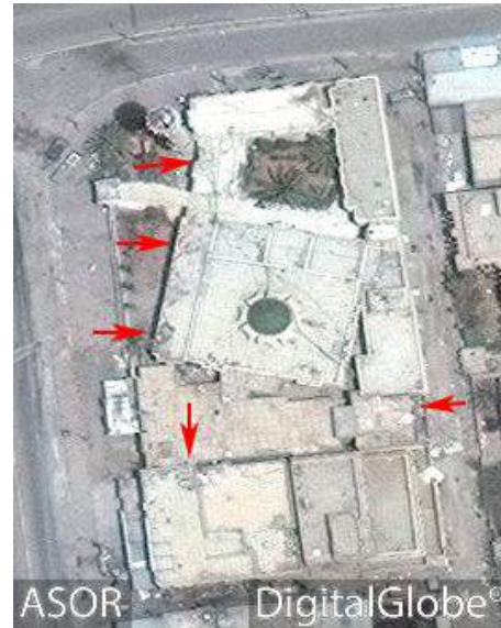
al-Hadra Mosque with damage to the eastern side of the mosque and multiple auxiliary buildings (DigitalGlobe; June 28, 2016)
