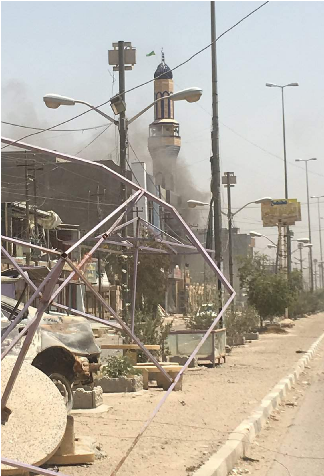
A fire burns in al-Furqan Mosque (WG Dunlap; June 28, 2016)
