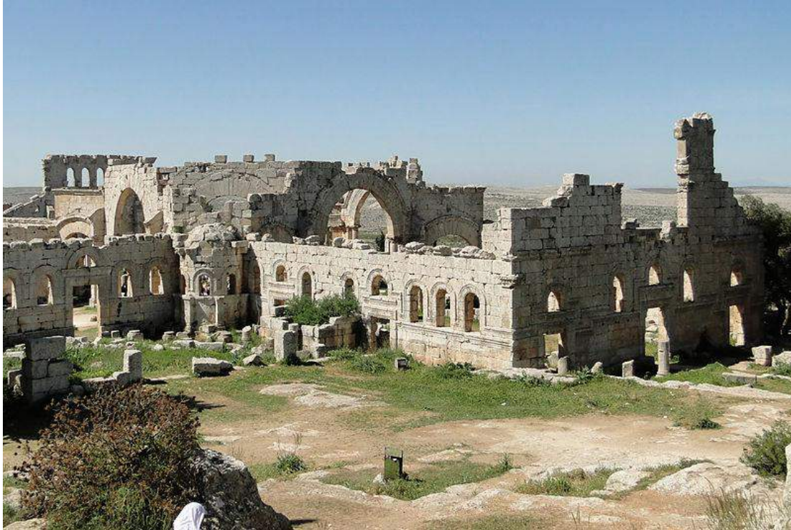
General view of church prior to airstrike
