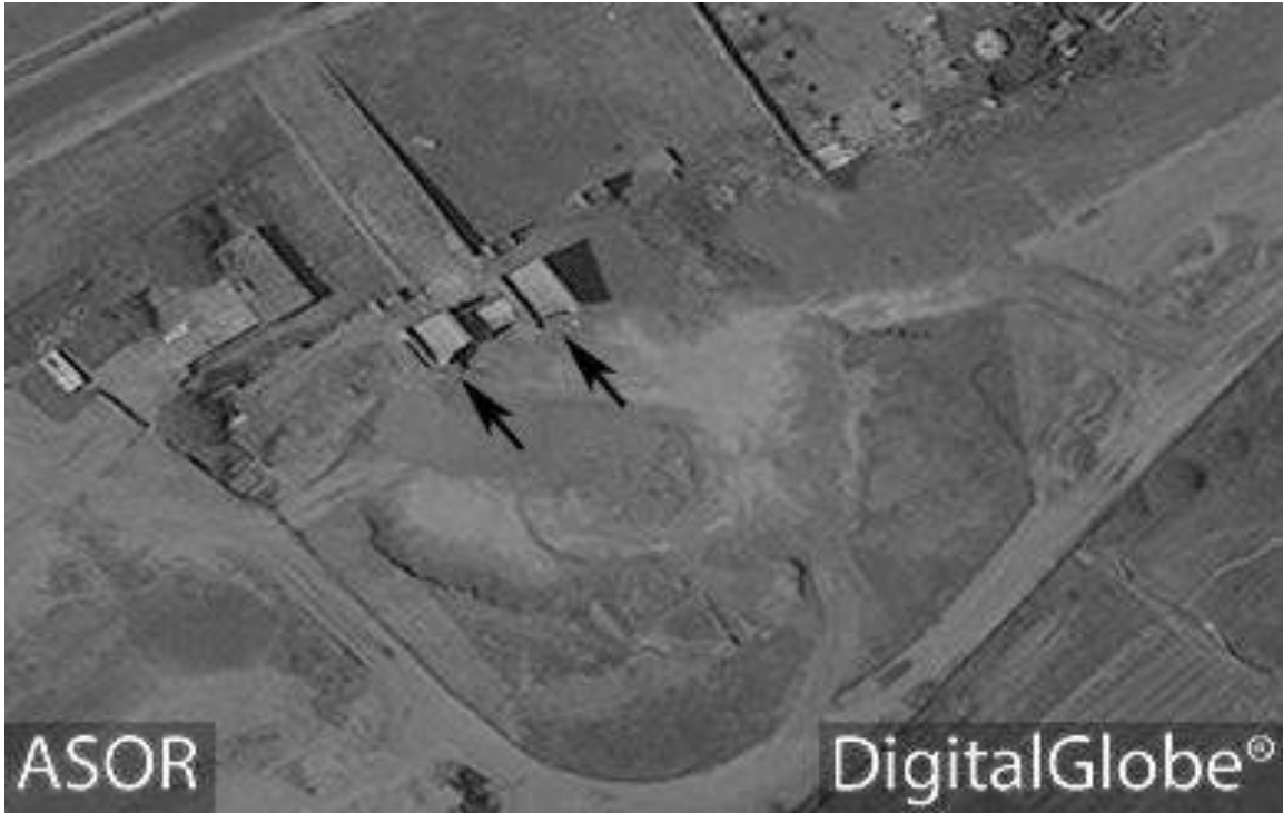
Nergal Gate with damage on the southern side indicated by the black arrows. (DigitalGlobe; May 25, 2016)
