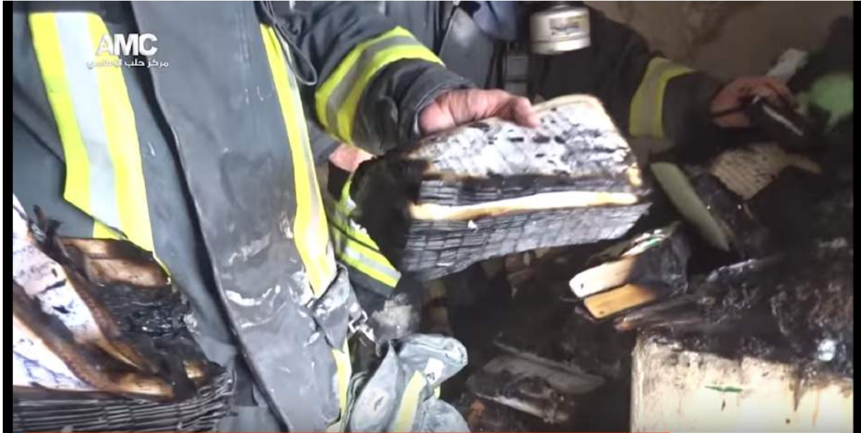
Fire damage in Sabareen Mosque (Aleppo Media Center; June 16, 2016)
