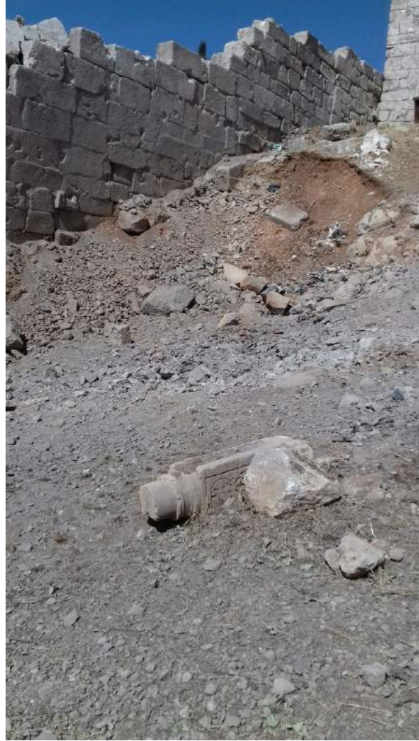
Northeast outer wall
