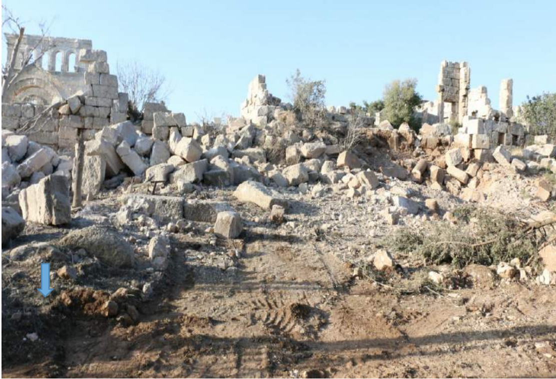
Extensive damage including collapsed and fragmented stone masonry, photo facing northeast
