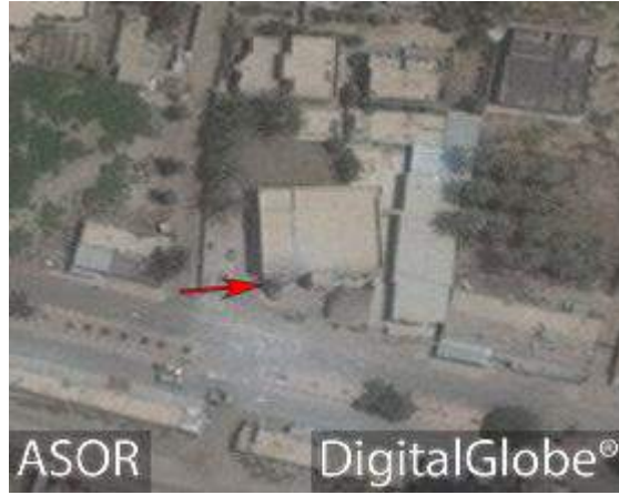
Visible damage to the minaret and roof of the mosque with debris seen in the street (DigitalGlobe; June 5, 2016)
