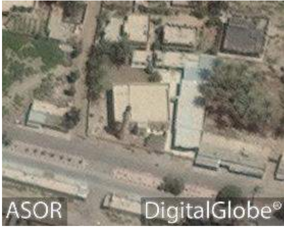
Image of mosque prior to damage (DigitalGlobe; May 28, 2016)
