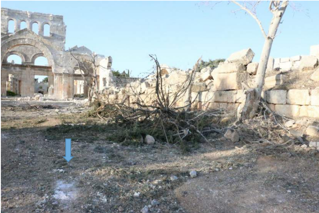
South façade of the Church of St. Simeon (Photo facing northeast)
