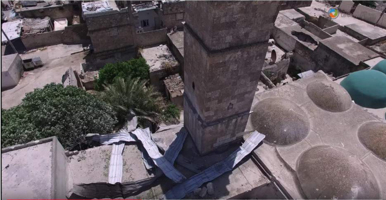
Damage to al-Kabir Mosque (Ammar Ahmadou; June 2, 2016)
