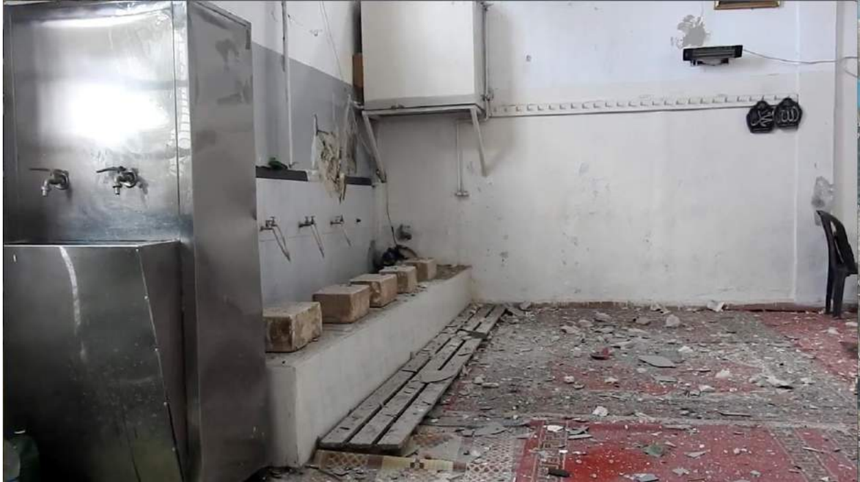
Video still of damage to the interior of Souq al-Hal Mosque (Ammar al-Nasser; May 9, 2016)
