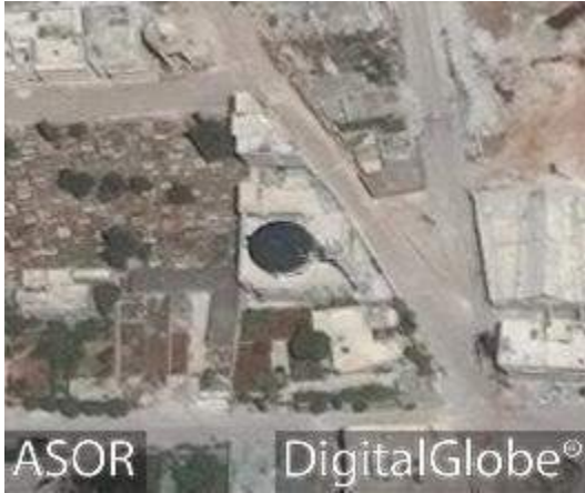
Amer Abu Obaida Ibn al-Jarah Mosque prior to damage. (DigitalGlobe; May 20, 2016)
