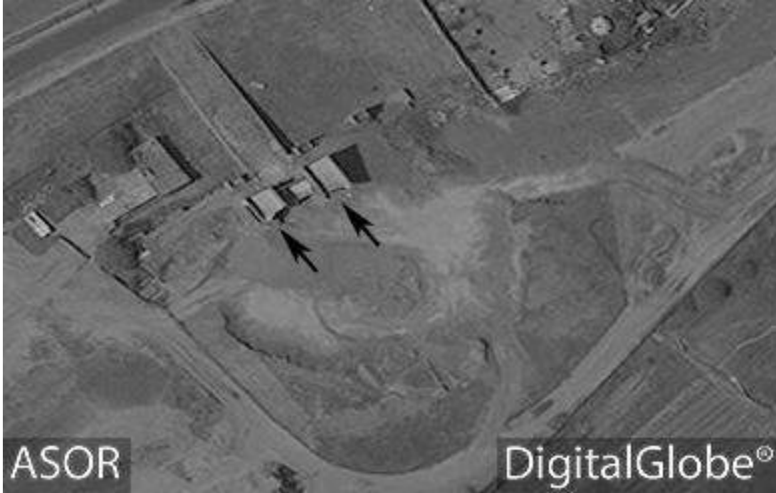
Nergal Gate with damage on the southern side indicated by the black arrows. (DigitalGlobe; May 25, 2016)
