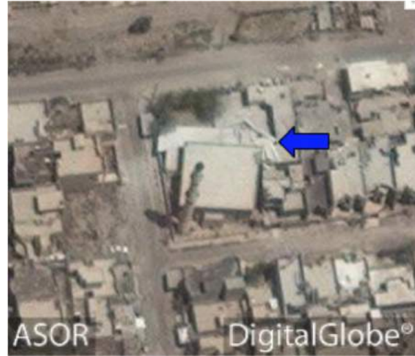
Visible damage to the metal roof directly north of the main mosque (DigitalGlobe; May 28, 2016)
