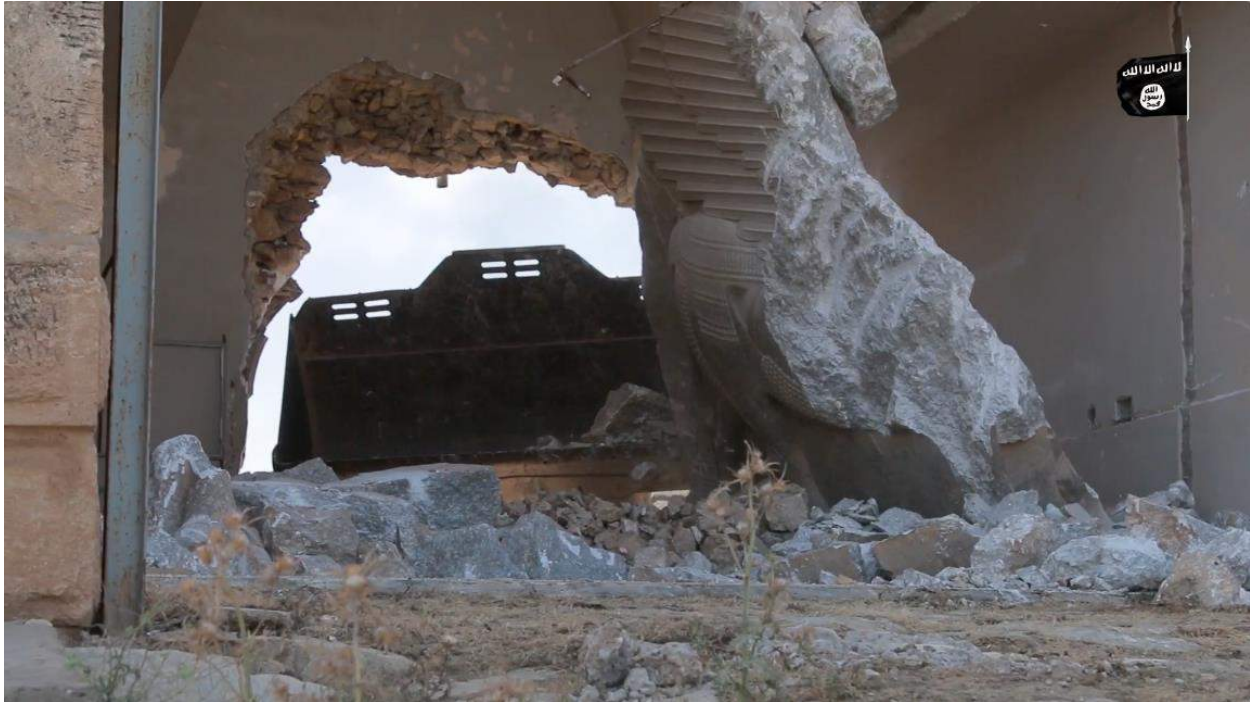
An earthmover knocking over a Winged Bull at the reconstructed Nergal Gate (Amaq News Agency; Downloaded June 7, 2016)
