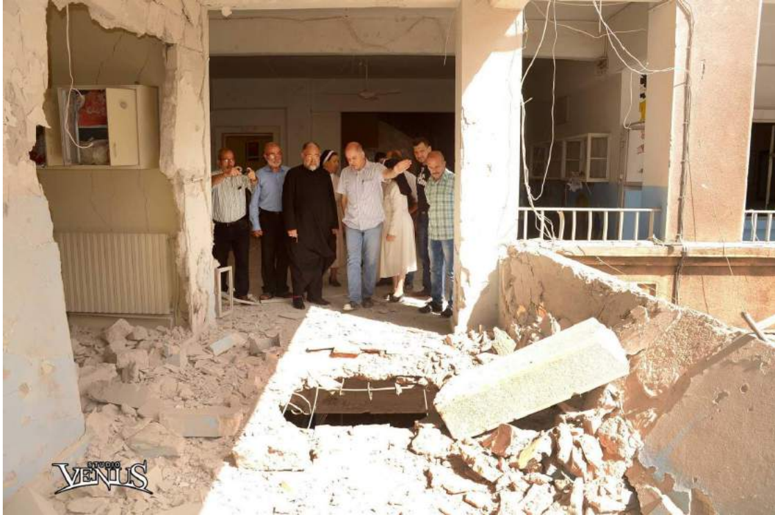
Severe structural damage to Zvartnots School (Kantsasar/Studio Venus; June 3, 2016)
