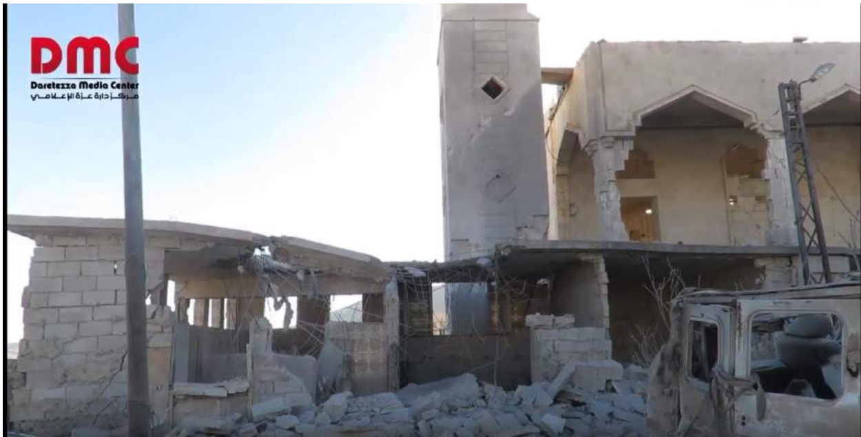
Video still showing damage to eastern side of al-Farouq Mosque (Daretezza Media Center; June 5, 2016)
