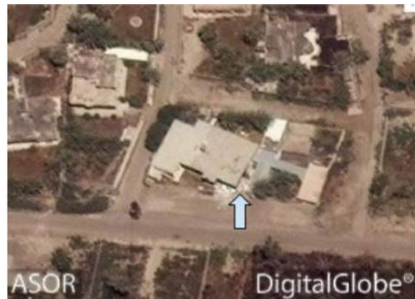
Debris can be seen outside the southeastern corner (DigitalGlobe; May 31, 2016)
