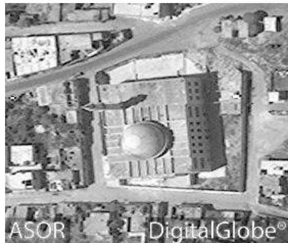
No visible damage to the mosque due to location of hole in the dome (DigitalGlobe; June 2, 2016)
