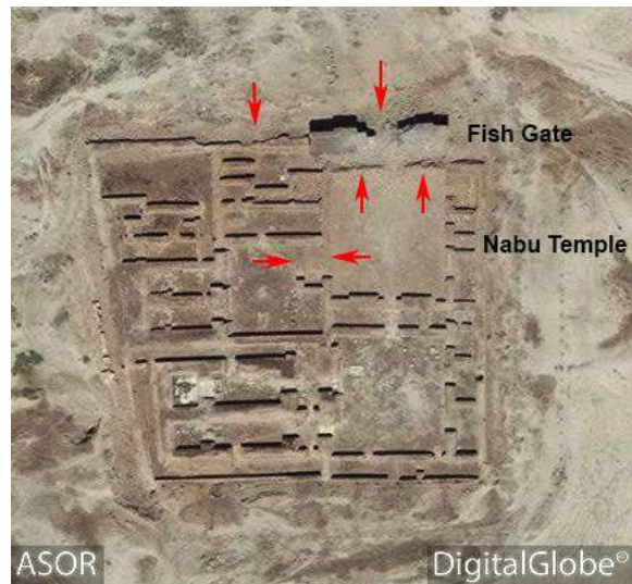
Damage to the Fish Gate and the Temple of Nabu, outlined with red arrows. Note the two missing interior walls in addition to areas damaged by the explosives. (ASOR CHI/DigitalGlobe; June 3, 2016)
