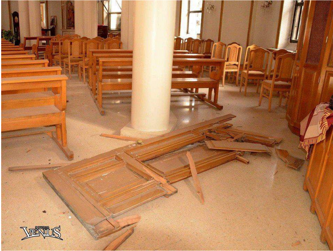
Damage to church door (Kantsasar/Studio Venus; June 5, 2016)
