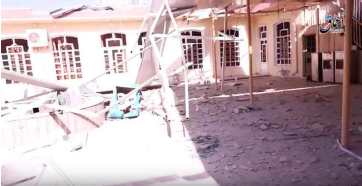
Video still of damage to al-Mudallal Mosque (Amaq News Agency; May 28, 2016)
