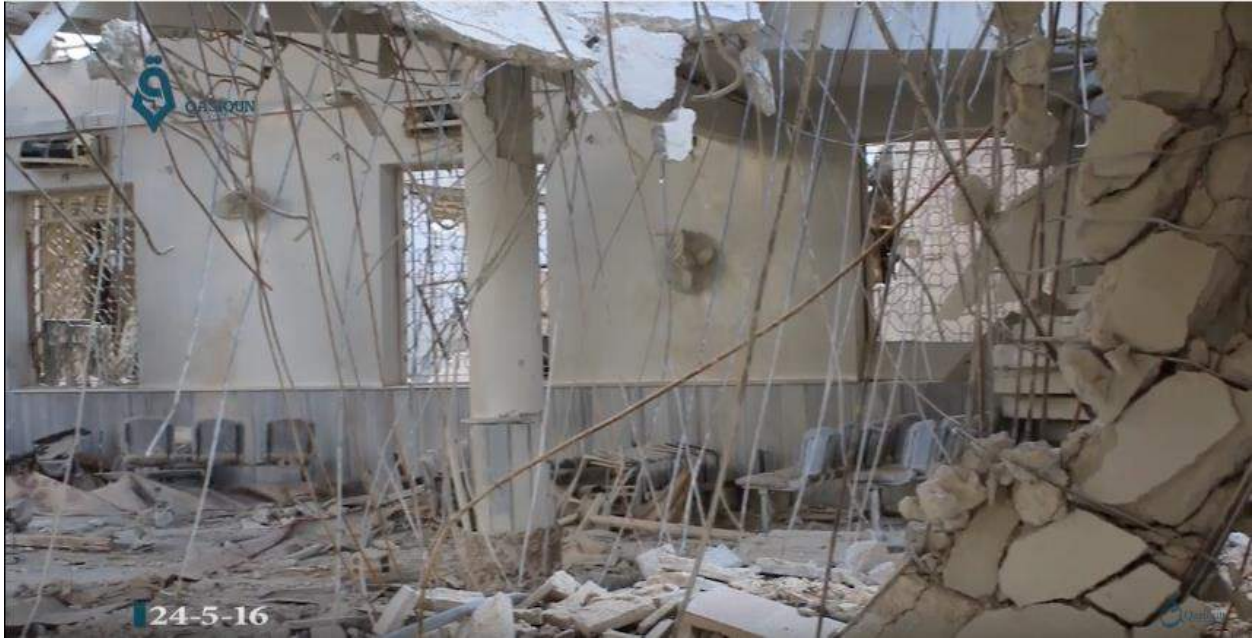
Video still of damage to the interior of al-Kabir Mosque (Qasioun News Agency; May 24, 2016)
