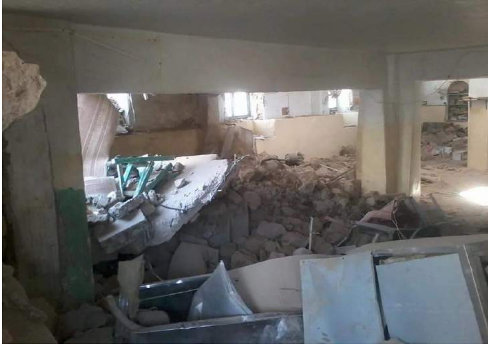
Interior damage to Uthman bin Affan Mosque (Sukhna al-Hadath; May 20, 2016)
