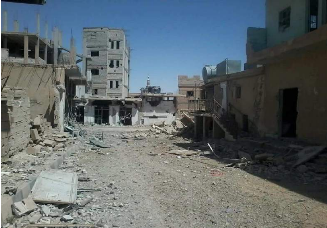
Surrounding damage to Uthman bin Affan Mosque (Sukhna al-Hadath; May 20, 2016)
