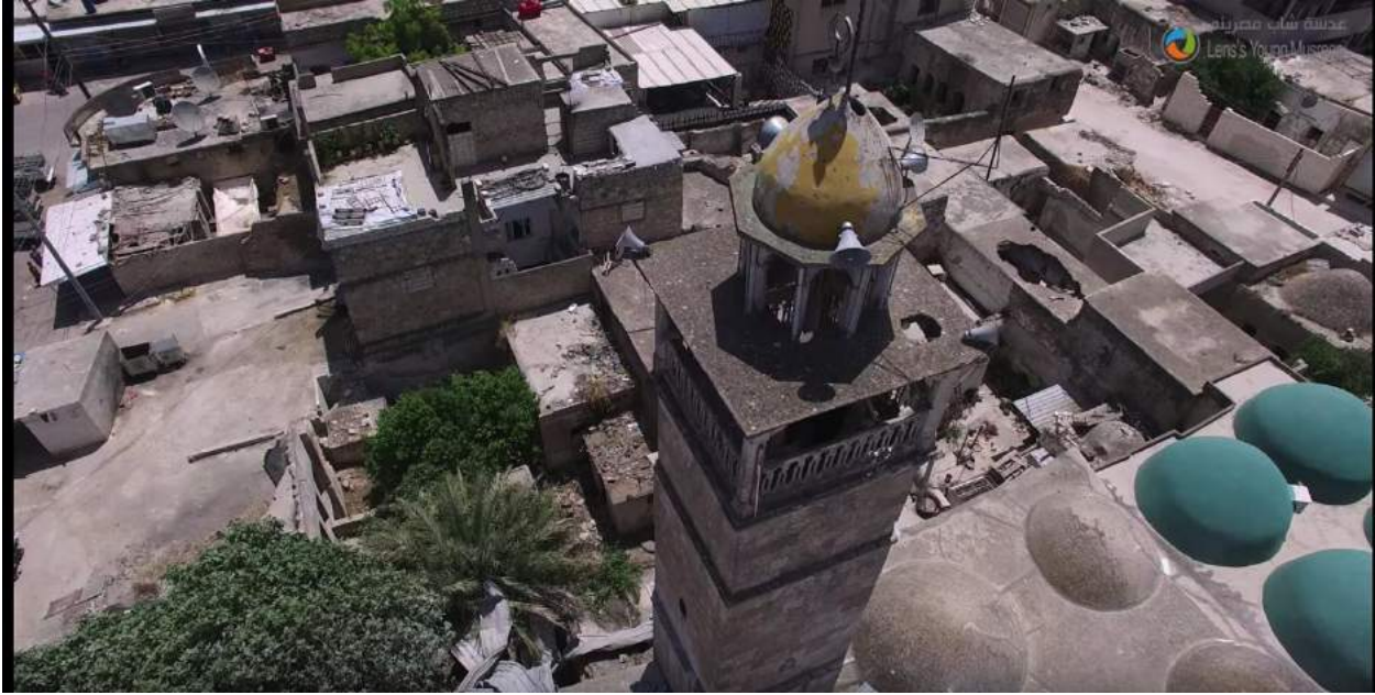
Damage to al-Kabir Mosque (Ammar Ahmadou; June 2, 2016)
