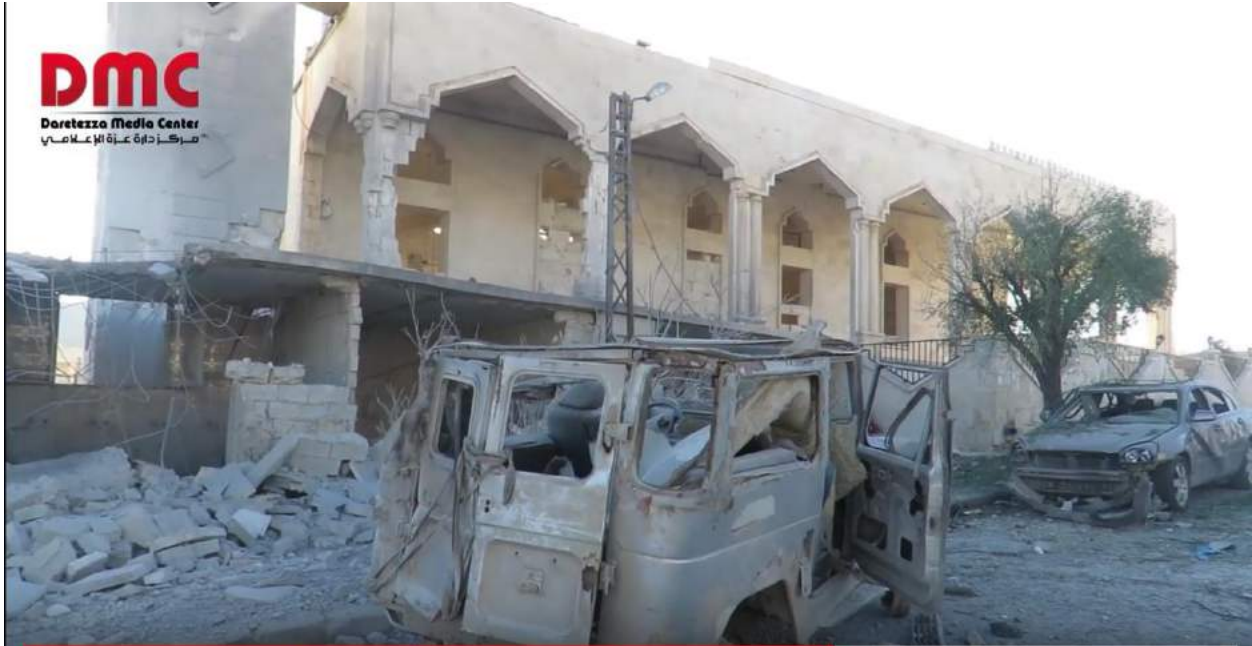
Video still showing damage to eastern side of al-Farouq Mosque and surrounding area (Daretezza Media Center; June 5, 2016)
