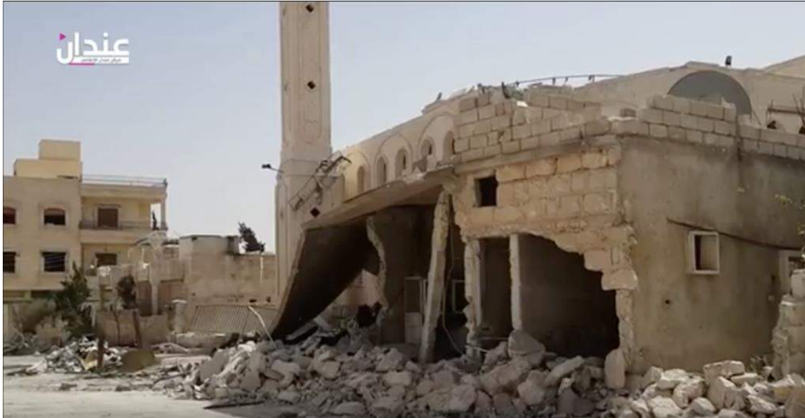
Video still of surrounding damage to Amer Abu Obaida Ibn al-Jarah Mosque (Anadan Media Center; June 5 2016)
