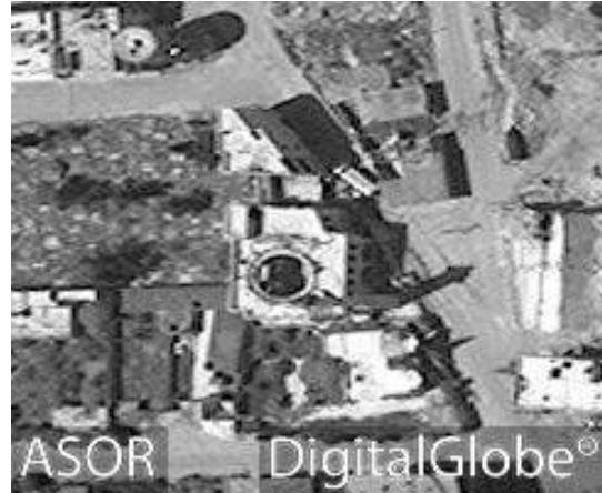
Visible damage to the dome of the mosque (DigitalGlobe; June 2, 2016)
