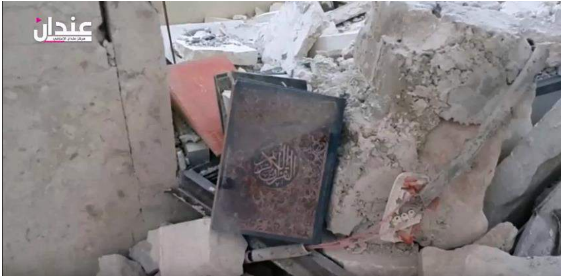
Video still of damage to Amer Abu Obaida Ibn al-Jarah Mosque (Anadan Media Center; May 30 2016)
