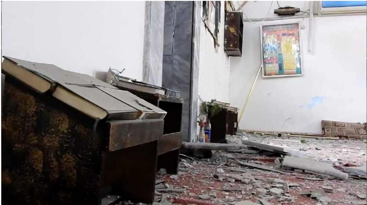
Video still of damage to the interior of Souq al-Hal Mosque (Ammar al-Nasser; May 9, 2016)
