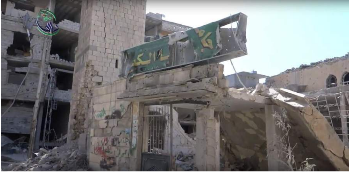
Video still of al-Kabir Mosque showing the base of the minaret and what remained of the surrounding structure as it appeared in May 2014 (Local Council Daraya; May 30, 2014)
