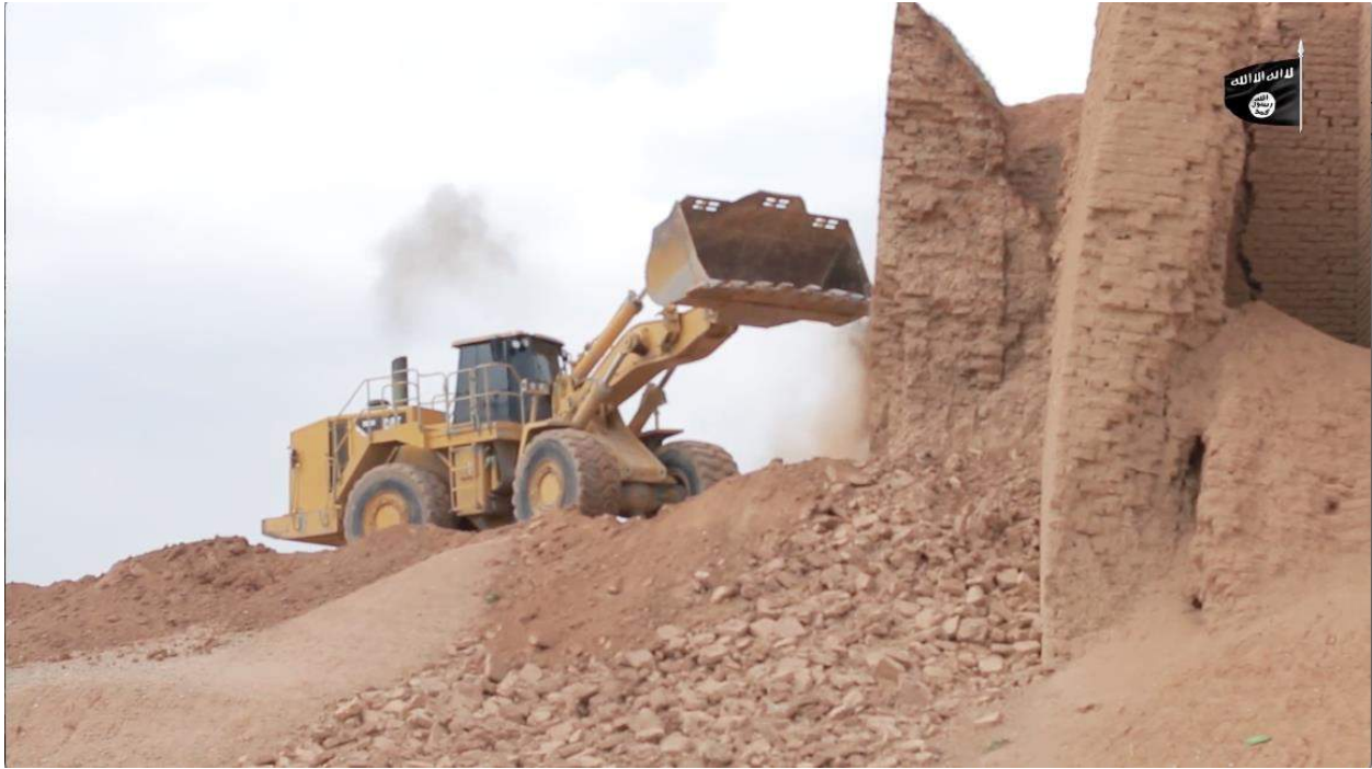
Video still of an earthmover driving into the reconstructed Adad Gate (Amaq News Agency; Downloaded June 7, 2016)
