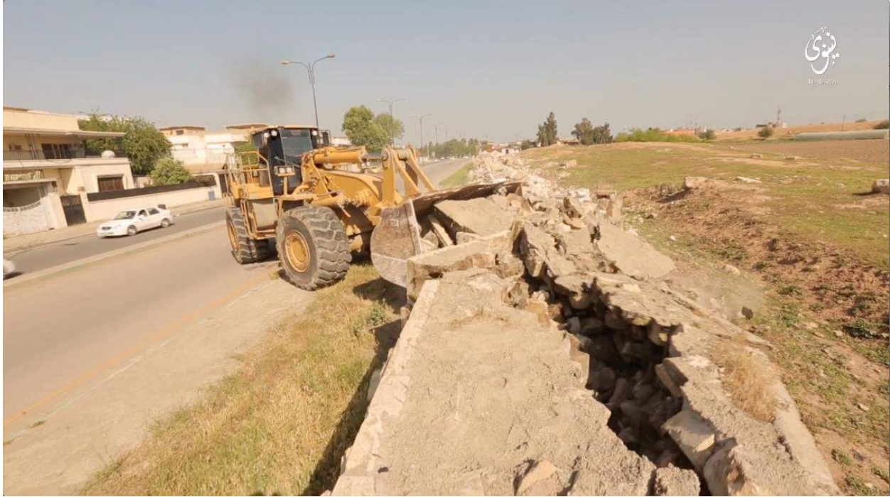
Video still of an earthmover destroying a modern wall at the ancient site of Nineveh (Amaq News Agency; Downloaded June 7, 2016)
