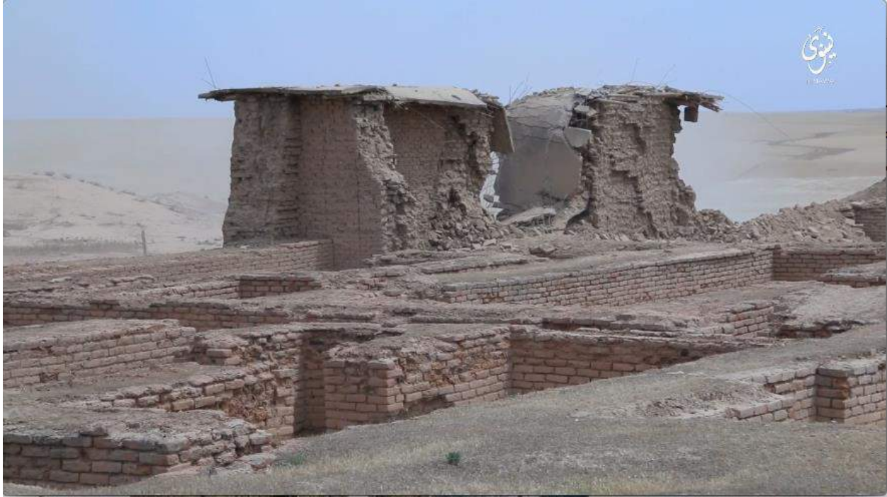
Remains of Fish Gate after detonation (facing northeast) (Mosul Eye; June 7, 2016)
