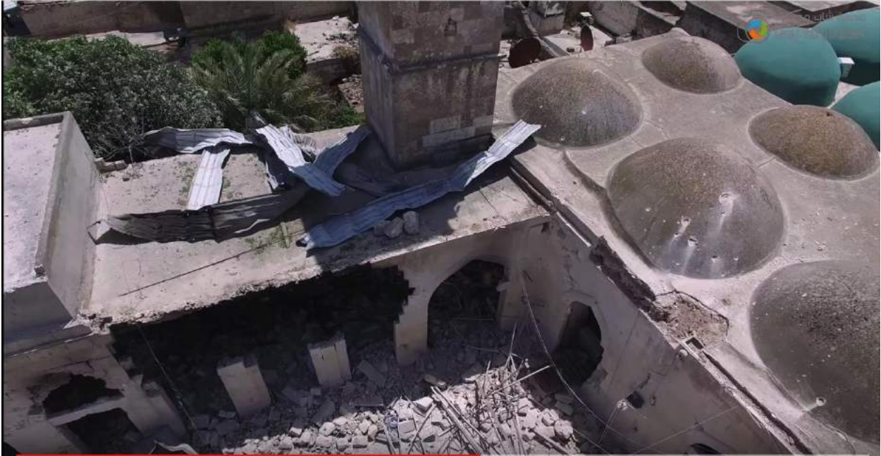
Damage to al-Kabir Mosque interior courtyard (Ammar Ahmadou; June 2, 2016)
