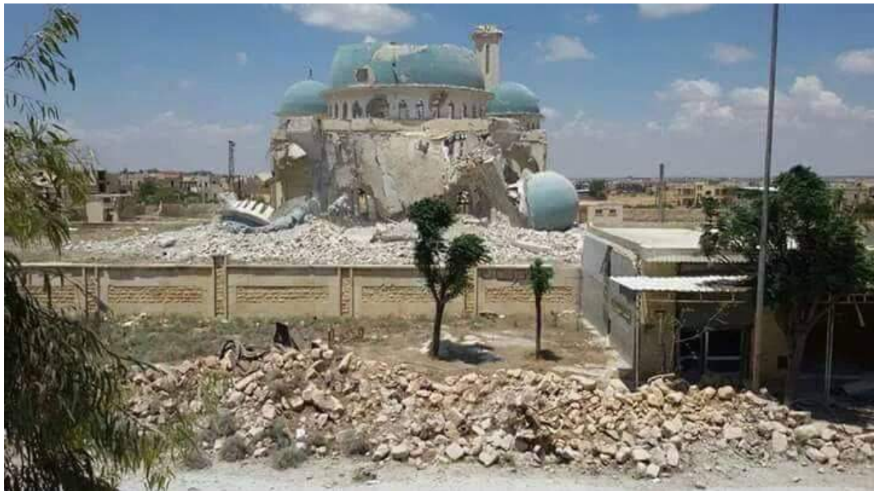
Damage to Sahib bin Sinan al-Roumi Mosque (Khaled Al Homsy; June 7, 2016)
