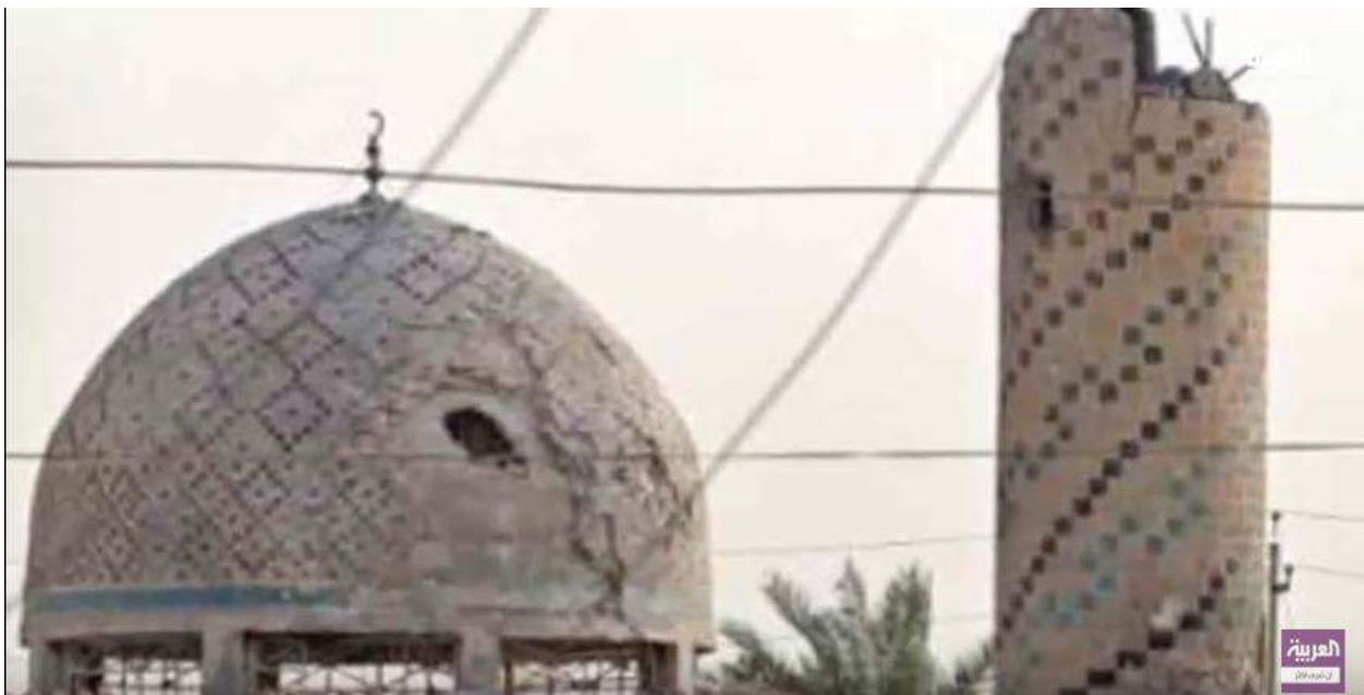
Video damage to the dome and minaret of one of the mosques allegedly damaged by the Popular Mobilization Front (Al Arabiya; May 28, 2016)
