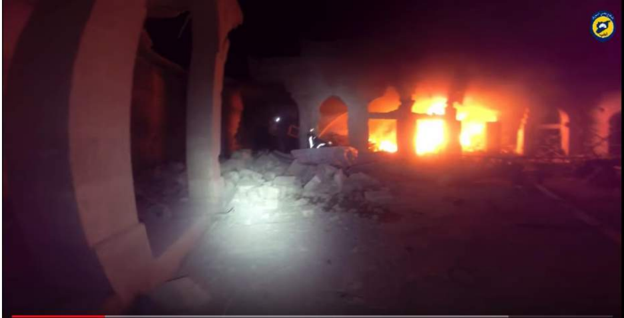
Fire damage to al-Kabir Mosque interior courtyard (Ammar Ahmadou; June 2, 2016)
