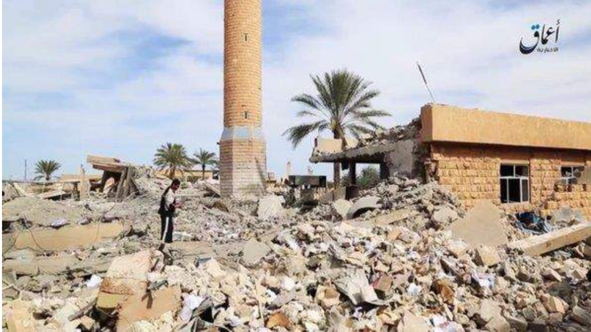
Damage to al-Farooq Mosque (Christiaan Triebert; March 15, 2016) 107
