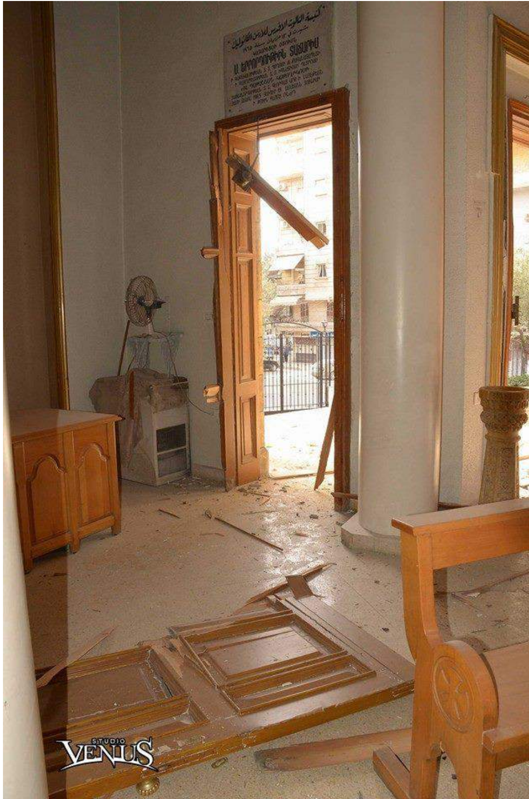
Damage to church doorway (Kantsasar/Studio Venus; June 5, 2016)
