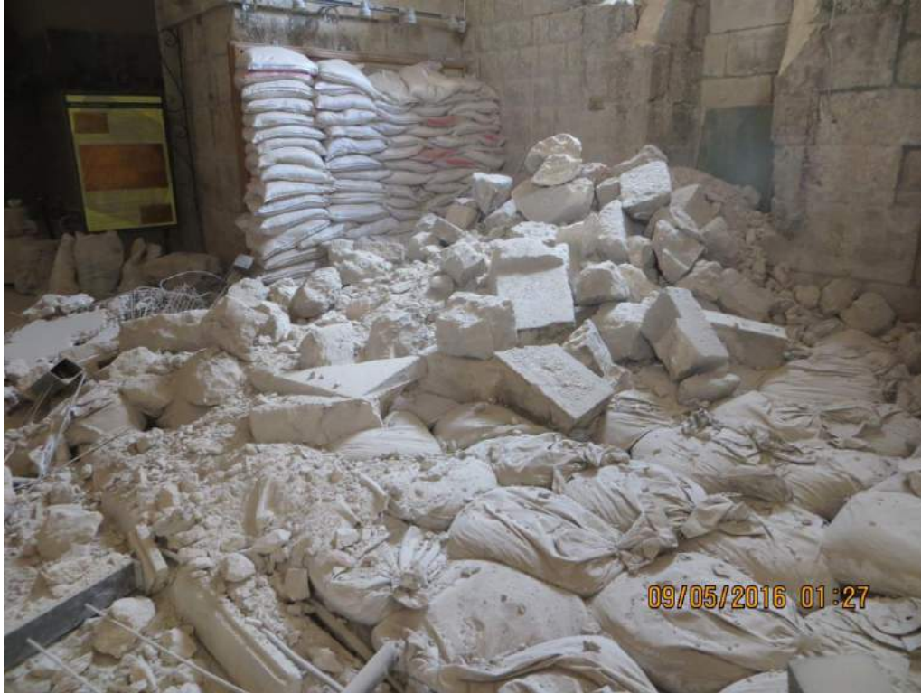
Rubble collapse over mosaic
