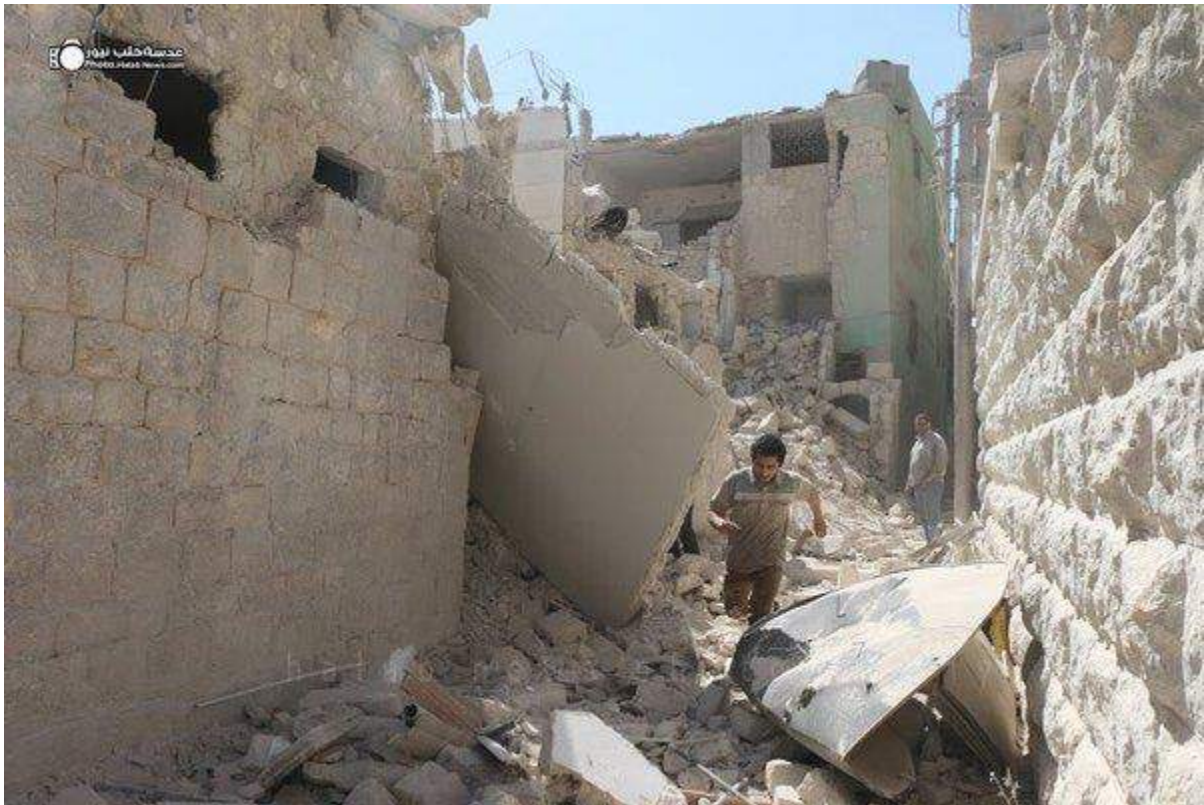
Significant damage and rubble present at the Nabhaniyah Institute (Twitter; April 29, 2016)
