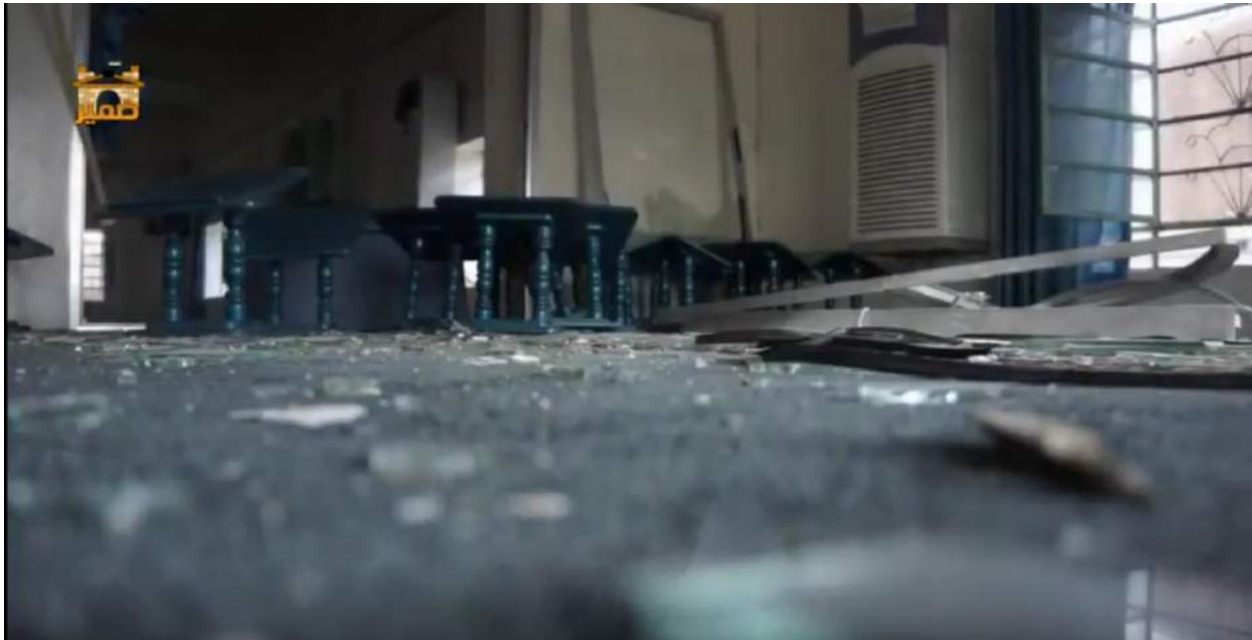
Interior damage and broken glass inside the Abu Bakr al-Sidiq Mosque (Media Abu Mohammad; April 28, 2016)
