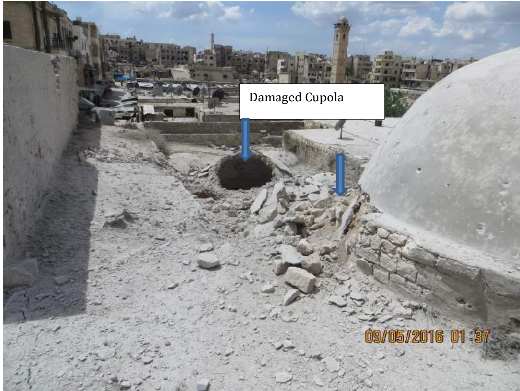
Roof of the Bathhouse (Hammam)
