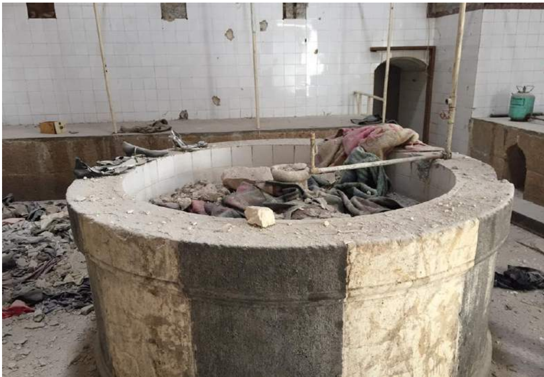
Interior damage at the Al-Ma'arra Museum (Al Watan FM; May 9, 2015)
