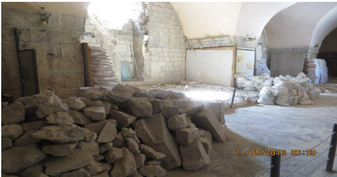
Stone masonry piled up for safekeeping
