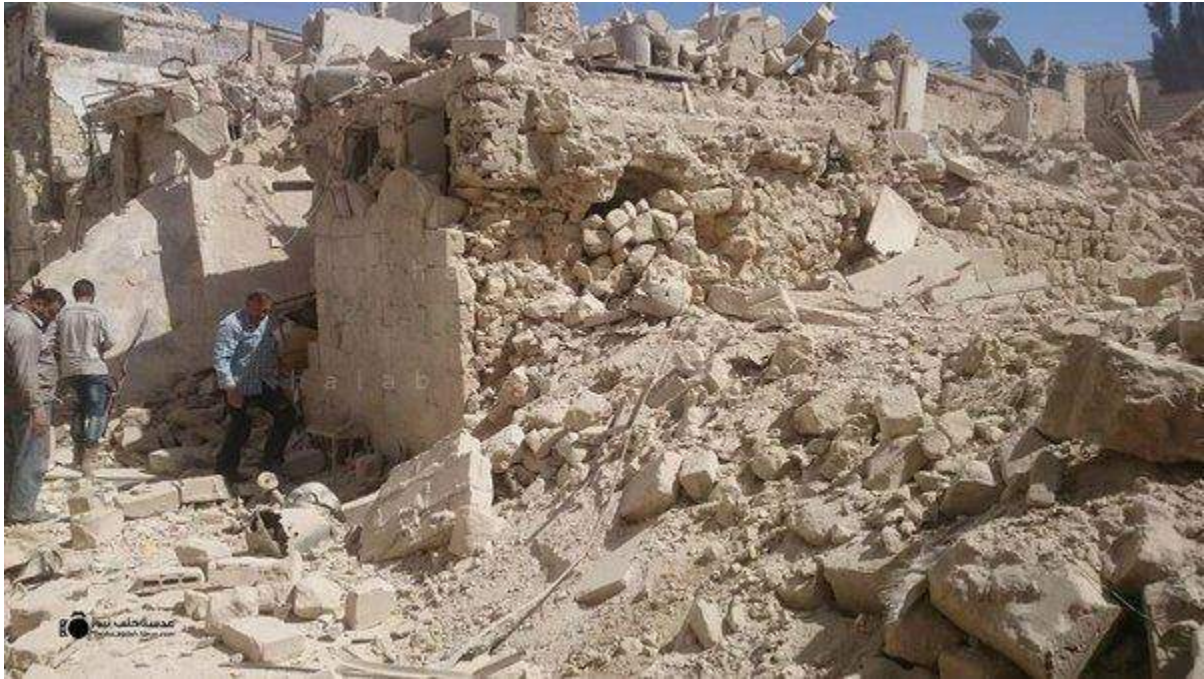
Severe damage at the Nabhaniyah Institute (Twitter; April 29, 2016)
