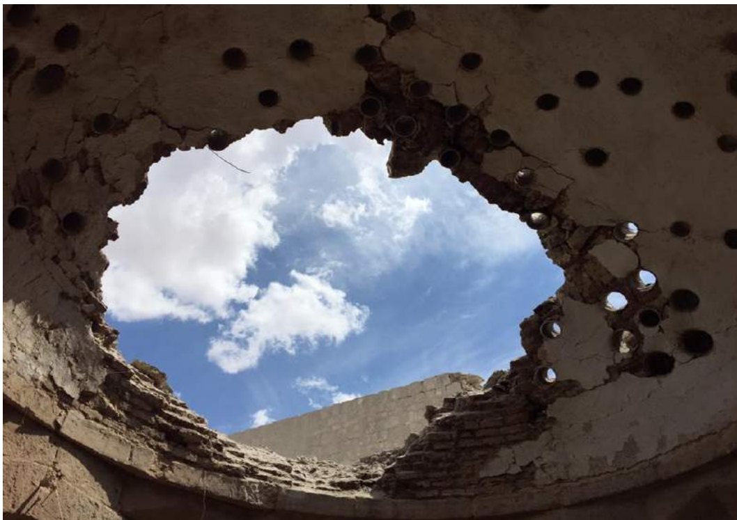
A hole through the domed ceiling at the Al-Ma'arra Museum (Al Watan FM; May 9, 2015)
