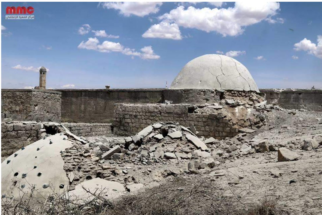
Airstrike damage at the Al-Ma'arra Museum (republished by APSA; May 9, 2016)
