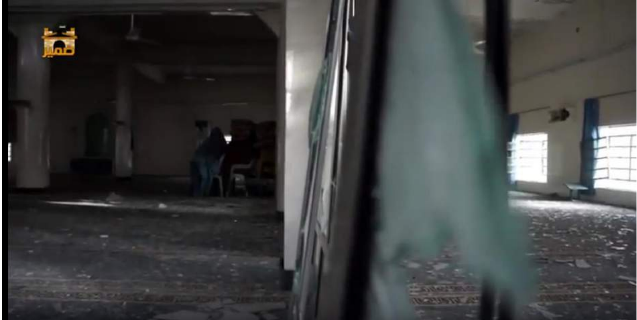
Interior damage to the Abu Bakr al-Sidiq Mosque (Media Abu Mohammad; April 28, 2016)
