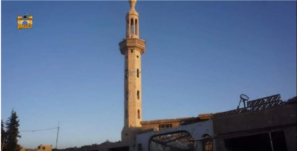
Damage to the exterior of the Abu Bakr al-Sidiq Mosque and minaret (Media Abu Mohammad; April 28, 2016)
