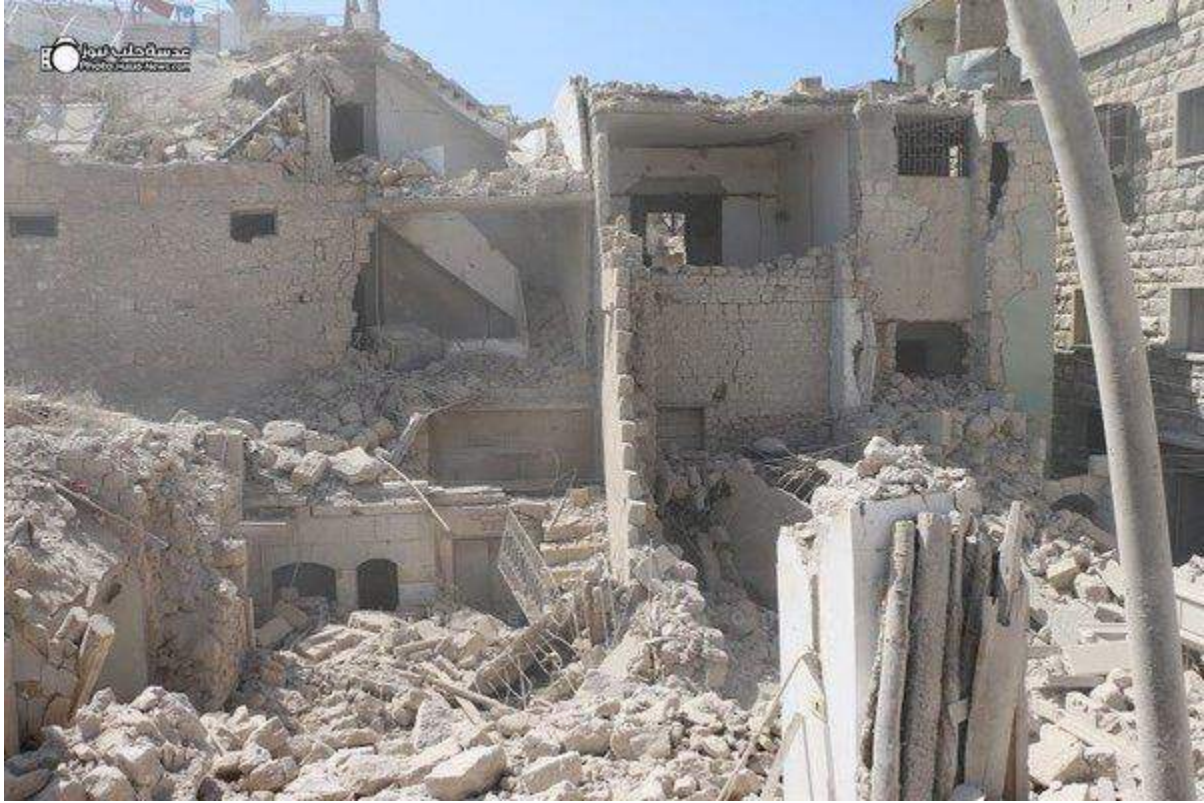
Damage to the Nabhaniyah Institute (Twitter; April 29, 2016)
