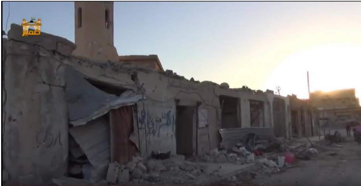
Damage to the exterior of the Abu Bakr al-Sidiq Mosque (Media Abu Mohammad; April 28, 2016)
