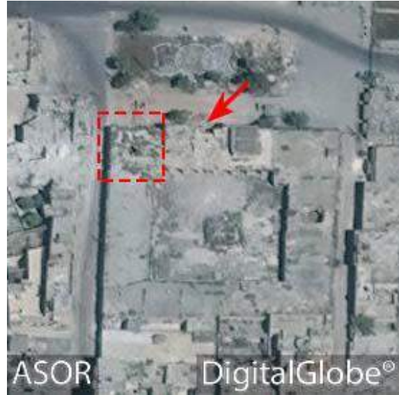
Damage to the northern wall and northwest corner (DigitalGlobe; April 22, 2016)
