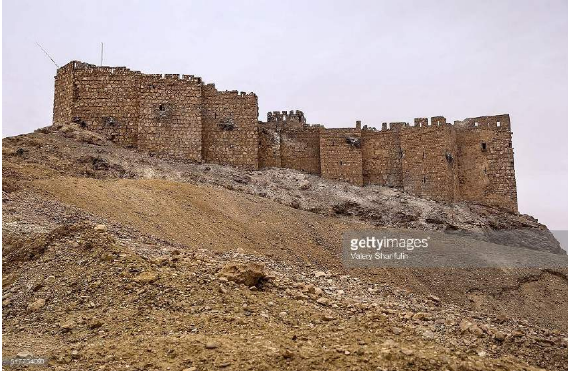
Airstrike damage on the western curtains walls (Valery Sharifulin/Getty; March 27, 2016) 146
