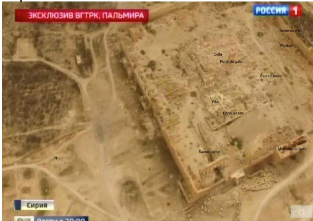
Temple of Bel complex showing damage to cella (Russia 24; March 25, 2016)
