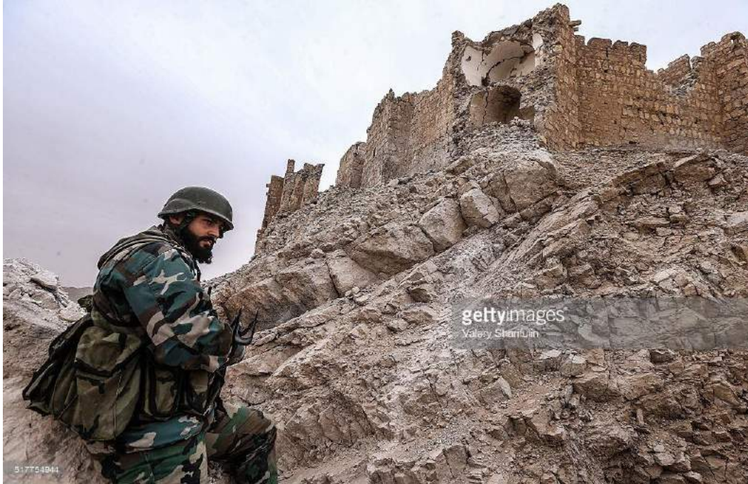
Major damage to northeastern corner of fortress (Valery Sharifulin/Getty; March 27, 2016) 153
