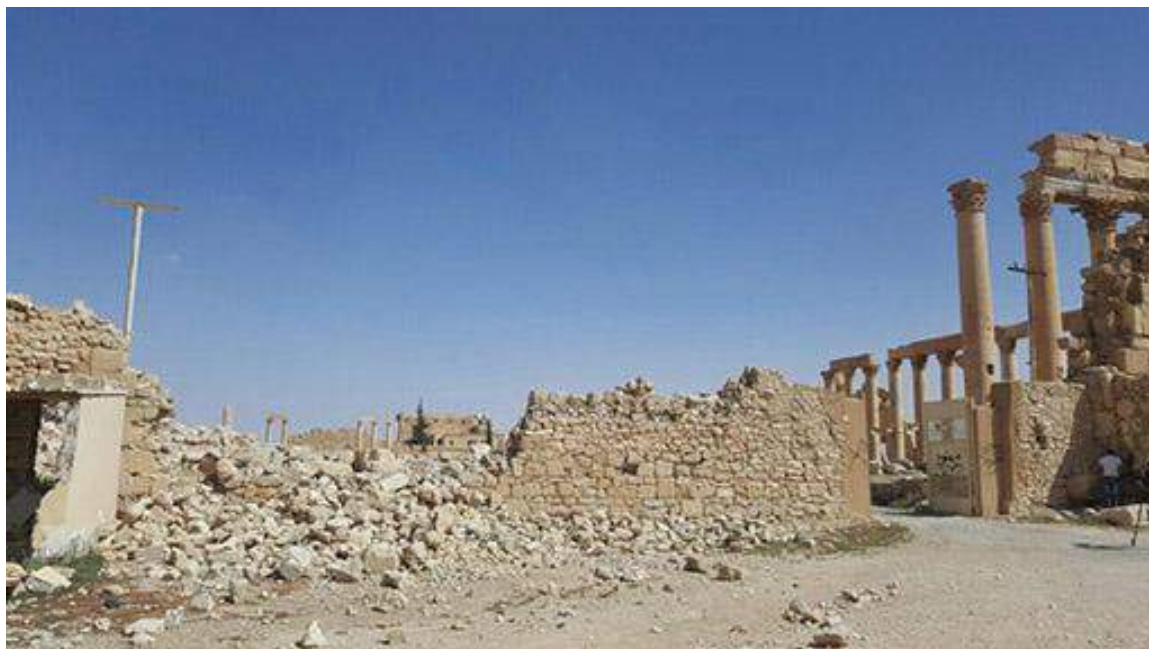
Collapsed section of exterior western wall of Temple of Bel complex, to the right of the Monumental Gateway (DGAM; March 27, 2016)
