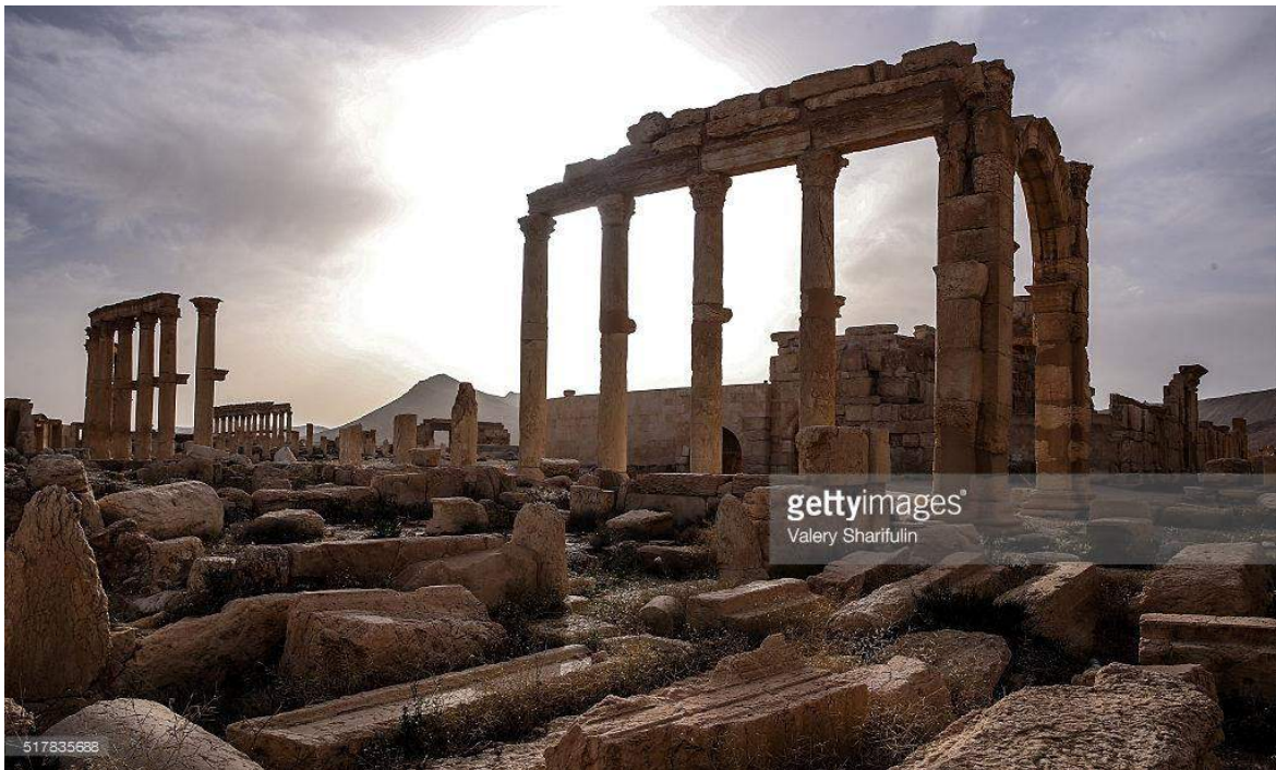
Eastern exterior portico of Theater complex (Valery Sharifun; March 27, 2016) 130
