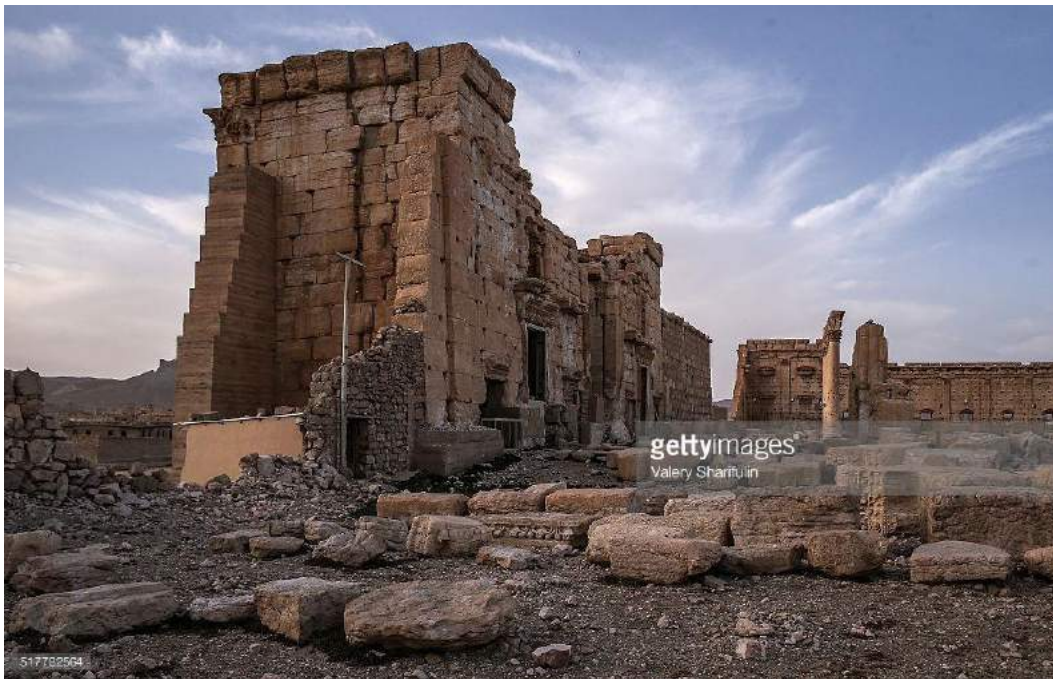
Interior of monumental gateway to Temple of Bel temenos with collapsed wall (left) (Valery Sharifulin/Getty; March 27, 2016) 121
