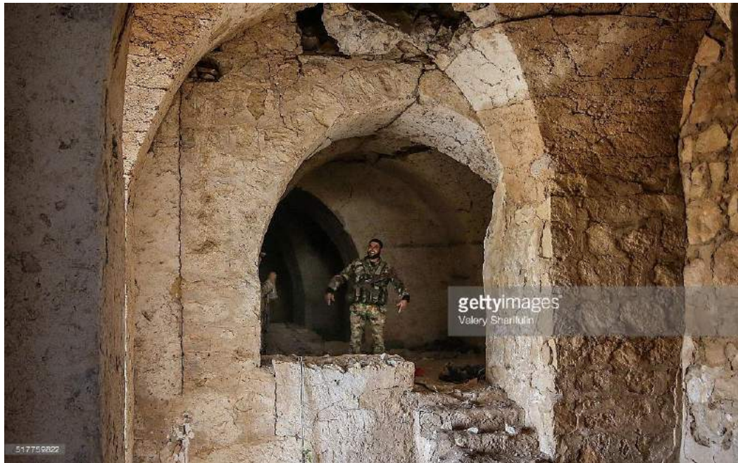
Partial ceiling collapse in fortress interior (Valery Sharifulin/Getty; March 27, 2016) 159
