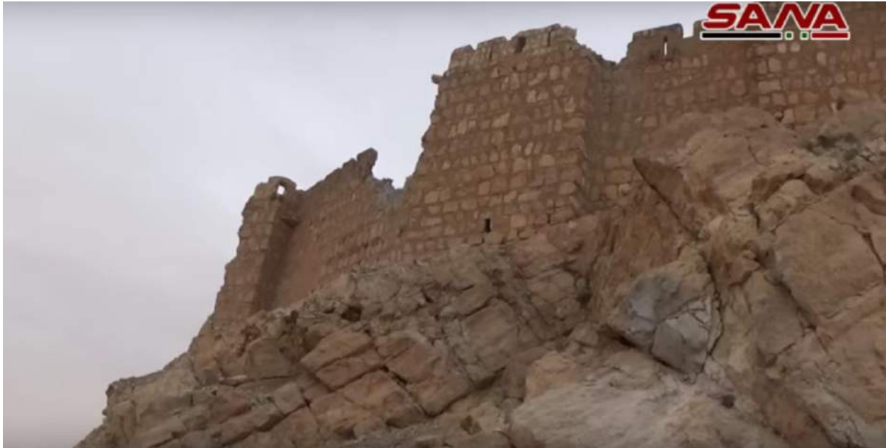
Partial collapse of eastern battlement (SANA; March 27, 2016)
