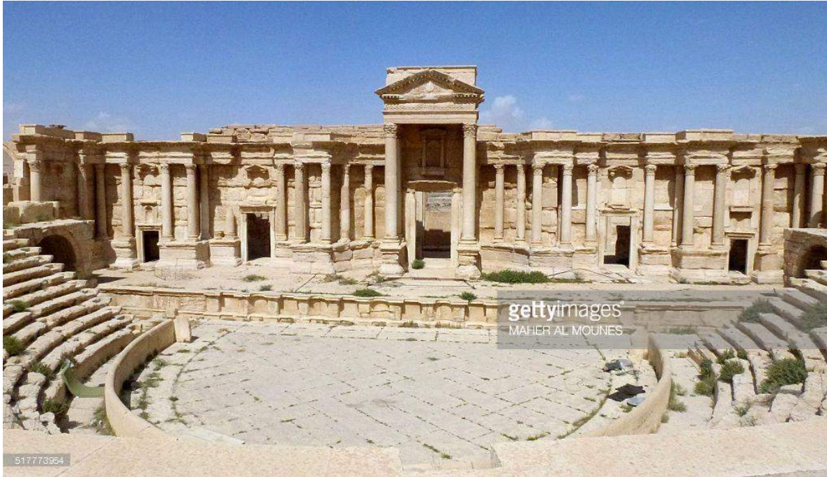
Interior of Theater with overgrown vegetation and debris on pulpitum and in orchestra (Maher Al Mounes; March 27, 2016) 129
