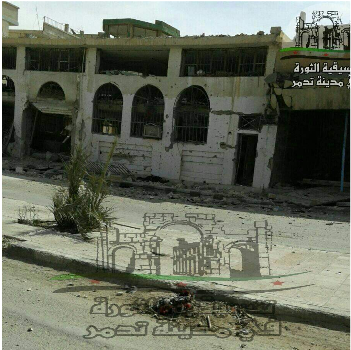
Damage to exterior of Bilal ibn Rabia Mosque (Palmyra Coordination; March 22, 2016)
