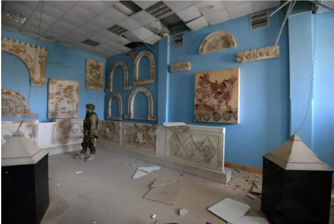
Damage to the Qasr Al Heir Hall (Sputnik; March 29, 2016)
