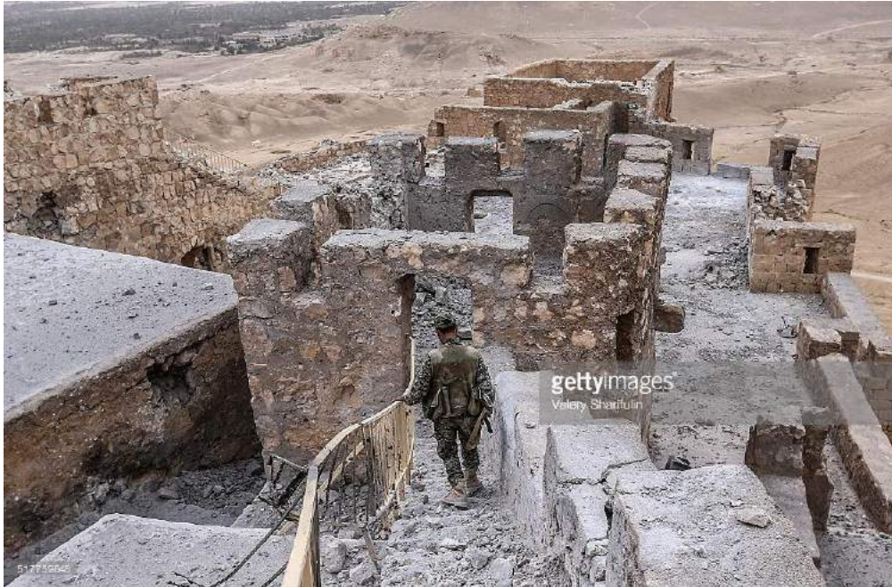
Debris on interior staircase (looking south) (Valery Sharifulin/Getty; March 27, 2016) 155
