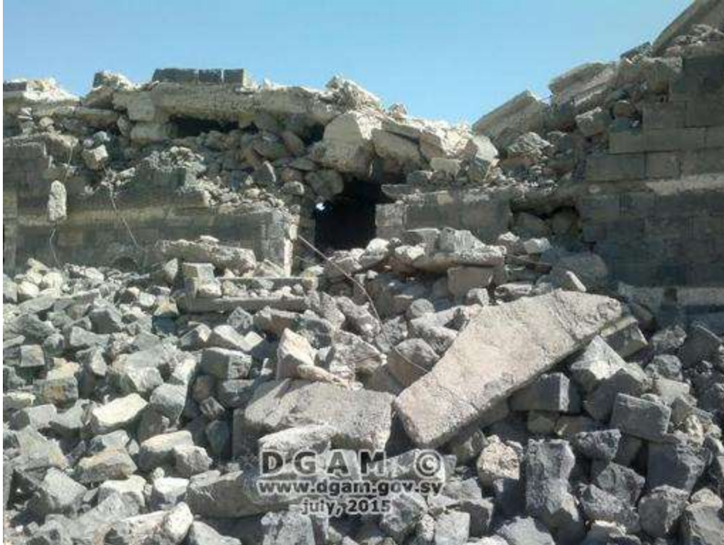
Al-Omari Mosque, Marbaa, after destruction (DGAM; July 20, 2015)
