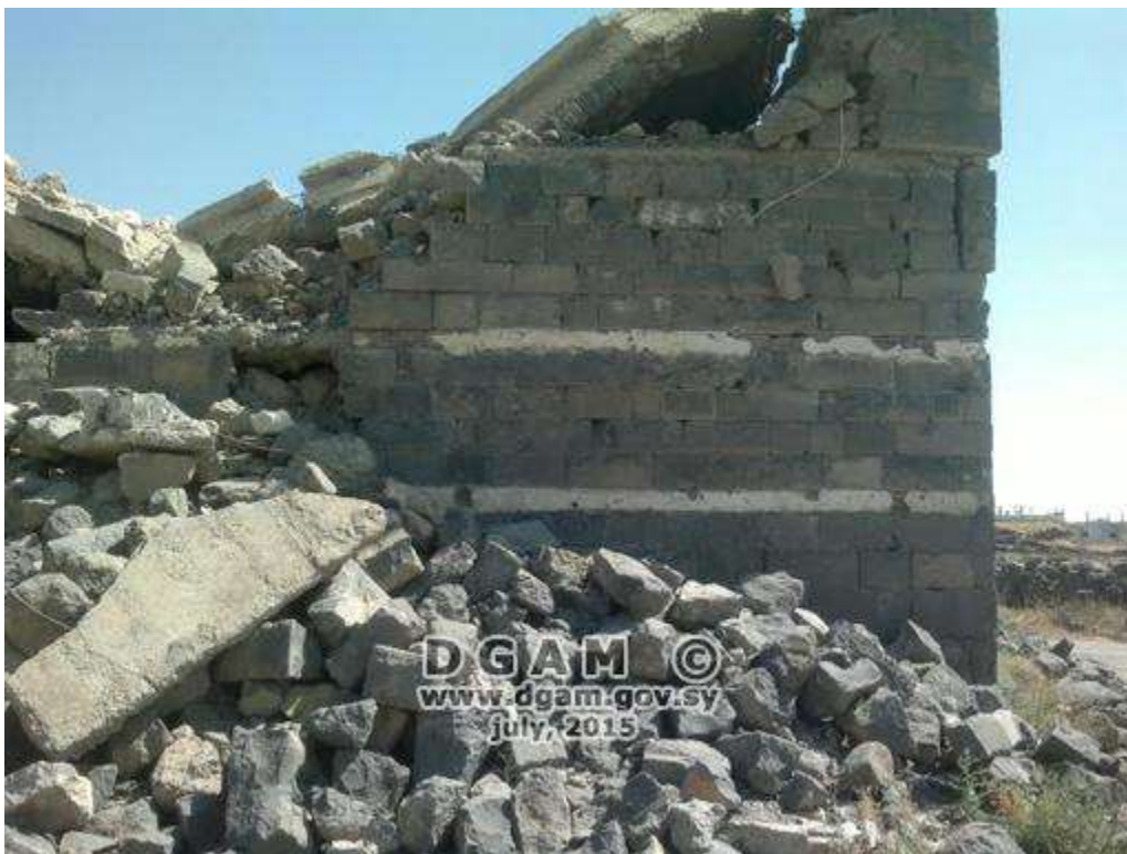
Al-Omari Mosque, Marbaa, after destruction (DGAM; July 15, 2015)
