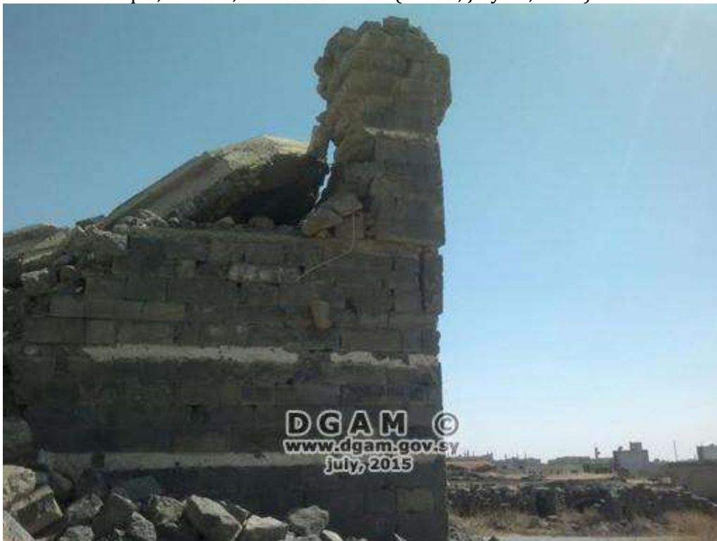
Al-Omari Mosque, Marbaa, after destruction (DGAM; July 15, 2015)
