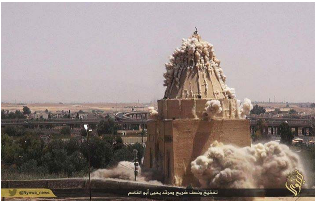
Demolition of the Shrine of Imam Yahya ibn al-Qasim (posted to the “Monuments of Mosul in Danger” Facebook page)
