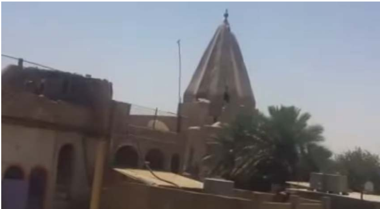
Mausoleum of Imam Ibn Hassan Awn al-Din, during demolition (YouTube, screenshot)
