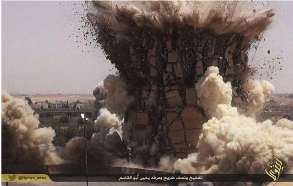
Demolition of the Shrine of Imam Yahya ibn al-Qasim (posted to the “Monuments of Mosul in Danger” Facebook page).
