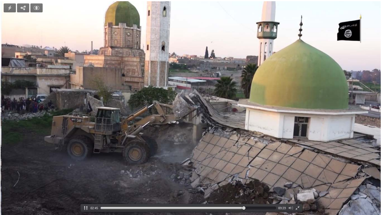
Mosque and Shrine of Imam al-Muhsin, during demolition (screenshot from video)
