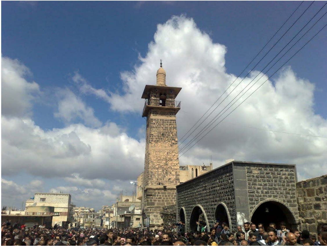
Omari Mosque from the southwest, Daraa, Syria (Panoramio; dated 3/15/2011). Note the differential masonry of arcade, minaret base, and minaret tower.
