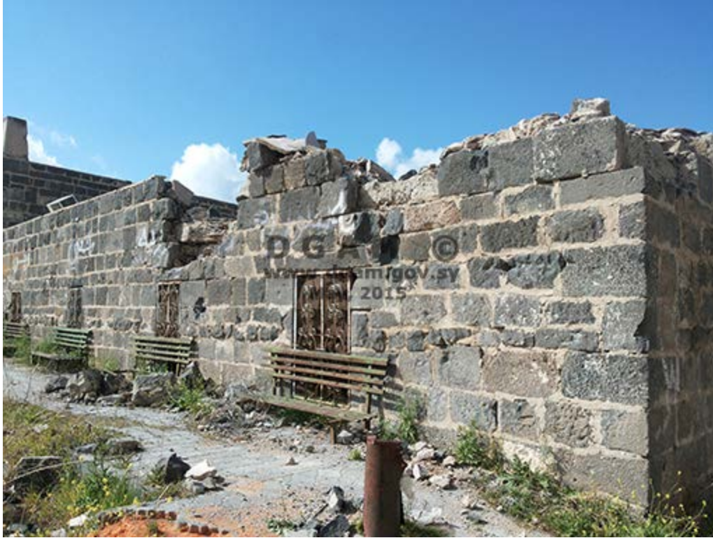
Omari Mosque, Daraa, Syria, showing damage to the facade (DGAM; posted April 29, 2015)
