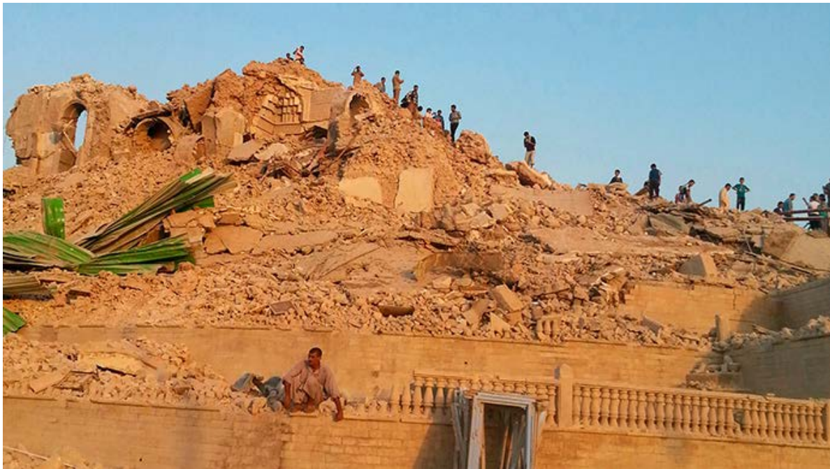
Shrine of Nebi Yunus following demolition (Reuters)
