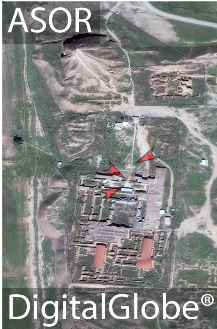
The Northwest Palace at Nimrud, Iraq, showing probable signs of intentional destruction of the structure and sculptures by ISIL. See ASOR CHI Incident Report IHI 15-0067 Update, below. (ASOR CHI; DigitalGlobe image taken in early March 2015)
