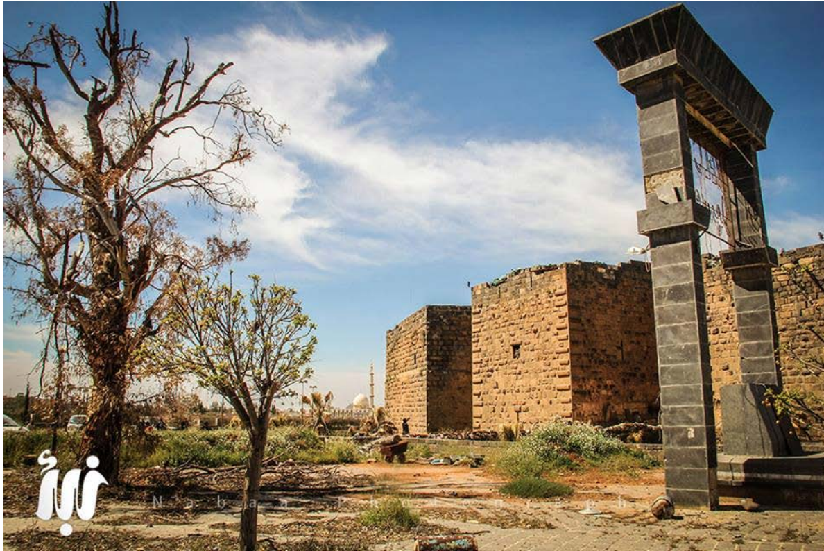
Bosra, exterior of Citadel/Roman Amphitheater (APSA; posted March 25, 2015)
