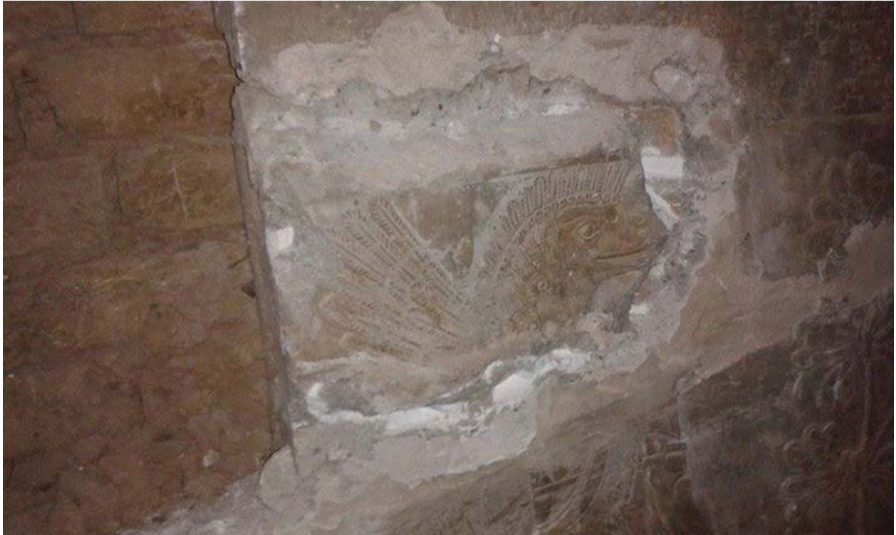
Alleged damage to the Northwest Palace at Nimrud, dating to October 2014 (Facebook)
