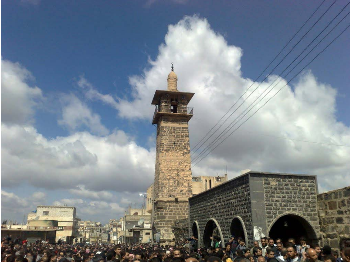
Omari Mosque from the southwest, Daraa, Syria. Note the differential masonry of arcade, minaret base, and minaret tower. (Panoramio; dated 3/15/2011)
