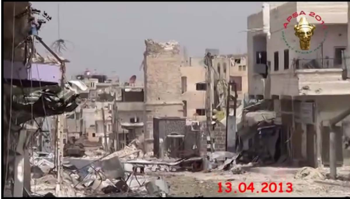
Omari Mosque, Daraa, Syria. This is a still image taken from footage filmed from the street south of the mosque, facing approximately the same direction as the first photograph above. Note the arcade, minaret base, and minaret tower, now truncated. (APSA; posted April 12–13, 2013)
