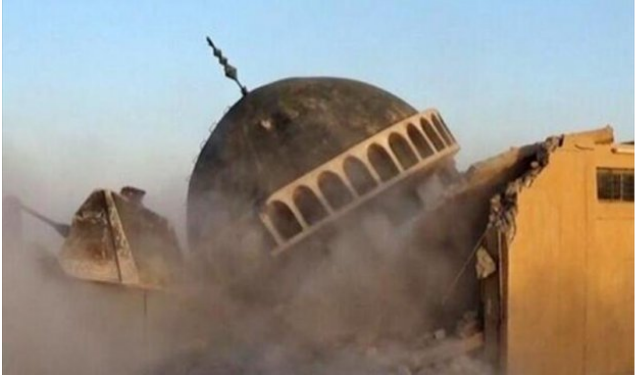
Demolition of the Tomb and Shrine of Ahmed ar-Rifa'i (posted on Twitter, original account now disabled)
