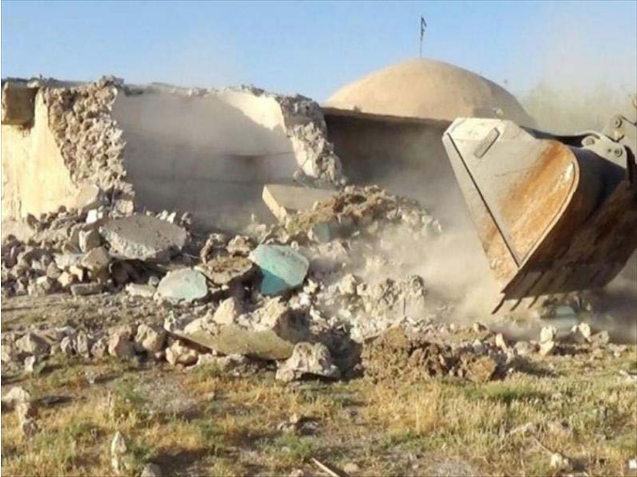
Demolition of Sheikh Ibrahim (Al-Wasat)
