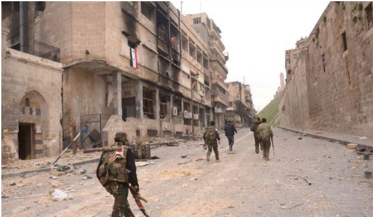
View from Matbakh al-Ajami (first building on the left) toward the Aleppo Citadel (APSA)
