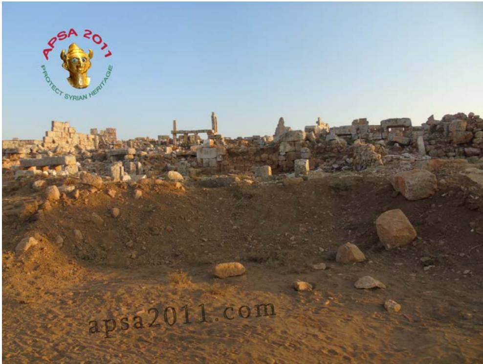
Deir Qita — an area of recent clearance, almost certainly using a front-end loader or bulldozer. (APSA)
