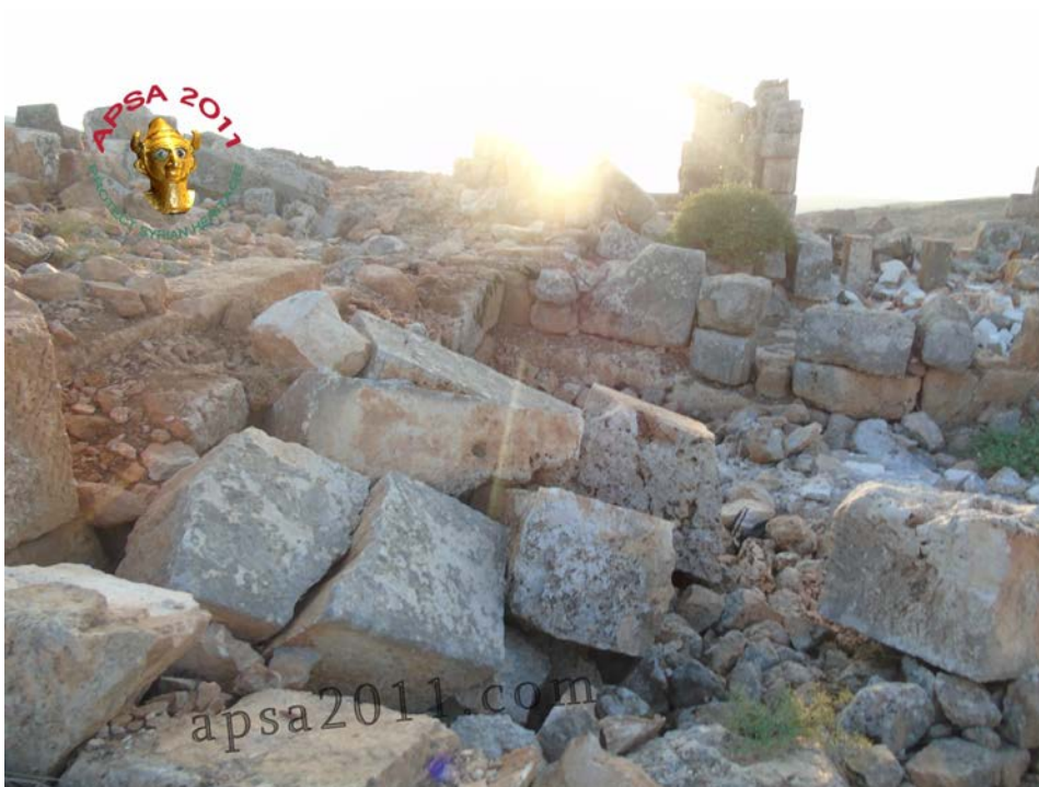
Deir Qita — fresh breaks in masonry visible on the right and newly toppled masonry and soil disturbance on the left. (APSA)
