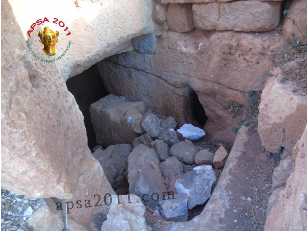
Site disturbance at Deir Qita with freshly broken limestone masonry in an ancient doorway. (APSA)
