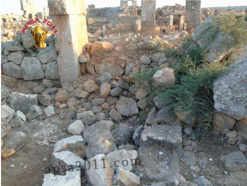
Deir Qita — fresh breaks in masonry visible in the foreground. Areas of darker red soil mark site disturbance. (APSA)
