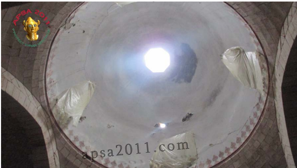
Damage to one of the domes of the Hammam Yalbougha (bathhouse) in Old Aleppo (APSA).
