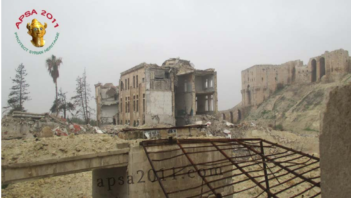
Damage to the Hammam Yalbougha (bathhouse) in Old Aleppo — showing the remains of the Old Serail in the distance (APSA).
