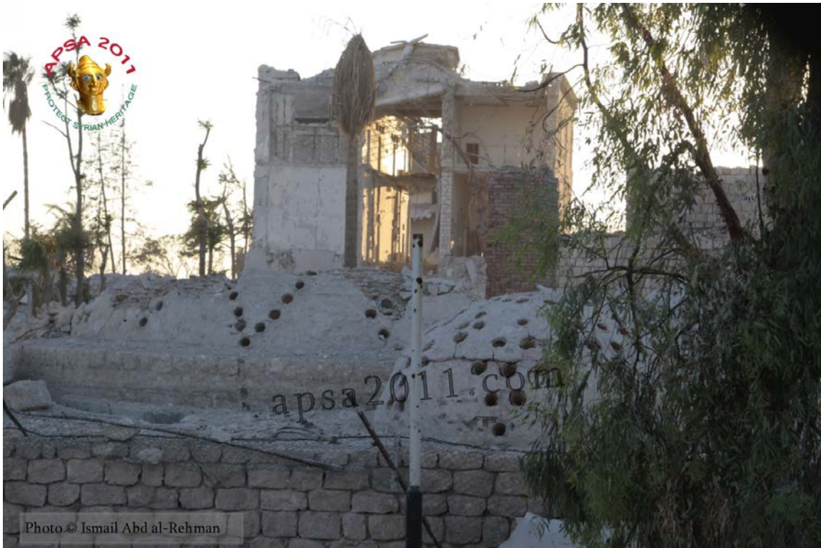
Damage to Hammam Yalbougha (bathhouse) in Old Aleppo (APSA).
