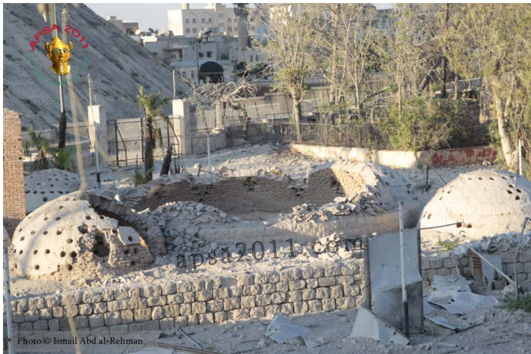
Damage to one of the domes of the Hammam Yalbougha (bathhouse) in Old Aleppo (APSA).
