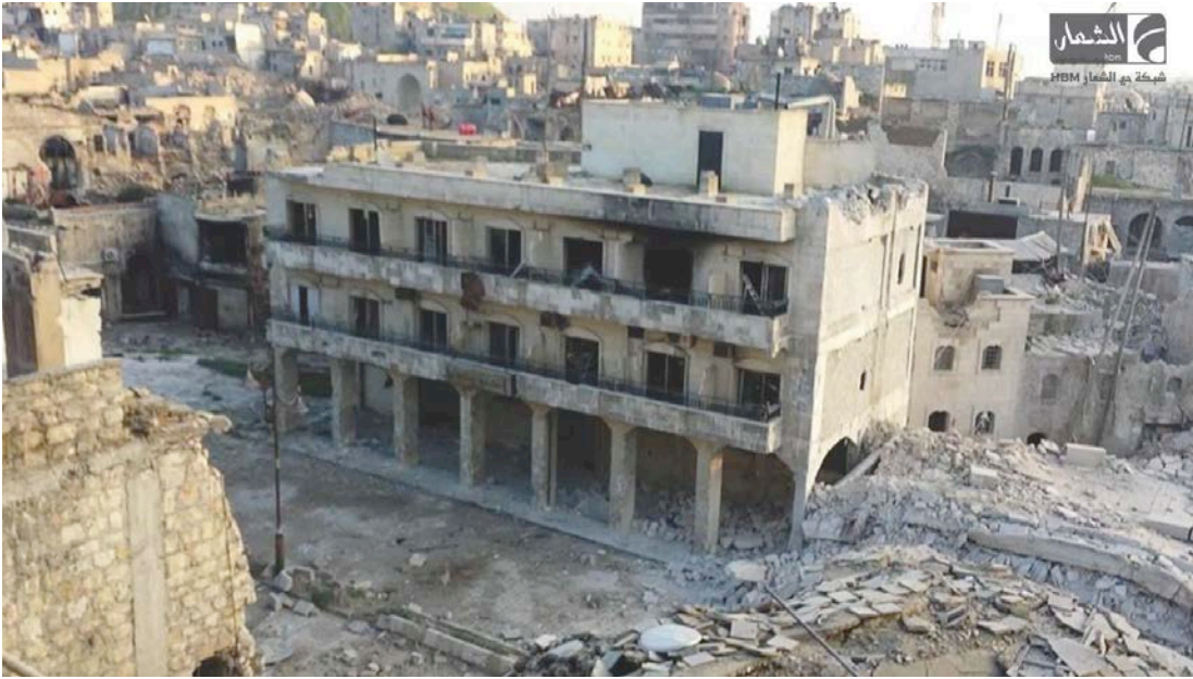
View of the new modern structure (left, No. 4 on the map) beside the modern structure destroyed in the Dec. 30, 2014 tunnel bomb blast (right, No. 3 on the map) (HBM).
