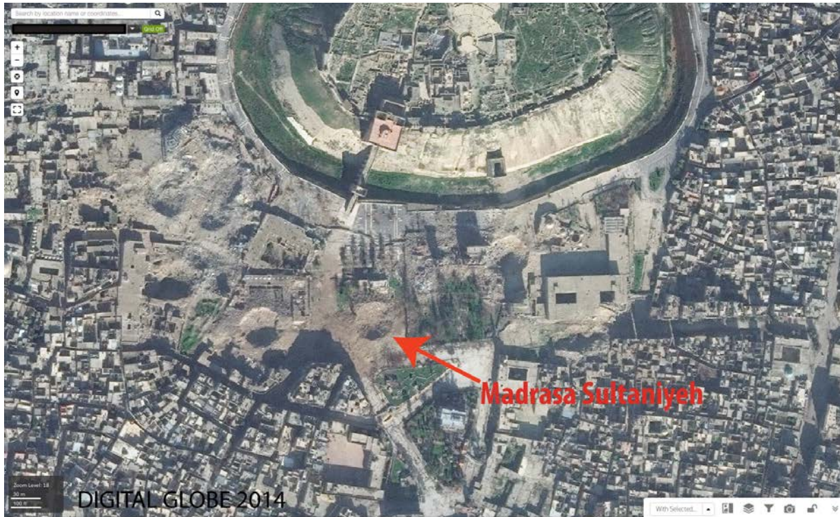
Digital Globe Image of the Madrasa Sultaniyeh dating to December 15, 2014. The tunnel bomb of December 7, 2014 destroyed the southern half of the building (Digital Globe).
