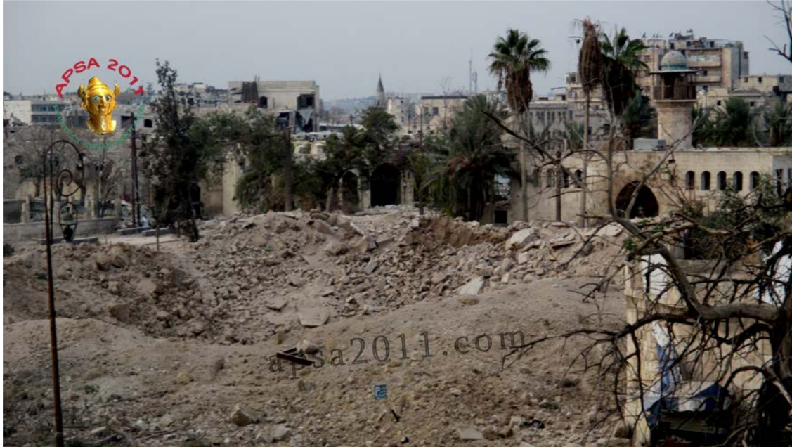
The remains of the Madrasa Sultaniyeh from the south following the tunnel bombing of December 7, 2014.
