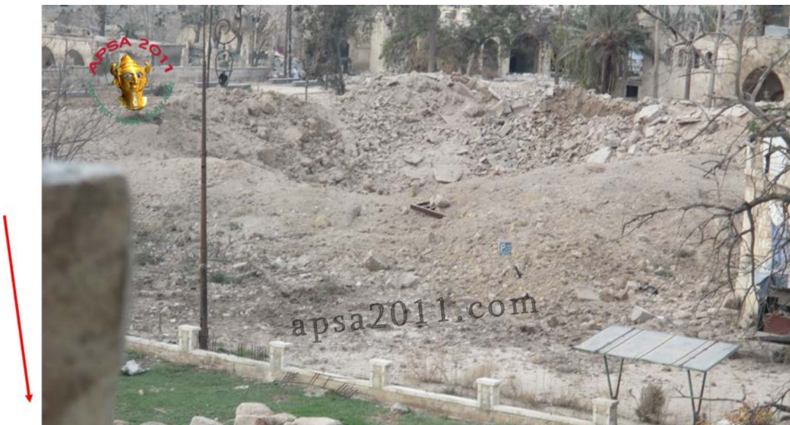
The remains of the Madrasa Sultaniyeh from the southeast looking northwest following the tunnel bombing of December 7, 2014.
