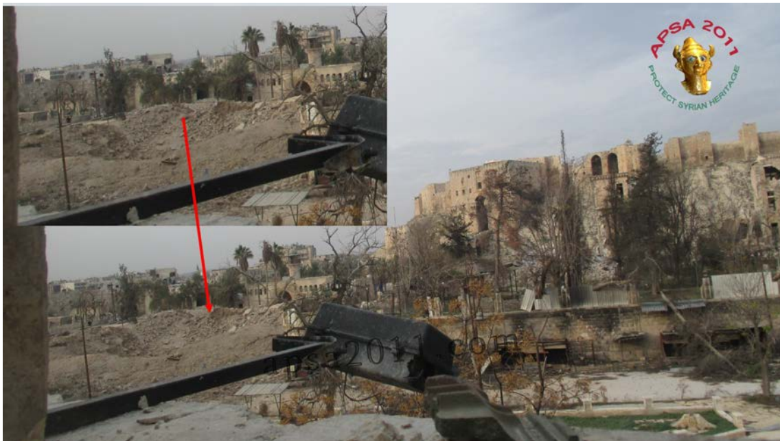
The remains of the Madrasa Sultaniyeh from the southeast looking northwest following the tunnel bombing of December 7, 2014.
