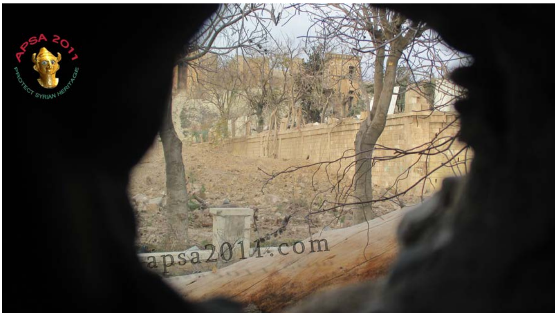
The remains of the Madrasa Sultaniyeh from the south following the tunnel bombing of December 7, 2014.
