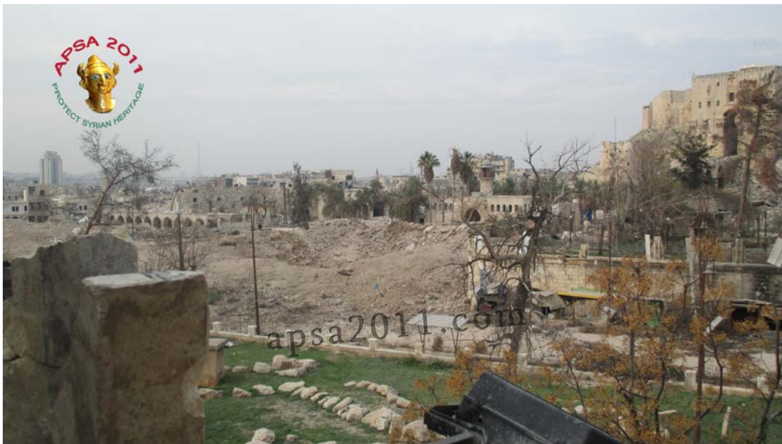
The remains of the Madrasa Sultaniyeh from the southeast looking northwest following the tunnel bombing of December 7, 2014.
