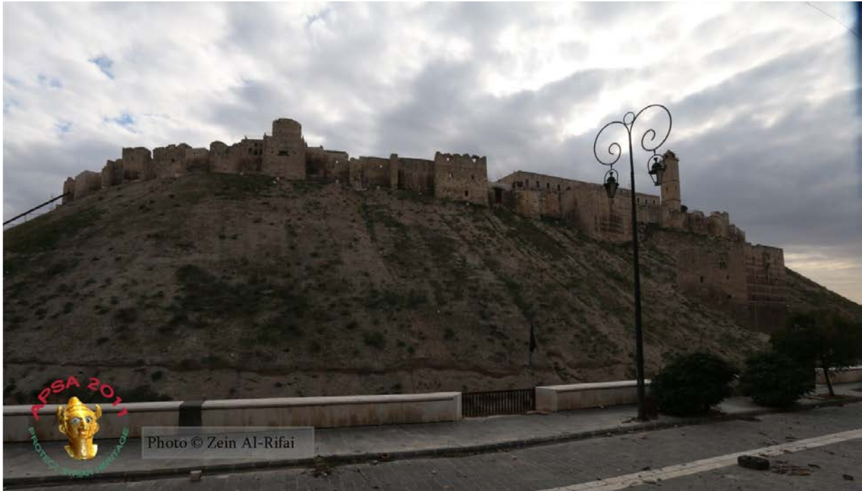
Image showing damage to the Aleppo Citadel (APSA).
