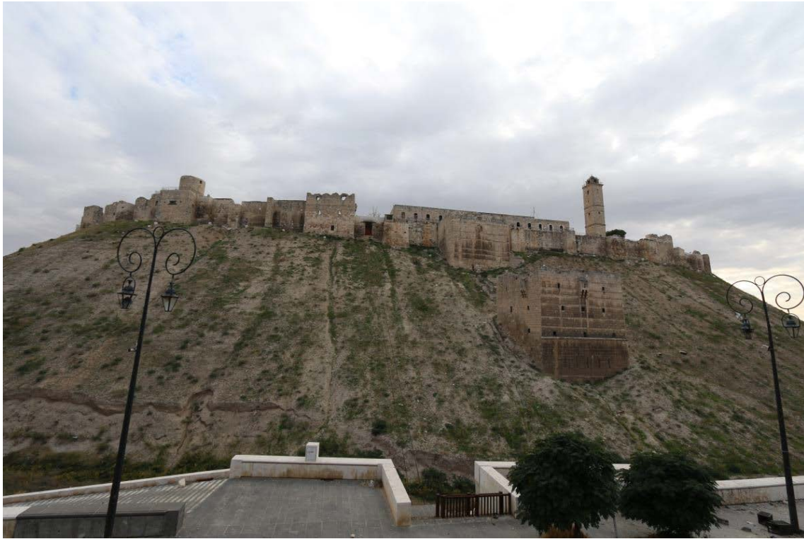
Image showing damage to the Aleppo Citadel (APSA).
