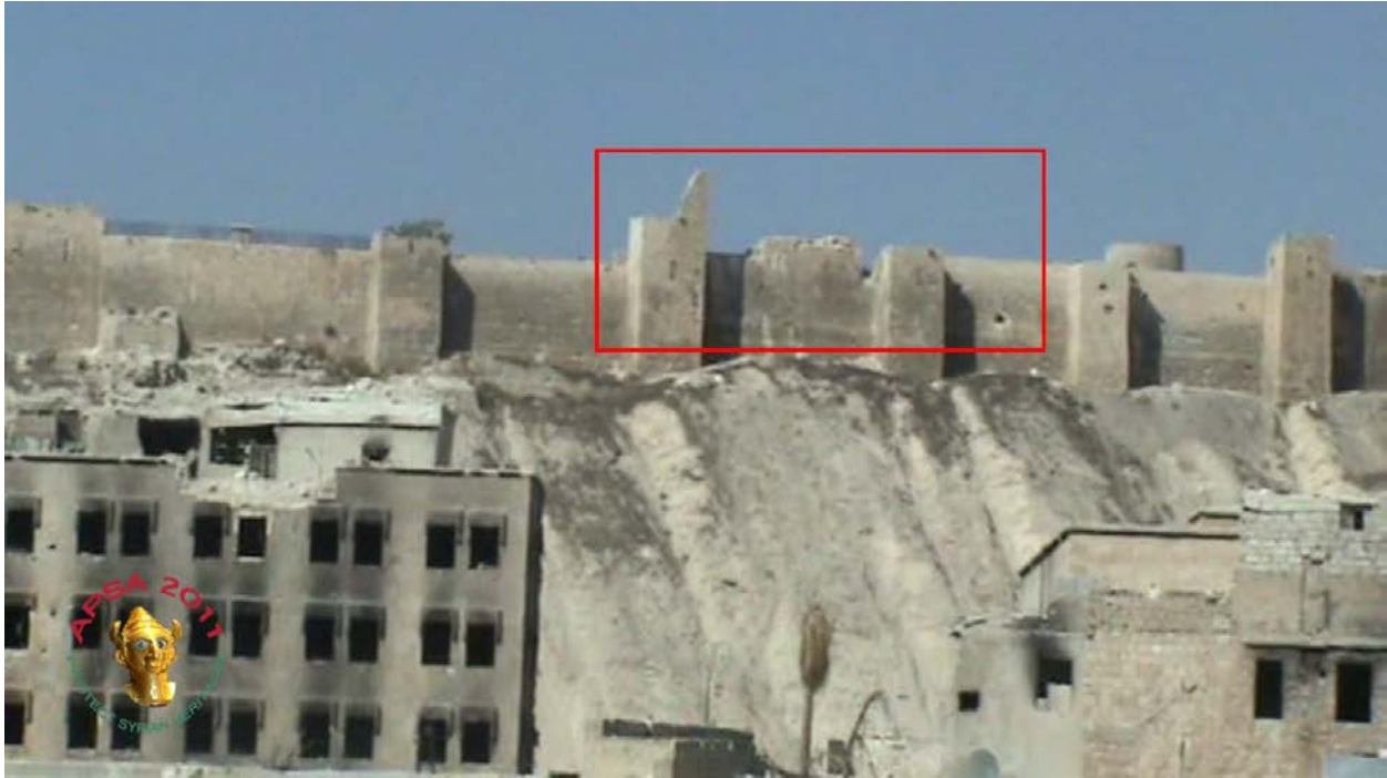
Image showing damage to the Aleppo Citadel (APSA).
