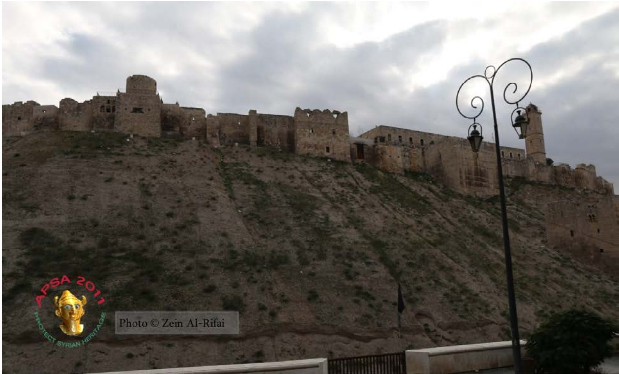
Image showing damage to the Aleppo Citadel (APSA).
