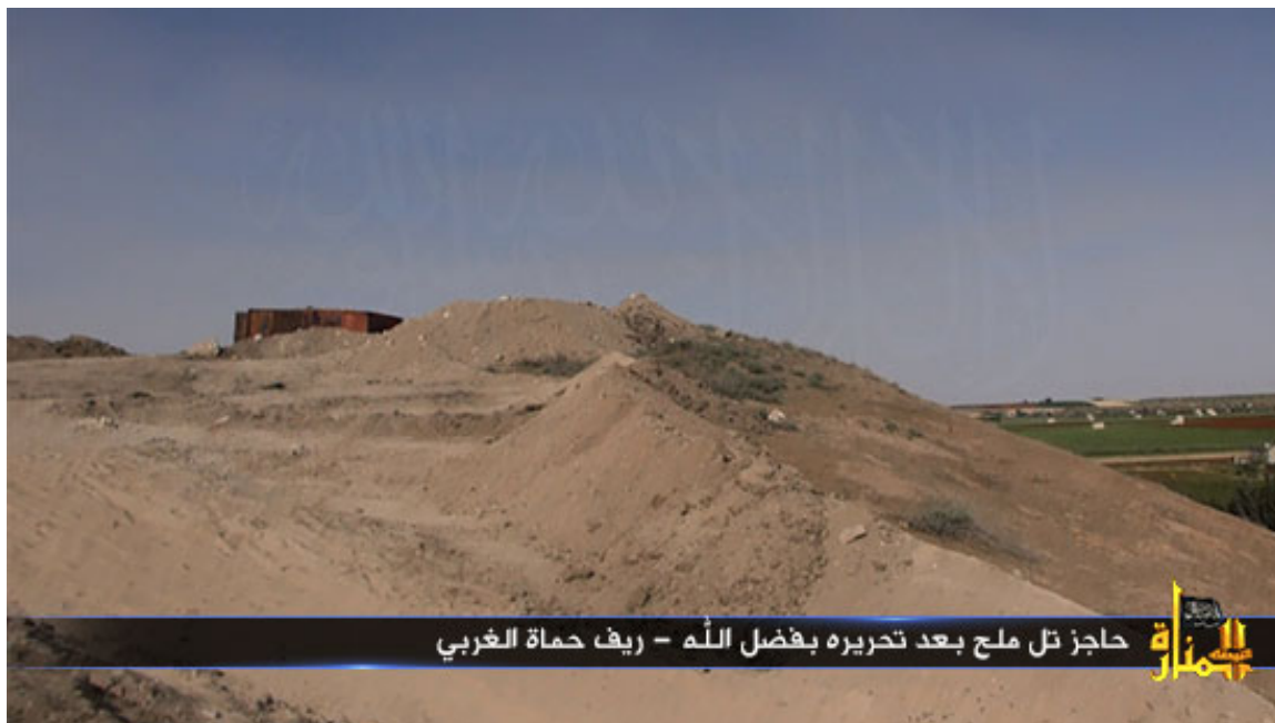
SARG earthworks on Tell Meleh (APSA).
