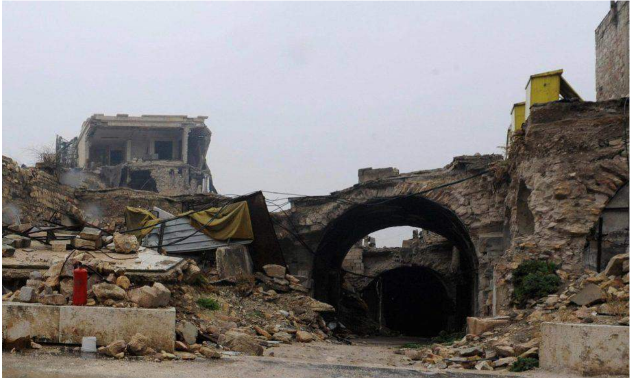
Severe damage to the entrance of Suq al-Zarb (Reuters; December 13, 2016)
