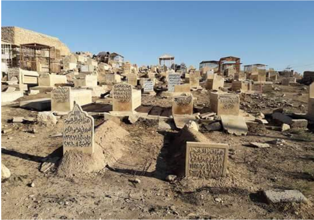
Intentional damage seen at a Yezidi Cemetery (Bashiqa and Bahzani News; December 5, 2016)
