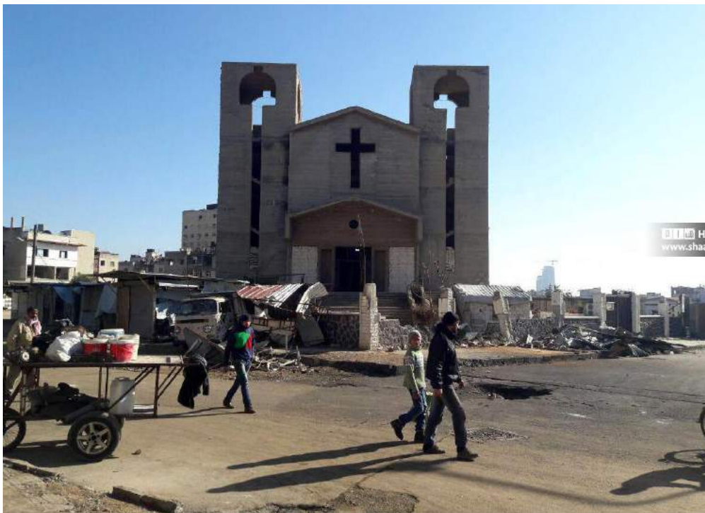
Damage outside the Greek Orthodox Church in al-Waer (Shaam News Network; October 6, 2016)
