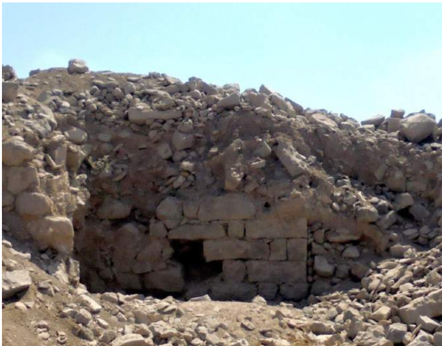
Wall of a building in the western side of Tell Ash'ari with a hole, possibly made by illegal excavation (DGAM; December 5, 2016)
