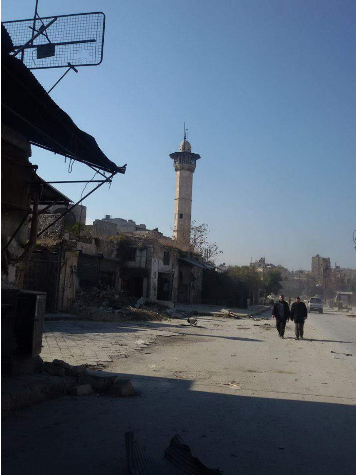
Damage surrounding Banqusa Mosque (Private Facebook Account; December 10, 2016)
