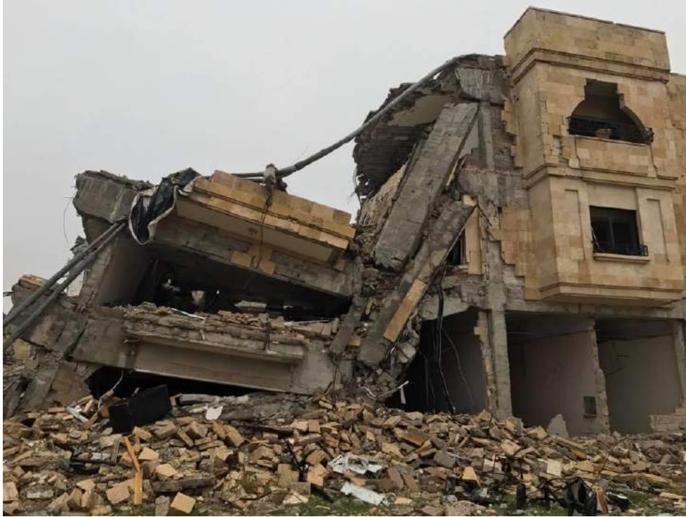
Collapsed wing of the Chamber of Industry (Faris Shihabi; December 13, 2016)
