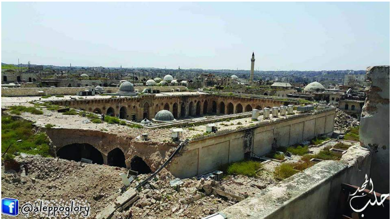
Severe damage to the Umayyad mosque showing missing minaret and extensive damage to the walls (Aleppo Glory حلب المجد/Facebook; December 10, 2016)
