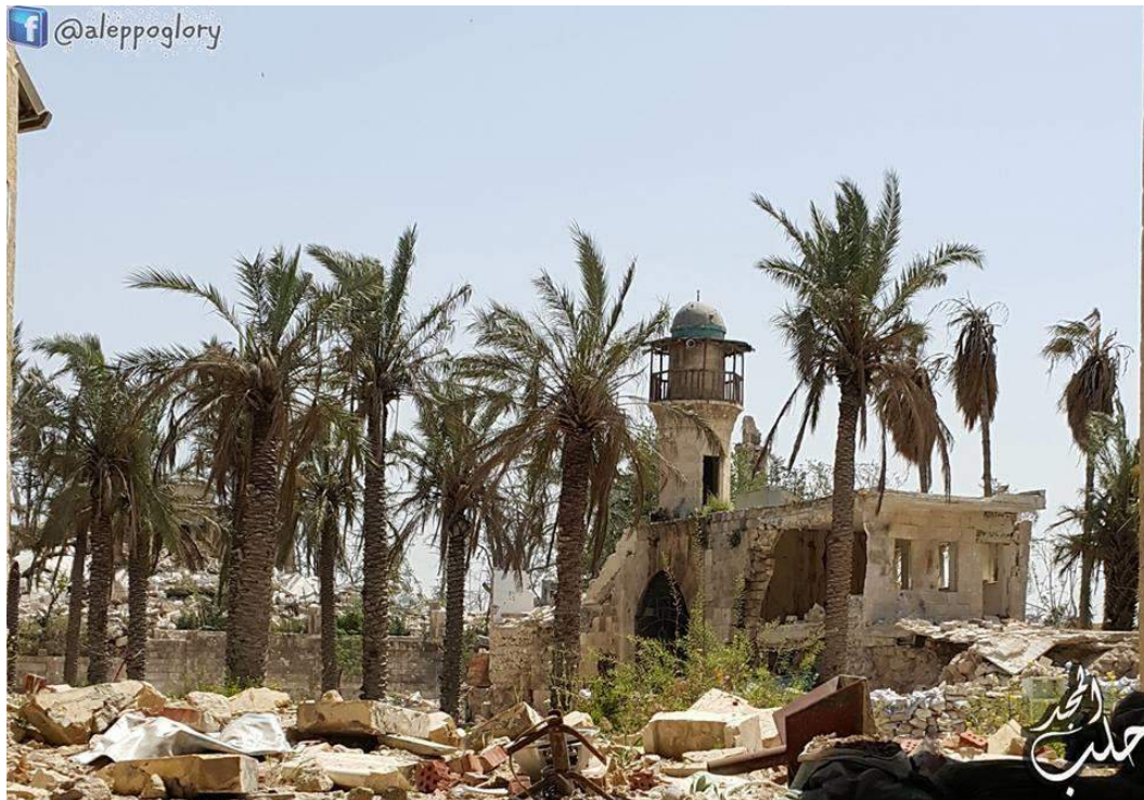
Severe damage to the Sultaniyah Madrasa showing only the far corner standing (Aleppo Glory حلب المجد/Facebook; December 10, 2016)
