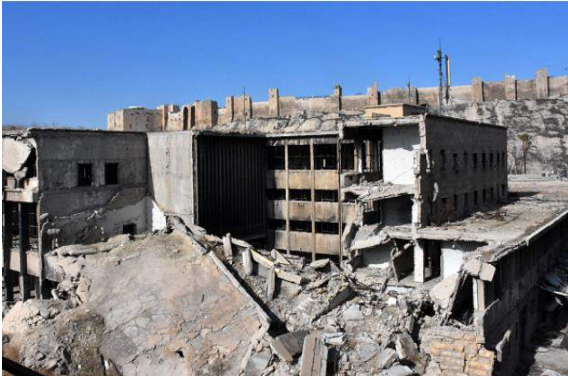
Damage to area south of the Aleppo Citadel (George Ourfalian/AFP; December 8, 2016)
