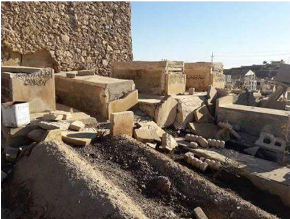
Intentional damage seen at a Yezidi Cemetery (Bashiqa and Bahzani News; December 5, 2016)
