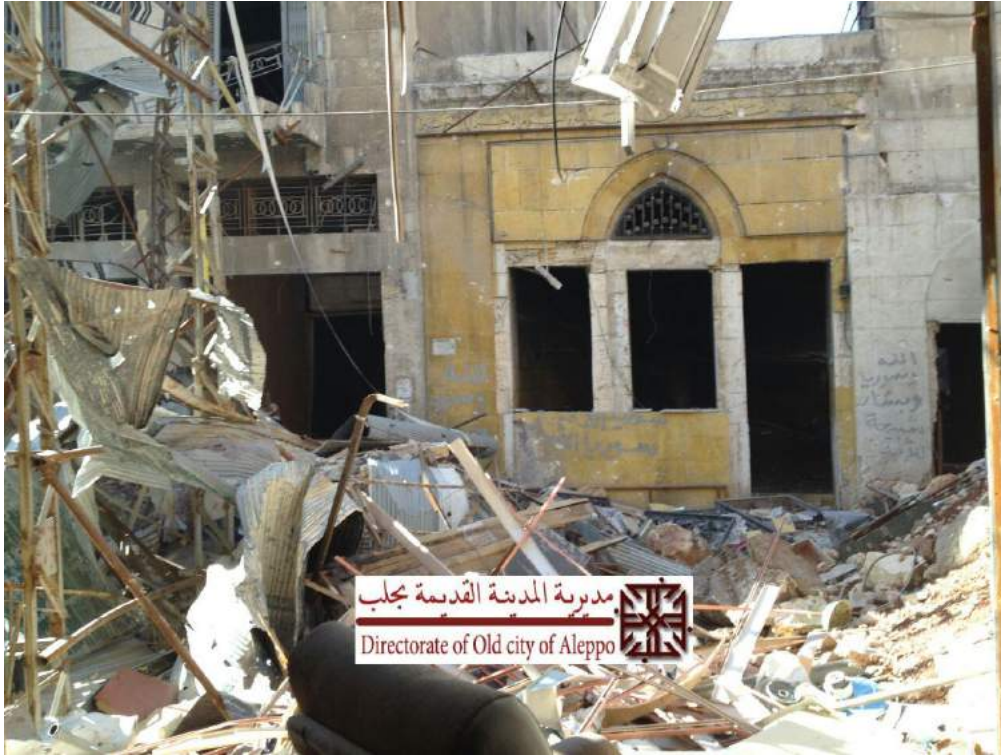
Severe damage to the Khan al-Harir (DGAM; December 12, 2016)
