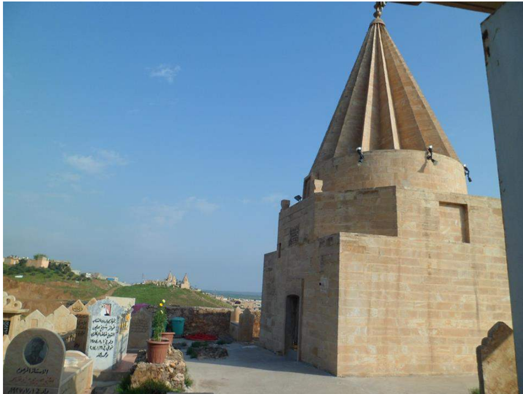
Sheikh Hassan Shrine prior to damage (Beloved Bahzani; July 8, 2014)
