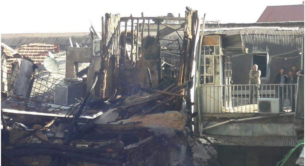
Fire damage in al-Hamidiyah Souq (DGAM; December 2, 2016)
