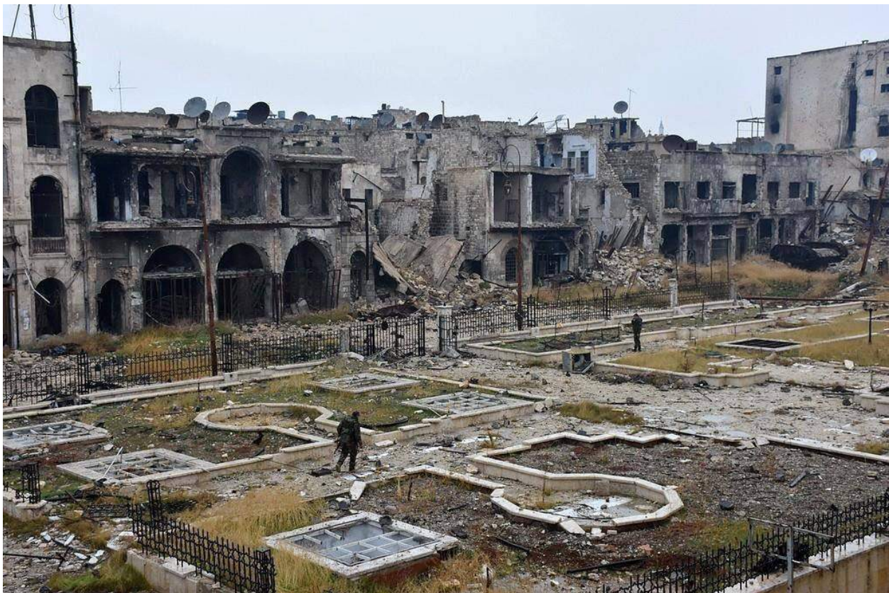
Severe damage to the area around the Umayyad Mosque (Khalid Masri; December 12, 2016)
