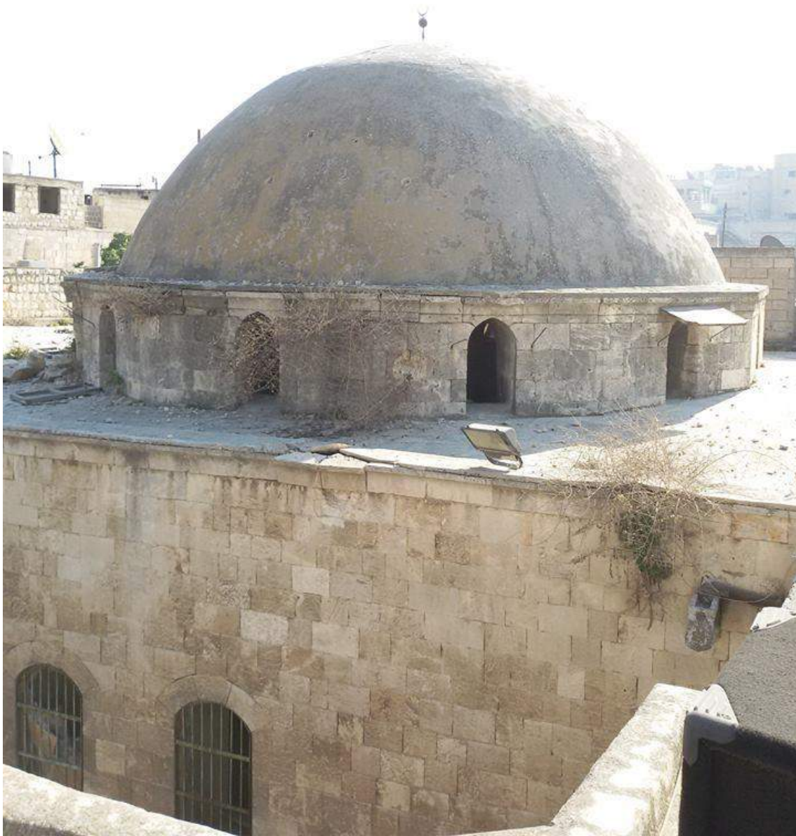
Overgrowth of vegetation on the dome of al-Sarawi Mosque (Private Facebook Account; December 10, 2016)
