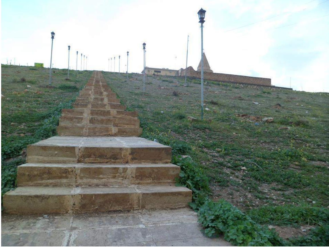
Sheikh Hassan Shrine prior to damage (Beloved Bahzani; March 15, 2014)
