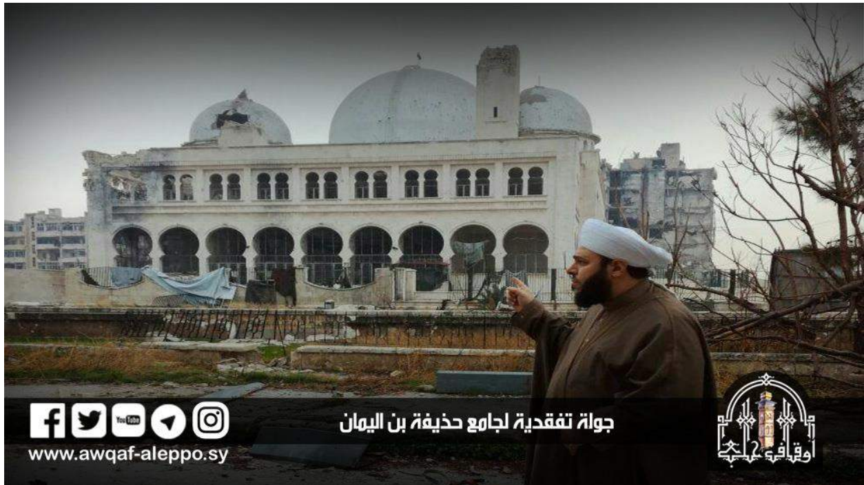
Damage to the exterior of Huzeifa ibn al-Yaman Mosque during an inspection (Awqaf Aleppo; December 13, 2016)
