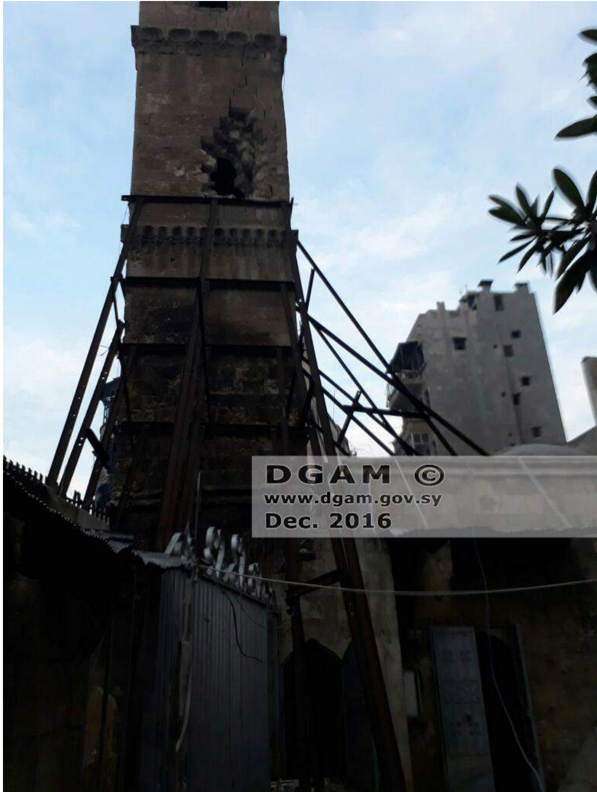
Damage to the minaret of Mosque Dabbagha al-'Atiqa, with a hole in the side and wooden supports (DGAM; December 10, 2016)
