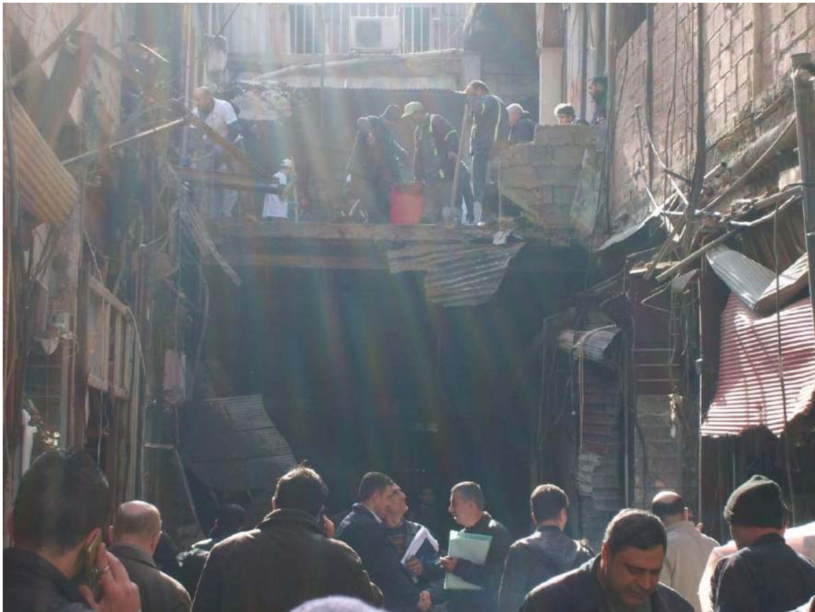
Fire damage in al-Hamidiyah Souq (DGAM; December 3, 2016)
