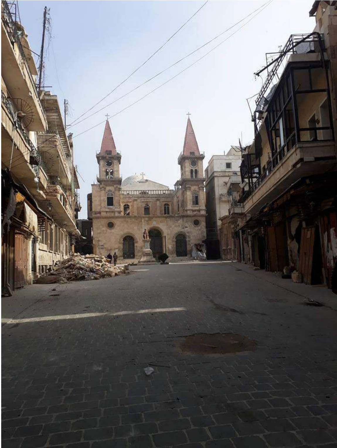
Minor damage to St. Elias Maronite Church showing missing glass panes and rubble in street (Khalid Masri; December 12, 2016)
