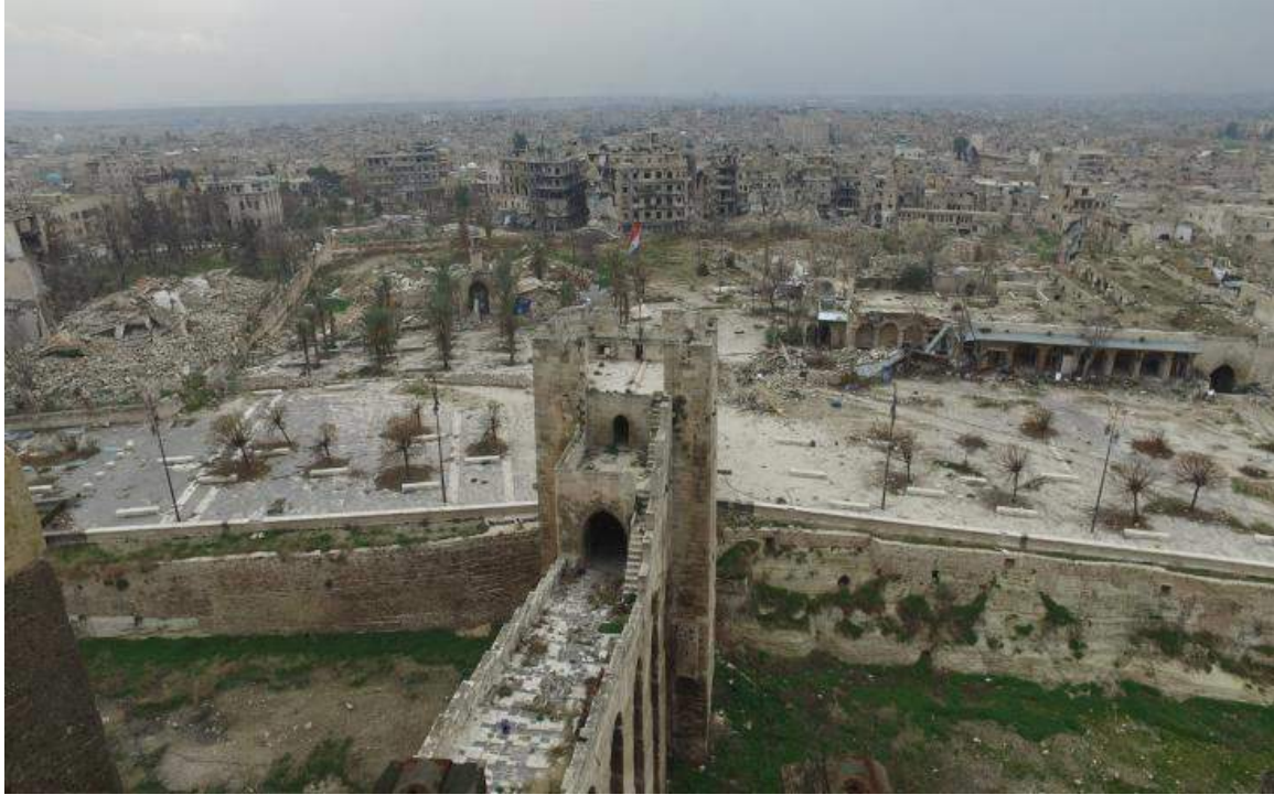
Damage to the causeway of the Aleppo Citadel (Aleppo Archaeology; December 12, 2016)
