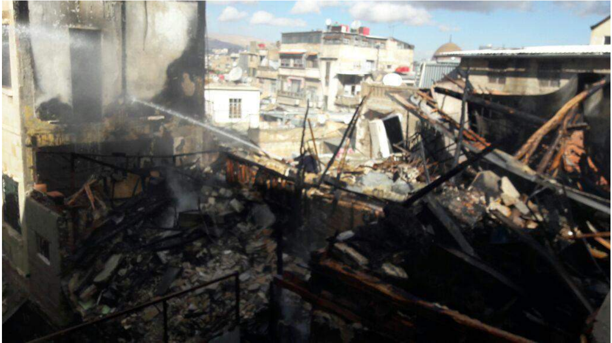
Fire damage in al-Hamidiyah Souq (DGAM; December 2, 2016)
