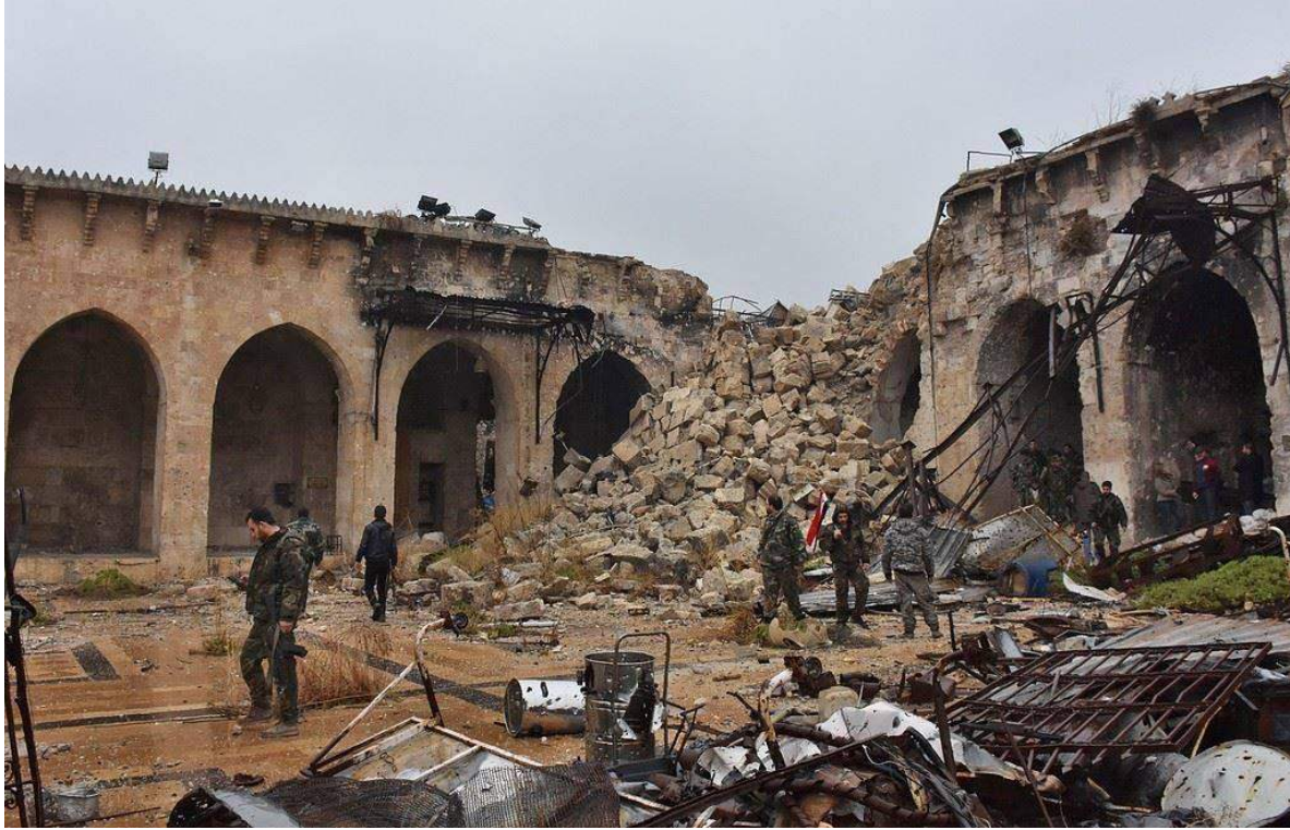
Severe damage to the Umayyad Mosque showing the missing minaret (Khalid Masri; December 12, 2016)
