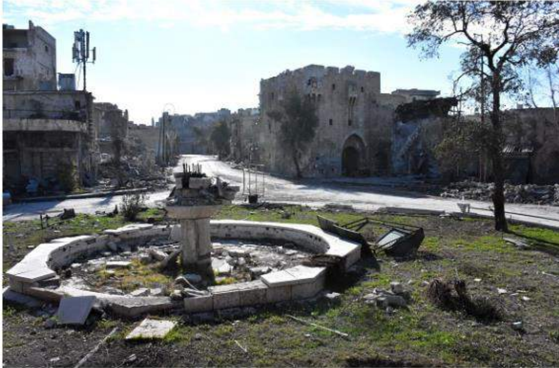
Damage to the Bab al-Hadid Neighborhood and Bab al-Hadid Gate (George Ourfalian/AFP; December 8, 2016)
