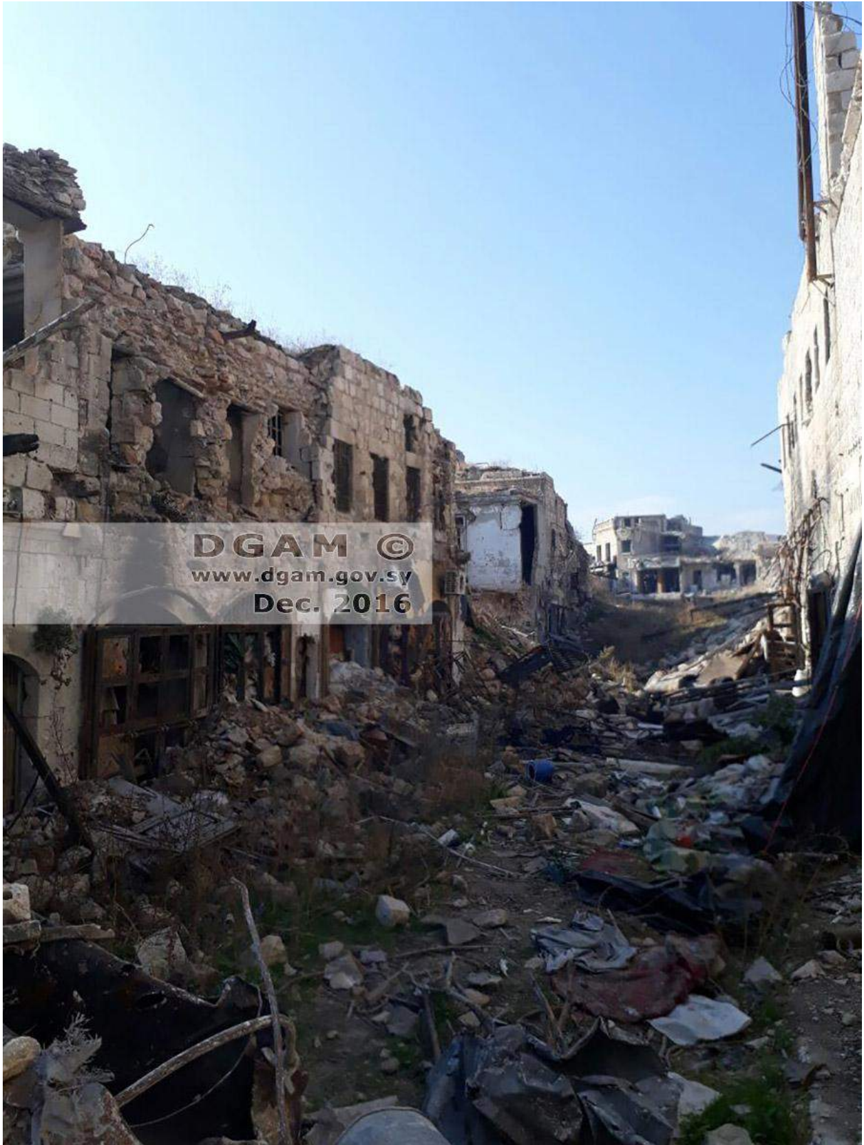
Severe damage to area surrounding al-Fadileh School (DGAM; December 9, 2016)
