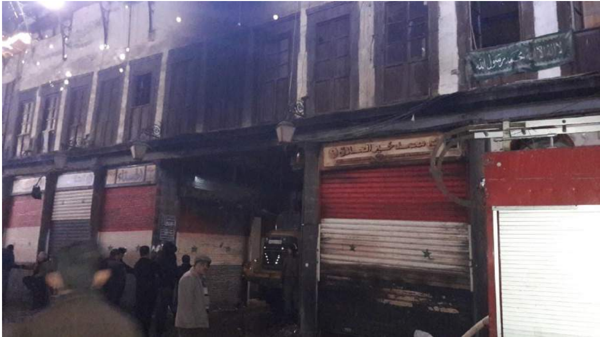
Fire damage to al-Tahan Avenue in al-Hamidiyah Souq (DGAM; December 3, 2016)
