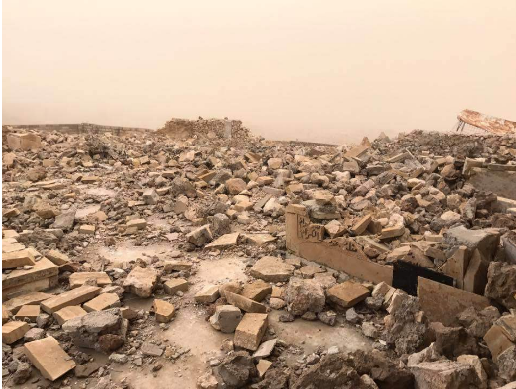
Damage seen to Sheikh Hassan Shrine (Bashiqa wa Bahzani; December 2, 2016)
