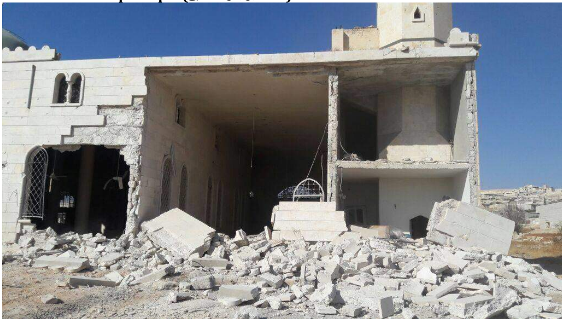
Damage to Abu Bakr al-Sadiq Mosque (SNHR; October 26, 2016)
