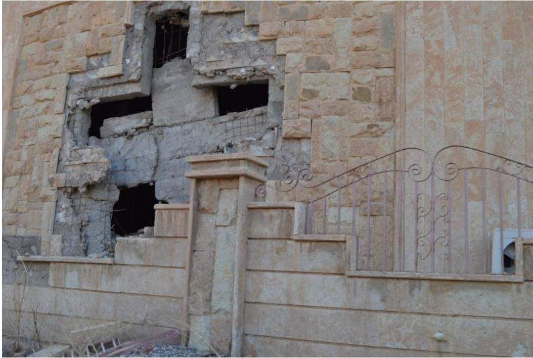
Damage to the Syriac Orthodox Cultural Center (Baretly.net; October 22, 2016)
