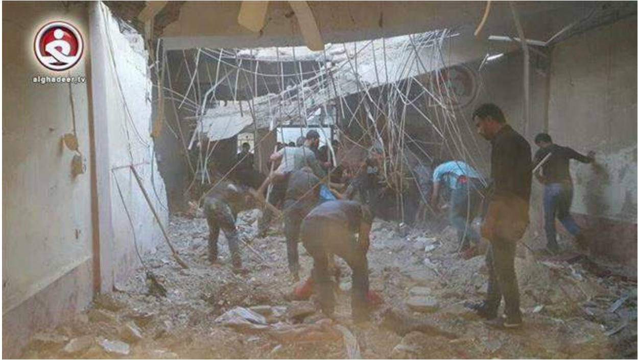
Damage inside al-Khanli Mosque following the airstrike (Iraqi al-Ghadeer/Press TV; October 21, 2016)
