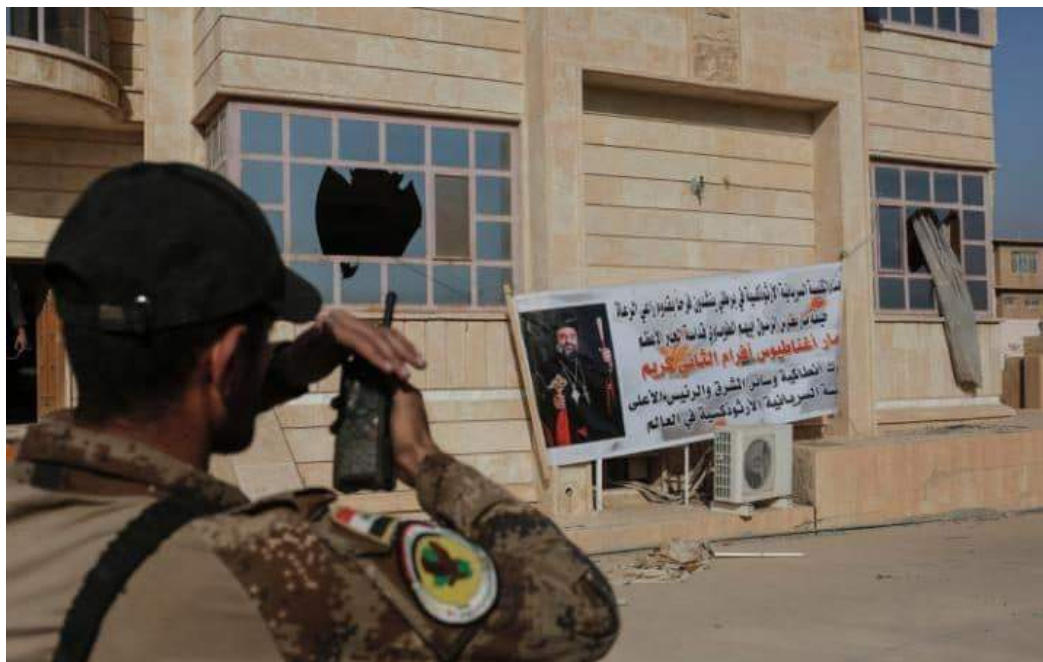
A view of the damaged Syriac Orthodox Cultural Center (Telegraph; October 22, 2016)
