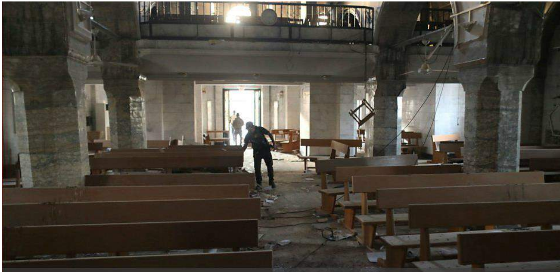
A soldier inspects the damage inside Mart Shmone Church (BBC/Reuters; October 23, 2016)
