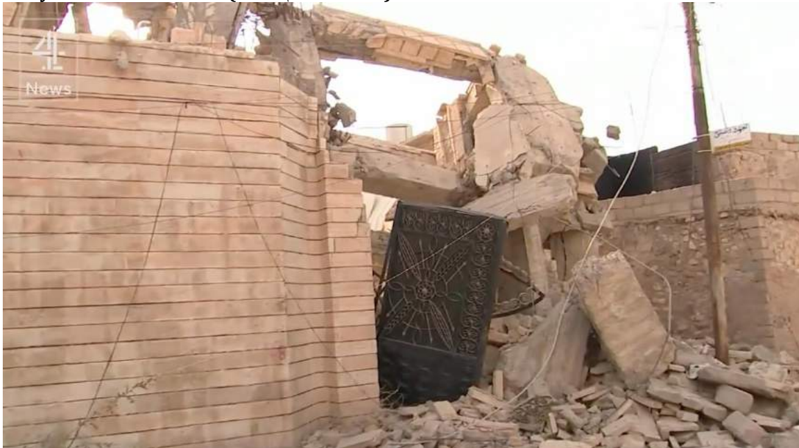
Video still of extensive damage to the exterior of Maryam al-Azra Church (Channel 4; October 23, 2016)
