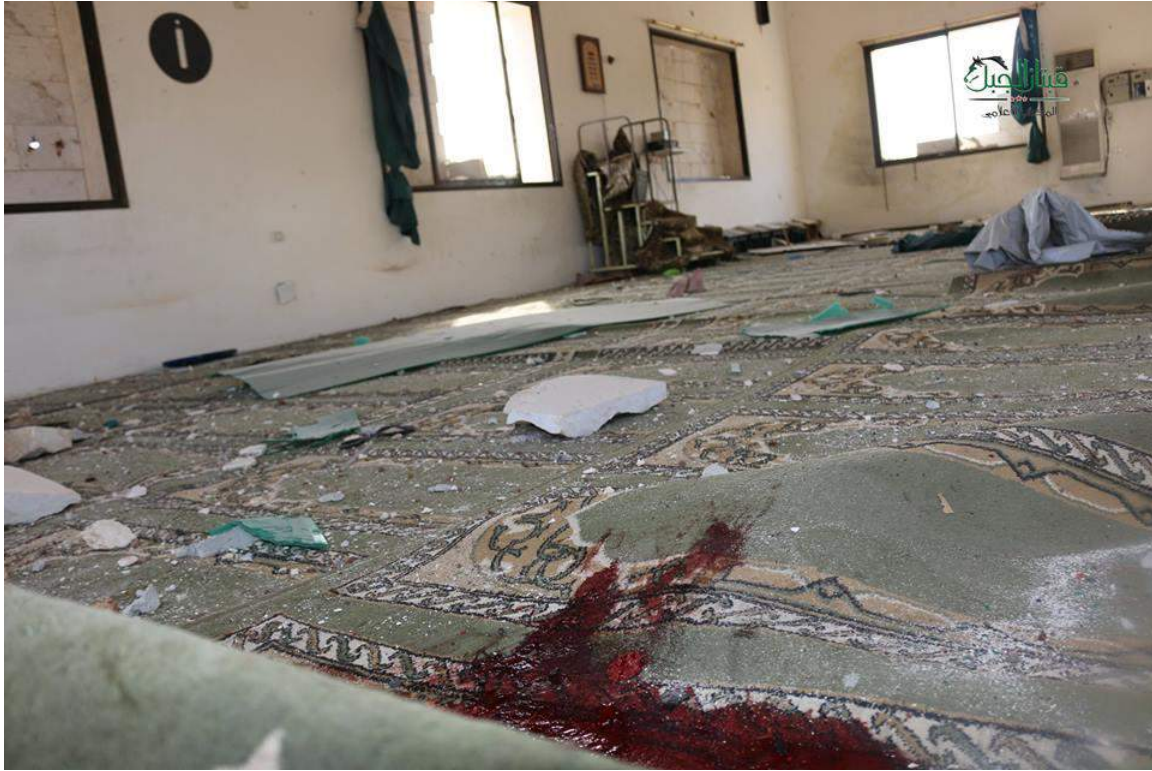
Damage to the interior of Qebtan Mosque (SNHR; October 25, 2016)
