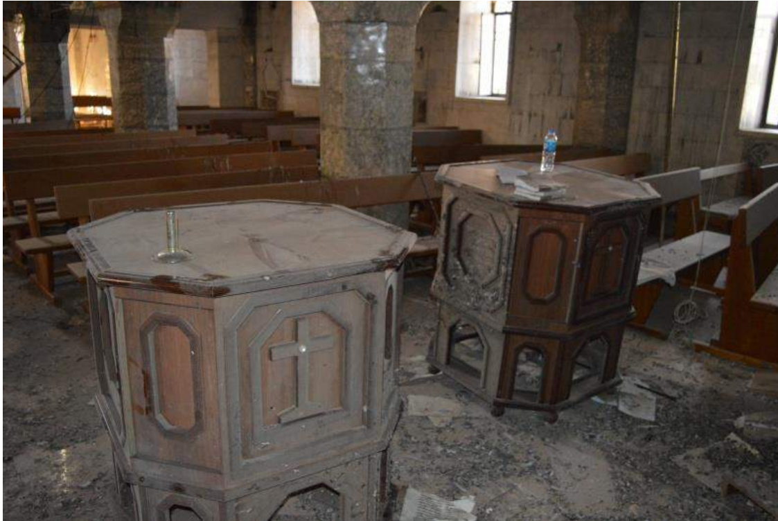
Severe damage to Mart Shmone Church (Barely.net; October 22, 2016)
