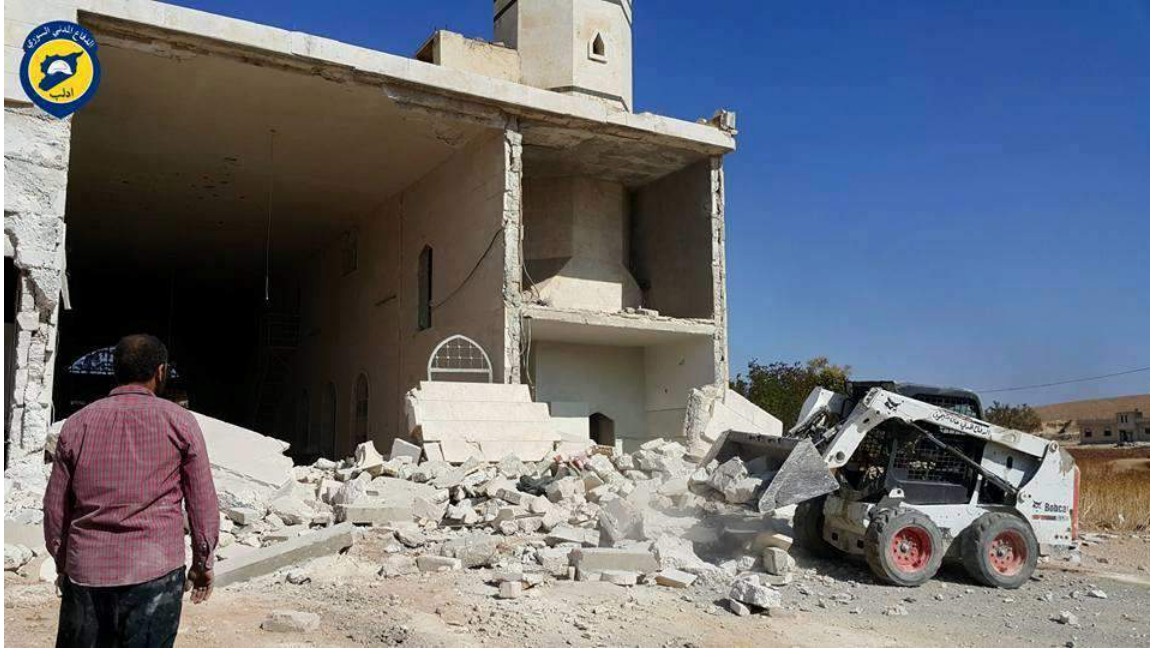
Damage to Abu Bakr al-Sadiq Mosque (The White Helmets; October 28, 2016)
