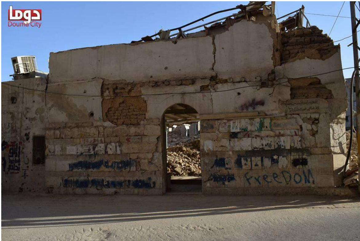
Damage to Zeen Musalla in Douma (Douma Revolution; October 17, 2016)
