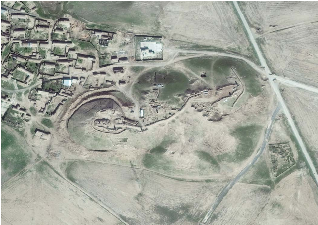
Satellite image of Mohammed Diyab (February 2014) showing the construction of a military garrison (Digital Globe®, Casana)
