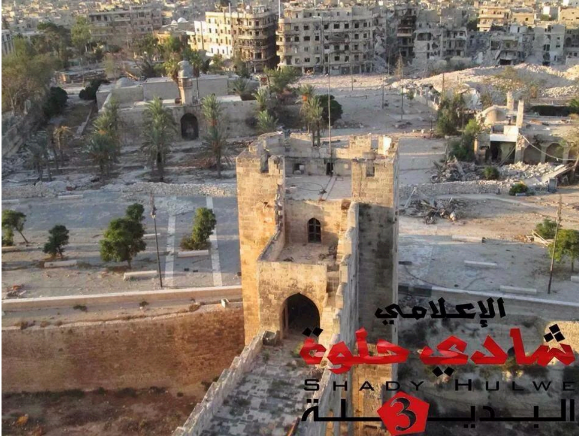
Madrasa Khusruwiye before and after the 2014 tunnel bombs. The structure has been completely destroyed (Shady Hulwe)
