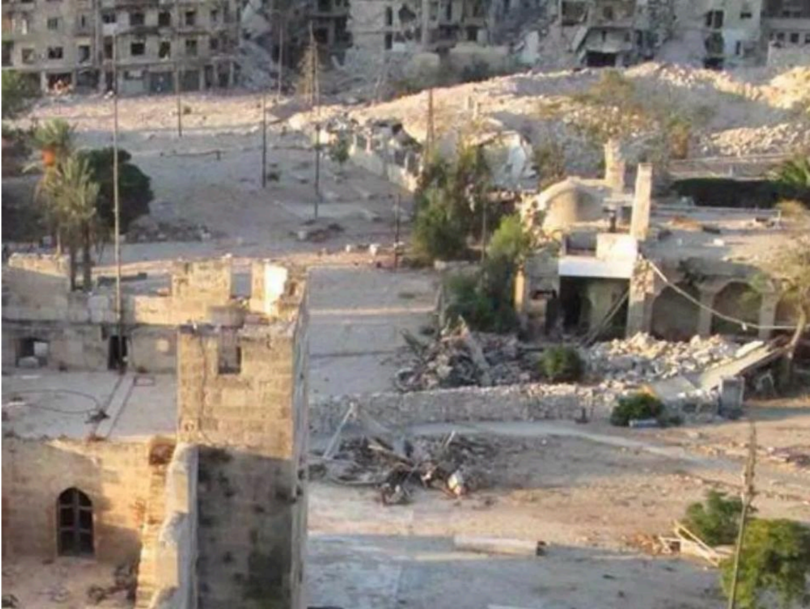
Madrasa Khusruwiye before and after the 2014 tunnel bombs. The structure has been completely destroyed (Shady Hulwe)
