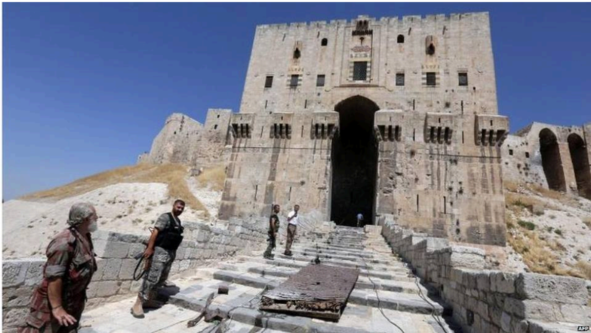
Image showing damage to the Citadel of Aleppo (APSA)
