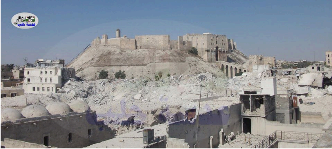
Image showing damage to the Citadel of Aleppo (APSA)
