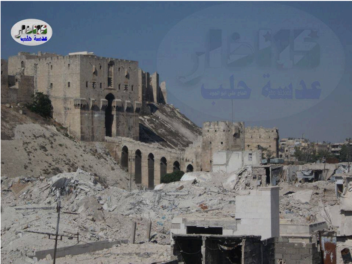
Image showing damage to the Citadel of Aleppo (APSA)
