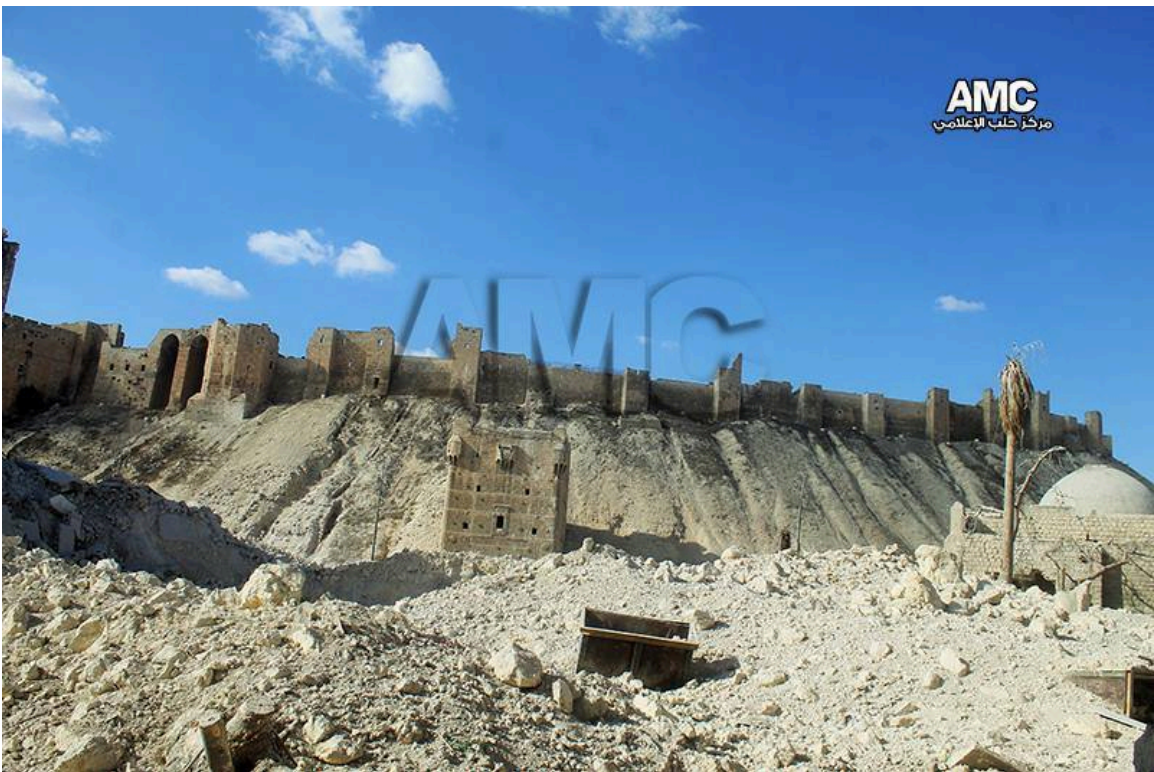
Image showing damage to the Citadel of Aleppo (APSA)
