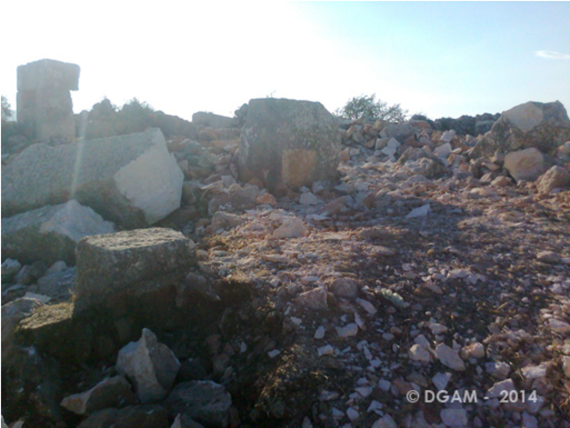
Photograph showing large ancient stones at St. Simeon Castle that have been broken for building material (DGAM).
