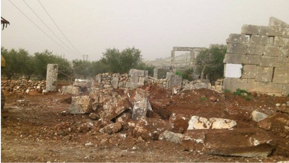
Photograph of the St. Samaan Monastery showing ancient stones broken by bulldozer (DGAM).
