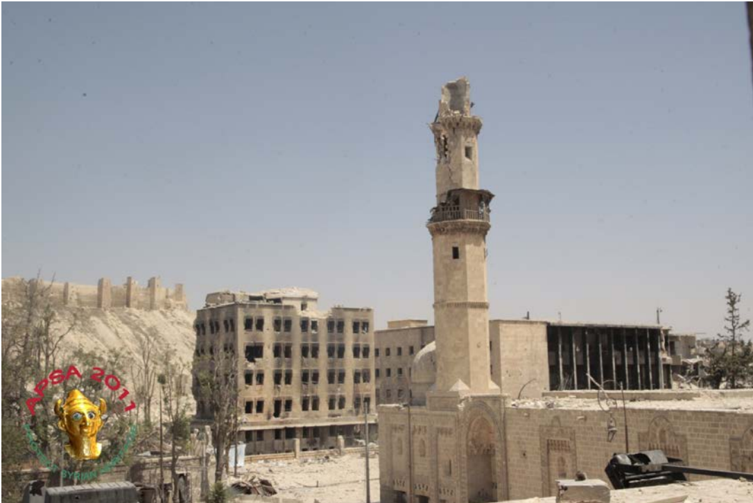
Damage to the al-Otrush Mosque (APSA).
