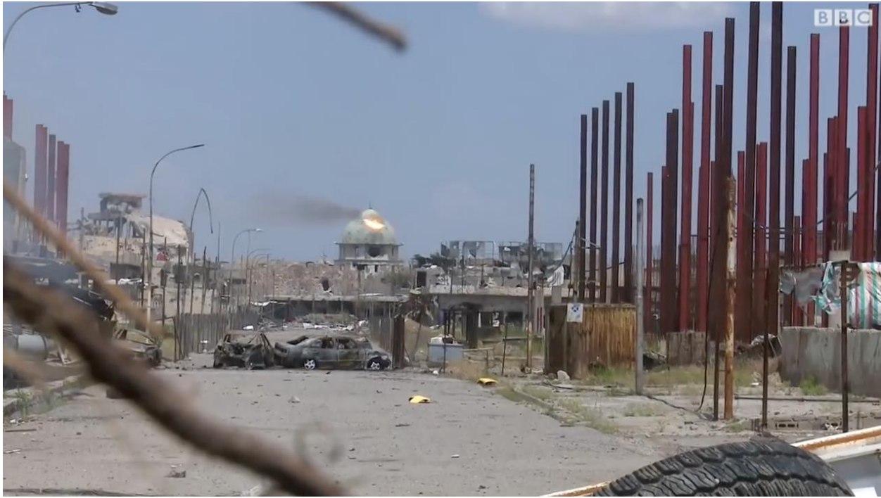
Video still of al-Nuri al-Kabir Mosque at the time of the RPG impact (BBC Arabic; May 5, 2017)
