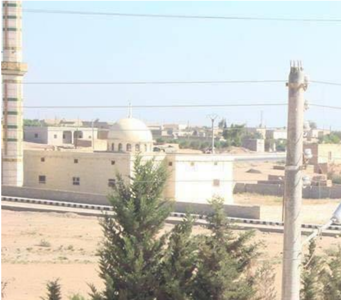
Hamada al-A'lowi Mosque prior to damage (RBSS; May 3, 2017)
