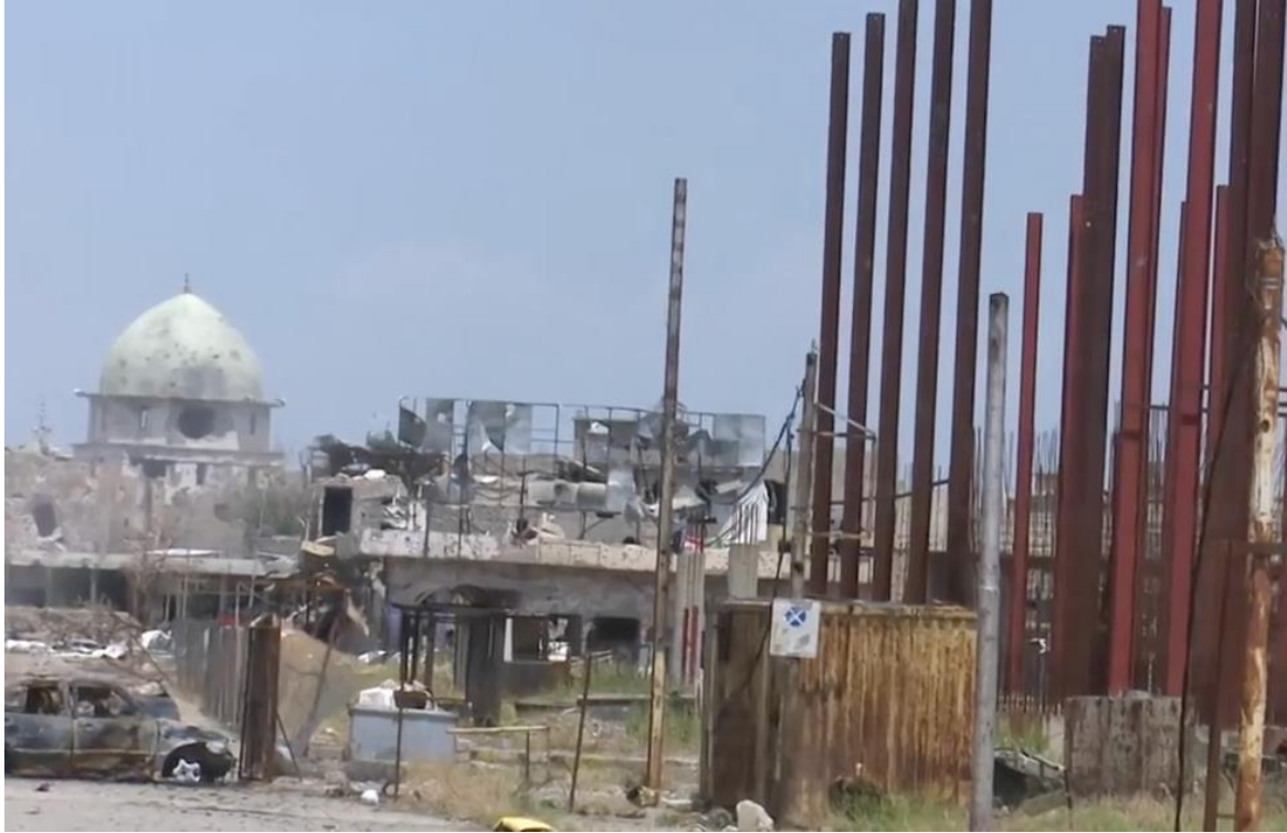
Video still of al-Nuri al-Kabir Mosque from the vantage point of ISF members, showing damage to the dome (BBC Arabic; May 5, 2017)
