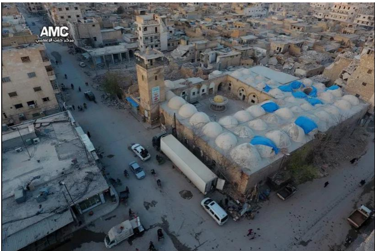
Damage to al-Kabir Mosque (APSA; May 8, 2017)
