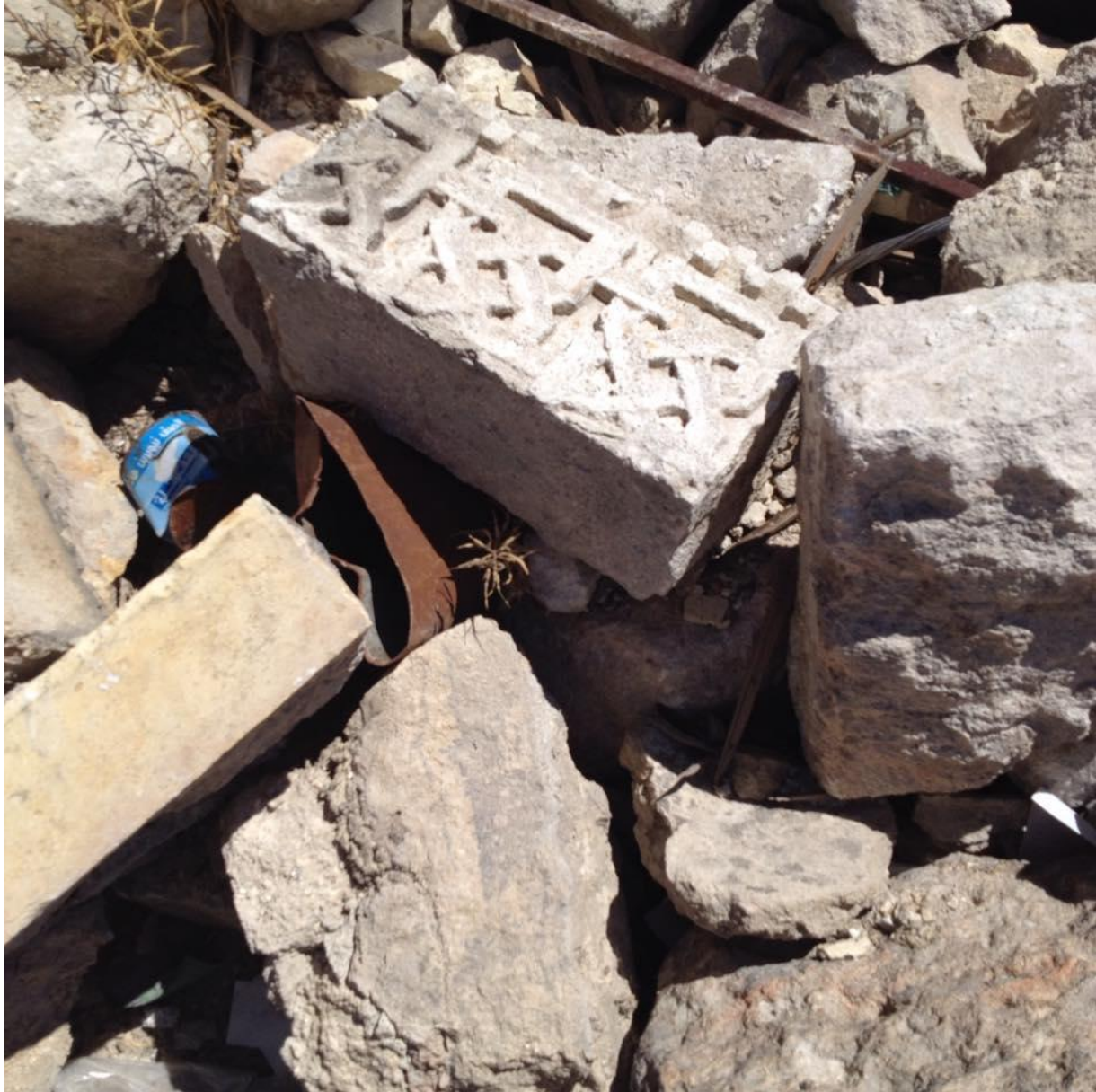
Part of the facade amidst other rubble from gate (Private Facebook Account; May 21, 2017)
