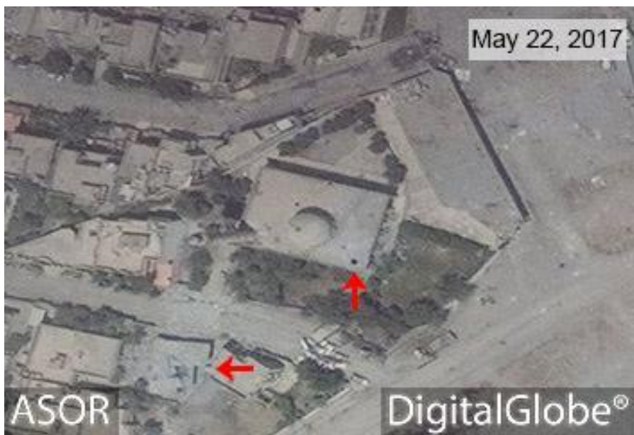
al-Shahid Muhammed Mosque with damage to the roof (DigitalGlobe; May 22, 2017)
