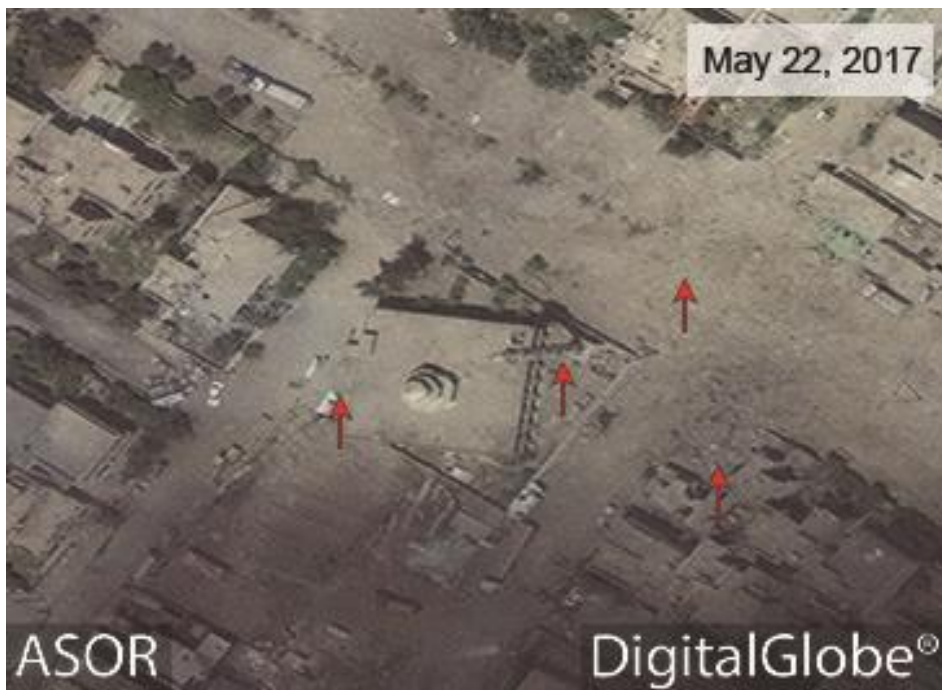
Damage to the mosque visible on the minaret and western side as well as the street and adjacent building (DigitalGlobe; May 22, 2017)
