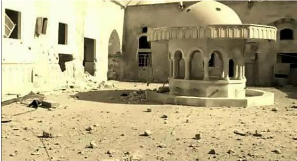
Damage to al-Kabir Mosque (APSA; May 8, 2017)
