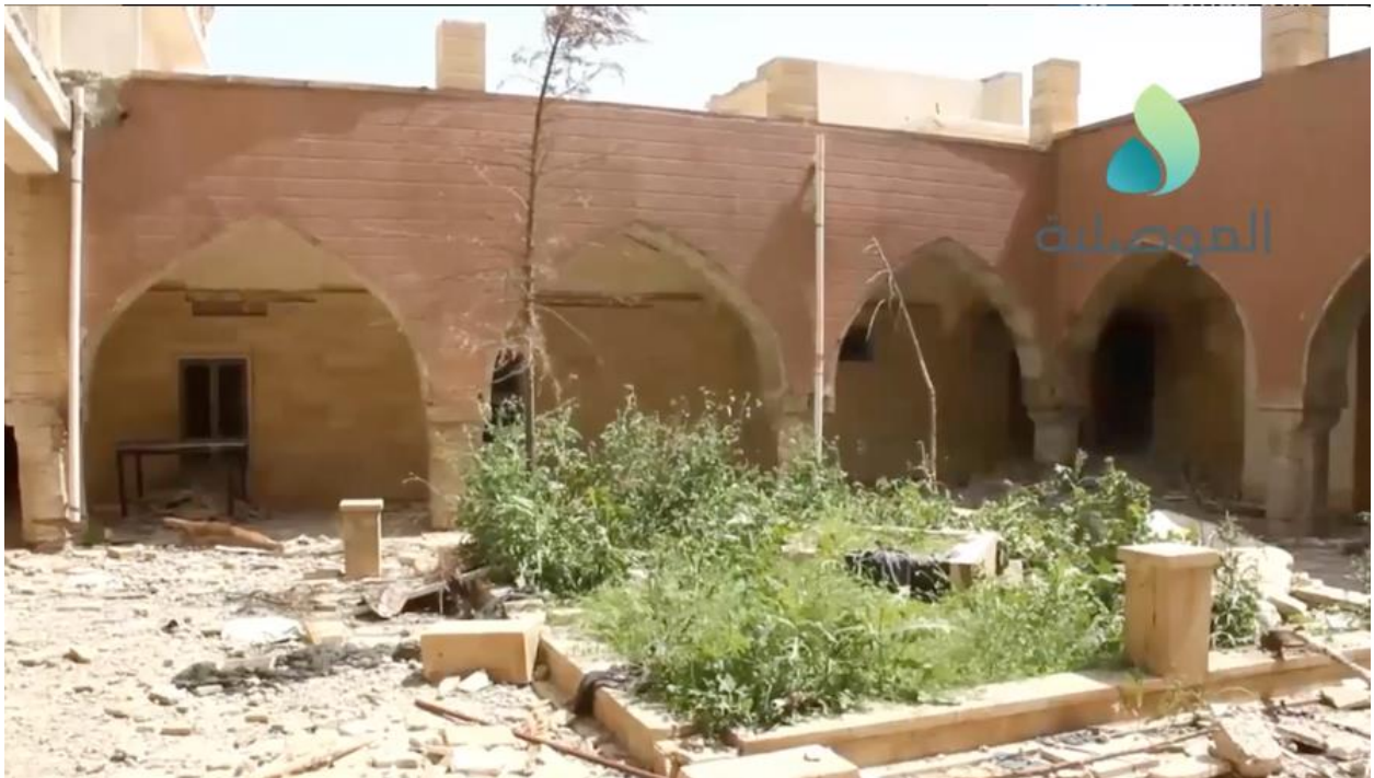
Video still of extensive damage at Mar Gorgis Monastery (al-Mosuliya; May 1, 2017)
