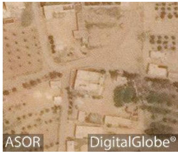
al-Orwa al-Wothqa Mosque prior to damage (DigitalGlobe; April 12, 2017)
