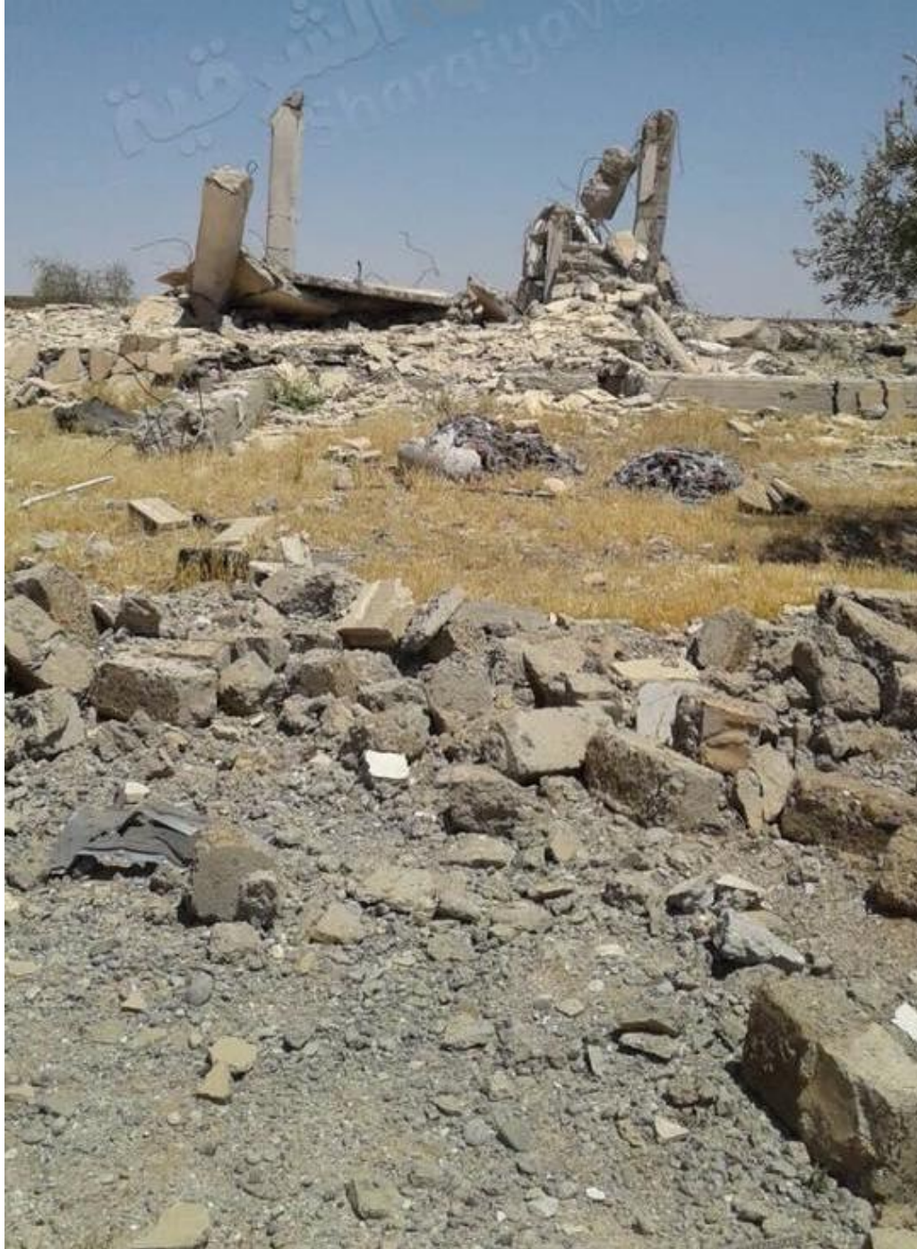
The destruction of the Bayyoud Village Mosque (Sharqiya Voice; May 19, 2017)
