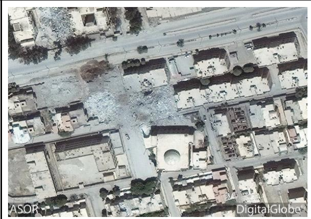
Post damage to the area with the mosque still appearing intact (DigitalGlobe; May 30, 2017)
