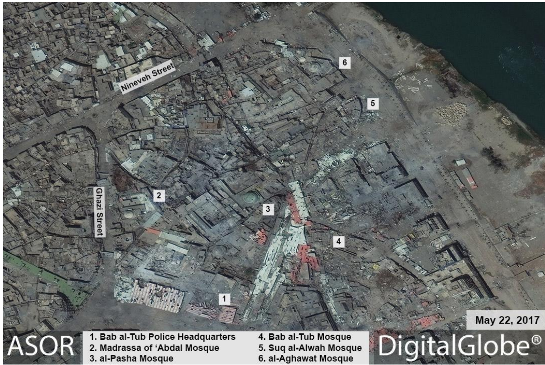
Additional damage and deterioration of the area with new damage to the al-Pasha Mosque (3) (DigitalGlobe; May 22, 2017)
