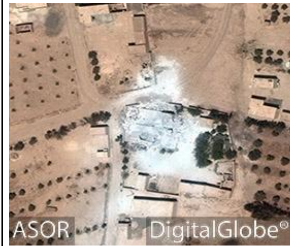
al-Orwa al-Wothqa Mosque severely damaged (DigitalGlobe; May 17, 2017)
