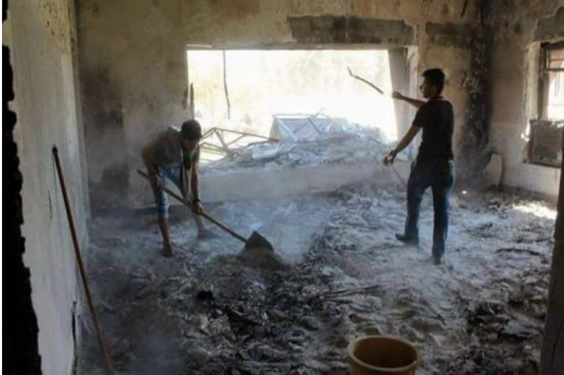
Volunteers cleaning up a building at Mosul University (France 24; April 17, 2017)
