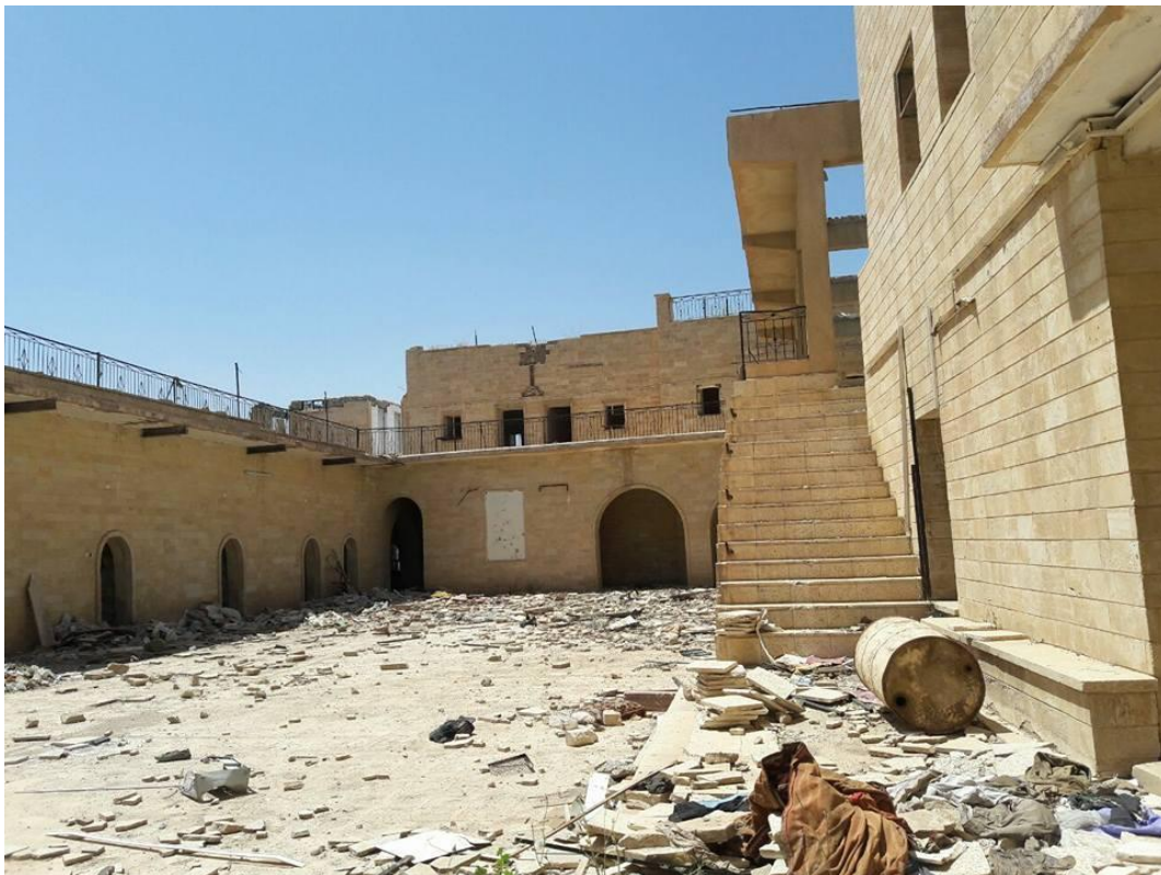
Damage seen to Mar Gorgis Monastery (Shlama Foundation; May 9, 2017)
