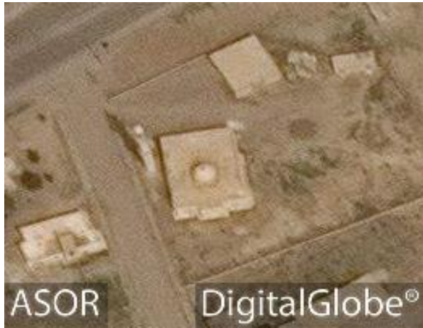
Hamada al-Al'ouwi Mosque prior to damage (DigitalGlobe; April 12, 2017)
