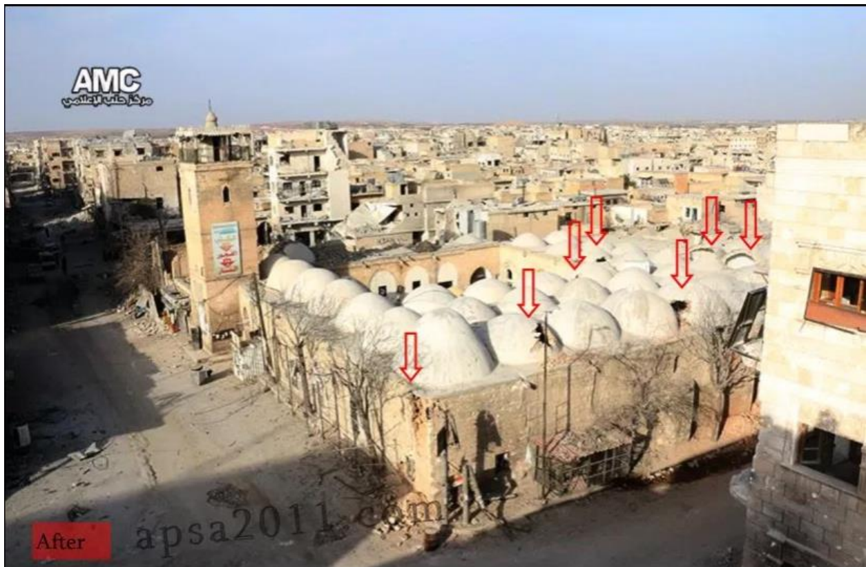
Damage to al-Kabir Mosque (APSA; May 8, 2017)
