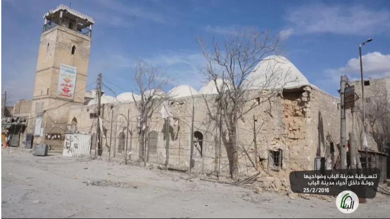
Exterior damage to al-Kabir Mosque (APSA; May 8, 2017)
