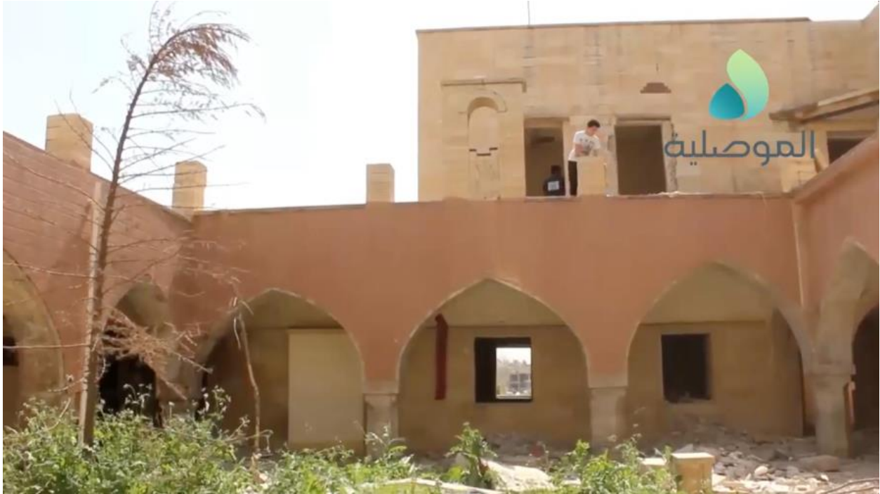
Video still of extensive damage at Mar Gorgis Monastery (al-Mosuliya; May 1, 2017)
