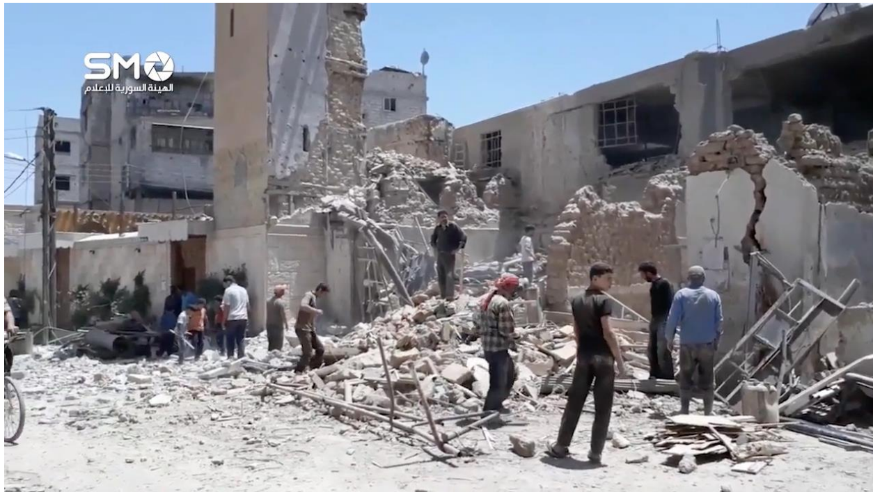
Video still of damage to Hamouriya Grand Mosque (SNHR; May 19, 2017)
