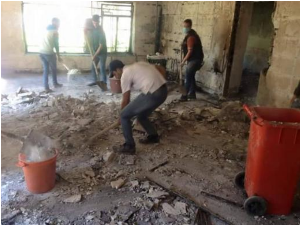
Volunteers cleaning up a building at Mosul University (France 24; April 17, 2017)
