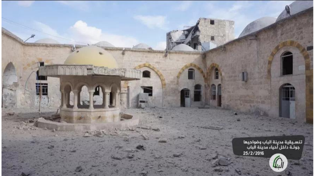
Damage to al-Kabir Mosque (APSA; May 8, 2017)
