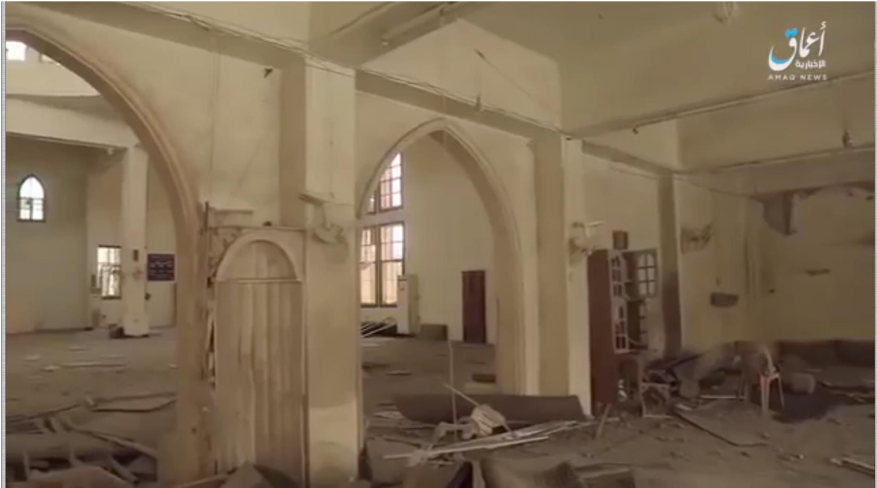
Video still showing damage to the interior of the mosque showing slight cracks in back wall, as well as rubble on floor (Amaq News Agency; May 28, 2017)
