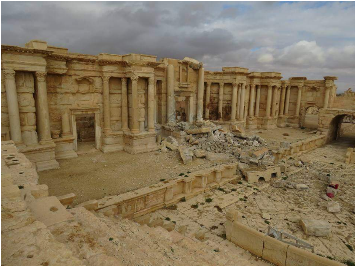
Damage to the front and stage of the theater (Private Twitter Account; March 2, 2017)
