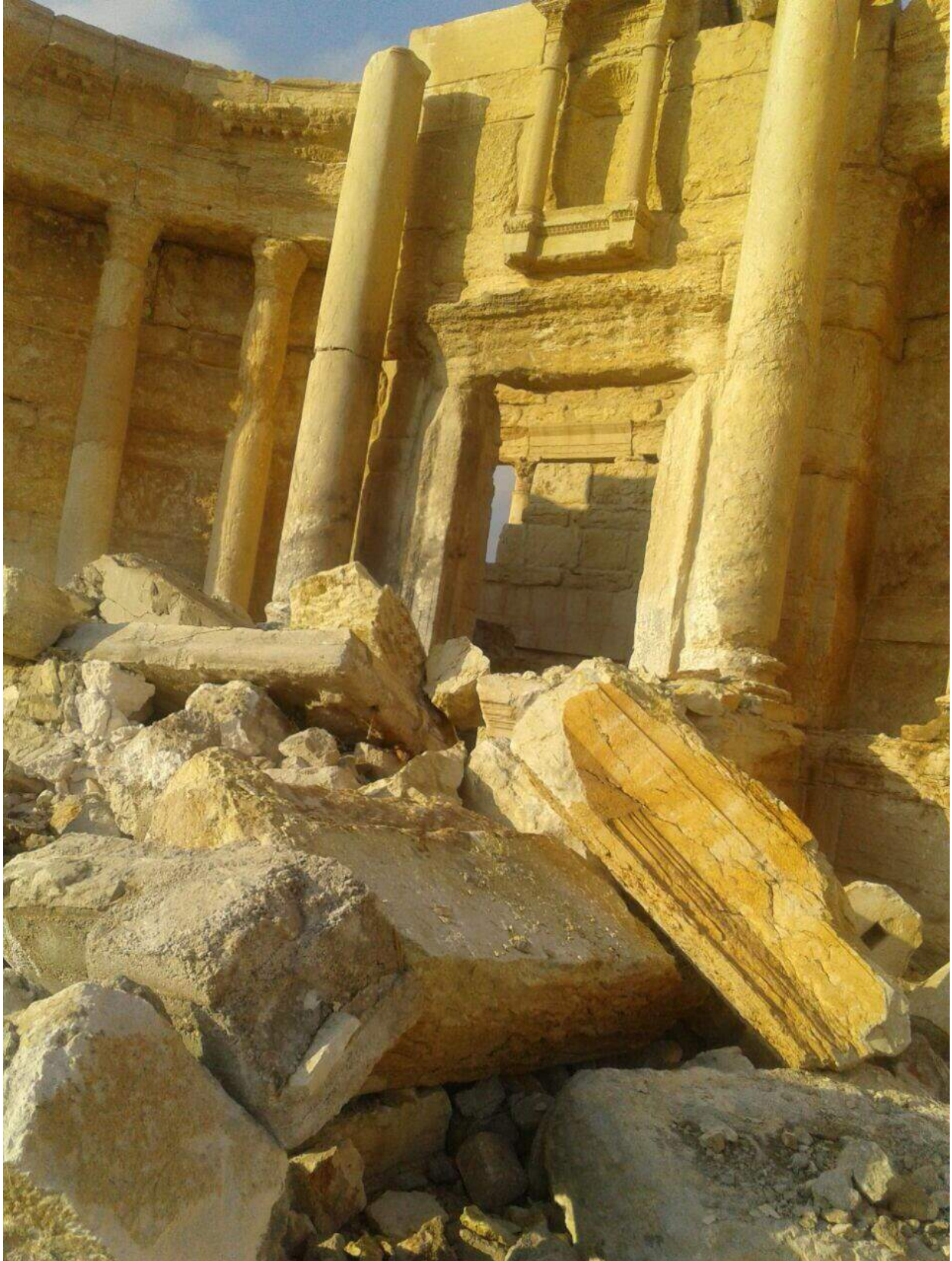
Detail of damage to front of stage (DGAM; March 2, 2017)
