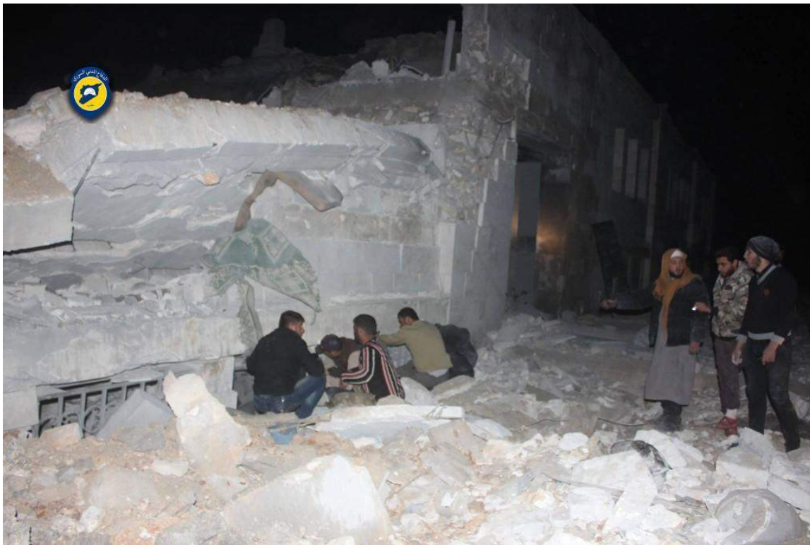
Damage seen to the mosque (SRC; March 16, 2017)
