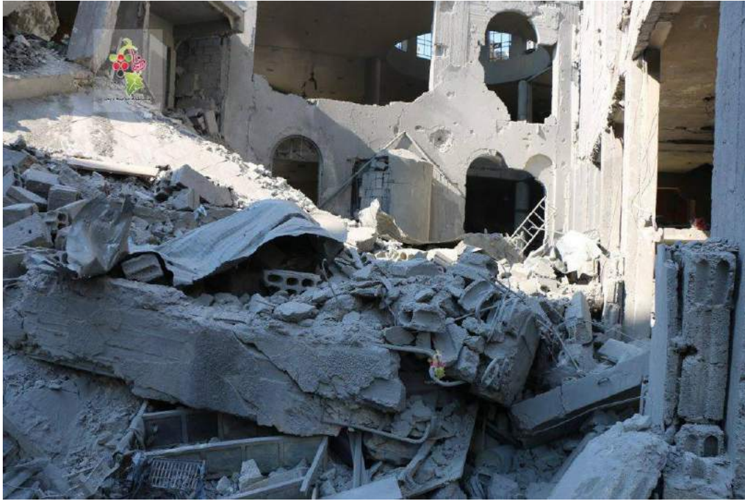
Damage to al-Rawda mosque from airstrikes on March 25, 2017 (SNHR; April 13, 2017)
