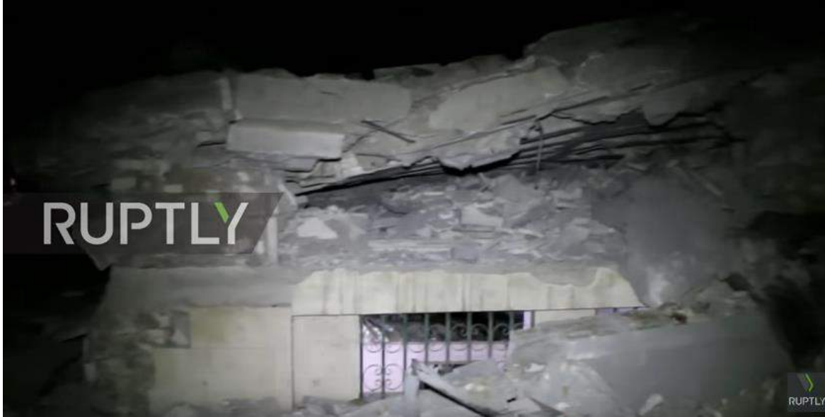
A video still shows what appears to be the leveling of the second floor of the mosque compound (Ruptly TV; March 17, 2017)
