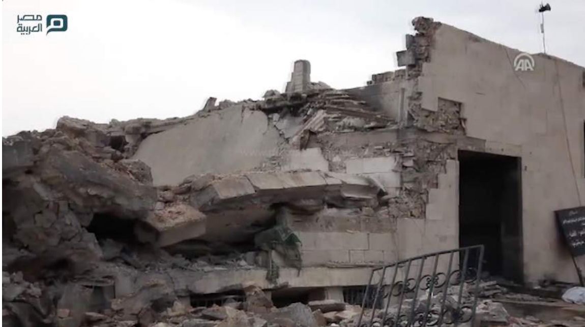
Video still shows damage to the mosque compound (Masr Alarabia; March 18, 2017)
