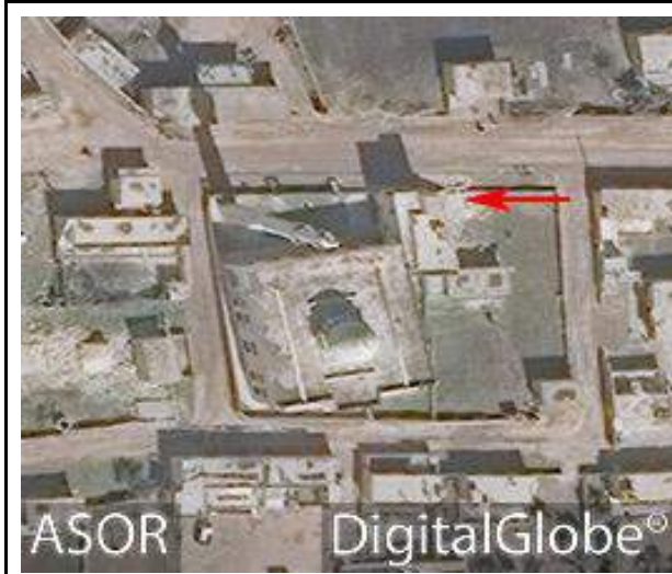
Mosque with prior damage to building and wall on the northeast (DigitalGlobe; February 15, 2017)
