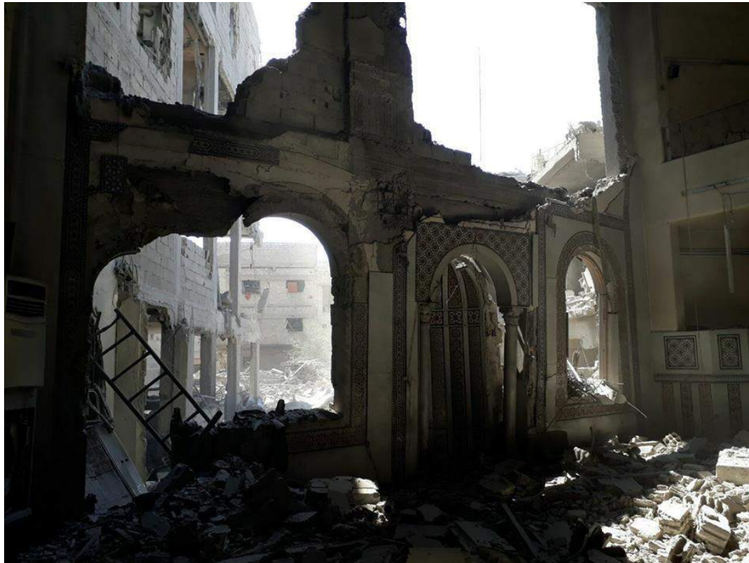
Damage to al-Rawda mosque from airstrikes on March 25, 2017 (SNHR; March 25, 2017)
