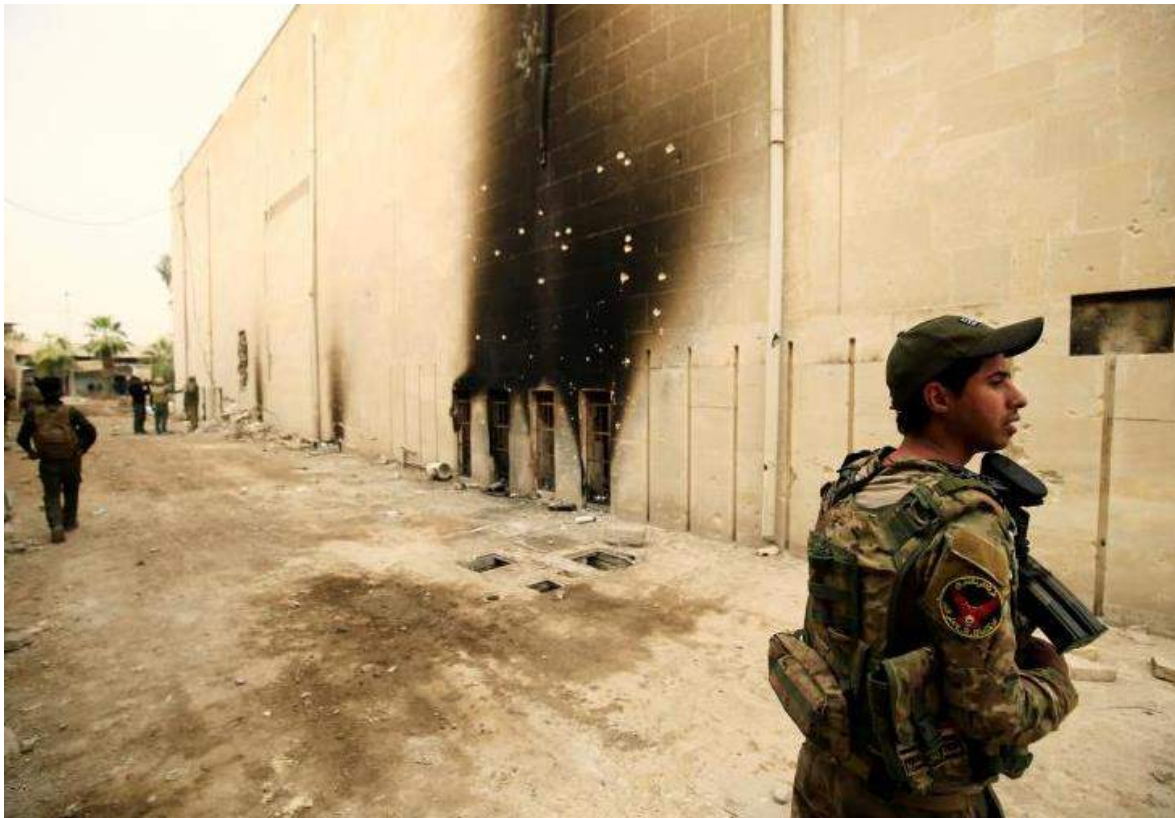
Fire damage to exterior of the Mosul Museum (Reuters; March 13, 2017)
