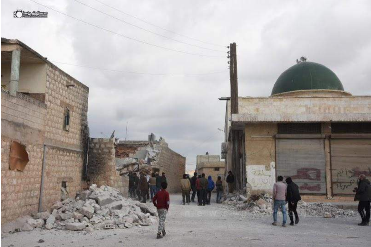
Damage near al-Kabir Mosque (SNHR; April 13, 2017)
