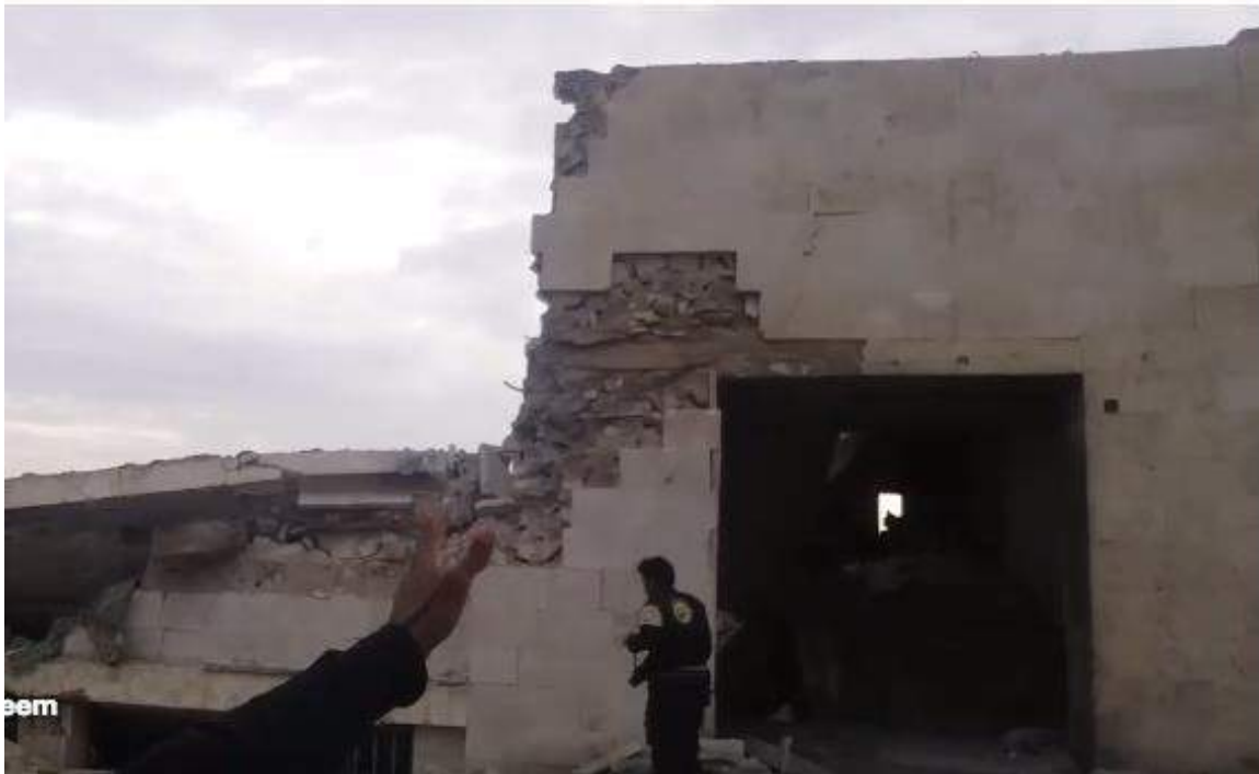
Video still of damage to the mosque compound (OGN TV; March 17, 2017)
