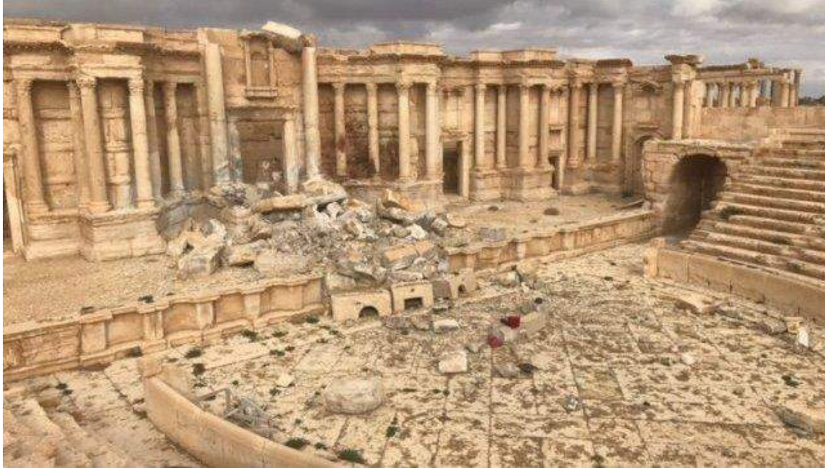
Damage to the front and stage of theater (RIA; March 3, 2017)
