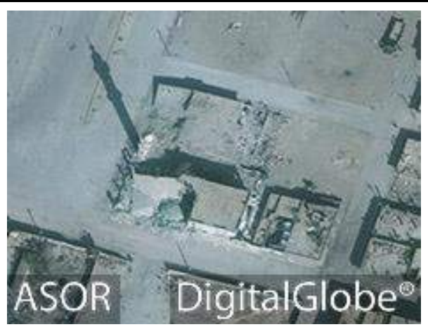
Othman bin Affan Mosque severely damaged with a collapsed dome (DigitalGlobe; February 26, 2017)
