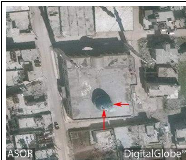
Previous damage to the mosque's dome (DigitalGlobe; February 21, 2017)
