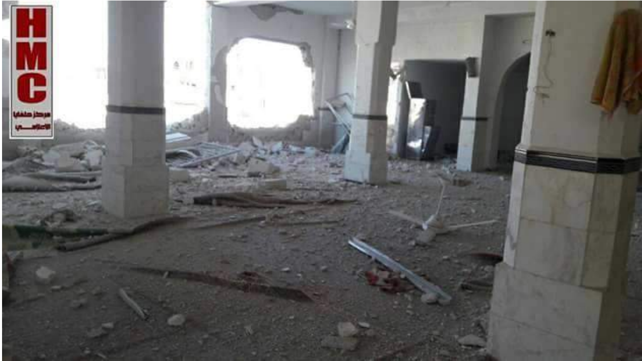
Damage to interior of Mosque (SHNR; March 25, 2017)
