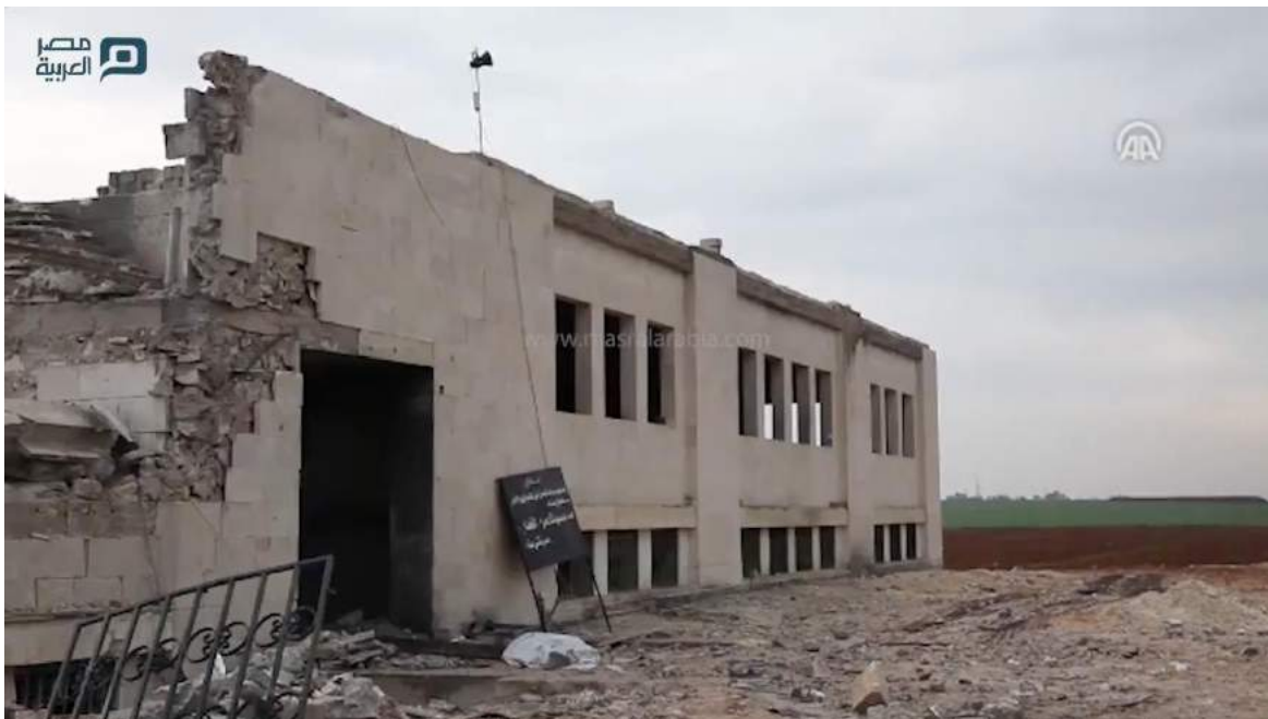
Video still shows damage to Omar Ibn al-Khattab Mosque (Masr Alarabia; March 18, 2017)
