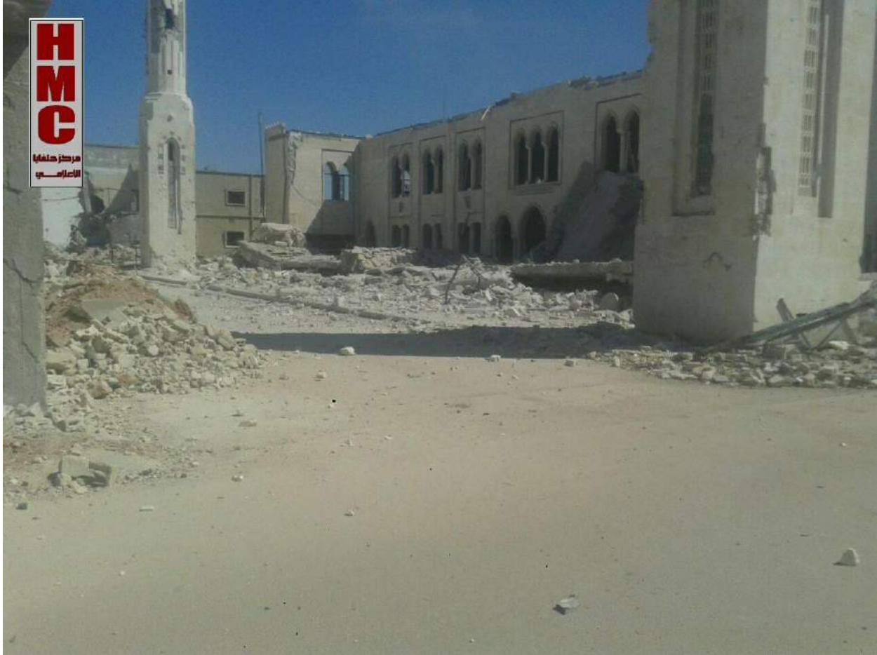
Damage to the courtyard and exterior of the mosque (SNHR; March 25, 2017)
