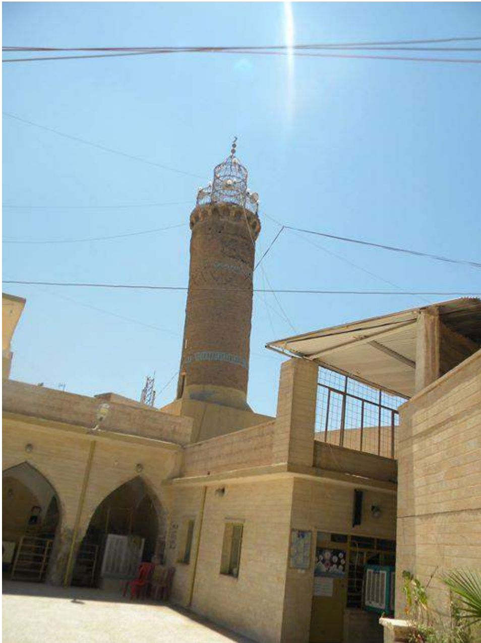
Minaret of the Omar al-Aswad Mosque before airstrike (Layla Salih; March 1, 2017)
