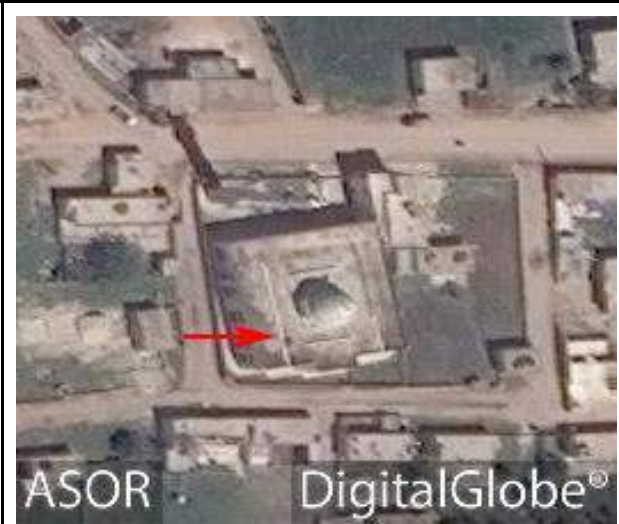
Visible hole in the roof of the mosque (DigitalGlobe; April 3, 2017)
