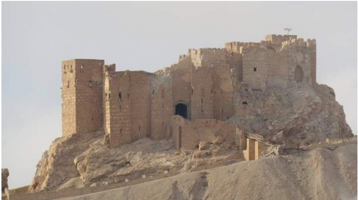
Damage to front of the Citadel (DGAM; March 2, 2017)
