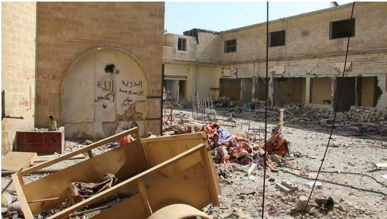
Video still of damage to the courtyard of Umm al-Mauna Church (Iraqi Day; March 8, 2017)
