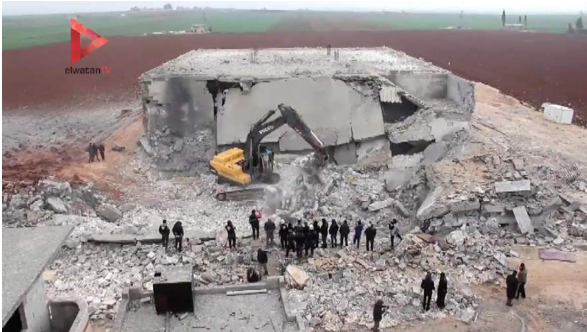
Debris being cleared from the mosque compound (Al Watan TV; March 18, 2017)
