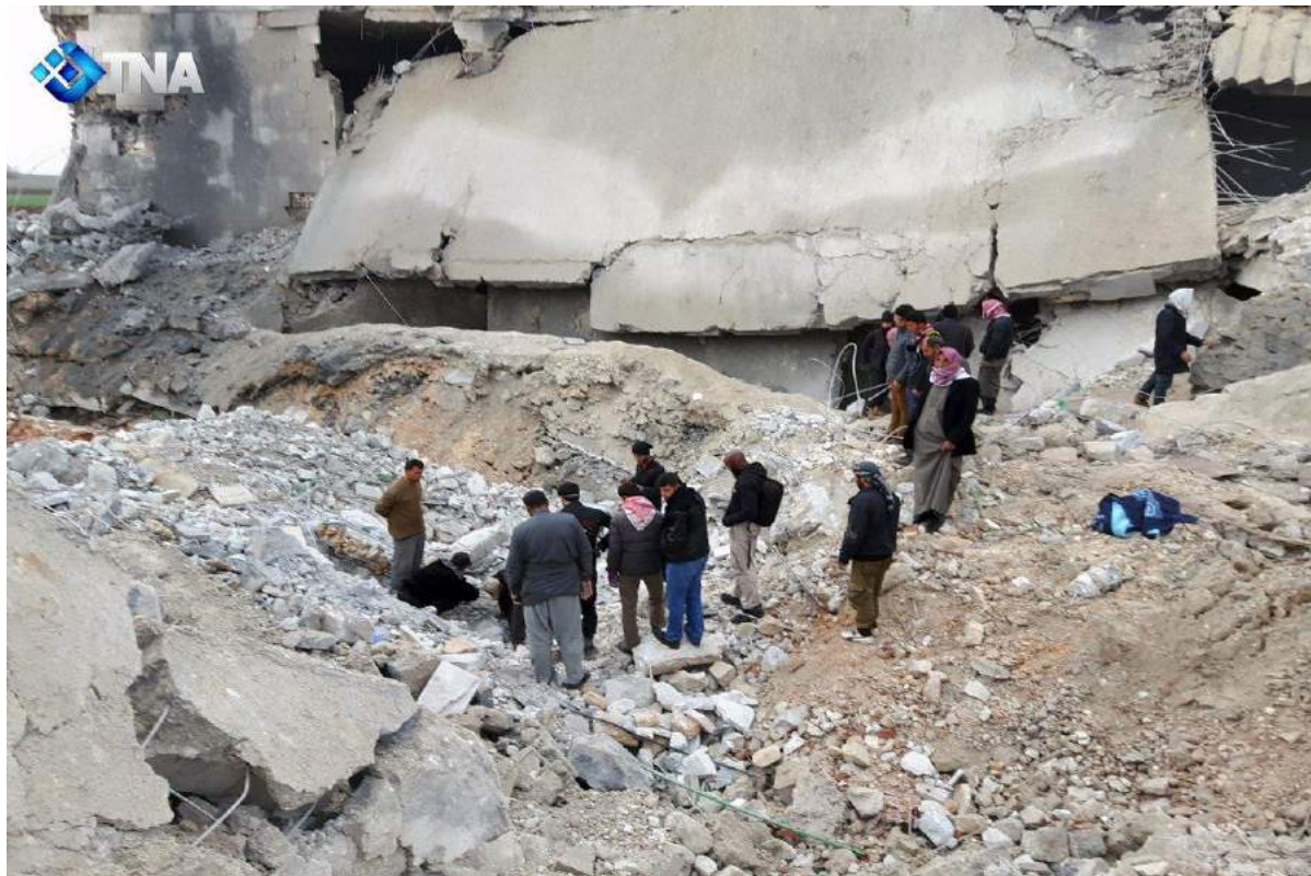
Extensive damage seen to mosque compound (Charles Lister; March 17, 2017)
