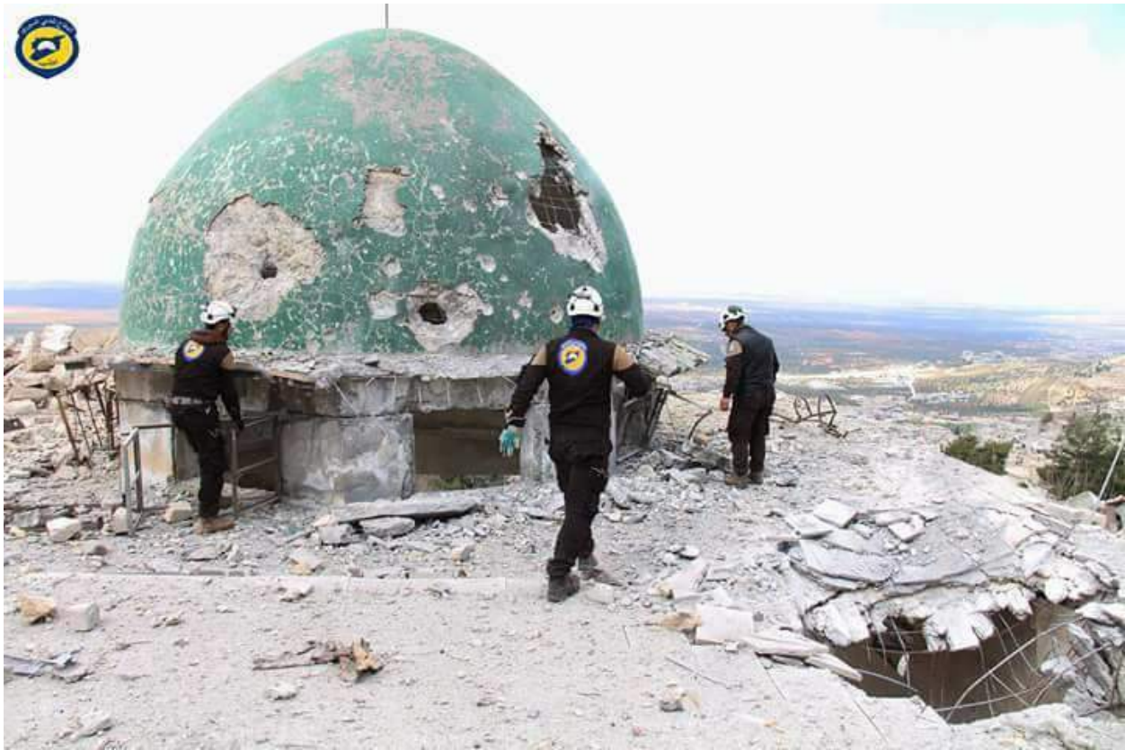
Damage to the dome of al-Rahman Mosque (SNHR; March 29, 2017)
