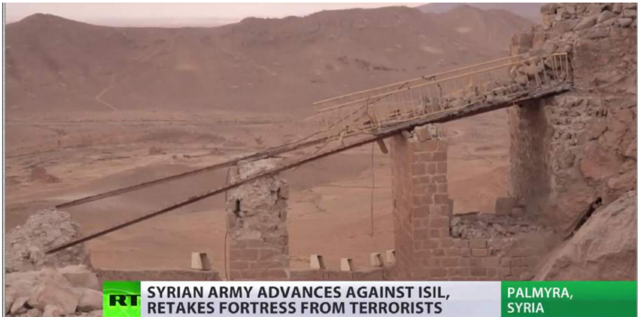
Video still of destruction to the causeway of the Citadel (Ruptly TV; March 1, 2017)
