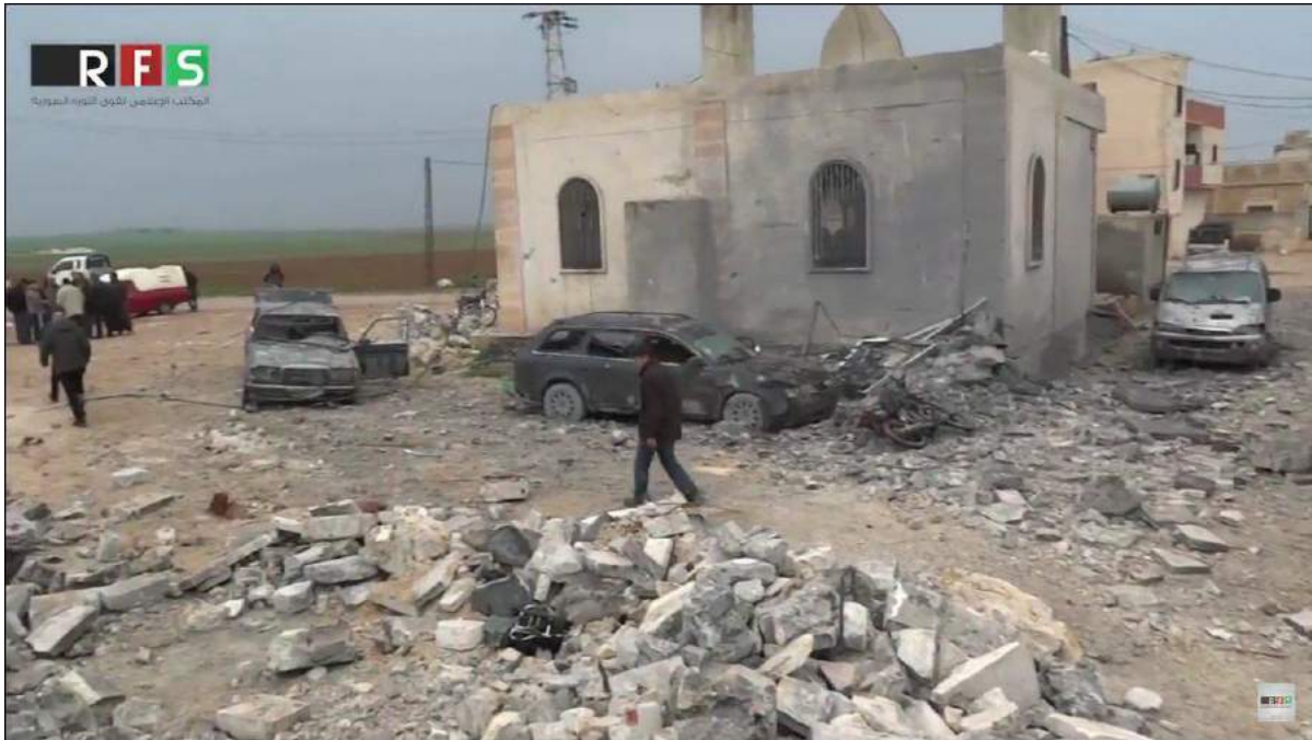
Damage seen to area surrounding the mosque compound, including to this smaller mosque seen in the photograph (RFS/Bellingcat; March 16, 2017)
