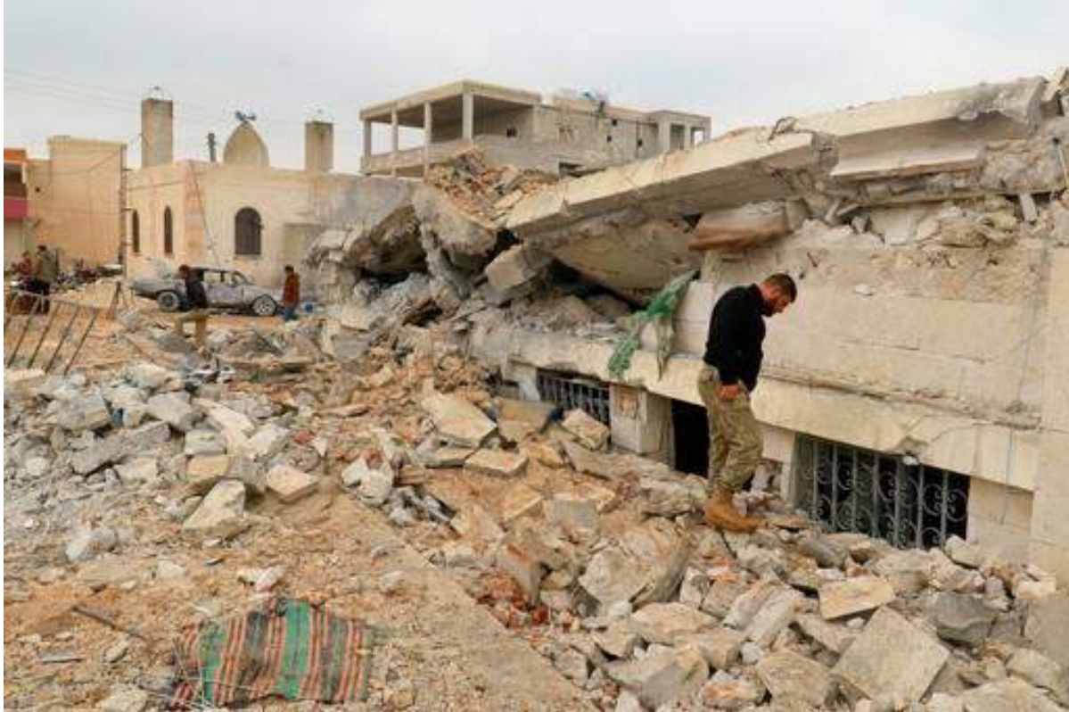
A man inspects damage to the mosque compound (Independent IE/Reuters; March 18, 2017)
