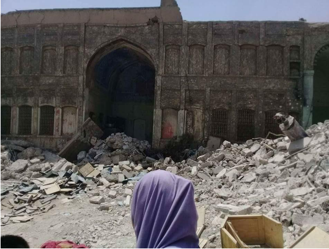
Damage to Dar Thun Hadid showing possible fire damage, rubble, shrapnel/bullet holes/ and graffiti (Private Facebook Account; July 3, 2017)
