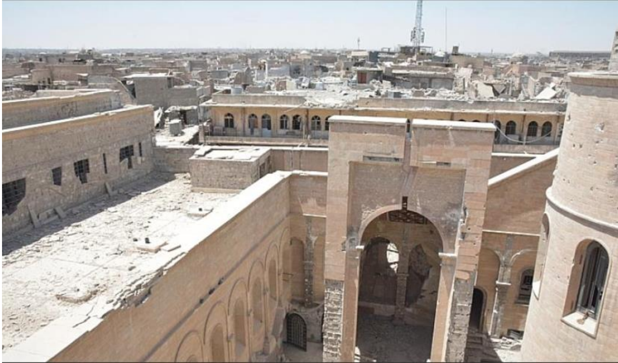
Damage to the interior courtyard from top of al-Sa'a Church (Seth Robson/Stars and Stripes; July 22, 2017)
