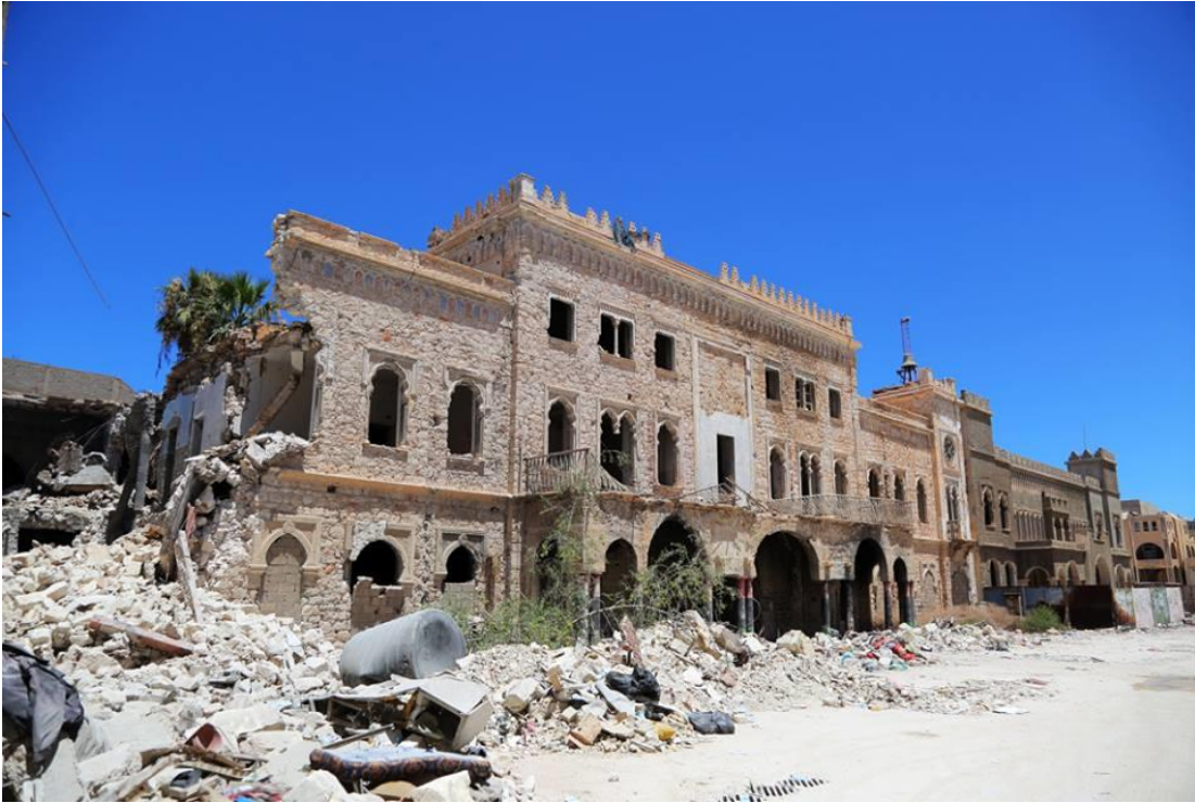
Damage to Ottoman Municipal Building (Private Facebook Account; July 18, 2017)
