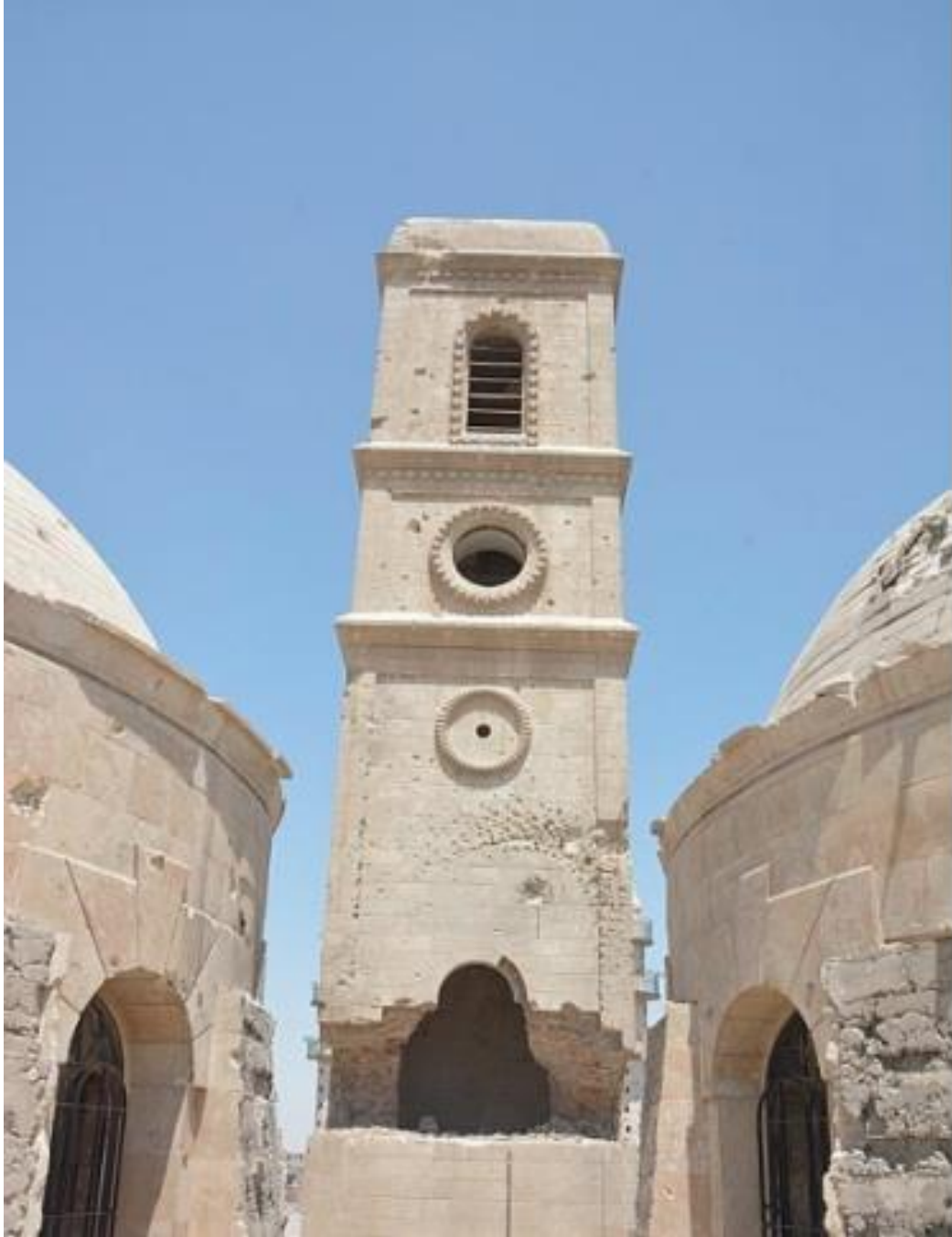
Damage to the clocktower of al-Sa'a Church (Seth Robson/Stars and Stripes; July 22, 2017)
