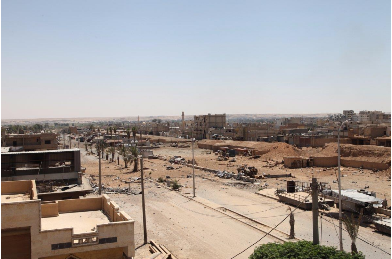
View of the southern breach from the northeast (Qasioun News Agency; July 20, 2017)
