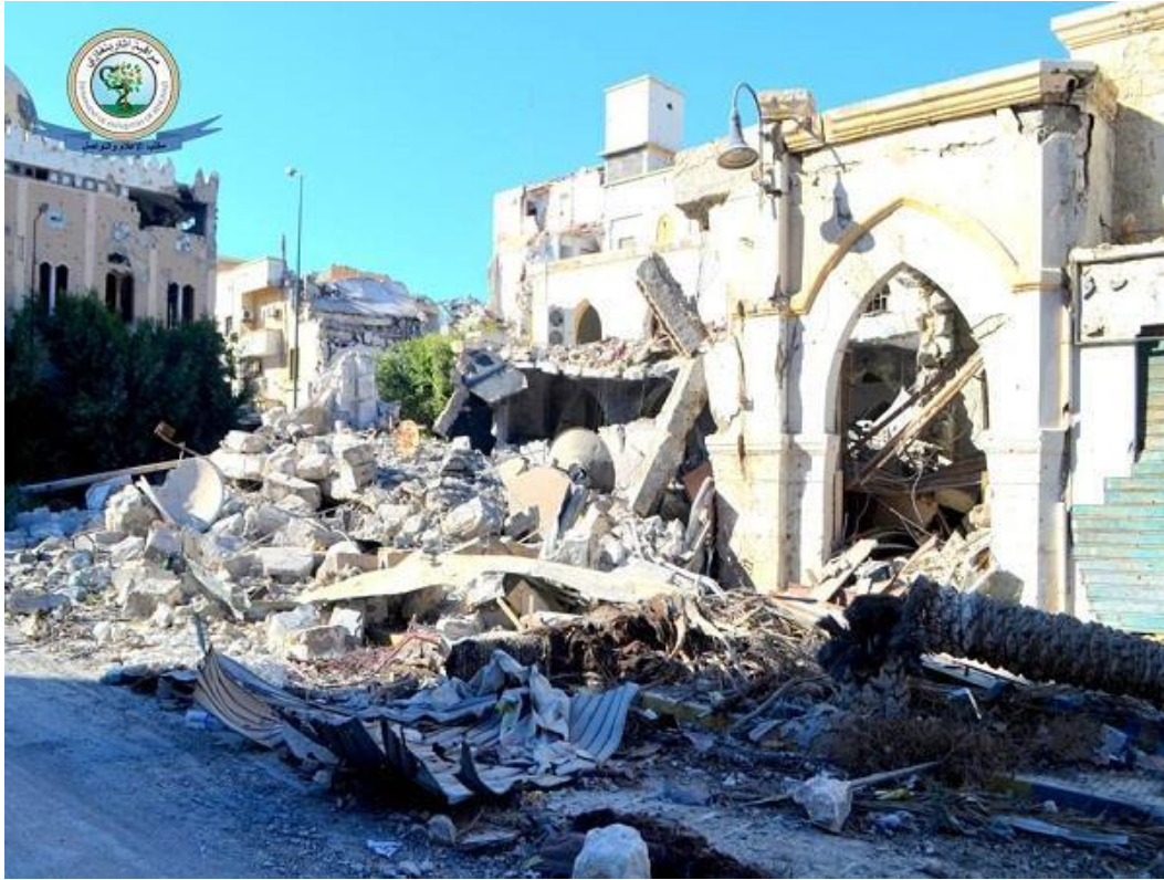
Damage to buildings adjacent to the storeroom in Souq al Hout (DOA Benghazi; June 27, 2017)
