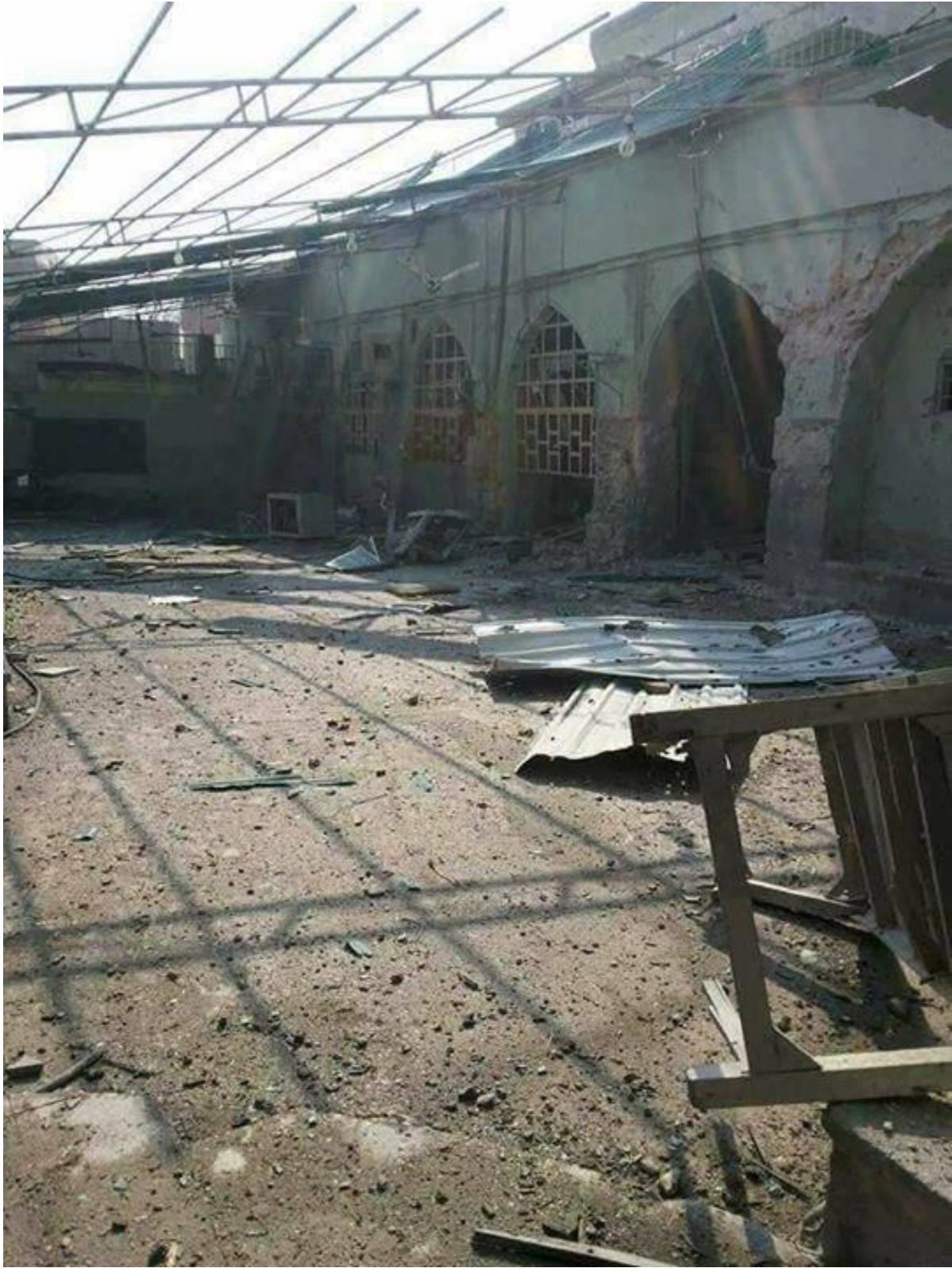
Damage to the courtyard of al-Hamdeen Mosque (Iraqi Day; June 24, 2017)
