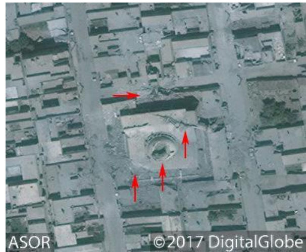
Mosque after the airstrike with damage to the dome, minaret, and multiple walls (DigitalGlobe NextView License; July 25, 2017)
