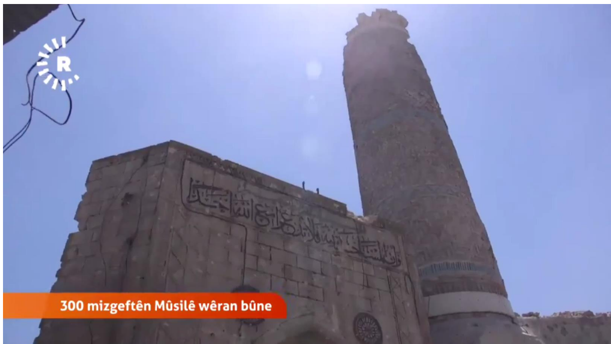
Video still of damage to the front of al-Ziwani Mosque, the top of the minaret has been destroyed (Rudaw; July 10, 2017)
