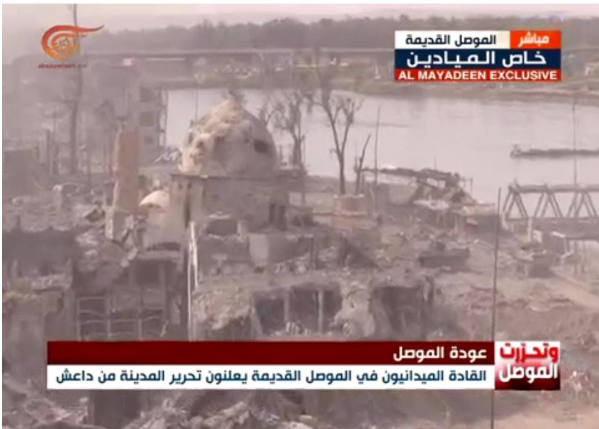
Video still of damage to al-Aghwat Mosque (al-Mayadeen; July 8, 2017)
