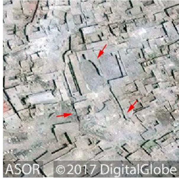
Red arrows indicating damage to the archdiocese on July 8, 2017 (DigitalGlobe NextView License; July 8, 2017)
