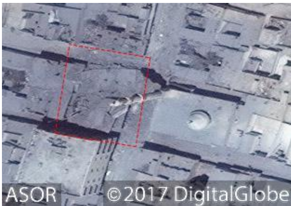
Damage to building directly west of the mosque while the mosque has dust covering the roof (DigitalGlobe NextView License; June 17, 2017)
