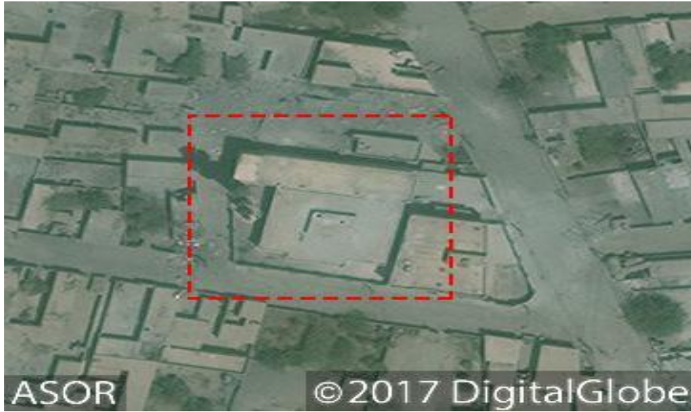
Al-Safa Mosque prior to damage (DigitalGlobe NextView License; July 19, 2017)
