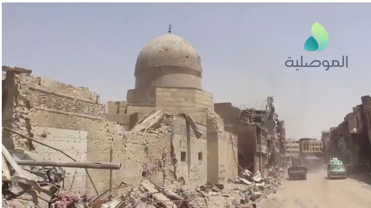
Video still of damage to the exterior of al-Qataneen Mosque (al-Mosuliya; July 12, 2017)
