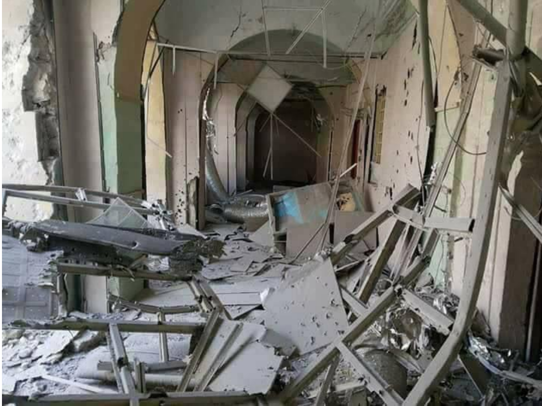
Damage to the interior of al-Hamdeen Mosque (Iraqi Day; June 24, 2017)
