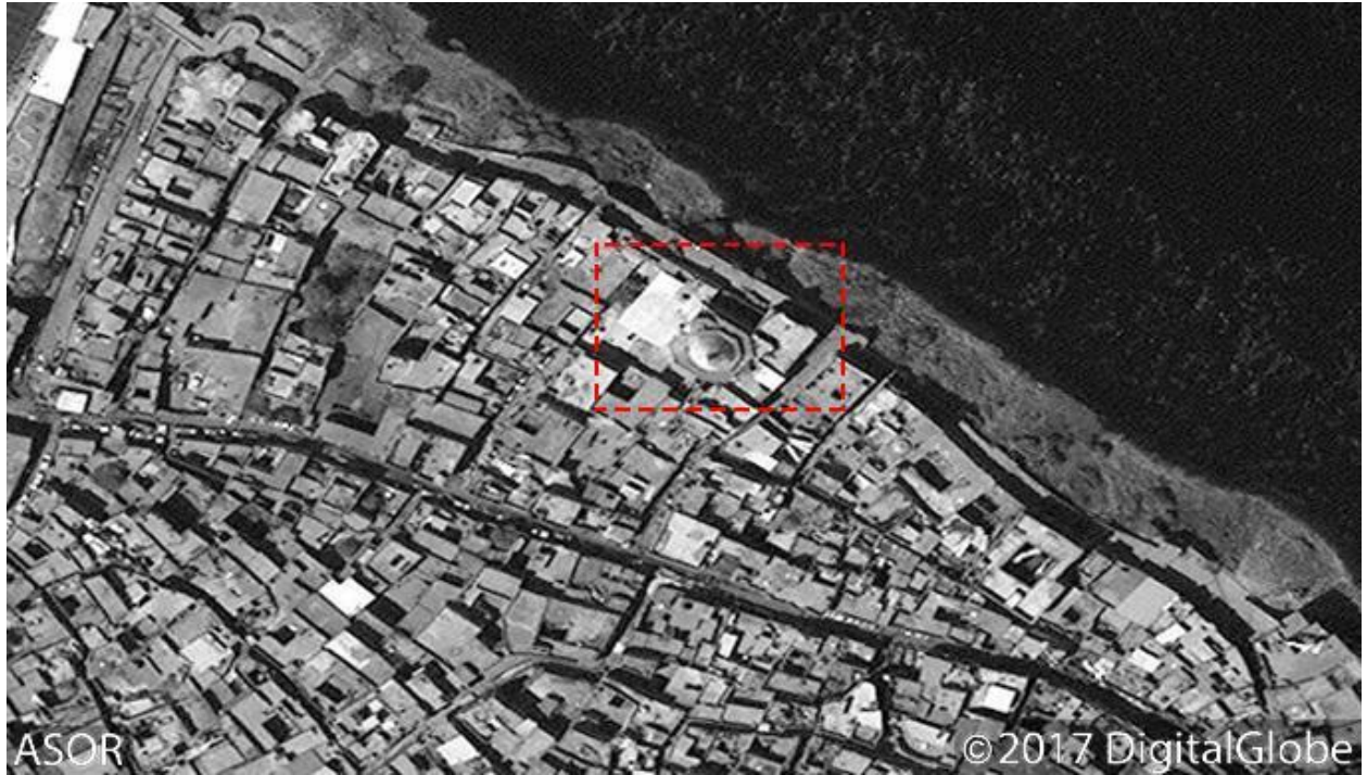
Sheikh al-Shut Mosque prior to damage (DigitalGlobe NextView License; July 1, 2017)
