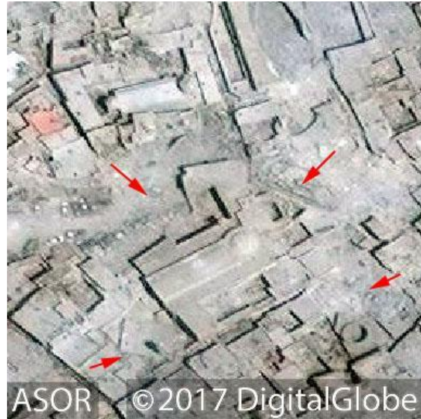
Arrows indicating damage to the church (DigitalGlobe NextView License; July 8 2017)
