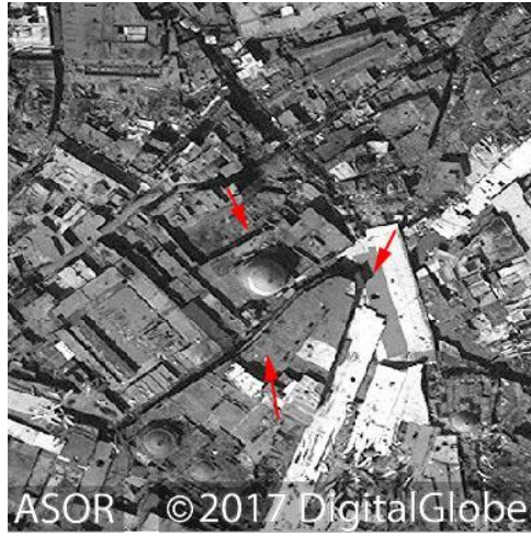
The first instance of damage to the mosque, indicated by red arrows (DigitalGlobe NextView License; March 25, 2017)
