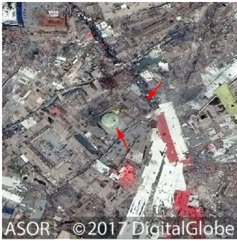
Increased damage to the mosque indicated by red arrows (DigitalGlobe NextView License; April 15, 2017)
