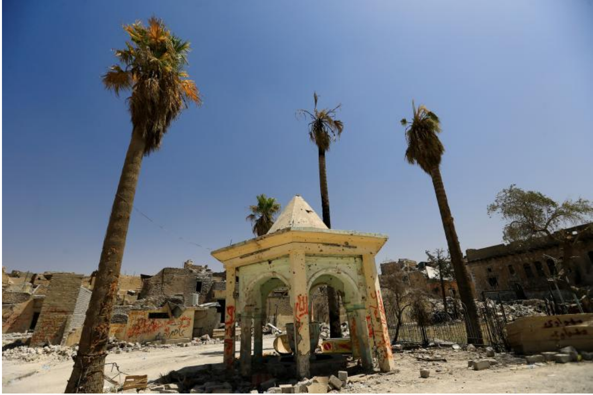
Graffiti on the structure over the ablution fountain in courtyard of al-Nuri Mosque (Reuters; July 24, 2017)
