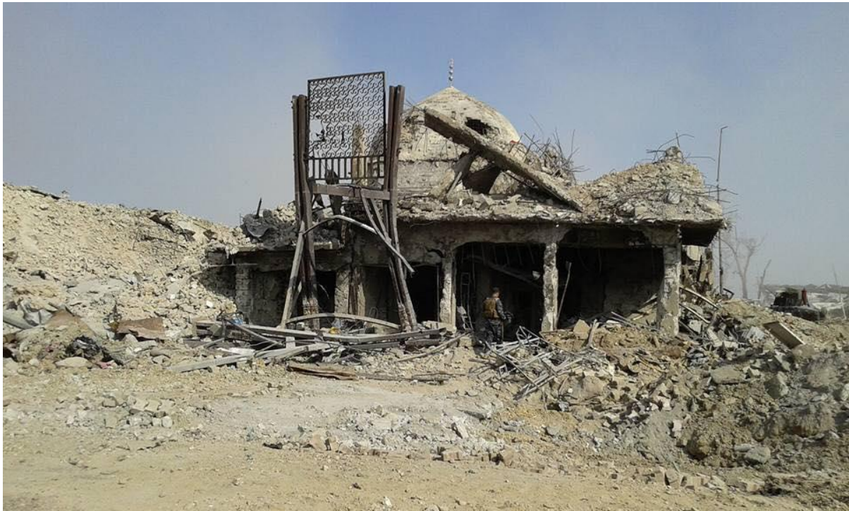
Damage to the southern side of al-Aghwat Mosque (Mosul Ateka; July 10, 2017)
