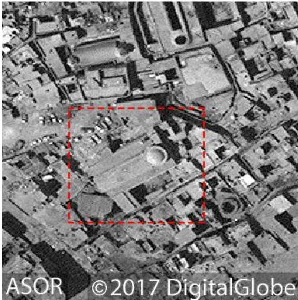
Syriac Orthodox Church shown in red box, prior to damage (DigitalGlobe NextView License; July 1, 2017)
