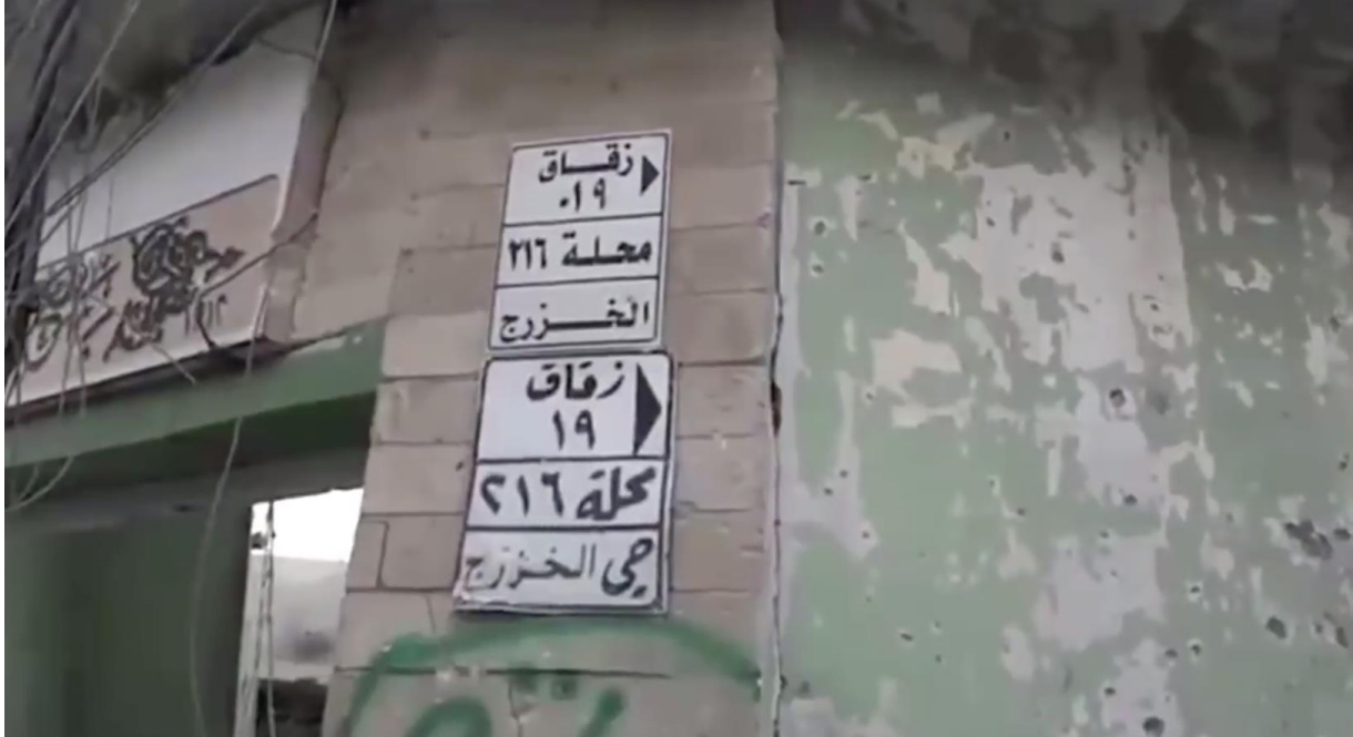
Video still of damage to the exterior of al-Hamdeen Mosque (WK Ahmed; June 23, 2017)
