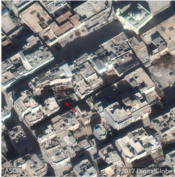
Detail of buildings in the Old City of Benghazi (DigitalGlobe NextView License; December 18, 2016)
