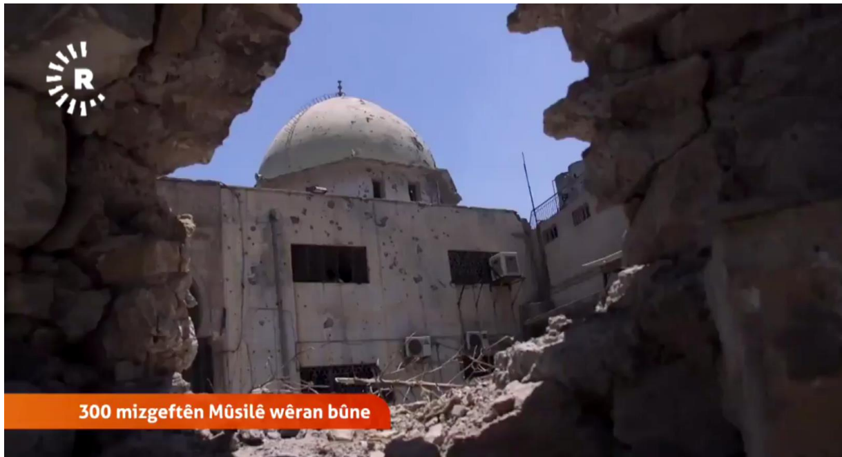
Video still of damage to the interior courtyard of al-Ziwani Mosque (Rudaw; July 10, 2017)
