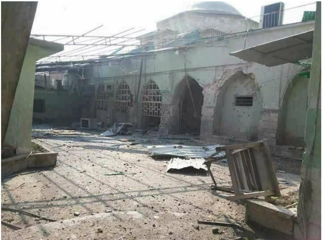
Damage to the courtyard of al-Hamdeen Mosque (Iraqi Day; June 24, 2017)
