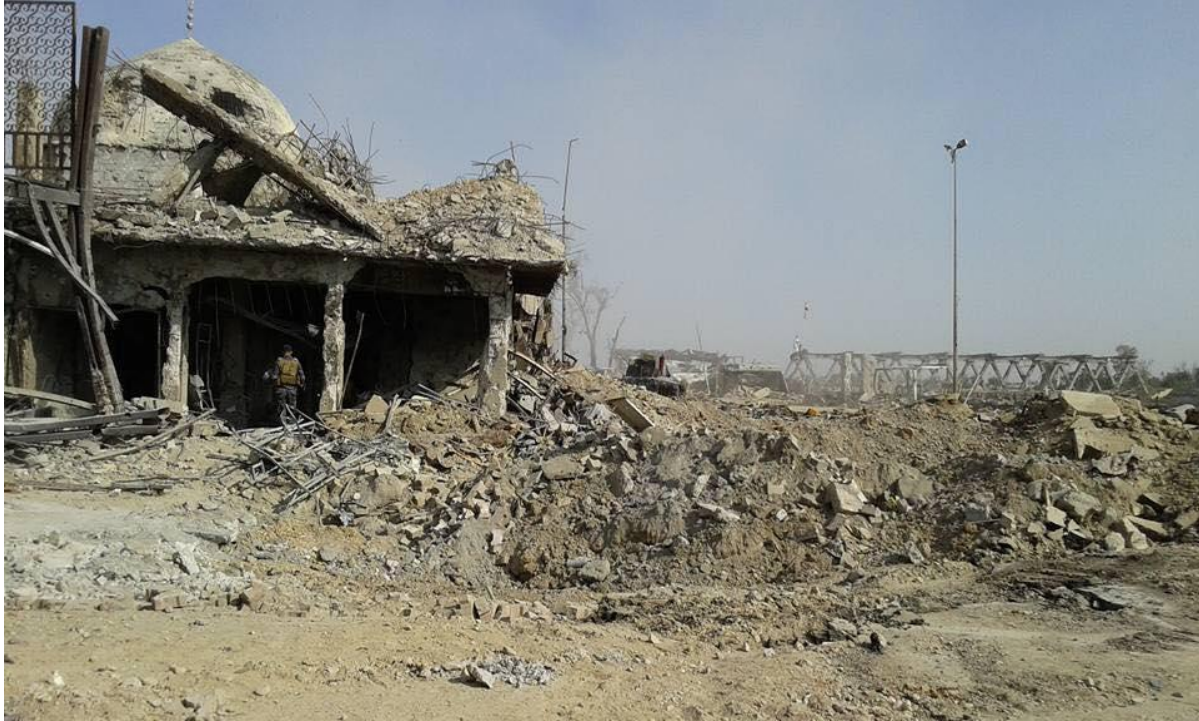
Damage to the southern side of al-Aghwat Mosque, and surrounding area (Mosul Ateka; July 10, 2017)
