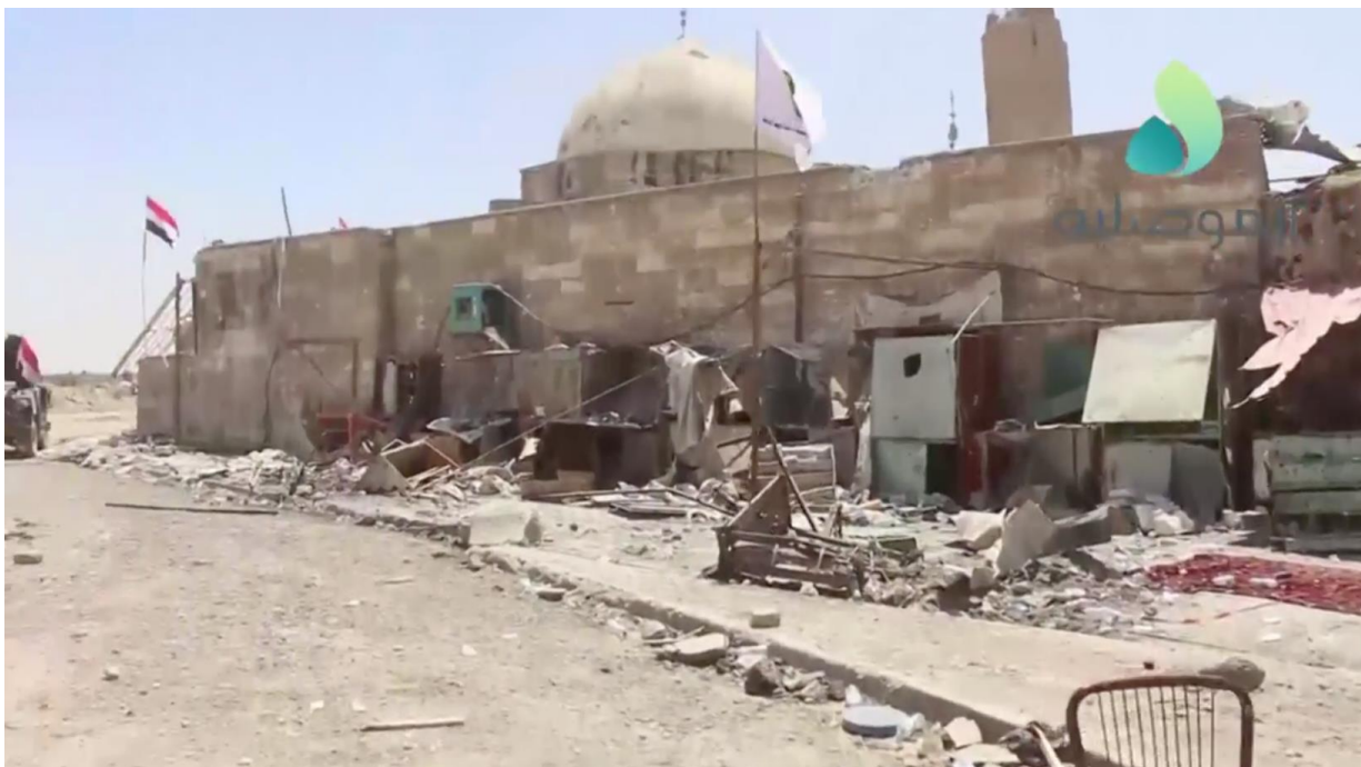
Video still of damage to the northern side of al-Aghwat Mosque (al-Mosuliya; July 17, 2017)
