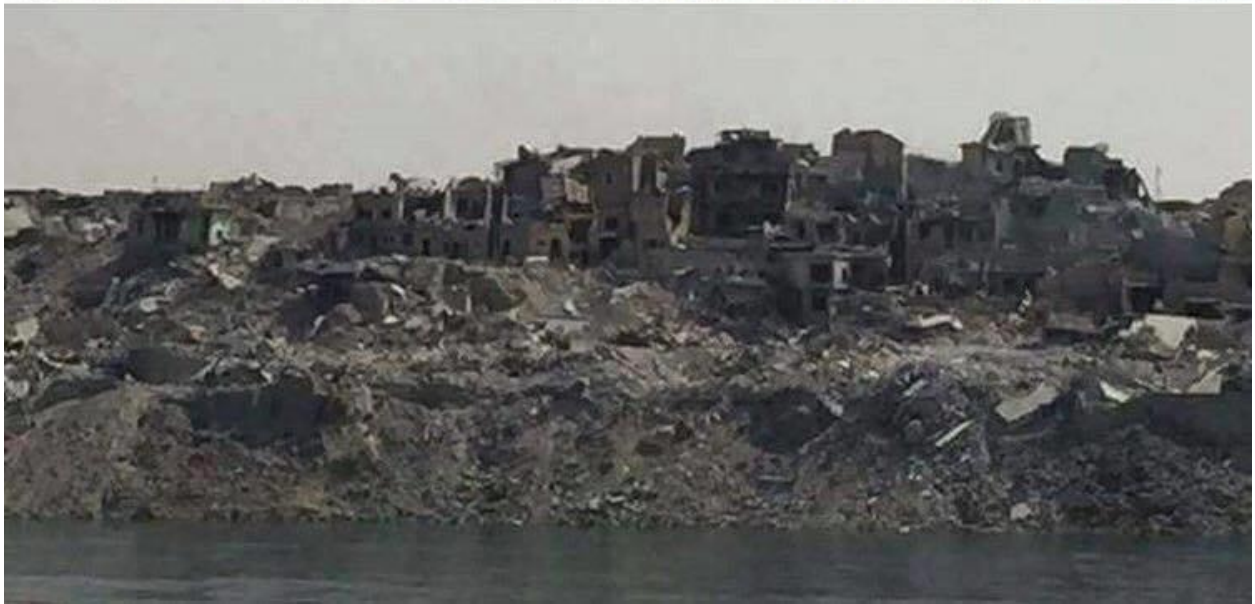
Before-and-after photographs of the Old City near the Sheikh al-Shut Mosque. Bottom photograph taken before July 27, when neighborhood was leveled. (Personal Facebook Account; August 1, 2017)
