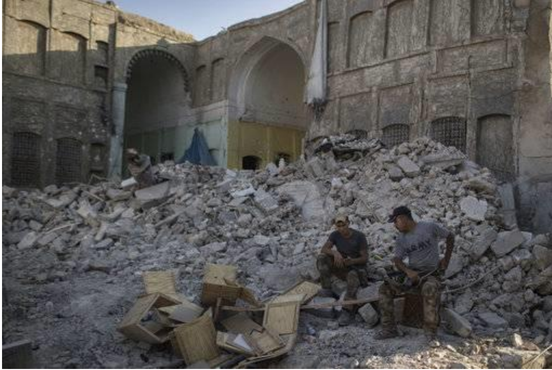
The inside of Dar Thun Hadid showing shrapnel/bullet holes, fire damage, and rubble (Daily Herald; June 30, 2017)
