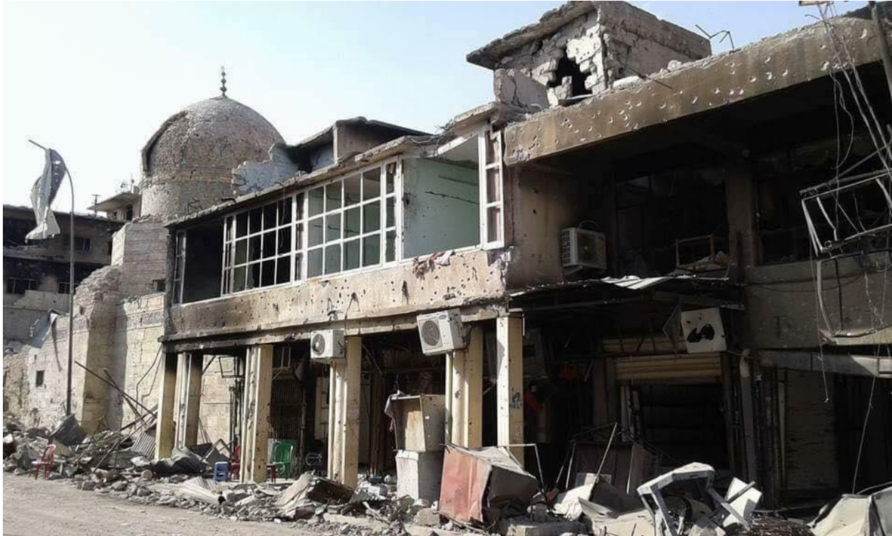
Damage to the dome of al-Qataneen Mosque (Mosul.ateka; July 14, 2017)
