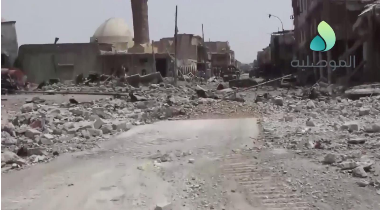
Video still of damage to the Omar al-Aswed Mosque and neighborhood (al-Mosuliya; July 3, 2017)
