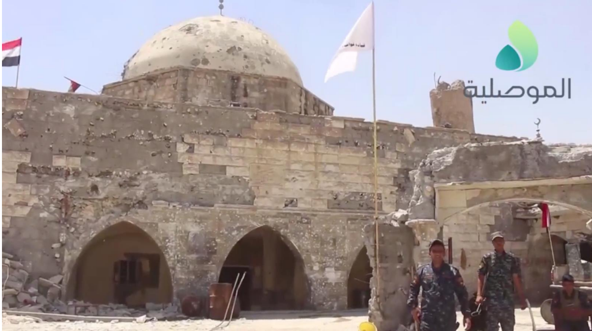
Video still of damage to the eastern side of al-Aghwat Mosque (al-Mosuliya; July 17, 2017)
