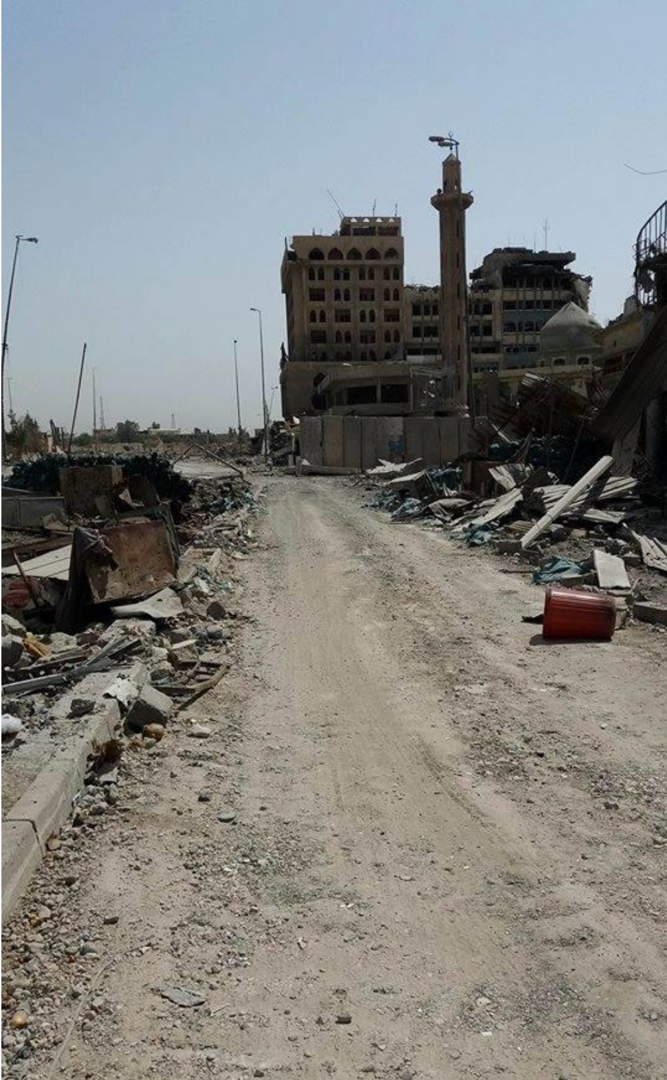
Damage to the mosque and surrounding neighborhood (Mosul Ateka; July 22, 2017)
