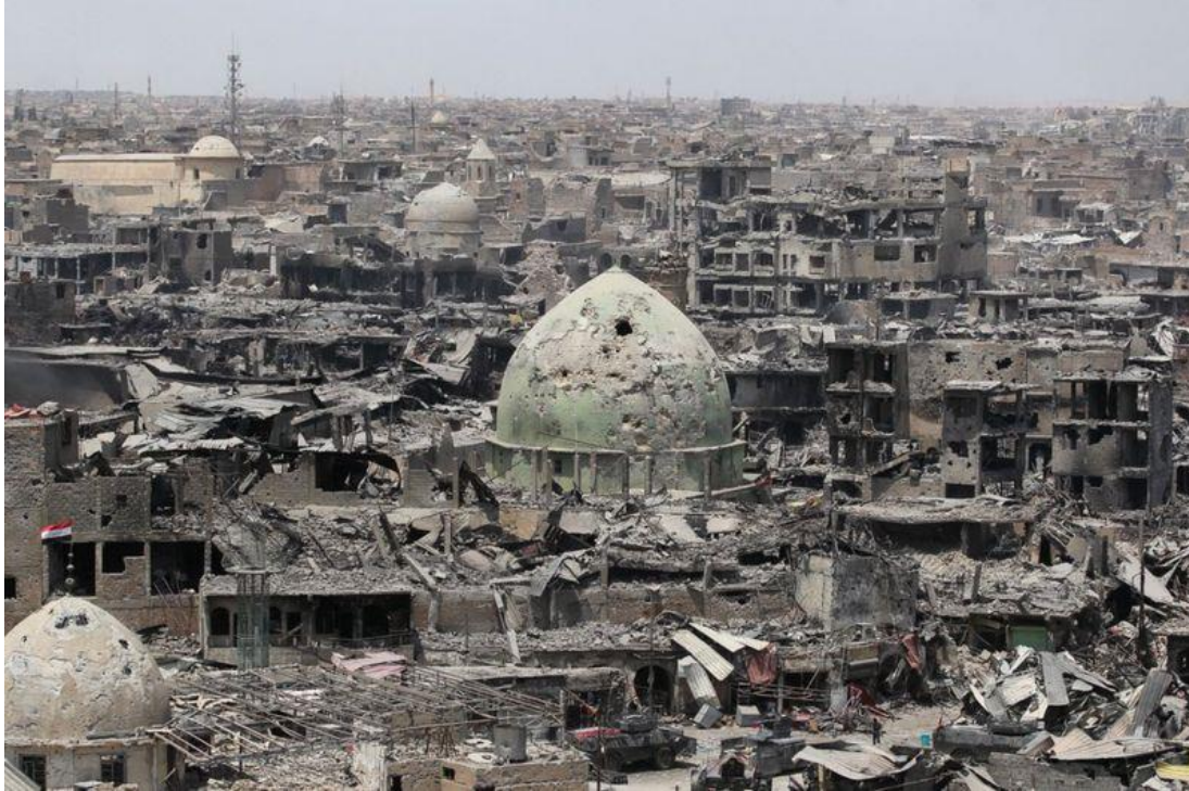
Damage to various sites in old Mosul, including Bab al-Tub Mosque, al-Pasha Mosque, 'Abdal Mosque, Syriac Orthodox Church of al-Tahira, and the Chaldean Catholic Church of al-Tahira (BBC; July 10, 2017)
