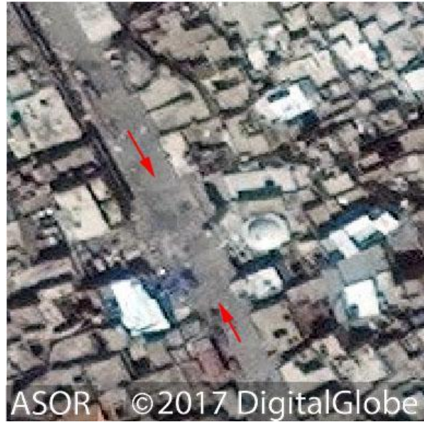
Red arrows indicating the area of explosion damaging the minaret and western facade of the mosque (DigitalGlobe NextView License; April 26, 2017)
