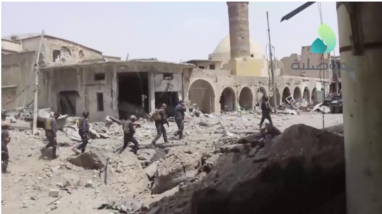
Video still of damage to the side of the Omar al-Aswed Mosque (al-Mosuliya; July 3, 2017)
