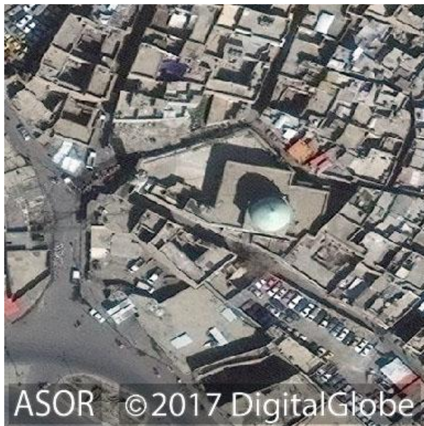
The mosque prior to any damage (DigitalGlobe NextView License; February 25, 2017)
