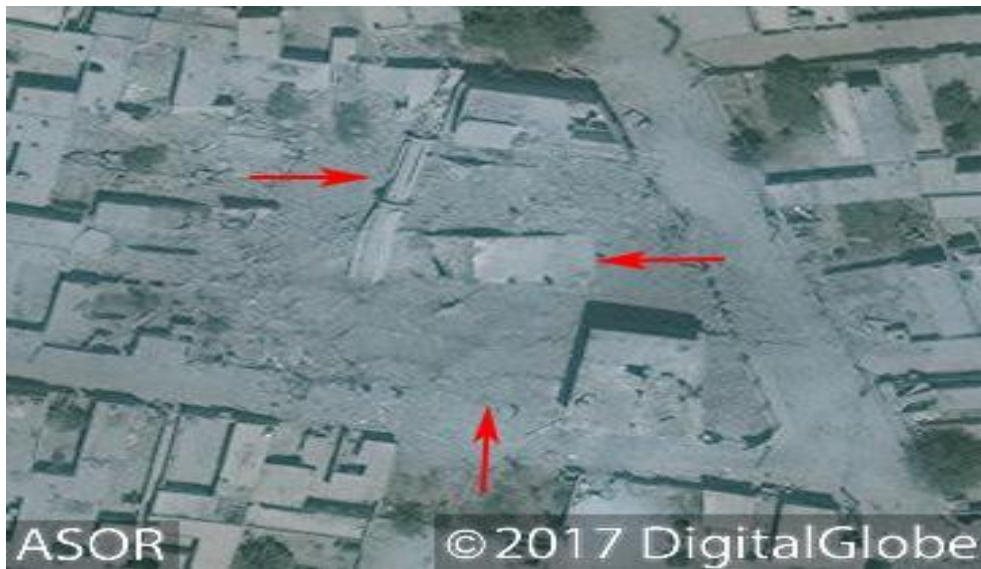
Severe damage to al-Safa Mosque, with the main building destroyed and the minaret lying on the debris (DigitalGlobe NextView License; July 25, 2017)
