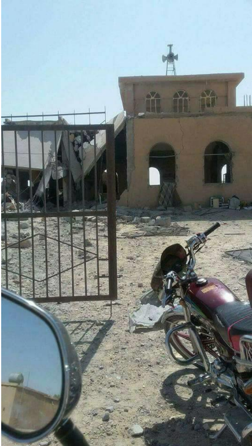
Damage to al-Rahman Mosque (SNHR; July 18, 2017)
