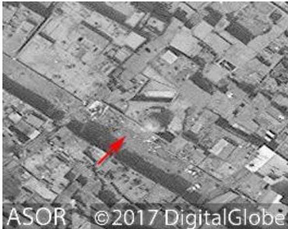
The metal roof removed, and pieces visible on the ground (DigitalGlobe NextView License; May 11, 2017)
