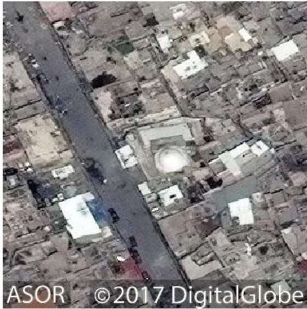
al-Juwayjati Mosque prior to any damage (DigitalGlobe NextView License; April 15, 2017)
