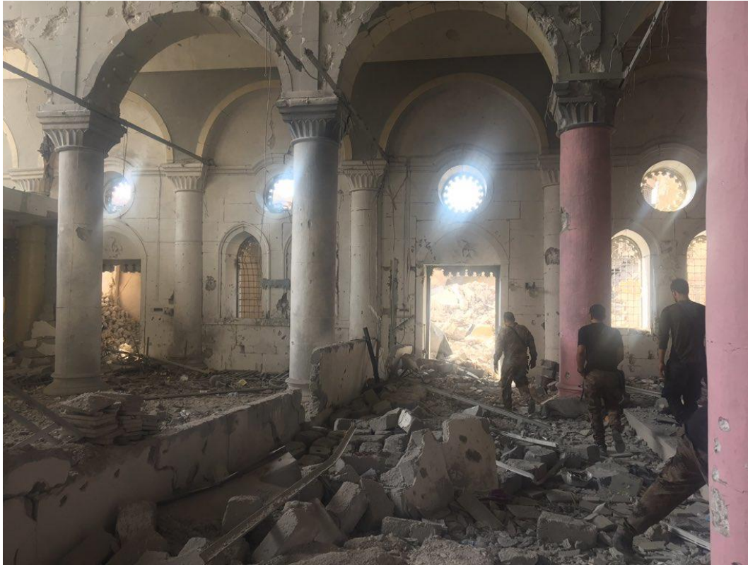
Damage to the interior of Syriac Orthodox Church (Rukmini Callimachi/NYT; July 11, 2017)
