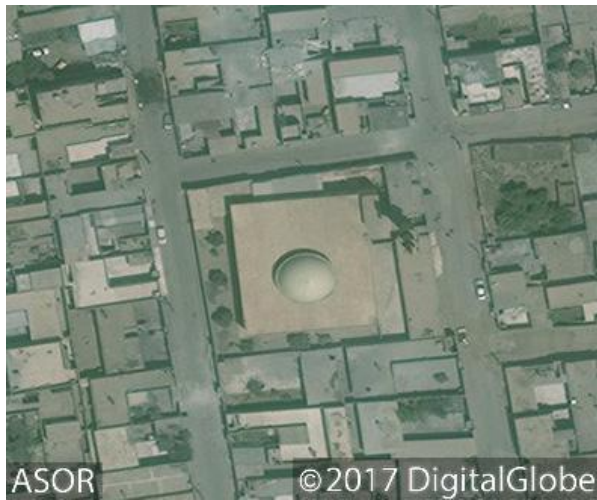
al-Mustafa Mosque prior to damage (DigitalGlobe NextView License; July 19, 2017)
