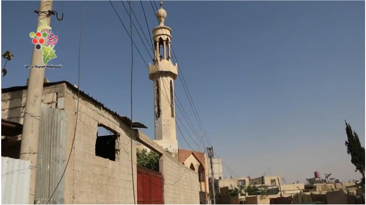
Damage to the minaret of al-Aqoula Mosque (SNHR; July 31, 2017)
