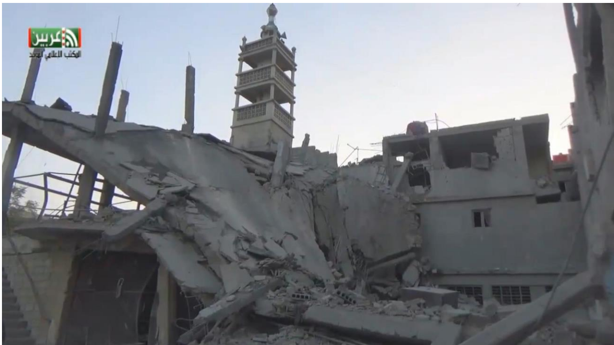
View of the damaged minaret behind a collapsed building (Arbin Media Information Office; July 25, 2017)
