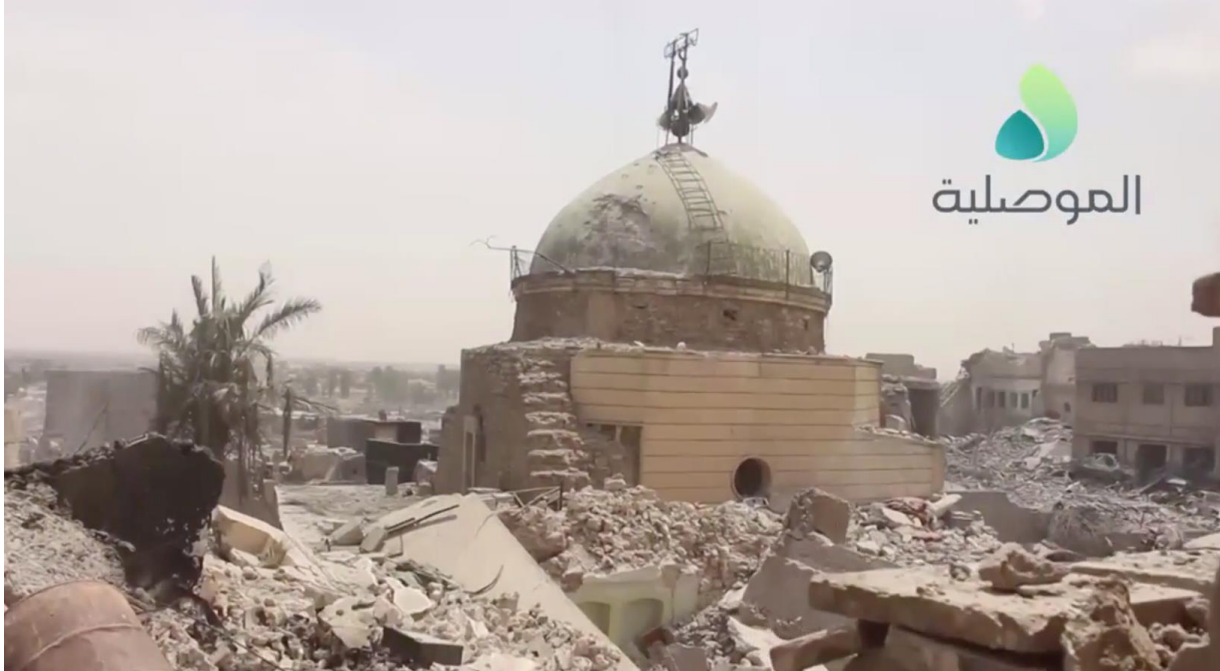
Video still of damage to Umayyad Mosque (al-Mosuliya July 7, 2017)
