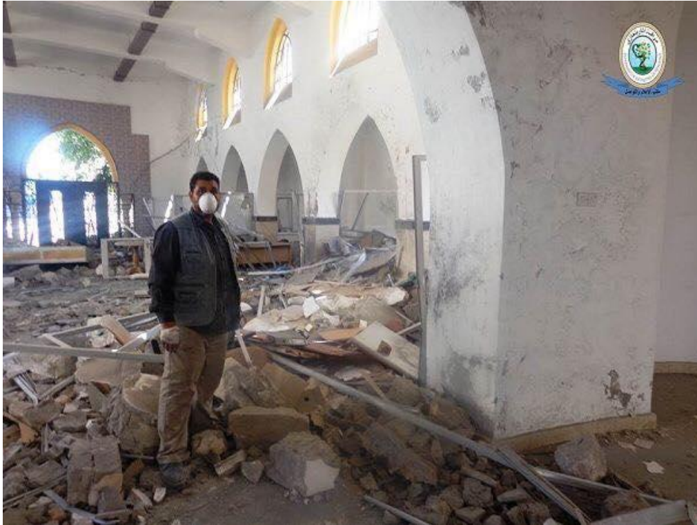
Damage to the interior of the building (Abdel Hafid al-Massalati; July 20, 2017)
