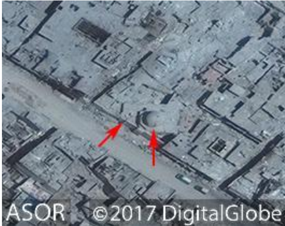
Minor damage to the dome and the front of the mosque (DigitalGlobe NextView License; July 12, 2017)
