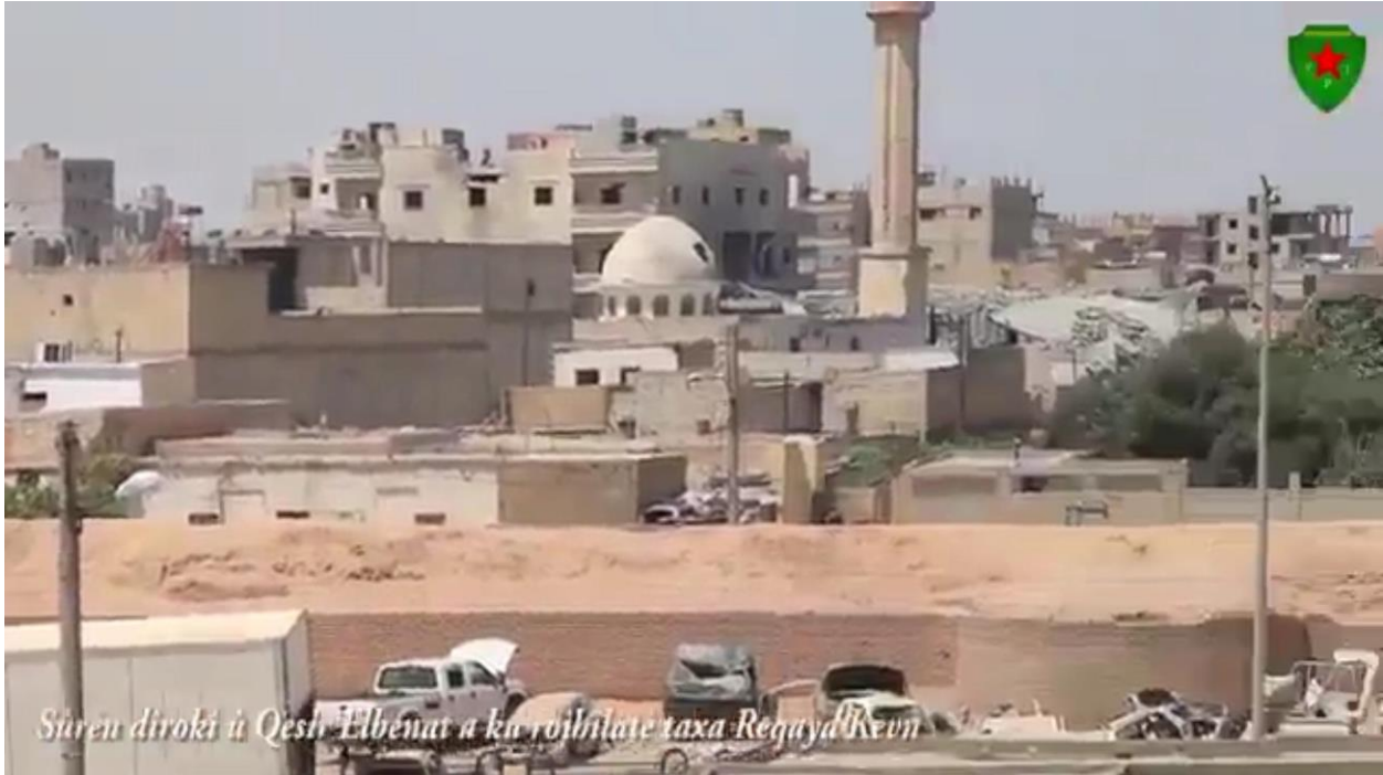
Video still of damage to the dome of the mosque, seen from the east (Personal Twitter Account; July 6, 2017)
