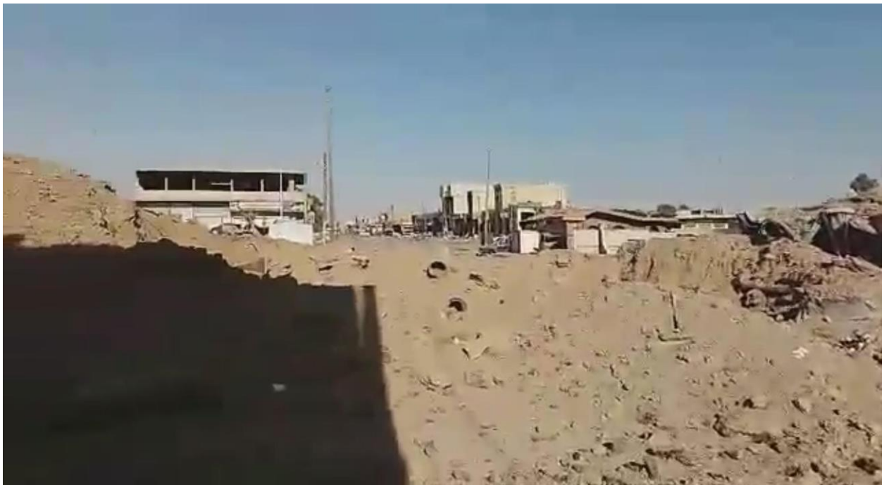
View of the blocked roadway through the wall south of the Qasr al-Banat, seen from the west (RBSS; July 26, 2017)
