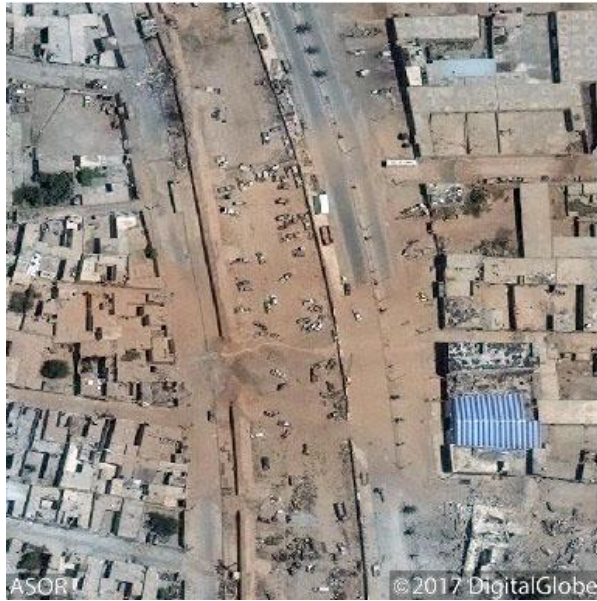
Close-up of the northern wall breach showing damage on July 7, 2017 with a small footpath across the remains of the wall (DigitalGlobe NextView License; July 7, 2017)
