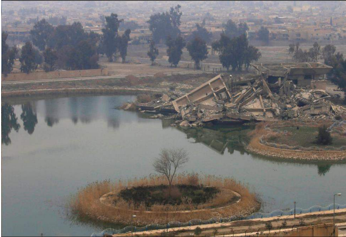
Complete destruction of part of al-Remah palace, and outbuilding (Reuters; January 25, 2017)
