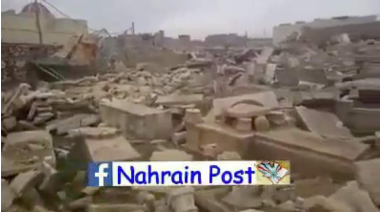
Video still of damage to Tel Kaif Cemetery (Nahrain Post; January 25, 2017)
