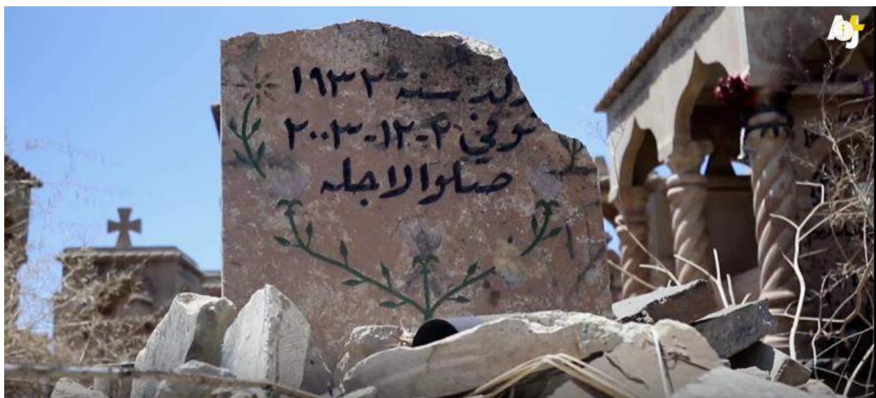
Video still of shelling damage to Tel Kaif Cemetery (AJ+; August 20, 2015)
