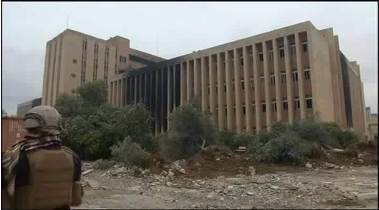
Fire damage and rubble seen at Mosul University Student Center (مجتهد الأنبار; January 16, 2016)
