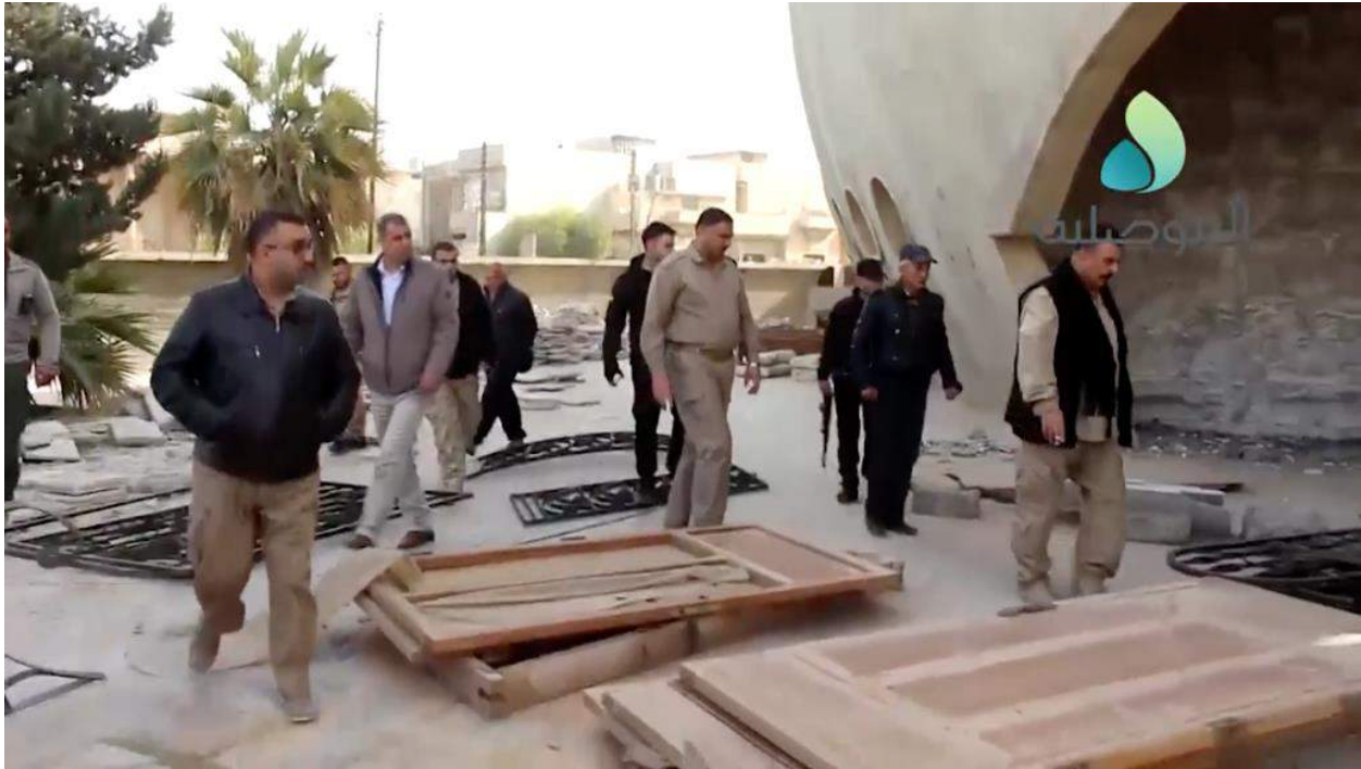
Video still of damage to the exterior of the church (al-Mosuliya; January 11, 2017)
