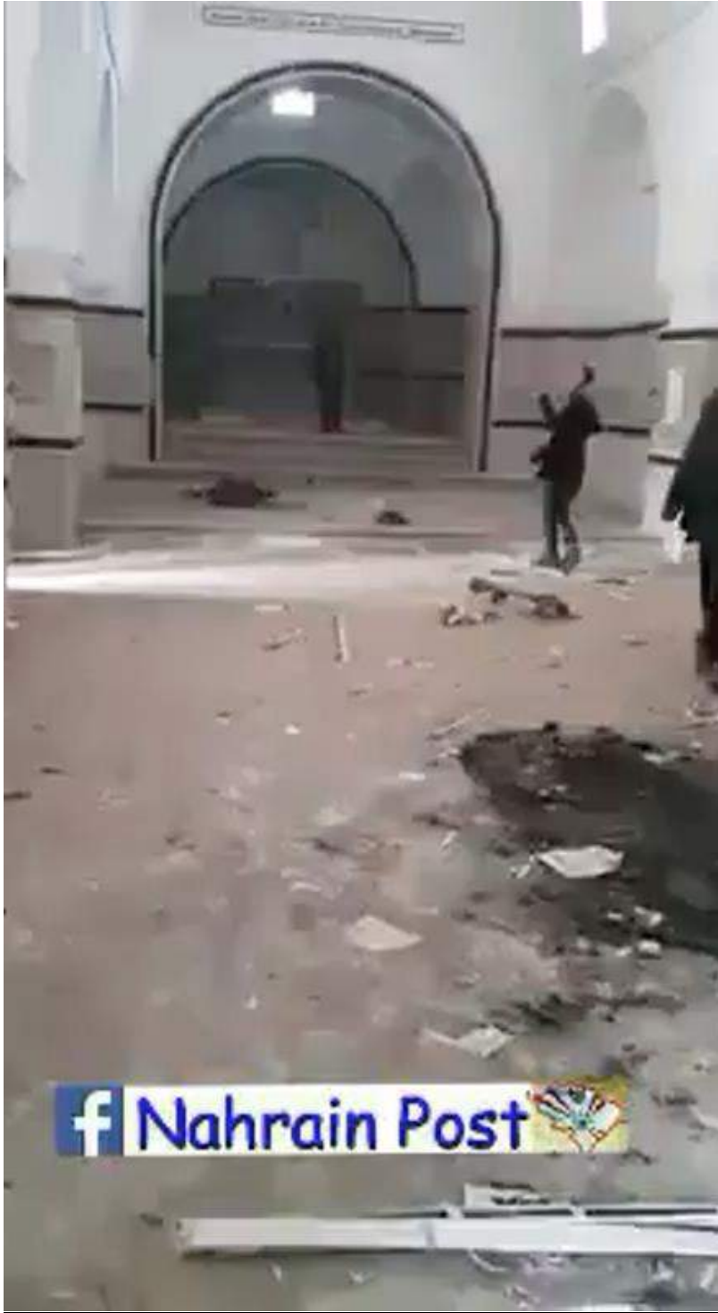
Damage to interior of Mar Yousif Church (Nahrain; January 24, 2017)
