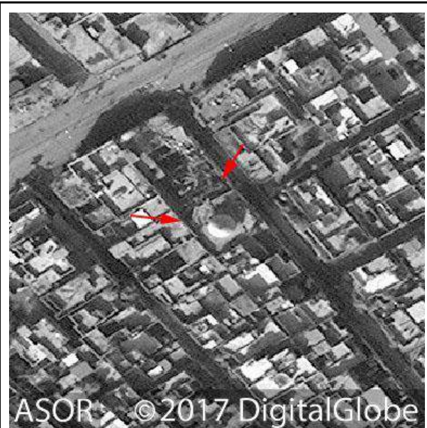
Destruction to mosque indicated by red arrows (DigitalGlobe NextView License; December 30, 2016)
