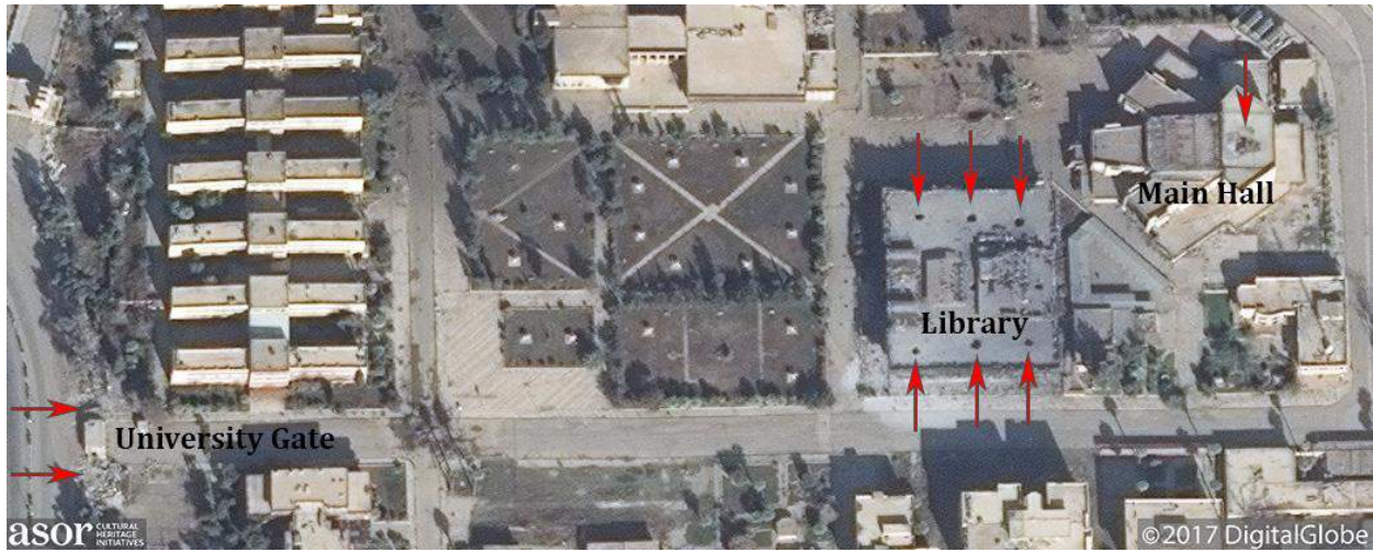
Damage to the Central Library of Mosul University and a University Gate (DigitalGlobe NextView License; January 13, 2017)
