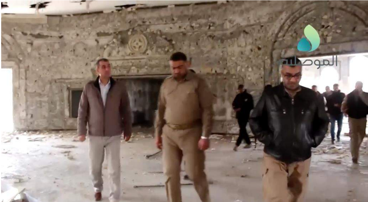
Video still of damage to the interior of the church (al-Mosuliya; January 11, 2017)
