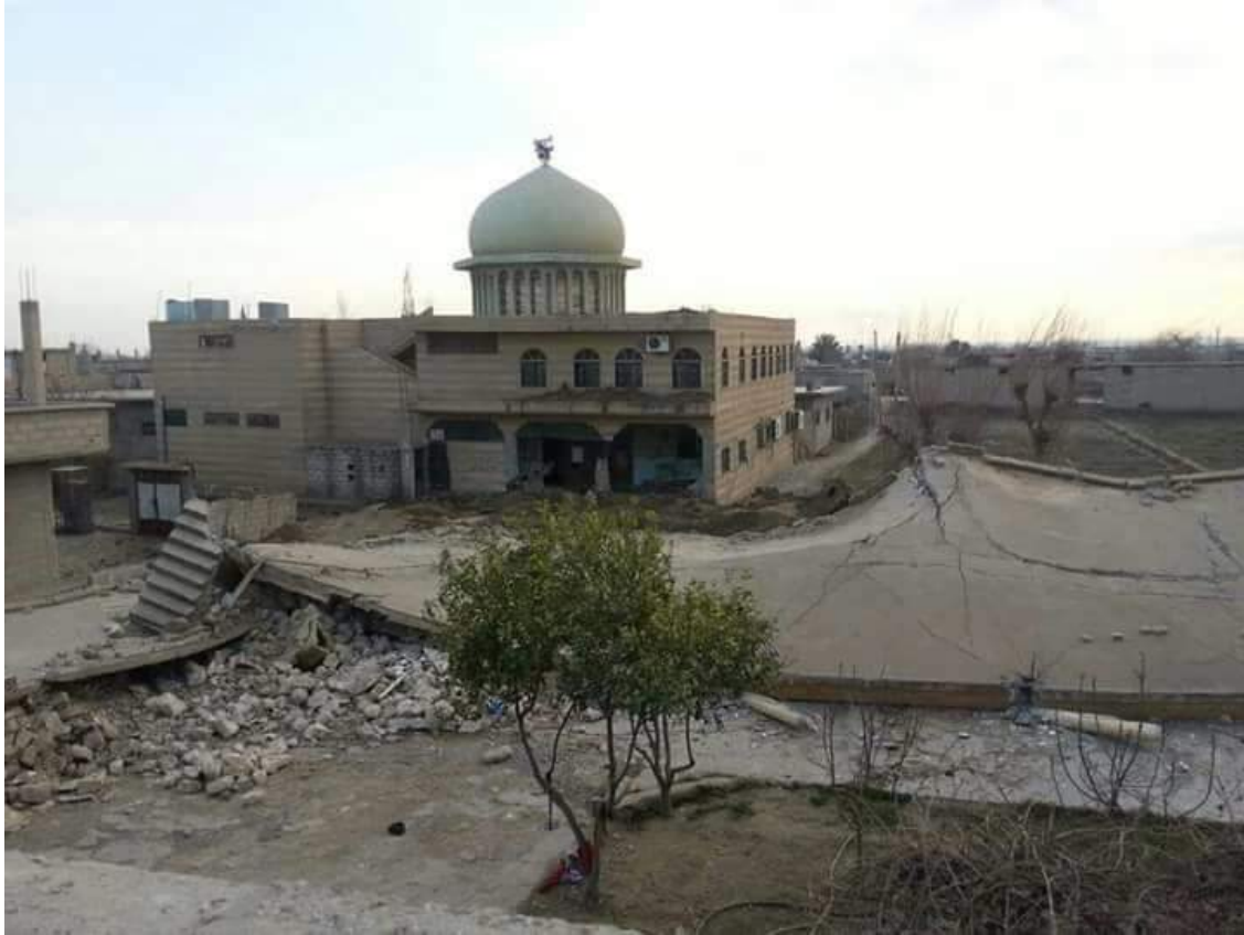
Damage to al-Nour Mosque (SNHR; January 20, 2017)
