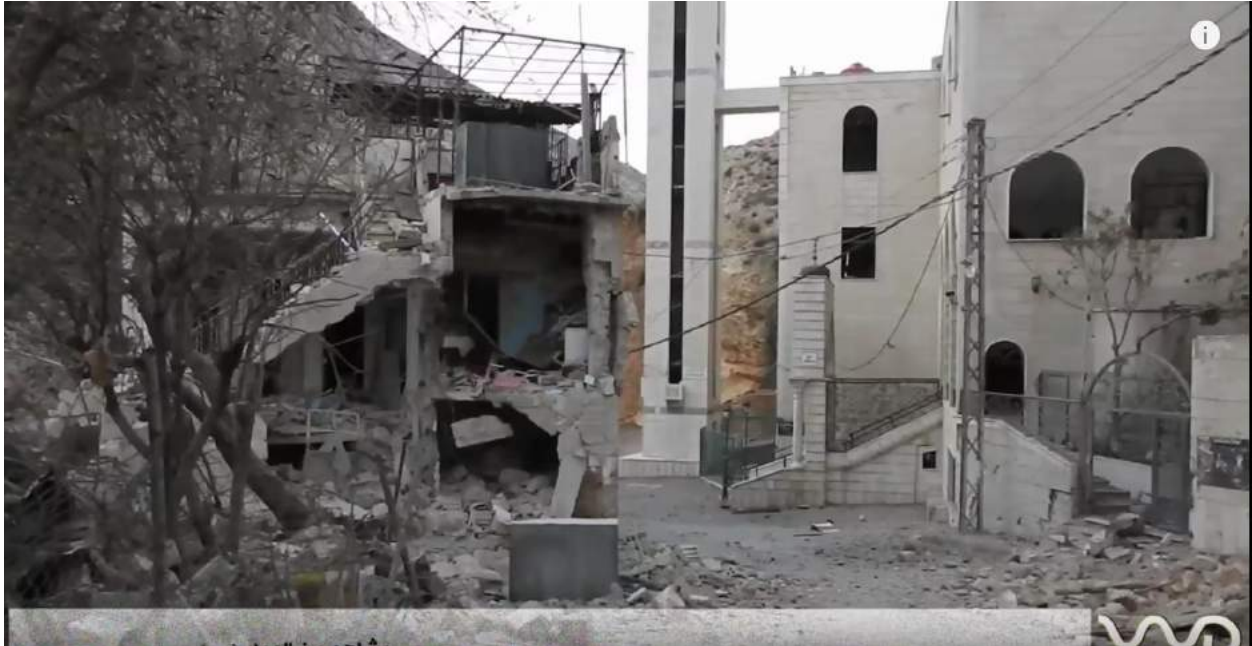
Damage to Ein al-Khadra Mosque and surrounding buildings (Orient News; January 7, 2016)
