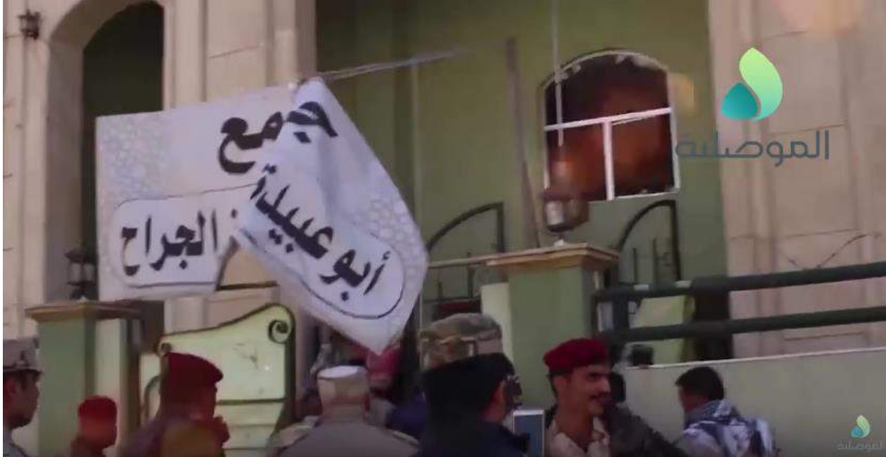
Video still of damage to the exterior of Abu Obeida Amer Bin al-Jarah (al-Mosuliya; January 9, 2017)
