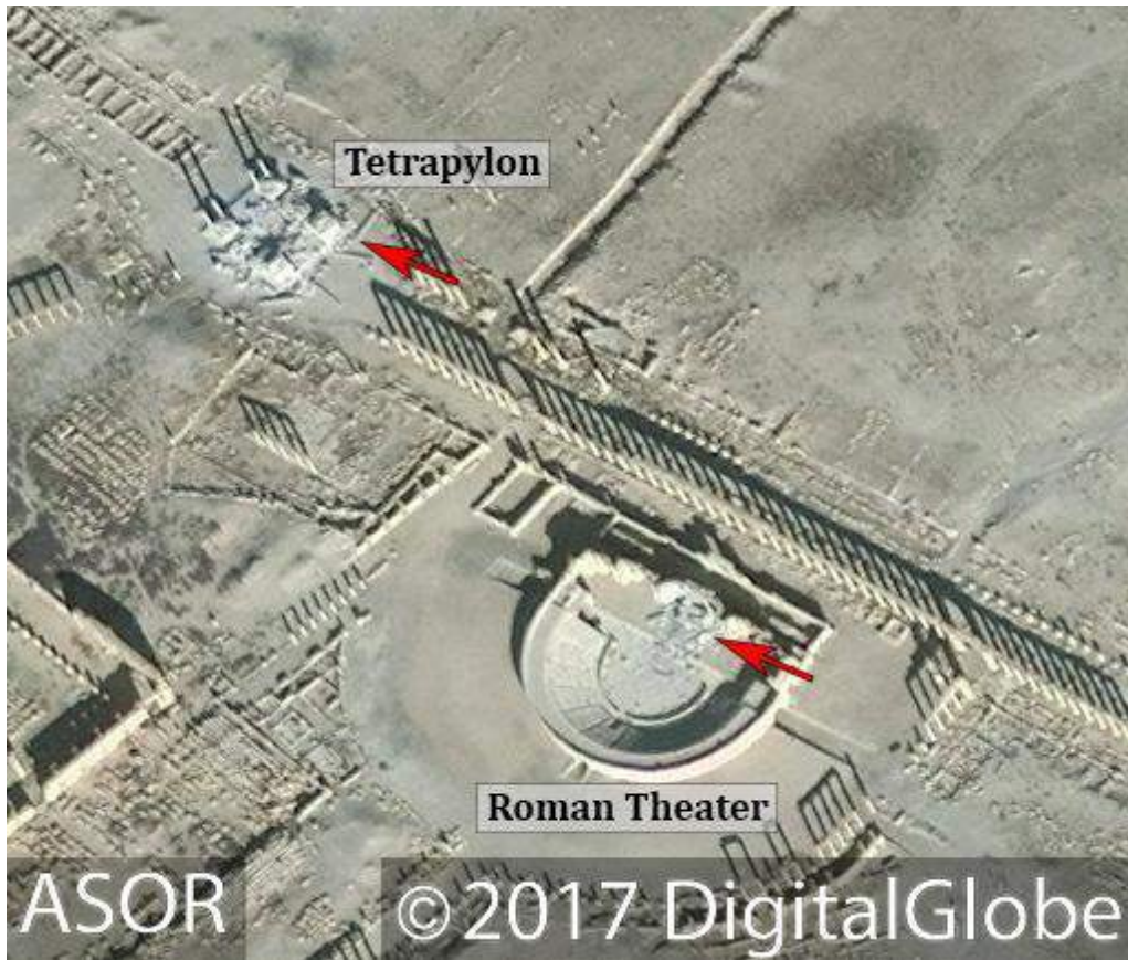
Significant damage to the Theater and Tetrapylon noted with red arrows (DigitalGlobe NextView License; January 10, 2017)
