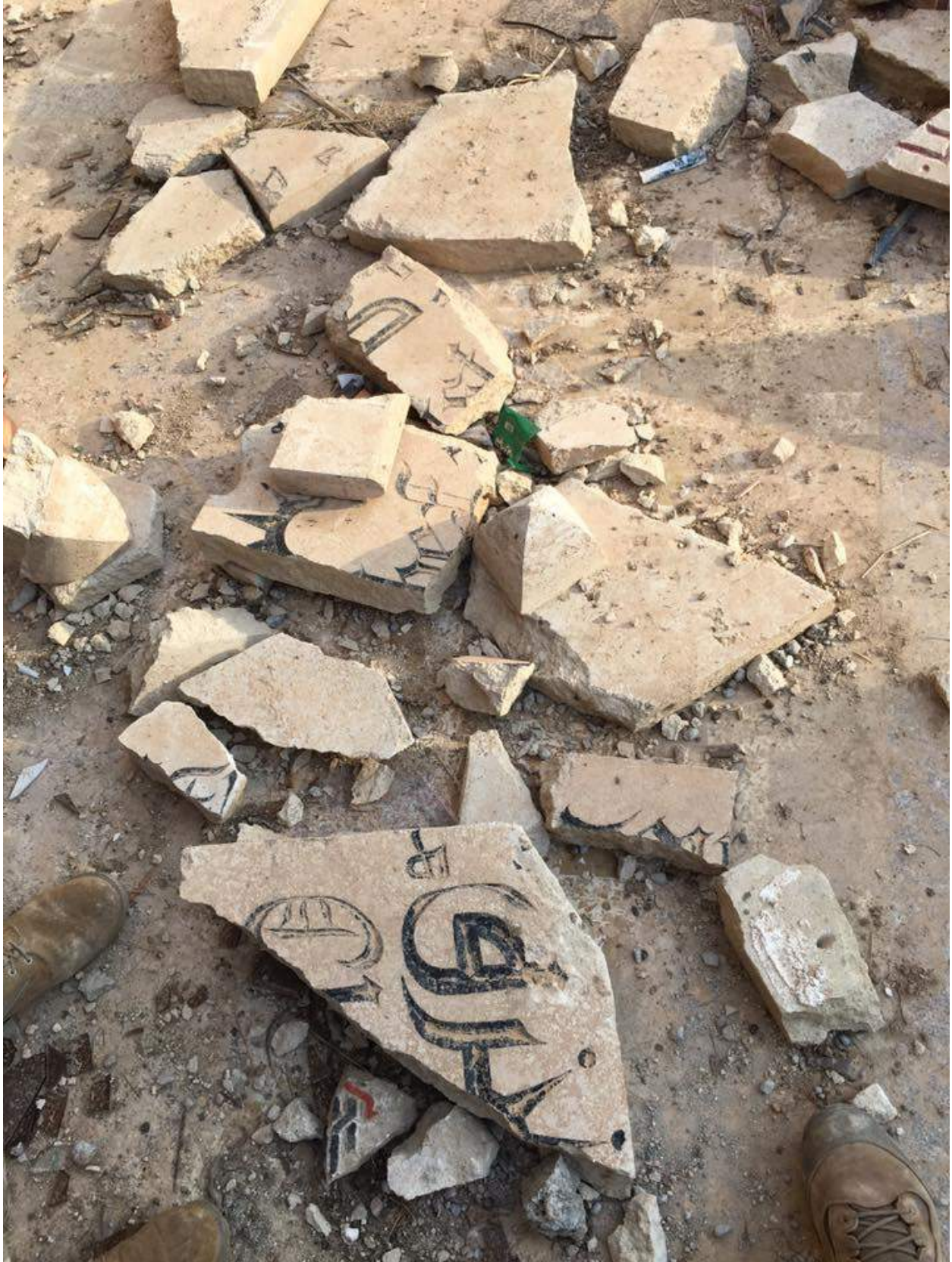
Damage to Mar Shmone Church (Twitter; January 22, 2017)
