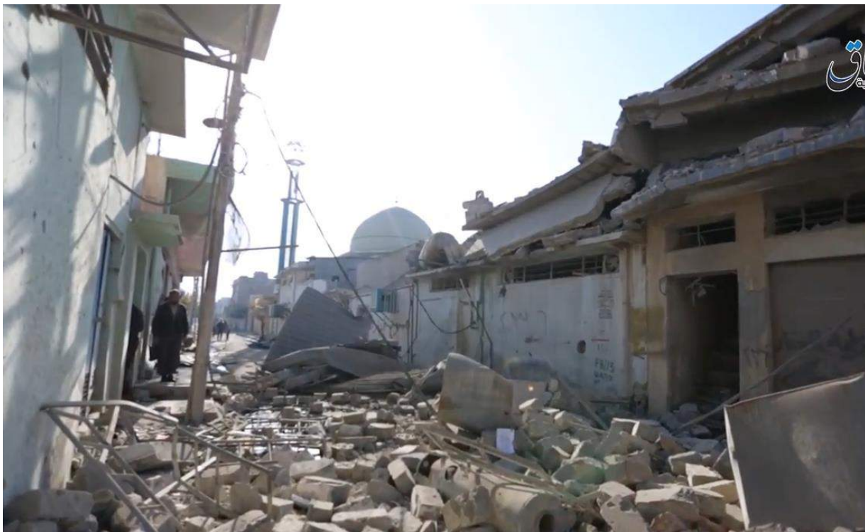
Video still of extensive damage to the area surrounding al-Khatib Mosque, the minaret and dome are seen in the background (Amaq News Agency; December 23, 2016)
