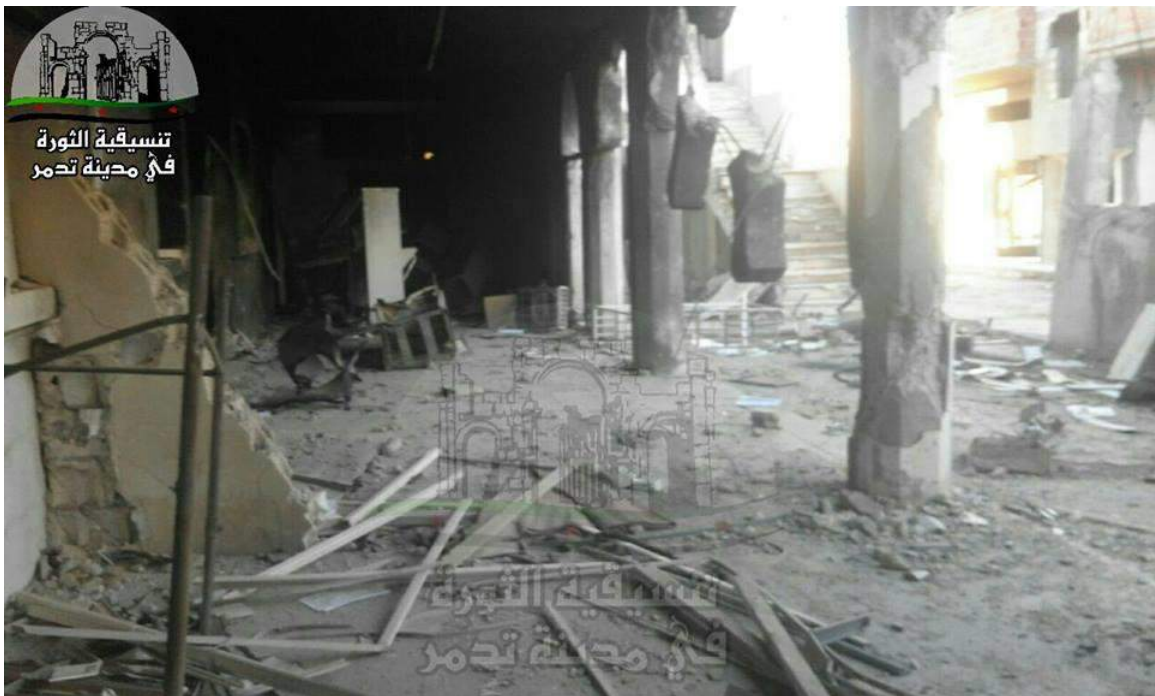
Severe damage to the structure of al-Eman Mosque (Palmyra Coordination; January 6, 2017)
