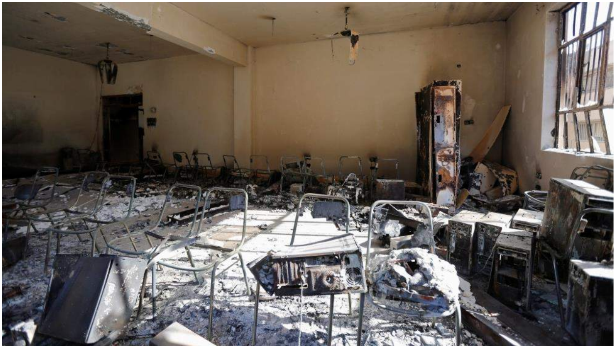
A heavily damaged classroom at Mosul University (Al Jazeera; January 26, 2017)
