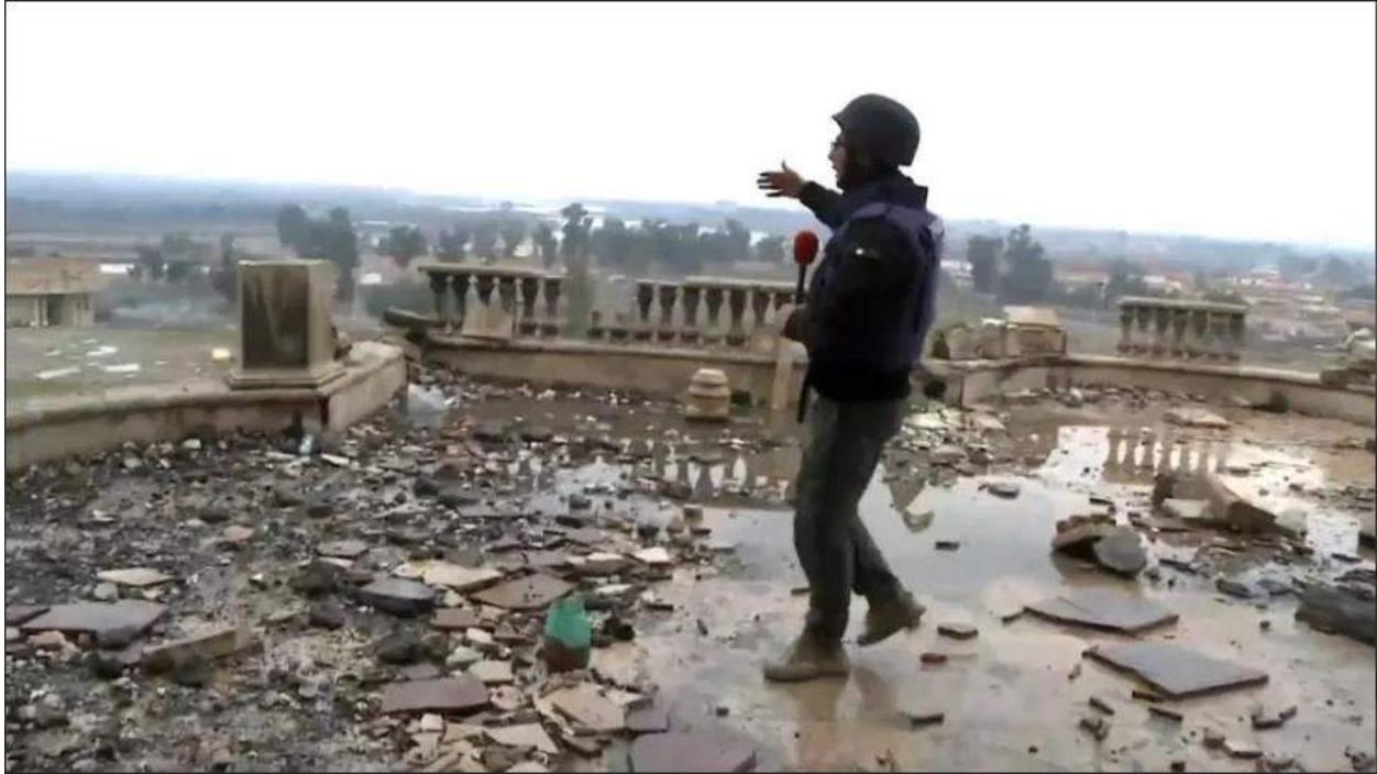
Video still of the roof of al-Remah Palace (The Sun/Rudaw; January 23, 2017)
