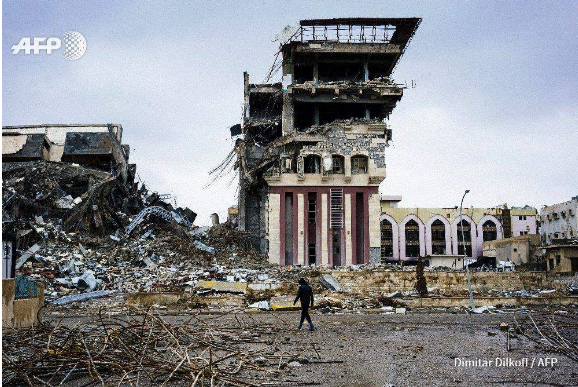
Damage to a building at Mosul University due to airstrikes (AFP; January 22, 2017)
