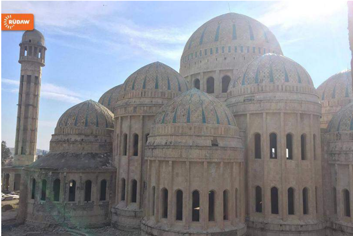
Damage to the exterior of the Grand Mosul Mosque (Rudaw; January 19, 2017)
