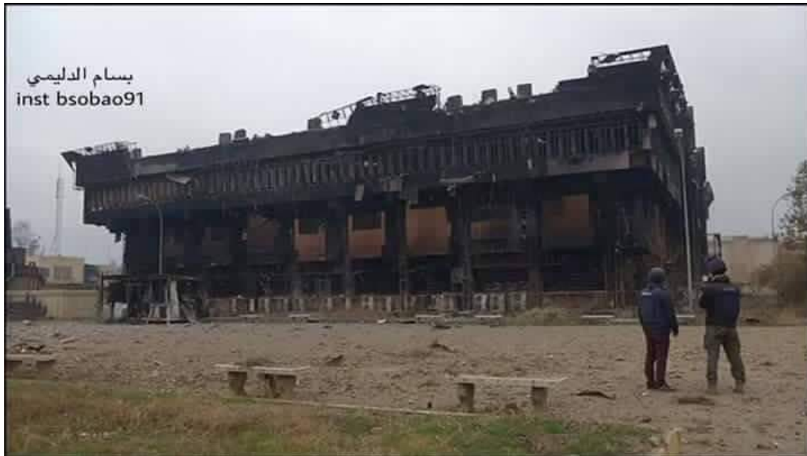
Damage to the Central Library at Mosul University (Mosul Eye; January 15, 2017)
