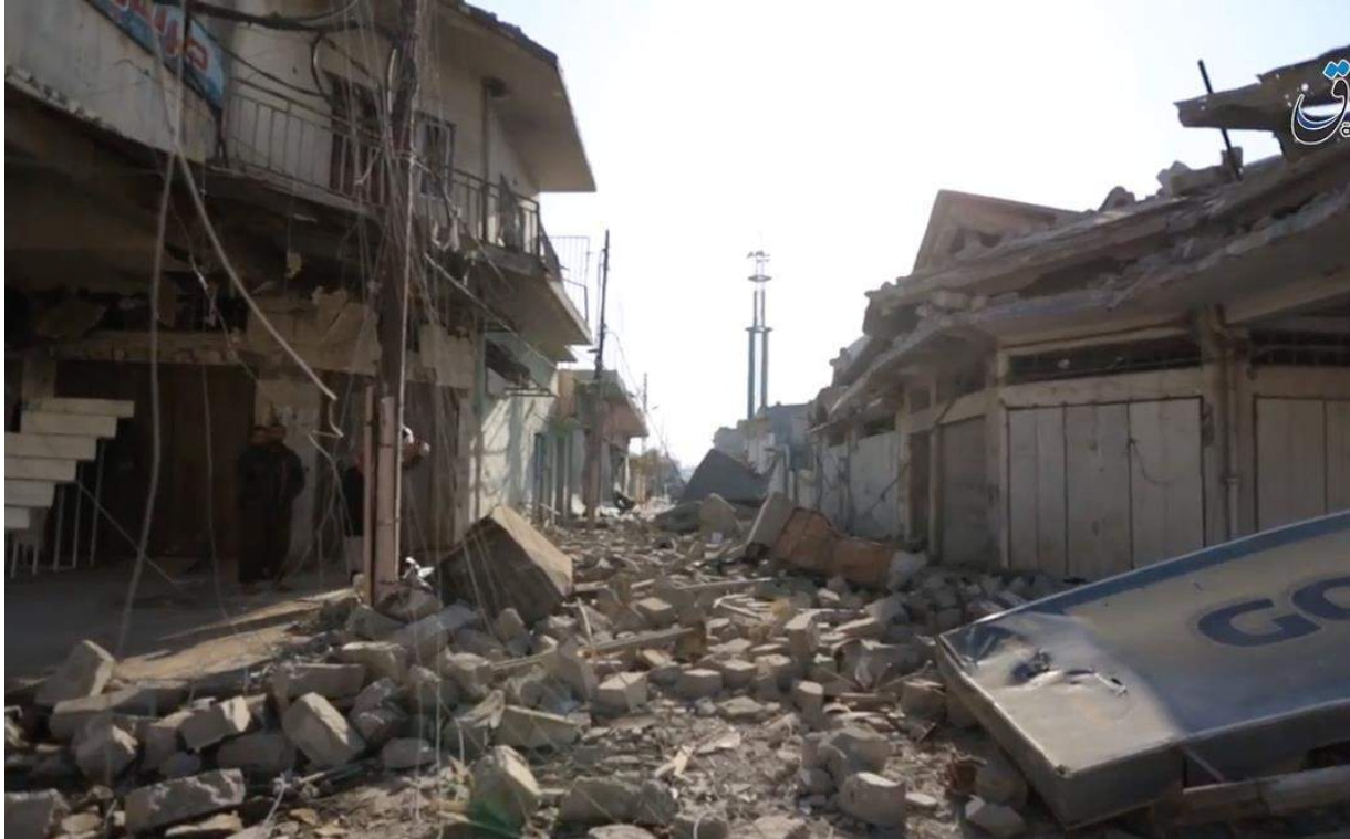
Video still of extensive damage to the area surrounding al-Khatib Mosque, the minaret is seen in the background (Amaq News Agency; December 23, 2016)
