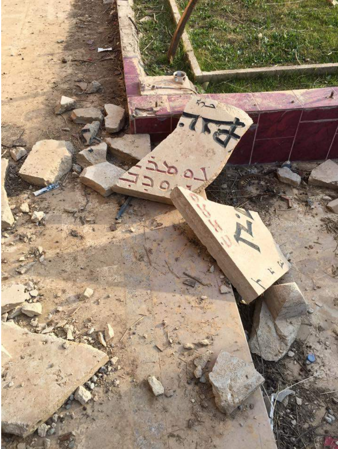
Damage to Mar Shmone Church (Twitter; January 22, 2017)
