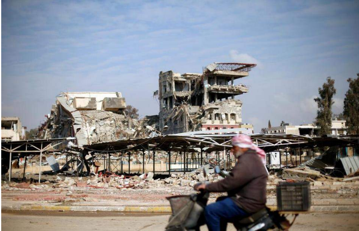
Damage seen at Mosul University (Reuters; January 31, 2017)
