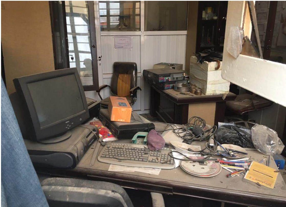
Damage seen inside a Mosul University building (W.G. Dunlop; January 16, 2017)
