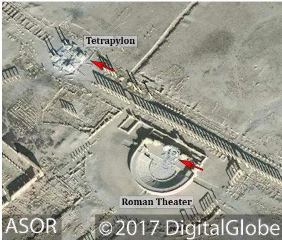
Significant damage to the Theater and Tetrapylon noted with red arrows (DigitalGlobe NextView License; January 10, 2017)
