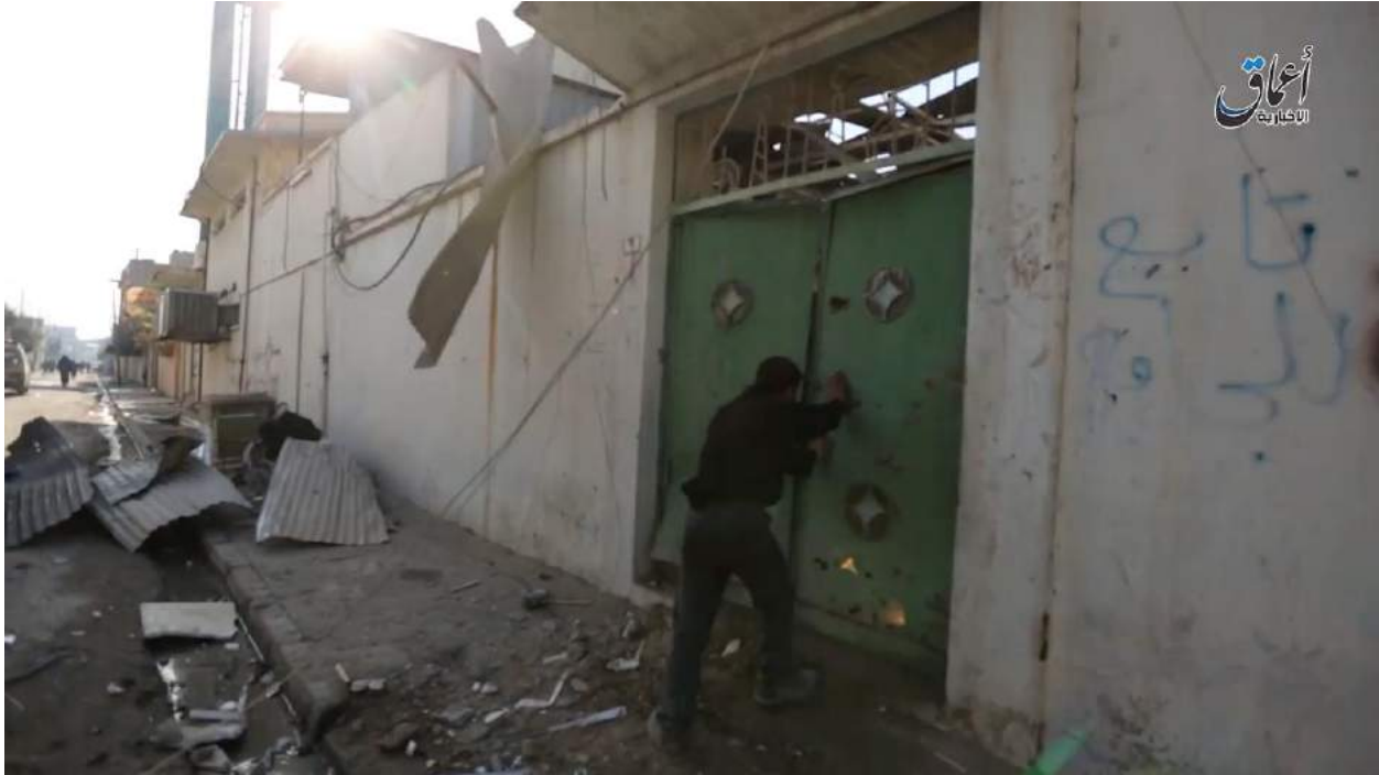
Video still of extensive damage to the area surrounding al-Khatib Mosque including the mosque's gate, the minaret is seen in the background (Amaq News Agency; December 23, 2016)
