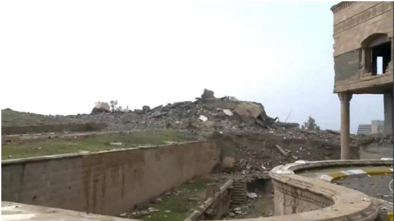
Video still showing complete destruction of outbuilding (The Sun/Rudaw; January 23, 2017)
