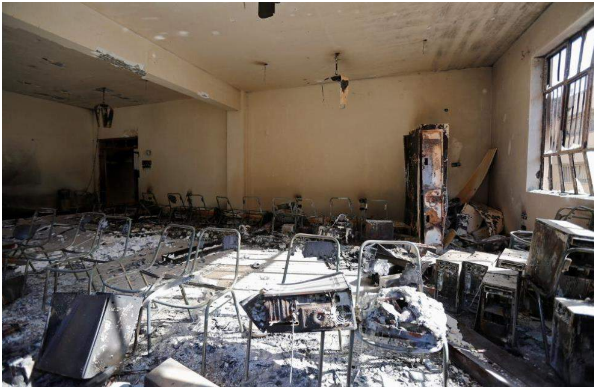
Damage to a classroom at Mosul University (Reuters; January 31, 2017)
