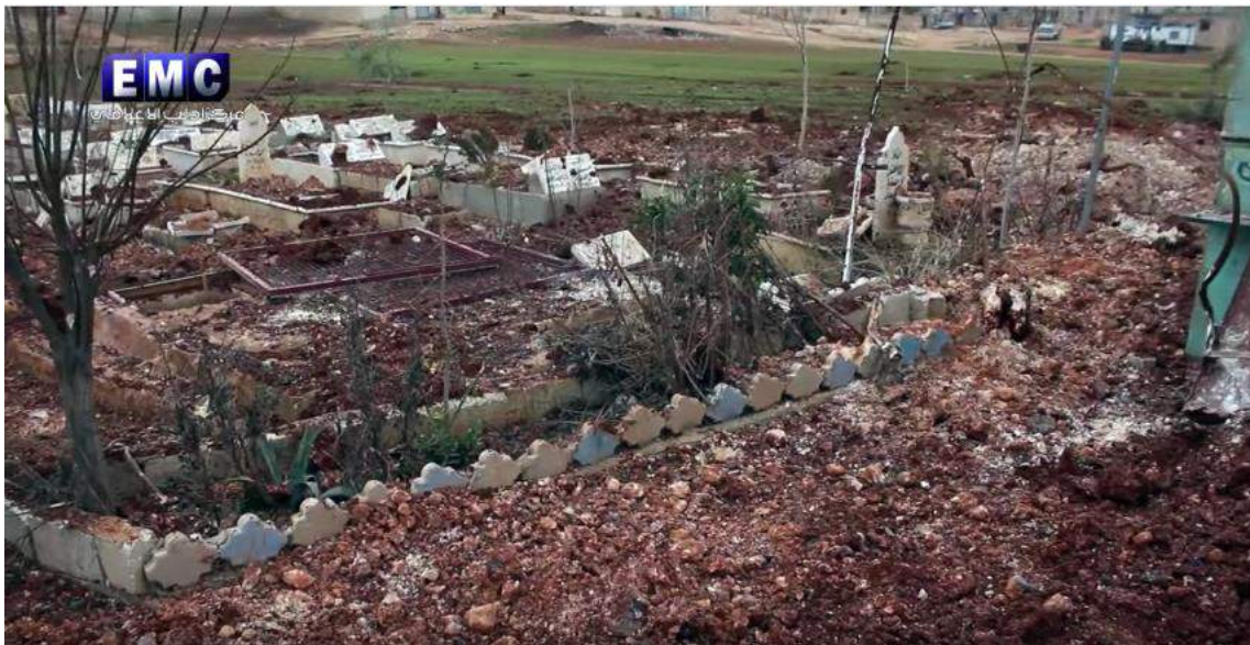
Video still of damage to the cemetery (Edlib Media Center; January 14, 2017)
