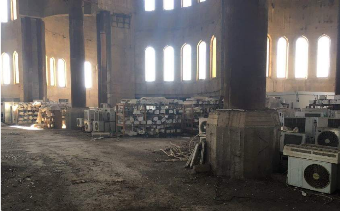
Air conditioners inside the unfinished Grand Mosul Mosque (W.G. Dunlop; January 20, 2017)
