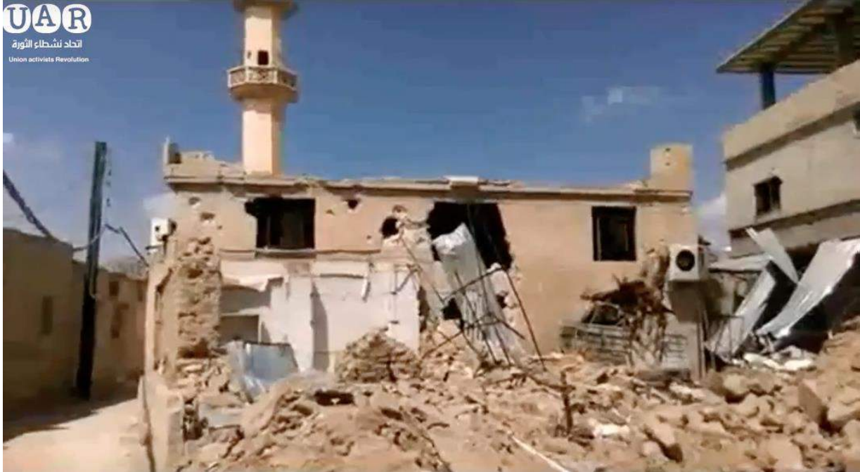
Video still of damage to al-Fateh Mosque (Union Activists Revolution; May 6, 2016)
