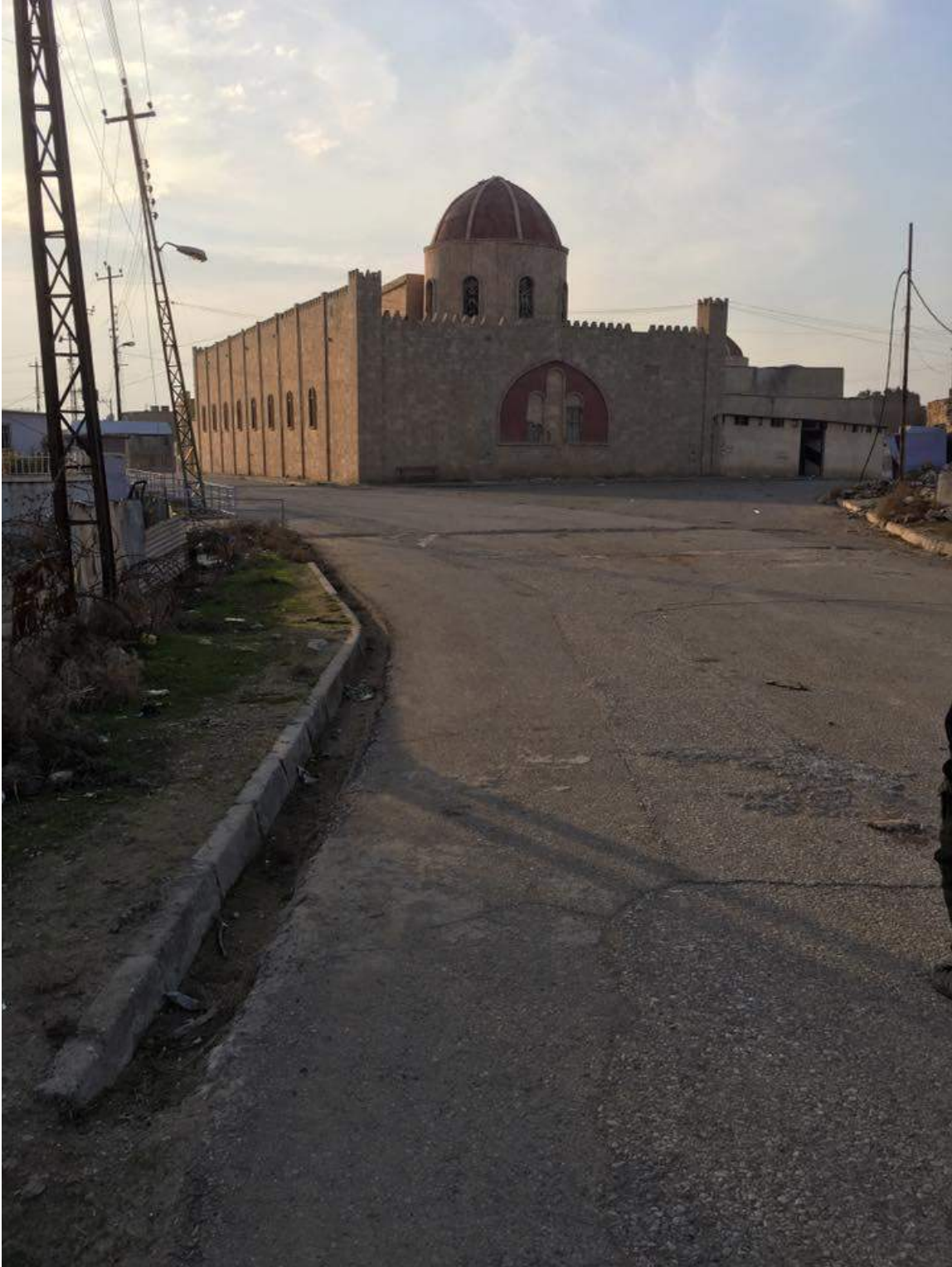
Another view of a damaged Sacred Heart Church (Twitter; January 23, 2017)
