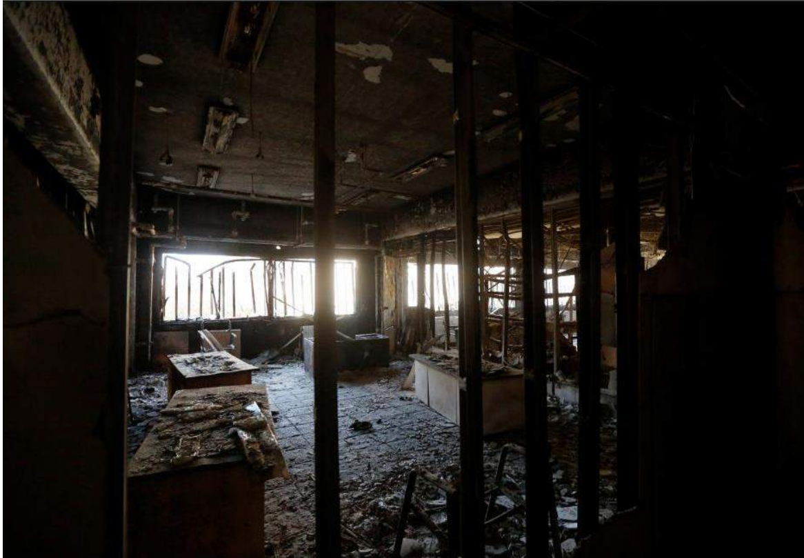
Fire damage to a classroom at Mosul University (Reuters; January 31, 2017)
