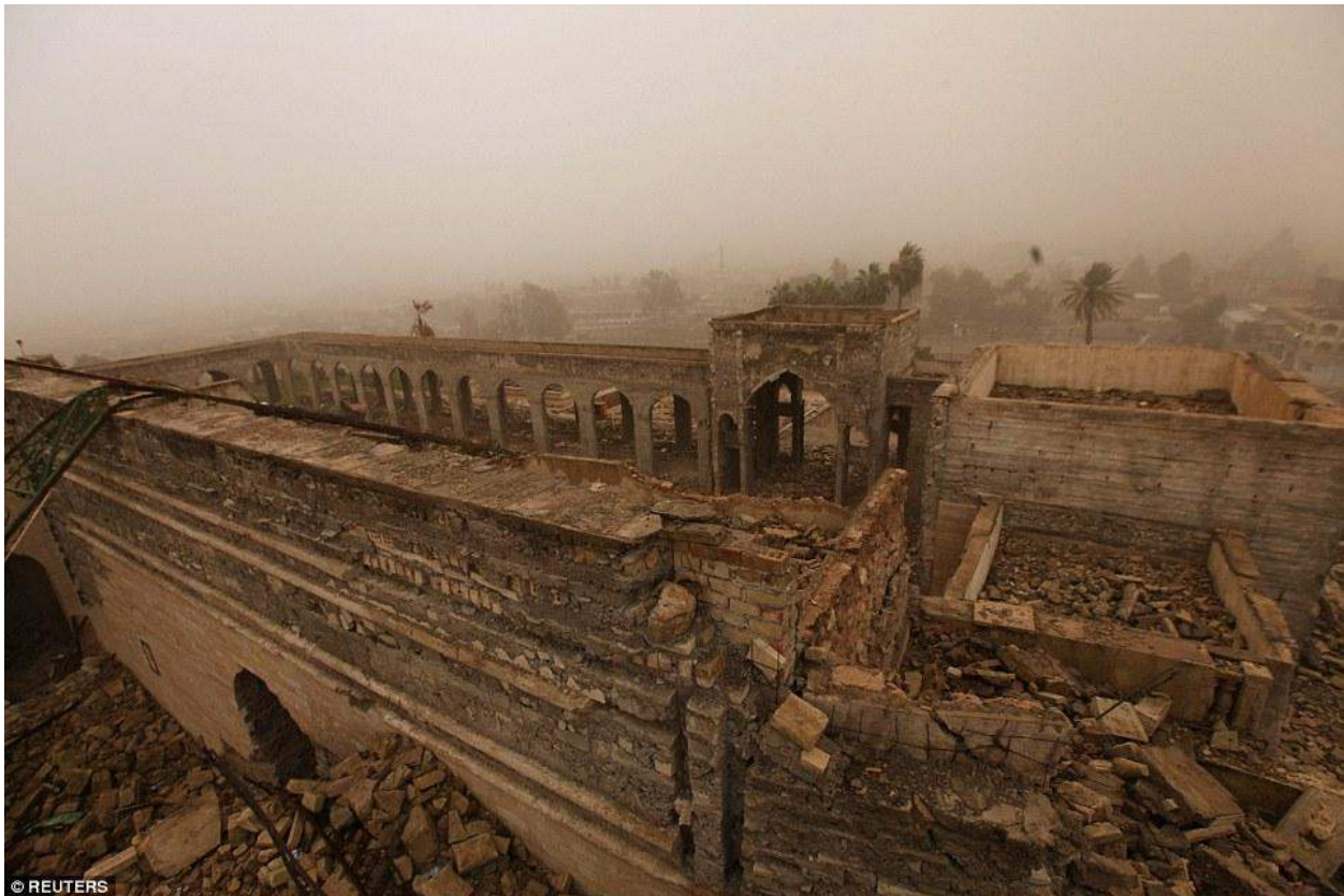
Damage to the Nebi Yunus Mosque Complex (Reuters/Daily Mail; January 28, 2017)
