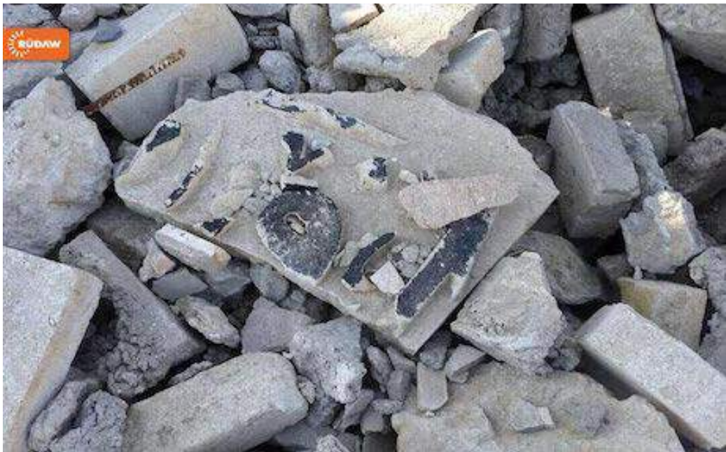
Damage seen inside the Nebi Yunus Mosque Complex (Rudaw; January 16, 2017)
