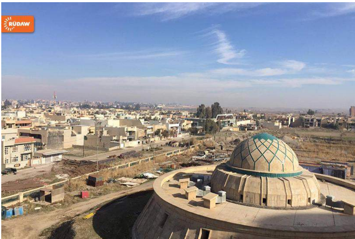
Damage to a mosque building (Rudaw; January 19, 2017)
