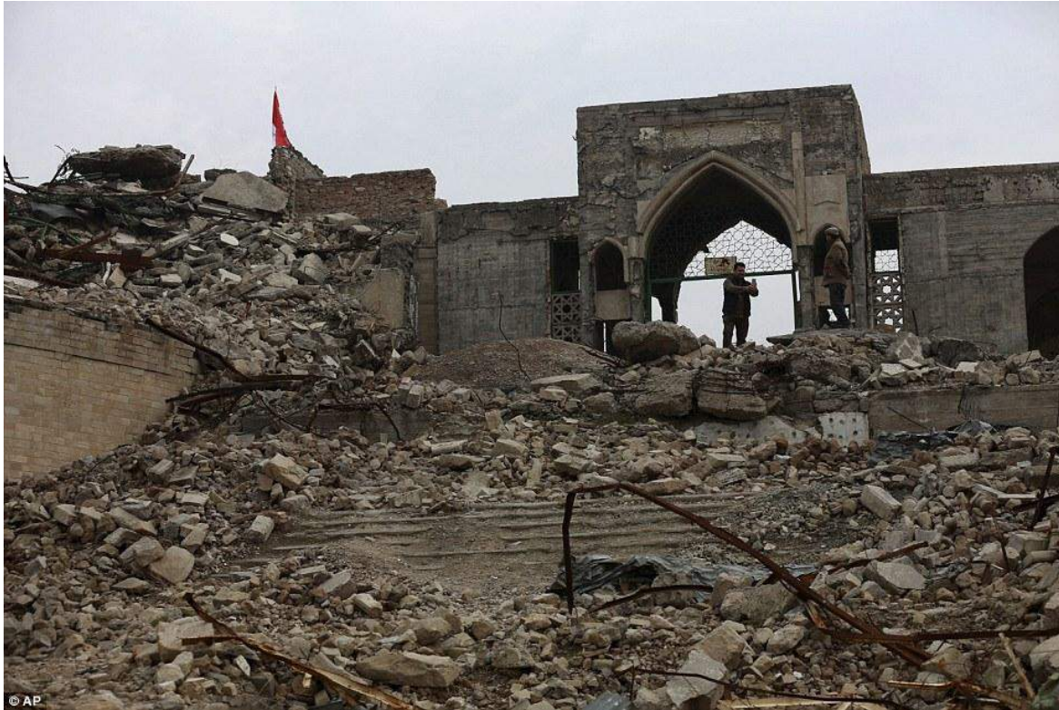
Damage to the Nebi Yunus Mosque Complex (AP/Daily Mail; January 28, 2017)
