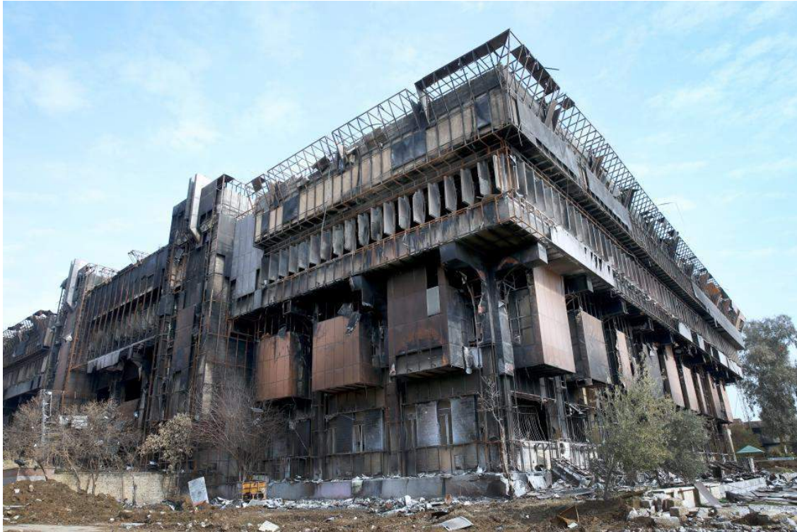
Damage to a building at Mosul University (Reuters; January 31, 2017)
