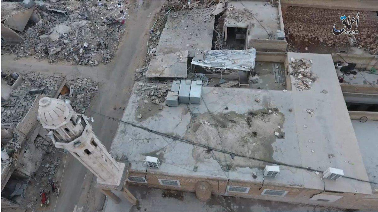
Video still of damage to al-Iman Mosque (Amaq Agency; January 2, 2017)
