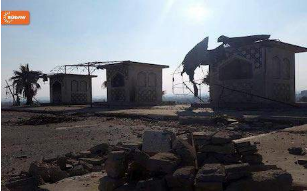
Damage seen inside the Nebi Yunus Mosque Complex (Rudaw; January 16, 2017)
