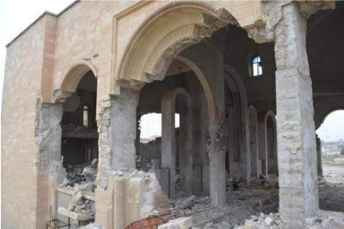
Damage to the side of the church showing missing walls and severe damage to area of altar (IshtarTV; February 10, 2017)
