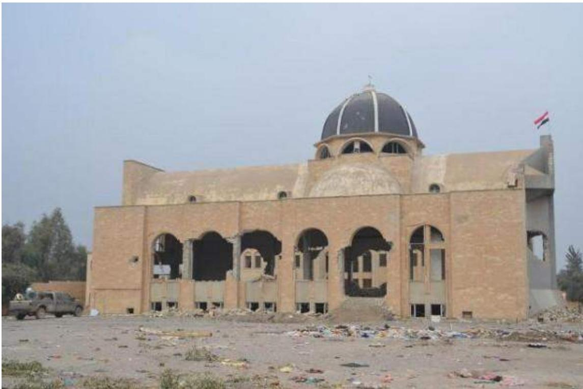
Damage to the side of the church showing missing walls (IshtarTV; February 10, 2017)
