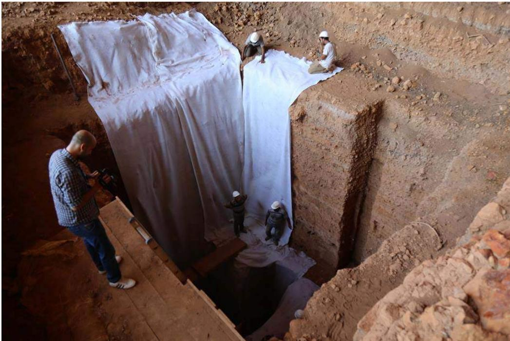
DoA staff place layer of geotextile to protect the exposed trench during reburial (DoA Shahat; August 13, 2017)
