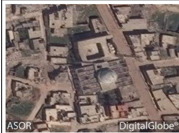
Abu Bakr al-Sadeiq Mosque with minor damage to the roof (DigitalGlobe; April 3, 2017)
