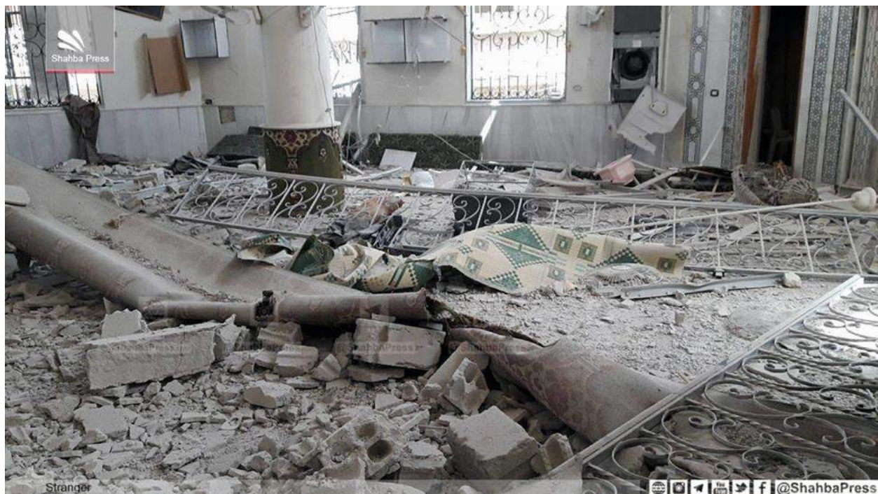
Damage to the interior of al-Sahabat al-Abrar Mosque mosque (SNHR; April 10, 2017)
