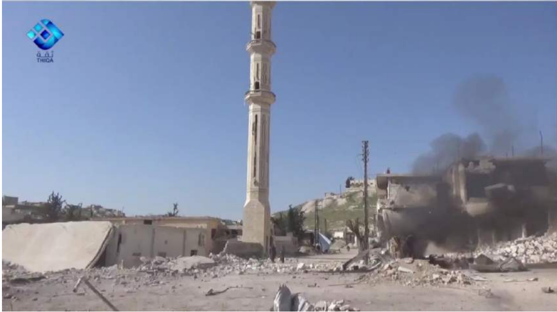
Video still of damage to al-Janubi Mosque in Lataminah showing collapsed roof and standing minaret (Thiqa News; April 6, 2017)
