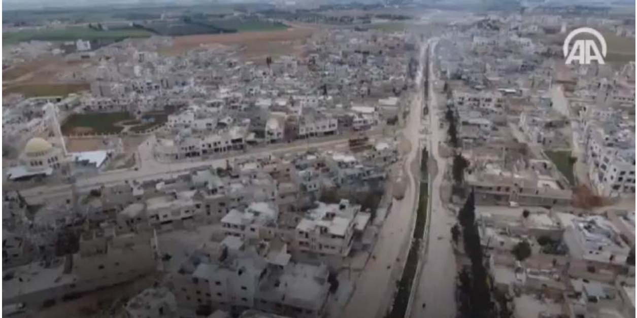
Video still of al-Bab showing the location of Zamzam mosque on left side of the image (Anadolu Agency; March 24, 2017)
