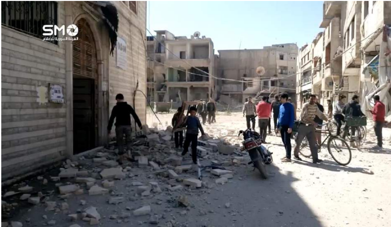
Video still of damage to the exterior of Arbin al-Kabir Mosque (SMO Syria; April 8, 2017)
