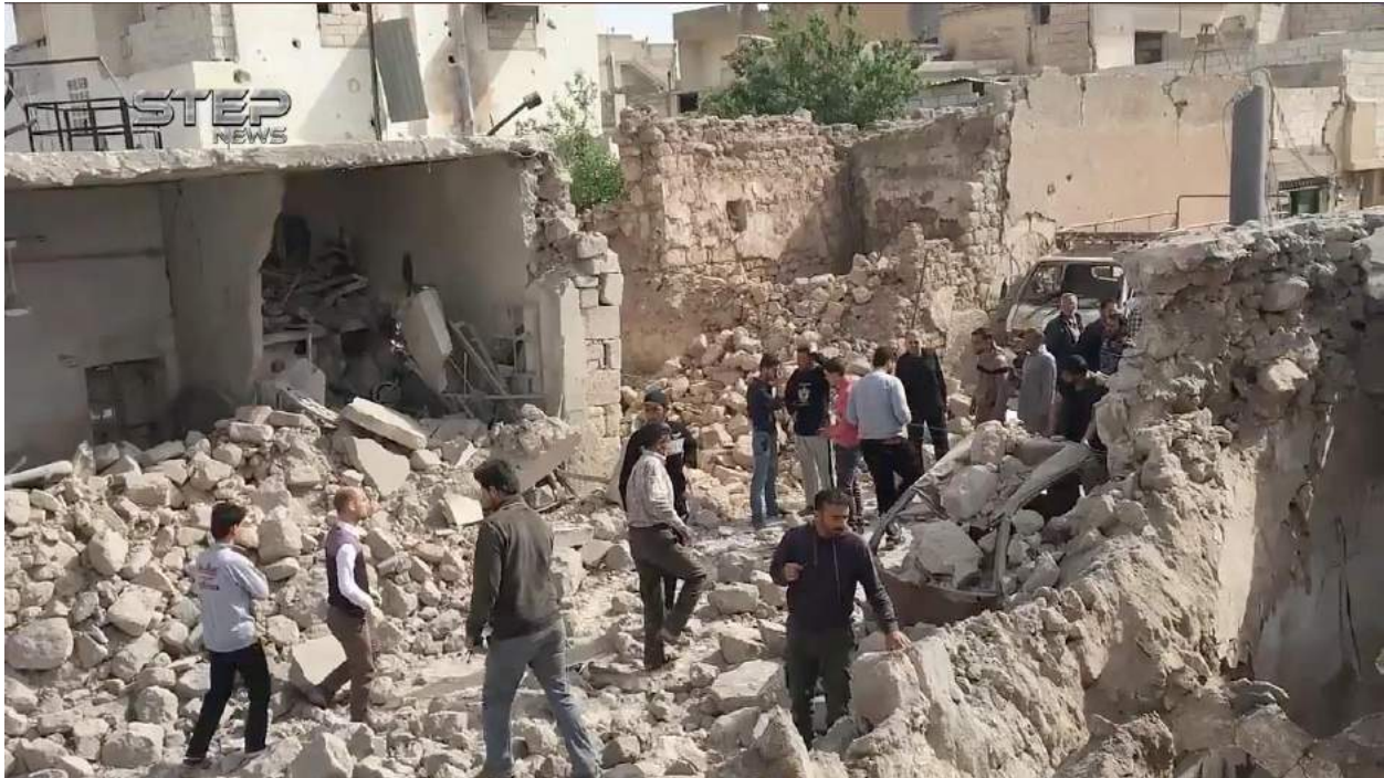
Video still of severe damage to Hammam al-Daraj al-Qadim (Step News Agency; April 27, 2017)
