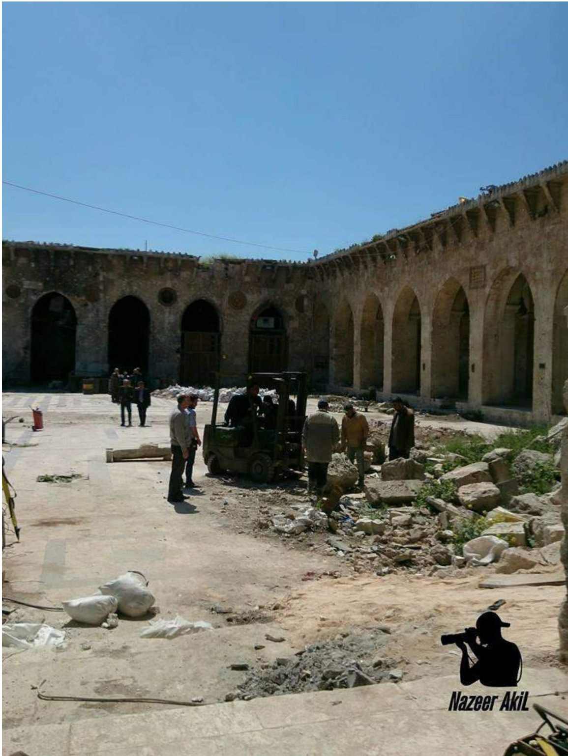
Clean-up efforts inside al-Umayyad Mosque (Aleppo Glory; April 3, 2017)
