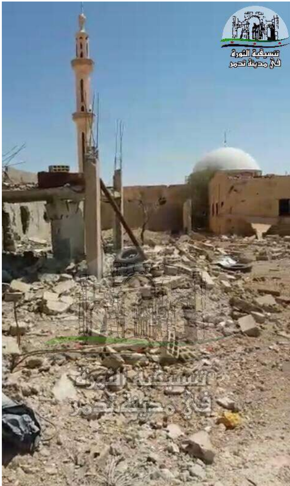
Damage to al-Amiriya Mosque (Palmyra Coordination Committee; April 23, 2017)
