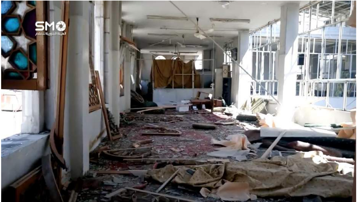
Video still of damage to the interior of Arbin al-Kabir Mosque (SMO Syria; April 8, 2017)
