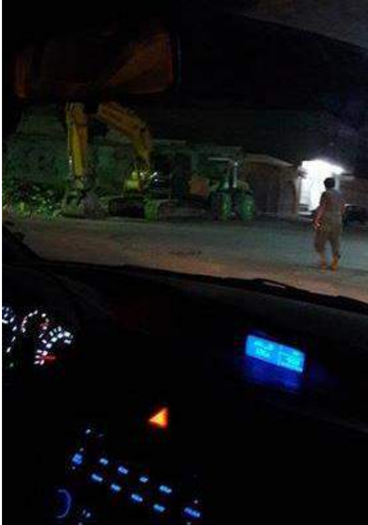
Heavy equipment has arrived on site to dig the foundations for the new building that will replace the Ben Halim house (ASOR CHI Sources; April 25, 2017)
