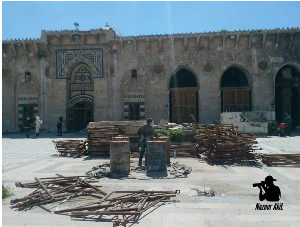
Clean-up efforts inside al-Umayyad Mosque (Aleppo Glory; April 3, 2017)
