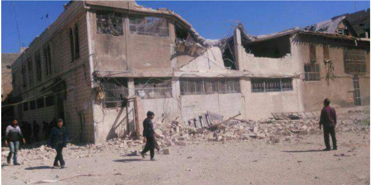
Damage to Arbin al-Kabir Mosque (Jobar News; April 7, 2017)
