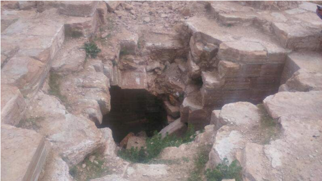
Damage to the Abu Jdari Tomb (DGAM; April 15, 2017)
