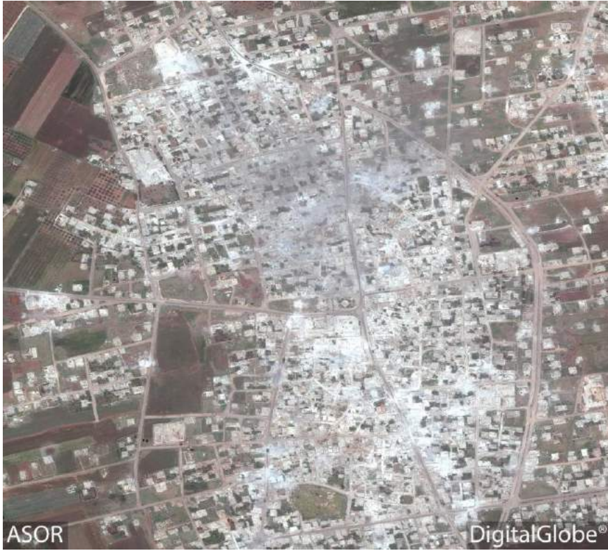
The severe damage to the city of Kafr Zaita since April 3, 2017 (DigitalGlobe; April 29, 2017)
