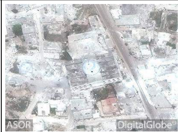
Abu Bakr al-Sadeiq Mosque with damage to the dome, courtyard, and surrounding areas (DigitalGlobe; April 29, 2017)
