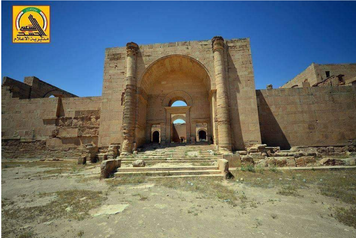
Damage and erosion at Hatra (Iraqi National Army/Twitter; April 27, 2017)
