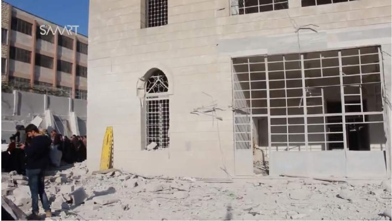
Video still shows damage to al-Rawda Mosque (Salqin City Coordination; April 7, 2017)
