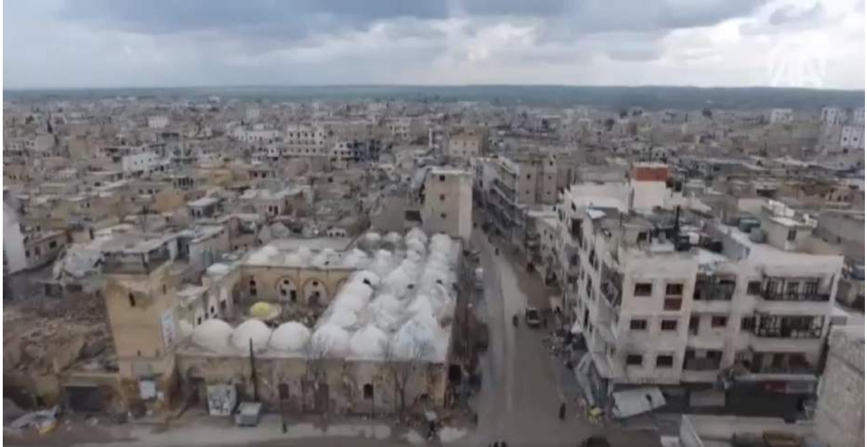
Video still of al-Kabir mosque showing damage to the domes (Anadolu Agency; March 24, 2017)
