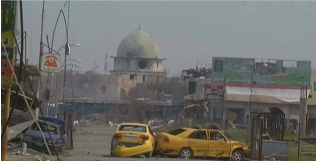
Video still of damage to the dome of al-Nuri al-Kabir Mosque (France 24; April 19, 2017)
