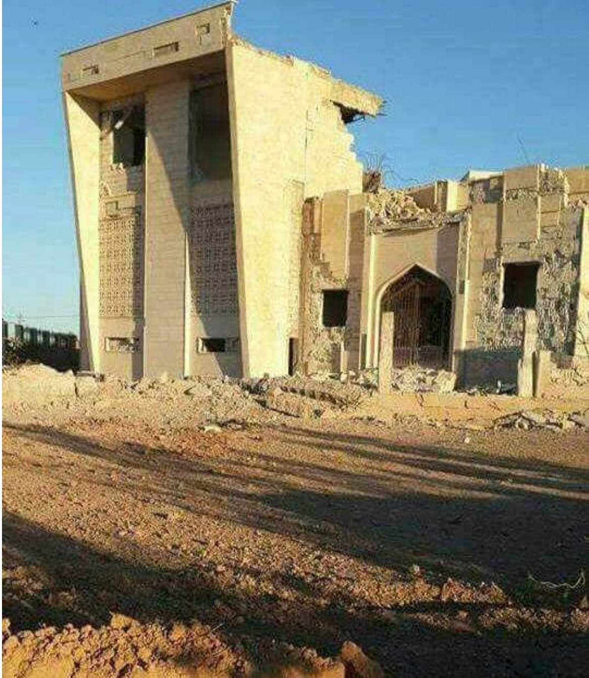
Damage to the cultural center (RBSS; April 26, 2017)
