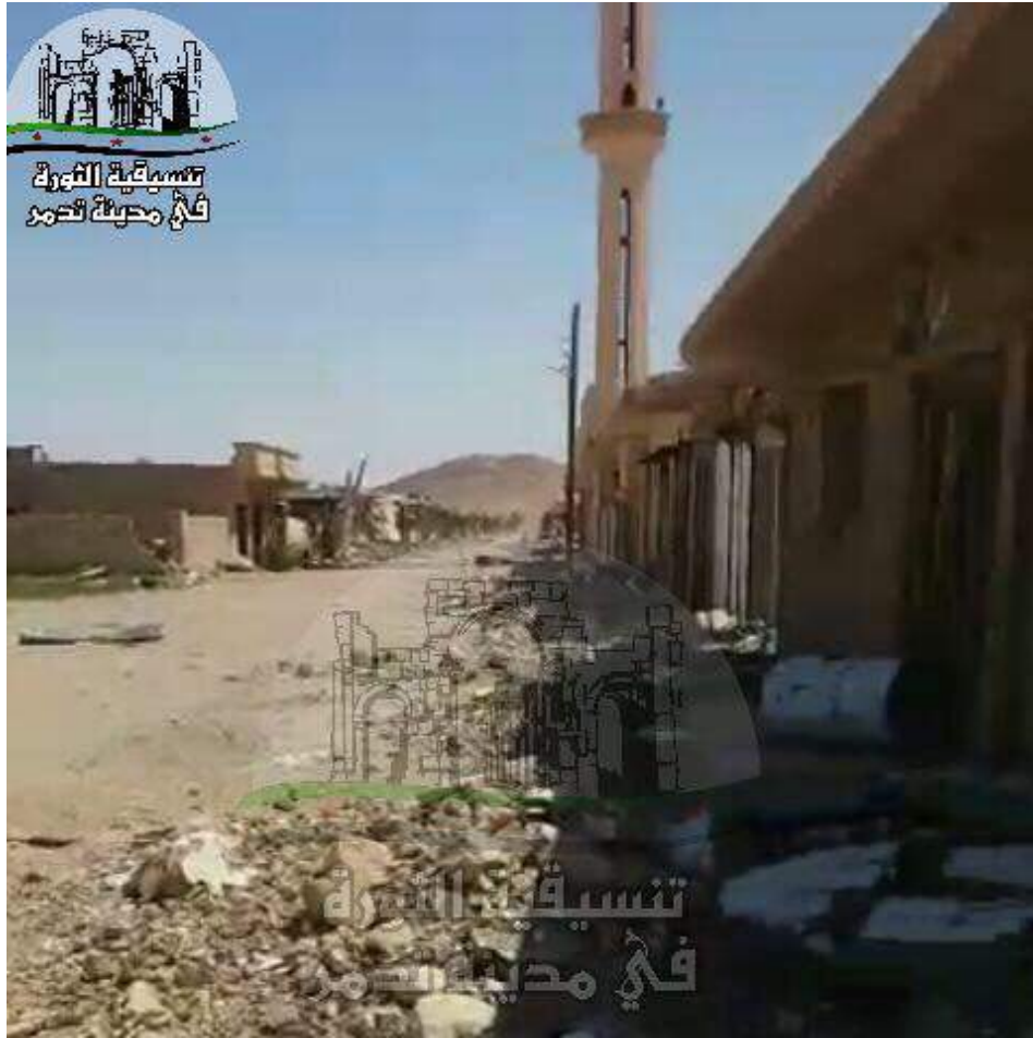
Damage to al-Amiriya Mosque (Palmyra Coordination Committee; April 23, 2017)
