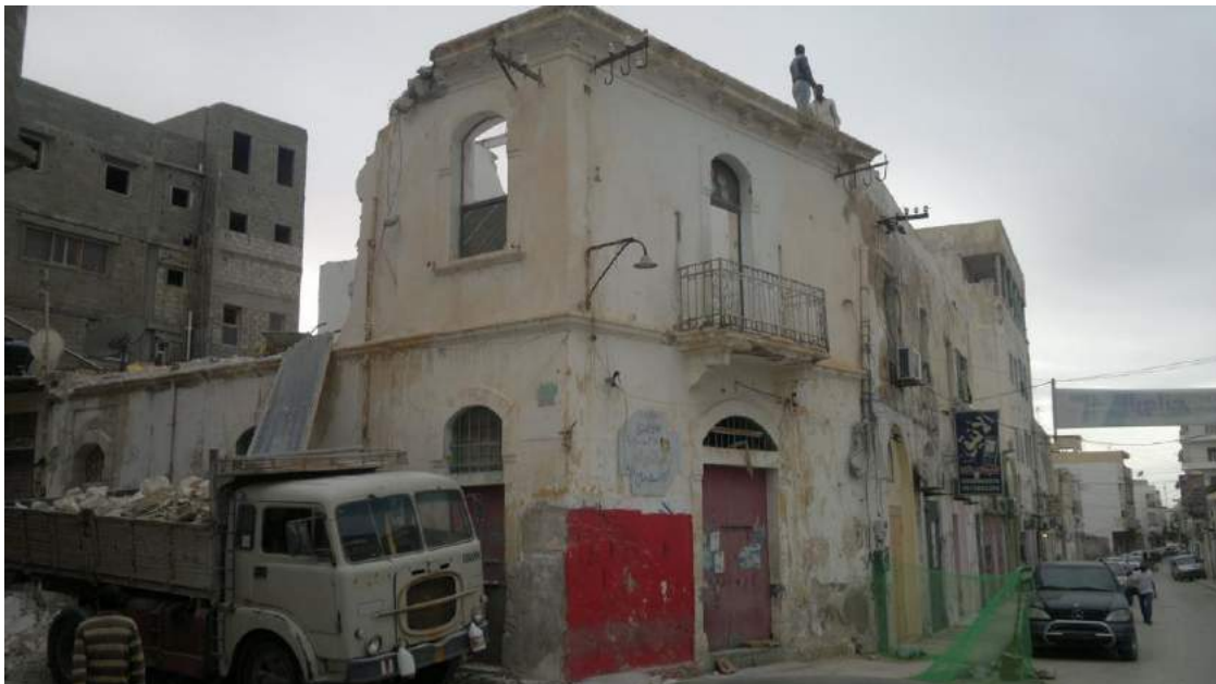
Ben Halim house being dismantled (ASOR CHI Sources; April 2017)
