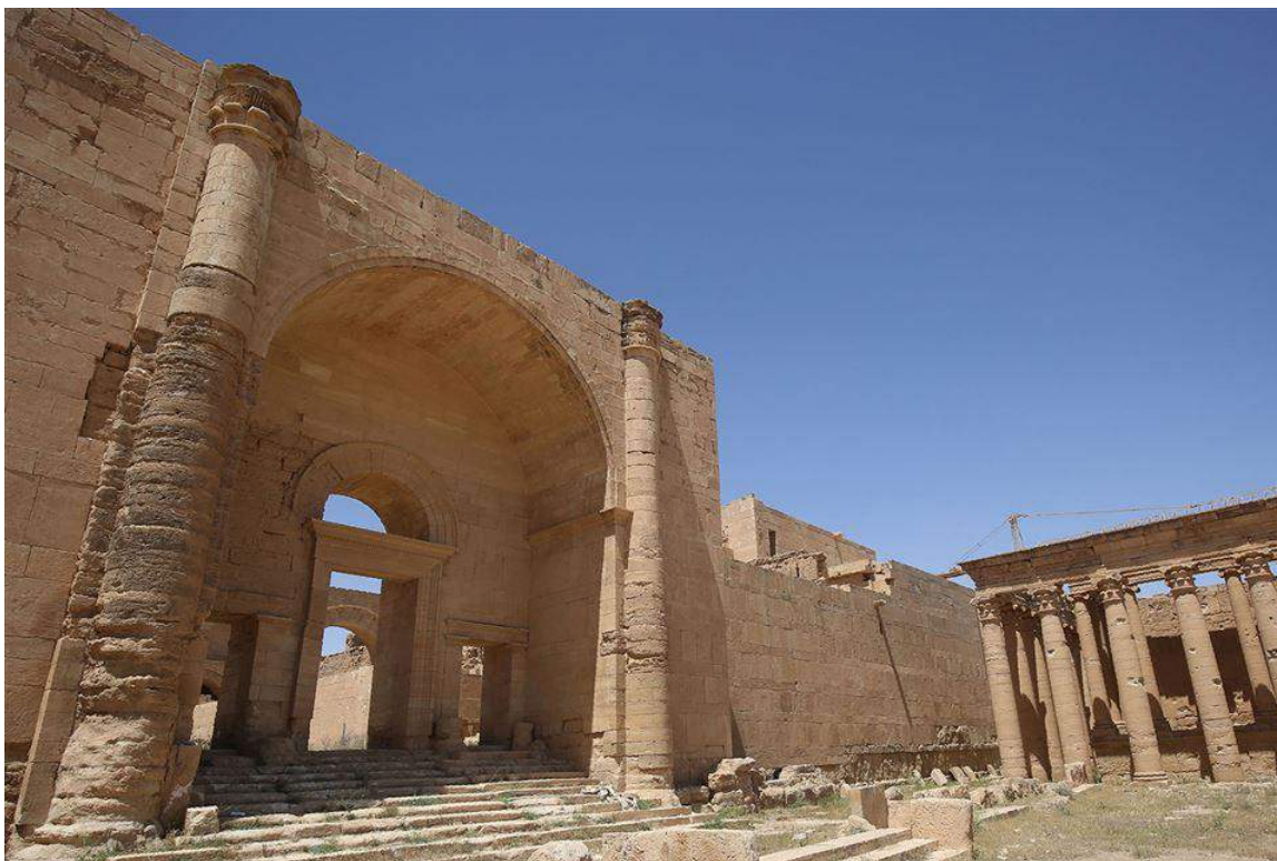
Damage and erosion at Hatra (Art Daily; April 27, 2017)
