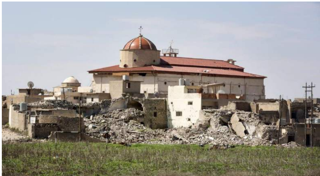
Damage surrounding Mar Qoryaqos Church (The Ferret; April 13, 2017)
