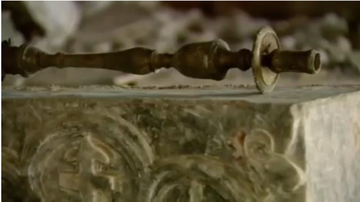
Video still of damage to the altar inside the Church of King Jesus (Sky 1; February 2016)
