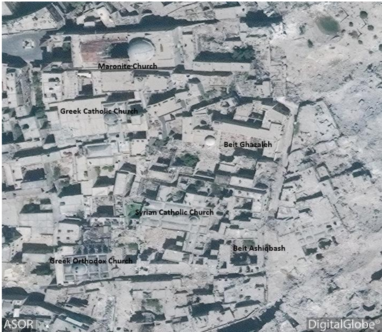
Jdeide Quarter with damage to multiple buildings due to tunnel bombs (DigitalGlobe; August 18, 2015)
