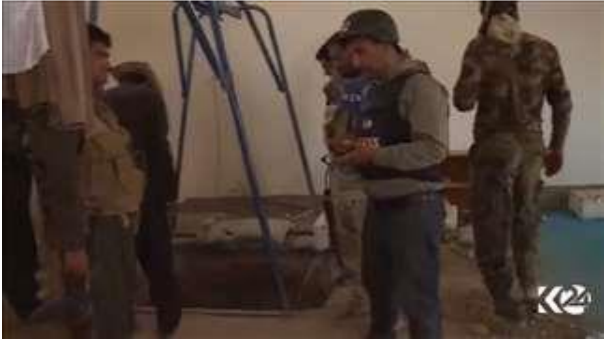
Pulley-system for dirt removal above large tunnel inside mosque (Kurdistan 24; August 21, 2016)
