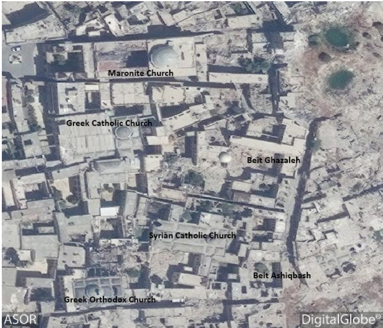
Jdeide Quarter with damage to multiple buildings due to tunnel bombs (DigitalGlobe; August 19, 2016)
