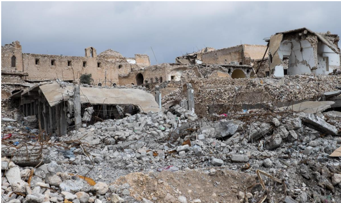
Damage surrounding the Church of King Jesus (Courtesy of Preemptive Love Coalition; February 25, 2016)
