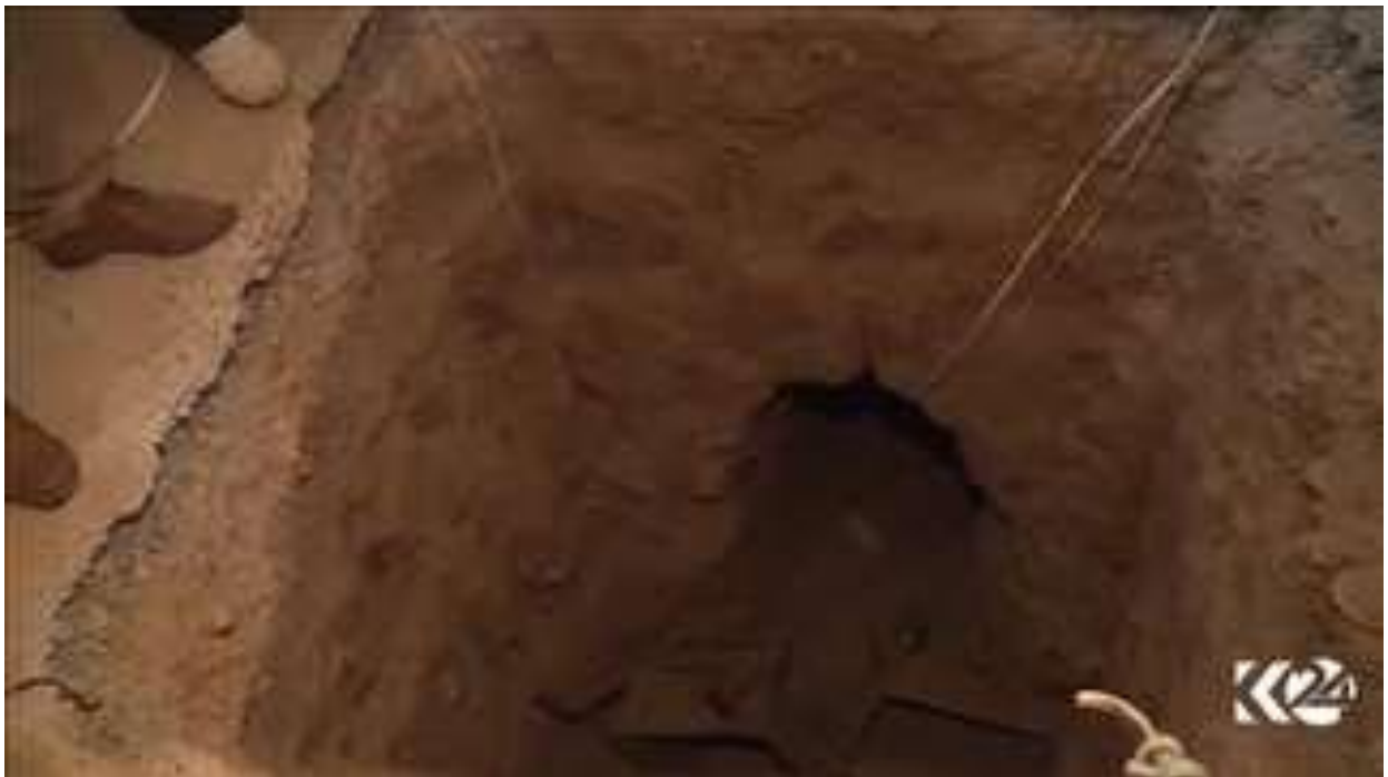
Large hole and tunnel inside mosque (Kurdistan 24; August 21, 2016)
