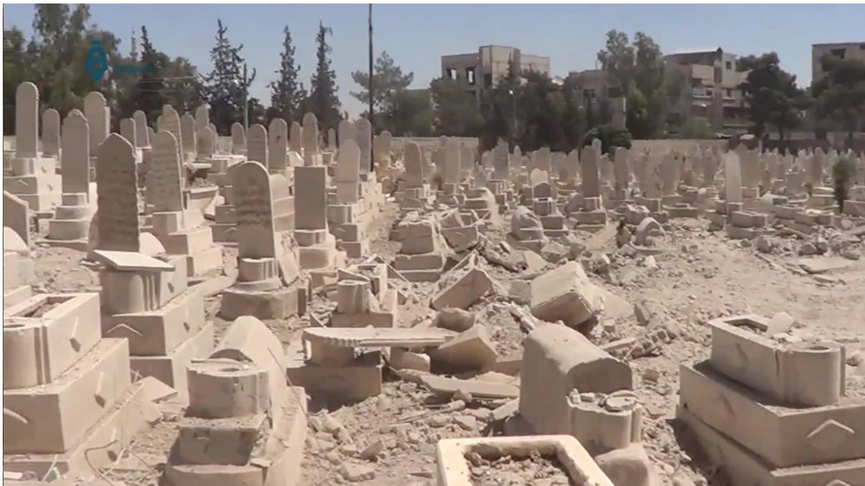
Video still of damage to Arbin Cemetery (Qasioun News Agency; August 18, 2016)
