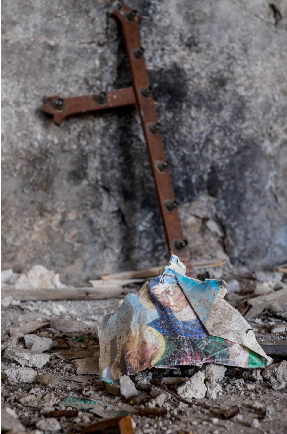
Detail of damage to a cross and religious materials inside the Church of King Jesus (Courtesy of Preemptive Love Coalition; March 30, 2016)
