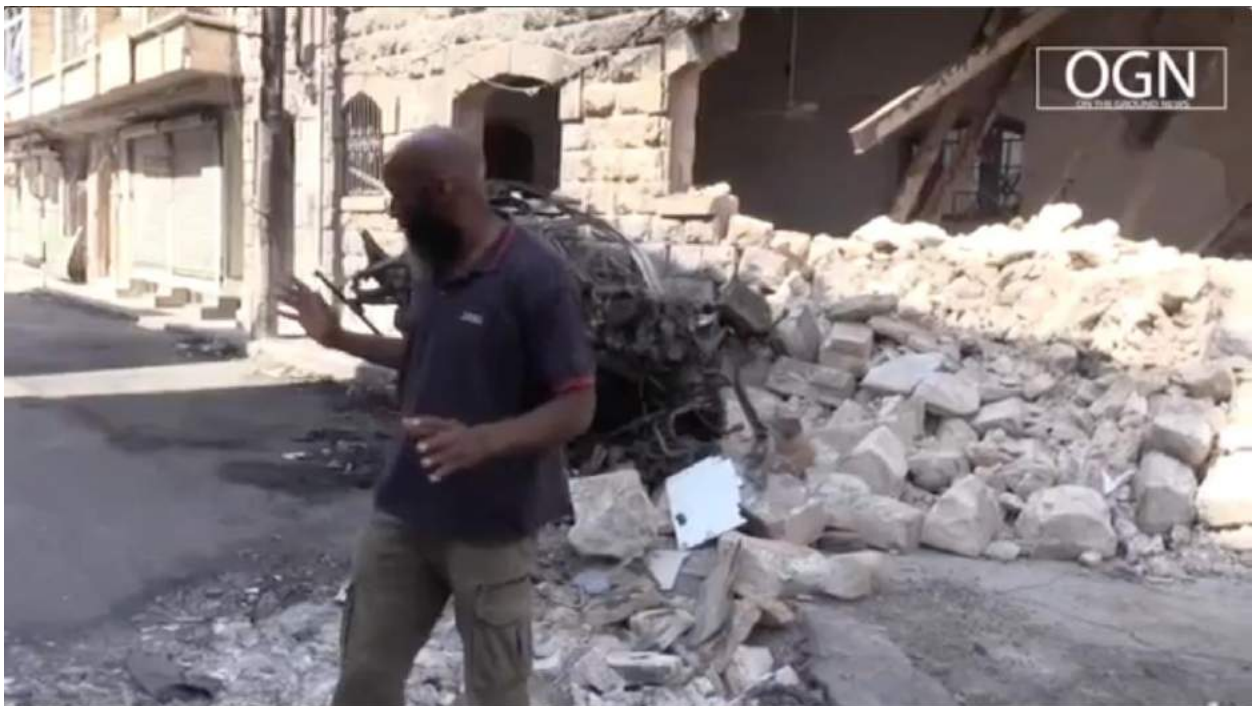
Video still of damage and debris surrounding the church (OGN; August 16, 2016)
