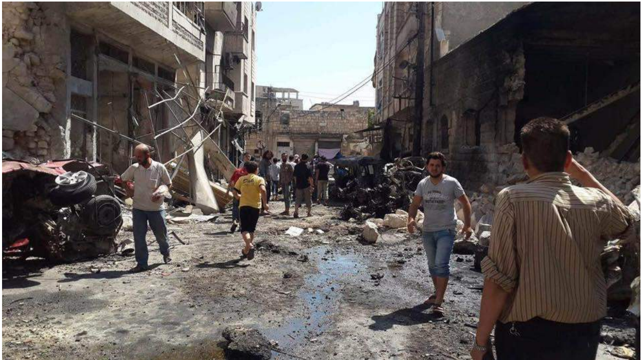
Damage to the street outside of the church (Facebook; August 10, 2016)
