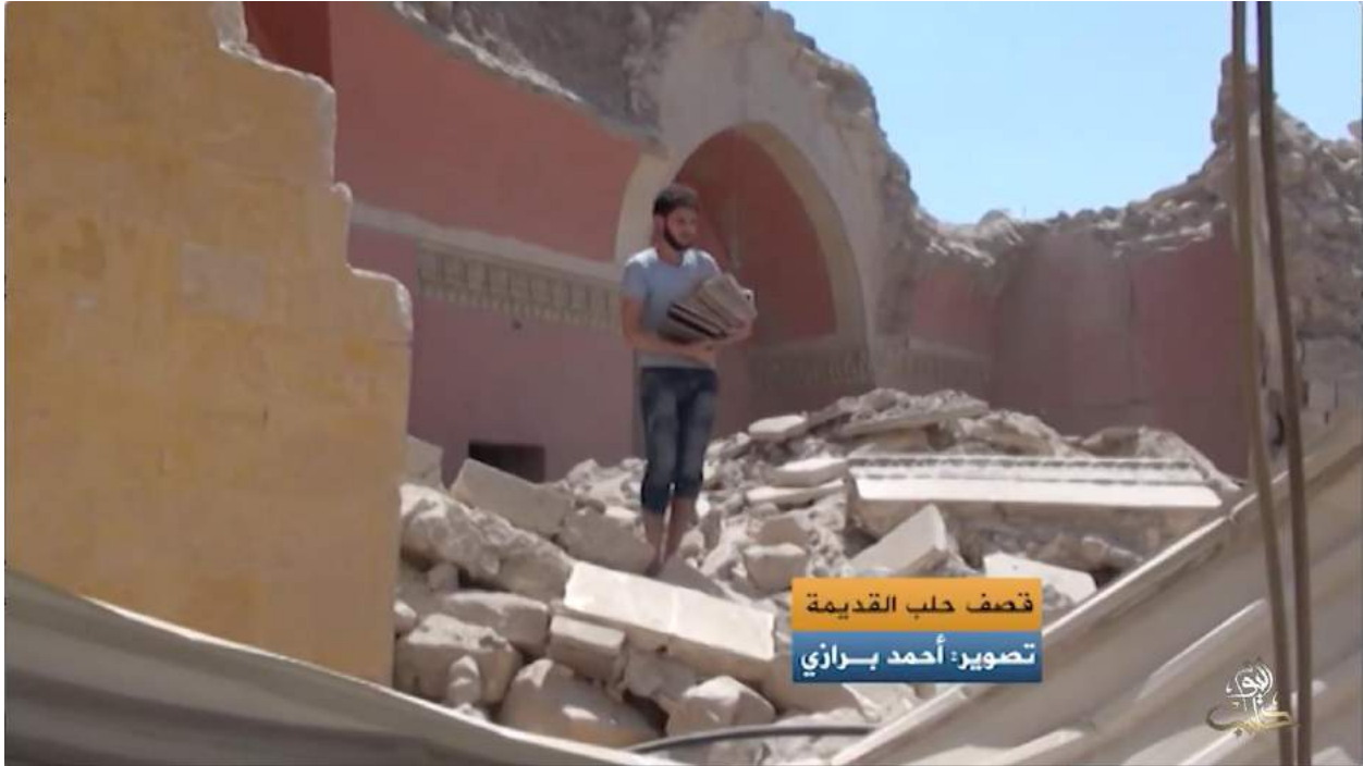
Video still showing extensive damage to Waraqa Cultural Center as an individual removes damaged books from the rubble (Halab Today TV; August 15, 2016)
