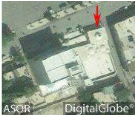
Old Hammam prior to painting of the dome (DigitalGlobe; April 4, 2014)
