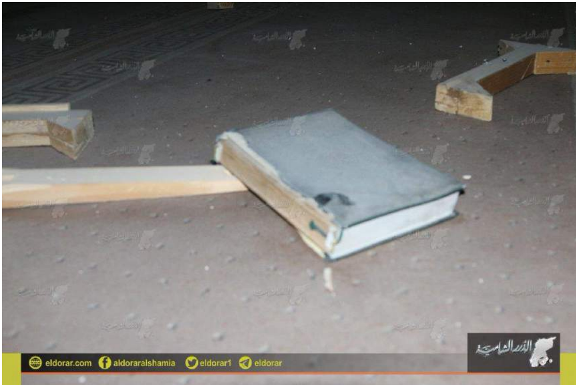
Material damage in al-Kabir Mosque (Al Dorar Al Shamia; August 8, 2016)
