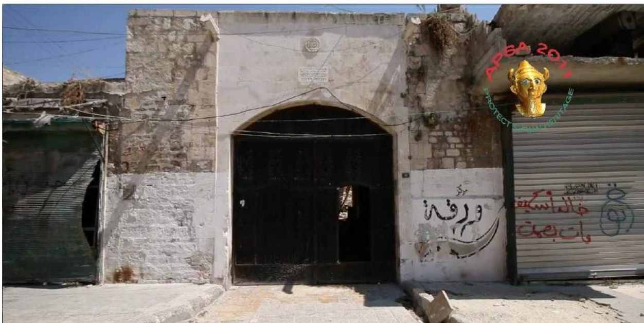
Video still of what is likely the entrance to Waraqa Cultural Center following damage to the building (APSA; August 16, 2016)
