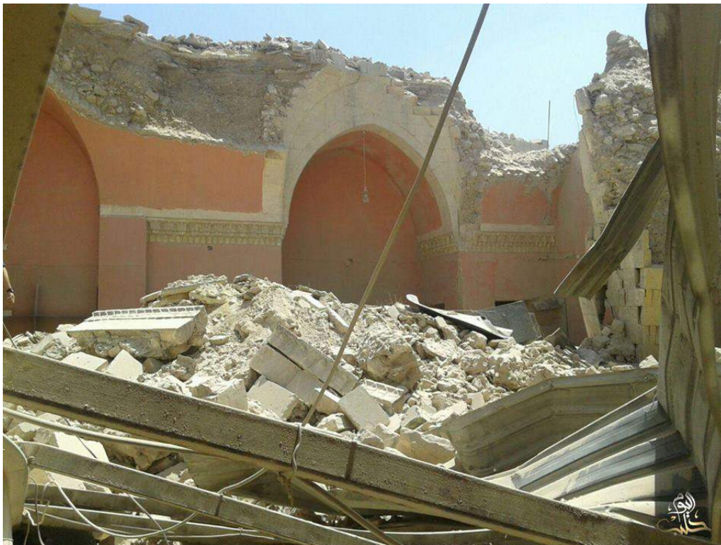
Extensive damage to Waraqa Cultural Center (Halab Today TV; August 15, 2016)
