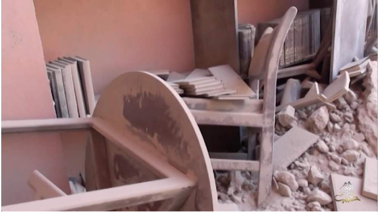
Video still of damage to the library at Waraqa Cultural Center (Halab Today TV; August 15, 2016)
