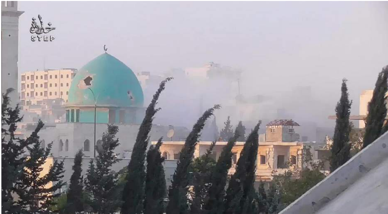
Video still of damage of the dome of al-Bara bin Malek Mosque (Step News Agency; August 15, 2016)
