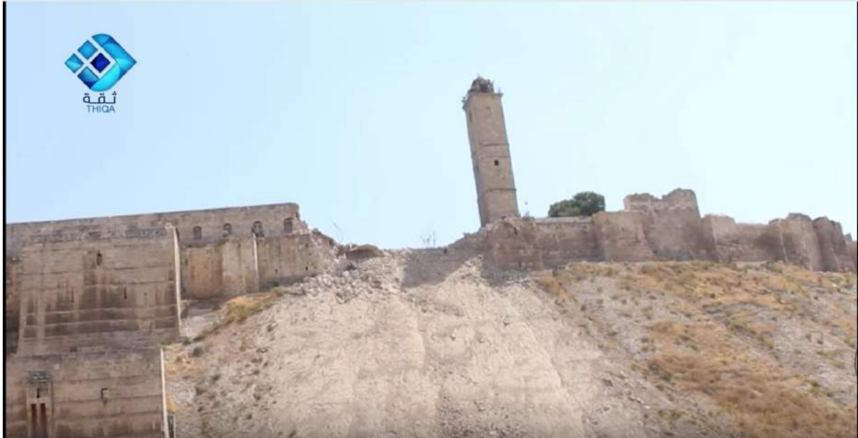
Video still of the damage to the northern side of the Citadel of Aleppo (Thiqa News Agency; August 11, 2016)
