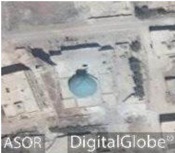
al-Bara bin Malek Mosque showing previous damage (DigitalGlobe; July 26, 2016)
