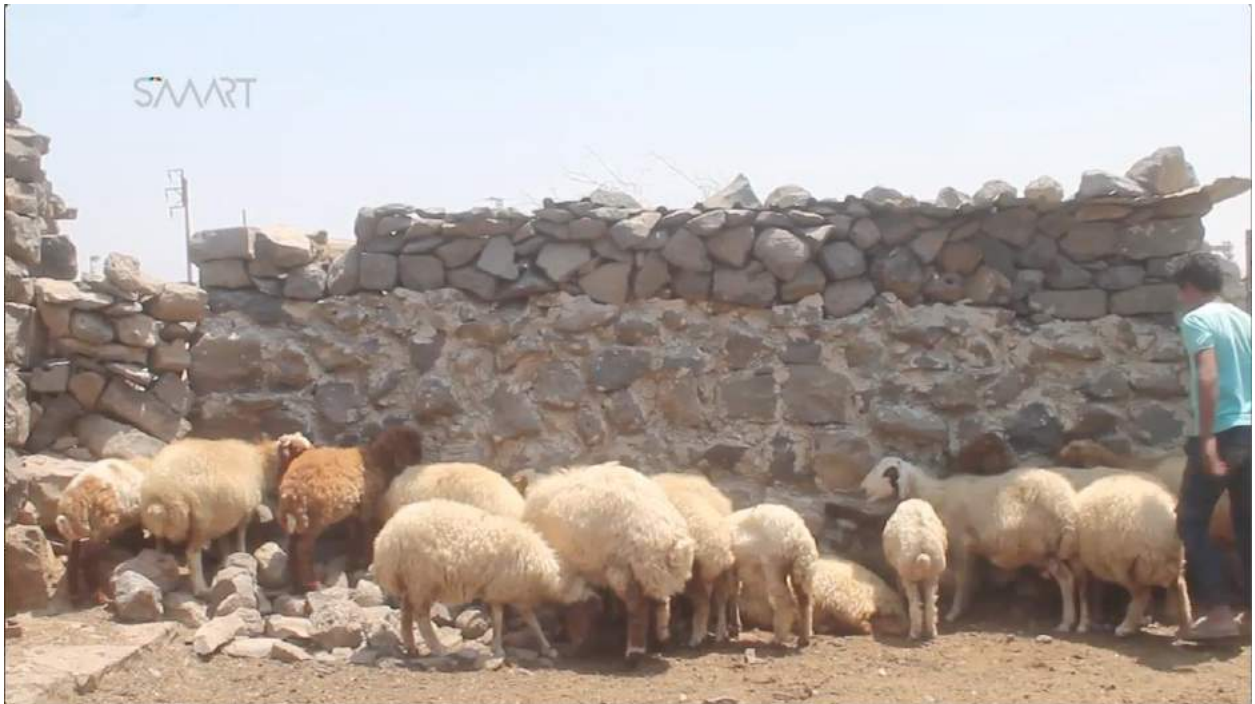
Video still of Byzantine structures reused by modern inhabitants (SMART News Agency; August 9, 2016)
