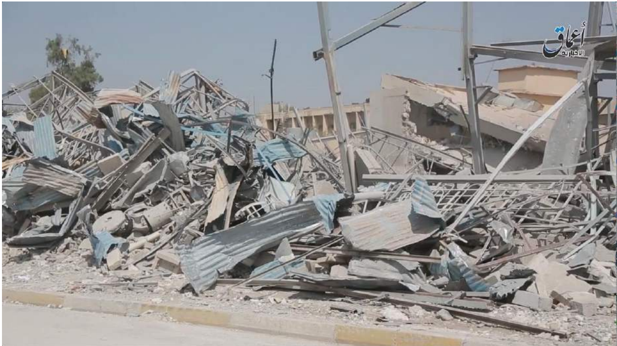
Video still of damage to the Faculty of Science (Amaq News Agency/Youtube; August 6, 2016)
