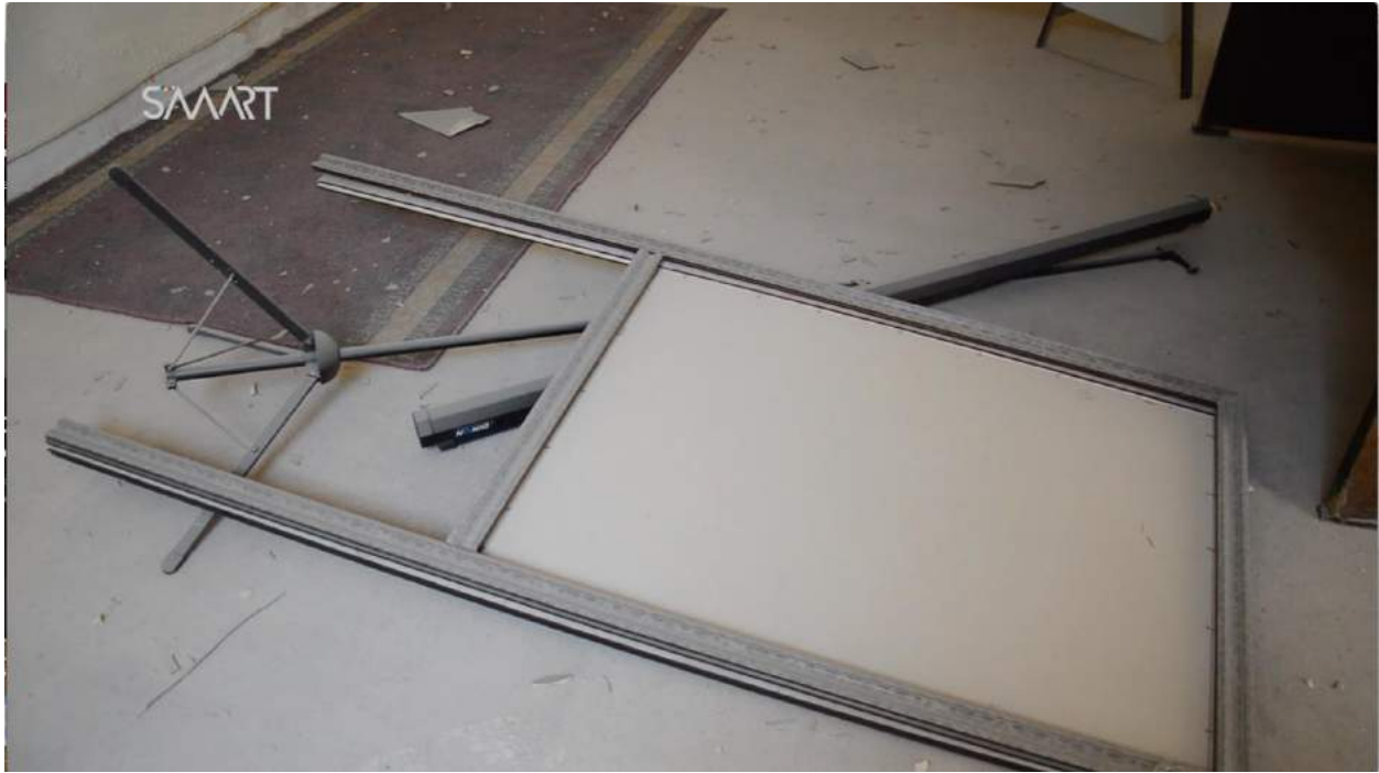
Video still of material damage at Waraqa Cultural Center (SMART News Agency; August 15, 2016)
