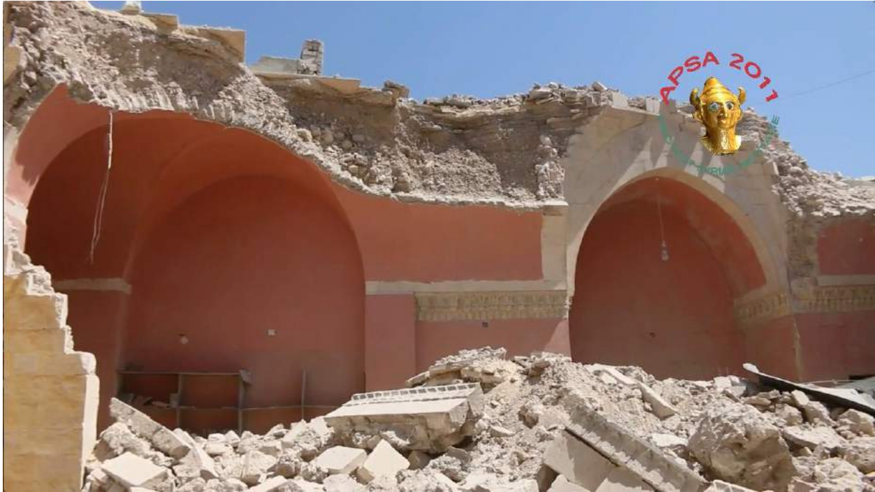
Video still of damage to the Waraqa Cultural Central (APSA; August 16, 2016)
