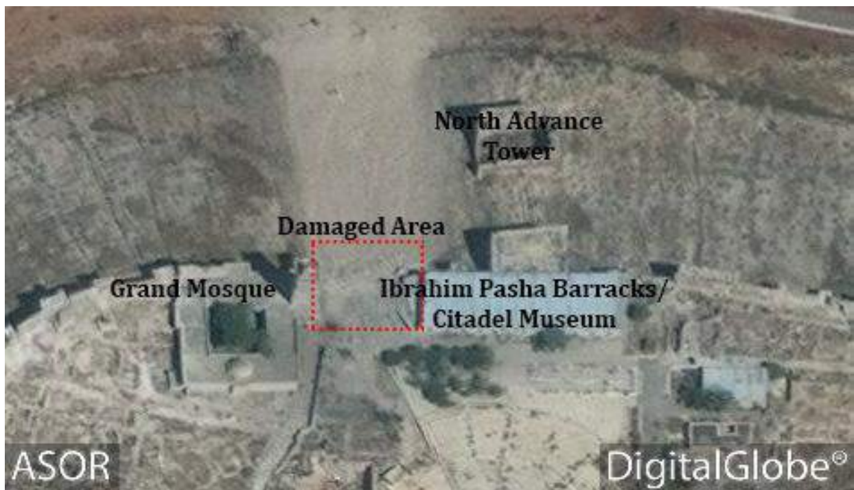
Damage to northern fortification wall and western side of Citadel museum (DigitalGlobe; August 11, 2016)
