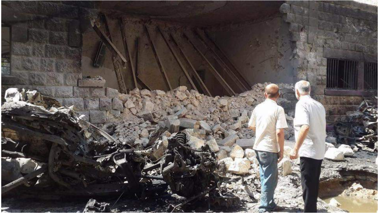
Damage to school building at Protestant Church (Facebook; August 10, 2016)
