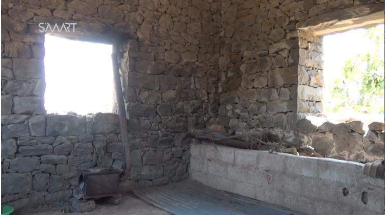
Video still of Byzantine structures reused by modern inhabitants (SMART News Agency; August 11, 2016)
