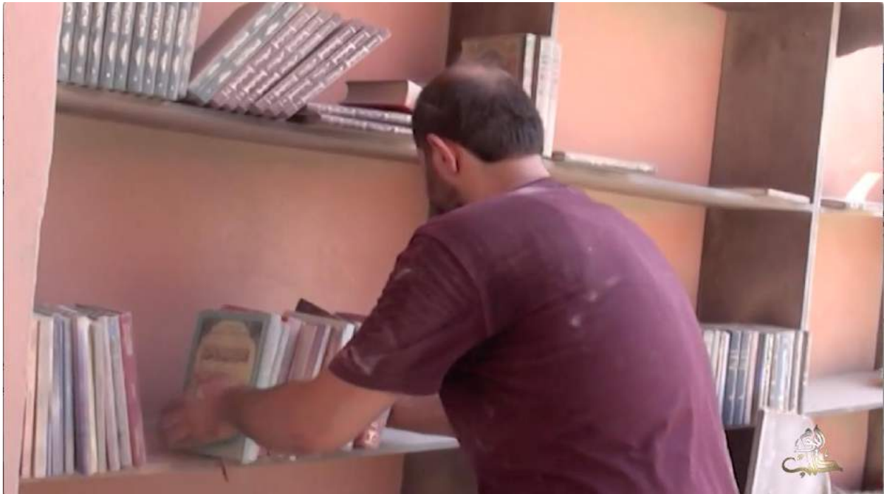
Video still of damage to the library at Waraqa Cultural Center (Halab Today TV; August 15, 2016)
