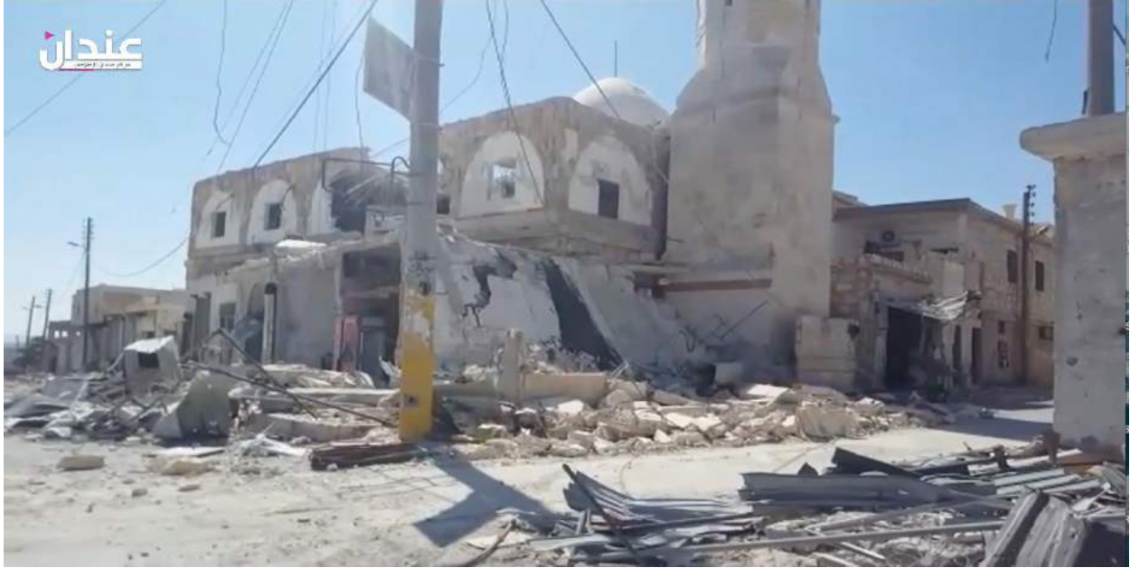
Video still of damage to Abu Bakr al Sidiq Mosque (Anadan Media Center/Youtube; July 25, 2016)
