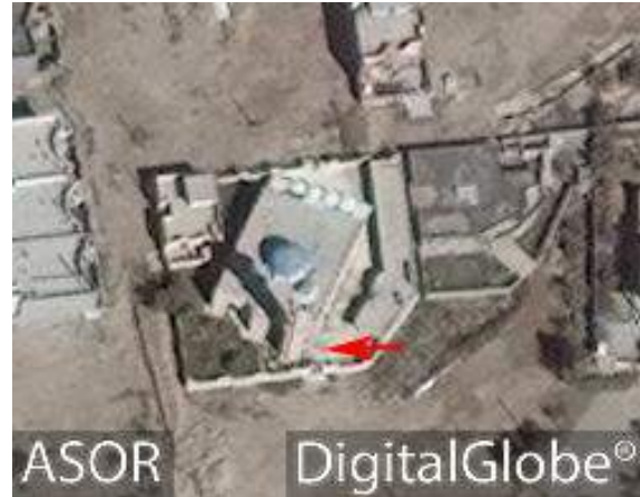
Yusuf al-Sidiq Mosque with debris visible near minaret (DigitalGlobe; March 5, 2016)
