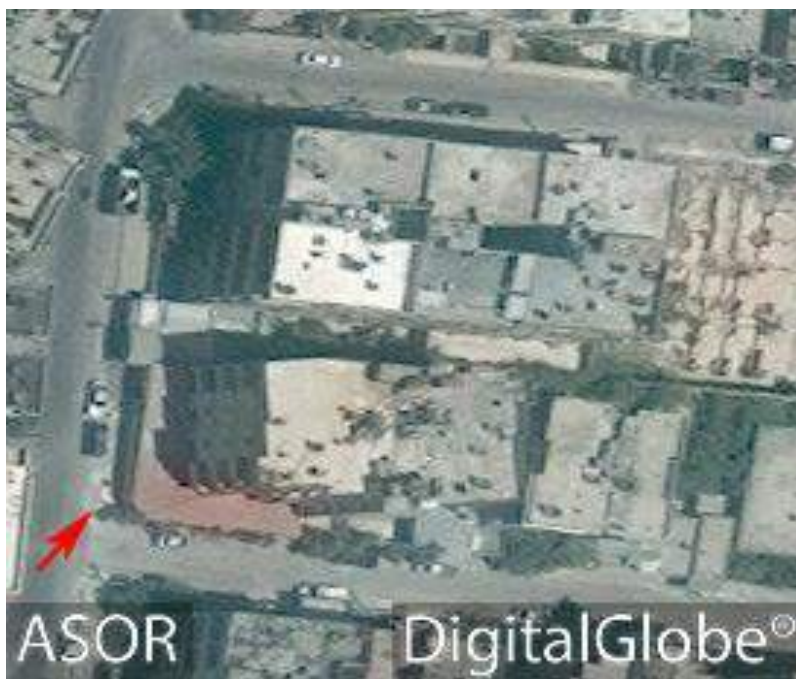
Bilal Mosque with possible damage visible on the western side (DigitalGlobe; August 1, 2016)
