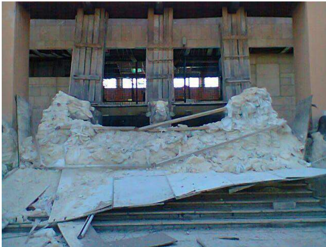
Entrance to Aleppo Museum after damage. (DGAM; July 24, 2016)
