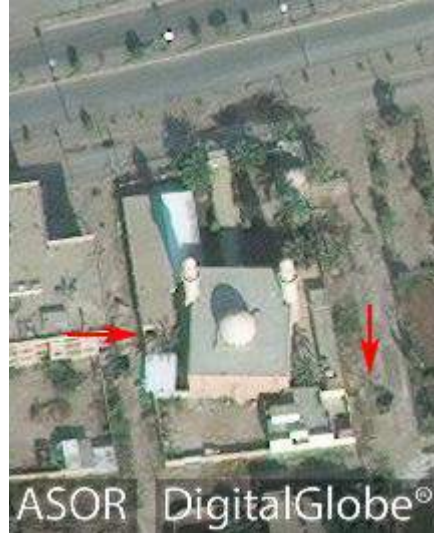
Hamoud Mahmoud Mosque with visible damage (DigitalGlobe; December 8, 2014)
