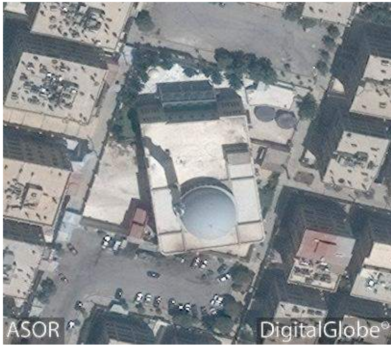
al-Shami Mosque showing previous damage on the south side (DigitalGlobe; July 19, 2016)
