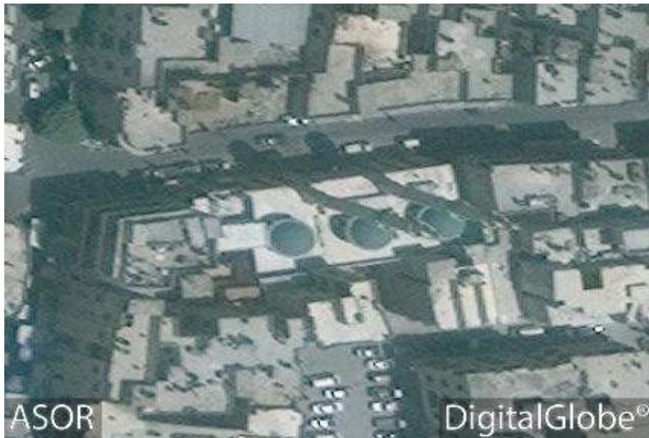
al-Omari Mosque prior to damage (DigitalGlobe; June 19, 2016)
