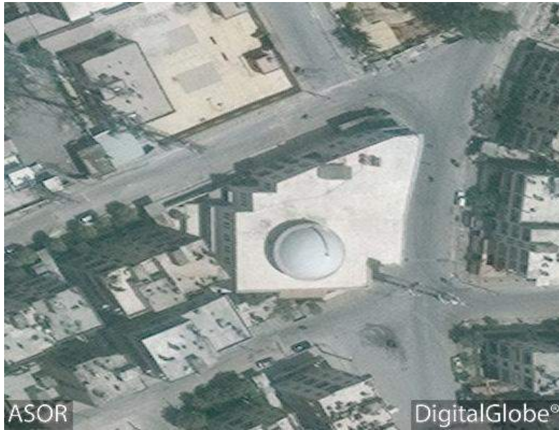
Saad bin Abi Waqas Mosque prior to damage (DigitalGlobe; June 19, 2016)
