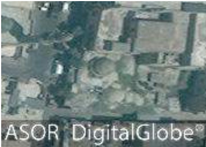
al-Kabir Mosque with no visible damage even after reports of airstrikes (DigitalGlobe; August 1, 2016)
