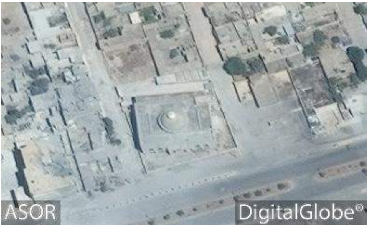
al-Fatah Mosque and the surrounding areas with visible damage to the western buildings (DigitalGlobe; July 26, 2016)
