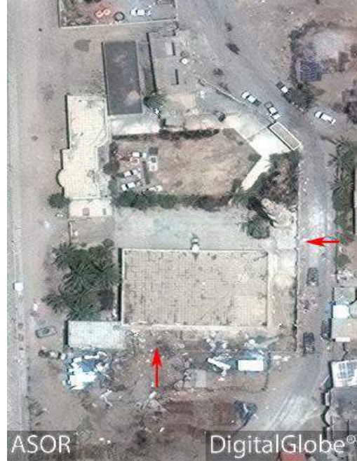
al-Kabir Mosque with damage with damage to the southern and exterior walls (DigitalGlobe; June 28, 2016)
