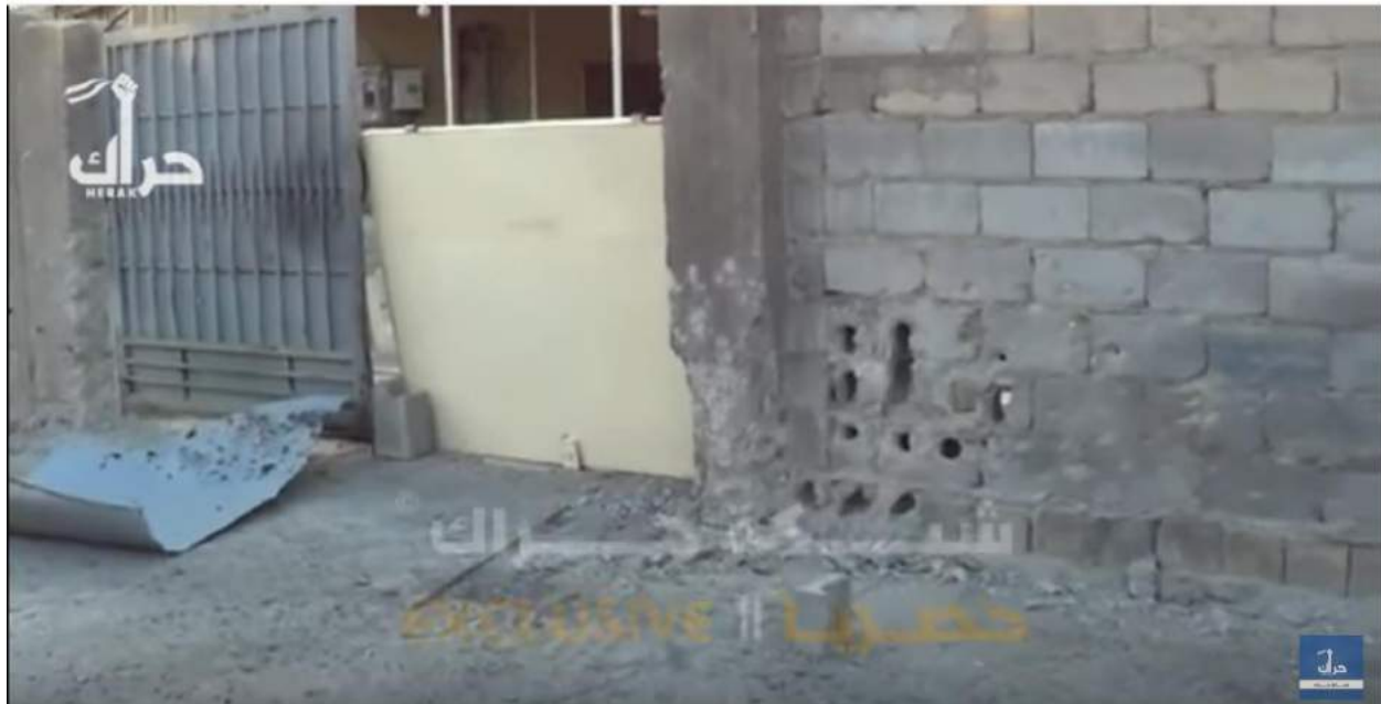
Video still of damage to al-Mursalin Mosque (Herak News/Youtube; February 24, 2014)
