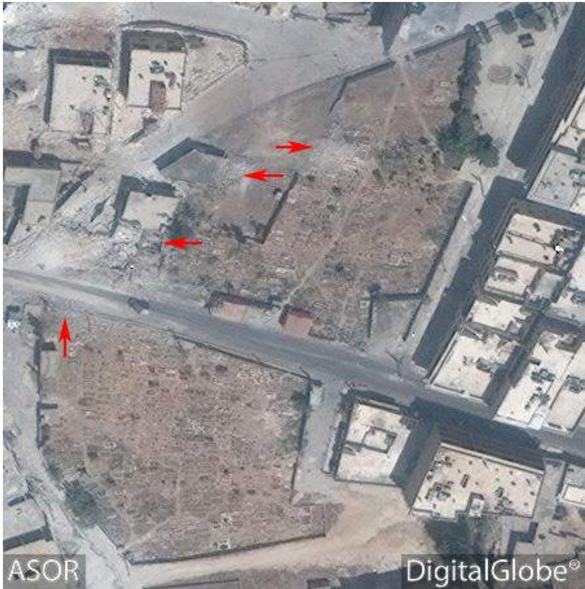
The cemetery with damage to graves, the cemetery wall, and associated buildings on the west side (DigitalGlobe; July 19, 2016)
