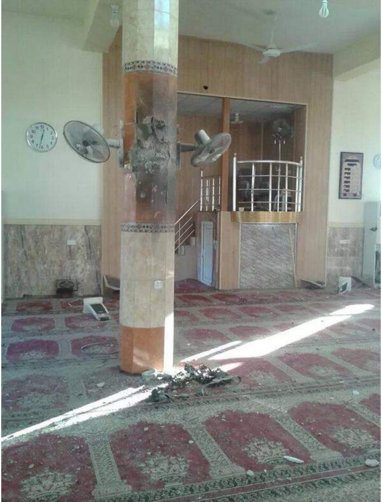
Interior damage to Ayyub al Ansari Mosque (Twitter; February 11, 2014)
