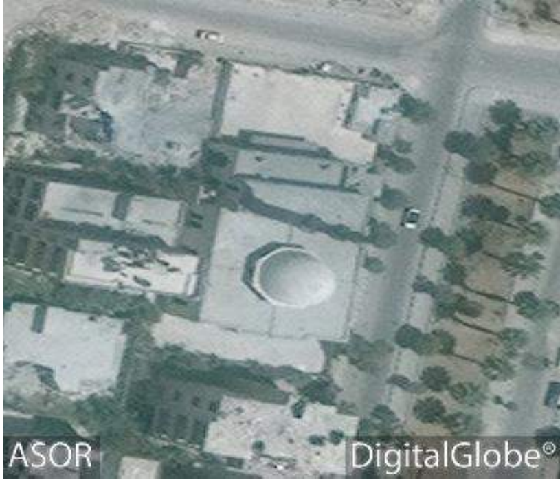
al-Rawda Mosque prior to damage (DigitalGlobe; June 19, 2016)
