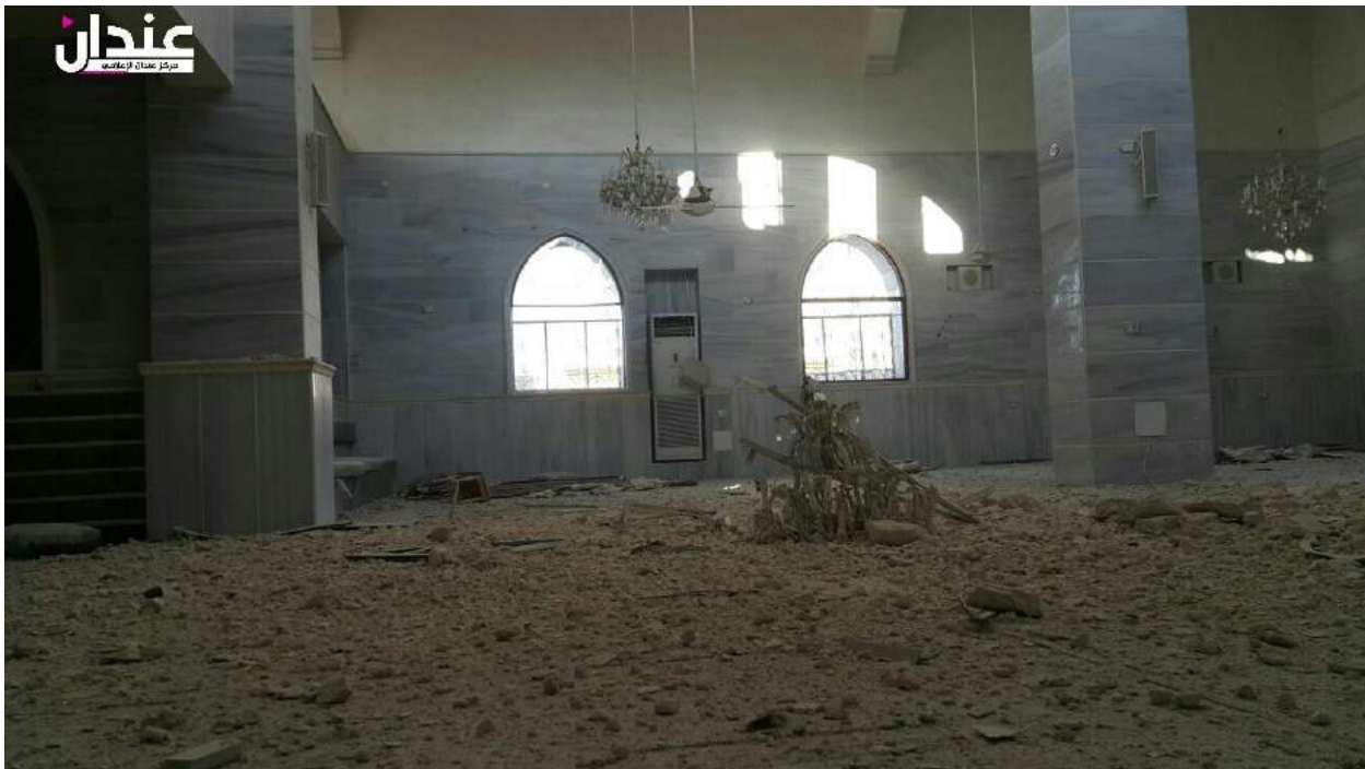
Interior damage to Abu Bakr al-Sidiq Mosque (Anadan Media Center/Facebook; July 15, 2016)
