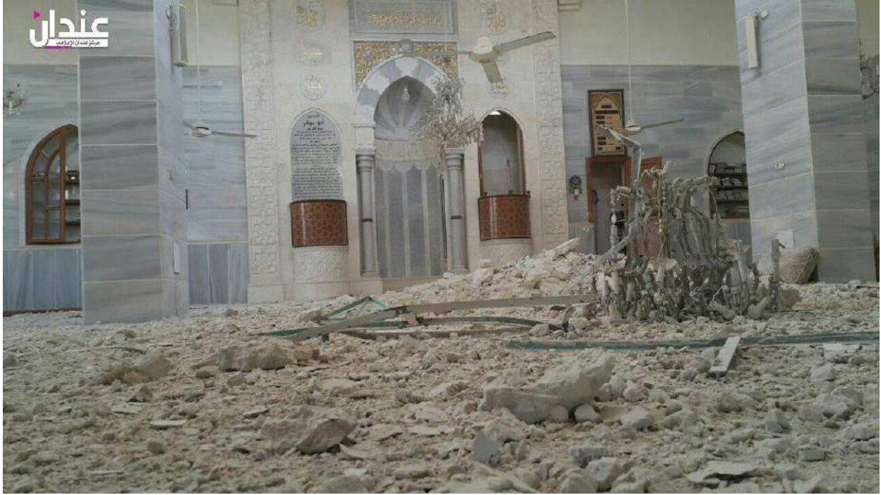
Interior damage to Abu Bakr al-Sidiq Mosque (Anadan Media Center/Facebook; July 15, 2016)
