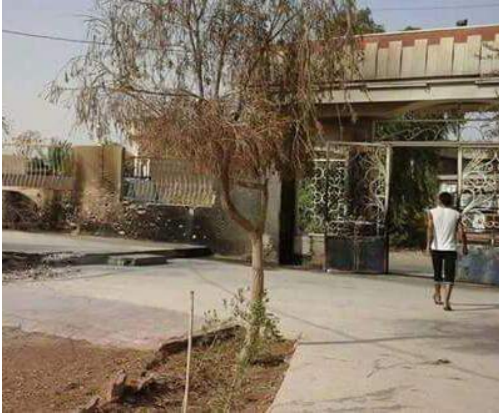
Minor damage to the exterior of al-Kabir Mosque (Twitter ; September 1, 2015)
