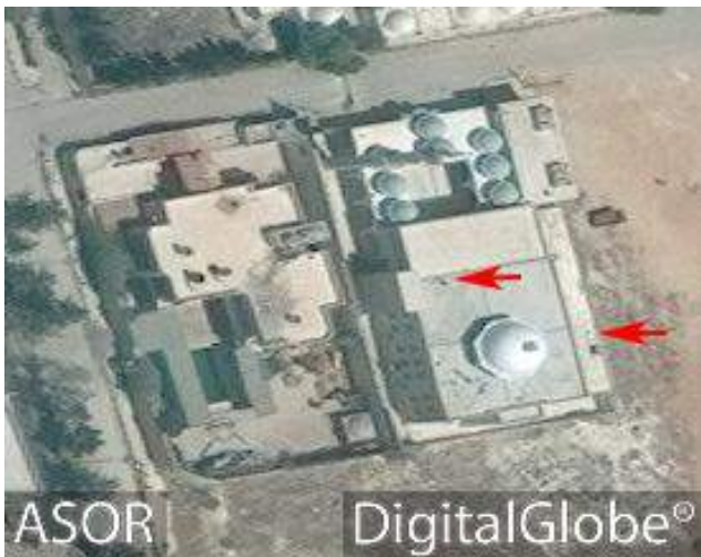
al-Tawhid Mosque with minor damage (DigitalGlobe; August 1, 2016)
