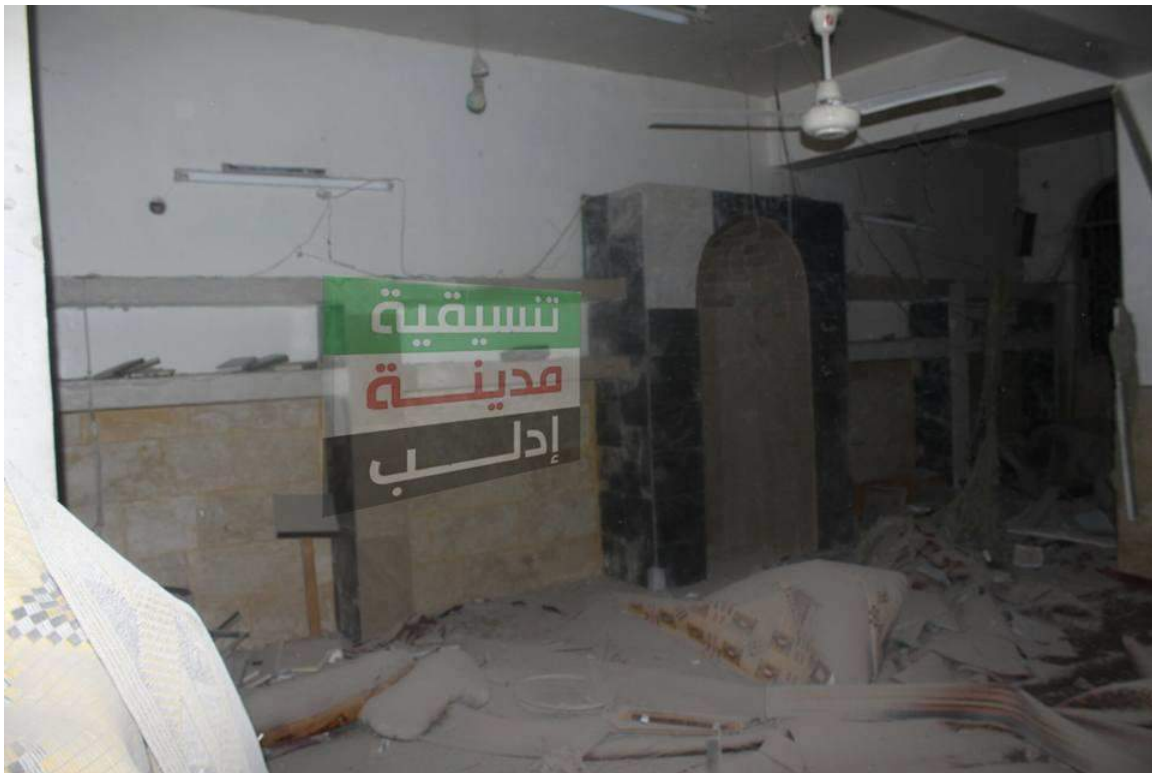
Damage to al-Hijazi Mosque (S.N.N; July 22, 2016)
