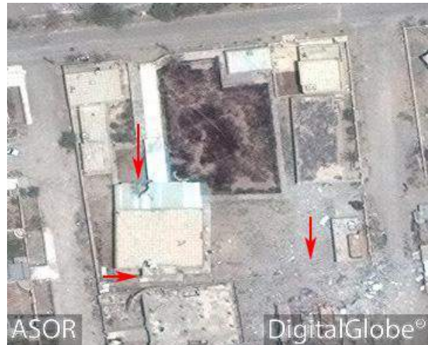
al-Mujahirin Mosque with damage to the mosque and exterior wall (DigitalGlobe; June 28, 2016)
