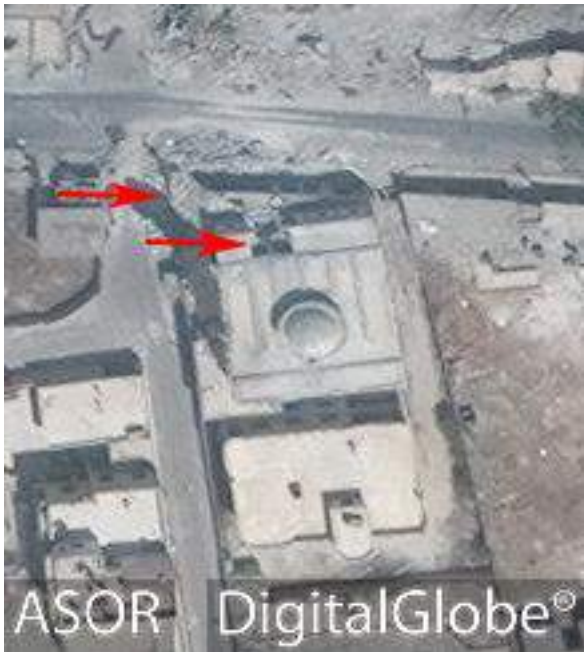
Abu Bakr al-Sidiq Mosque with damage to the northern side and roof (DigitalGlobe; July 19, 2016)
