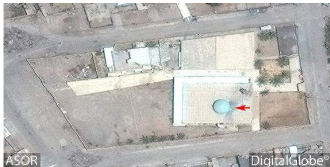
Abu Ayyub al-Ansari Mosque with damage to roof (DigitalGlobe; June 28, 2016)
