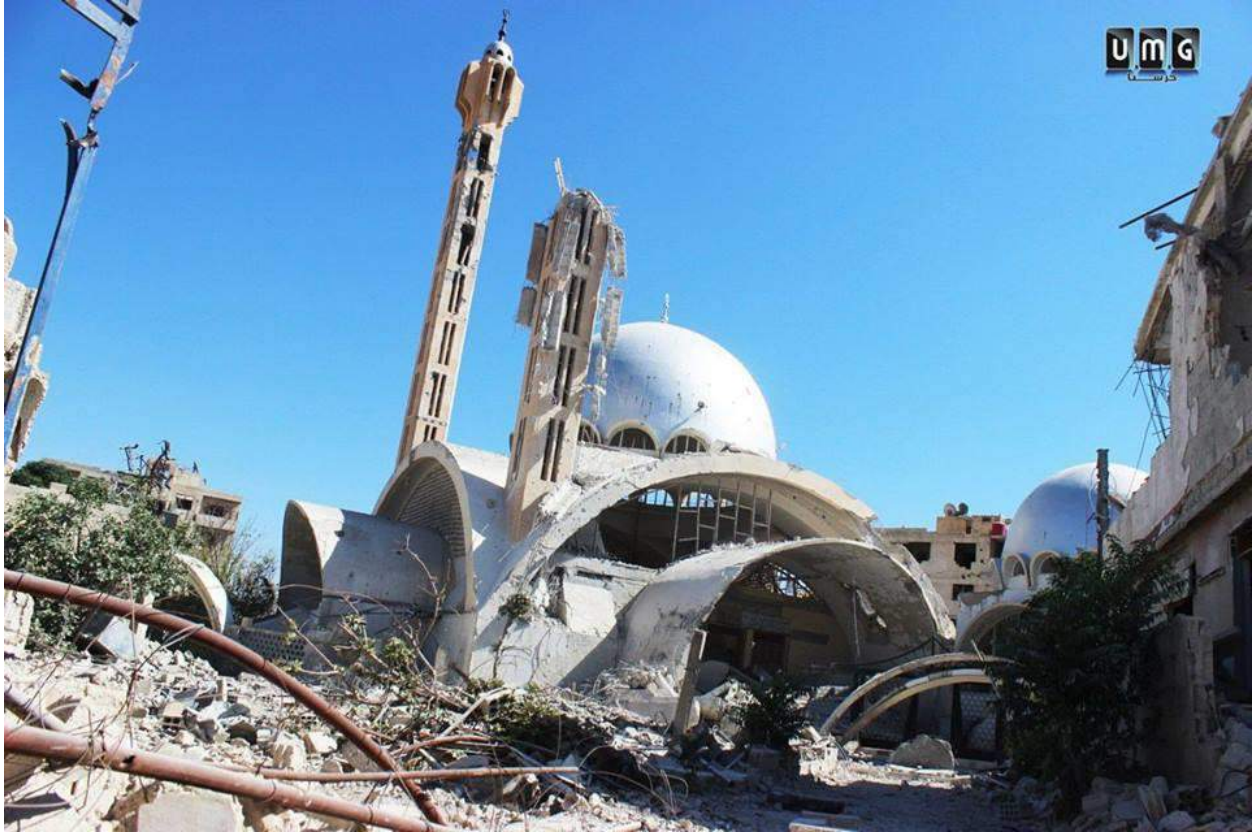
Extensive damage to Aqil ibn Abi Talib Mosque (SNHR; July 22, 2016)
