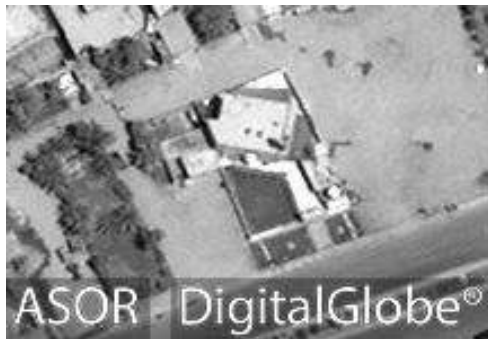
al-Mukarim Mosque prior to damage (DigitalGlobe; July 20, 2012)
