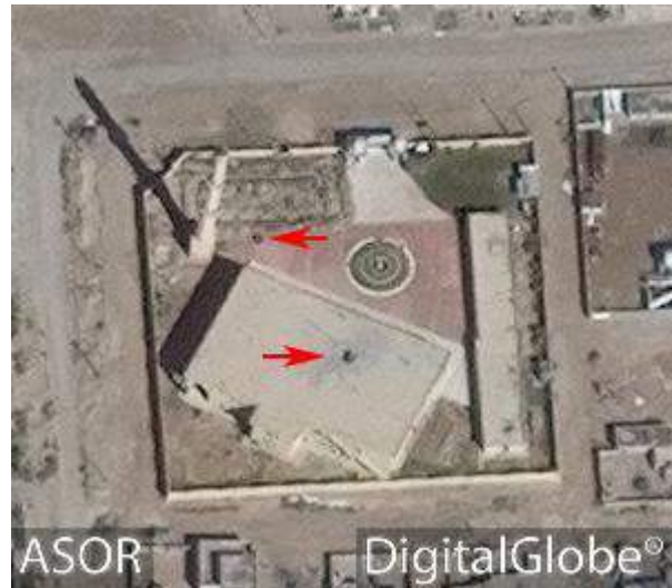
al-Shamari Mosque with a hole in the roof and in the courtyard (DigitalGlobe; March 5, 2016)
