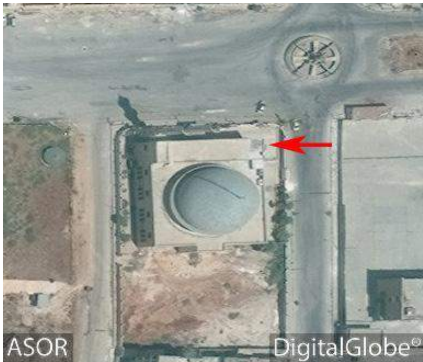
Shoab Mosque with visible damage to the northwest corner (DigitalGlobe; August 1, 2016)
