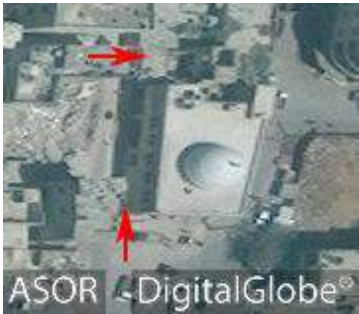
al-Hijazi Mosque with damage on the western and northern sides. Visible damage to the buildings on the west as well (DigitalGlobe; August 1, 2016)
