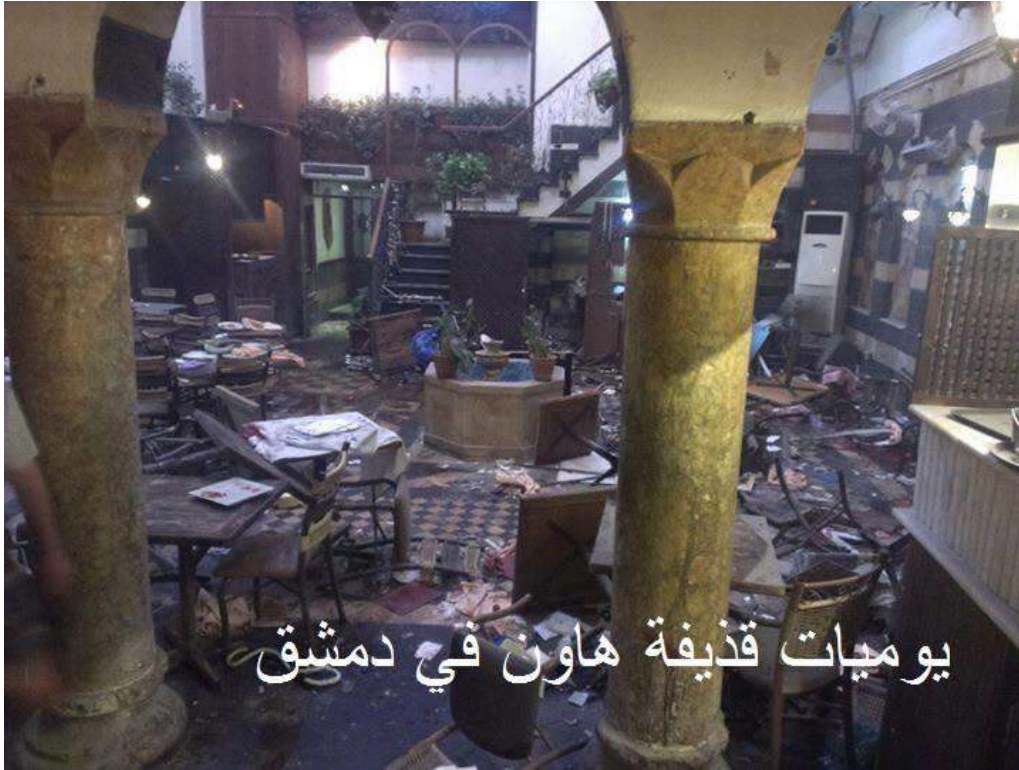
Damage to the interior of Qamar al-Sham Restaurant (Yomet Kzefeh Hawen; July 24, 2016)
