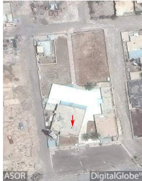
al-Tawfiq Mosque with a hole in the roof (DigitalGlobe; June 28, 2016)
