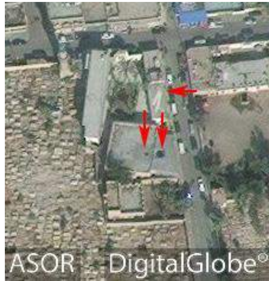
al-Farouk Mosque with visible damage to the roof (DigitalGlobe; December 8, 2014)
