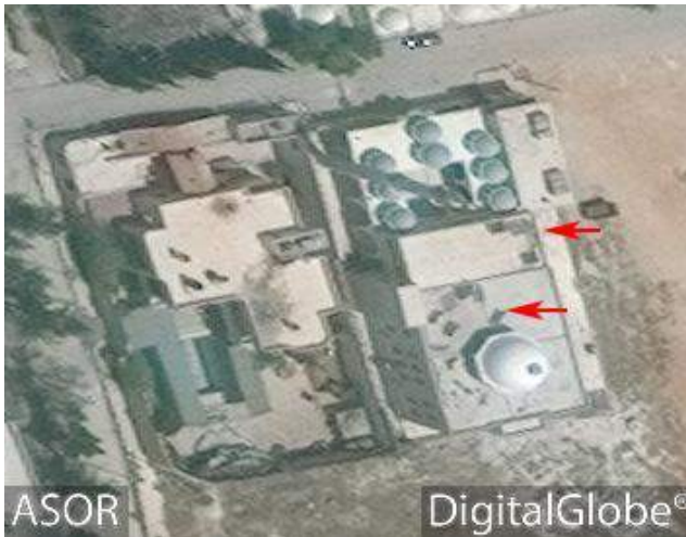
al-Tawhid Mosque with discoloration on the roof (DigitalGlobe; June 19, 2016)
