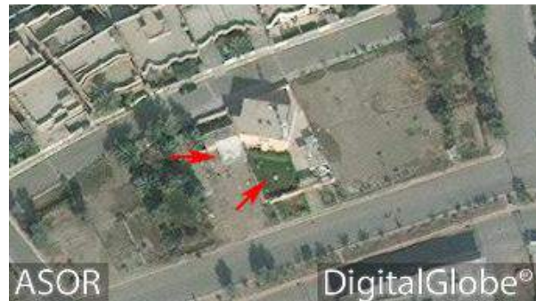
al-Mukarim Mosque with damage to the exterior (DigitalGlobe; December 8, 2014)
