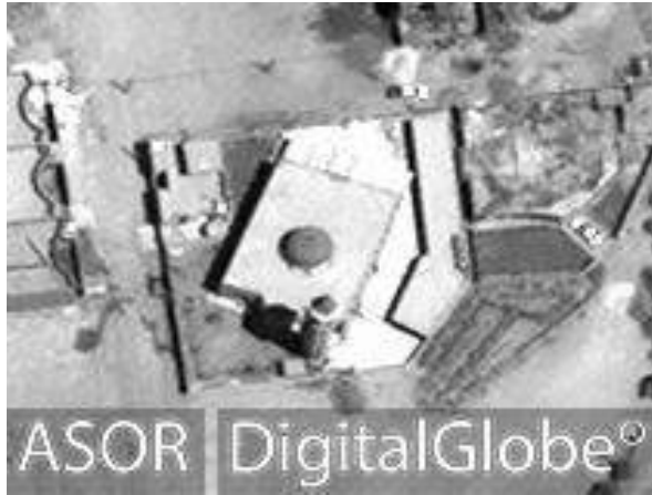
Yusuf al-Sidiq Mosque prior to damage (DigitalGlobe; July 20, 2012)
