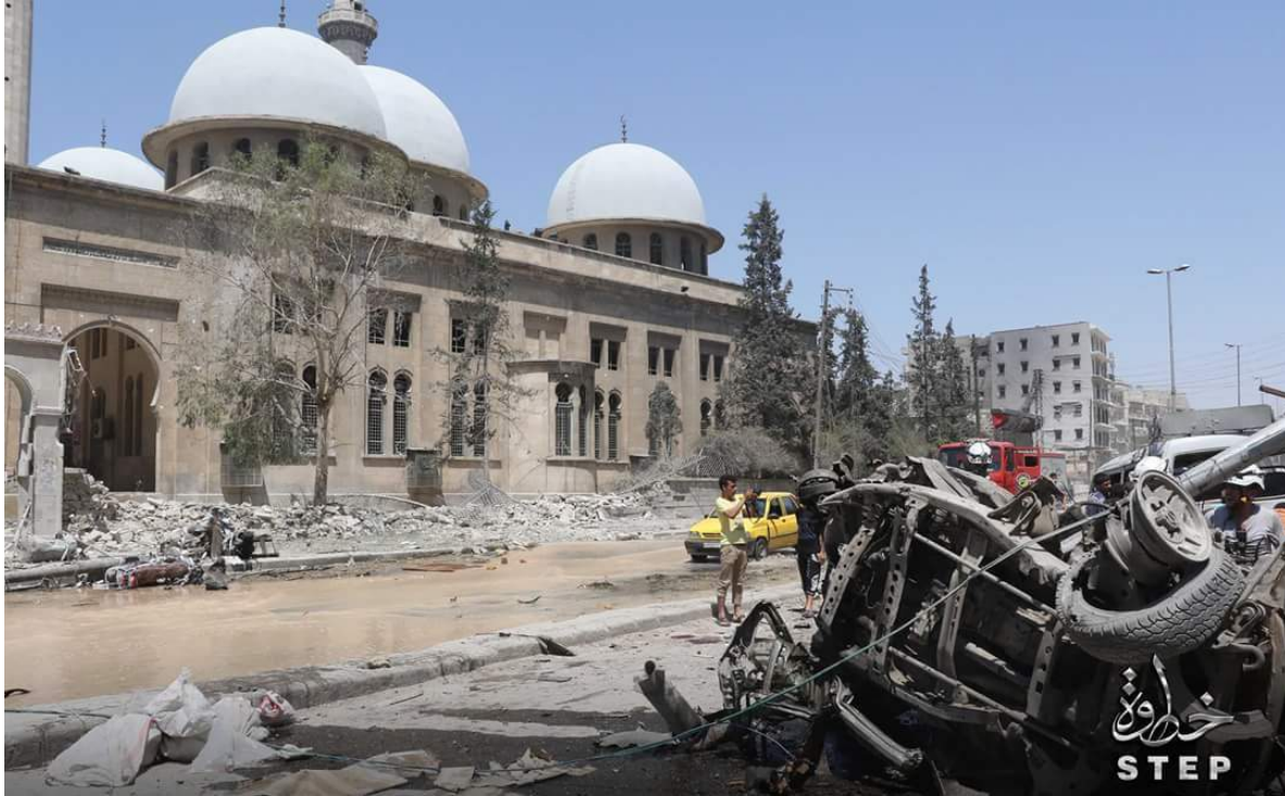
Damage to the exterior of Abdul Qadir Gilani Mosque showing large piles of rubble outside the building (Step News Agency/Twitter; July 21, 2016)
