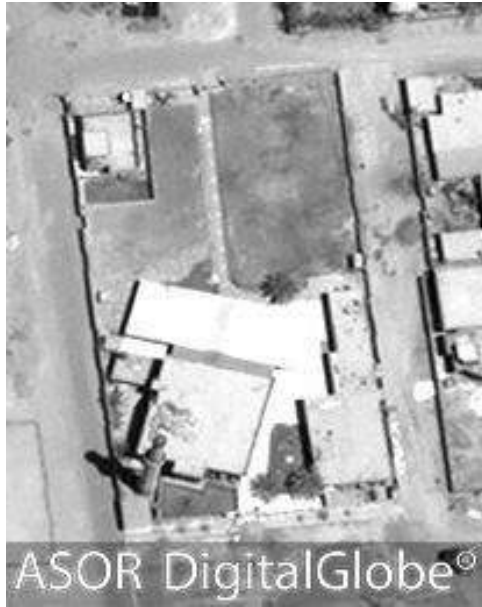
al-Tawfiq Mosque prior to damage (DigitalGlobe; July 20, 2012)
