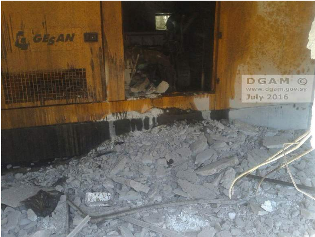
Damage to interior of National Museum of Aleppo (DGAM; July 13, 2016)
