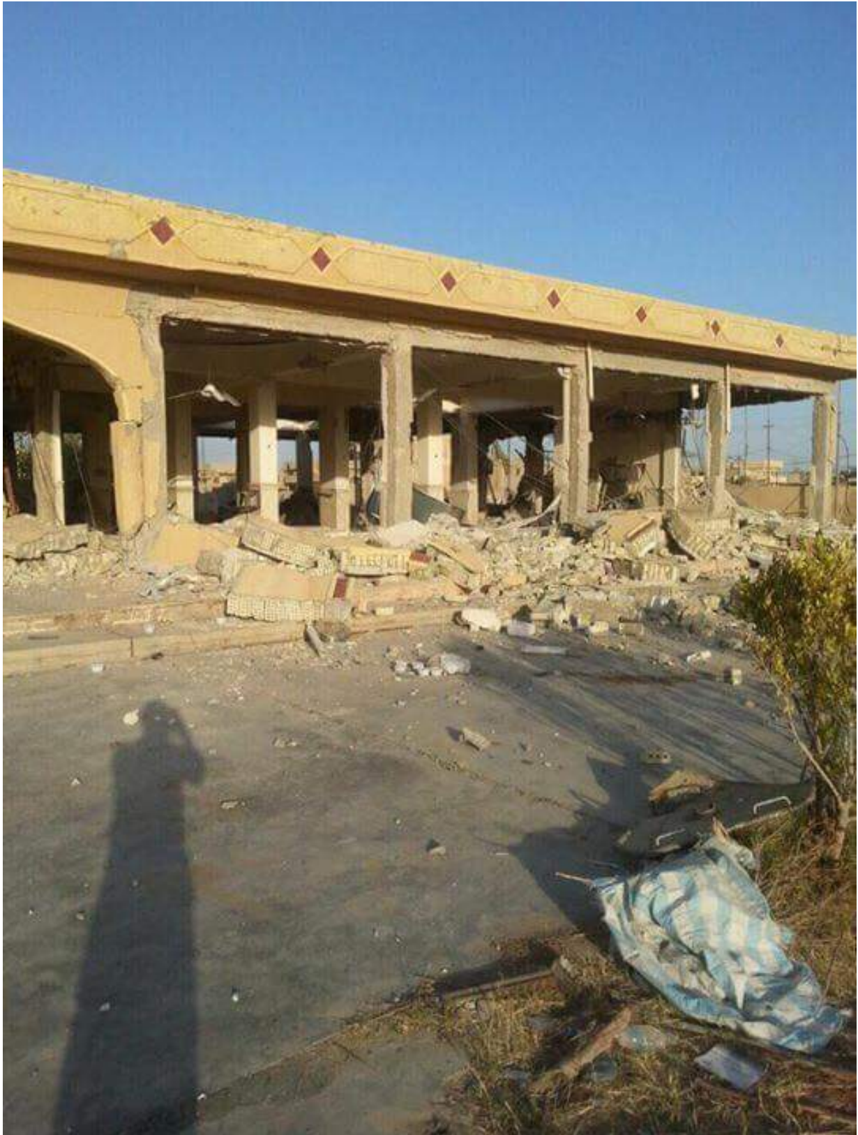
Destruction of al-Taqwa Mosque (Twitter; July 9, 2016)
