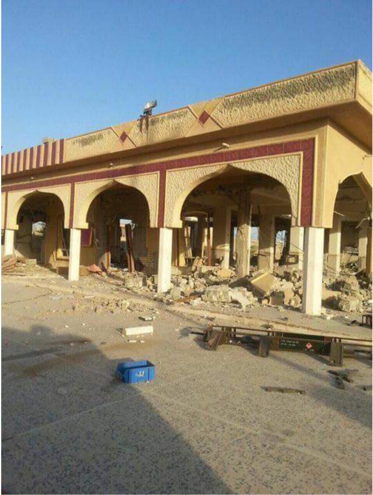
Destruction of al-Taqwa Mosque (Twitter; July 9, 2016)
