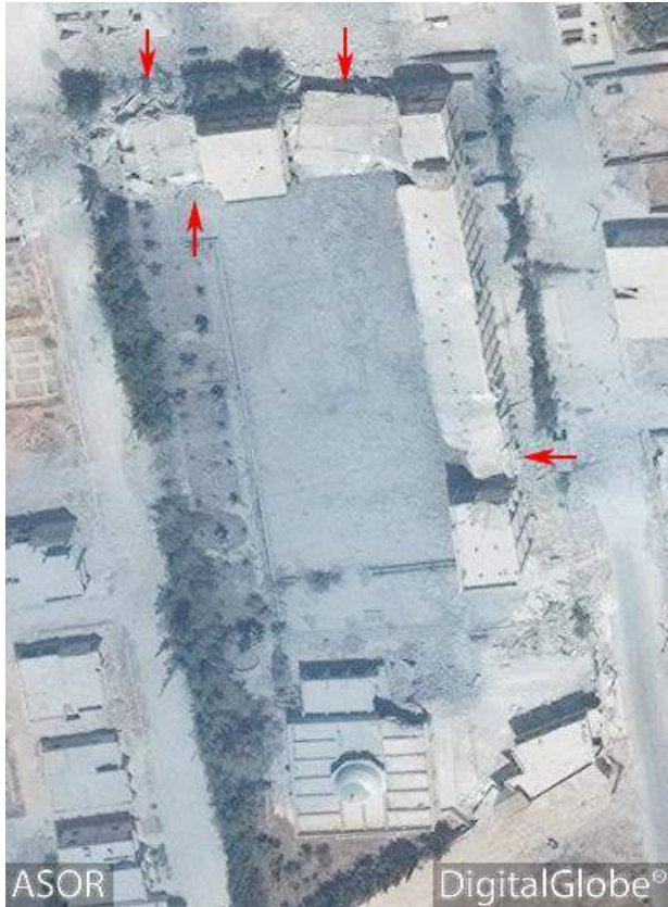
Severe damage to the al-Sharaya School with several portions of the building collapsed (DigitalGlobe; July 6, 2016)
