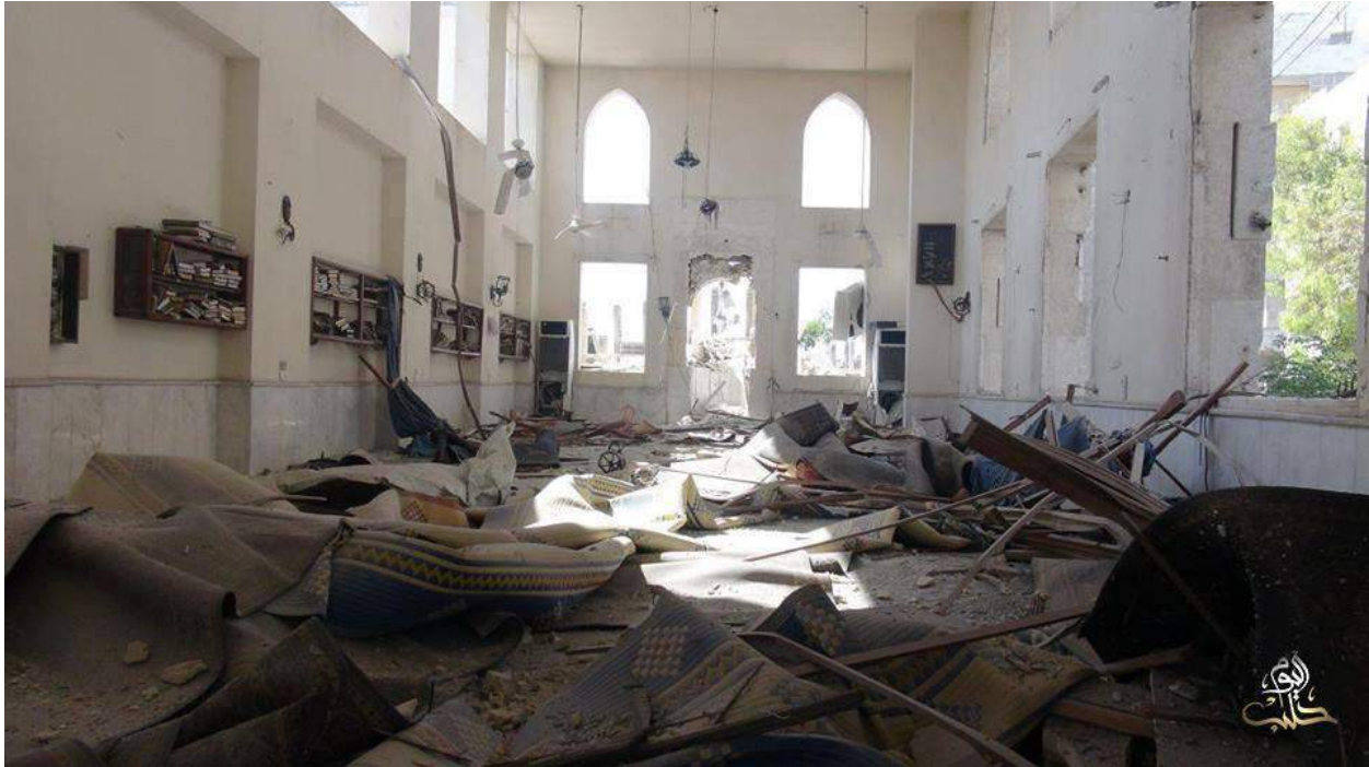
Severe damage to al-Saleheen Mosque (SNHR; July 16, 2016)
