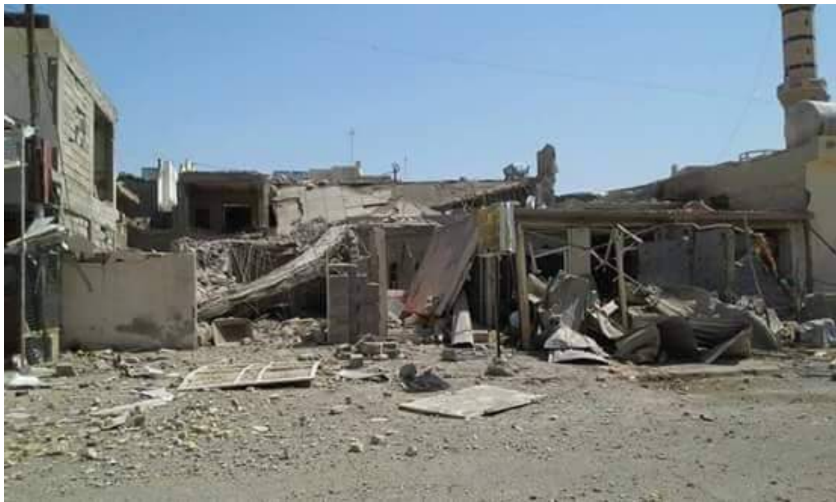
Destruction of building adjacent to al-Mudallal Mosque (Twitter; July 5, 2016)
