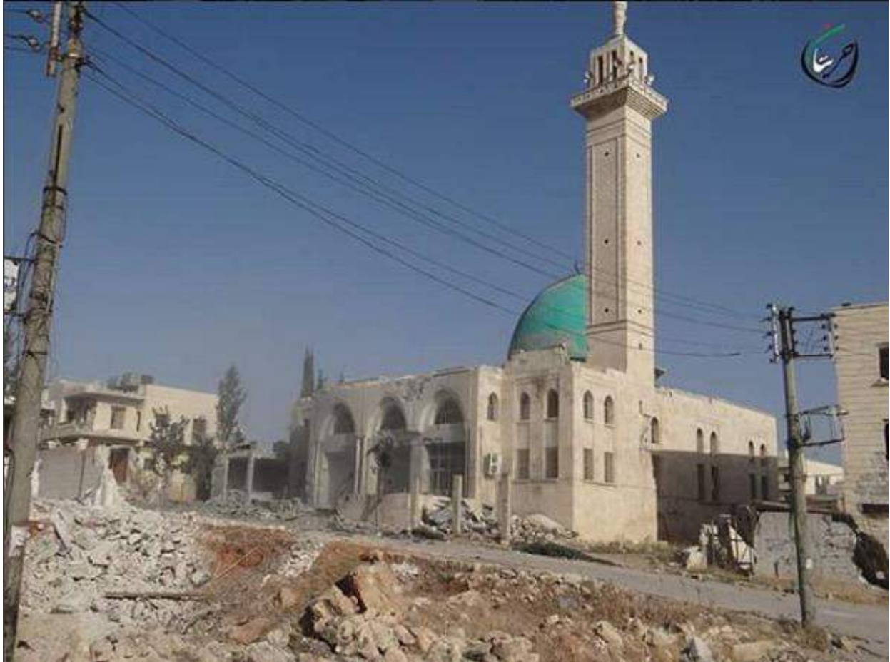
Damage to Al Bara bin Malek Mosque (Hraitan City; May 22, 2016)
