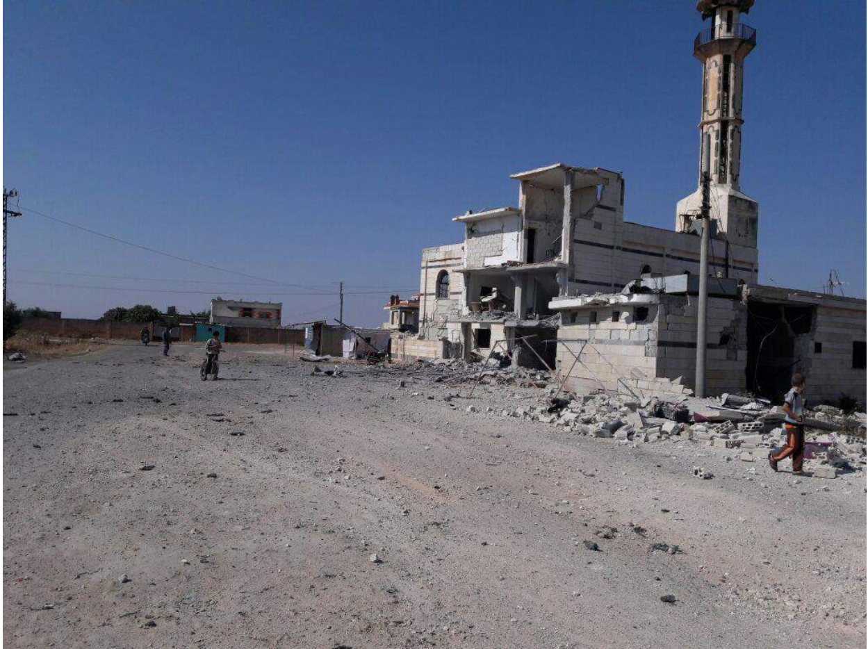
Damage to al-Musafir Mosque (Twitter; July 9, 2016)
