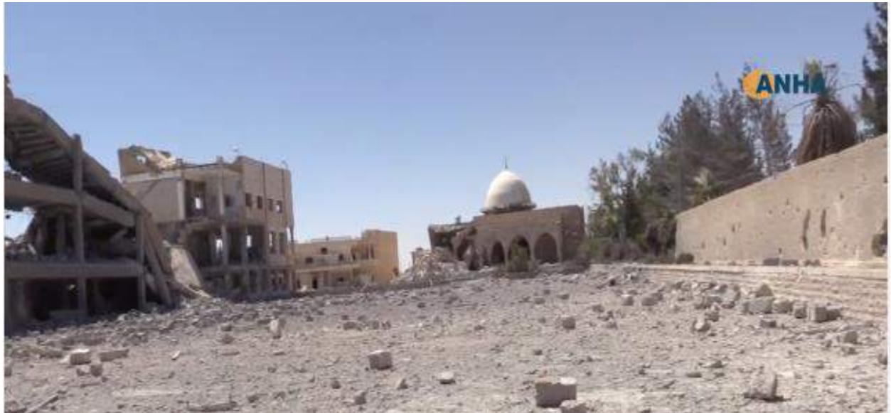
Damage to al-Sharaya School and al-Miqdad Mosque (ANHA; July 11, 2016)
