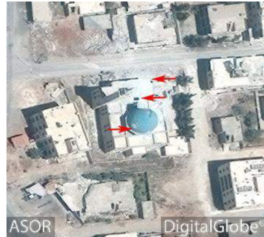
Visible damage to the north wall, roof, and dome of the mosque (DigitalGlobe; July 13, 2016)
