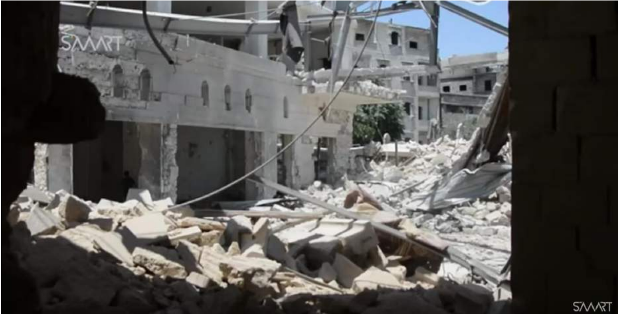
Video still of damage to exterior of al-Saleheen Mosque (SMART News Agency; July 16, 2016)
