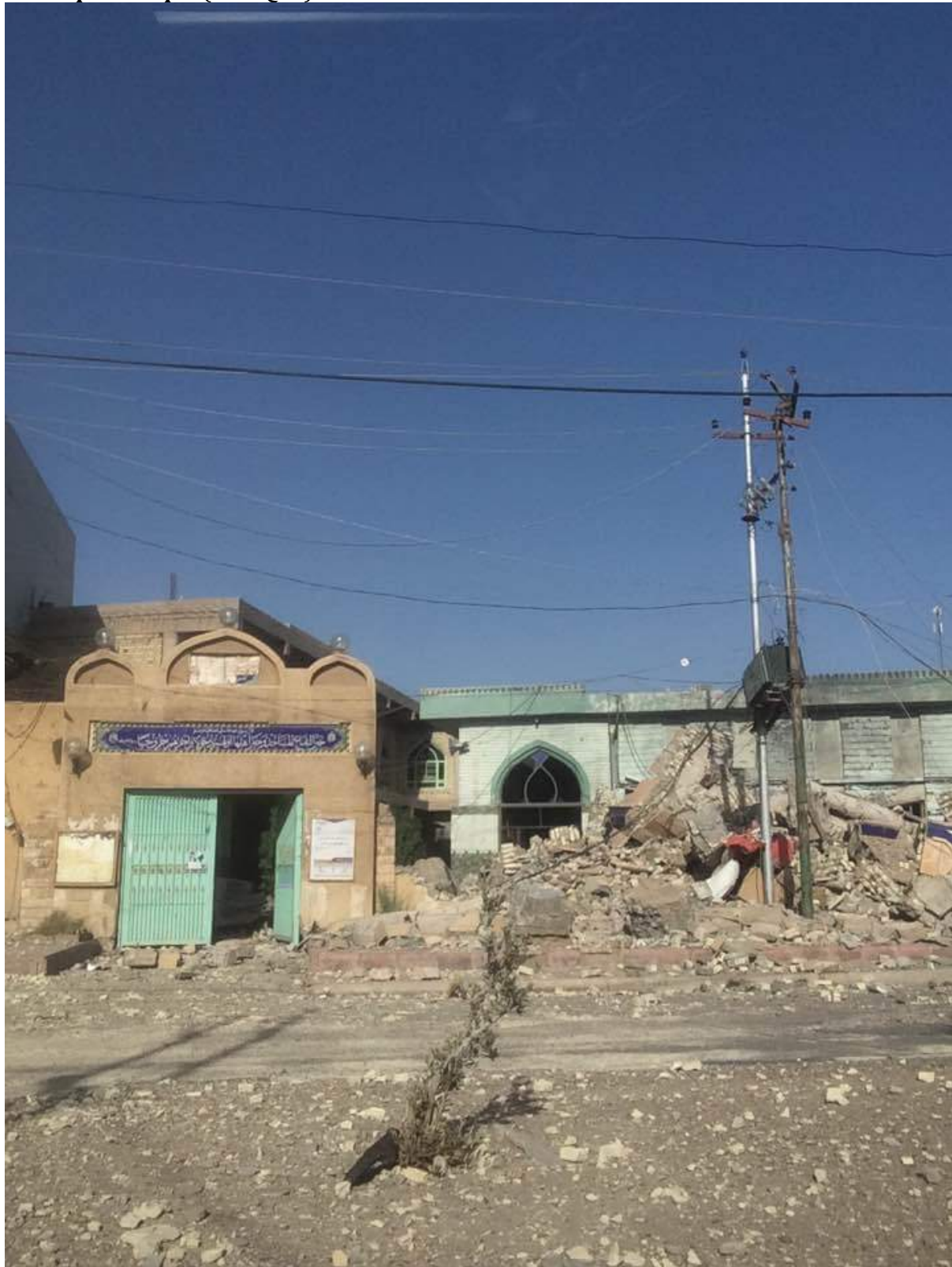
Destroyed minaret of al-Furqan Mosque (Twitter; July 13, 2016)
