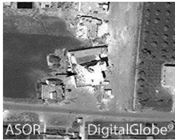
al-Musafir Mosque with damage to its western wall (DigitalGlobe; July 14, 2016)
