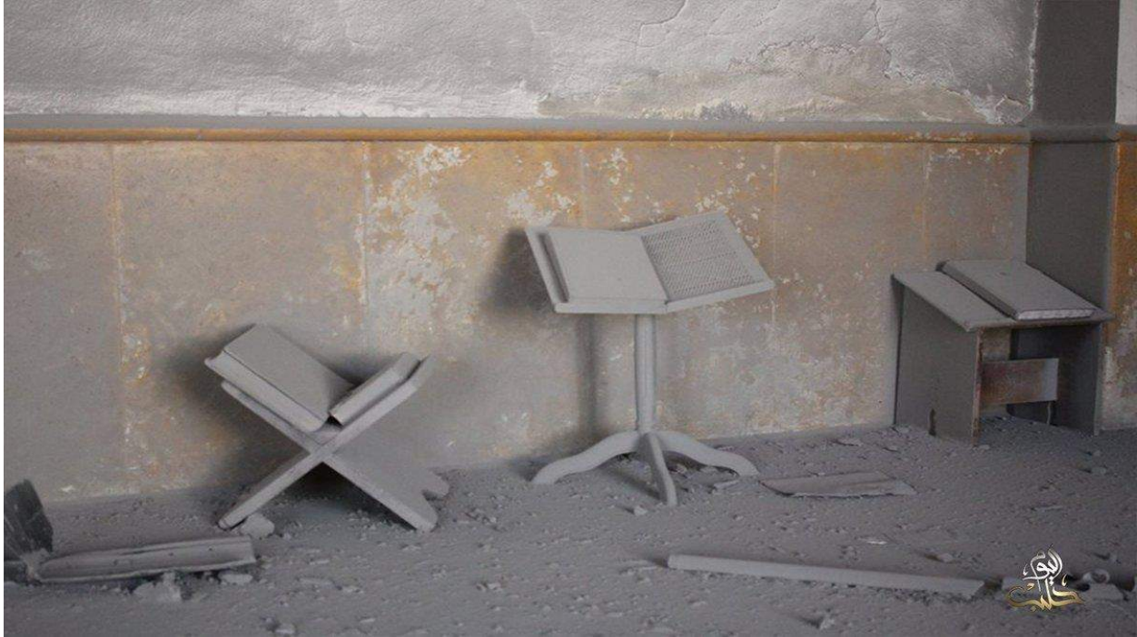
Damage to Shuhada al-Aqsa Mosque (Halab Today/Twitter; July 14, 2016)
