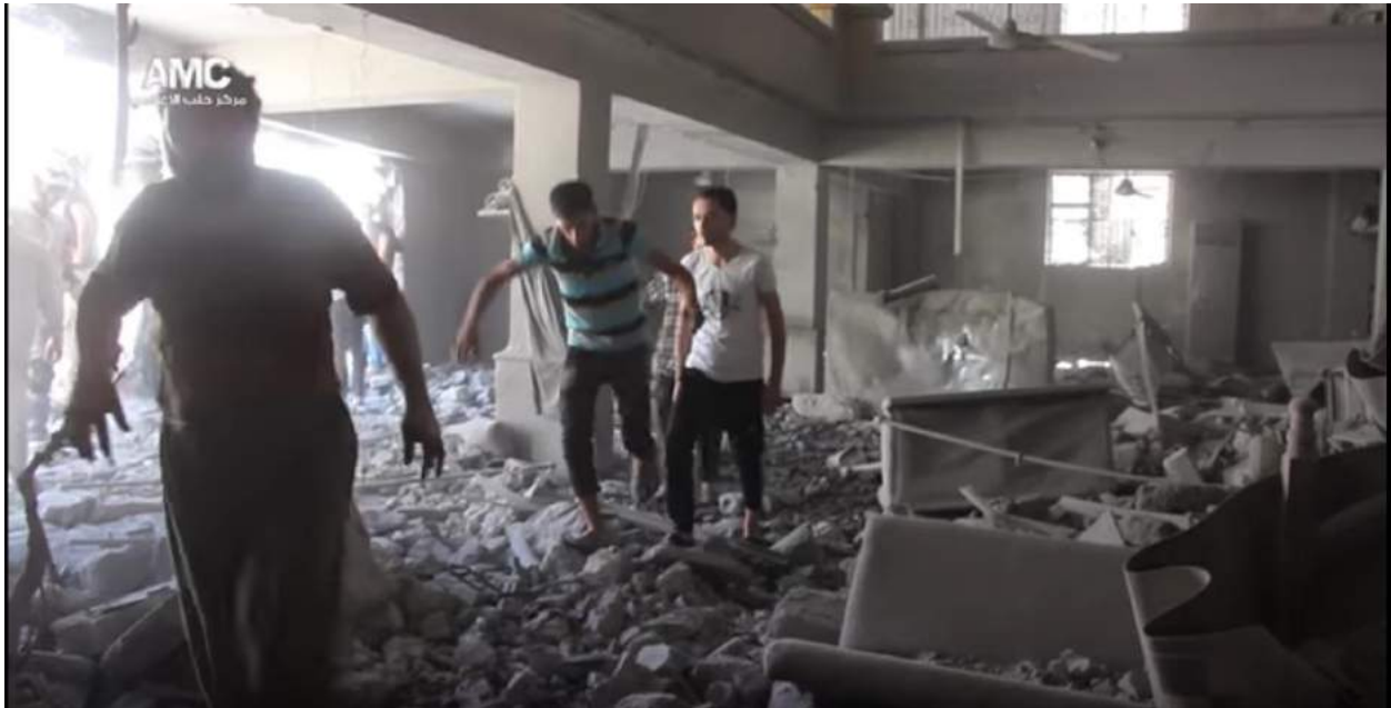
Video still of damage to mosque's interior (Aleppo Media Center/Youtube; July 14, 2016)
