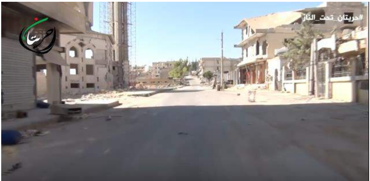
Video still of the base of al-Quds Mosque showing rubble surrounding the area (Hreitani City; July 3, 2016)
