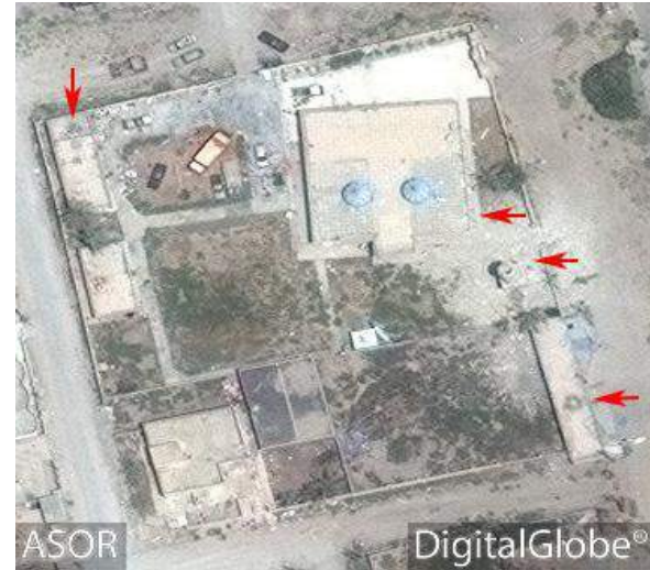
al-Taqwa Mosque with severe damage to the minaret, the mosque, and exterior buildings (DigitalGlobe; June 28, 2016)
