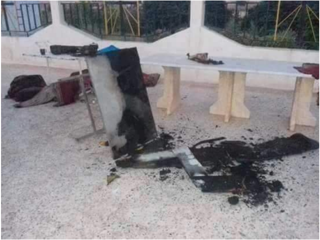
Damage outside of Mar Sharbel Church (Bas News; July 18, 2016)
