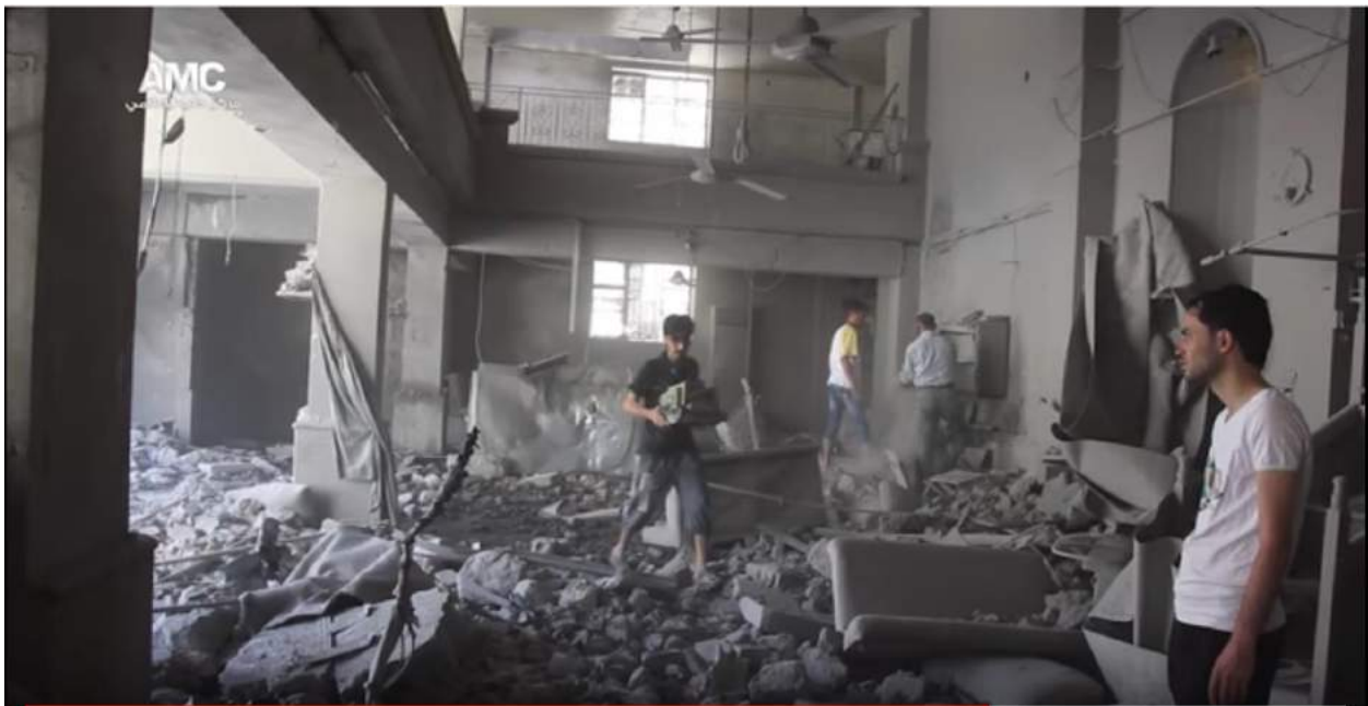
Video still of damage to mosque's interior (Aleppo Media Center/YouTube; July 14, 2016)
