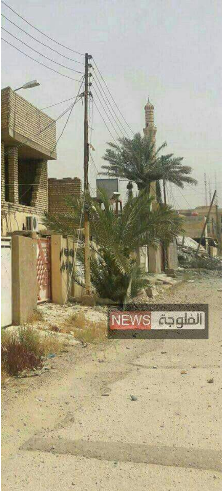
Minaret of Abu Obeida Mosque before its destruction (Fariq al-Muraslin/Twitter; July 7, 2016)
