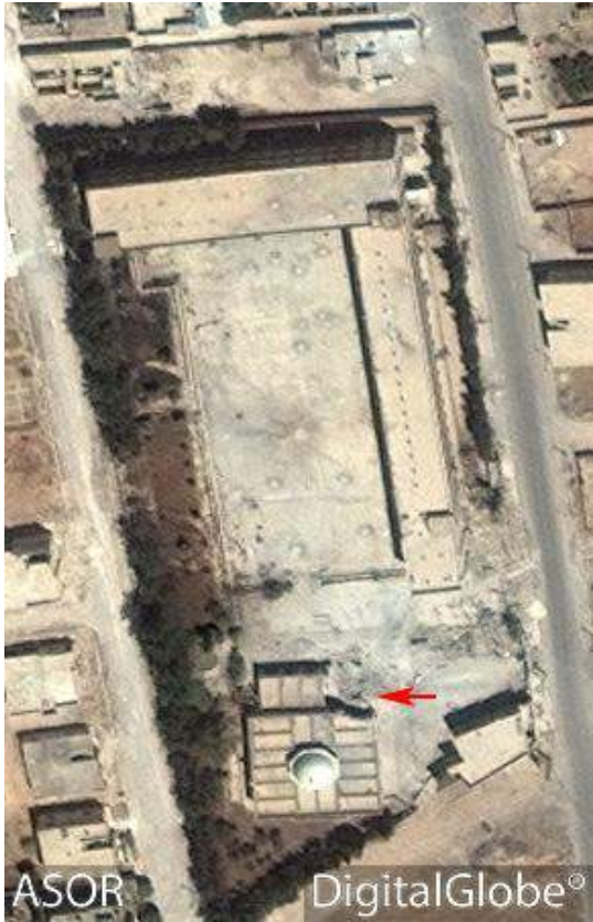
Damage to the minaret of the al-Miqdad Mosque and visible impact craters in the courtyard of the al-Sharaya School (DigitalGlobe; June 26, 2016)
