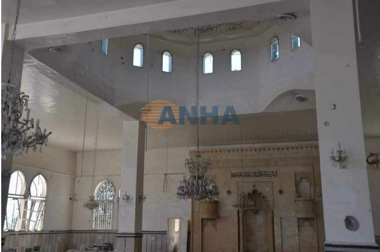
Damage to al-Miqdad Mosque (Twitter; July 12, 2016)
