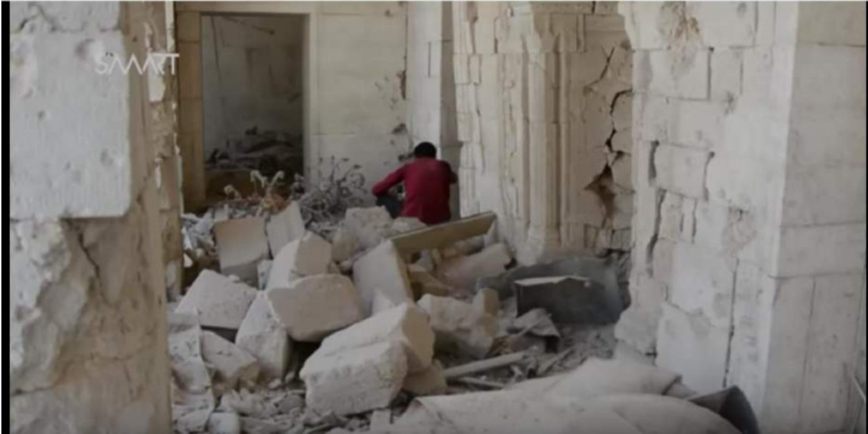
Video still of damage to al-Saleheen Mosque (SMART News Agency; July 16, 2016)
