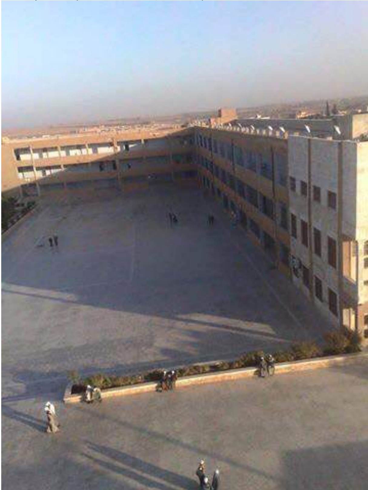
al-Sharaya School prior to any damage (Manbij News; shared July 12, 2016)
