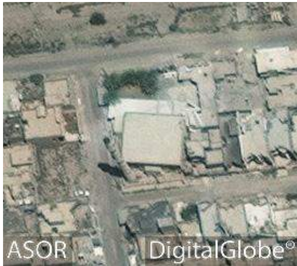
Previous damage to the metal roof over the courtyard of the al-Mudallal Mosque (DigitalGlobe; May 31, 2016)
