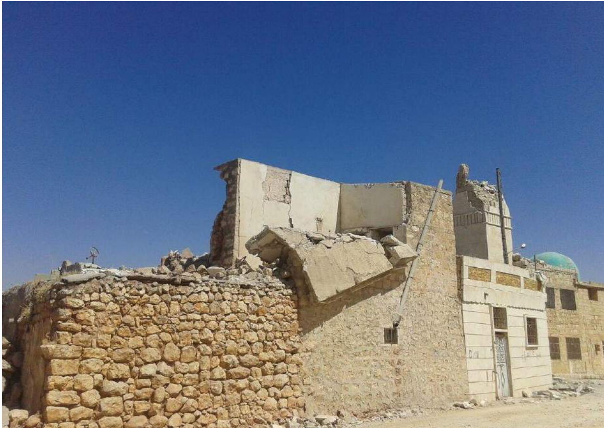
Damage to minaret of Tawabin Mosque (Leiramoun al-Hadath/Facebook; July 13, 2016)
