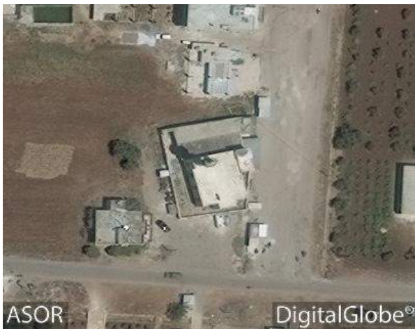
al-Musafir Mosque prior to damage (DigitalGlobe; May 30, 2016)
