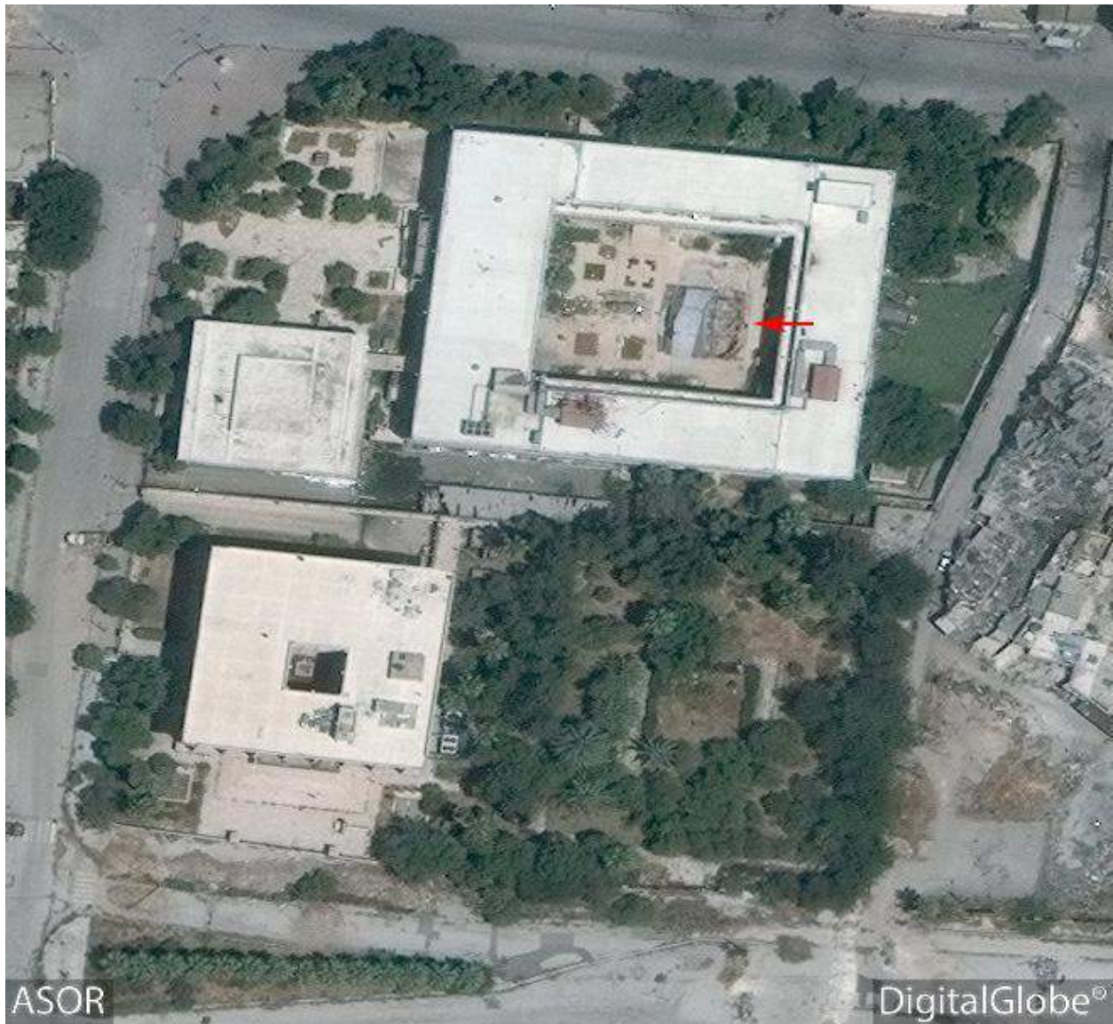
Aleppo Museum prior to the most recent damage. Clear visible damage to the main courtyard and there are possibly stone statues under the metal roof that may have suffered damage as well (DigitalGlobe; June 24, 2016)
