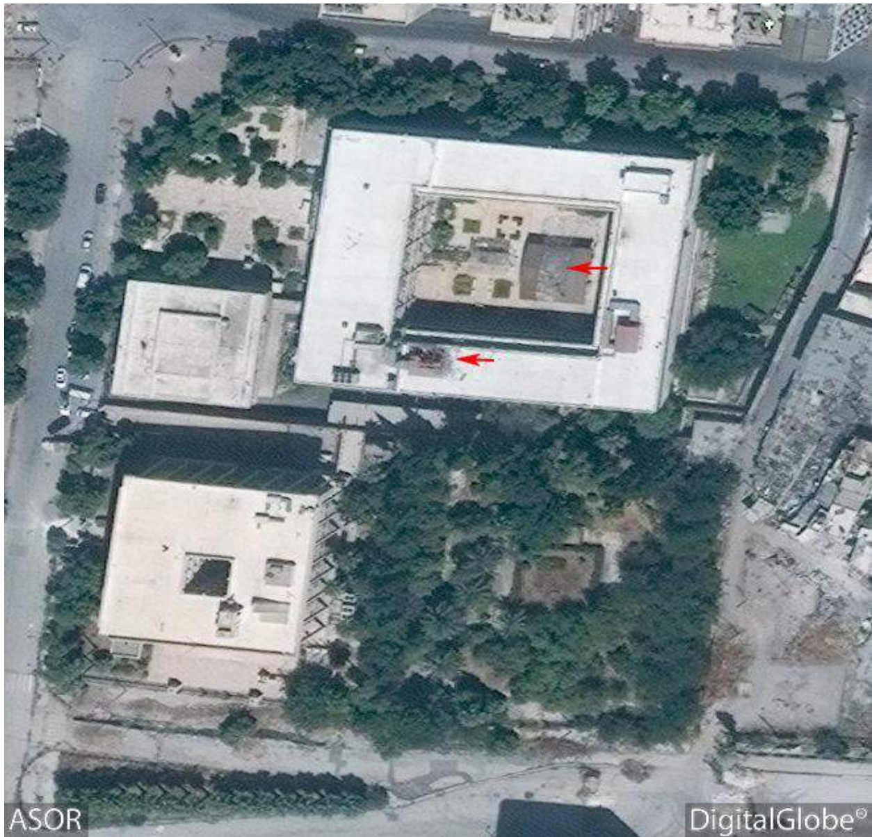
Aleppo Museum Complex showing previous damage from 2014 to the electrical transformer. Additional damage appears in the courtyard (DigitalGlobe; August 18, 2015)
