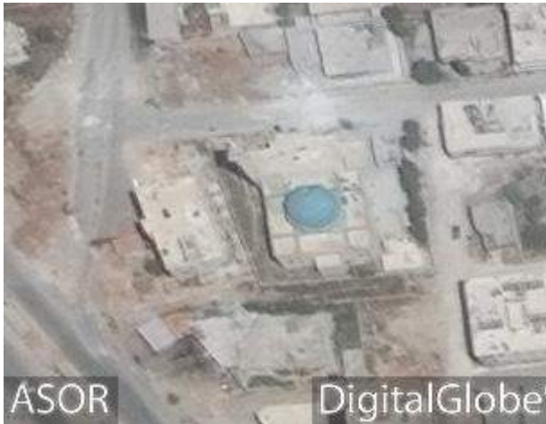
Al Baraa Bin Malek Mosque partially damaged (DigitalGlobe; May 22, 2016)
