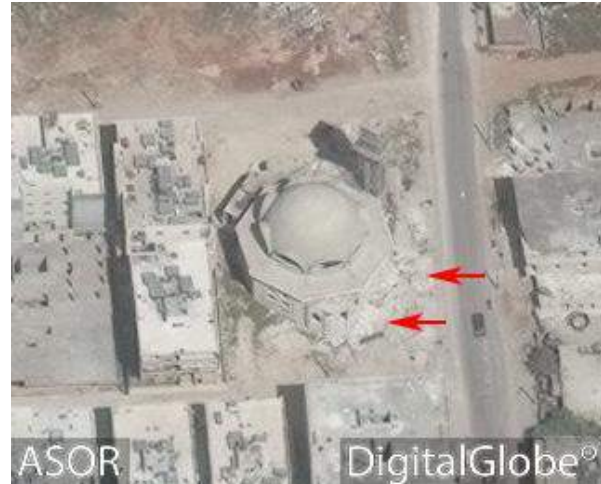
Visible damage to the windows and eastern wall of the mosque (DigitalGlobe; April 15, 2016)
