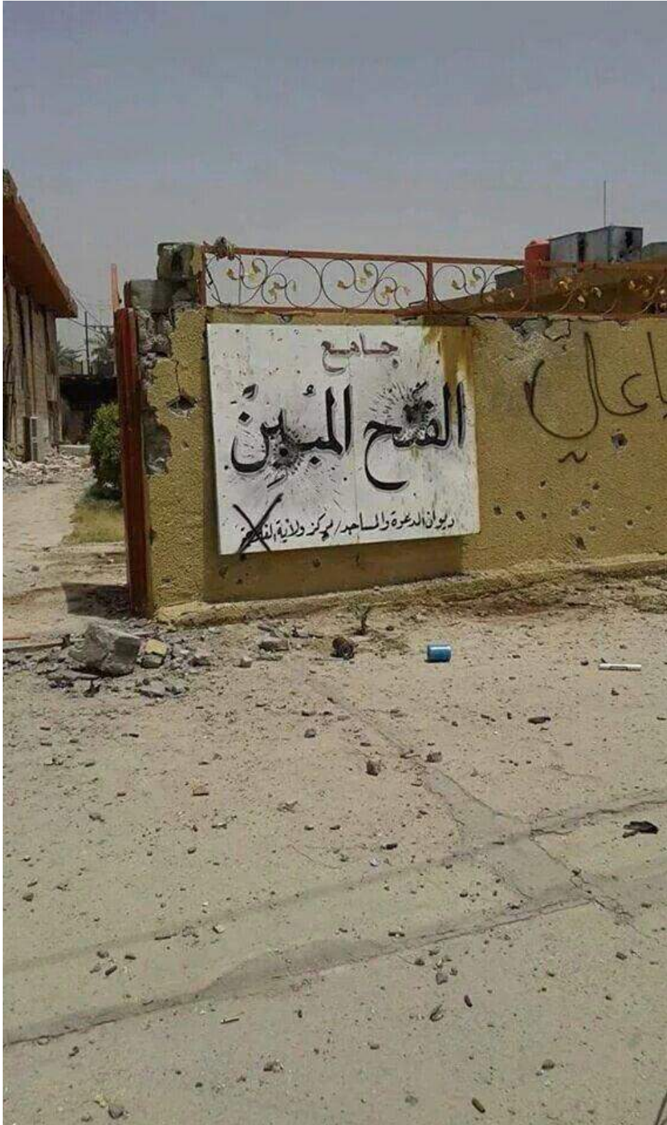
Vandalism and damage to al-Fath al-Mudin Mosque entrance (Twitter; July 10, 2016)
