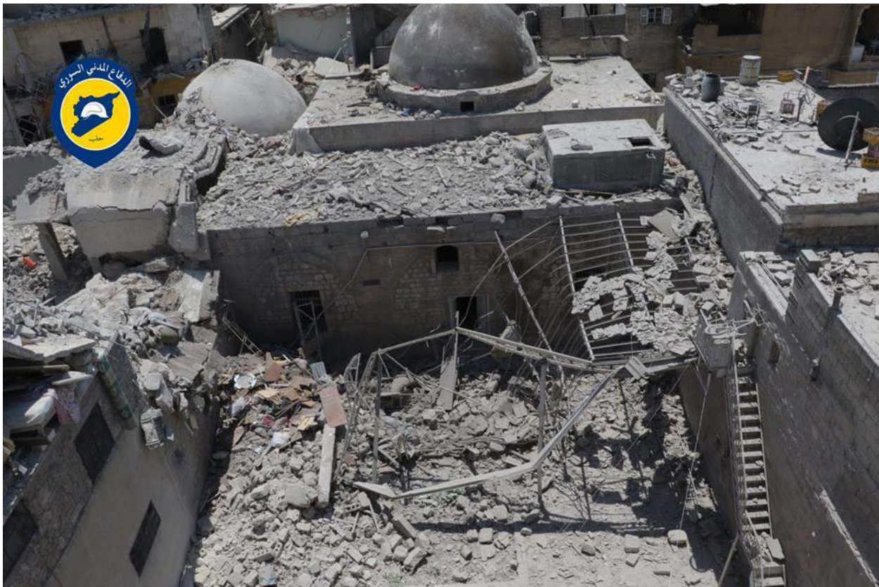
Severe damage to al-Maqamat Mosque (SNHR; July 16, 2016)
