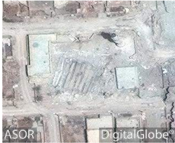
Complete destruction of al-Anbia Mosque (DigitalGlobe; June 28, 2016)
