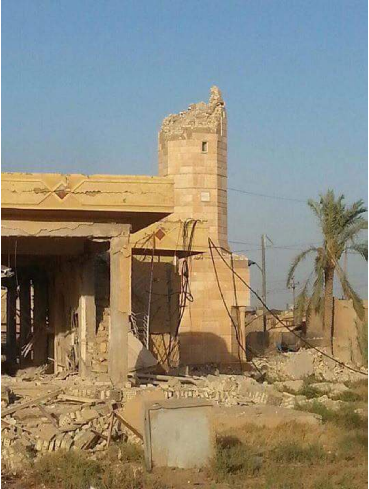
Destruction of al-Taqwa Mosque (Twitter; July 9, 2016)
