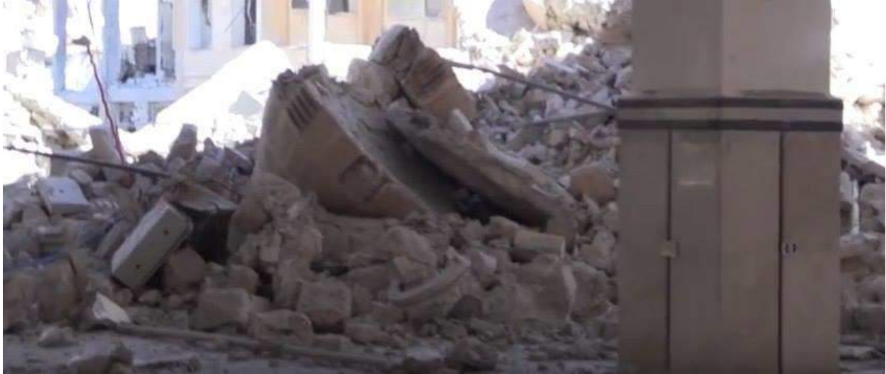
Detail of damage to al-Miqdad Mosque (Manbej Mubashar; July 13, 2016)
