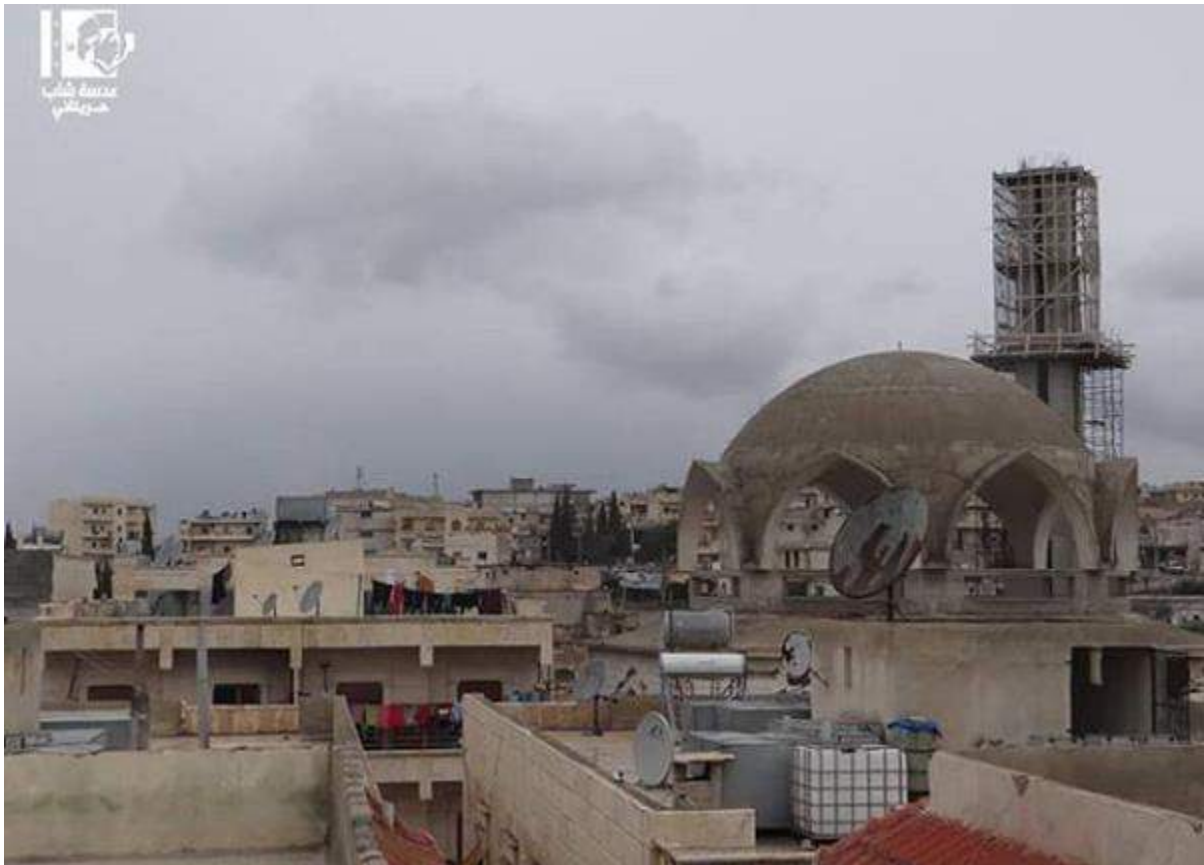
al-Quds Mosque and scaffolding (Hreitan City; January 13, 2016)
