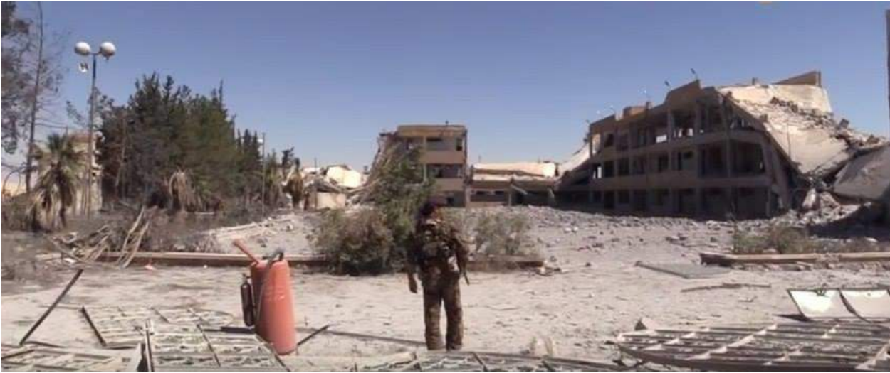
Damage to al-Sharaya School (Manbej Mubashar; July 13, 2016)
