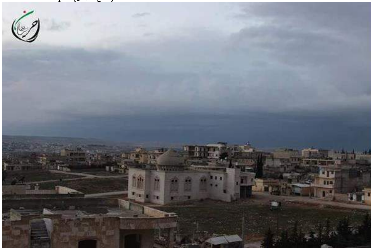
al-Abbas Mosque as it appeared on January 18, 2016 showing some minor damage to the dome (Hreit City; January 18, 2016)
