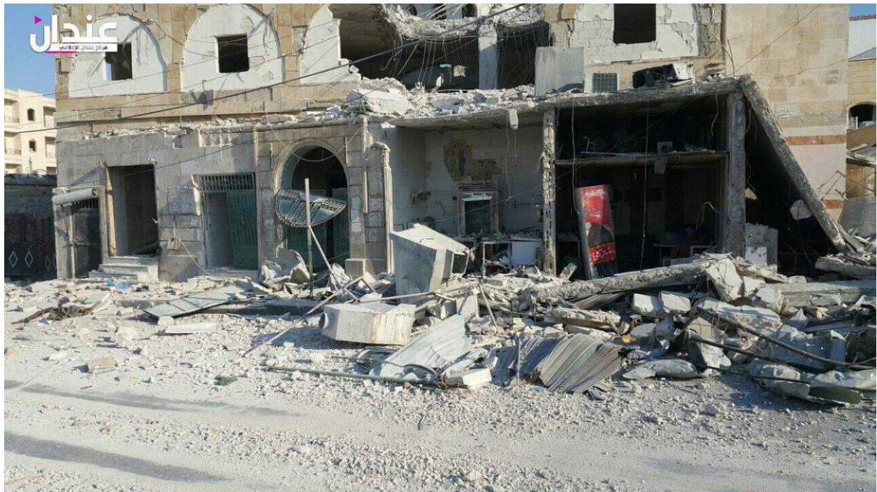
Severe damage to Abu Bakr al-Sidiq Mosque (SNHR/Twitter; July 14, 2016)
