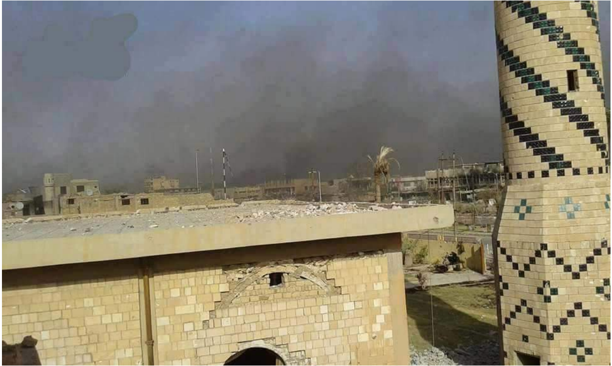
Damage to facade and roof of al-Fath al-Mubin Mosque (Ahrar al-Rafidain Network for Human Rights/Facebook; July 4, 2016)
