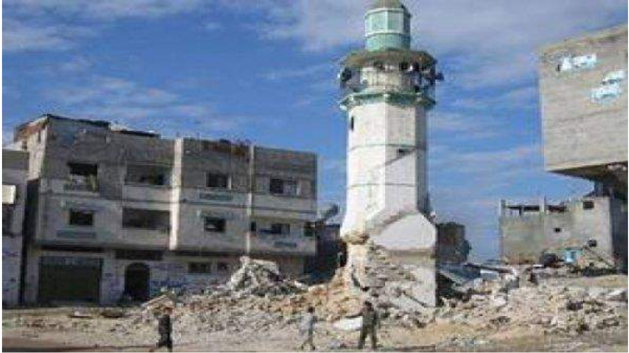
Damage to Shuhada al-Aqsa Mosque in 2013 (El Dorar; March 9, 2013)
