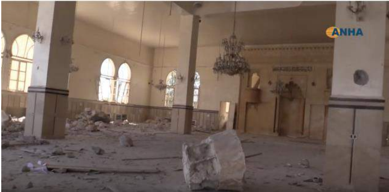
Interior damage to al-Miqdad Mosque (ANHA; July 11, 2016)
