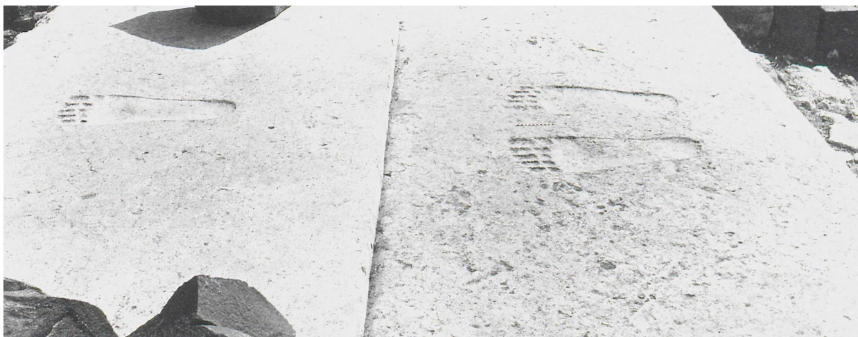
The carved thresholds in the entrance at the end of excavation, seen from the southwest (Assaf 1990: Taf. 11b)
