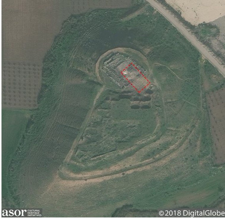
Damage from attack on Tell Ain Dara temple, with debris field indicated by the red box (DigitalGlobe NextView License; January 29, 2018)
