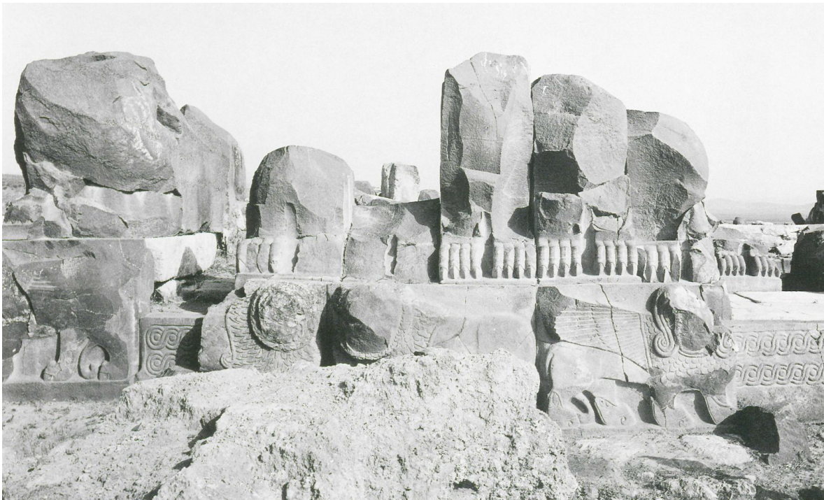
The facade west of the entrance at the end of excavation, seen from the southeast (Assaf 1990: Taf. 36b)
