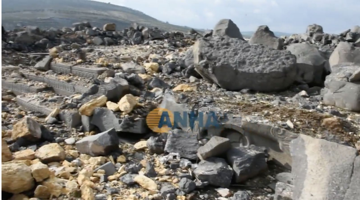
Video still of the temple facade east of the entrance after the attack, seen from the east (ANHA; January 27, 2018)
