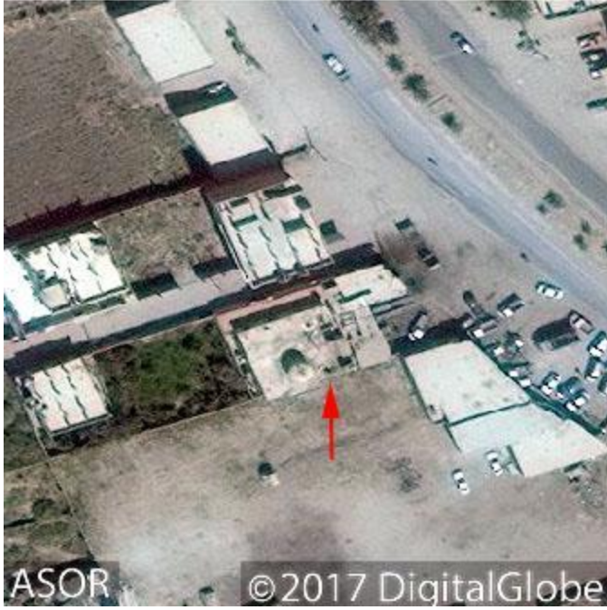
The unnamed mosque with a red arrow indicating previous damage to the roof (DigitalGlobe NextView License; September 7, 2017)
