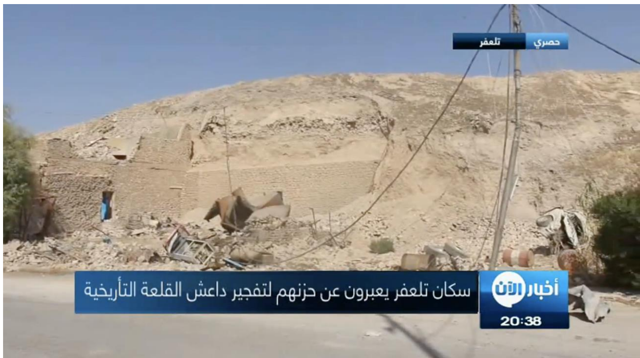
Video still of damage to buildings around the base of the mound, seen from the west (Al-Aan Arabic Television; October 4, 2017)
