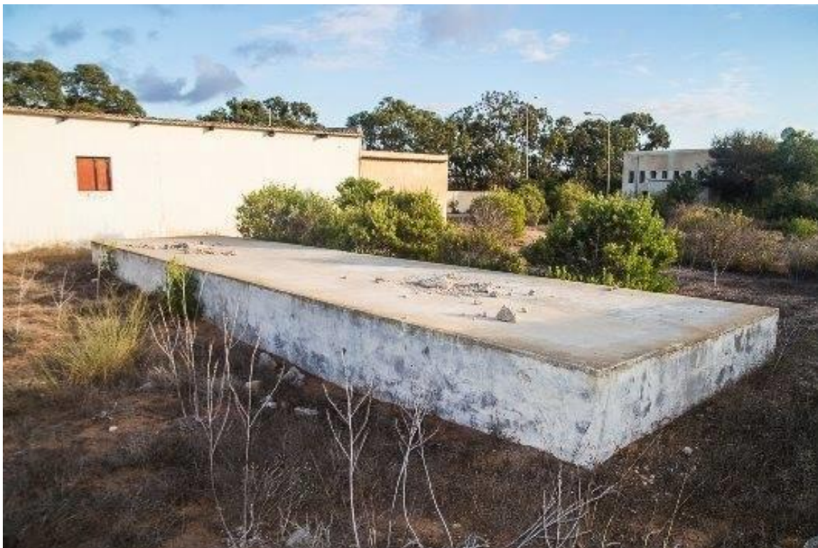
Platform after the removal of the bronze statues (Khalid Aljohre; October 15, 2017)
