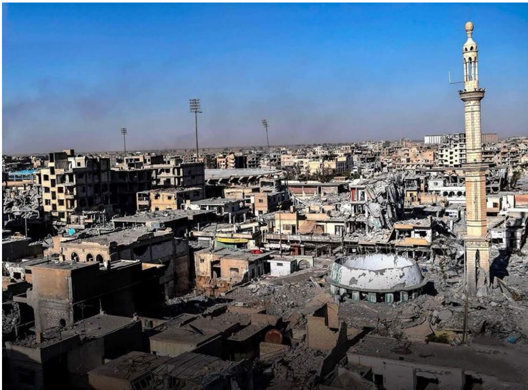
Damage to al-Firdous Mosque (RBSS; October 17, 2017)
