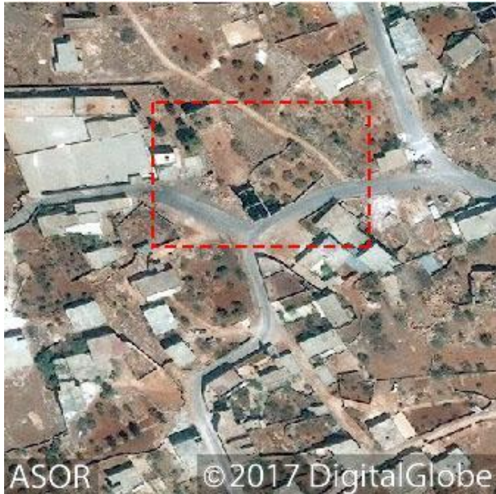
Villa in Deir Sunbul prior to any significant damage shown within the red box (DigitalGlobe NextView License; September 10, 2014)
