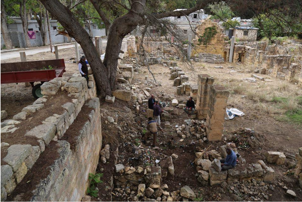
Overview of the area targeted for maintenance (DoA Shahat; October 11, 2017)
