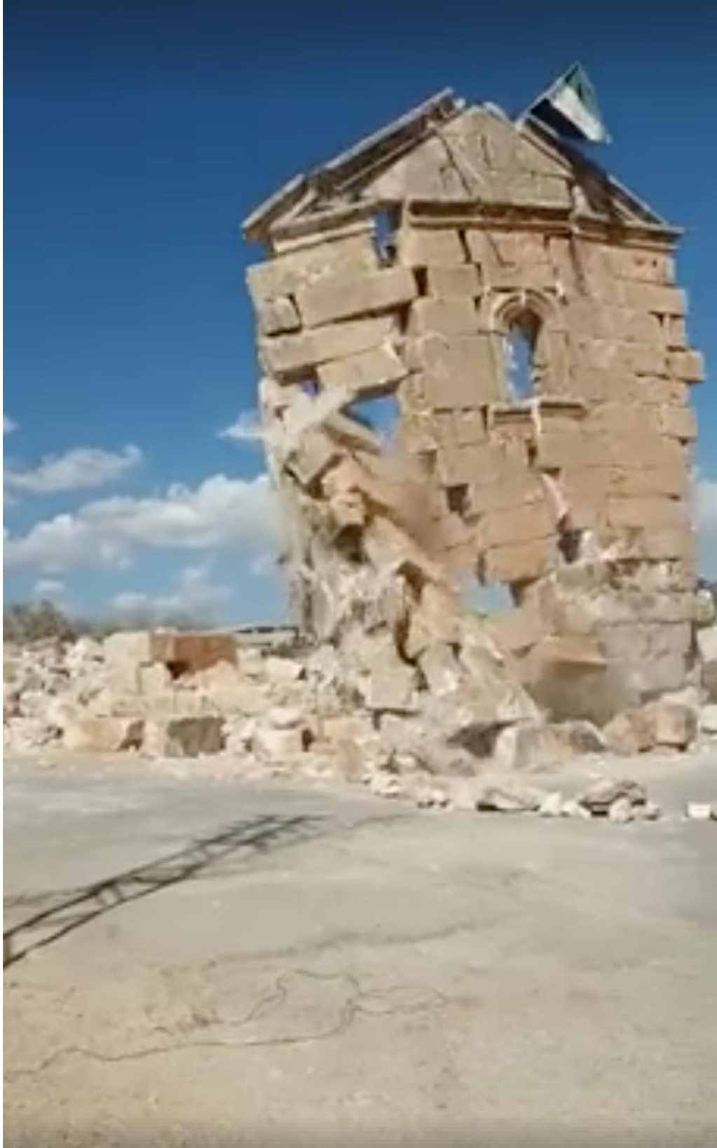
Video still of the collapse of the monument (Aleppo Archaeology; October 4, 2017)
