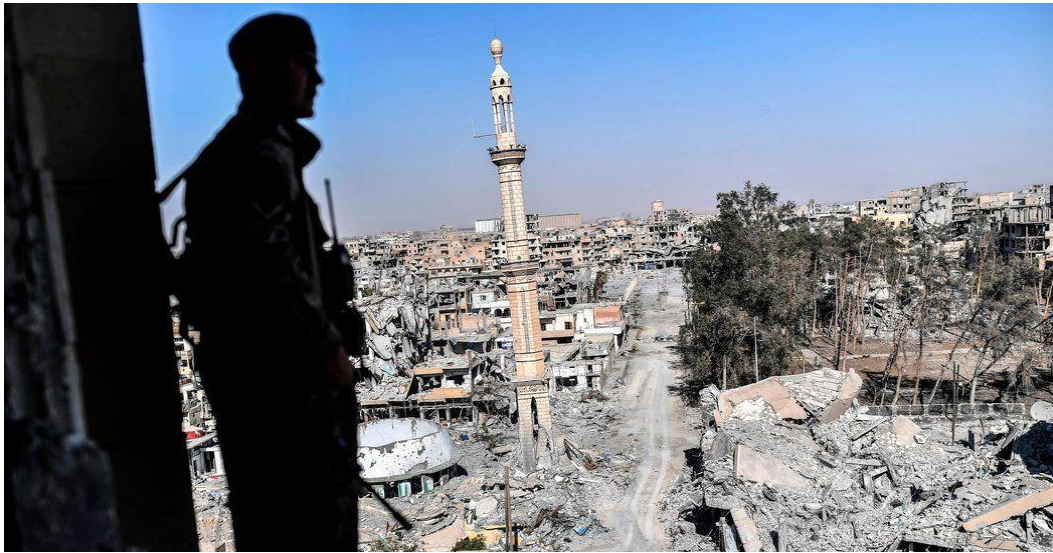
Damage to al-Firdous Mosque (CIVIC; October 17, 2017)
