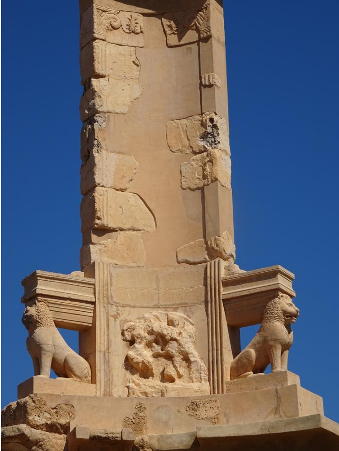
Superficial damage to the Punic funerary Mausoleum of Bes (Hafed Walda; October 9, 2017)
