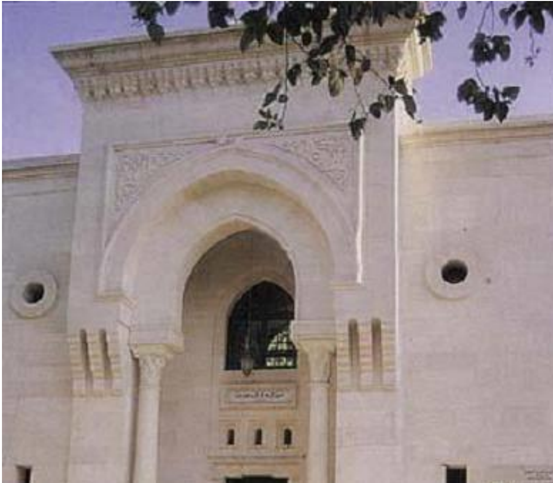
Pre-damage photograph of north facade of cultural center (al-Maara Education Center/Facebook; undated)
