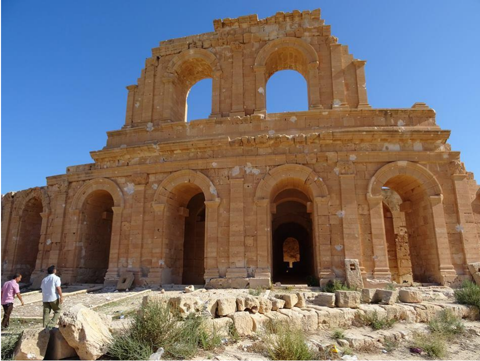
Damage to the Sabratha theatre (Hafed Walda; October 9, 2017)
