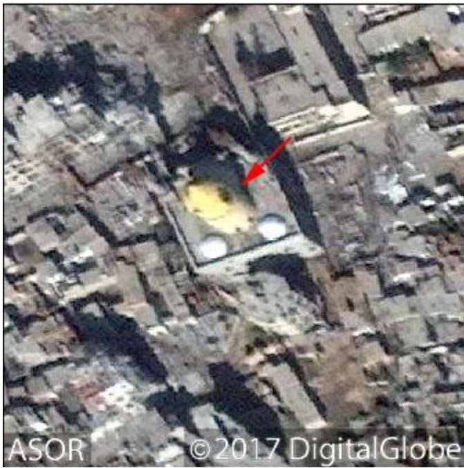
Initial damage to the dome of the shrine as indicated by the red arrow, possibly from an airstrike (DigitalGlobe NextView License; November 20, 2013)
