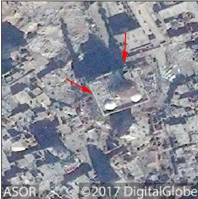
Increased damage to the roof of the shrine in the form of holes, possibly from airstrikes, indicated by red arrows (DigitalGlobe NextView License; December 23, 2014)
