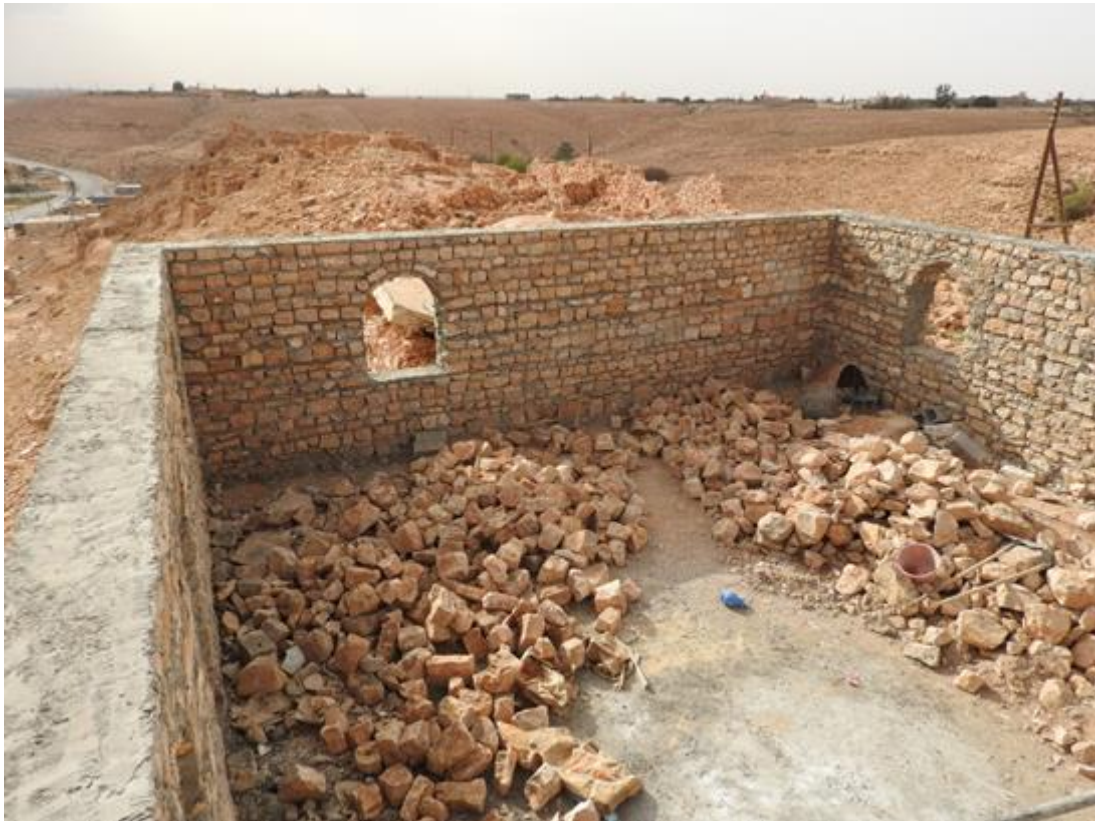
Work to rebuild walls (Sufian ad Debib; October 29, 2017)
