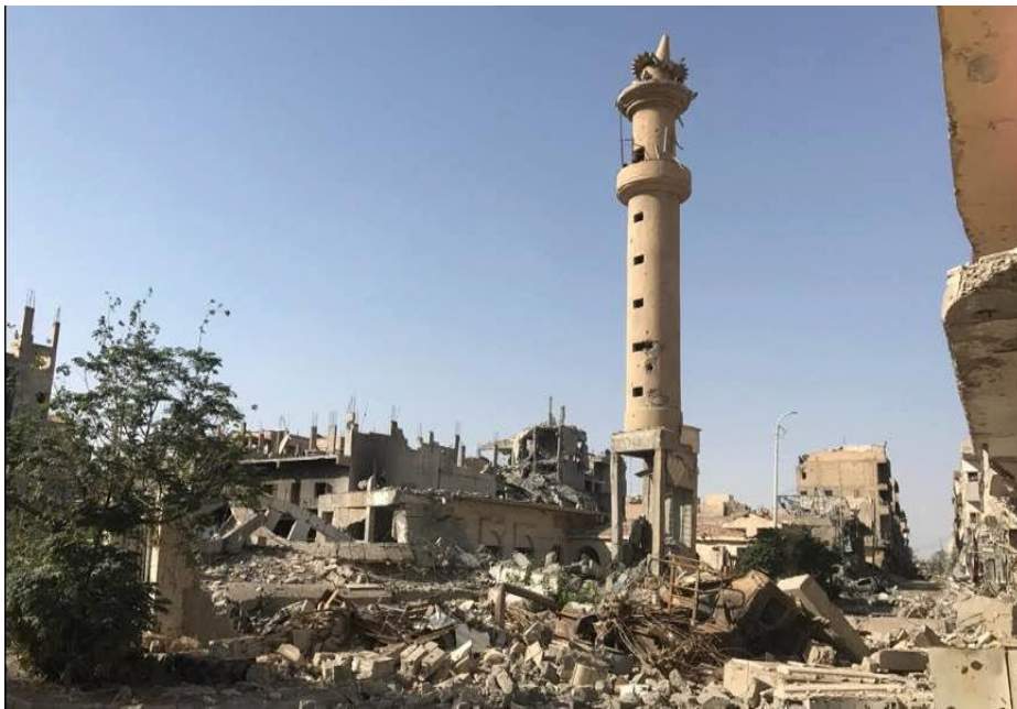
Destruction of the Circassian Mosque and damage to minaret (RBSS; October 19, 2017)
