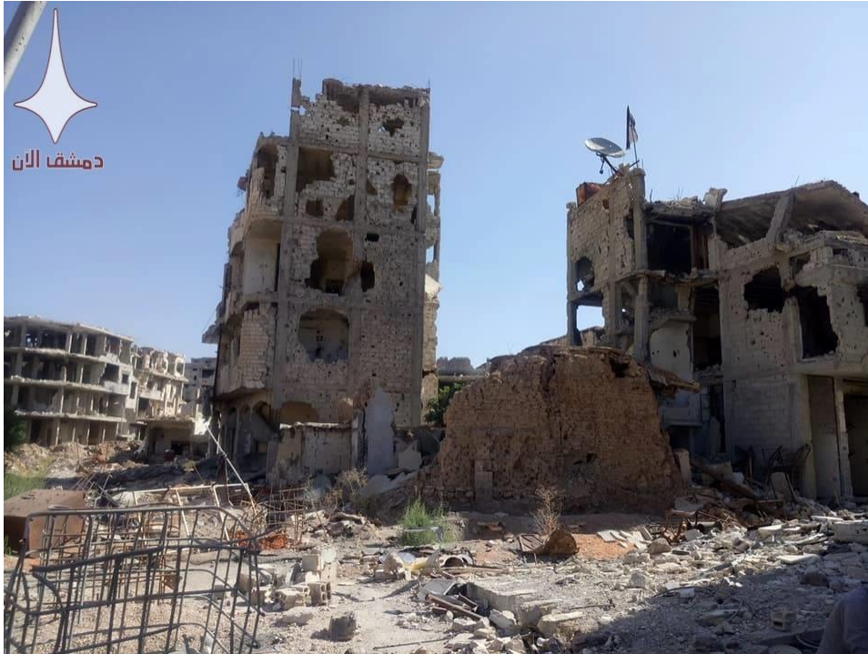
Photograph of damage to the area surrounding the shrine (Private Facebook Account; October 8, 2017)
