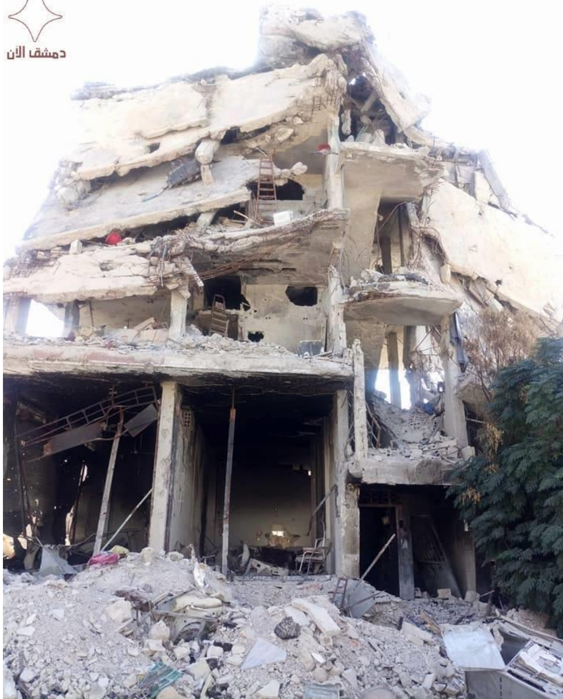
Photograph of damage to the shrine (Private Facebook Account; October 8, 2017)
