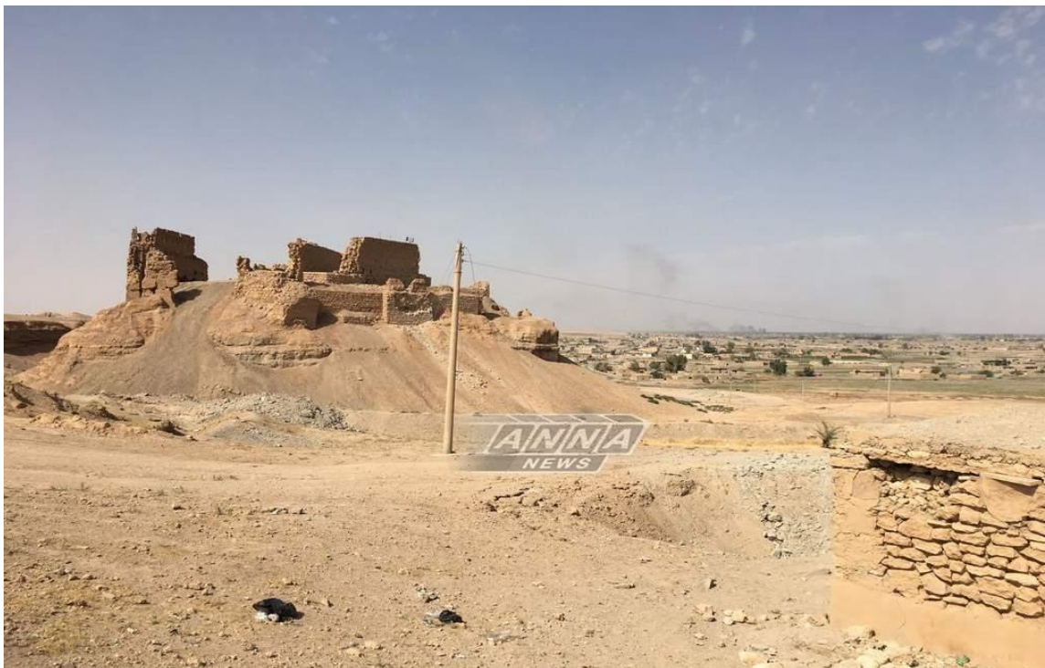
Qalaat Rahba, seen from the southeast. The soil discoloration along the left side of the image is likely the result of foot traffic into the site's interior (ANNA News; October 8, 2017)
