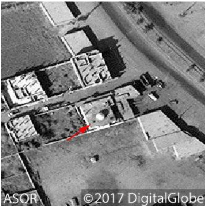
A new hole in the roof of the mosque indicated by a red arrow (DigitalGlobe NextView License; October 15, 2017)
