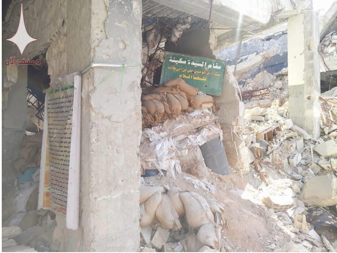
Photograph of damage to the shrine (Private Facebook Account; October 8, 2017)
