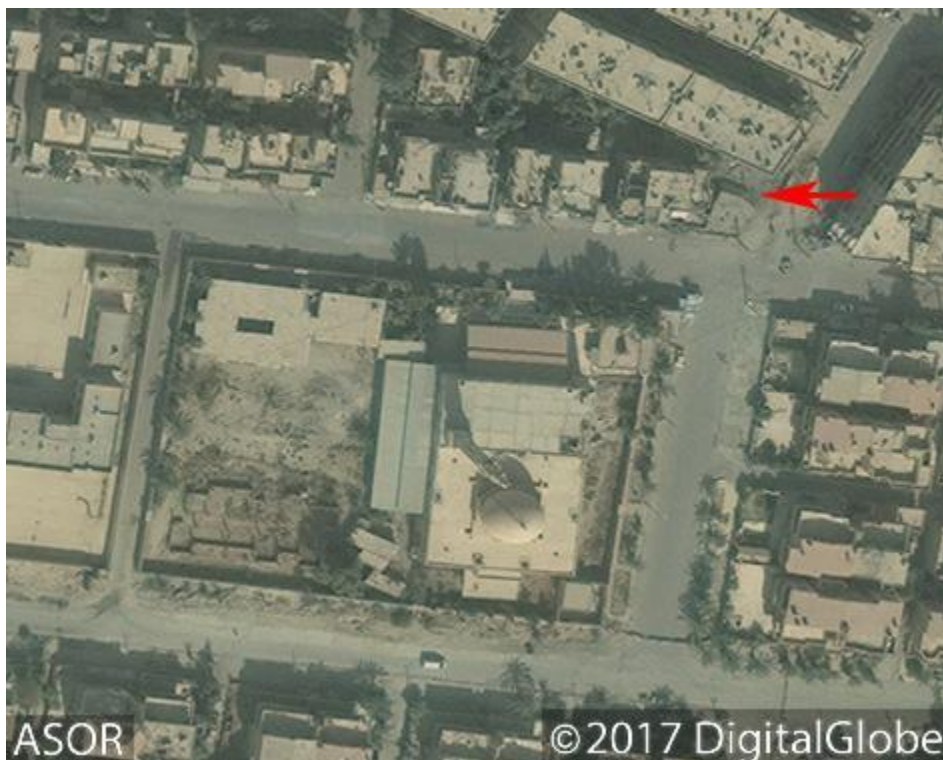
Damage to building close to al-Fateh Mosque after reports of shelling (DigitalGlobe NextView License; October 27, 2017)
