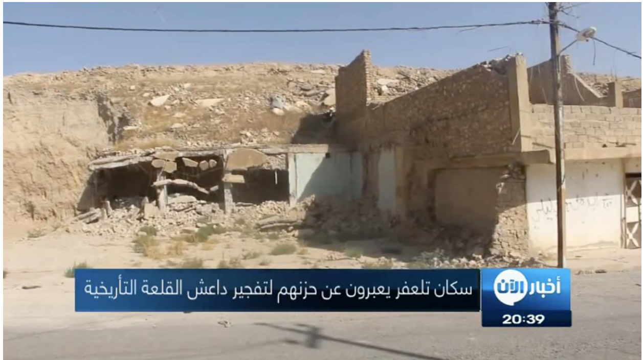
Video still of damage to buildings around the base of the mound as well as an area where ISIS looted the site with earthmoving equipment, seen from the west (Al-Aan Arabic Television; October 4, 2017)
