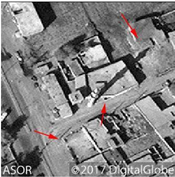
A hole visible in the southern roof of the mosque just east of the minaret is indicated by a red arrow. Nearby damage is indicated by red arrows (DigitalGlobe NextView License; October 15, 2017)
