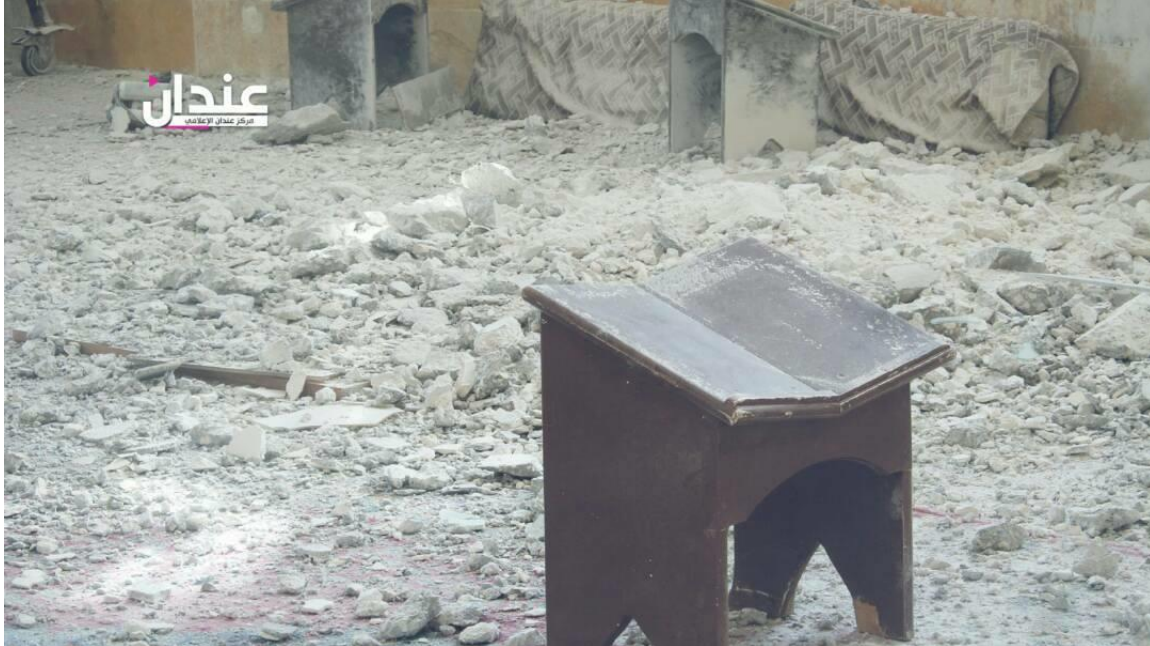
Rubble in mosque interior (Anadan Media Center; October 12, 2017)
