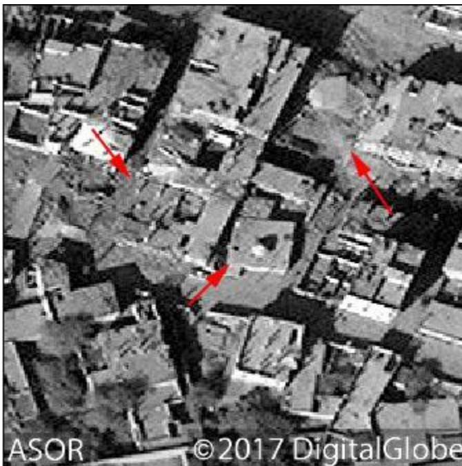
An arrow indicates the hole in the roof of the mosque. Other arrows indicate damage in surrounding area (DigitalGlobe NextView License; October 15, 2017)
