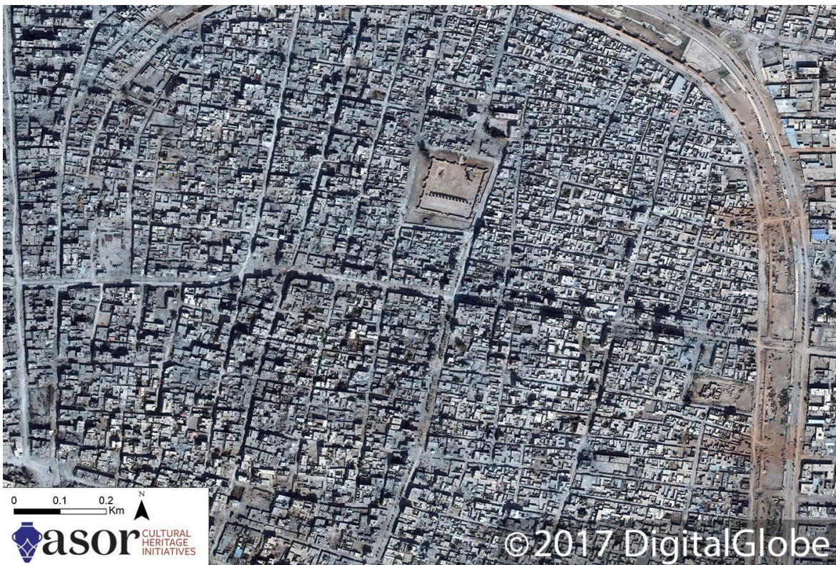
Old City of Raqqa with severe damage (DigitalGlobe NextView License; October 21, 2017)
