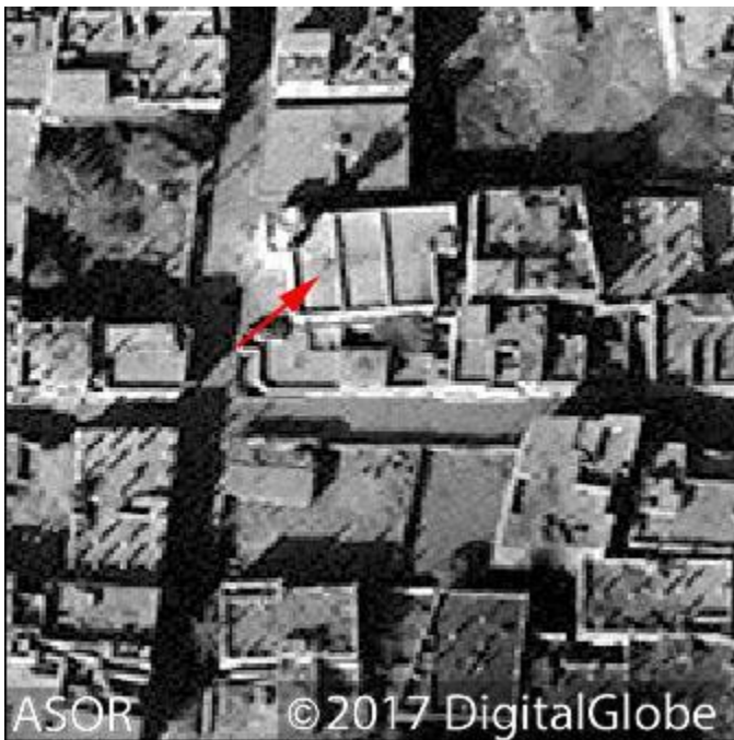
A hole in the roof of the mosque indicated by a red arrow (DigitalGlobe NextView License; October 15, 2017)
