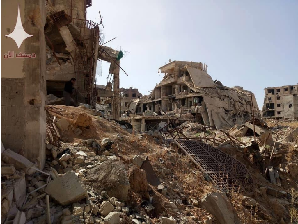
Photograph of damage to area surrounding the shrine (Private Facebook account; October 8, 2017)
