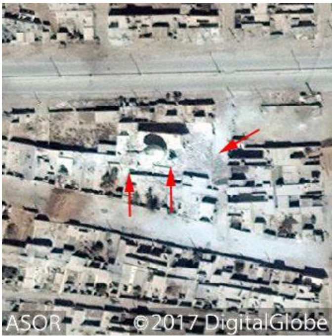
The southern half of the mosque is severely damaged likely by an airstrike, as indicated by the red arrows (DigitalGlobe NextView License; September 30, 2017)
