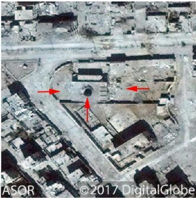
Damage to the dome of the mosque as well as to the surrounding area of the mosque as indicated by red arrows (DigitalGlobe NextView License; October 19, 2017)
