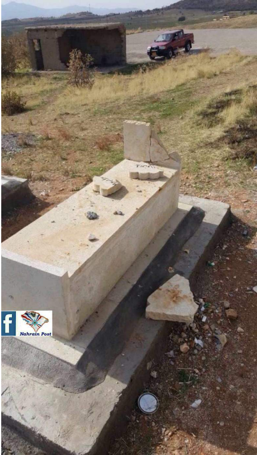
Damage to graves in Christian cemetery (Nahrain Post; November 28, 2017)
