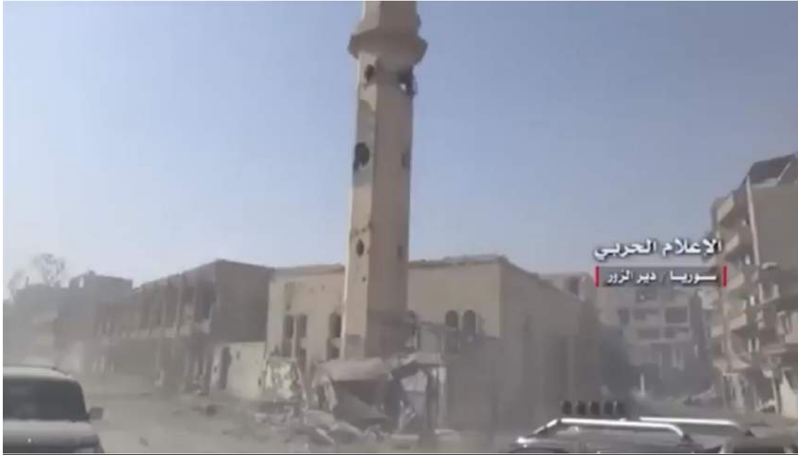
Video still of damage to the mosque's minaret, seen from the northeast (Private Twitter Account; November 3, 2017)
