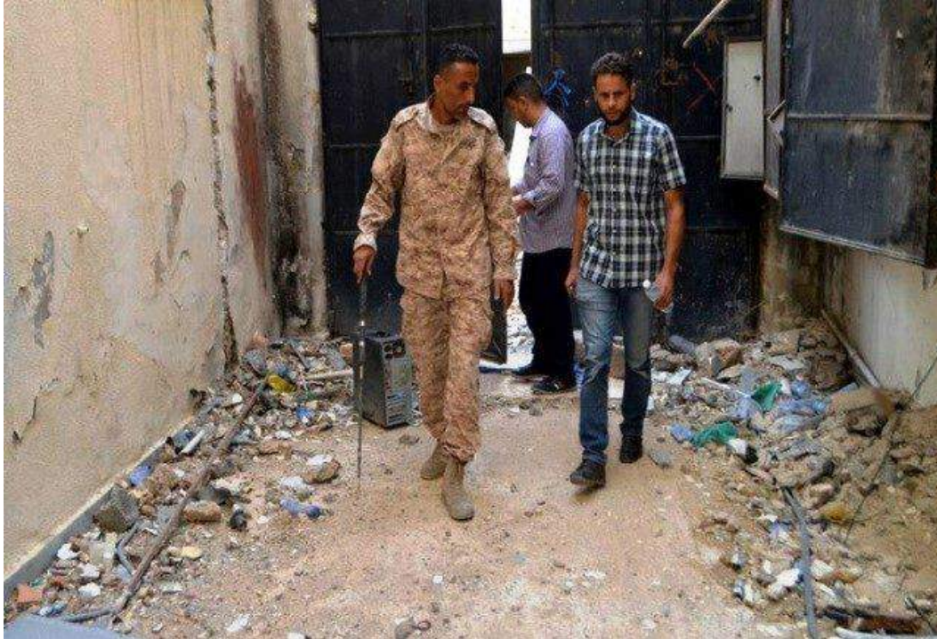
Damaged interior of the Qasr al Manar (Libyan Antiquities Authority; November 2, 2017)
