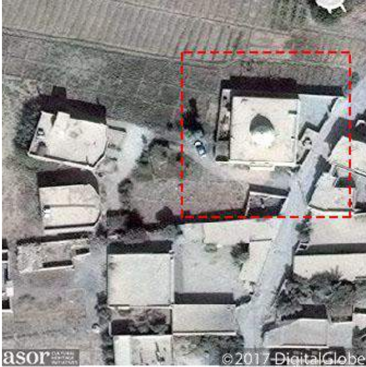
al-Taas Mosque shown in rectangle prior to any visible damage (DigitalGlobe NextView License; October 26, 2017)
