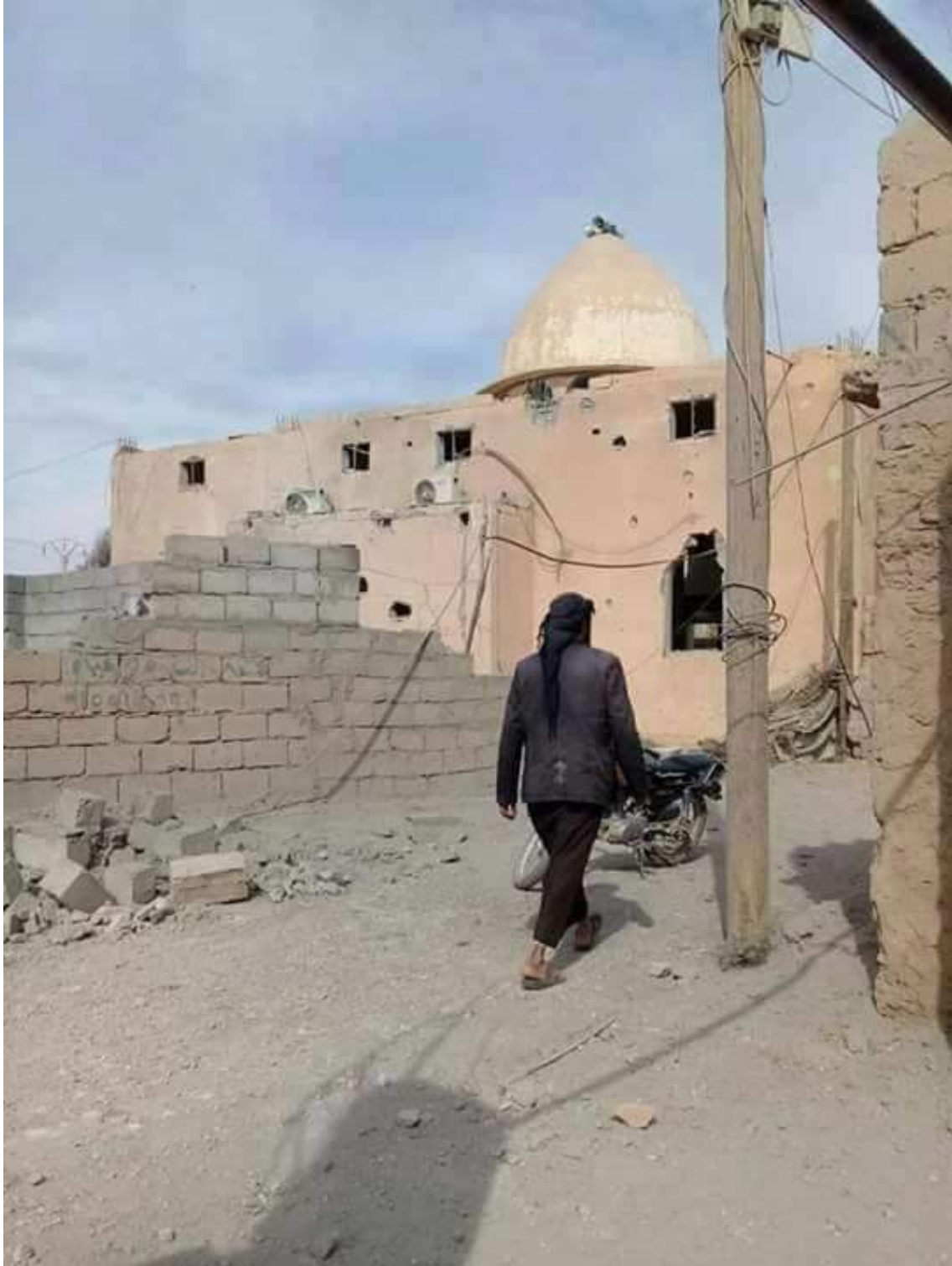
Missile damage to al-Taas Mosque (SNHR; November 1, 2017)
