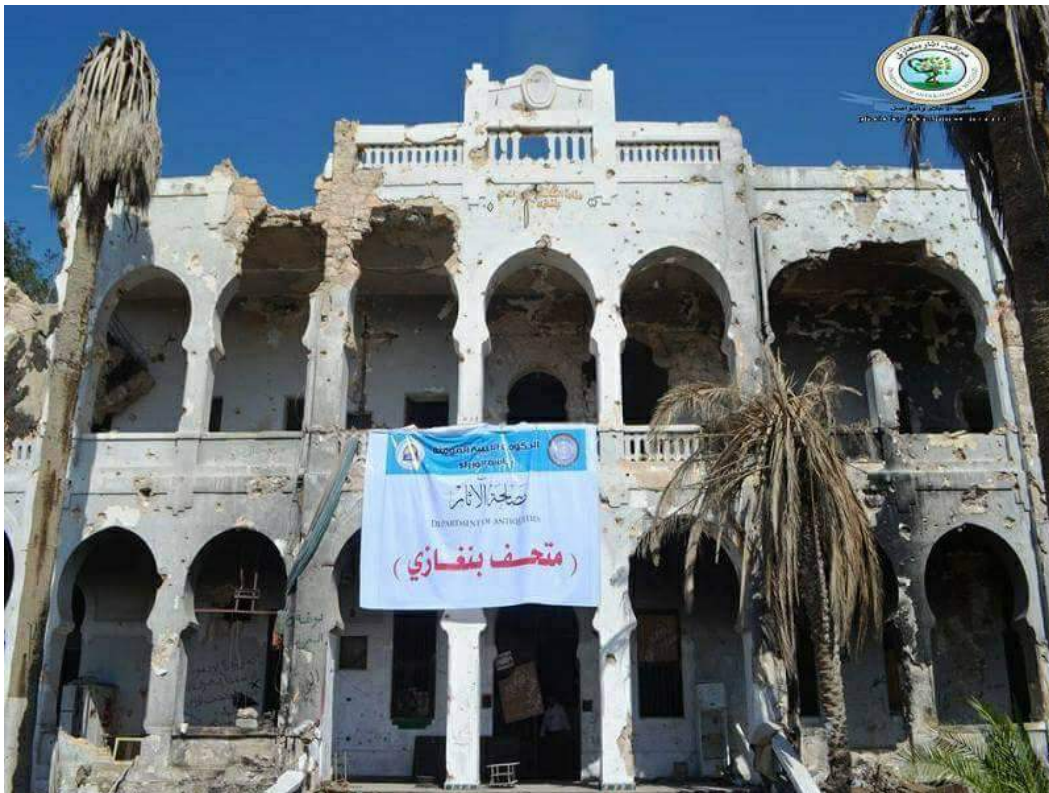
Damaged exterior of Qasr al Manar (November 21, 2017)
