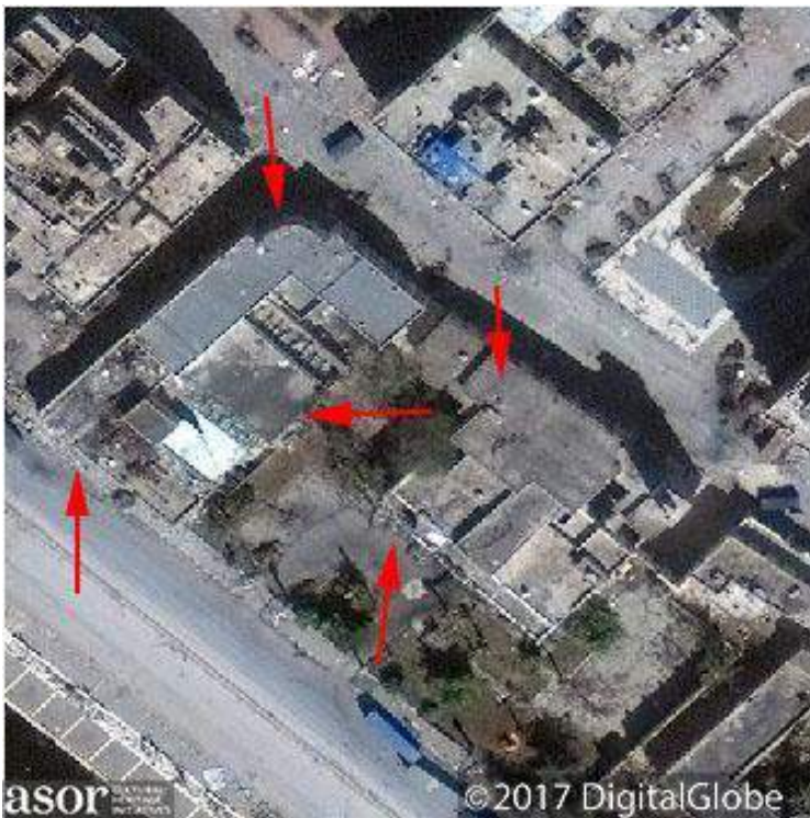
Various instances of damage to the building as a result of continuous warfare, as indicated by red arrows (DigitalGlobe NextView License; March 6, 2016)
