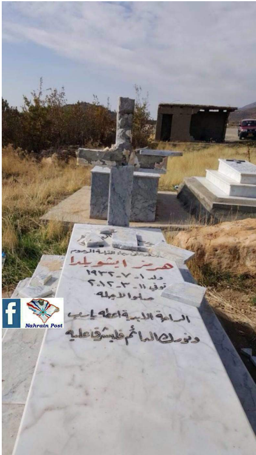
Damage to graves in Christian cemetery (Nahrain Post; November 28, 2017)
