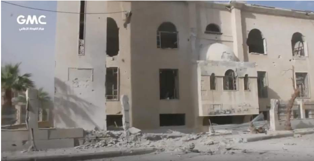
Damage to the exterior of al-Kabir Mosque (SNHR; November 16, 2017)
