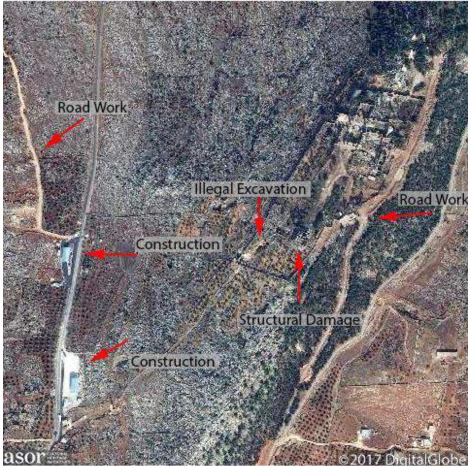
All recent damage to the site of Deir Semaan indicated by red arrows (DigitalGlobe NextView License; November 9, 2017)
