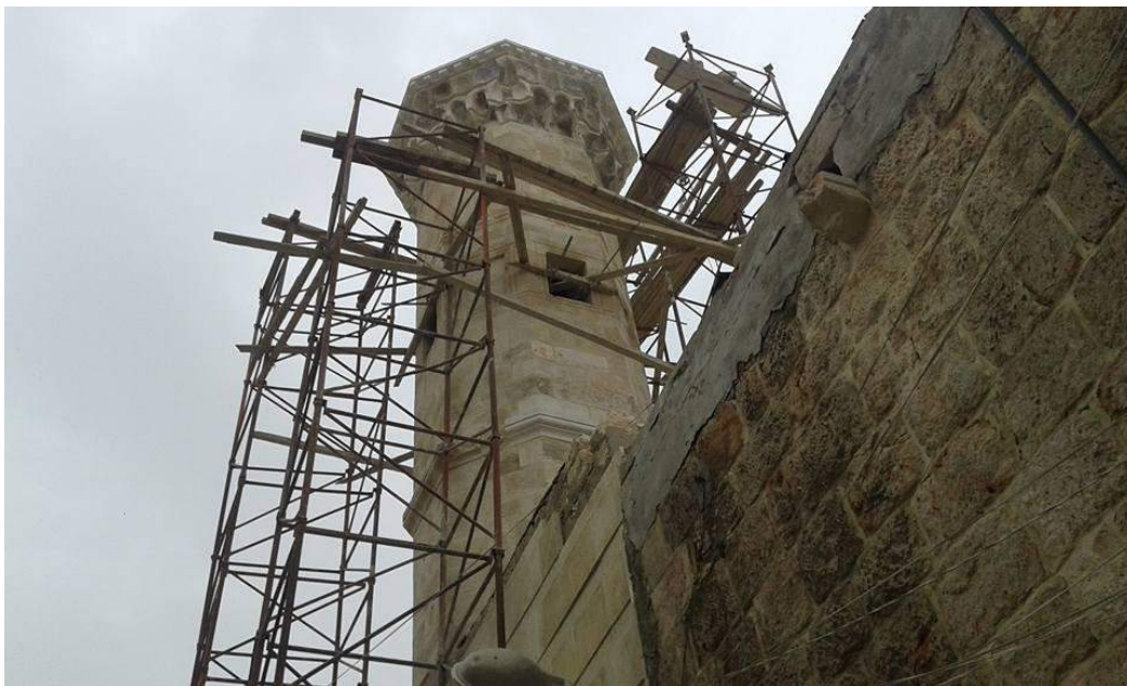
Restoration of the minaret (Private Facebook Account; November 20, 2017)
