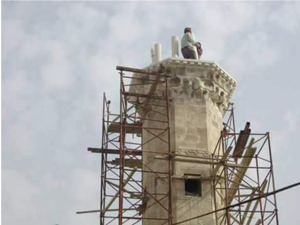
Restoration of the minaret (Private Facebook Account; November 20, 2017)
