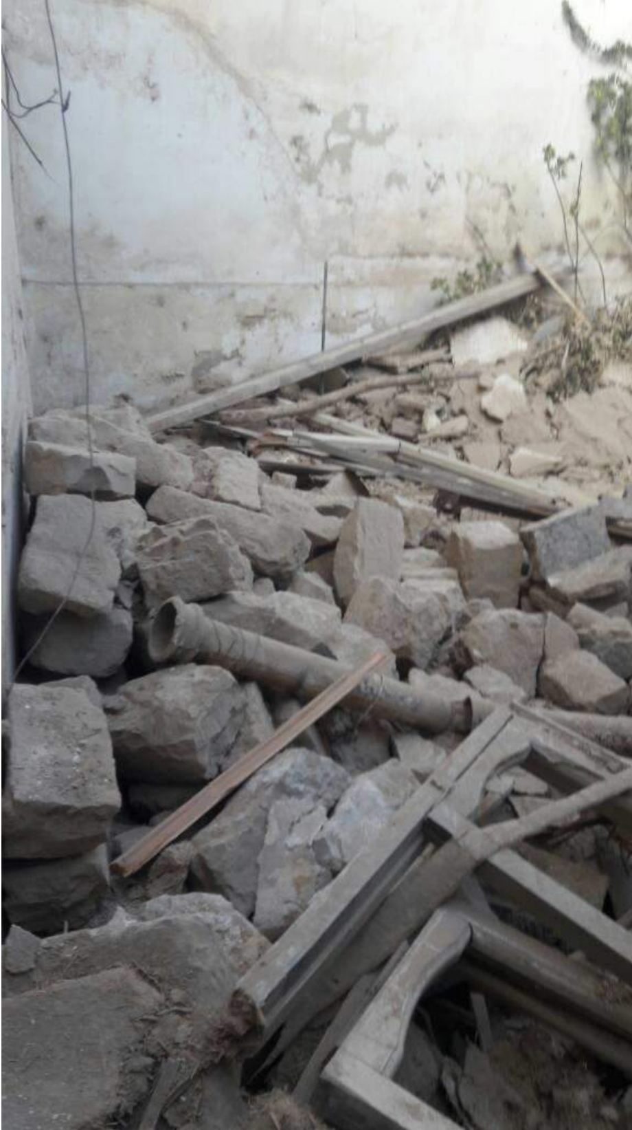
Collapse of house in Old Damascus (DGAM; November 2, 2017)
