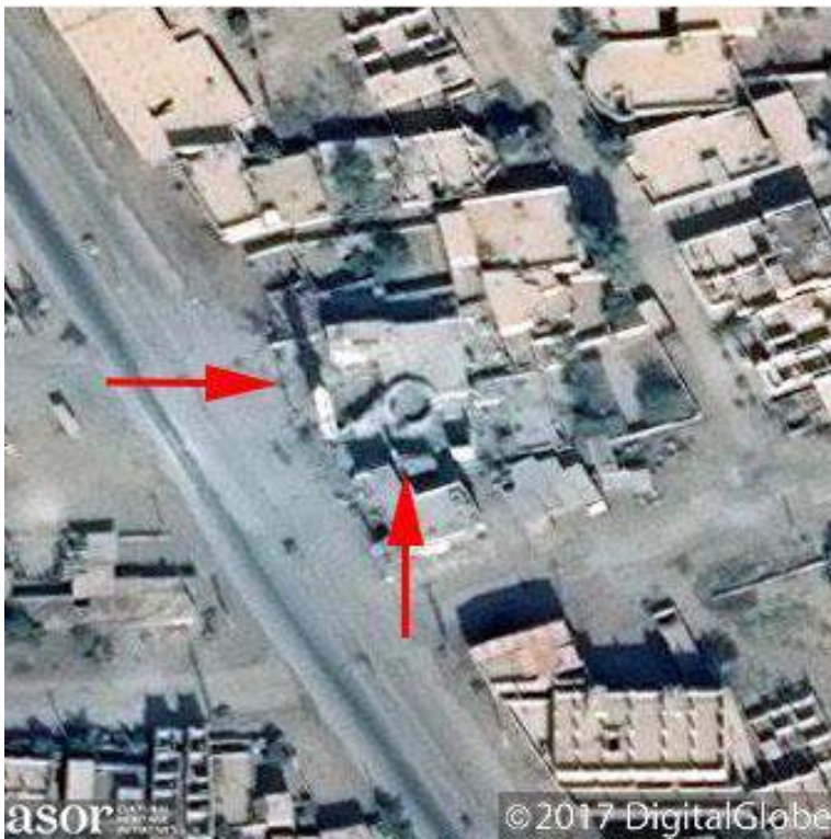
Damage to the dome and southwest quarter of the mosque as indicated by red arrows (DigitalGlobe NextView License; November 7, 2017)
