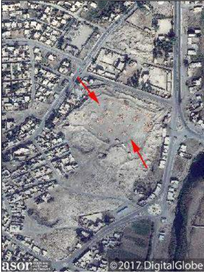
Red arrows indicate the destroyed modern structures on the site (DigitalGlobe NextView License; November 2, 2017)
