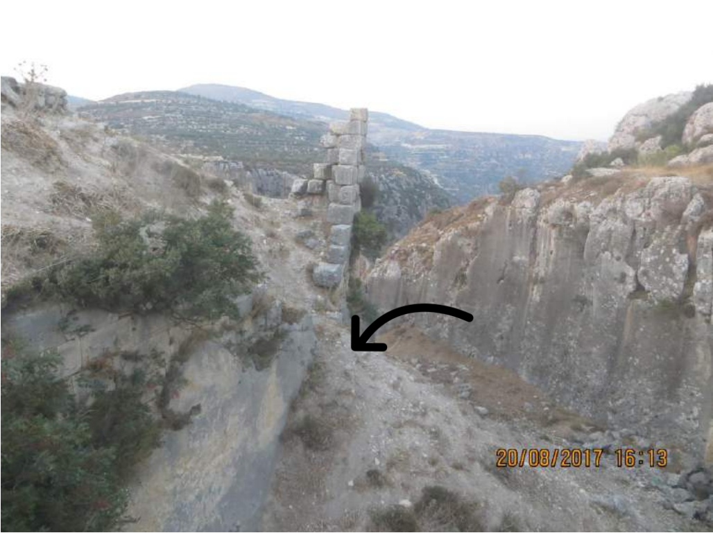
Collapse due to environmental /weathering
