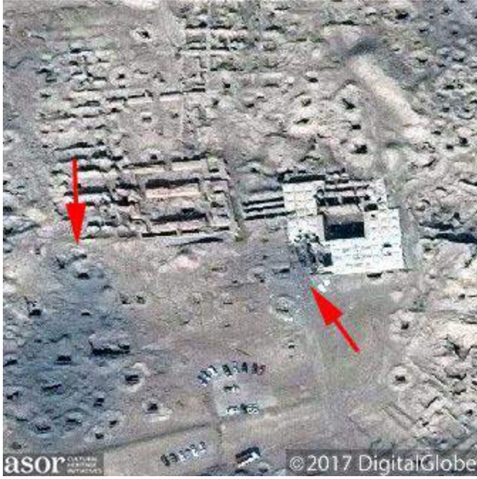
Damage to the southwestern part of the structure, as well as visible smoke and scorch marks, indicated by red arrows (DigitalGlobe NextView License; November 13, 2017)
