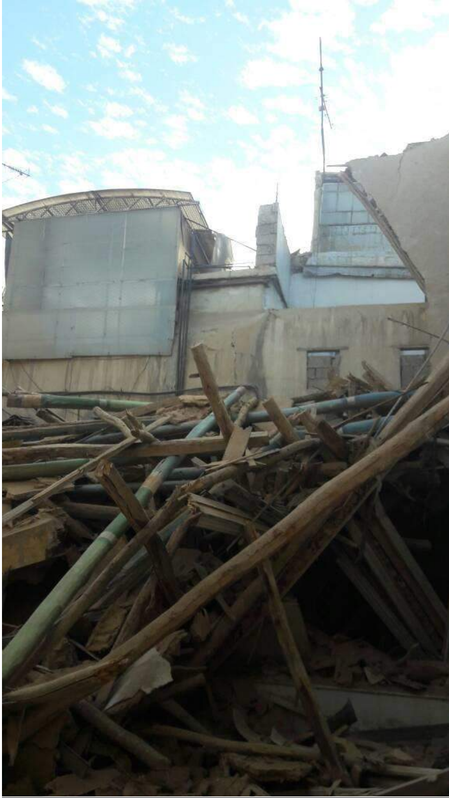
Collapse of house in Old Damascus (DGAM; November 2, 2017)
