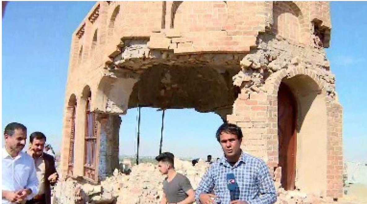
Video still of damage to top section of castle (Kurdistan24; November 14, 2017)
