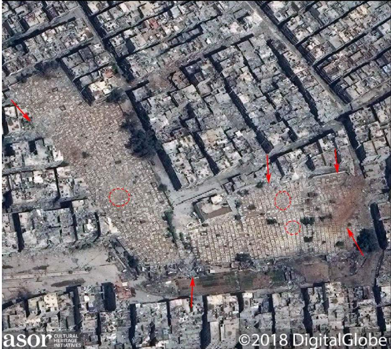
Previous damage to the Palestinian Martyrs Cemetery (DigitalGlobe NextView License; April 27, 2018)
