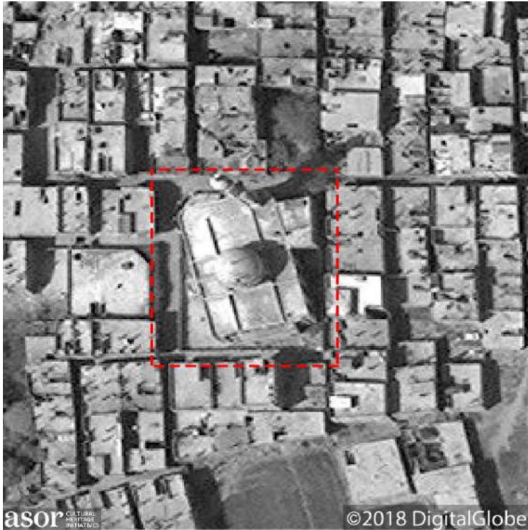
The unnamed mosque prior to military damage (DigitalGlobe NextView License; April 20, 2018)
