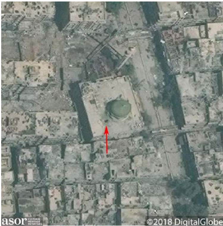
Initial military damage to the roof of al-Wasim Mosque, as indicated by the red arrow (DigitalGlobe NextView License; April 27, 2018)
