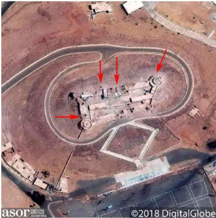
Increased damage visible on the northern wall of Sabha Castle. The central tower appears to have suffered from shelling and explosives, as evidenced by the holes and visible structural damage. There also appears to be damage to the northeast tower and the extent of damage to the western wall is clearly visible by a new hole, indicated by a red arrow (DigitalGlobe NextView License; May 21, 2018)
