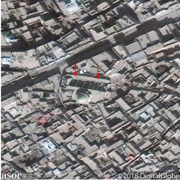
Al-Mahmudin Mosque with a missing roof section indicated by red arrows (DigitalGlobe NextView License; February 8, 2018)
