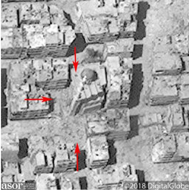
Increased damage to the Jerusalem Mosque indicated by red arrows. A hole is visible on the northwestern side of the roof of the mosque and the buildings south and west of the mosque have been destroyed (DigitalGlobe NextView License; May 11, 2018)
