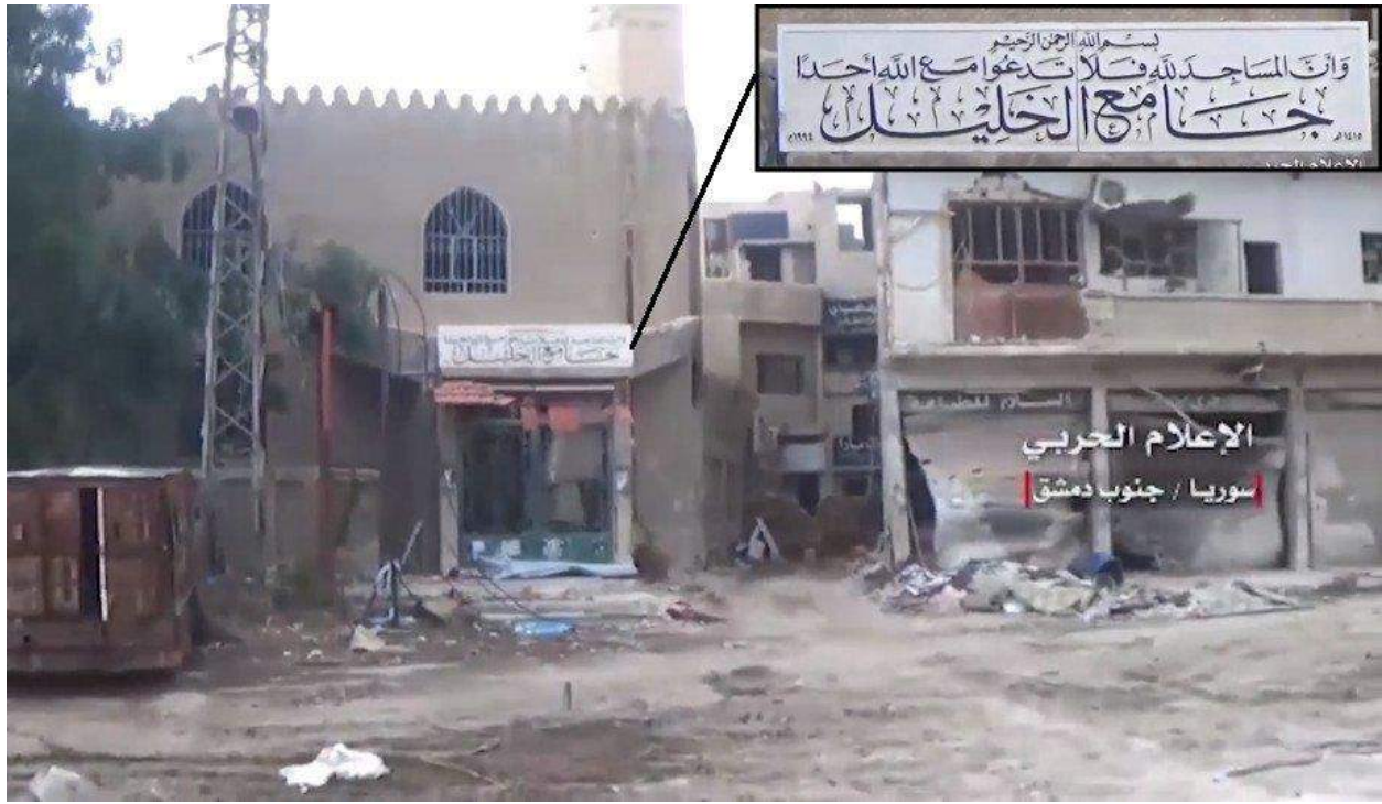
A photograph of damage to the area around Ibrahim al-Khalil Mosque (Private Twitter Account; May 5, 2018)
