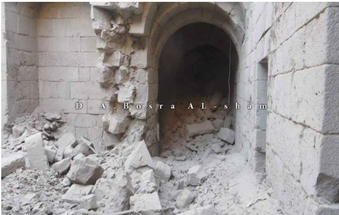
West courtyard after the airstrikes.
