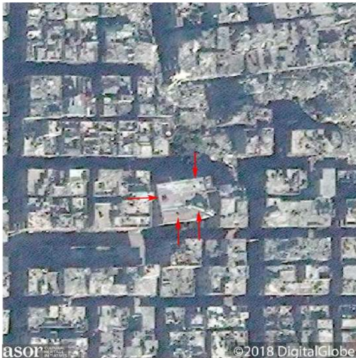
At least three holes in the roof of al-Habib al-Mustafa Mosque are indicated by red arrows, as well as the collapse of the minaret onto the southeastern part of the roof (DigitalGlobe NextView License; December 23, 2014)
