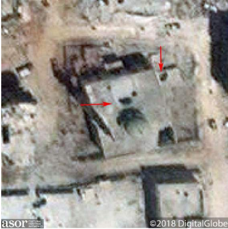
A much larger hole from shelling immediately north of the dome of al-Zubair Mosque and a large hole in the roof of the northeast entrance hall (DigitalGlobe NextView License; May 21, 2018)
