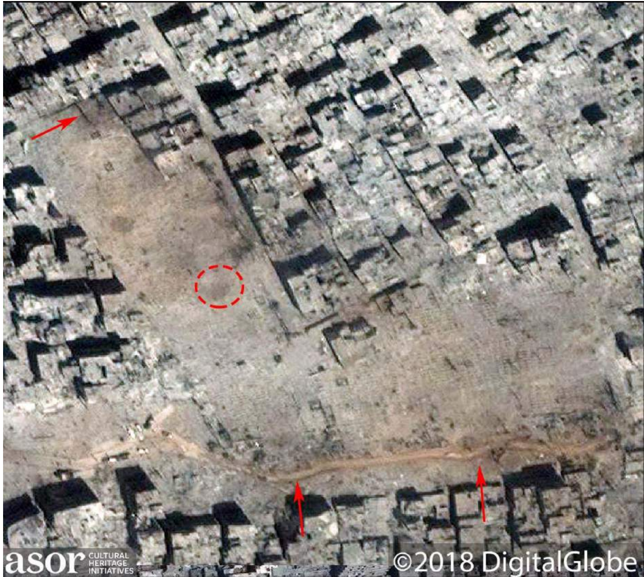
Extreme damage to the Palestinian Martyrs Cemetery as a result of military activity. An airstrike crater is indicated by a red circle. The southern half of the cemetery was almost entirely obliterated and a road was constructed along the boundary. There is a possible trench in the northern part of the cemetery (DigitalGlobe NextView License; May 21, 2018)
