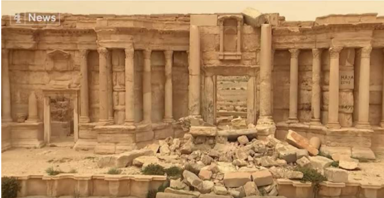
Video still of damage to stage of the Theater, as well as graffiti on the stage background (Channel 4 News; May 28, 2018)
