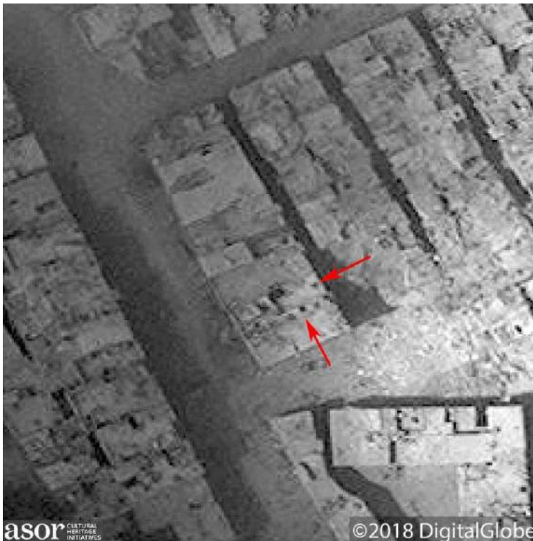
At least three holes are visible in the roof of al-Rahman Mosque, as indicated by red arrows (DigitalGlobe NextView License; May 11, 2018)
