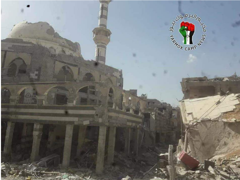
Damage to the Palestinian Mosque and the surrounding area, including the collapse of the dome (Private Twitter Account; May 11, 2018)
