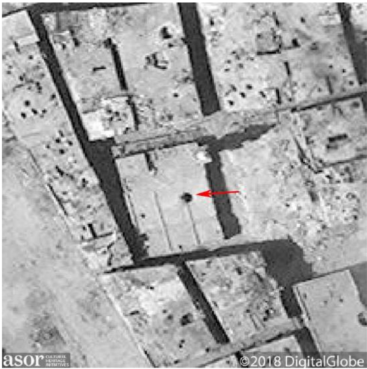
A red arrow indicates the large hole in the unnamed mosque's roof, and the building to the east has been reduced to rubble (DigitalGlobe NextView License; May 11, 2018)
