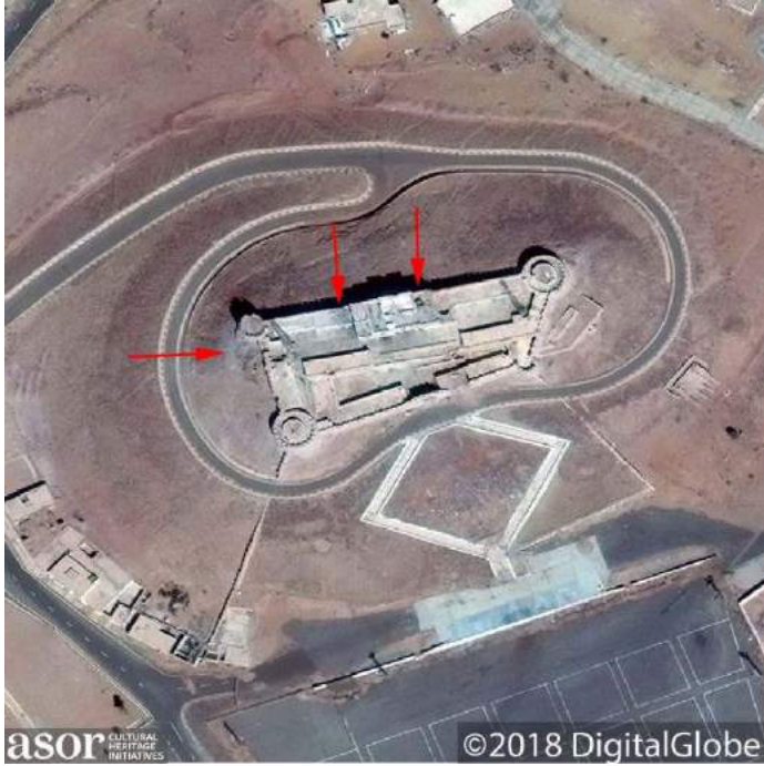
Previously reported damage to Sabha Castle indicated by red arrows (DigitalGlobe NextView License; March 25, 2018)
