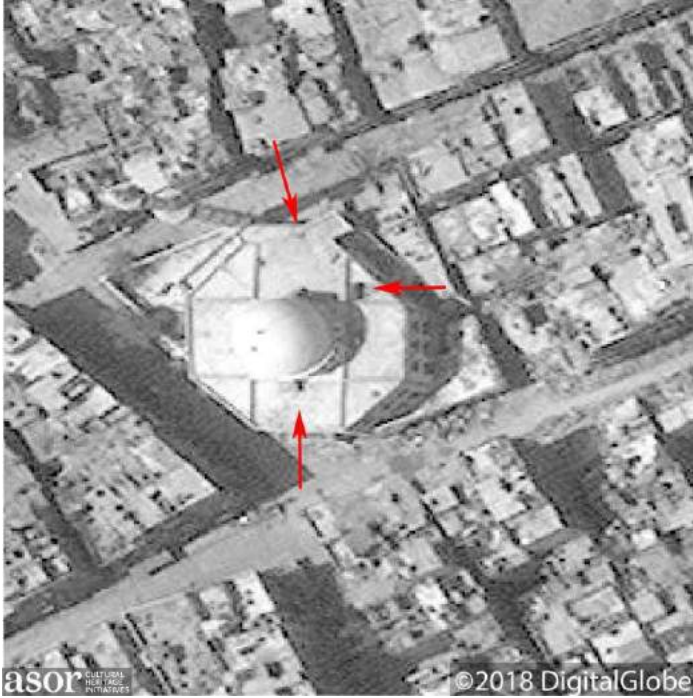
Previously reported damage to the Palestinian Mosque indicated by red arrows (DigitalGlobe NextView License; May 3, 2018)
