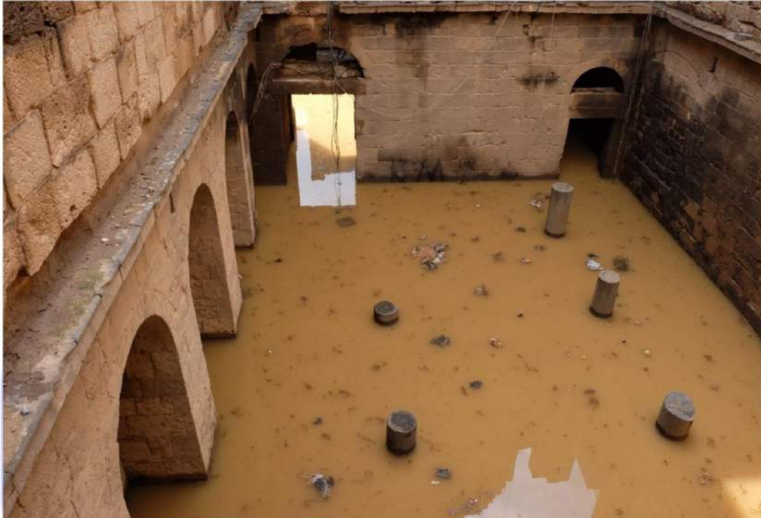
The east courtyard is under 1.5m of water.
