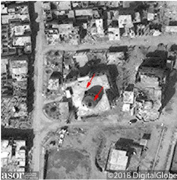
Increased damage to the mosque from heavy shelling. There are at least two large holes in the roof, one in the dome and one just north of the dome, indicated by red arrows (DigitalGlobe NextView License; March 4, 2018)
