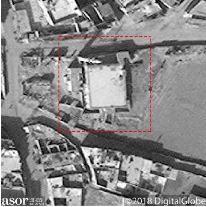
Al-Khanshur Mosque prior to visible damage (DigitalGlobe NextView License; February 6, 2018)
