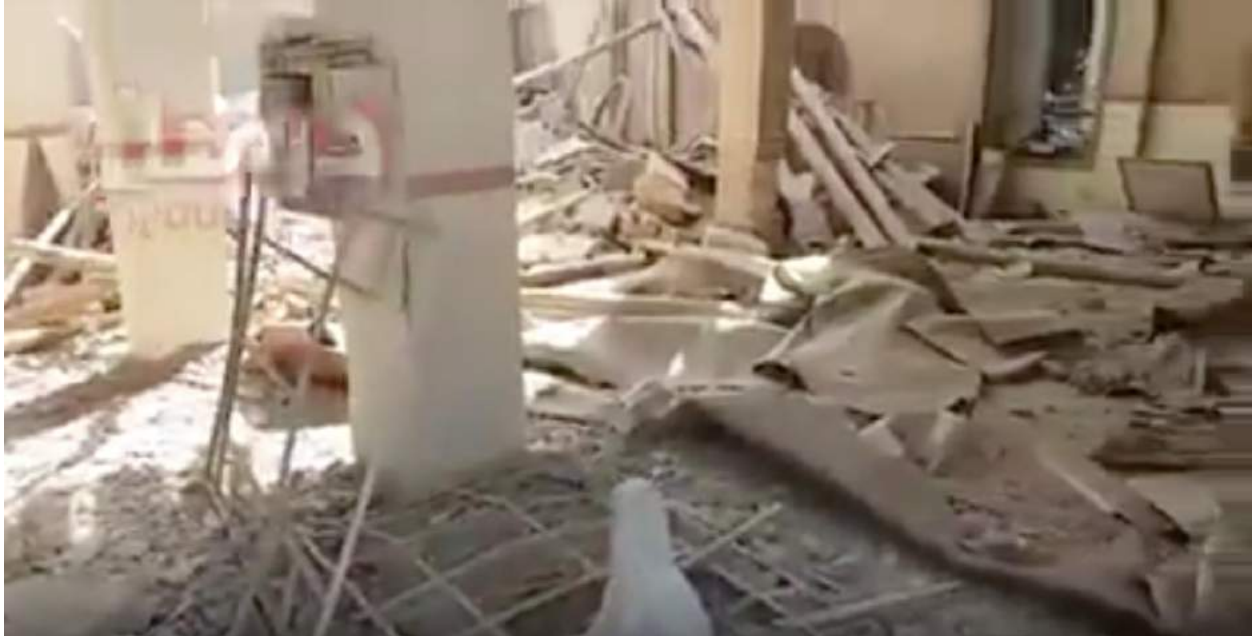
A video still shows severe damage to the interior of al-Sleiq Mosque (SNHR; March 12, 2018)
