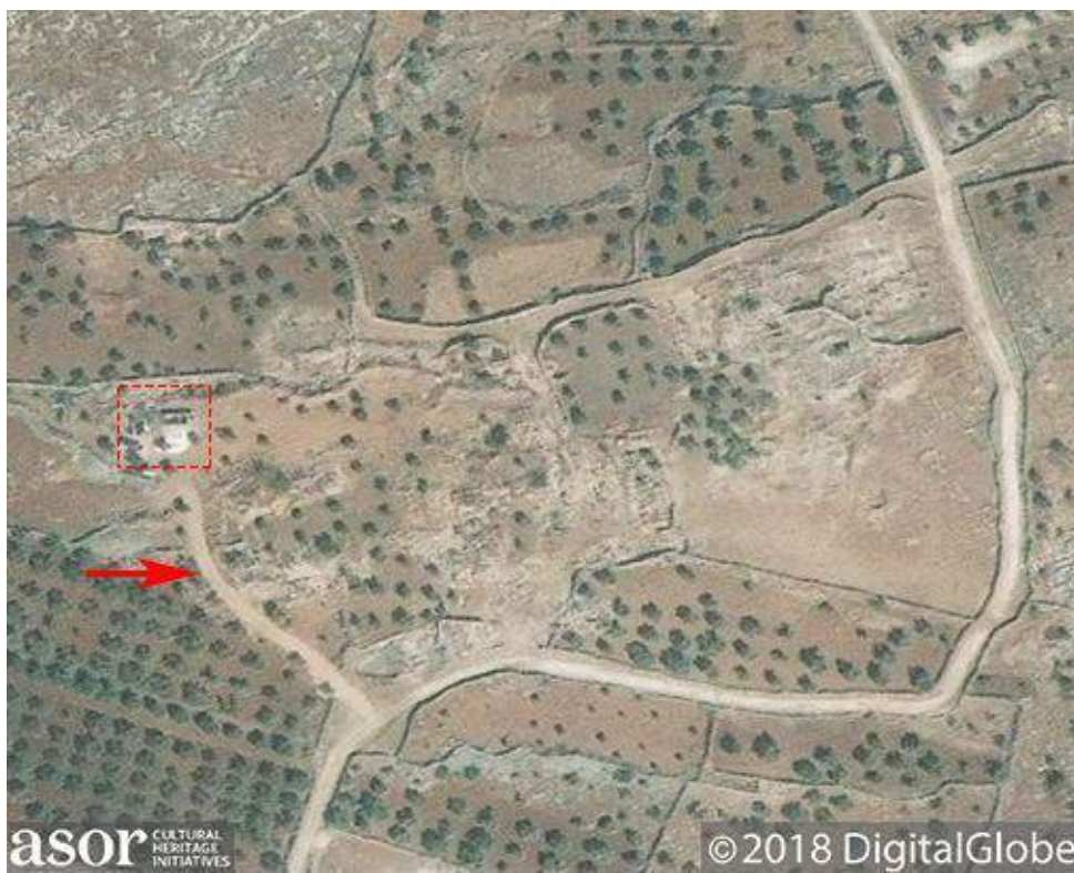
New building and road construction along eastern side of Batuta remains (DigitalGlobe NextView License; September 26, 2017)
