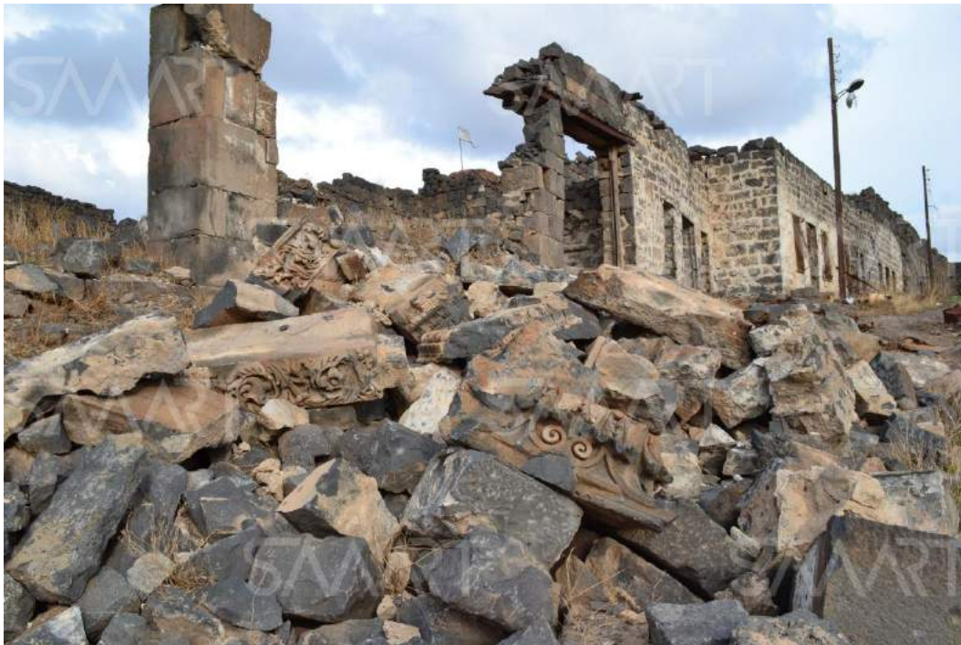
Collapsed section of the nymphaeum (SMART News Agency; February 11, 2018)
