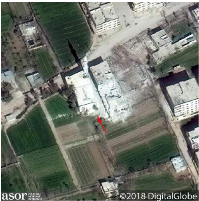
A red arrow indicates damage to the southern facade of al-Radha Mosque. There is also significant damage to the adjacent buildings (DigitalGlobe NextView License; March 1, 2018)
