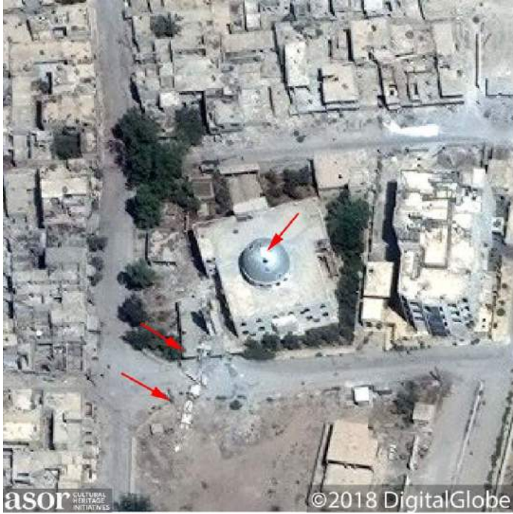
The minaret has collapsed southward, as indicated by two red arrows, and there are at least two holes in the dome of the mosque from heavy shelling (DigitalGlobe NextView License; August 18, 2015)
