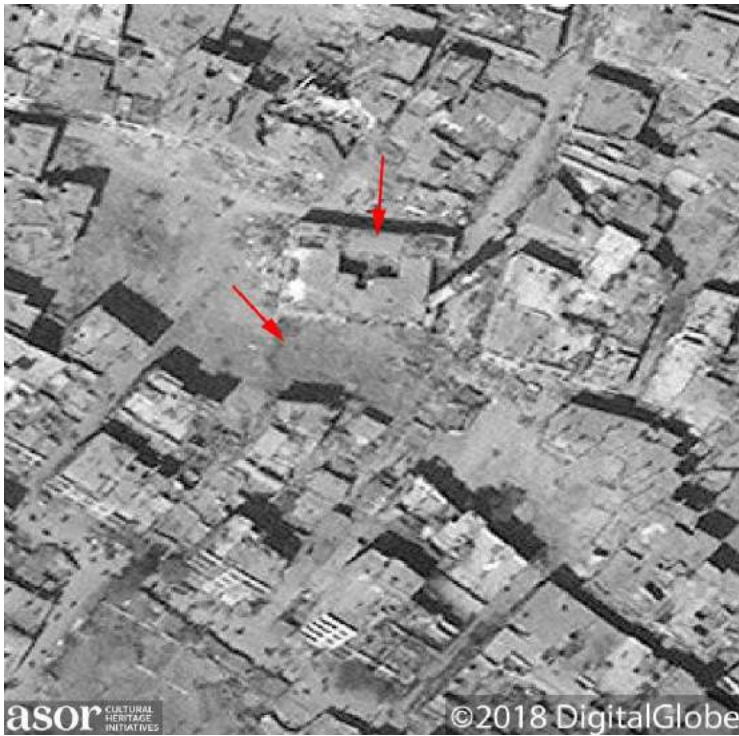
Rubble from the southern part of al-Kabir Mosque that previously collapsed has been cleared away and the central part of the remaining roof collapsed (DigitalGlobe NextView License; March 25, 2018)
