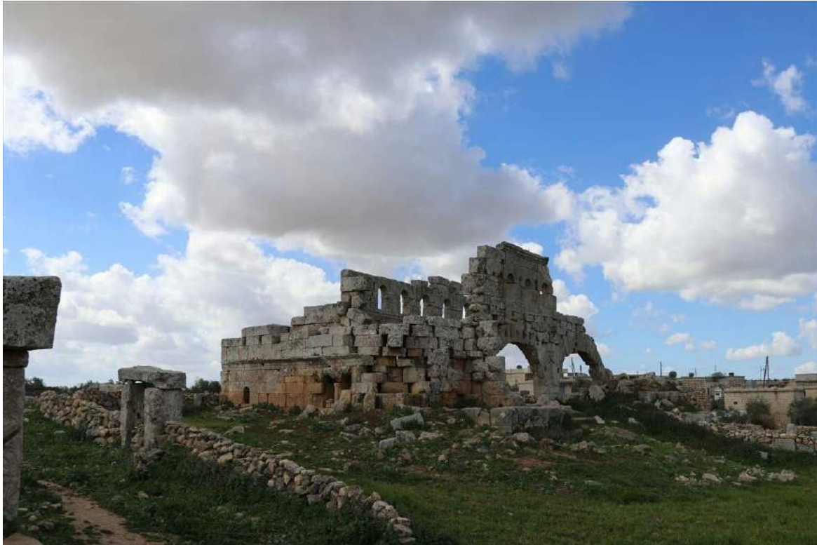
The North Church, seen from the northeast (ASOR CHI Source; March 30, 2018)
