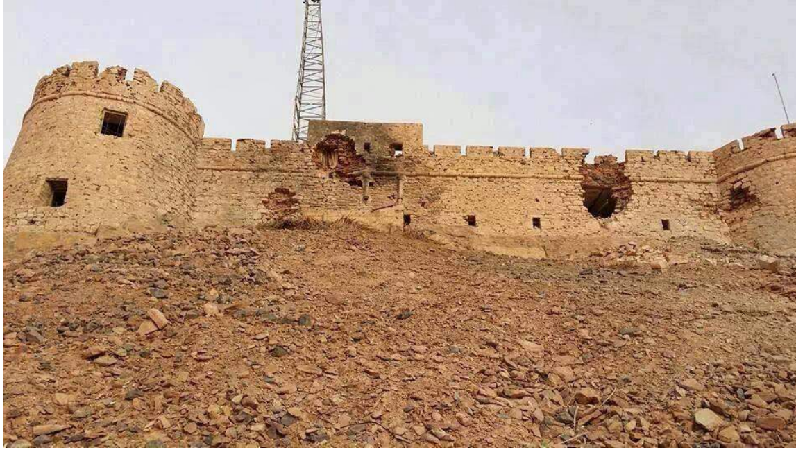
Damage to the western wall of Sabha Castle (Libya Observer; March 5, 2018)
