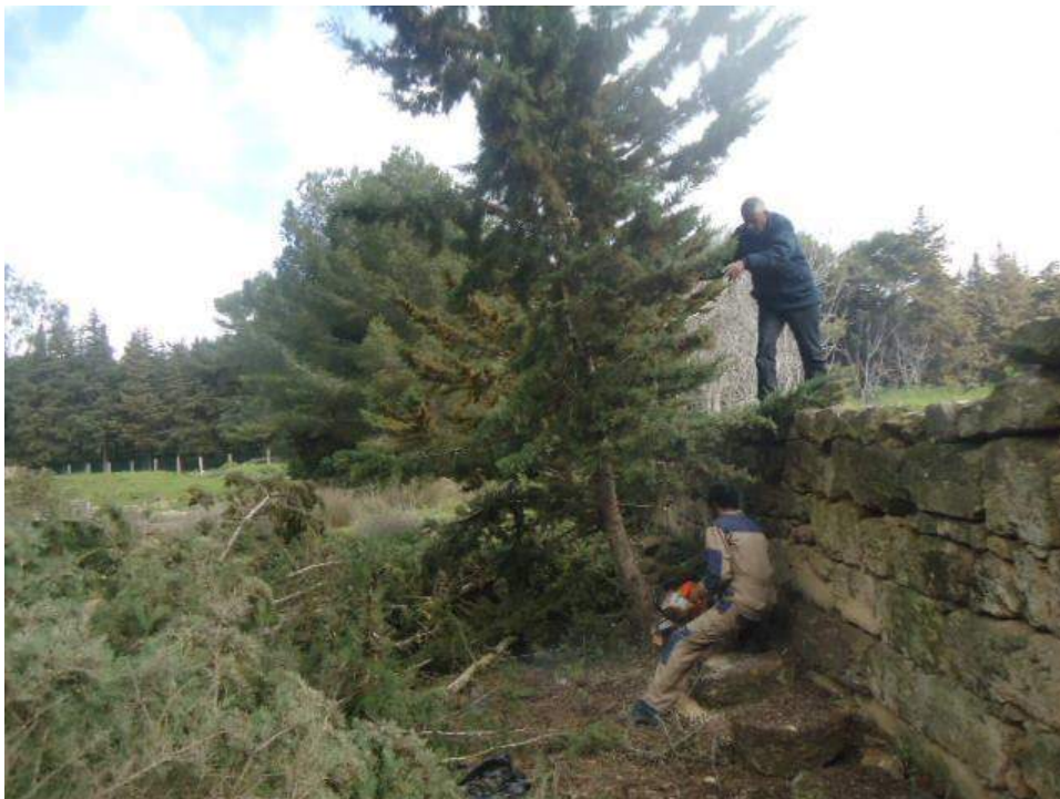
Members of DoA Shahat's conservation team remove another tree undermining the precinct wall (DoA Shahat; March 15, 2018)
