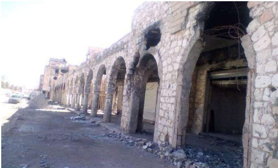
Another view of damaged arcade and storefronts (Private Facebook Account; March 28, 2018)
