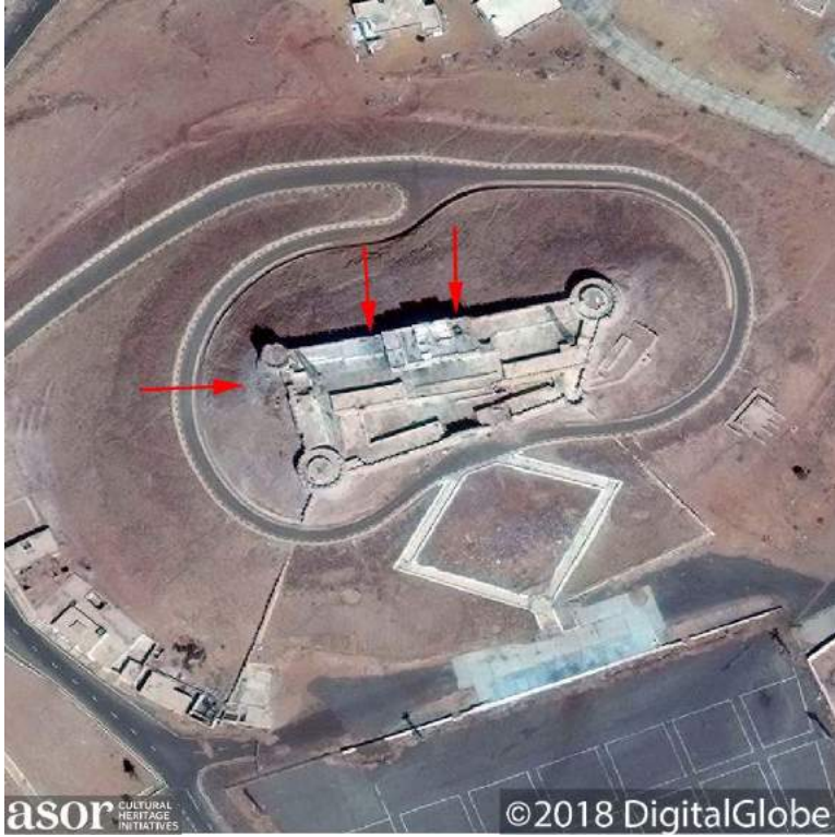
Damage to the northern wall of Sabha Castle, with a red arrow indicating a hole in the western wall. Additionally, rubble can be seen on the northwest corner of castle (DigitalGlobe NextView License; March 25, 2018)
