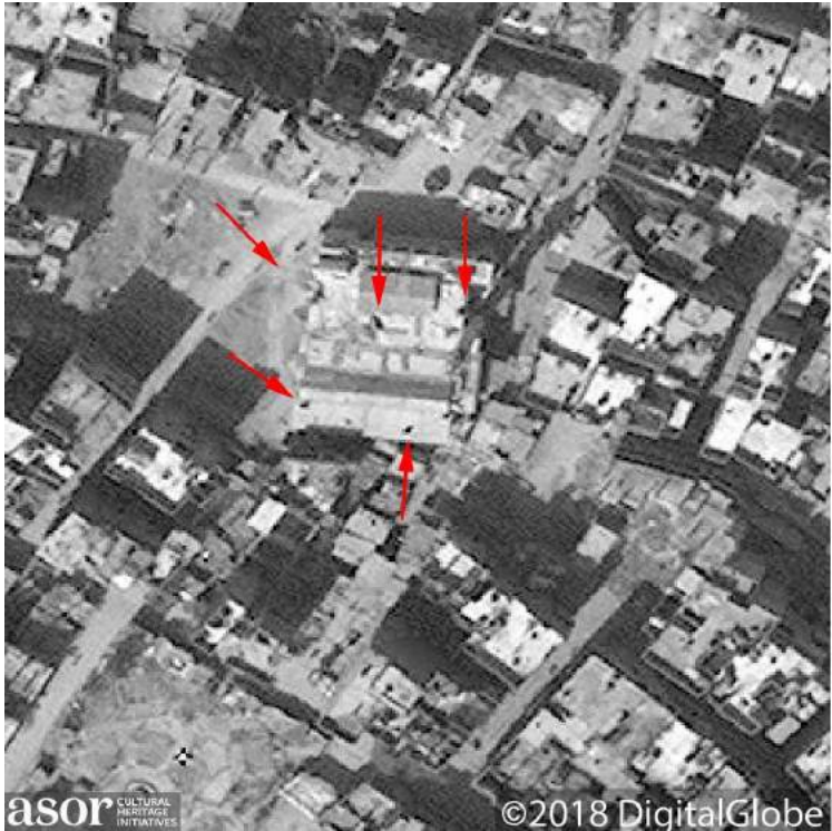
Al-Kabir mosque with previously occurring damage from heavy shelling indicated by red arrows (DigitalGlobe NextView License; March 4, 2018)
