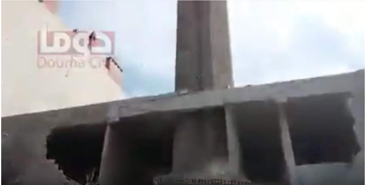
A video still shows severe damage to the exterior of al-Sleiq Mosque (SNHR; March 12, 2018)
