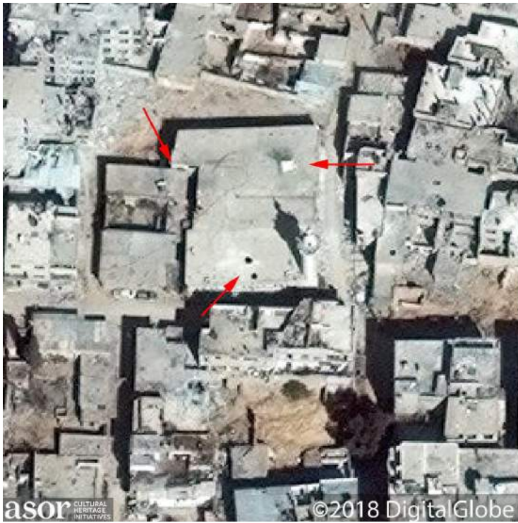
Two holes and scorch marks on the roof of al-Kabir Mosque are indicated by red arrows (DigitalGlobe NextView License; March 1, 2018)
