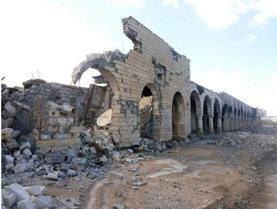
Given the extent of the damage, much stabilization and repair work remains to be done (Private Facebook Account; March 28, 2018)
