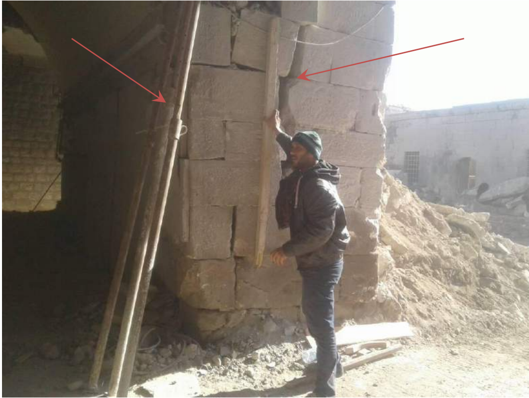
Workers stabilize damaged areas using wooden beams and scaffolding (TDA-HPI; January 6, 2018)
