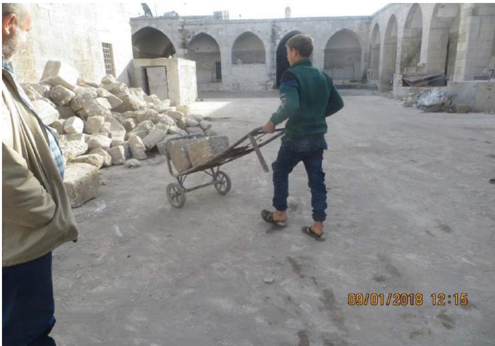
Workers sort collapsed stones.
