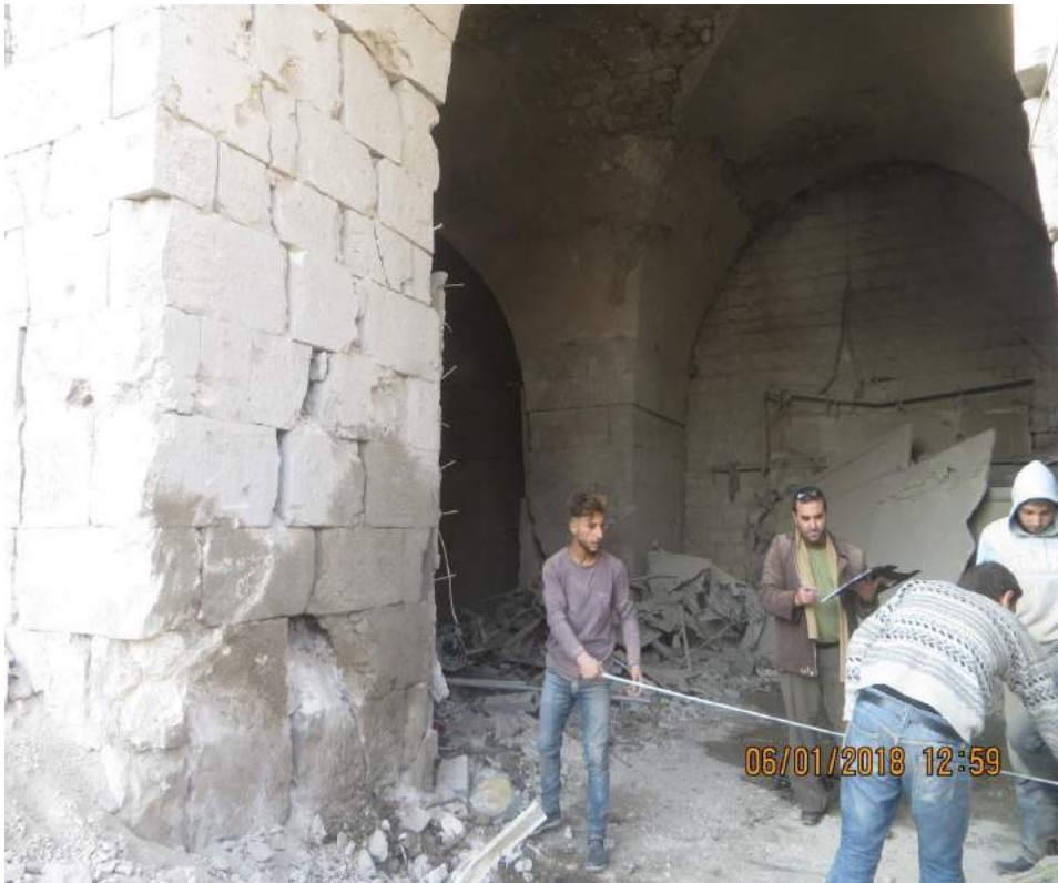
Workers dig through the rubble and collect fallen masonry (TDA-HPI; January 6, 2018)
