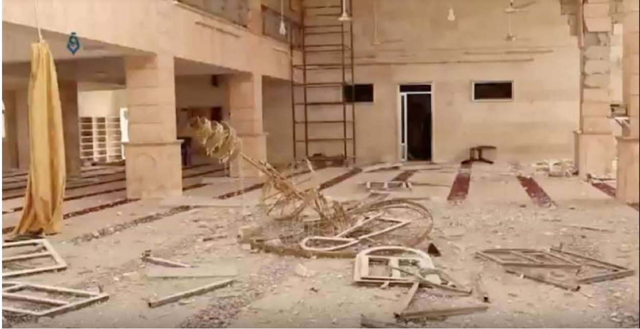
Video still of debris in the interior of al-Kabir Mosque, including a destroyed chandelier (Halab Today TV; January 4, 2018)
