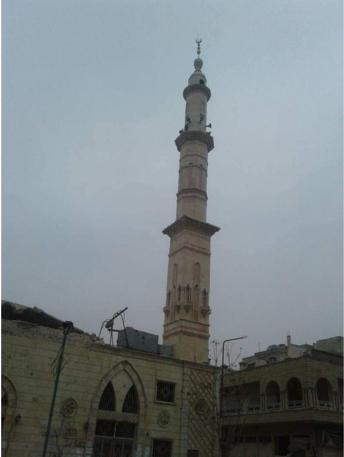
The condition of the exterior of Uwais al-Qarni Mosque (ASOR CHI Source; January 4, 2018)
