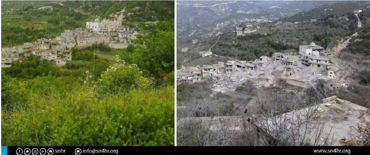
Before and after photographs of al-Tefahiya, with damaged mosque seen in top right (SNHR; January 6, 2018)
