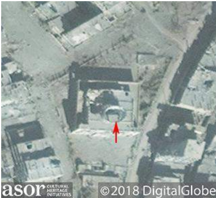
Severe damage to the dome of Othman Bin Affan Mosque (DigitalGlobe NextView License; December 1, 2017)
