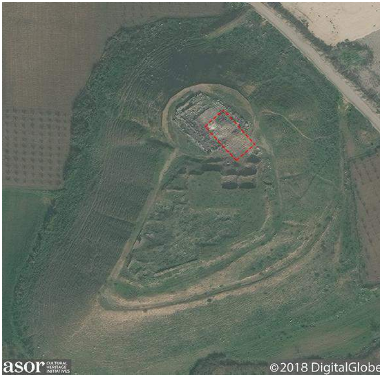
Damage from attack on Tell Ain Dara temple, with debris field indicated by the red box (DigitalGlobe NextView License; January 29, 2018)
