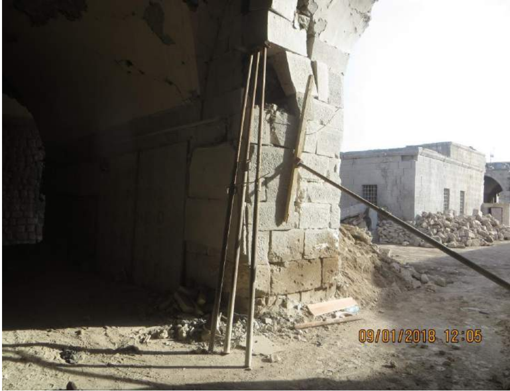
Workers stabilized damaged areas using wooden beams and scaffolding (TDA-HPI; January 9, 2018)
