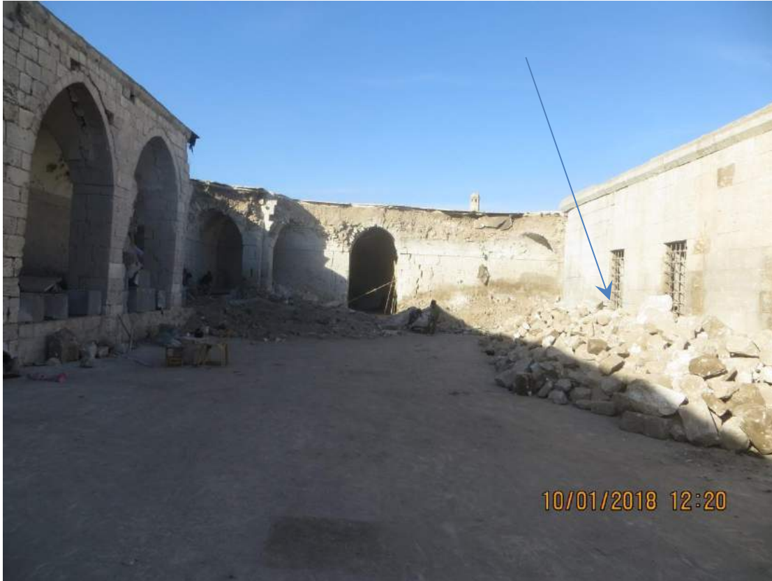
Workers gathered masonry from the north and west façades (TDA-HPI; January 10, 2018)
