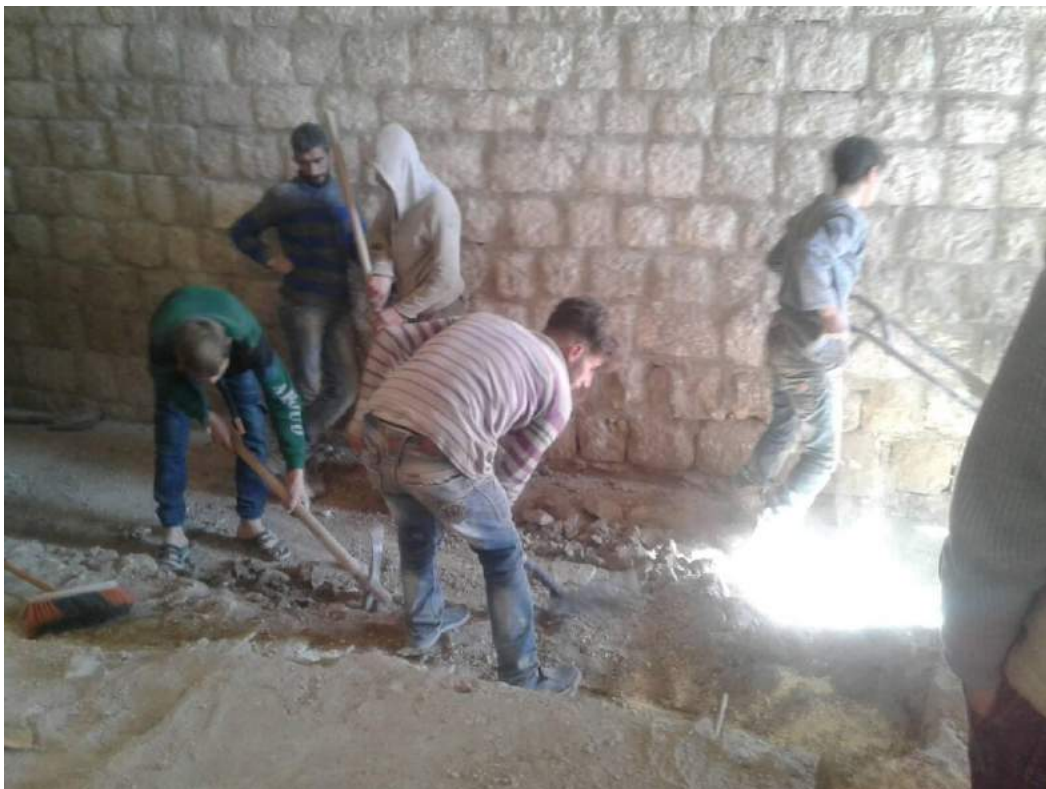
Workers clear out rubble (TDA-HPI; January 6, 2018)
