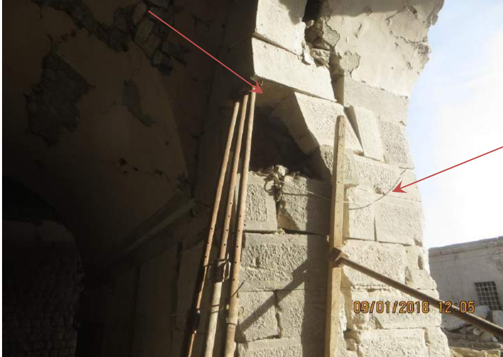
Workers stabilized damaged areas using wooden beams and scaffolding (TDA-HPI; January 9, 2018)
