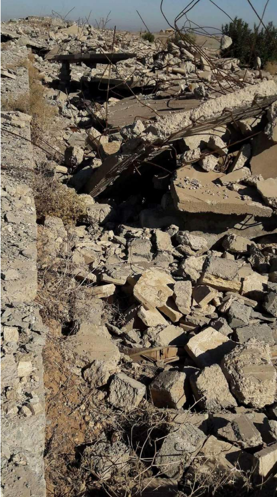
Damage to burials at Wadi 'Ikab Cemetery (This is Christian Iraq/Facebook; January 16, 2018)
