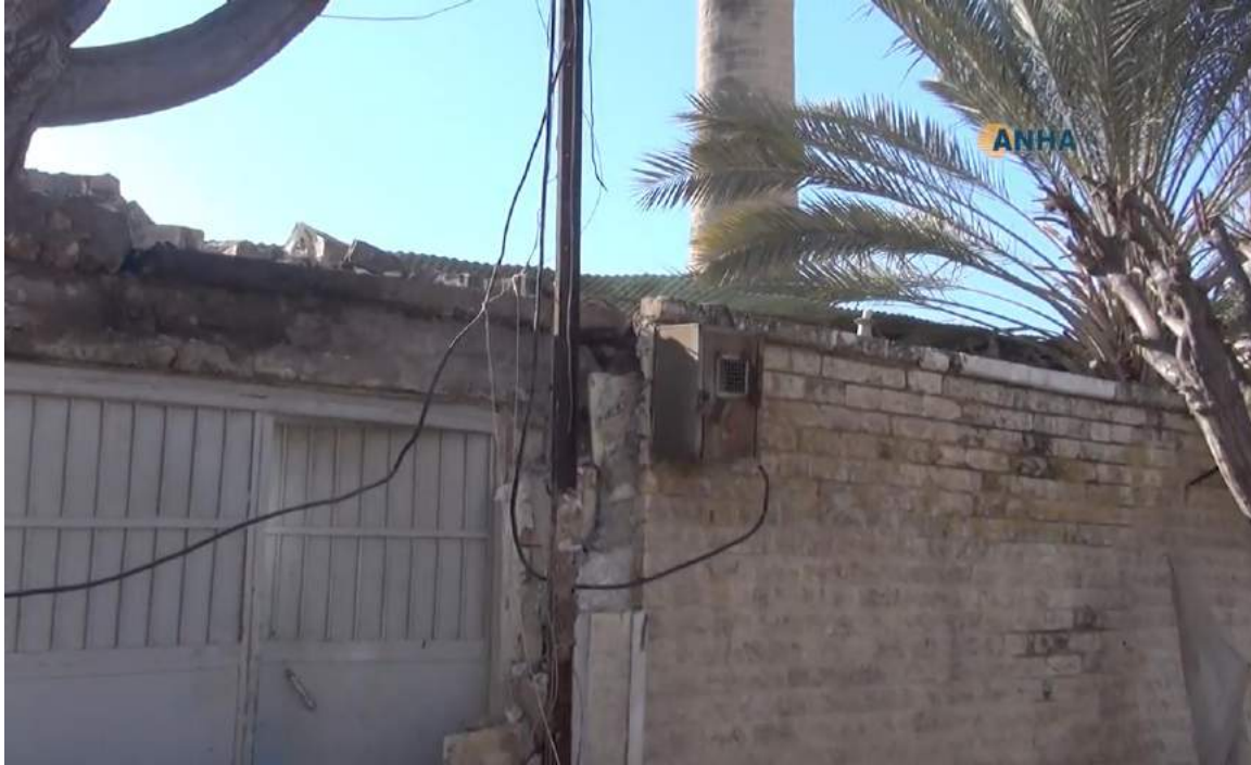
Video still of the exterior of Salah al-Din al-Ayoubi Mosque (ANHA; January 29, 2018)
