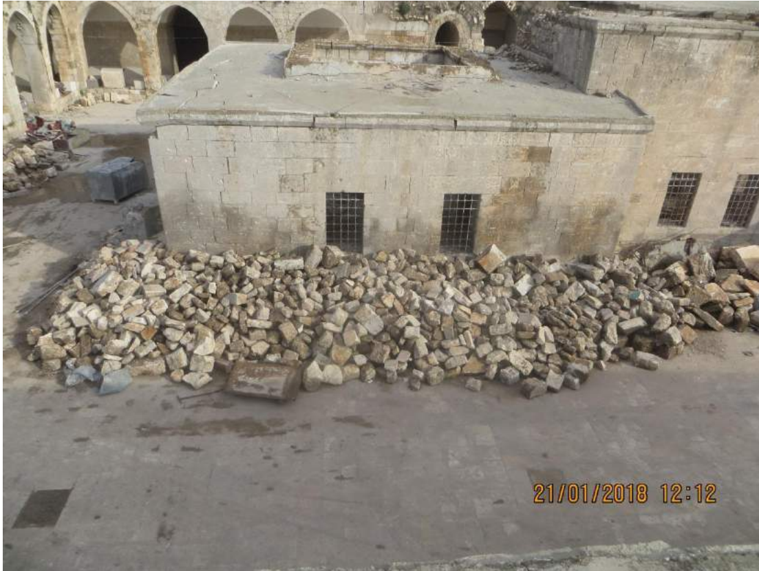
Workers completed the process of sorting collapsed masonry (TDA-HPI; January 21, 2018)
