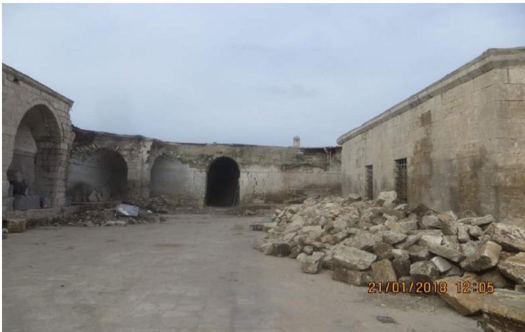
Area after sorting and clearing rubble (TDA-HPI; January 21, 2018)
