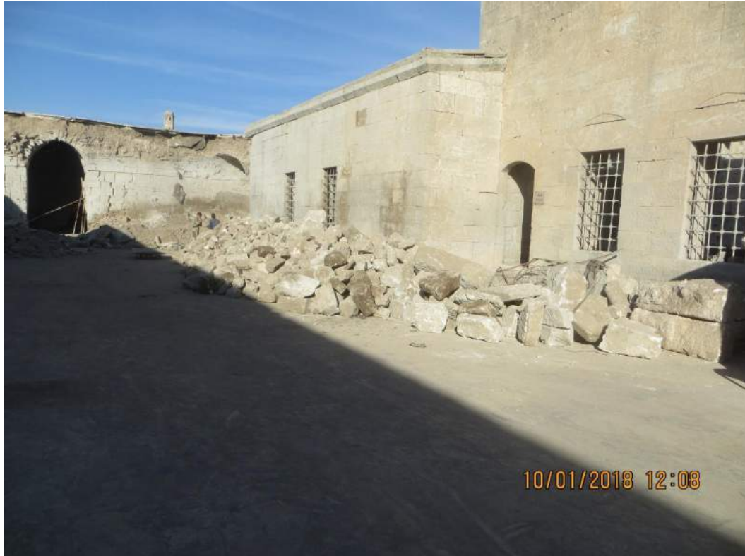
Workers collected pieces of the damaged sarcophagus (TDA-HPI; January 10, 2018)
