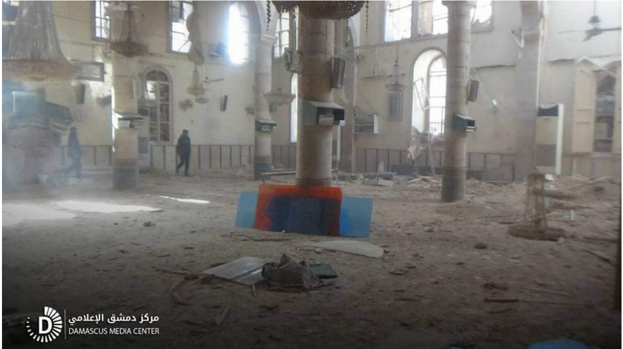
Damage to interior of al-Kabir Mosque (SNHR; January 22, 2018)
