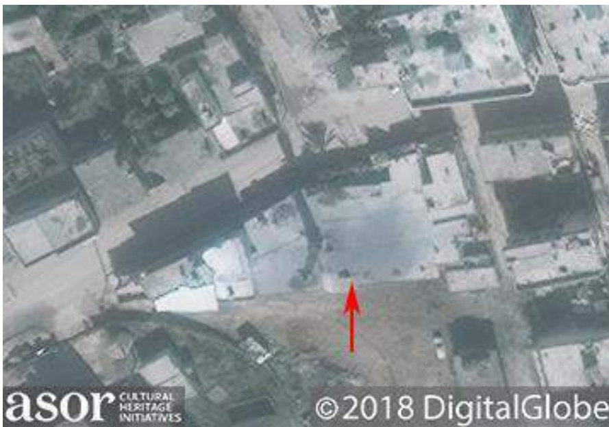
Holes in the roof of Salah al-Din al-Ayoubi Mosque and smoke damage indicated by red arrow (DigitalGlobe NextView License; January 29, 2018)
