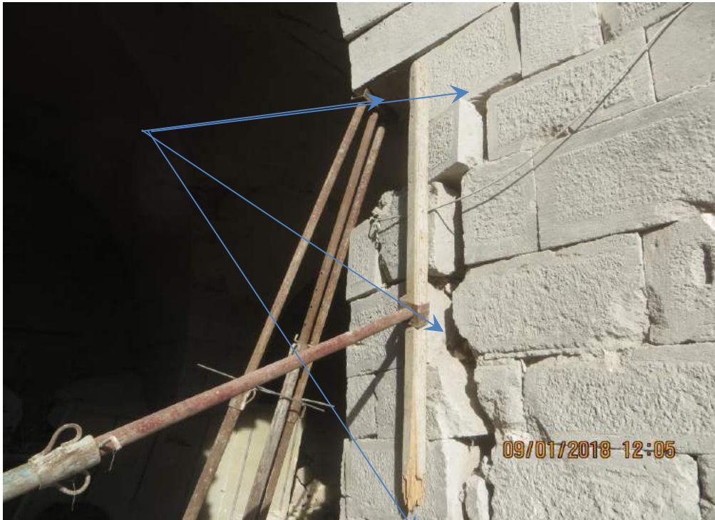
Workers stabilized damaged areas using wooden beams and scaffolding (TDA-HPI; January 9, 2018)
