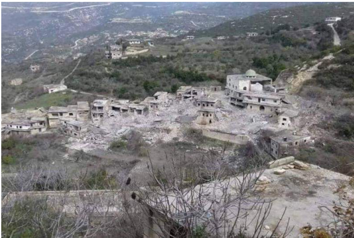
A view of the large-scale destruction of al-Tefahiya and damage to mosque (Shaam Network; January 6, 2018)
