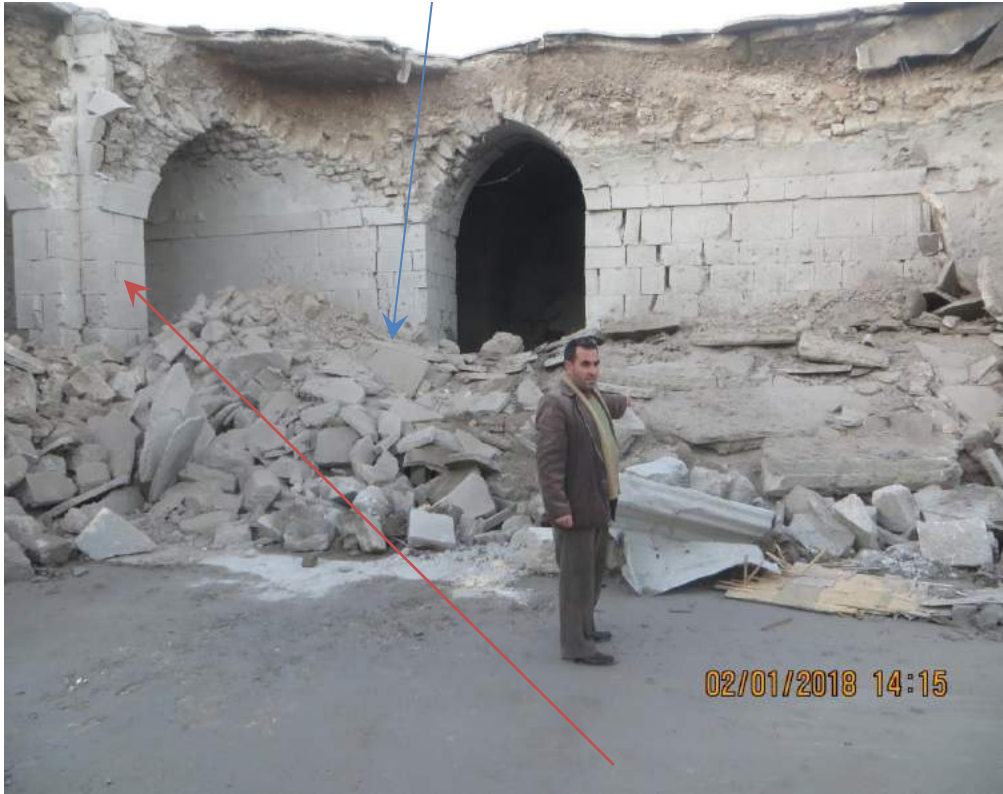
The damaged northwest corner of the museum (TDA-HPI; January 2, 2018)
