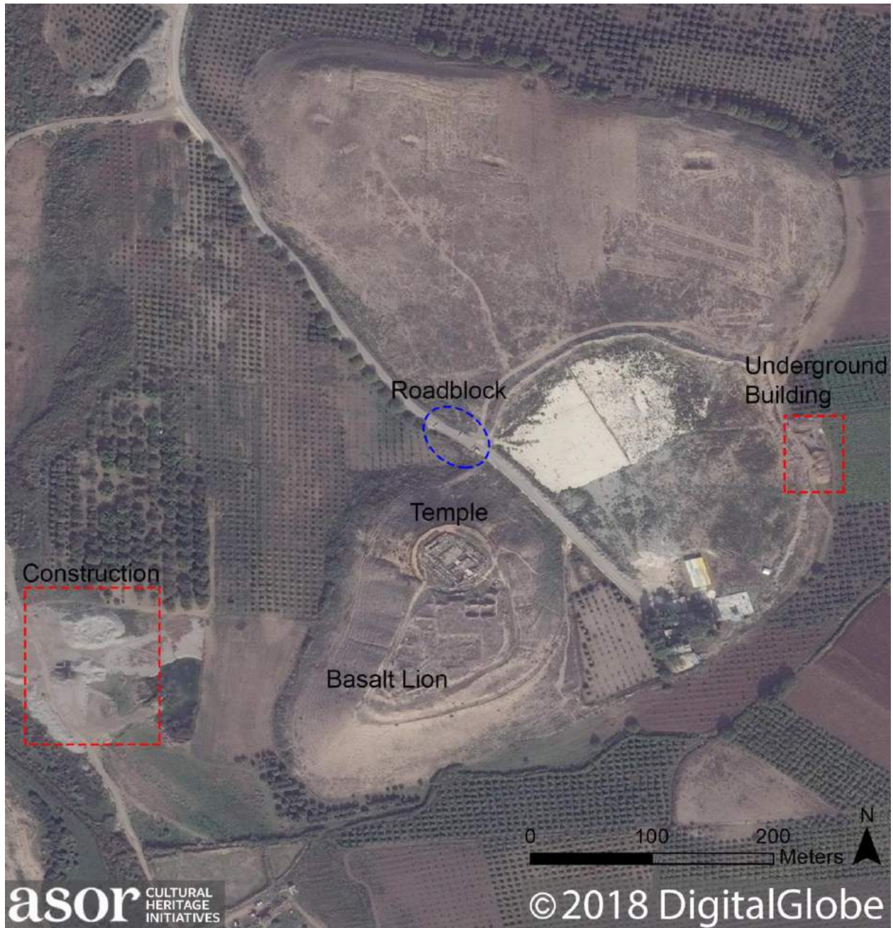
Construction on the eastern side of Tell Ain Dara and a roadblock near the site (DigitalGlobe NextView License; November 9, 2017)
