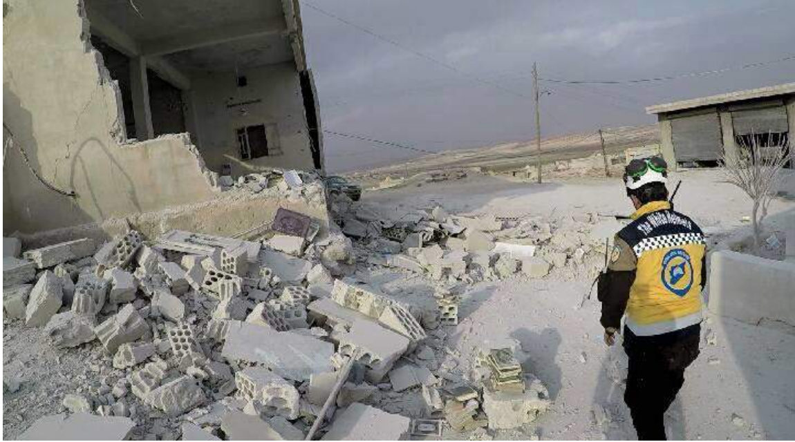
Damage to a mosque in Abu Habbah (SNHR; January 12, 2018)
