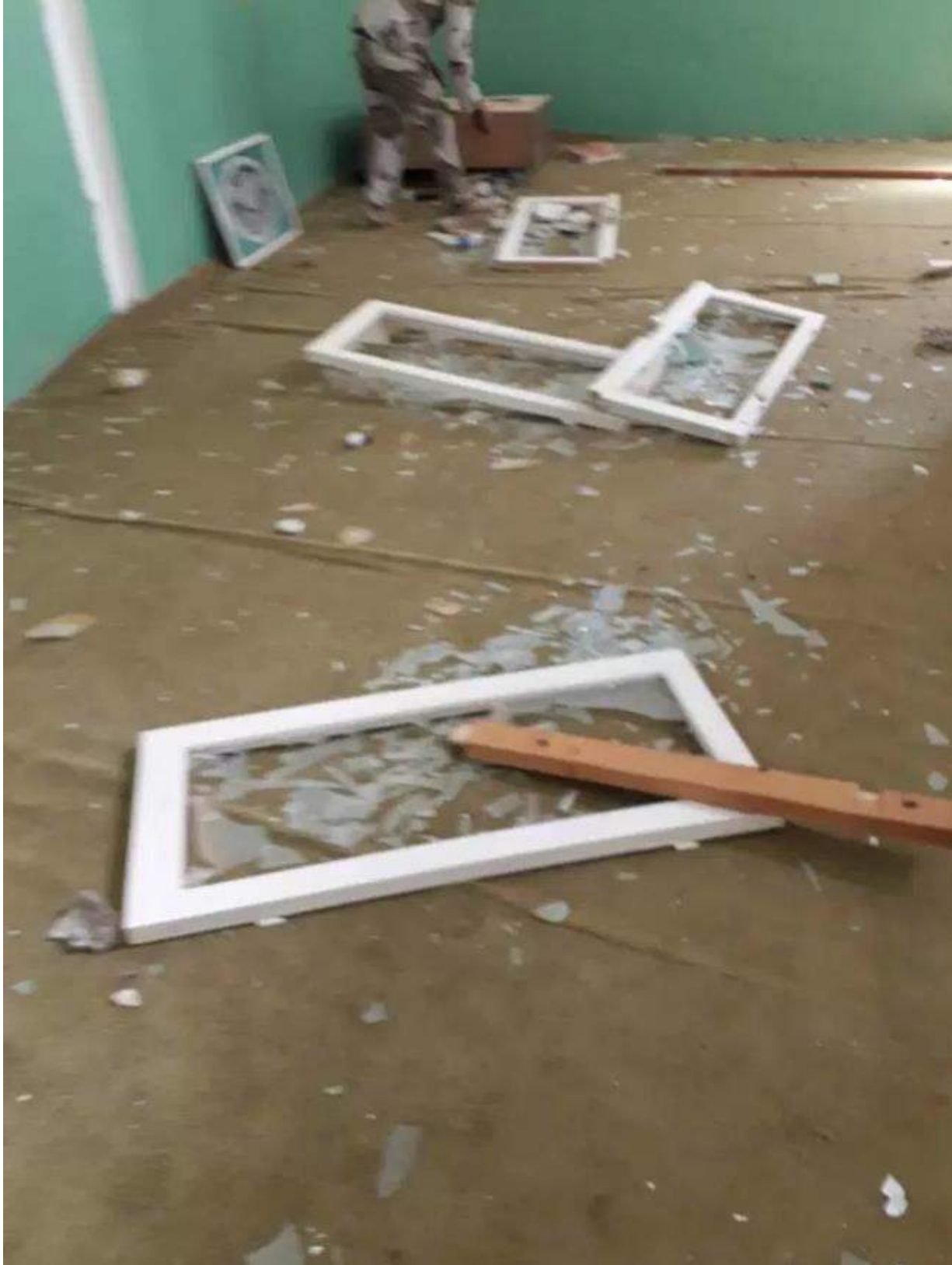
A view of the damage to the interior of the Mausoleum of al-Mahdi (Libyan Cloud News Agency; December 31, 2017)
