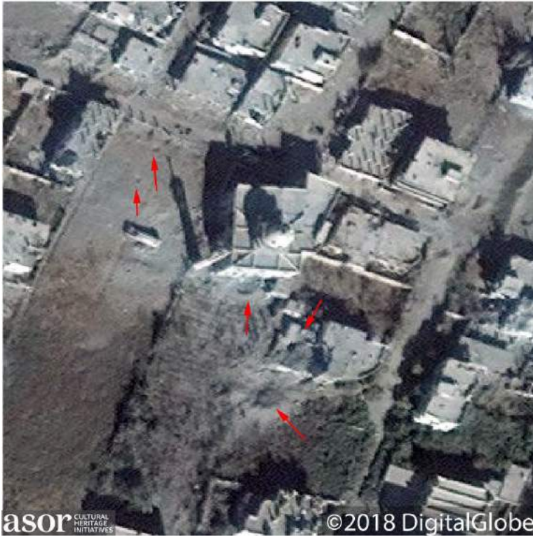
Badour al-Kurdi Mosque with a clear airstrike crater along the southern facade, although the mosque appears to be largely intact. Red arrows indicate areas of severe damage in the surrounding area (DigitalGlobe NextView License; December 2, 2017)
