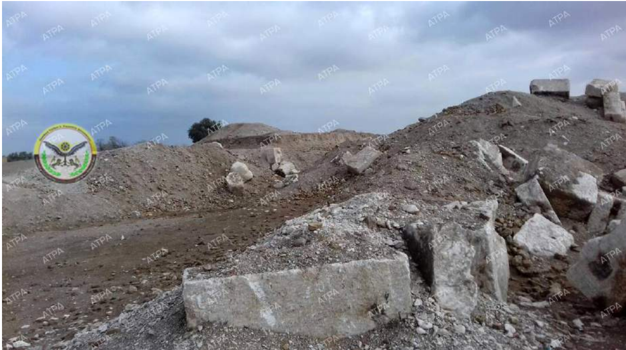
A view of toppled stones and a looting pit at Sura (ATPA; December 31, 2017)
