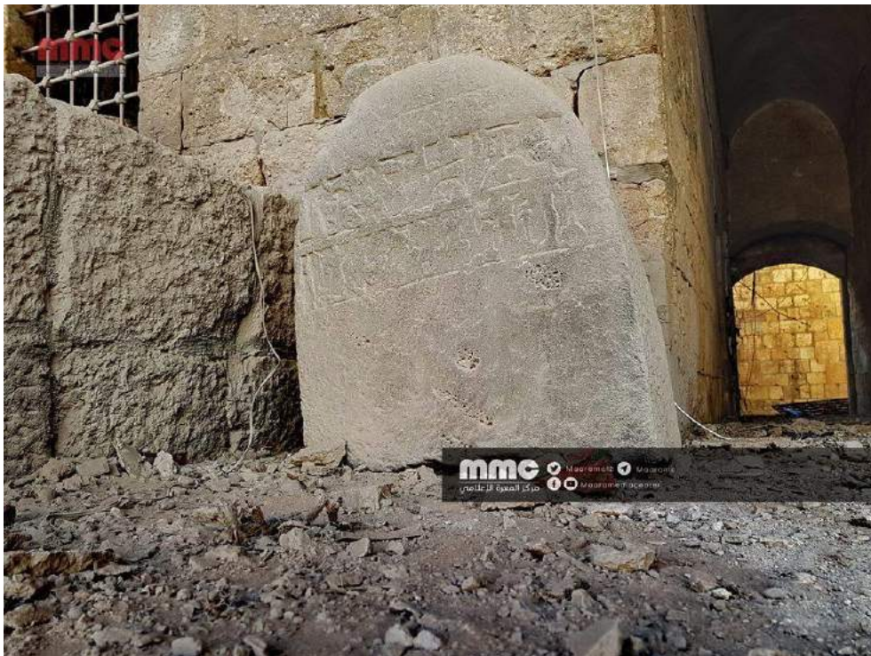
Debris around Luwian stele in western arcade of al-Ma'arra Museum (Maara Media Center/Twitter; January 2, 2018)
