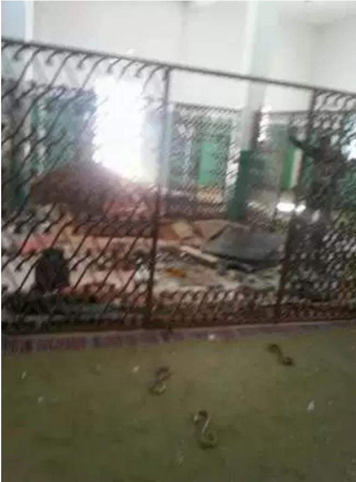
A view of the damage to the interior of the Mausoleum of al-Mahdi (Al Marsad; December 30, 2017)
