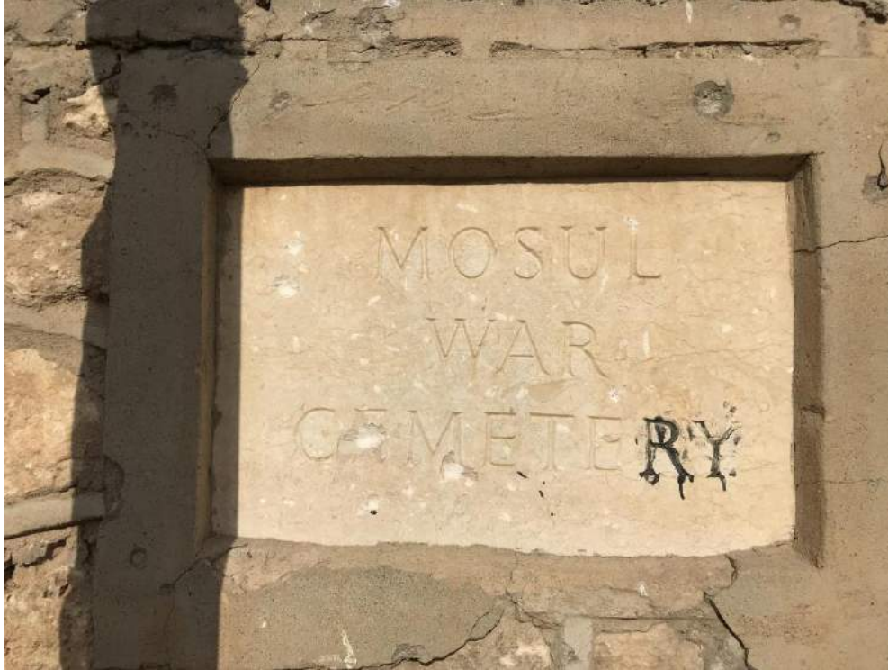
Damage to the Mosul War Cemetery entrance sign (Campbell MacDiarmid; December 22, 2017)
