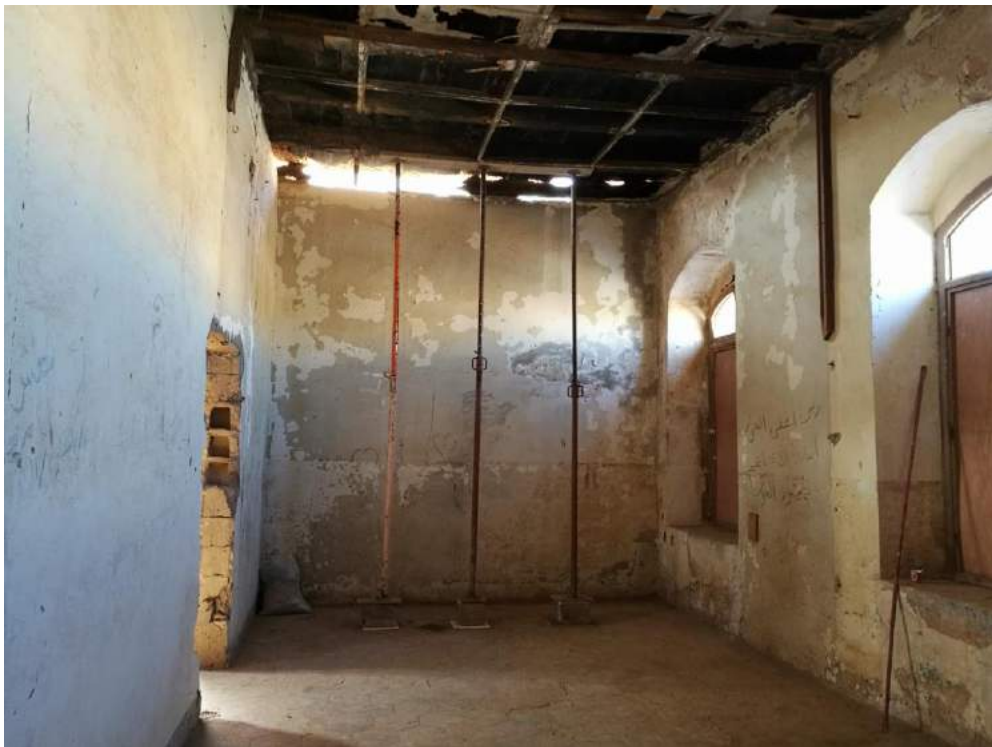
Shoring installed inside Qasr al-Birka (Private Facebook Account)
