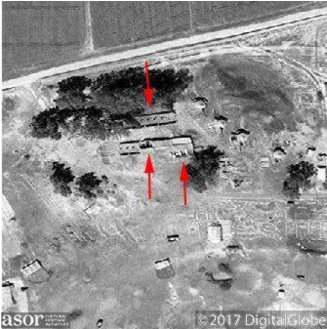
Red arrows indicate parts of the roofs that are missing (DigitalGlobe NextView License; April 16, 2016)
