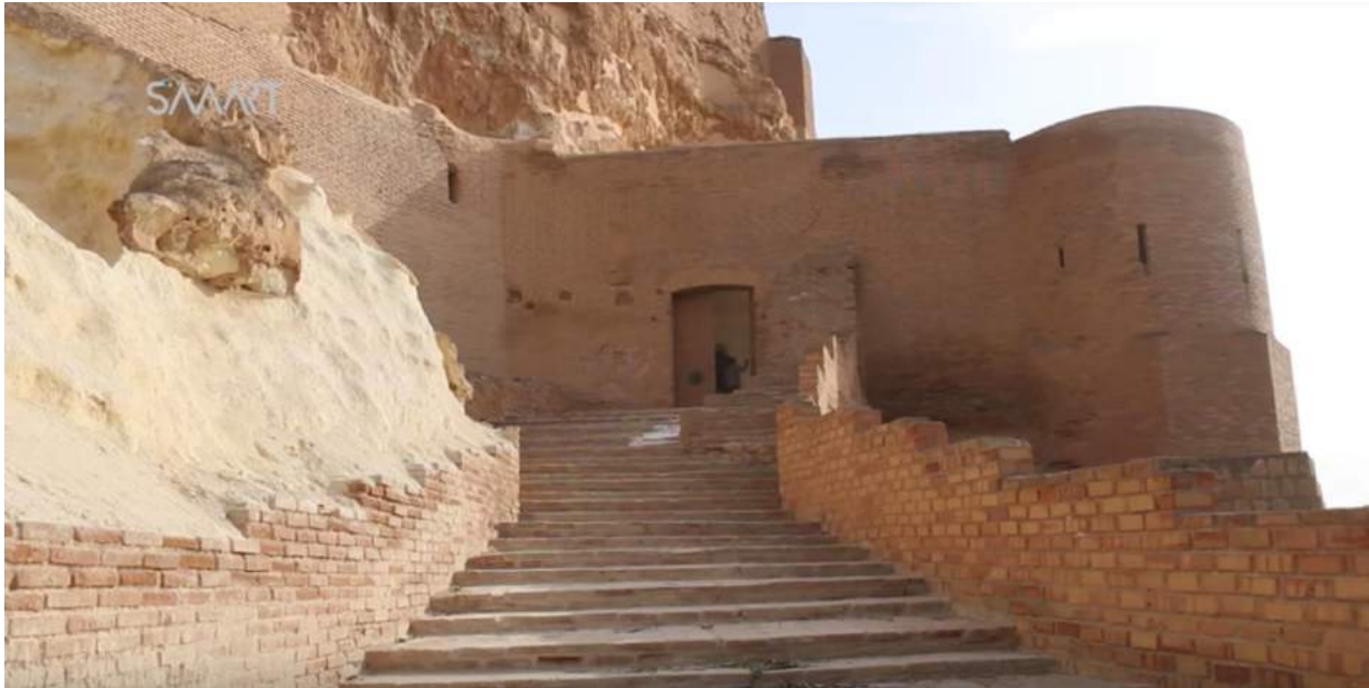
Damage to the entrance has been repaired (SMART News Agency; December 13, 2017)
