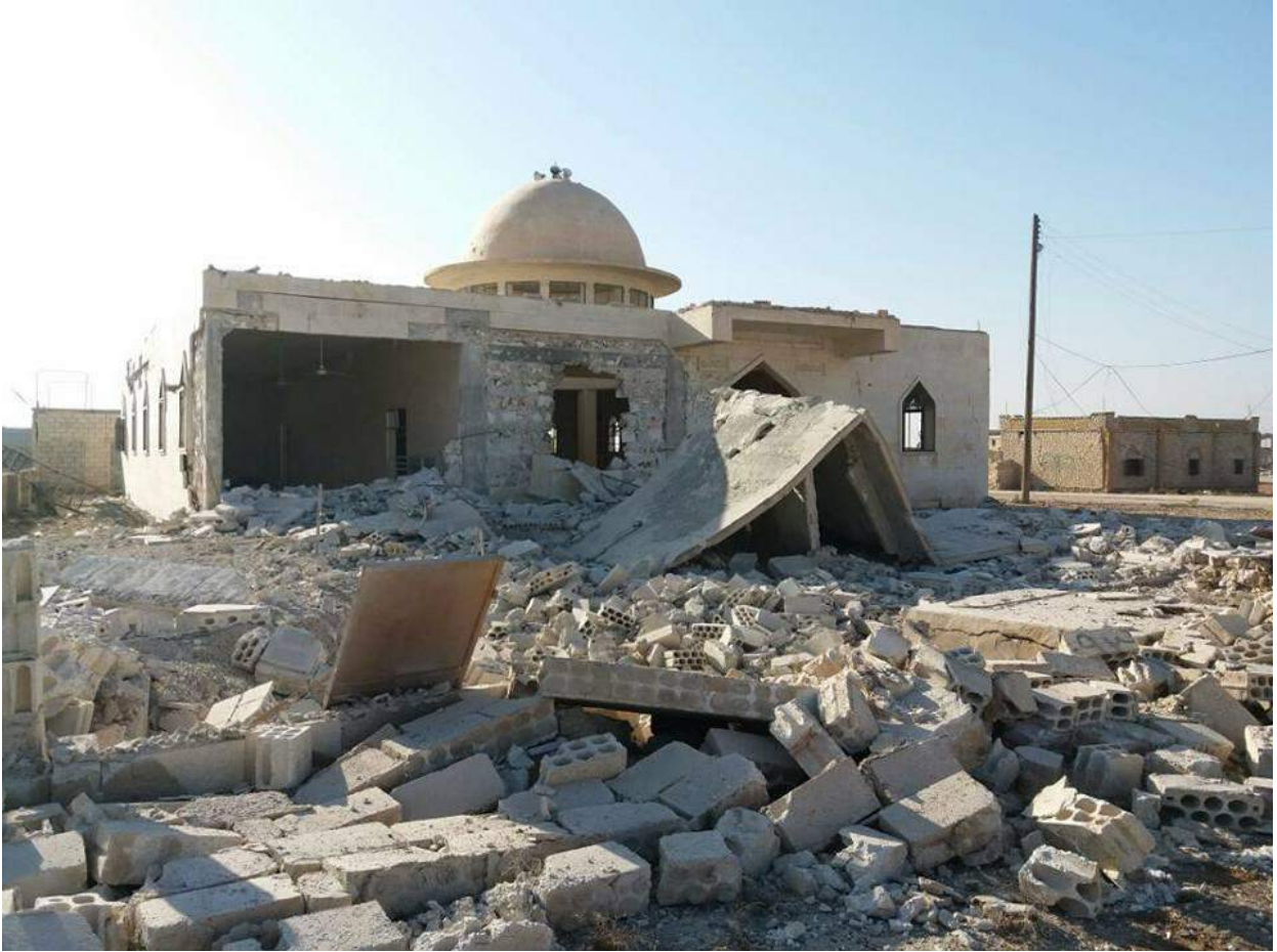
Significant damage to the north side of the mosque (SNHR; December 13, 2017)
