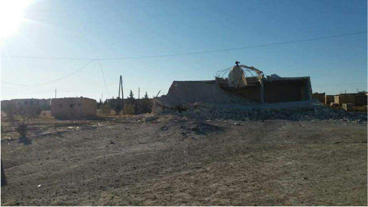
Damage to the Jub Abyad Mosque (SNHR; December 8, 2017)
