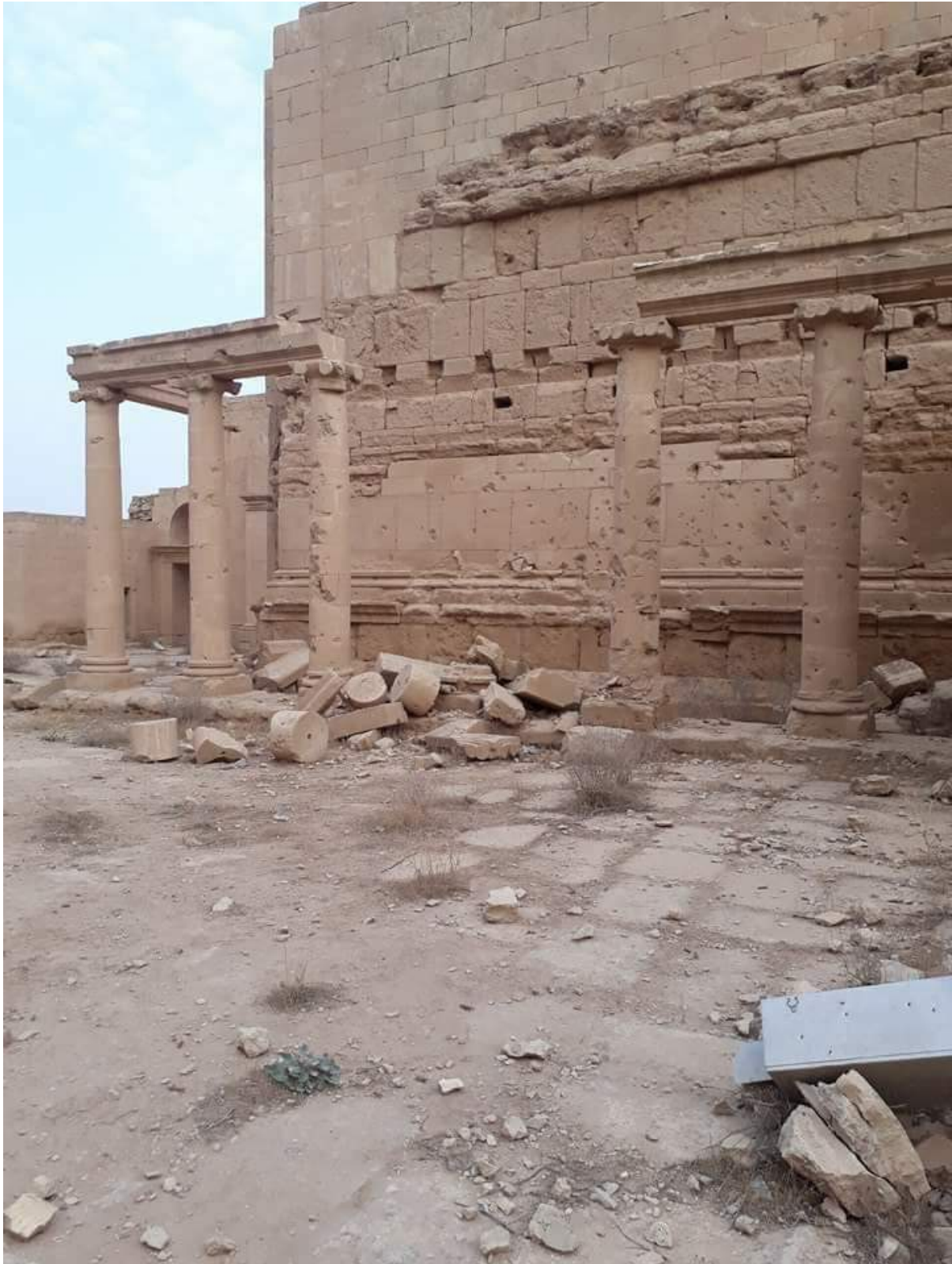
Damage to a building at Hatra showing a destroyed column and gunfire/shrapnel holes in the facade (ASOR CHI Source; December 14, 2017)
