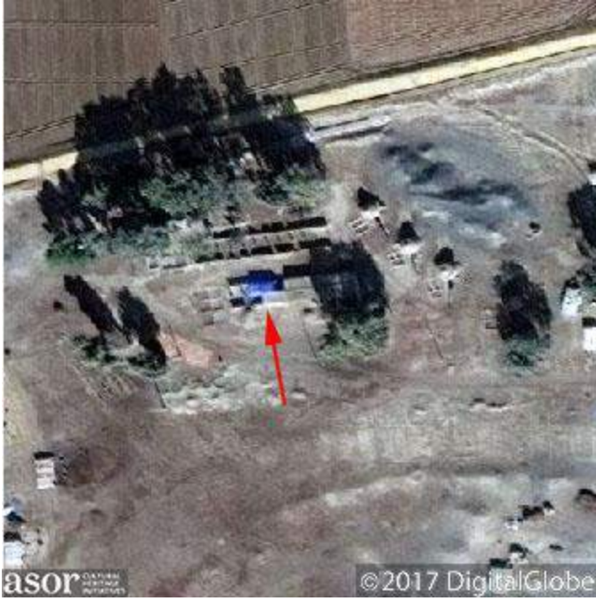
Red arrow indicates a blue covering over part of the southern warehouse. This is the first visible evidence of restoration efforts (DigitalGlobe NextView License; December 26, 2017)
