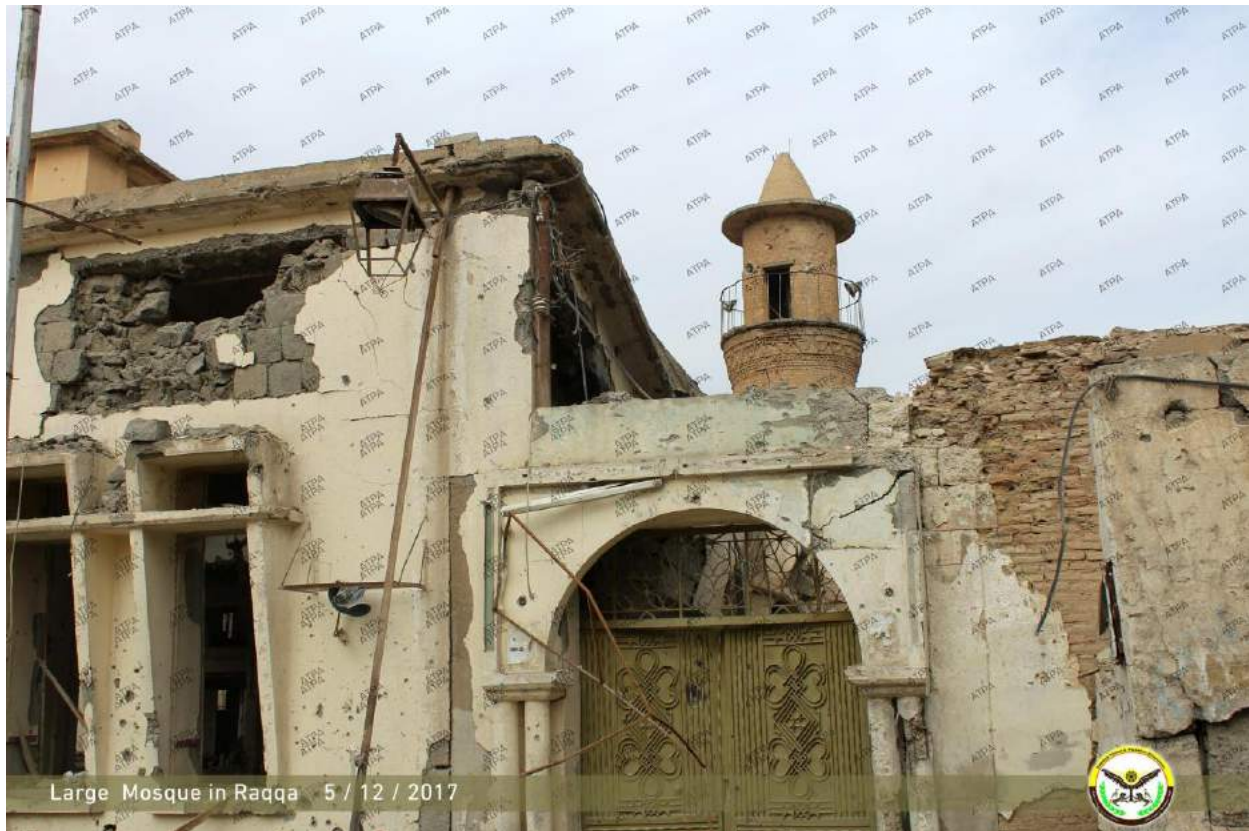
A view of the mosque's facade and smaller minaret, seen from the south (ATPA; December 10, 2017)
