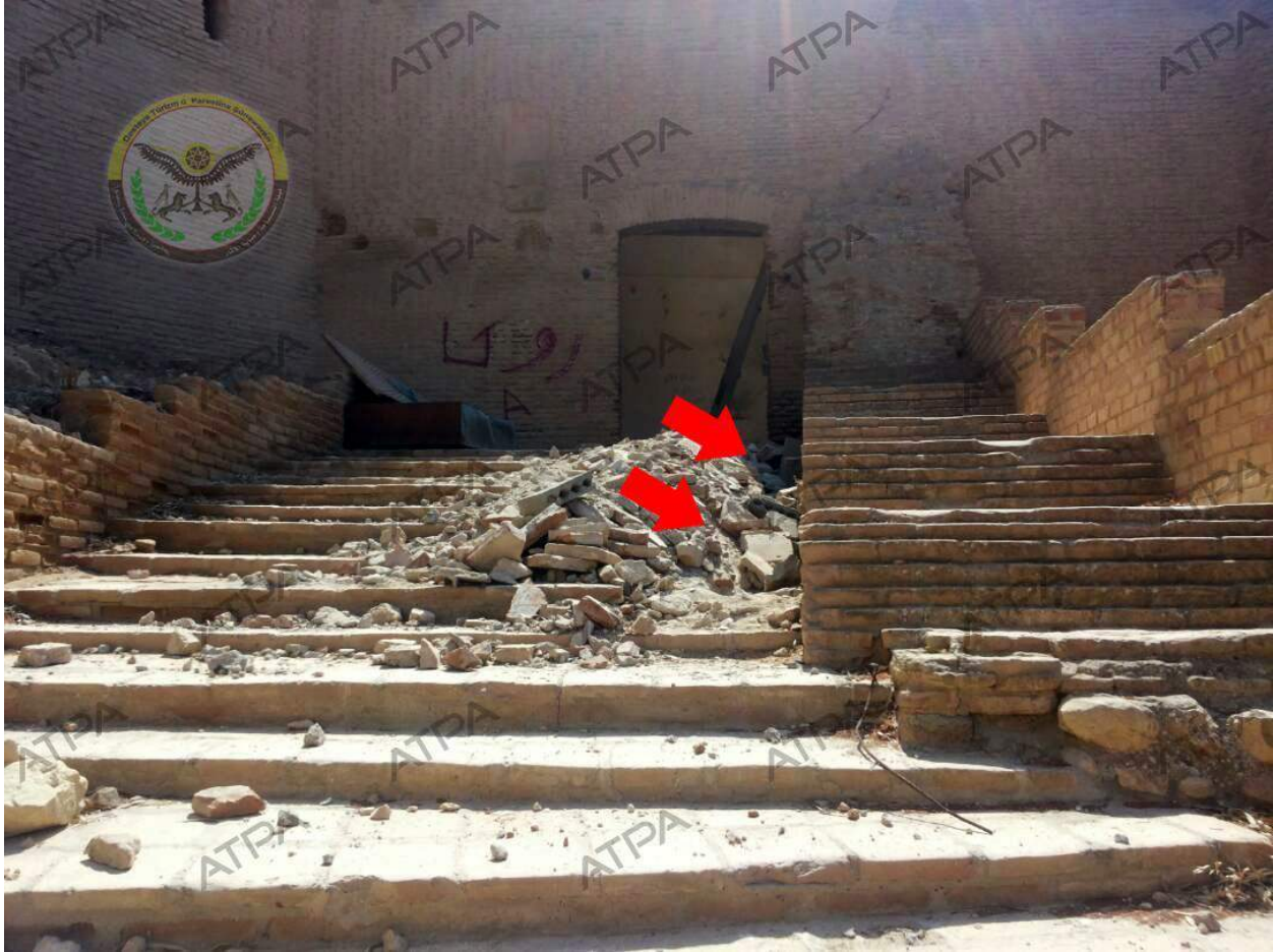
Damage to the main entrance of the castle and graffiti (ATPA; September 21, 2017)
