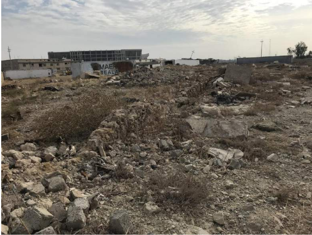
The Mosul War Cemetery showing damage to buildings (Campbell MacDiarmid; December 22, 2017)
