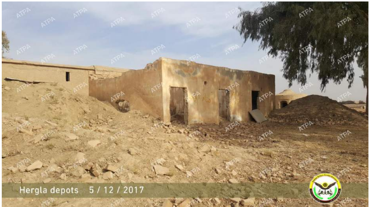
The storage facility, seen from the southwest (ATPA; December 11, 2017)
