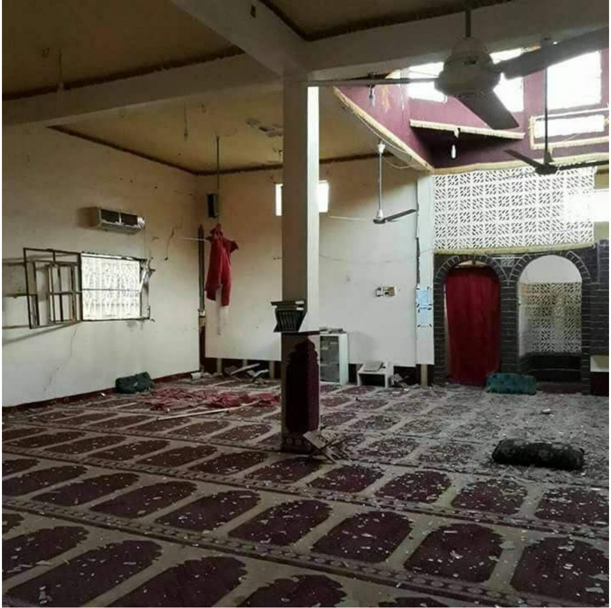
Damage to the interior of the mosque (Euphrates Post; November 4, 2017)
