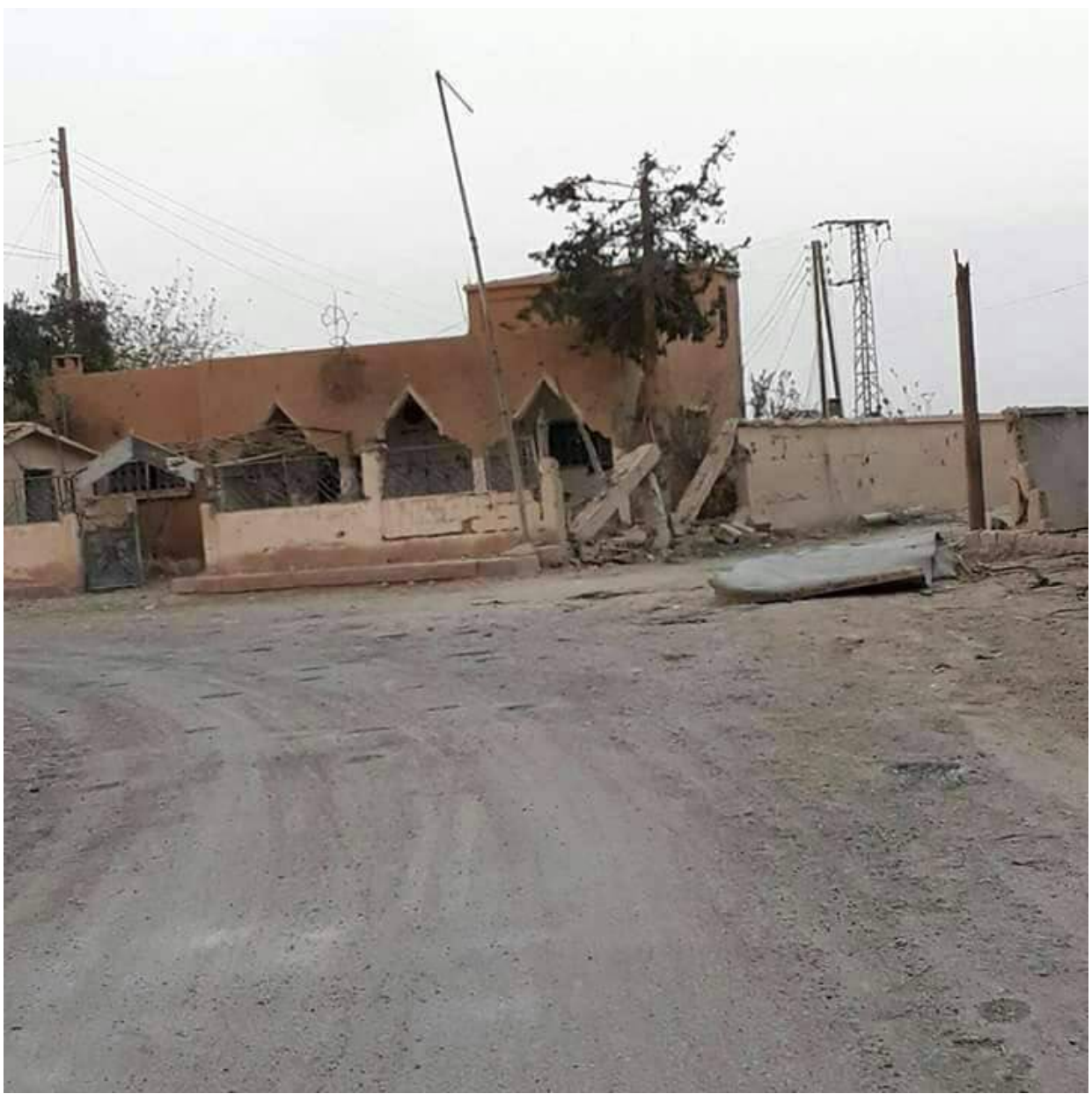
Damage to the exterior of the mosque (Euphrates Post; November 4, 2017)
