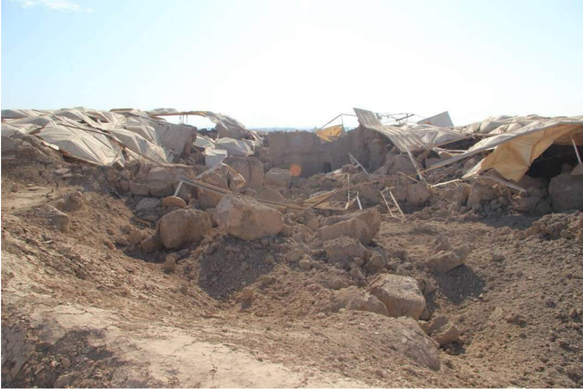
A photograph showing the collapsed modern structure covering a section of the Palace of Zimri-Lim (DGAM; March 27, 2018)
