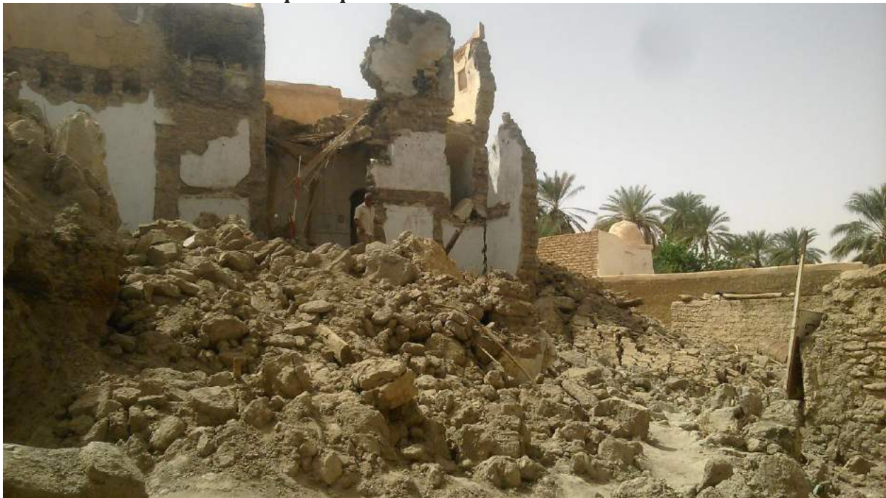
A view of a collapsed house near al-Atiq Mosque (Hassan Hamoudeh; April 4, 2018)
