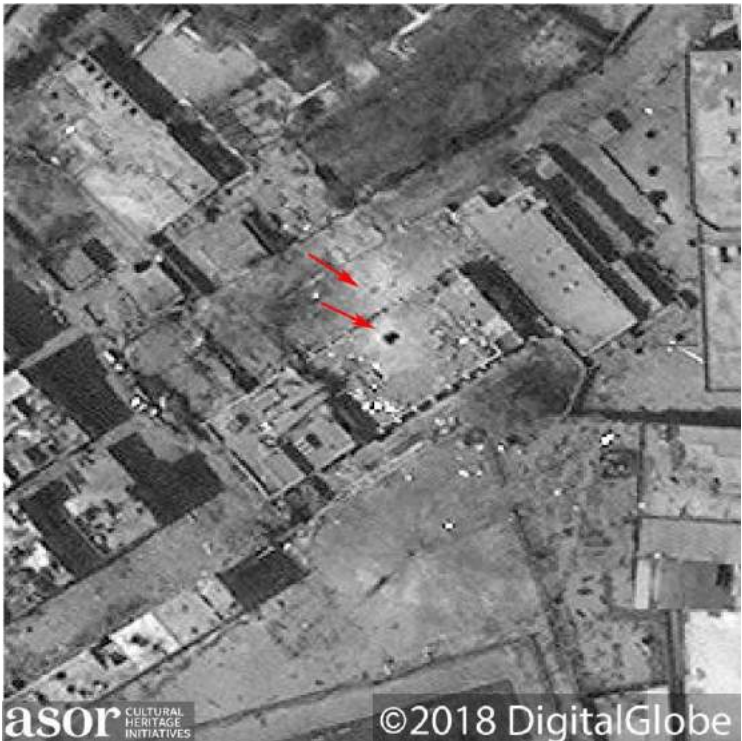
A large hole in the roof of the Palestinian Arab Cultural Center is indicated by an arrow. Evidence of shelling is visible immediately north of the center, also indicated by an arrow (Imagery courtesy of DigitalGlobe; April 27, 2018)
