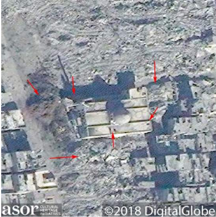
Visible in this image is severe damage surrounding Ali Bin Abi Talib Mosque, as well as the collapse of the minaret on the northwest part of the mosque and at least three holes in its roof (Imagery courtesy of DigitalGlobe; December 23, 2014)
