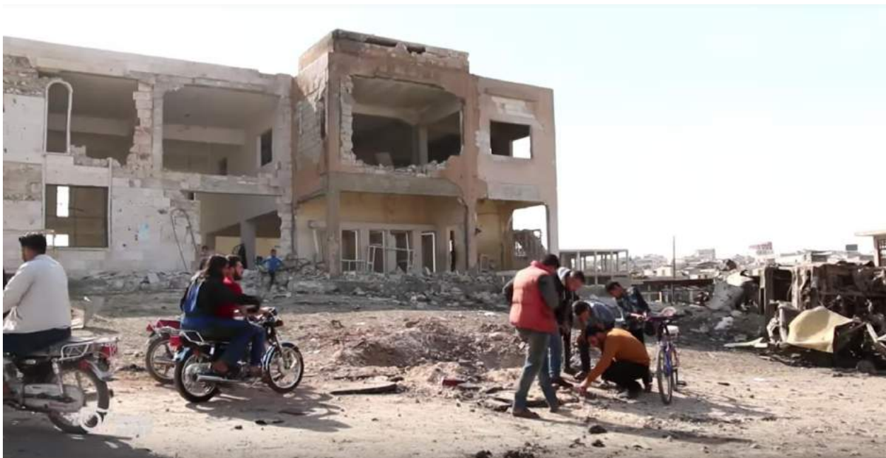
Video still showing damage to the exterior of Suhaib al-Rumi Mosque (Orient News; April 19, 2018)
