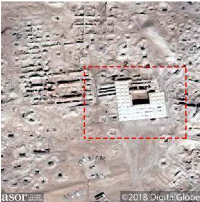
The modern covering over the Palace of Zimri-Limon prior to any explosive damage (Imagery courtesy of DigitalGlobe; October 19, 2017)
