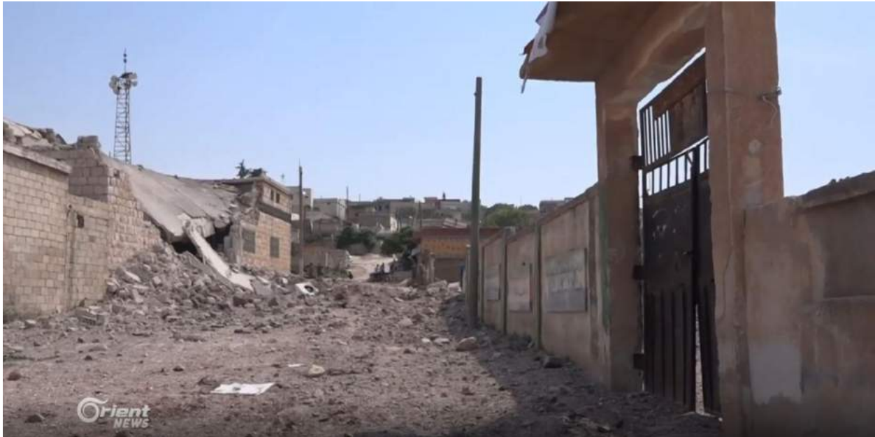
Damage to the area surrounding al-Kabir Mosque (Orient News; April 30, 2018)
