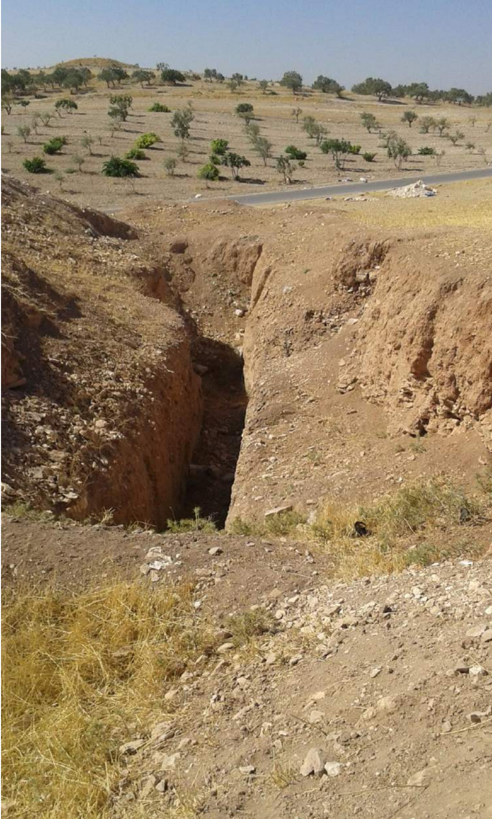
The northern side and a hole caused by illegal excavation
