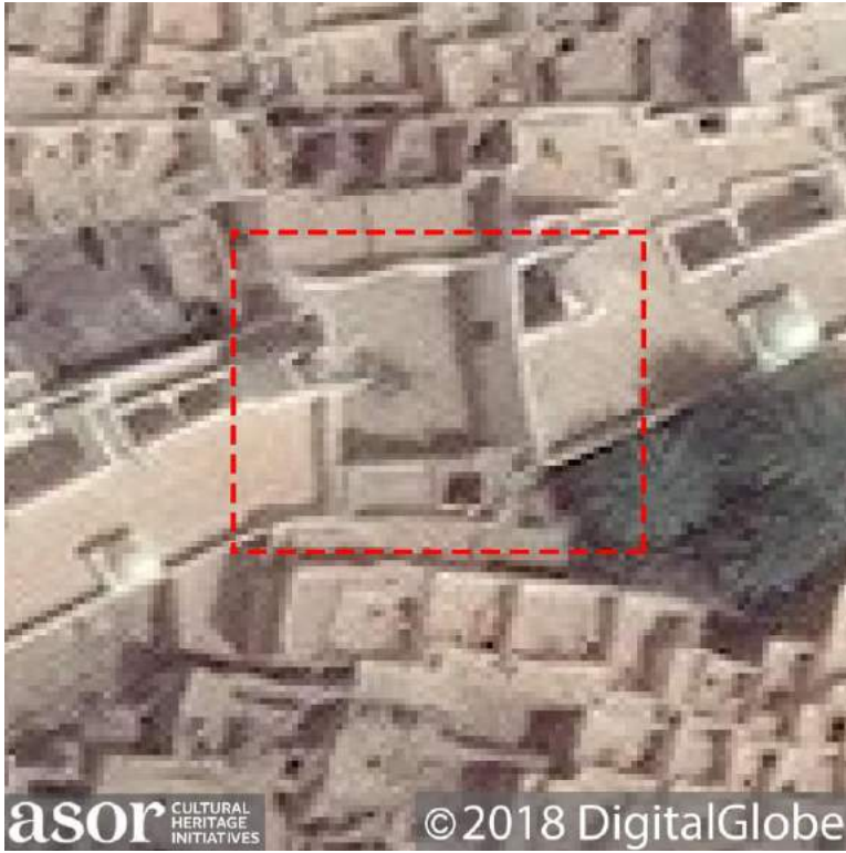
Location 4 after damage (Imagery courtesy of DigitalGlobe; April 5, 2018)
