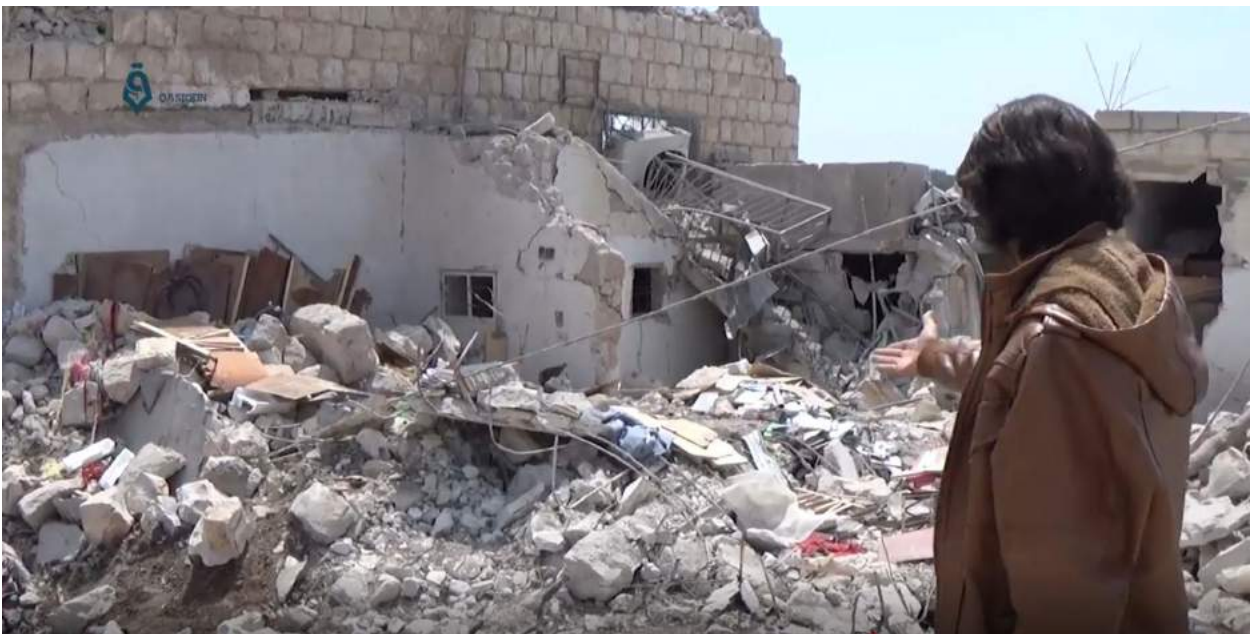
Damage to the area surrounding al-Kabir Mosque (Qasioun News Agency; April 30, 2018)
