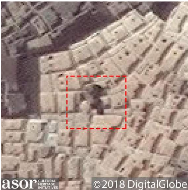
Location 1 after damage and collapse (Imagery courtesy of DigitalGlobe; April 5, 2018)
