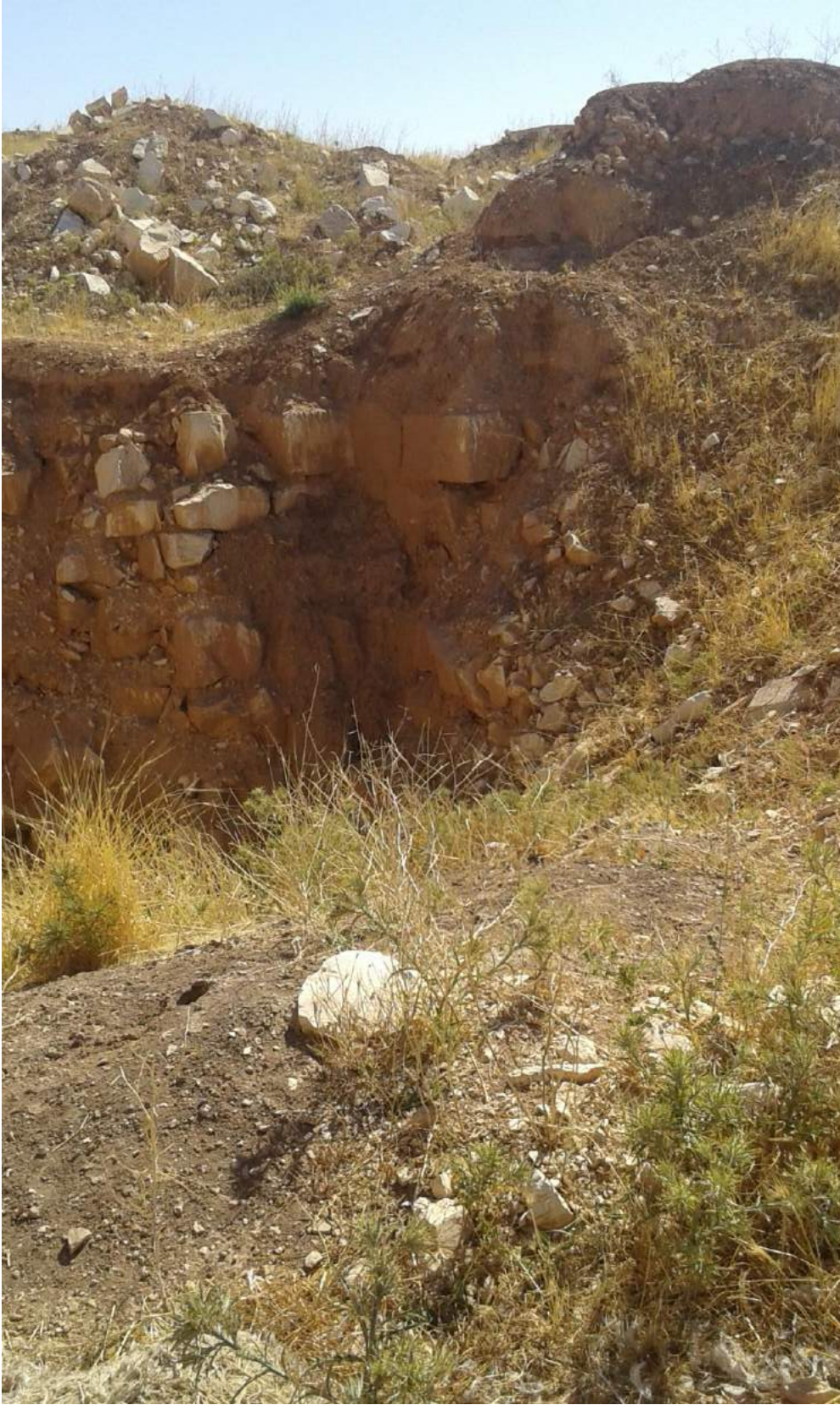
An illegal excavation on the eastern side
