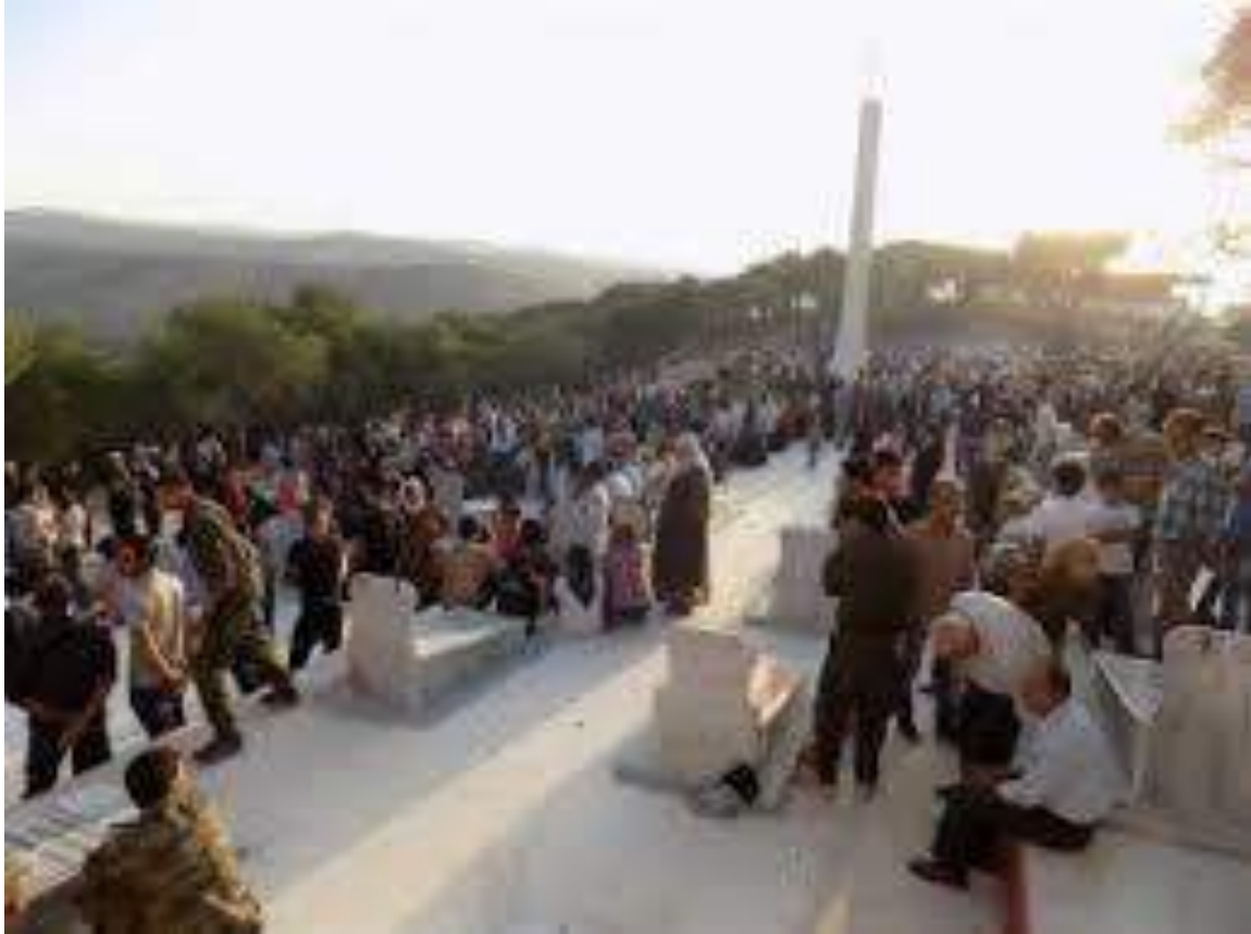
A pre-damage photograph of Martyr Seydo Cemetery (ANF Arabic; September 24, 2015)
