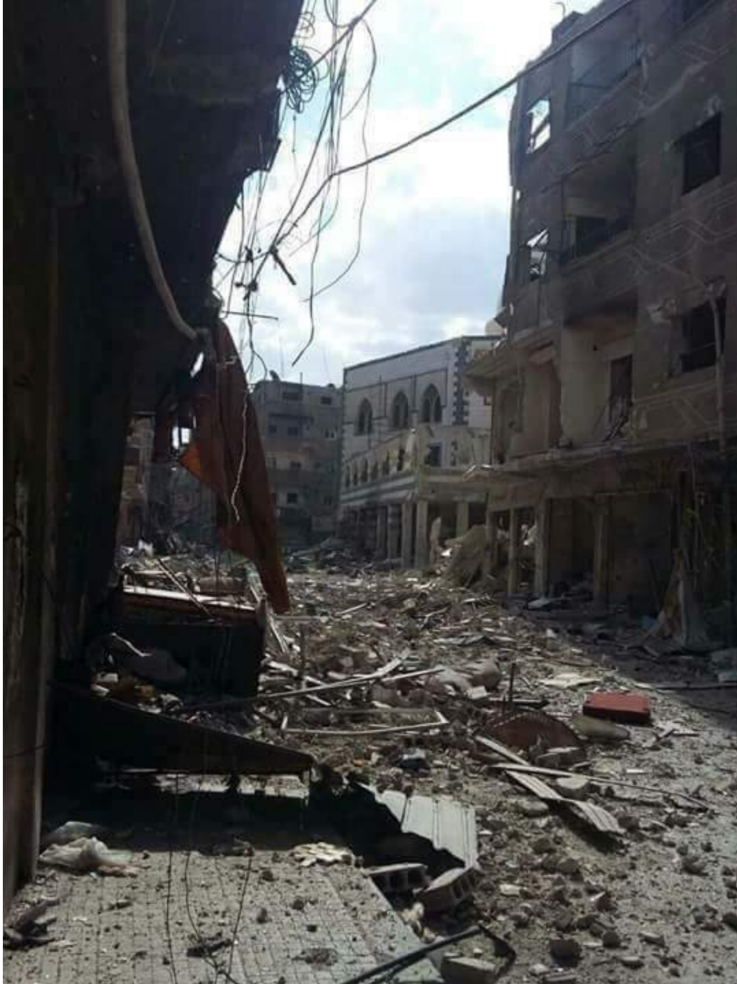
Severe damage to the exterior of the Palestinian Mosque and surrounding area (Private Twitter Account; April 21, 2018)
