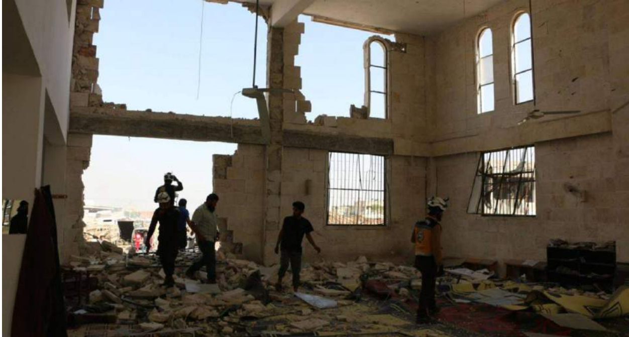
A photograph showing severe damage to the interior of Suhaib al-Rumi Mosque after an explosion (SNHR; April 19, 2018)
