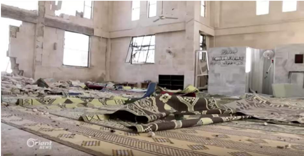
Video still showing damage to the interior of Suhaib al-Rumi Mosque (Orient News; April 19, 2018)
