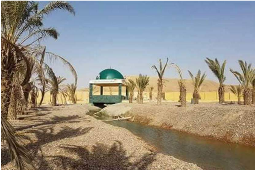
The completed shrine, seen from the east (Baghdad Post; April 24, 2018)
