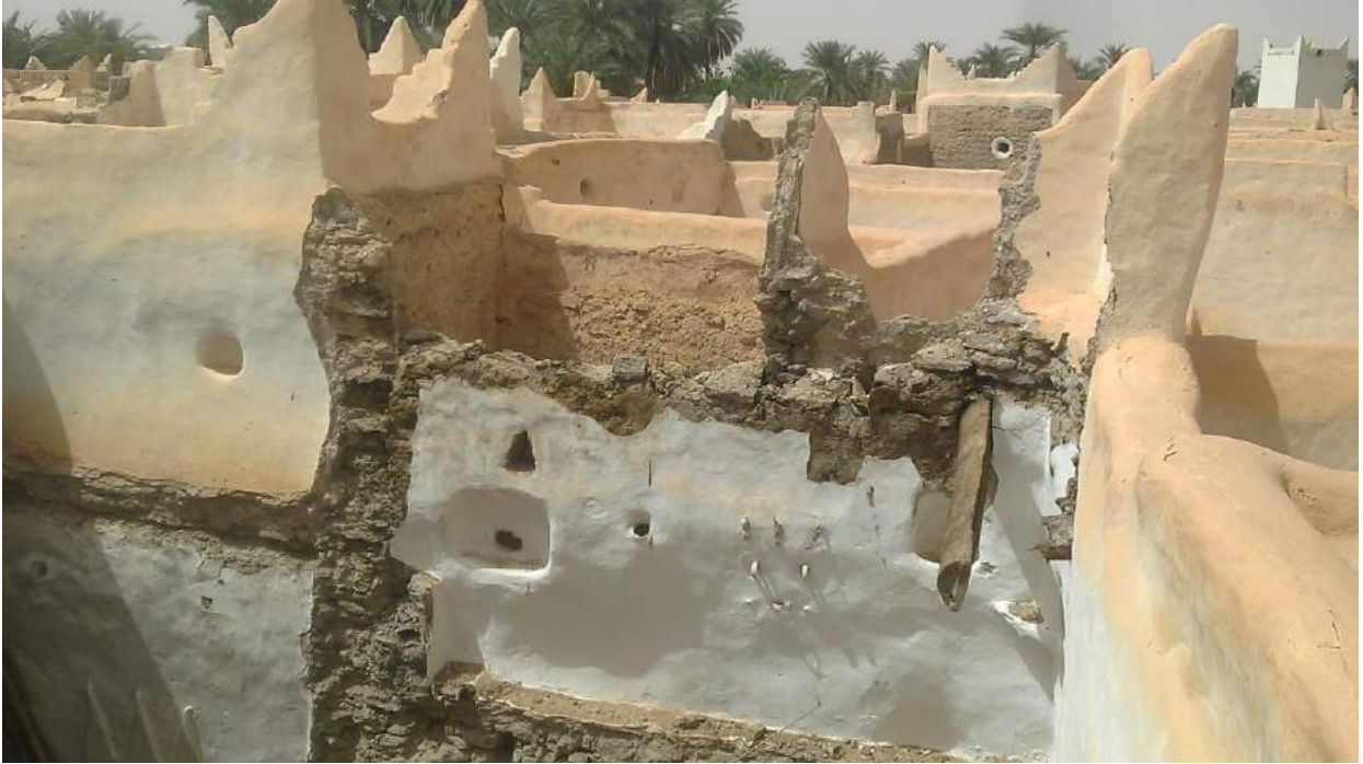
A view of the scar of the collapsed partition wall that once separated two houses (Hassan Hamoudeh; April 4, 2018)
