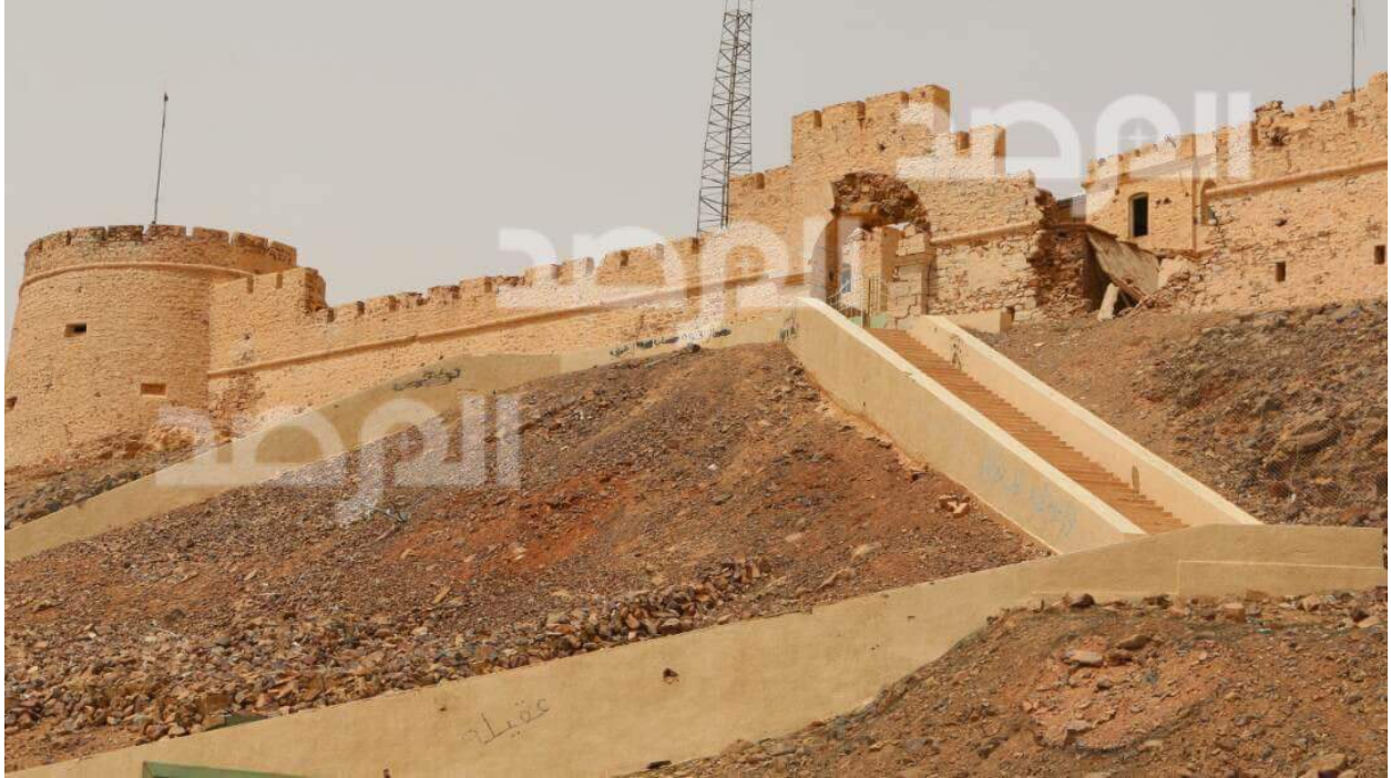
Collapse of a section of southern wall and entrance of Sabha Castle (Al Marsad; April 1, 2018)
