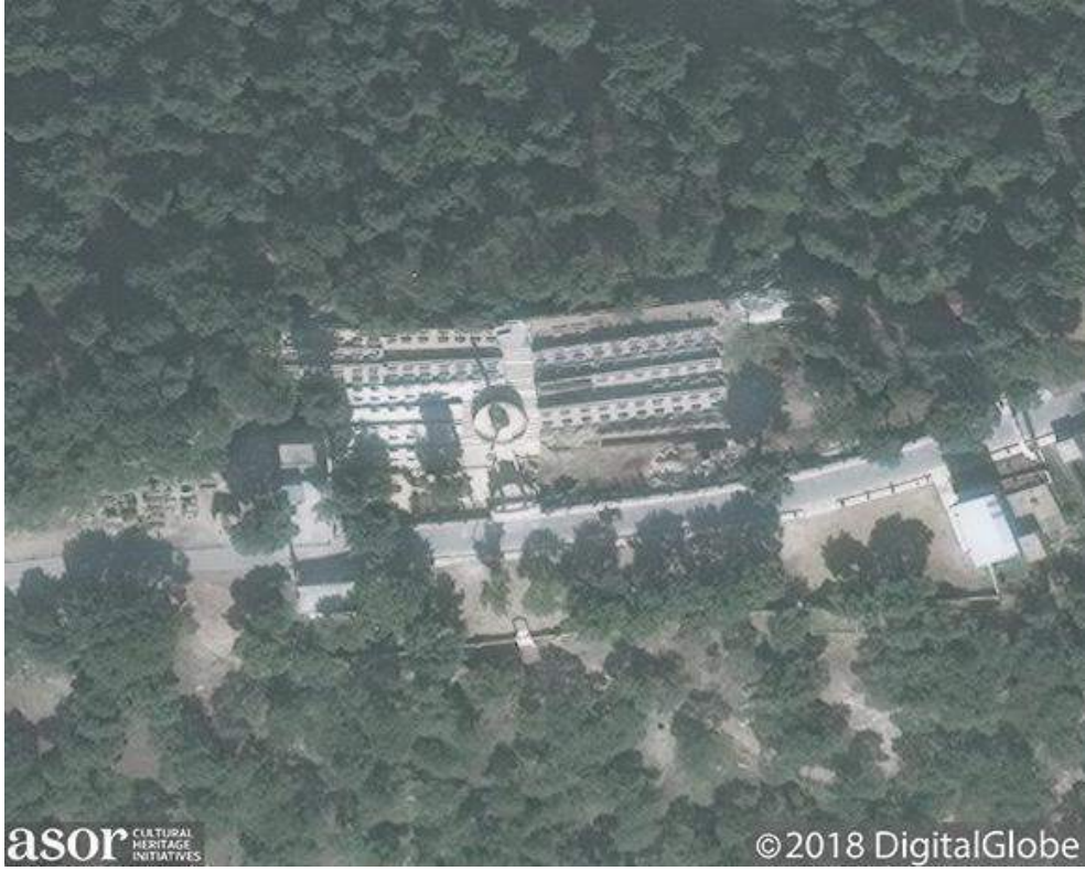
Martyr Seydo Cemetery before damage (Imagery courtesy of DigitalGlobe; January 29, 2018)
