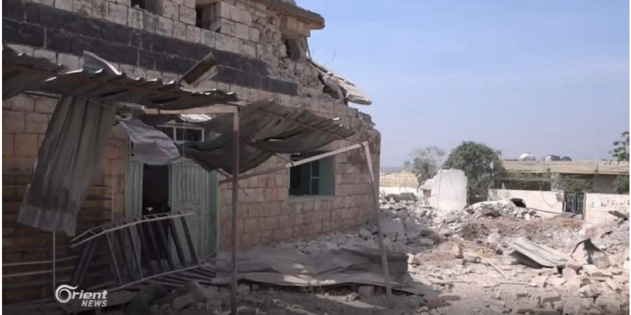
Damage to al-Kabir Mosque (Orient News; April 30, 2018)
