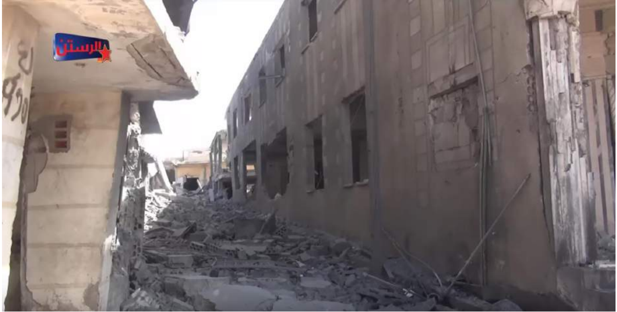
Damage to the eastern exterior side of al-Omari Mosque (Suhaib al-Ali - Homs; April 30, 2018)
