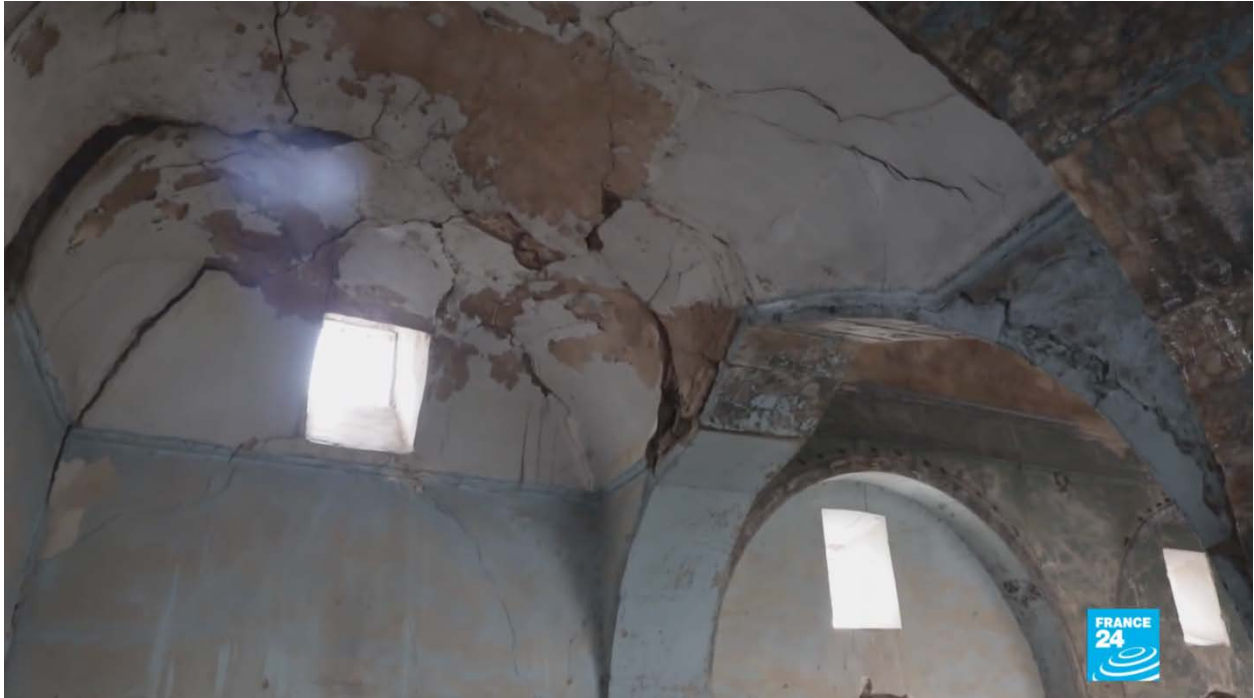
Fig. 44. Video still of the heavily damaged roof of the synagogue (France 24; April 24, 2019).
