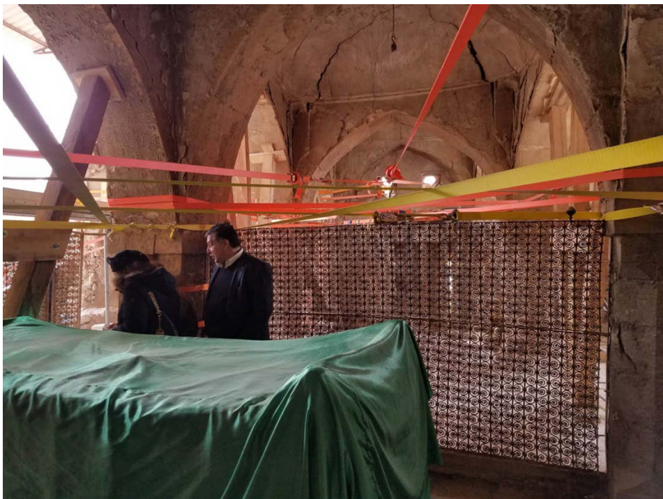
Fig. 53. Stabilization activities performed in the shrine by ARCH in December 2017–January 2018; the tomb of the prophet is visible in the foreground (ARCH).
