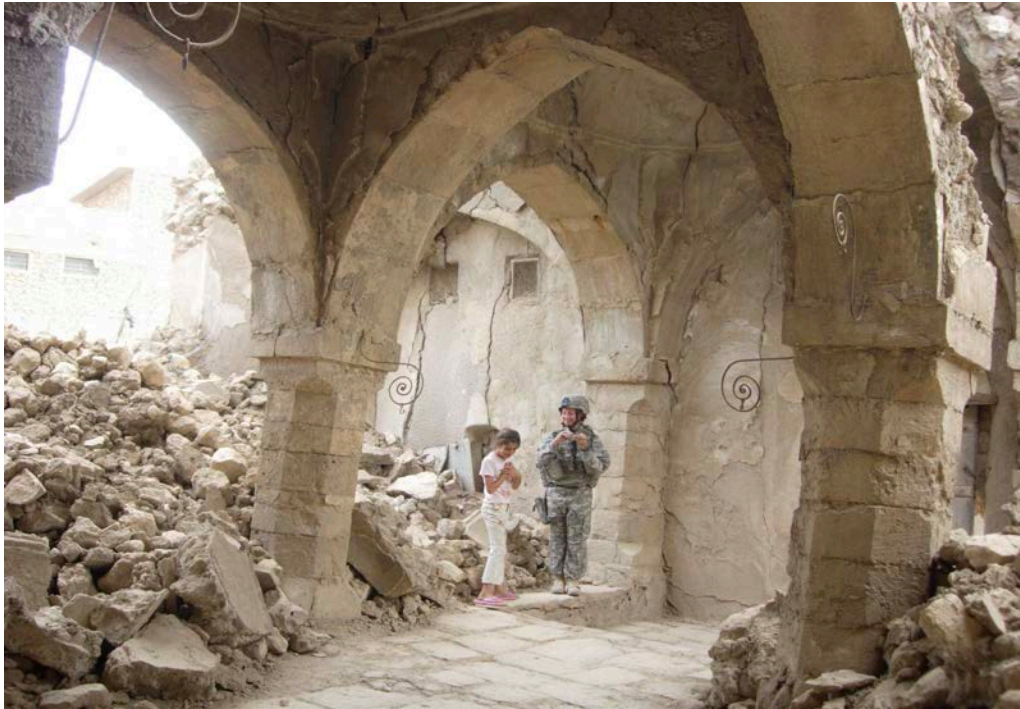
Fig. 51. The central aisle and collapsed southeastern corner of the synagogue, seen from the northwest (Suzanne E. Bott; September 2008).
