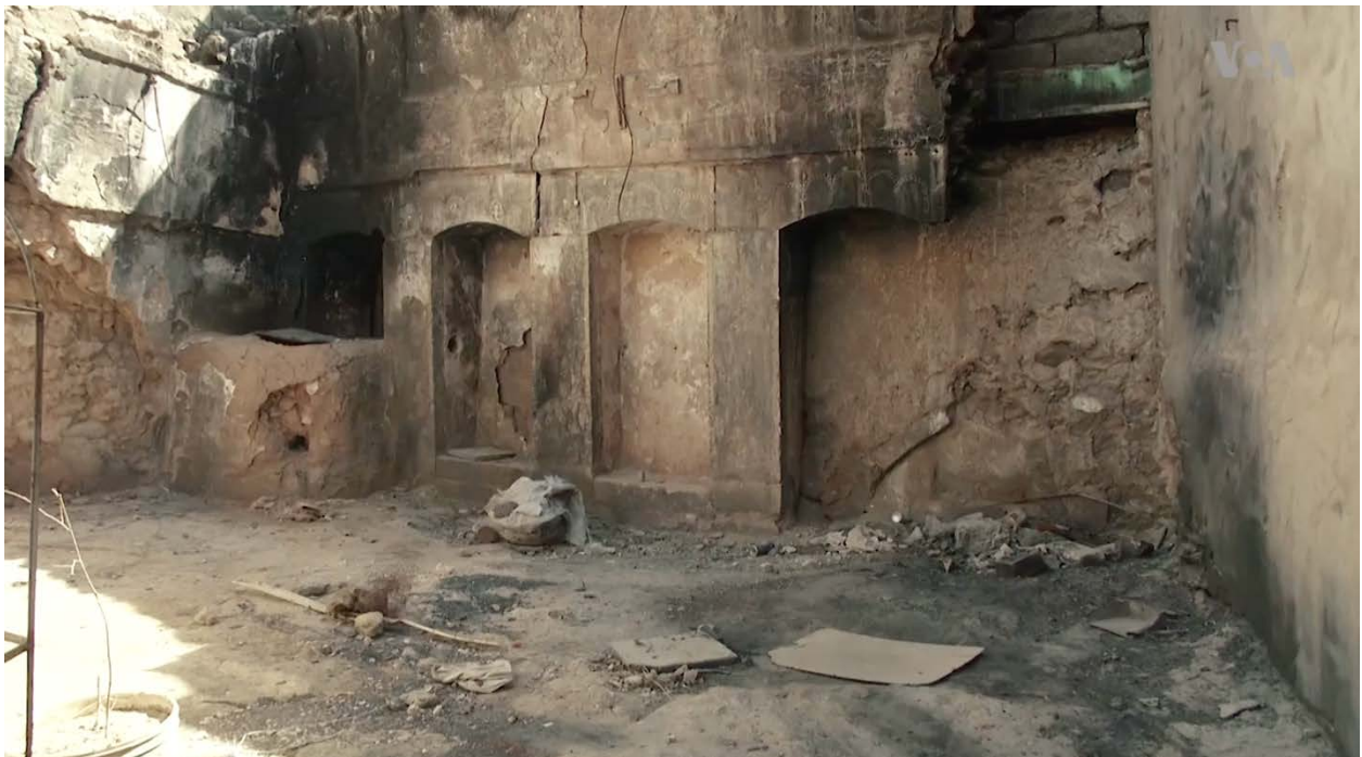
Fig. 46. A video still of fire damage inside the property (Voice of America; July 6, 2018).
