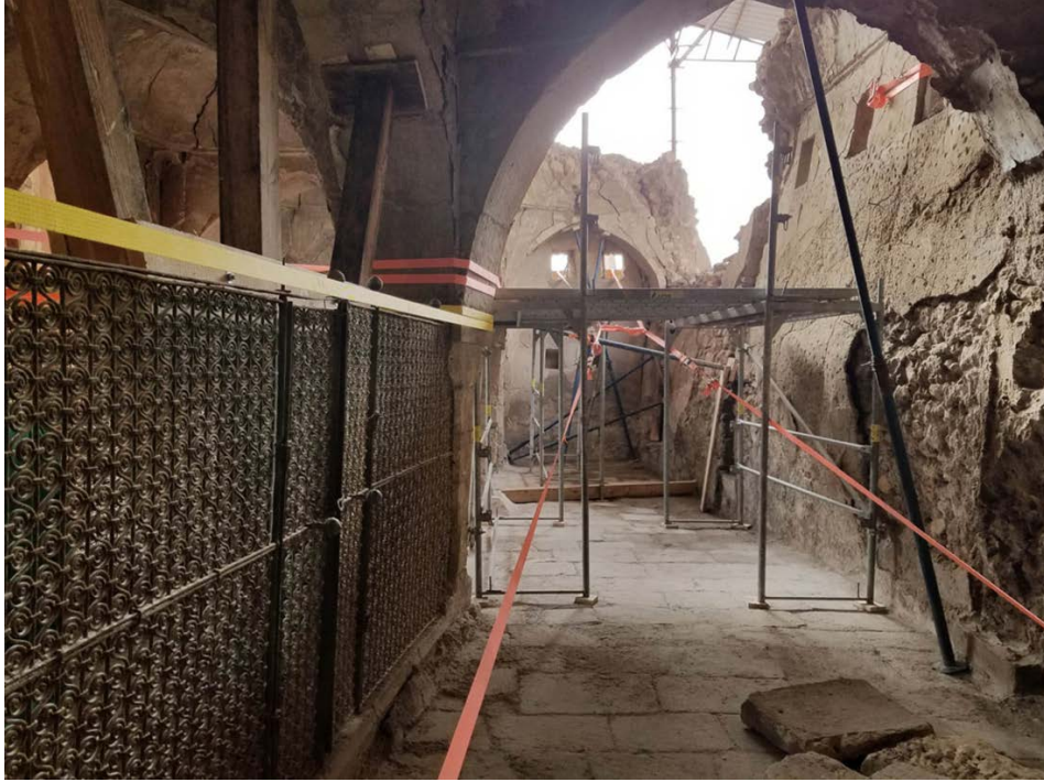
Fig. 52. Stabilization activities performed in the shrine by ARCH in December 2017–January 2018 (ARCH).
