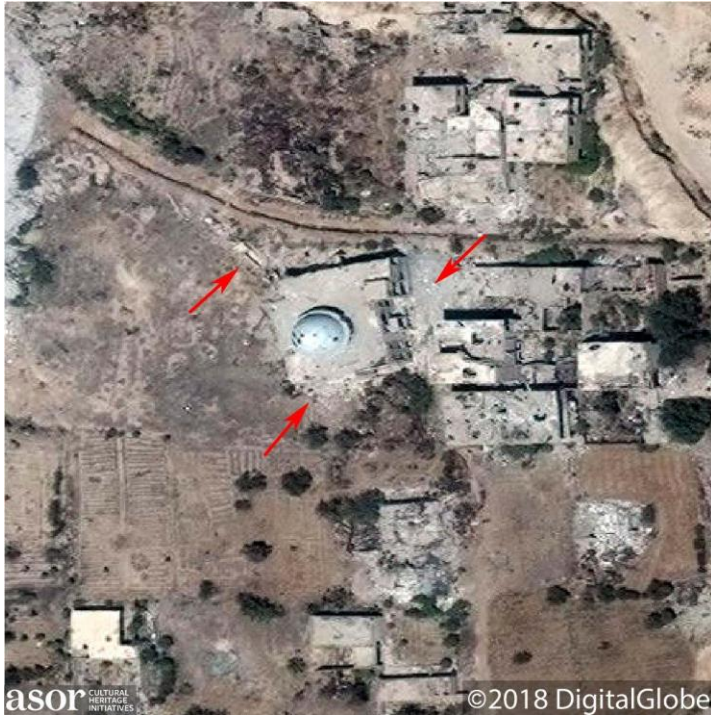
Al-Rahma mosque with prior visible damage from heavy shelling visible on all sides of the mosque, as well as to the dome (Imagery courtesy of DigitalGlobe; August 29, 2018)
