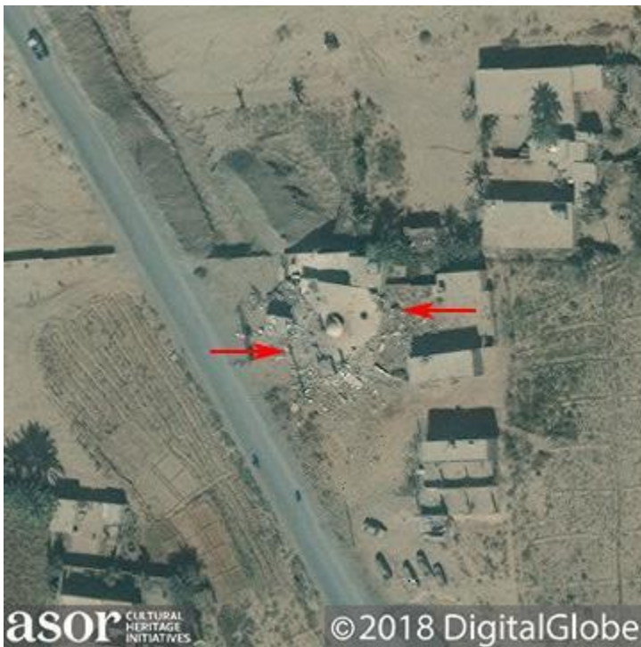
The western side of Ammar bin Yasser Mosque has collapsed (Imagery courtesy of DigitalGlobe; October 30, 2018)
