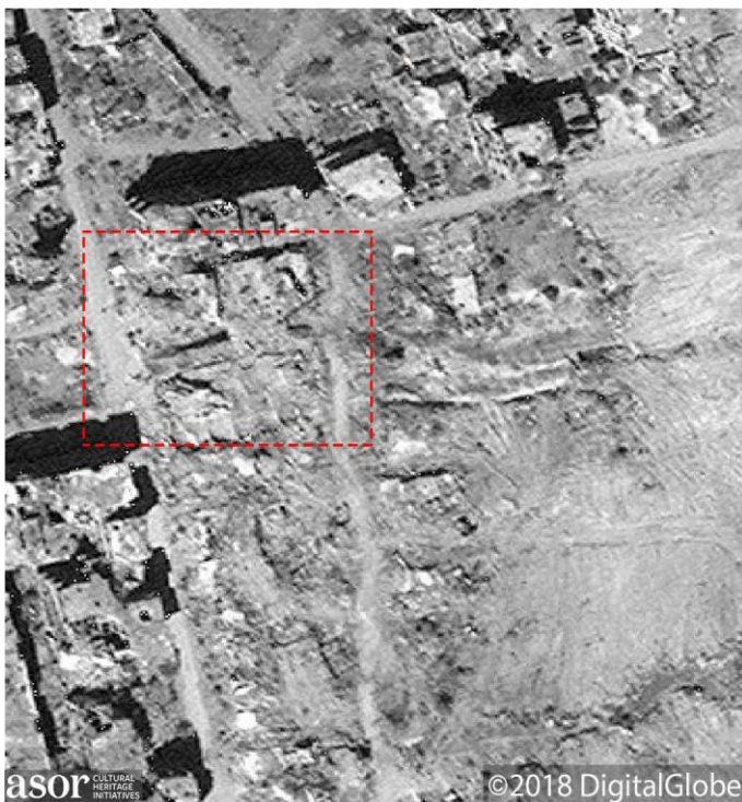
Al-Taqwa mosque is destroyed, although the means by which are unclear in satellite imagery (Imagery courtesy of DigitalGlobe; September 11, 2018)
