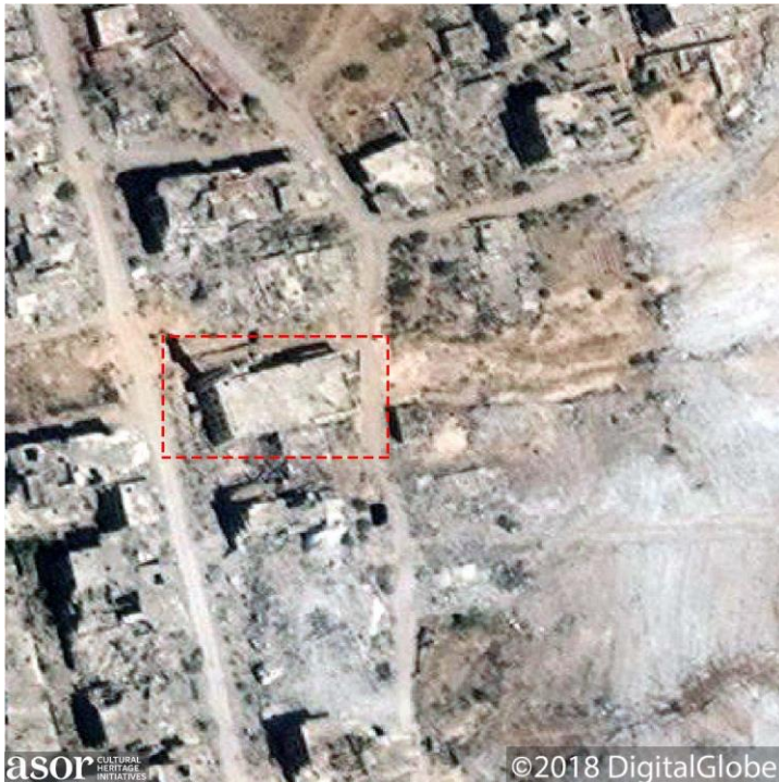
Al-Taqwa mosque prior to destruction; bulldozer scars are clearly visible east and southeast of the mosque (Imagery courtesy of DigitalGlobe; August 27, 2018)
