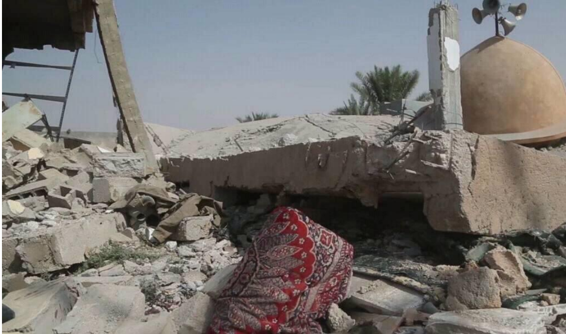
A view of the collapsed Ammar bin Yasser Mosque with the dome present in the background (SNHR; October 21, 2018)
