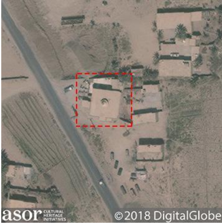
Ammar bin Yasser Mosque prior to damage (Imagery courtesy of DigitalGlobe; September 10, 2018)
