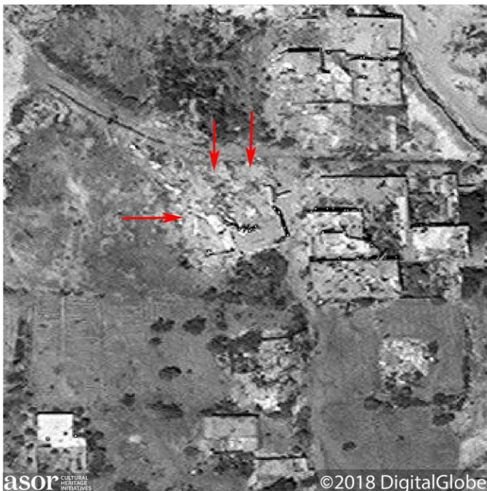
Al-Rahma mosque is almost entirely destroyed, likely the result of an airstrike based on the extensive damage to the main portion of the structure (Imagery courtesy of DigitalGlobe; August 8, 2018)
