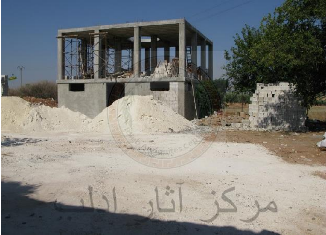
Non-military construction near Cyrrhus (Idlib Antiquities Center; July 13, 2018)
