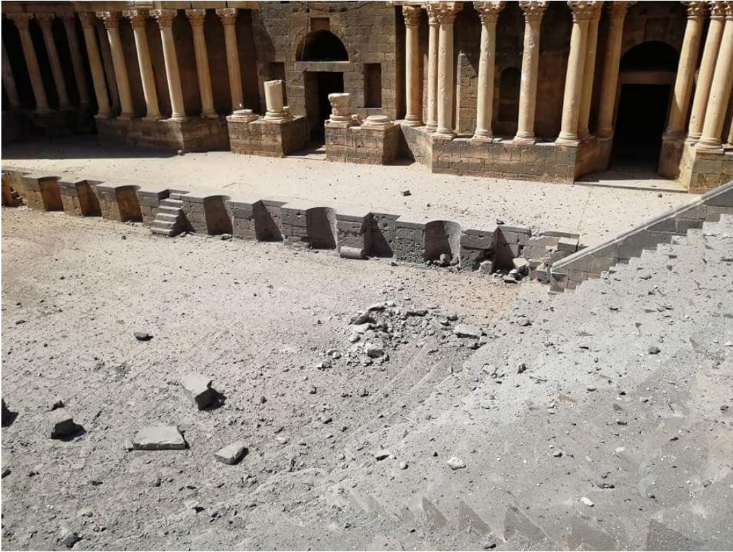
An airstrike crater in the eastern section of the orchestra pit (Bosra al-Sham Facebook; July 1, 2018)
