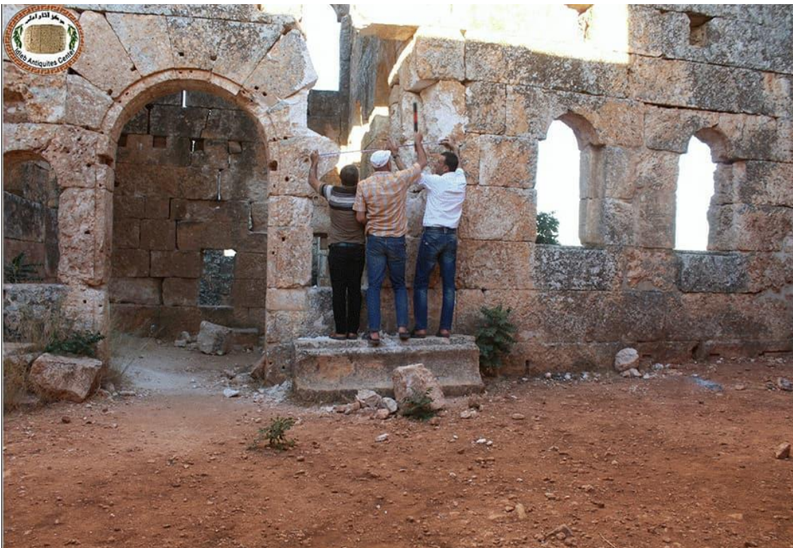
Preparing the facade for reconstruction work (Idlib Antiquities Center; July 14, 2018)
