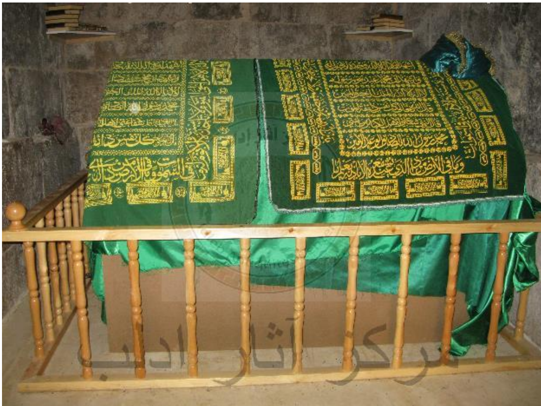
Condition of a shrine near Cyrrhus (Idlib Antiquities Center; July 13, 2018)
