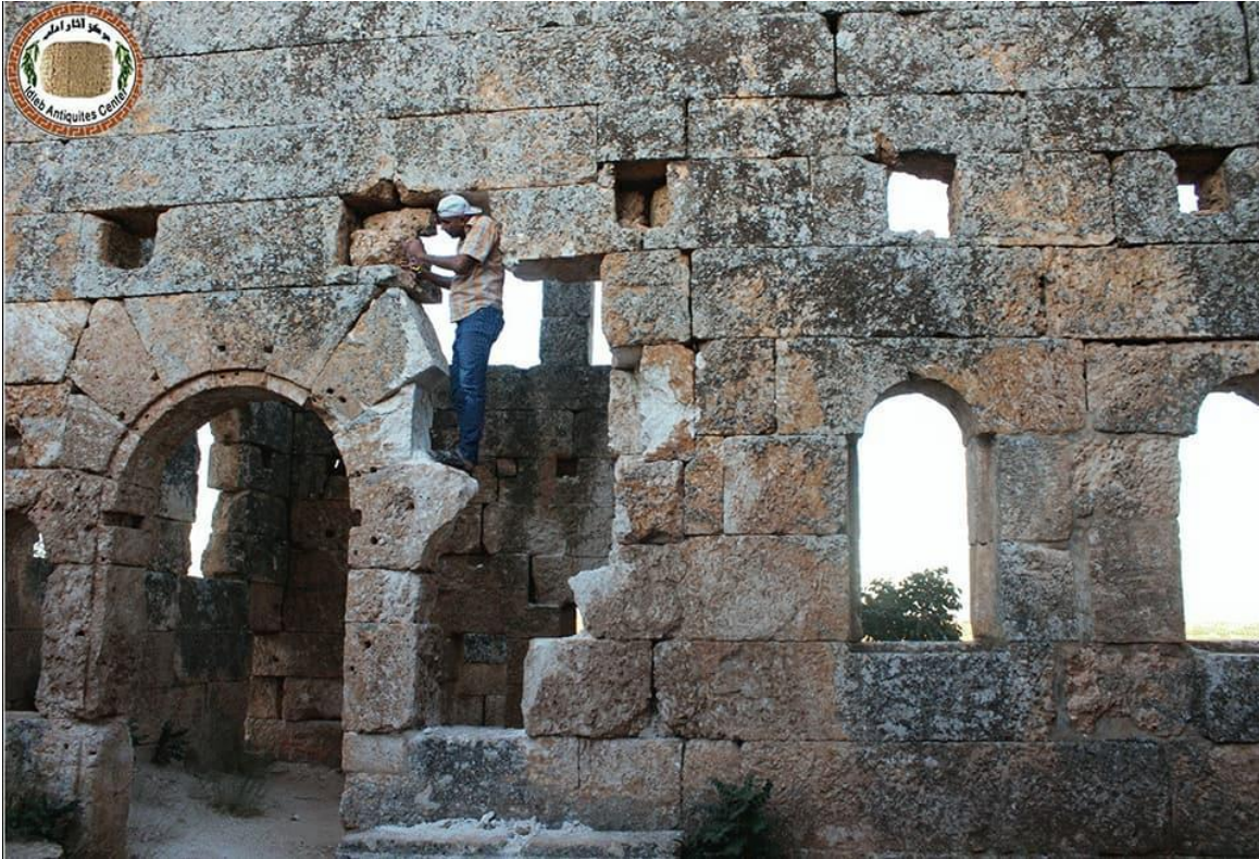
Preparing the facade for reconstruction work (Idlib Antiquities Center; July 14, 2018)
