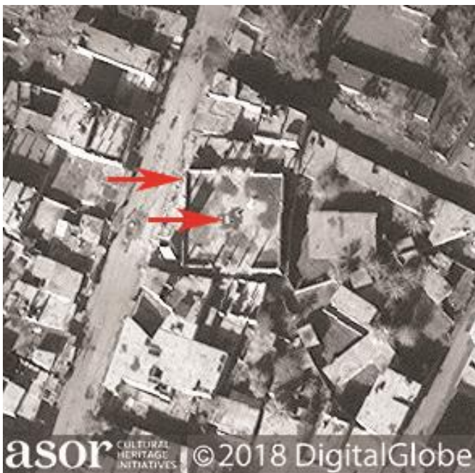
The mosque with damage on the northwestern corner and possible debris or hole in the roof, noted with red arrows (©DigitalGlobe 2018; December 11, 2018)
