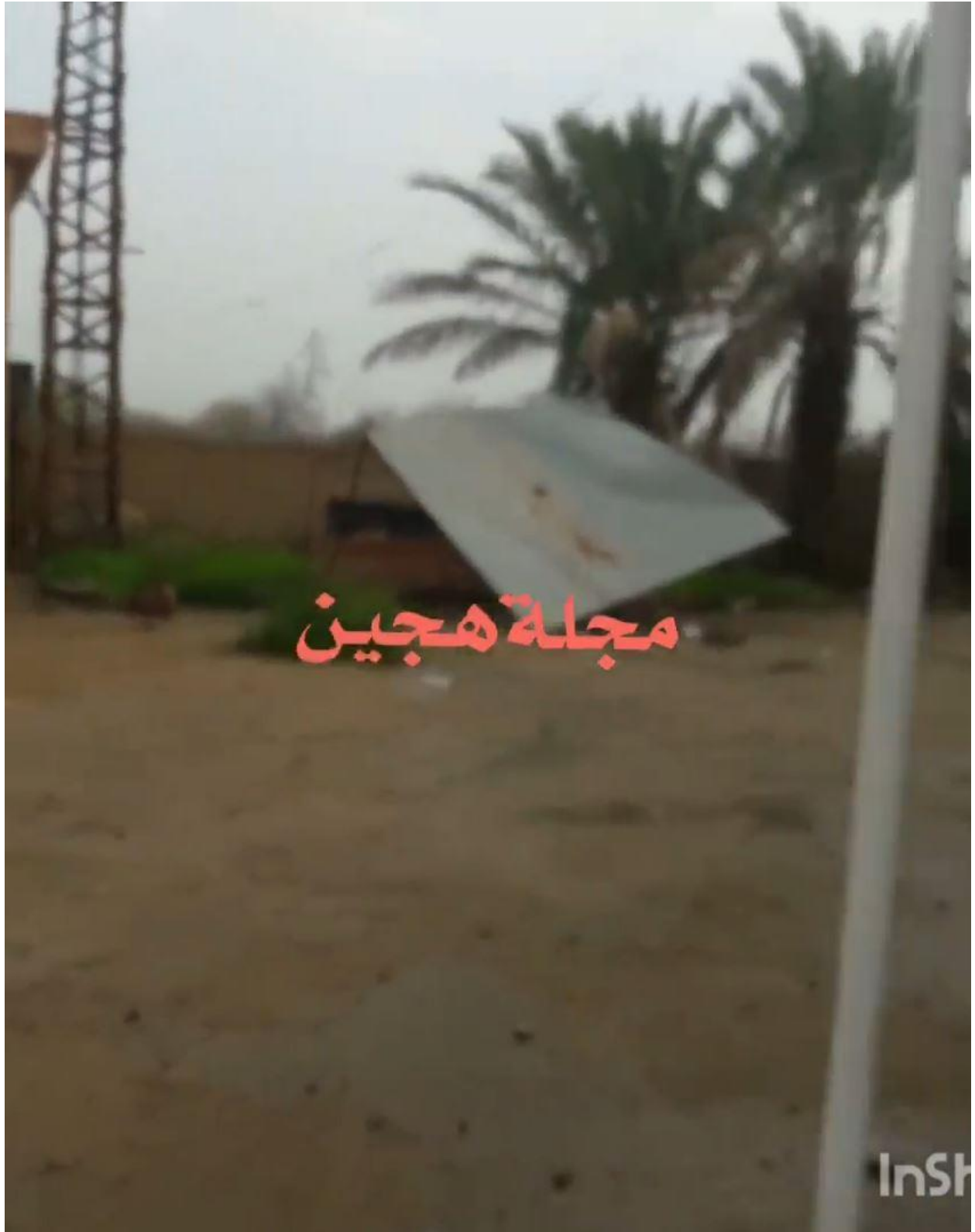
Video still of damage to secondary structures near the main entrance, seen from the southwest (Majlat Hajin; December 20, 2018)
