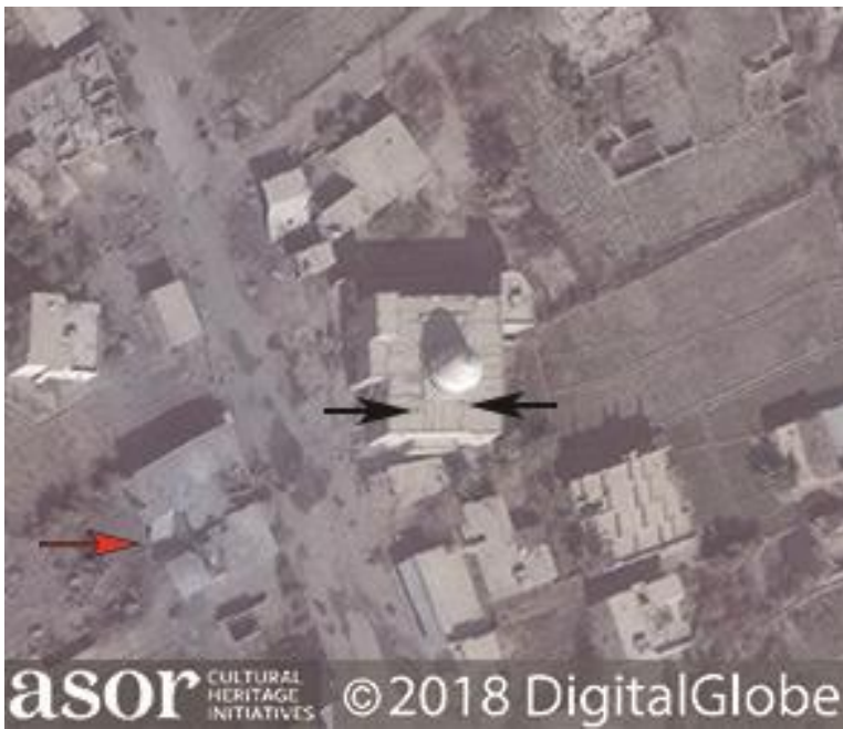
Possible damage to the roof of the mosque noted with black arrows (©DigitalGlobe 2018; November 13, 2018)
