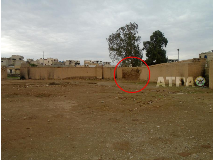
Wall deterioration at al-Qadim Mosque (ATPA; December 16, 2018)
