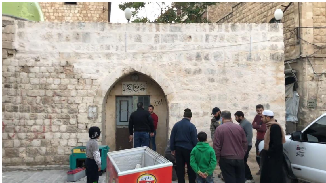
Video still of the mosque after repairs (Sohayb Masri; December 9, 2017)
