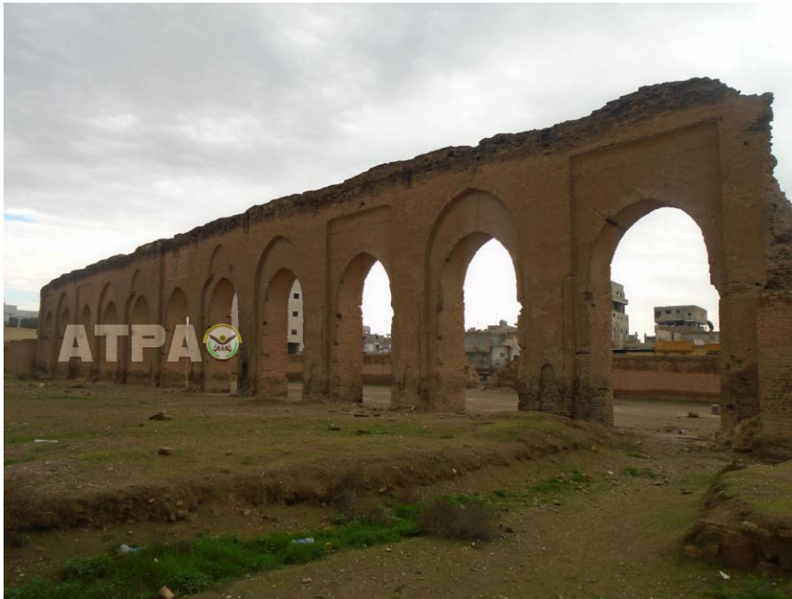
Deterioration of the colonnade at al-Qadim Mosque (ATPA; December 16, 2018)
