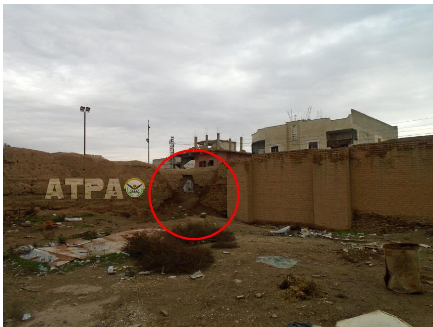
Wall collapse at al-Qadim Mosque (ATPA; December 16, 2018)
