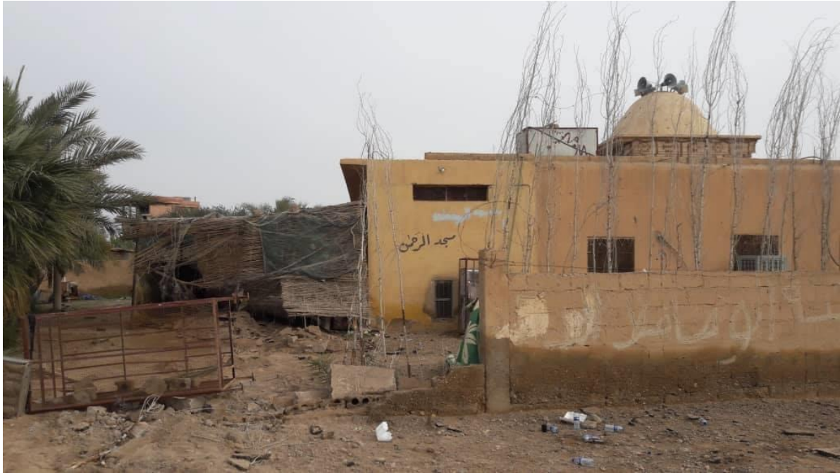
The western wall of al-Rahman Mosque (Majlat Hajin; December 16, 2018)
