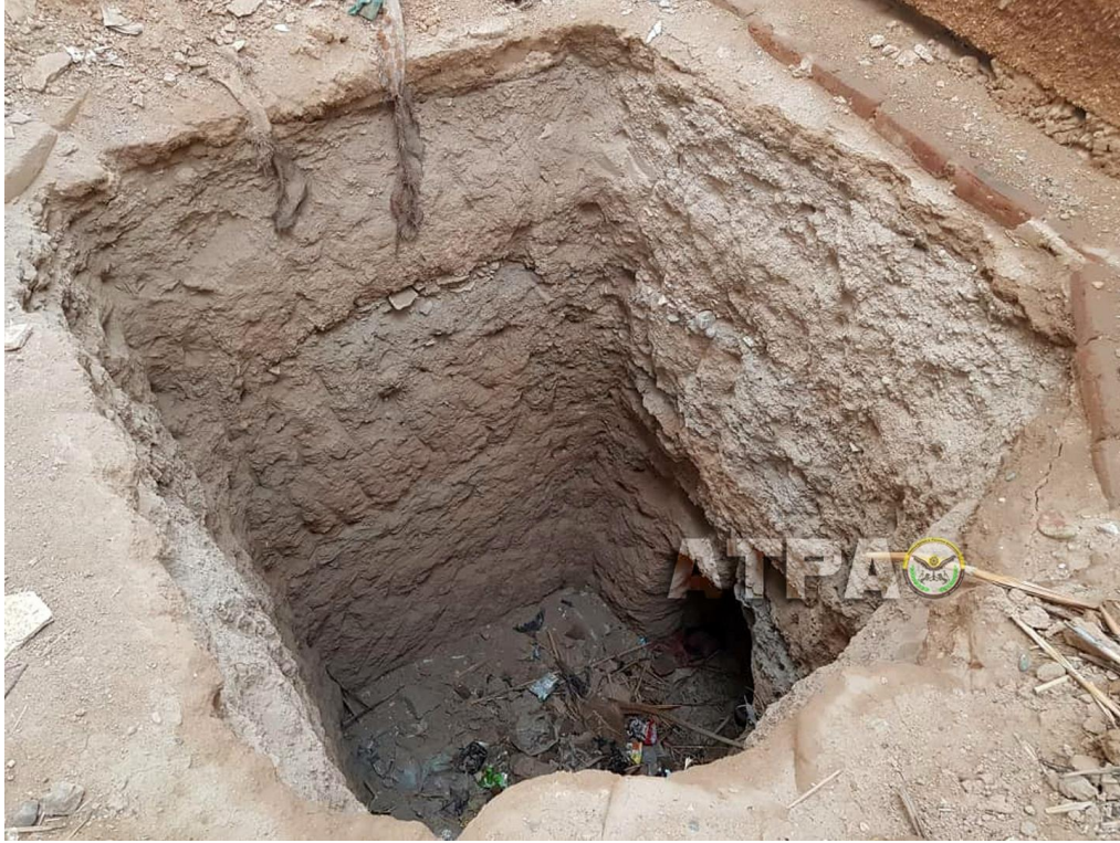
An illegal excavation in the former dig house (ATPA; December 14, 2018)
