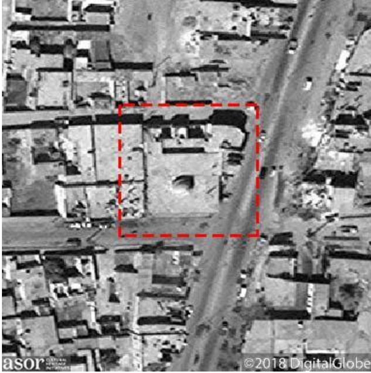
Al-Hamza bin al-Mutallib Mosque mosque prior to damage from an IED, shown within the red box (©2018 DigitalGlobe; March 25, 2018)
