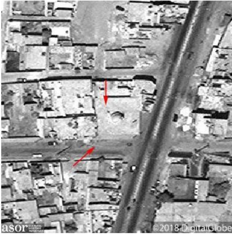
Red arrows indicate locations of possible damage to the mosque. There is a hole in the northwestern part of the roof, and visible rubble and debris on the street lining the southern facade (©2018 DigitalGlobe; August 21, 2018)
