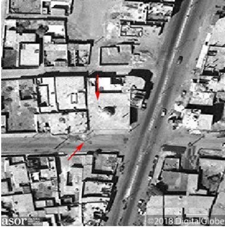
A later satellite image shows the damage to the mosque more clearly, as indicated by red arrows (©2018 DigitalGlobe; September 16, 2018)
