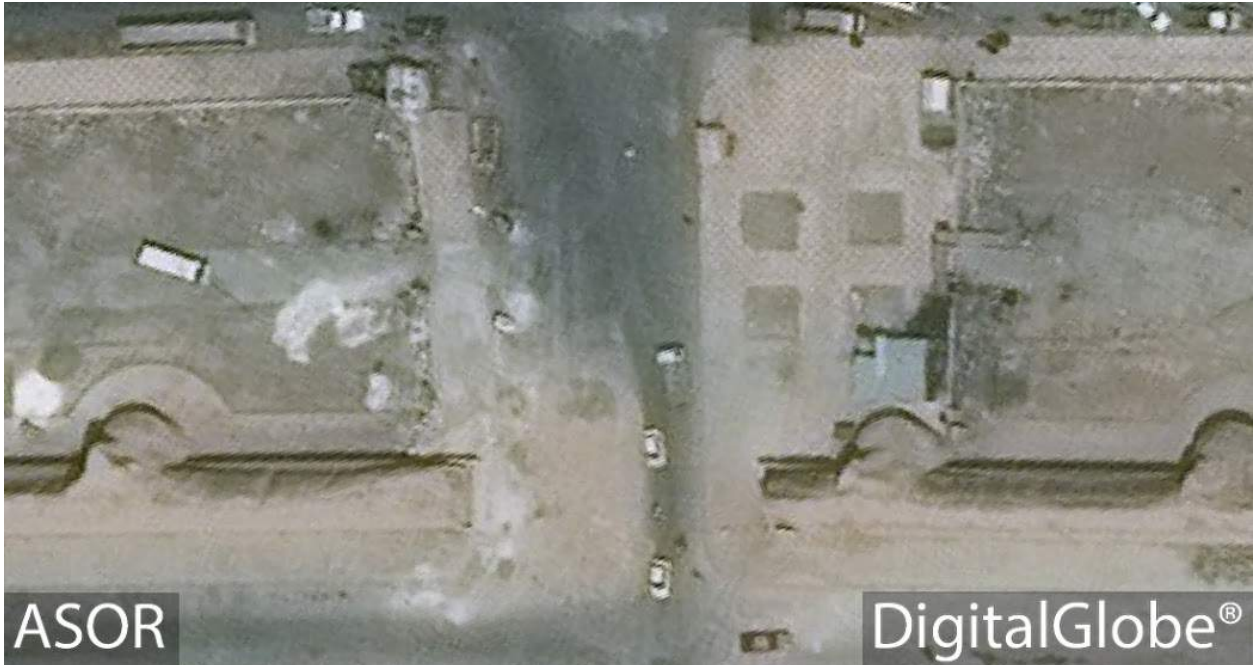
Bab Harran northern gate, Raqqa, with visible damage and debris cleared (DigitalGlobe; September 5, 2015)
