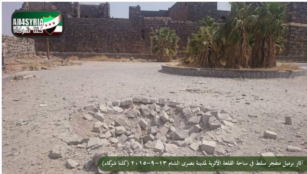
Busra al-Sham Citadel Courtyard showing bomb damage. (All4Syria; September 16, 2015)
