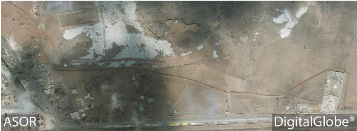
Construction of embankments on the northern edge of the city (DigitalGlobe; September 5, 2015)
