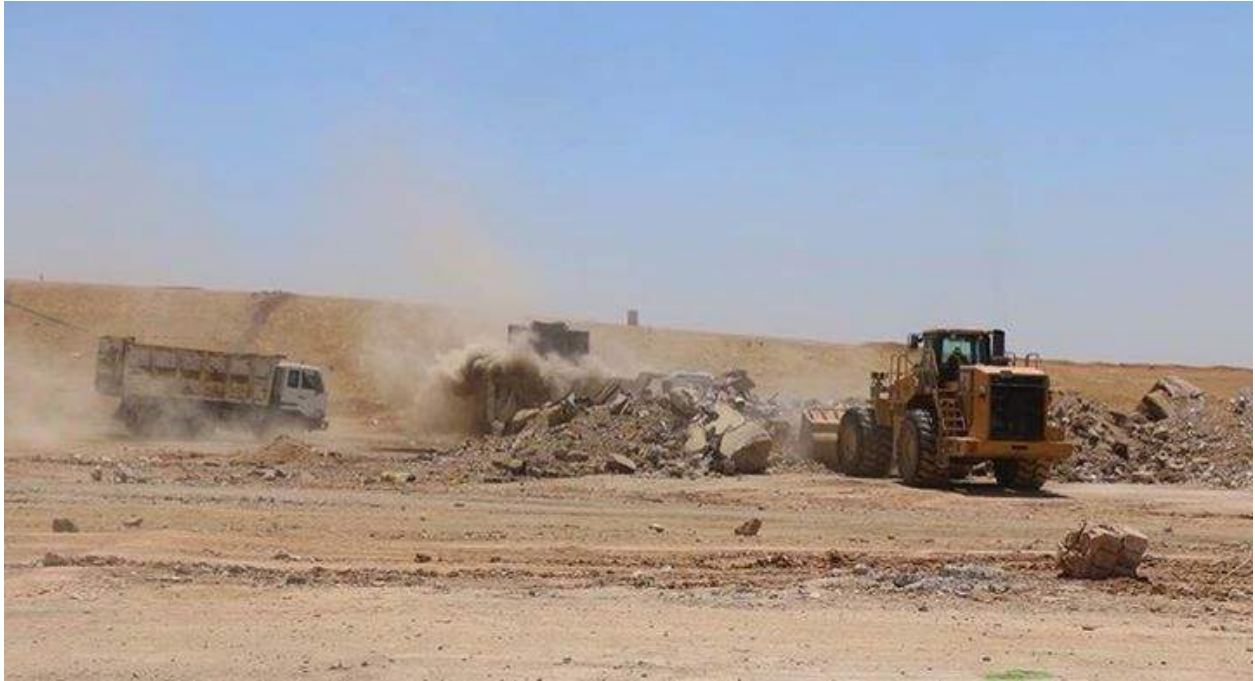
Demolition of the stadium (Facebook; June 23, 2015)
