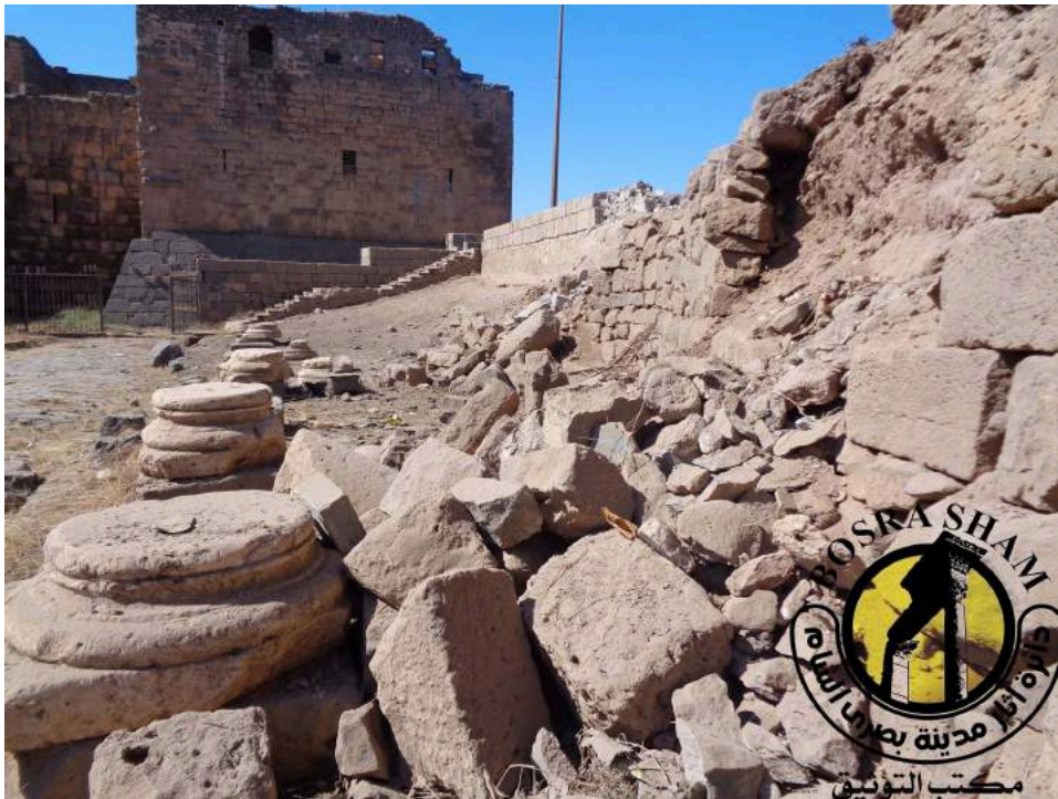
Busra al-Sham Citadel Courtyard showing bomb damage. (Facebook page; September 16, 2015)
