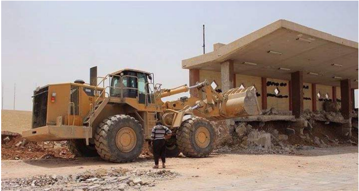
Demolition of the stadium, located outside the Northern Wall (Facebook; June 23, 2015)
