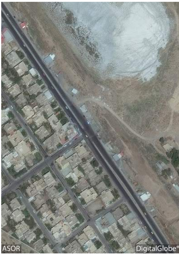
Western Area, new construction along edge of Nineveh (DigitalGlobe; August 29, 2015)
