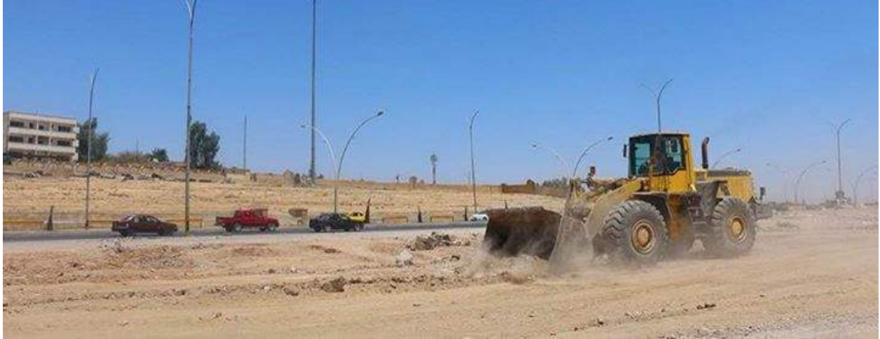
Demolition of the stadium (Facebook; June 23, 2015)
