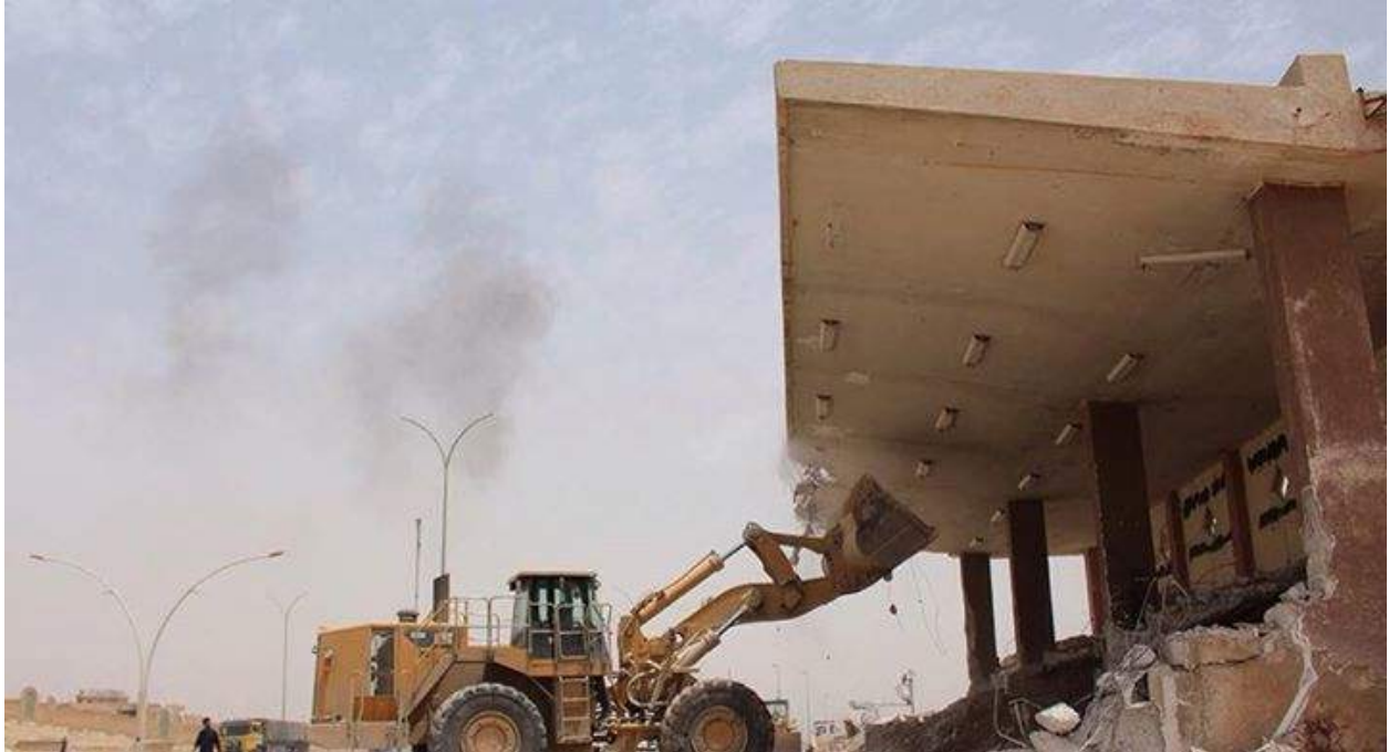
Demolition of the stadium, located outside the Northern Wall (Facebook; June 23, 2015)
