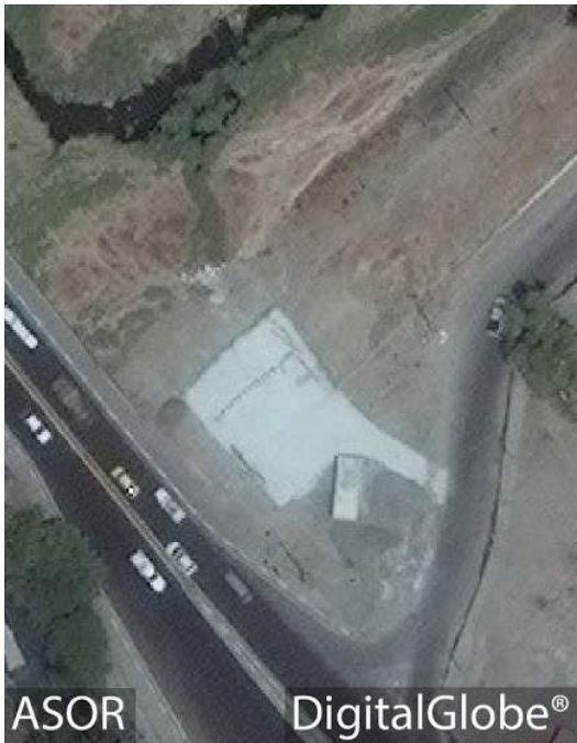
South Area, construction of large building in the south western corner (DigitalGlobe; August 29, 2015)
